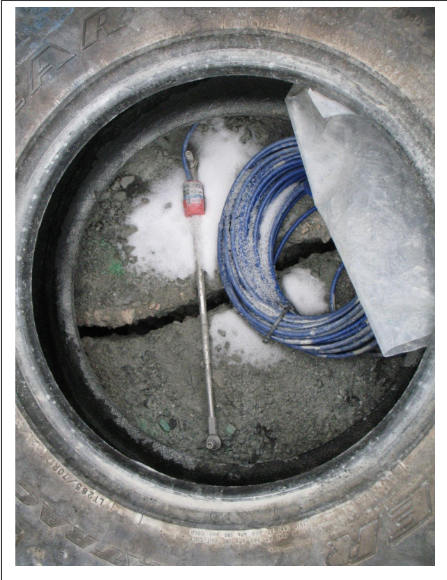
Photo No. 3 Crackmeter on Stormwater dike
