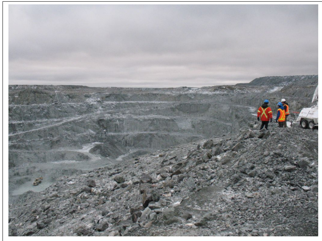
Photo No. 6 Push back area of Portage Pit E. Radar movement detector at right.
