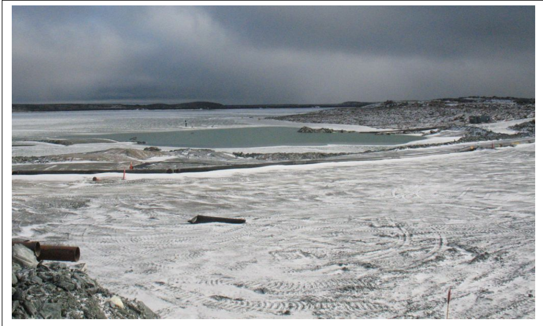
Photo No. 5 Reclaim water pump. Saddle Dam 3 in foreground
