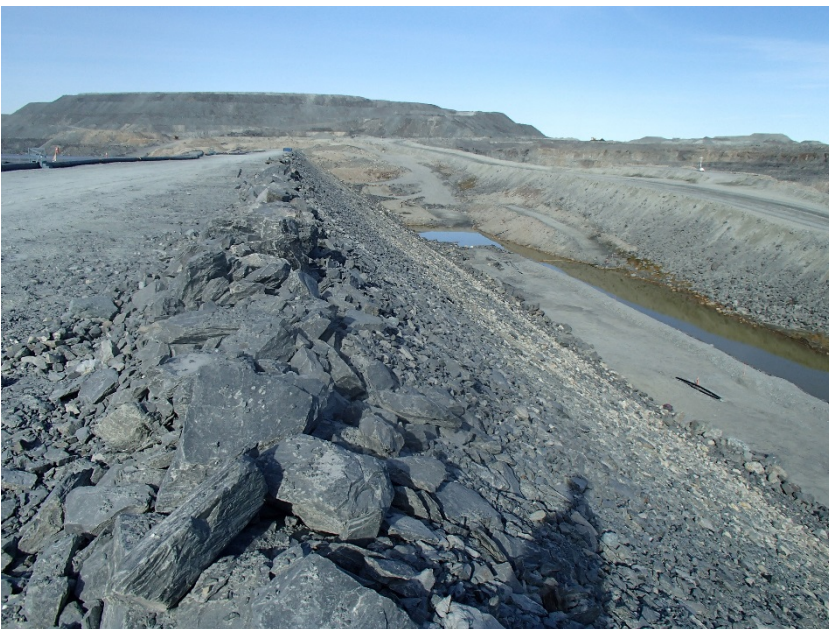
Photograph B7-10 Central Dike and Saddle Dam 5
