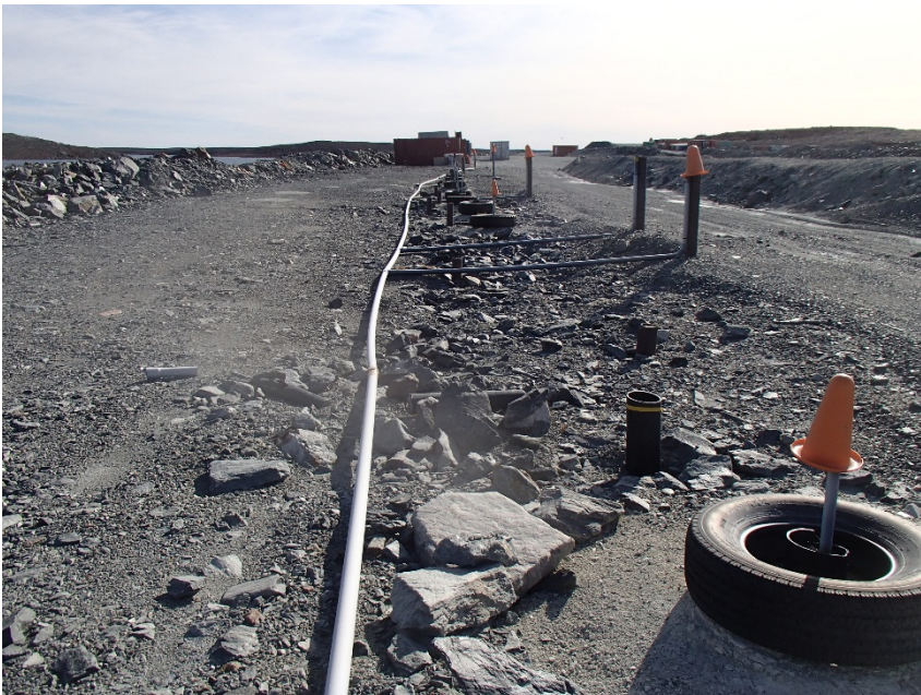
Photograph A1-4 East Dike
