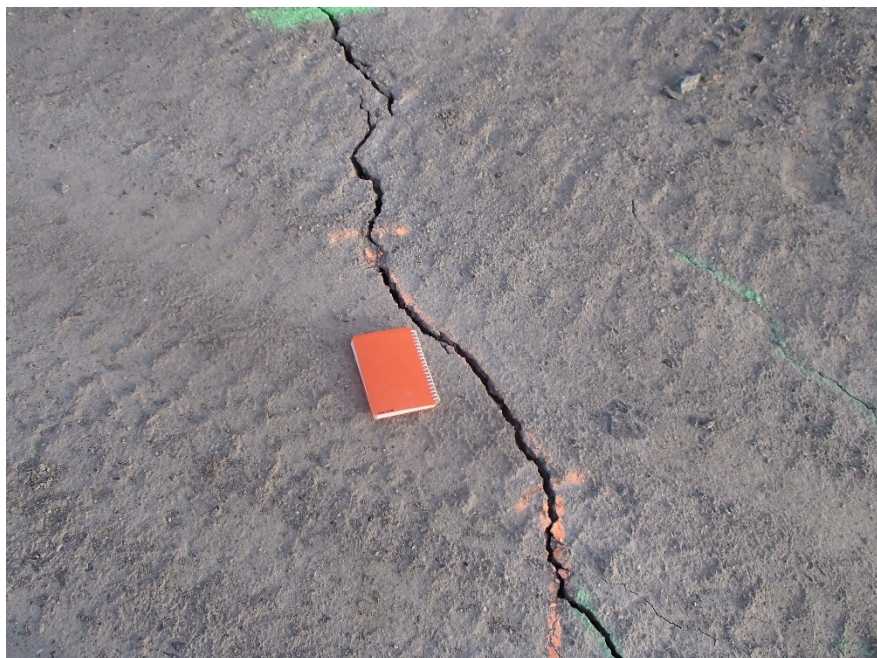
Photograph B7-8 Stormwater Dike
