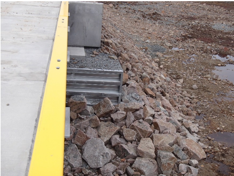
Photograph E2-14 Bridges 4 – km 20+000
