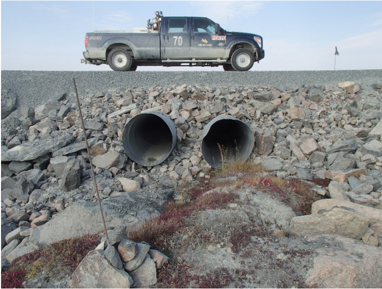
Photograph D1-69: R-24 km 98+100
