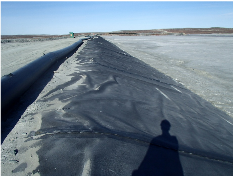
Photograph B1-4 Tailings Storage Facility
