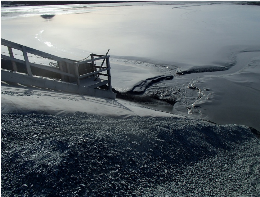
Photograph B7-7 Central Dike and Saddle Dam 5
