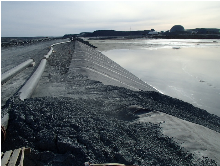
Photograph B7-6 Central Dike and Saddle Dam 5
