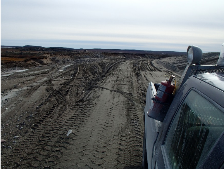
Photograph F2-9 Eskers and Quarries 4 – km 46+000
