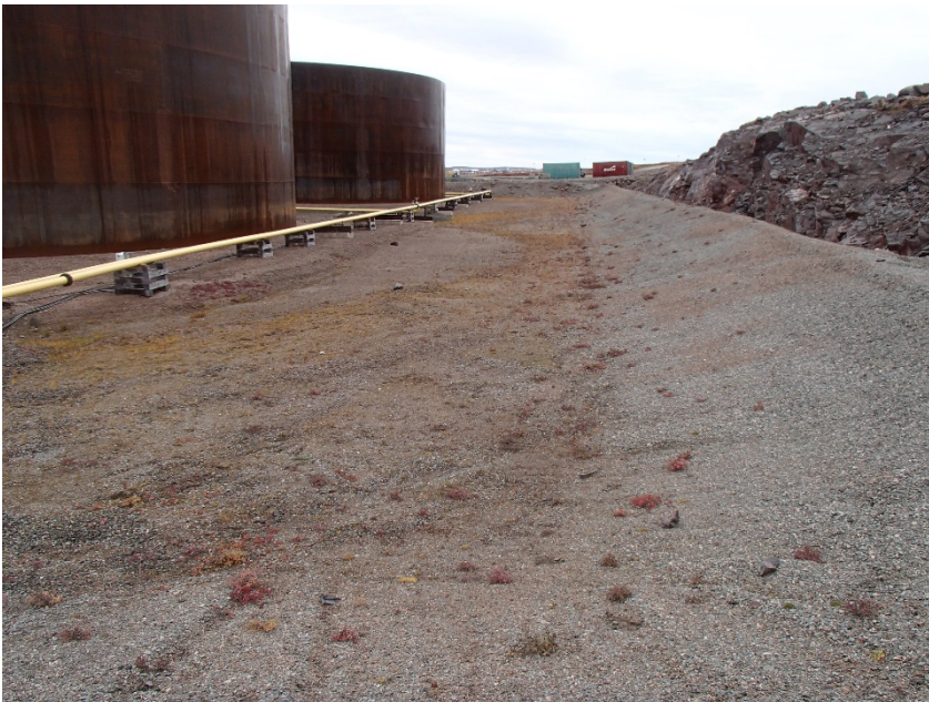
Photograph G1-16 Baker Lake Tank Farm
