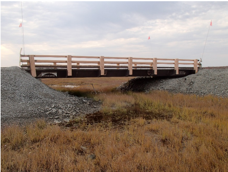
Photograph D2-18 Bridges 5 – R13 km 62+060
