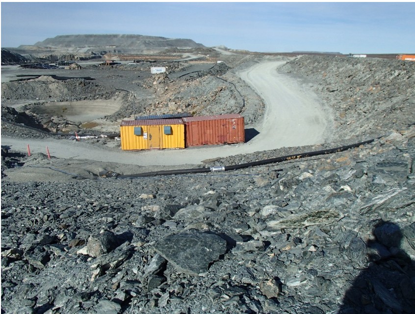
Photograph A1-10 East Dike
