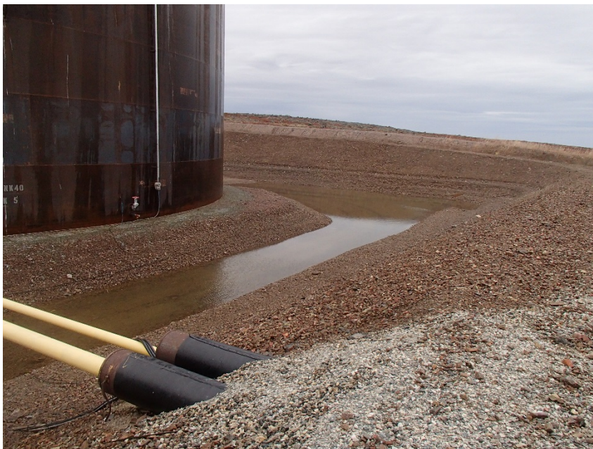
Photograph G1-20 Baker Lake Tank Farm
