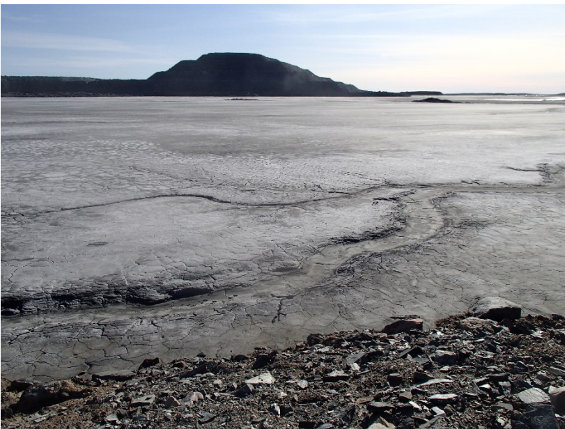
Photograph B1-6 Tailings Storage Facility
