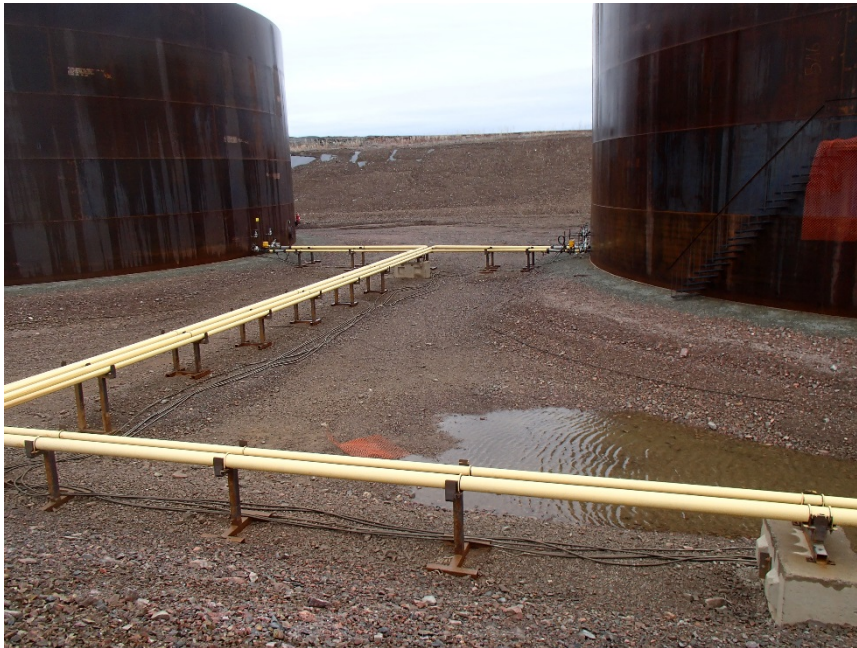
Photograph G1-19 Baker Lake Tank Farm
