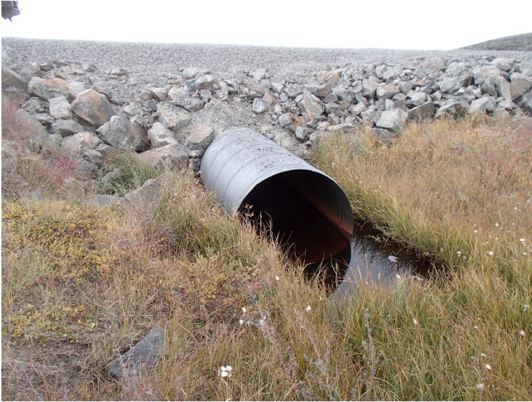
Photograph D1-31: R-05A km 15+745
