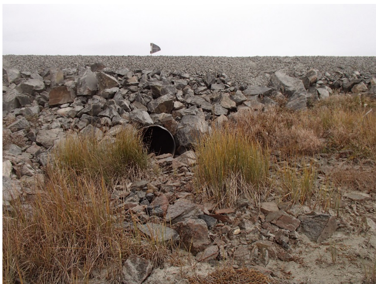
Photograph D1-24: PC-2 km 13+405
