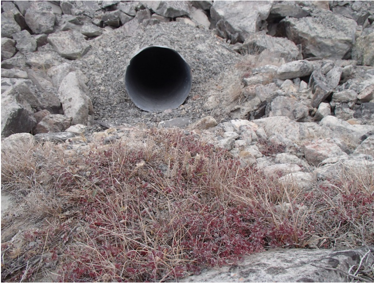
Photograph D1-45: PC-9 km 35+690
