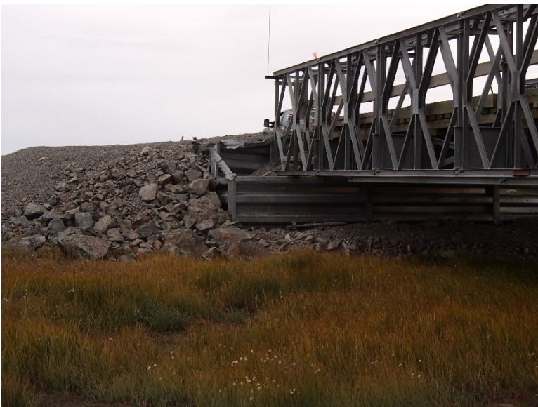
Photograph D2-6 Bridges 2 – R05 km 17+600
