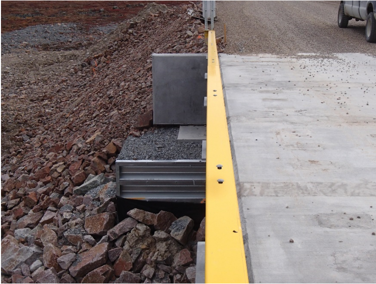
Photograph E2-15 Bridges 4 – km 20+000
