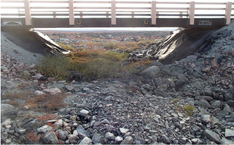
Photograph D2-25 Bridges 8 – R18 km 79+500
