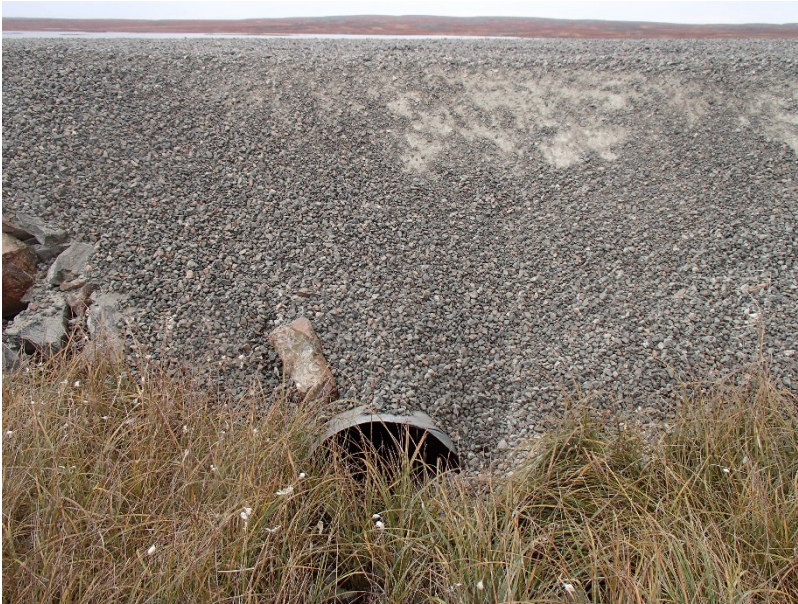
Photograph D1-25: PC-3 km 13+685
