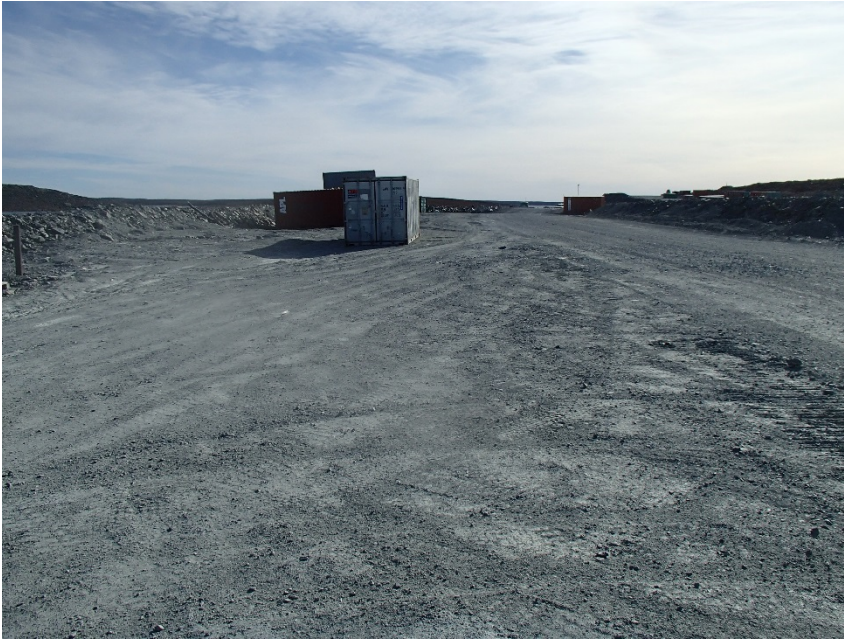
Photograph A1-1 East Dike
