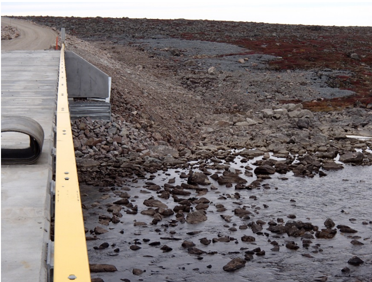
Photograph E2-18 Bridges 5 – km 23+900
