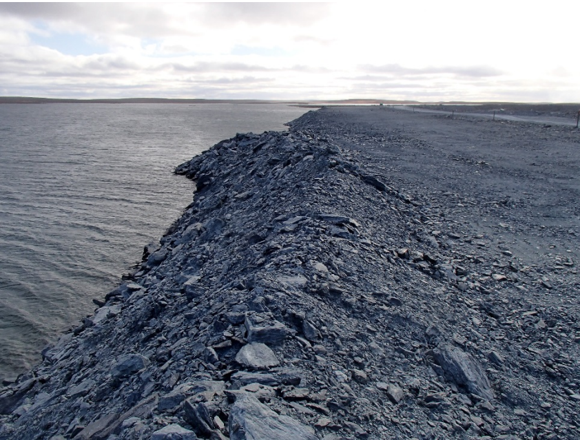
Photograph A3-10 Bay Goose Dike
