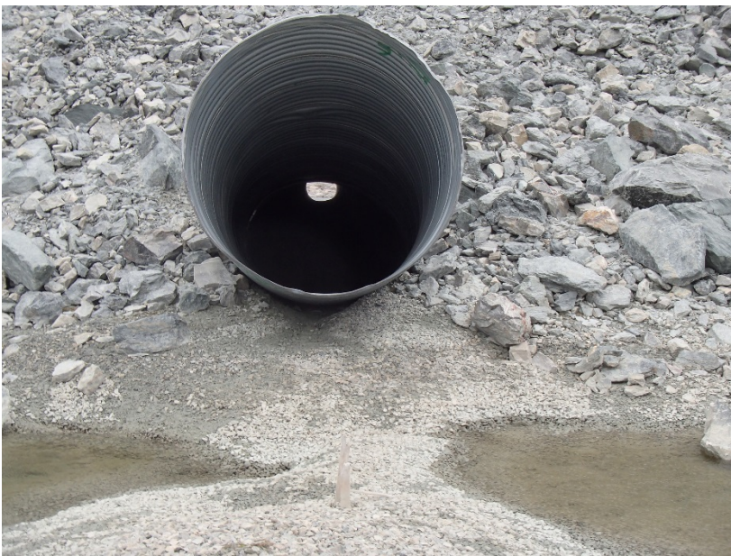
Photograph H1-2 Vault Road Culverts
