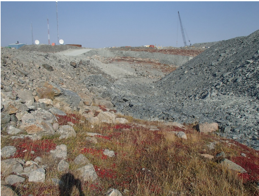
Photograph A2-6 South Camp Dike
