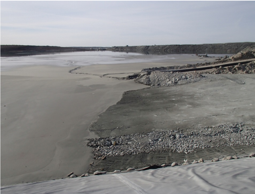
Photograph B7-2 Central Dike and Saddle Dam 5
