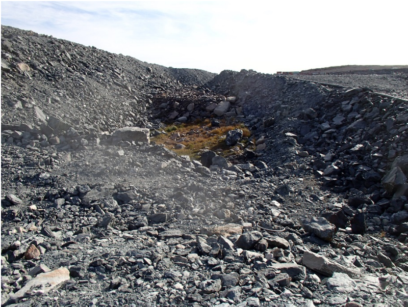
Photograph A1-14 East Dike
