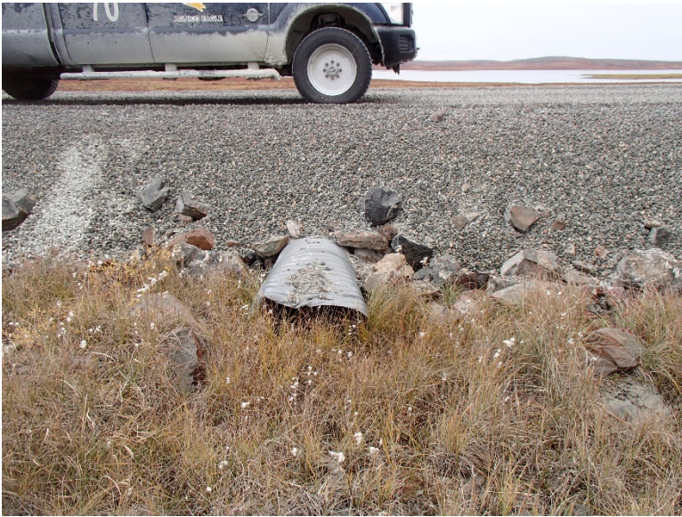
Photograph D1-21: PC-13 km 12+745
