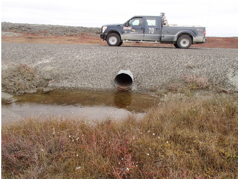
Photograph D1-28: unnamed km 13+950
