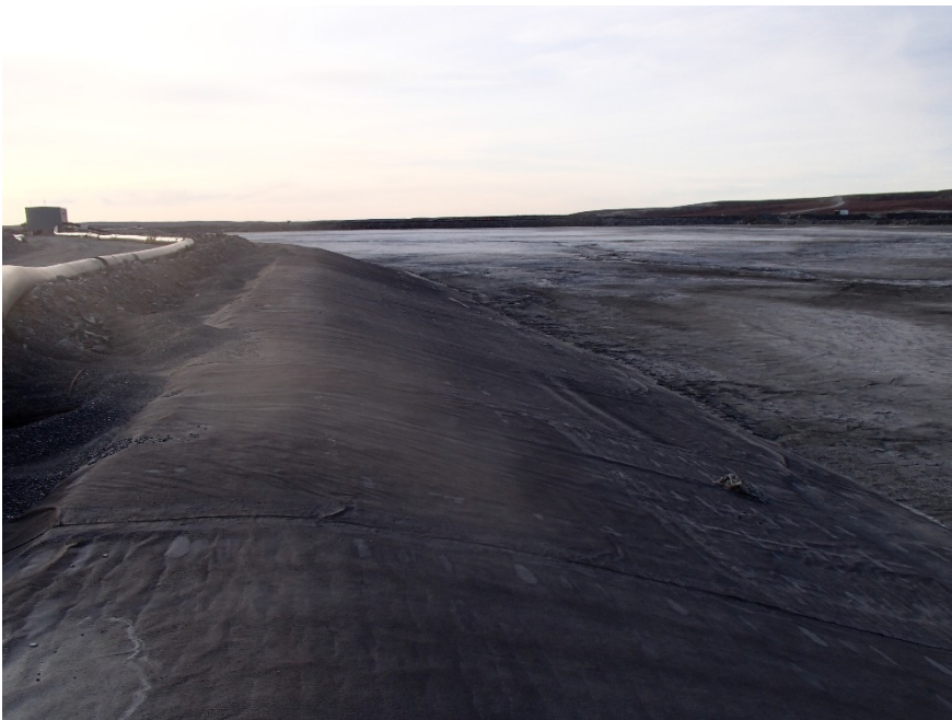
Photograph B7-6 Stormwater Dike
