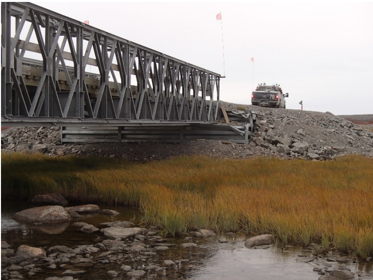
Photograph D2-8 Bridges 2 – R05 km 17+600
