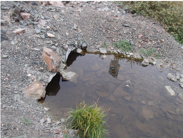
Photograph D1-4: PRC2 km 0+470
