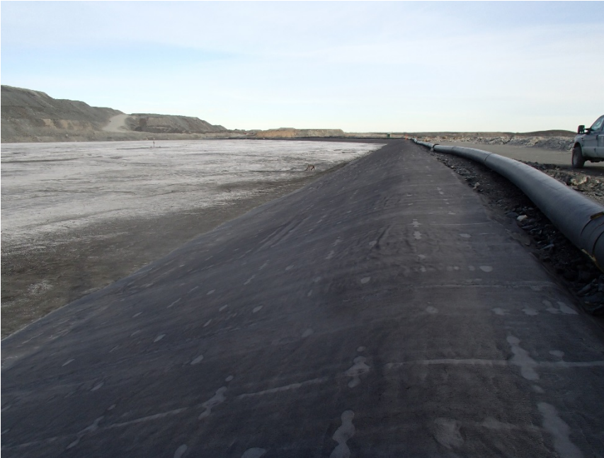
Photograph B7-5 Stormwater Dike
