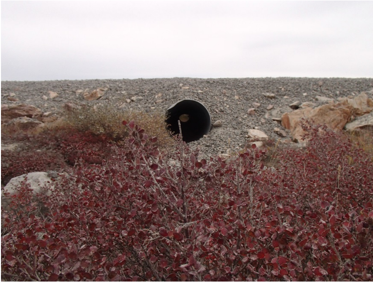
Photograph D1-49: PC-11 km 39+552
