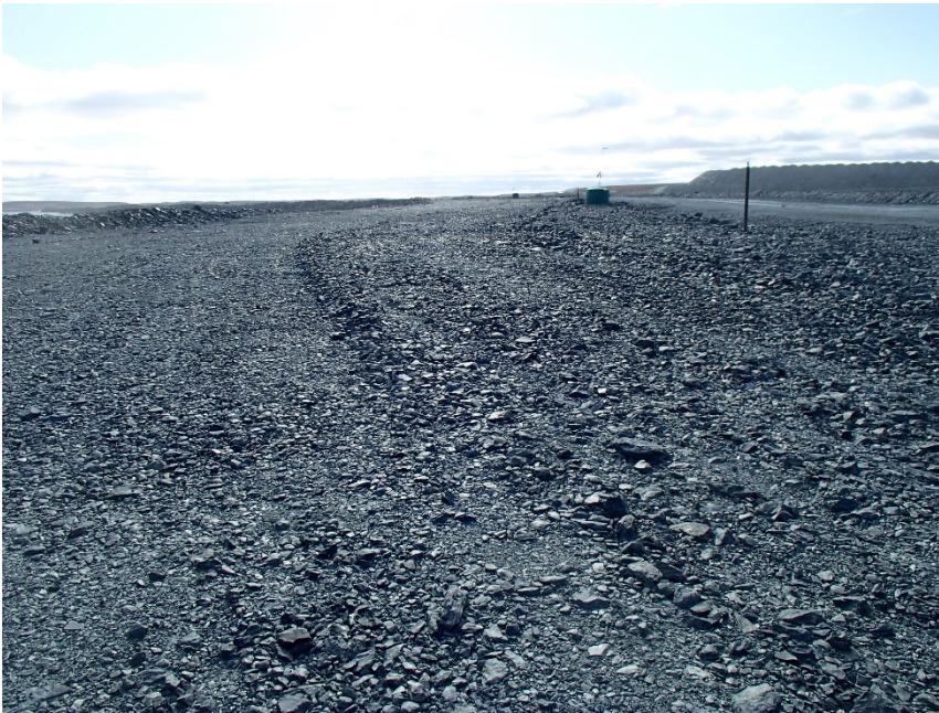
Photograph A3-1 Bay Goose Dike
