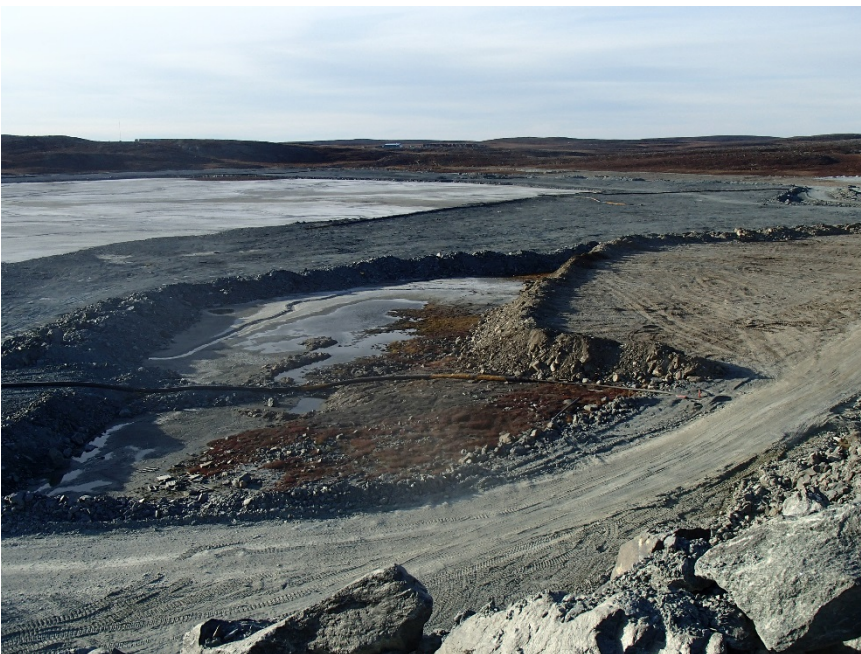
Photograph B1-14 Tailings Storage Facility
