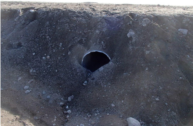
Photograph E1-8: Culvert #203 km 48+800
