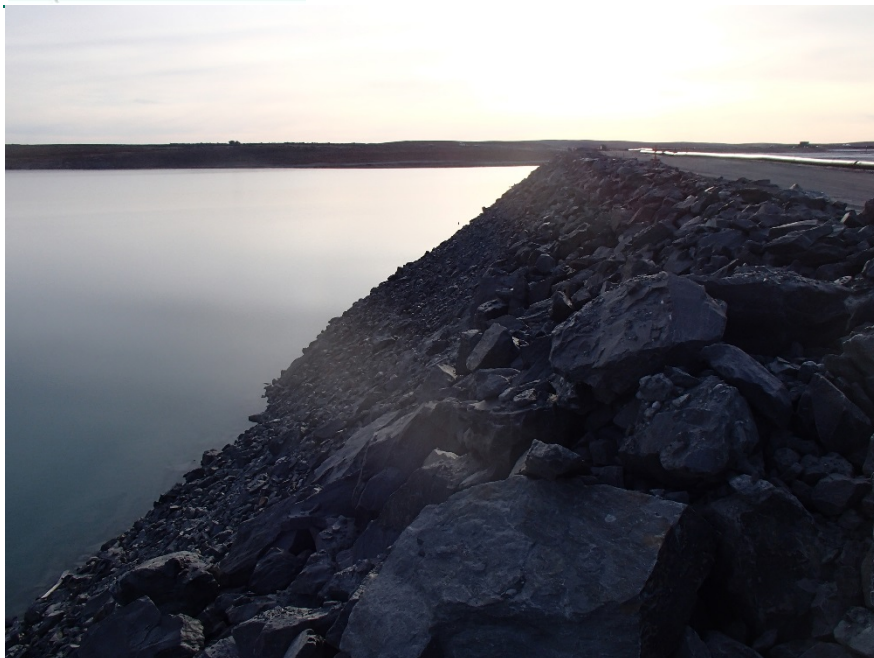
Photograph B7-7 Stormwater Dike
