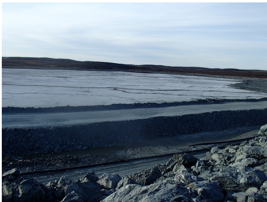
Photograph B1-12 Tailings Storage Facility
