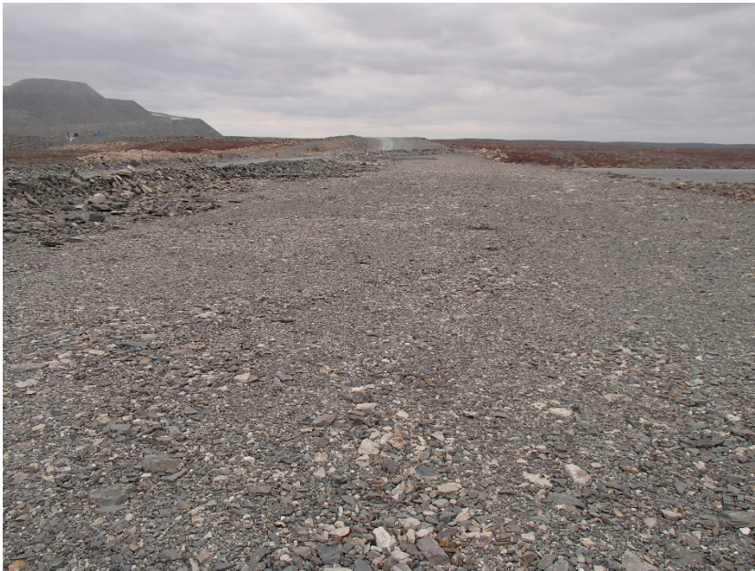
Photograph A4-6 Vault Dike
