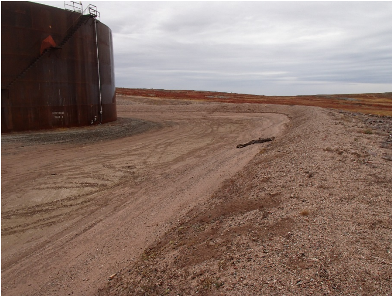
Photograph G1-10 Baker Lake Tank Farm
