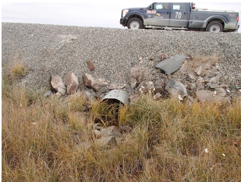
Photograph D1-16: PC-1 km 9+952
