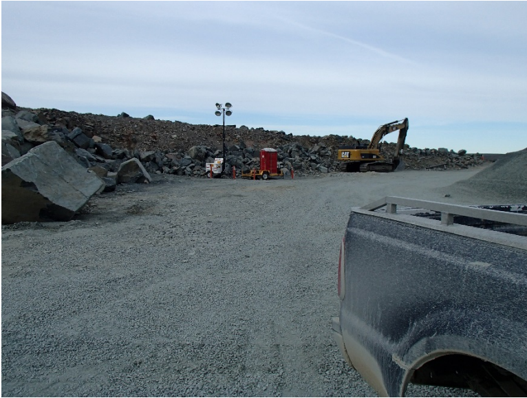
Photograph F2-5 Eskers and Quarries 3 – km 35+000
