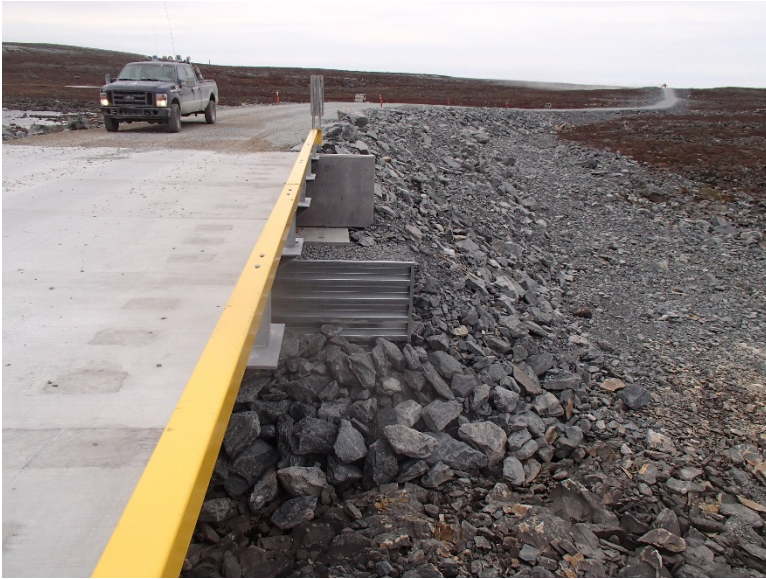
Photograph E2-1 Bridges 1 – km 3+400
