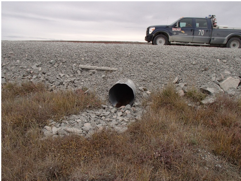
Photograph D1-40: PC-7 km 20+250
