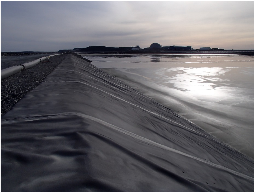
Photograph B1-16 Tailings Storage Facility
