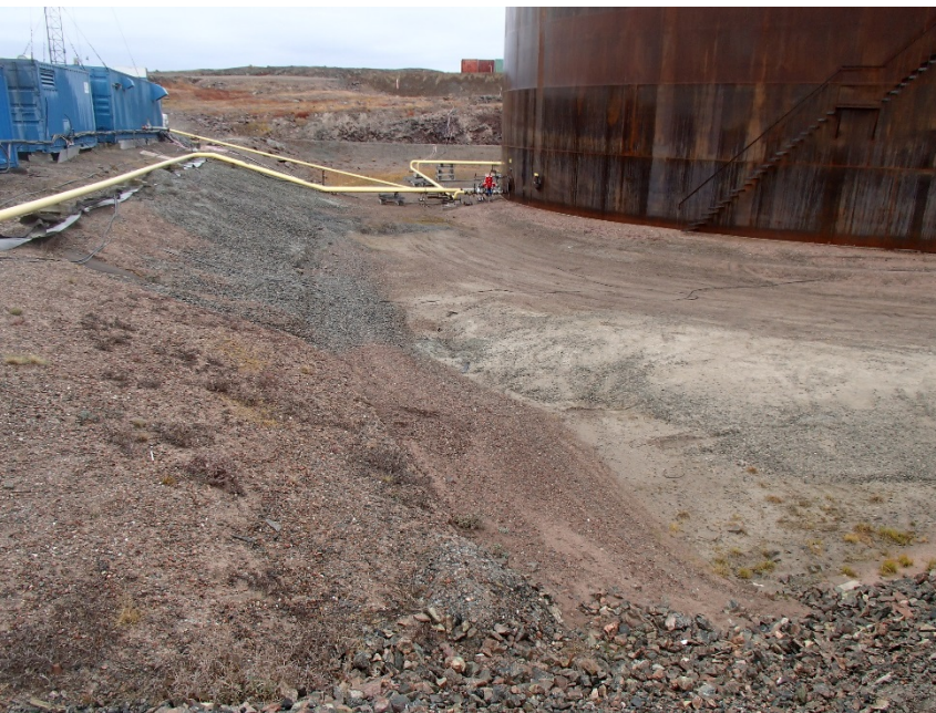
Photograph G1-2 Baker Lake Tank Farm
