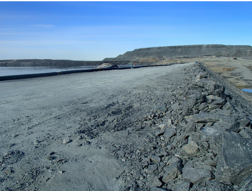
Photograph B7-12 Central Dike and Saddle Dam 5
