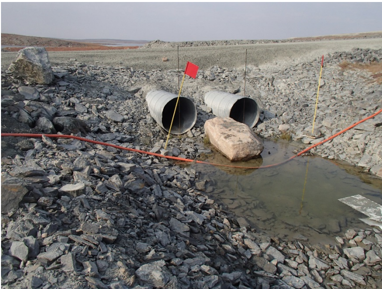
Photograph D1-72: R-26 km 104+400
