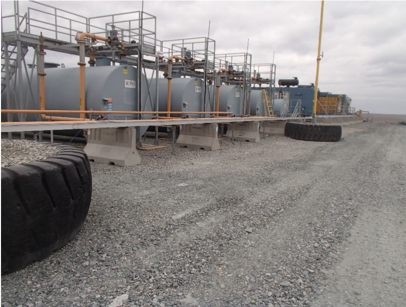
Photograph G3-3 Vault Tank Farm
