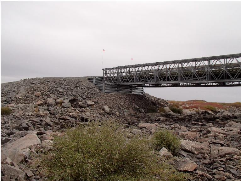
Photograph D2-2 Bridges 1 – R02 km 8+750
