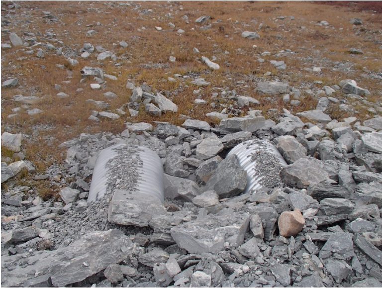
Photograph E1-1: Culvert #39 km 9+193
