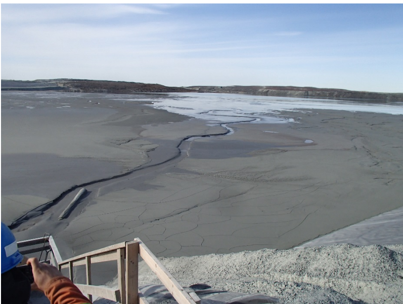
Photograph B1-18 Tailings Storage Facility
