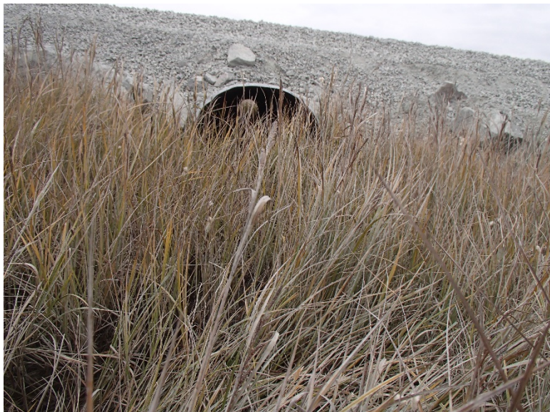
Photograph D1-43: PC-8 km 29+420
