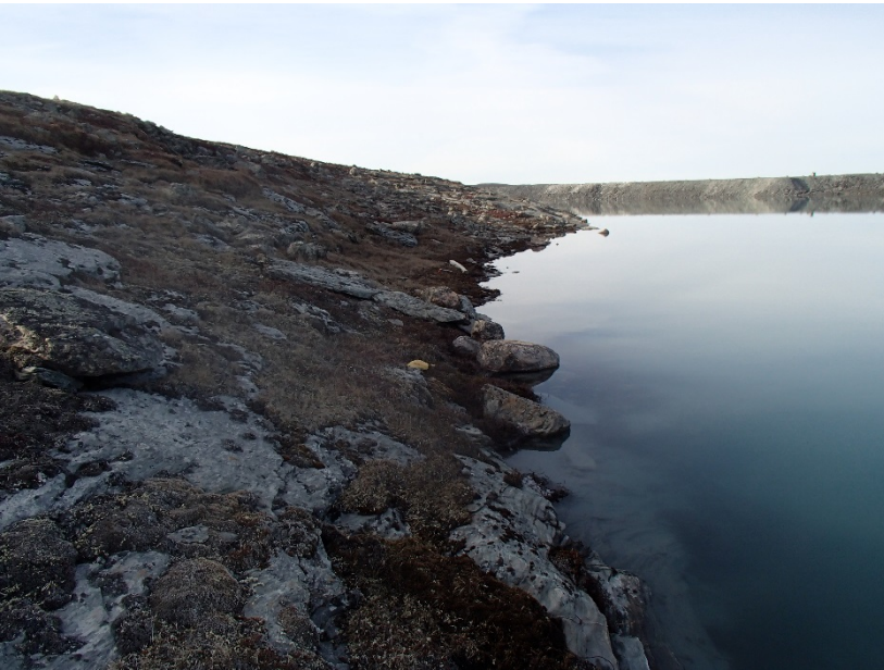
Photograph B1-22 Tailings Storage Facility
