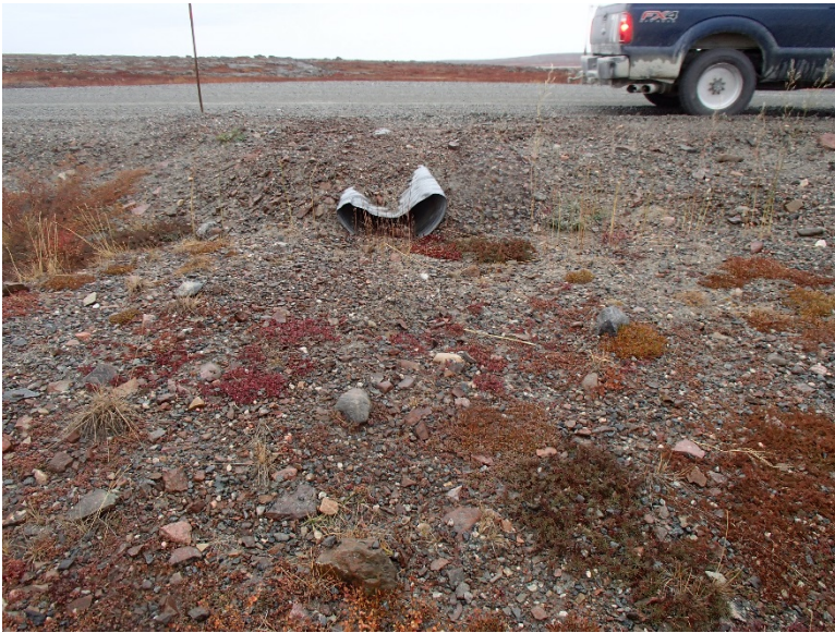
Photograph D1-7: R-00A km 2+550
