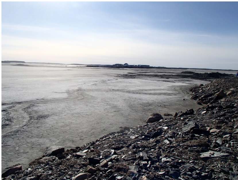
Photograph B1-7 Tailings Storage Facility
