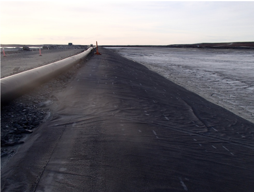
Photograph B7-4 Stormwater Dike
