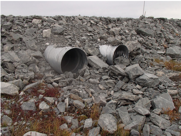
Photograph E1-2: Culvert #39 km 9+193
