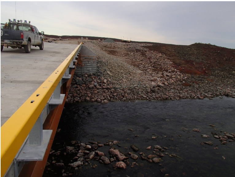
Photograph E2-28 Bridges 7 – km 32+300
