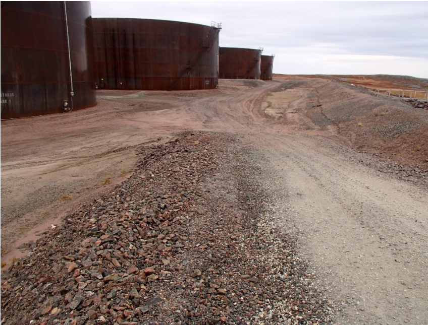
Photograph G1-1 Baker Lake Tank Farm
