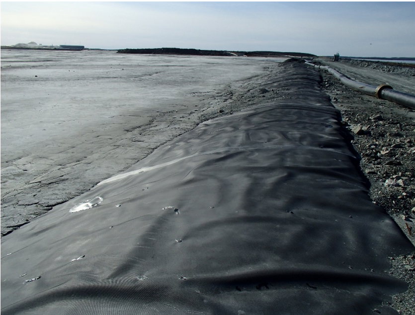
Photograph B2-5 Saddle Dam 1
