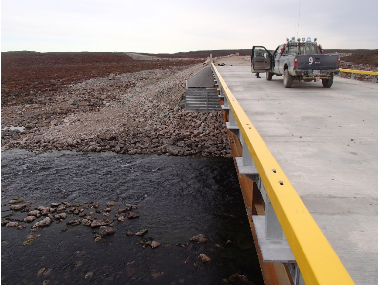
Photograph E2-27 Bridges 7 – km 32+300
