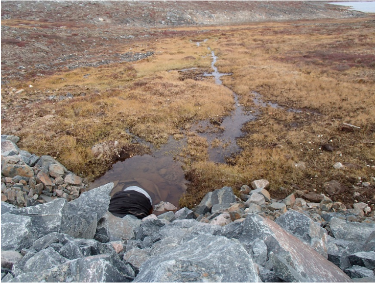
Photograph E1-7: Culvert #167 km 41+843
