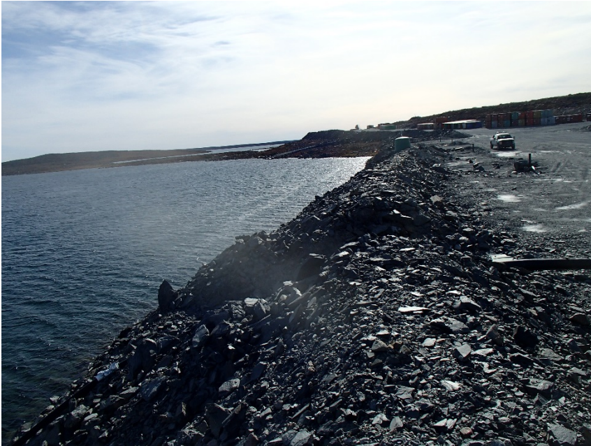
Photograph A1-9 East Dike
