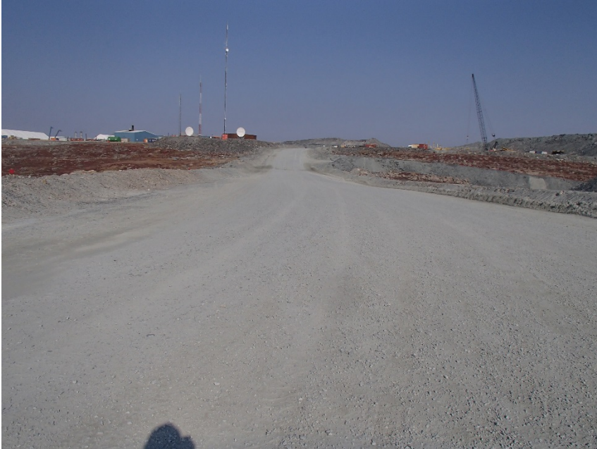
Photograph A2-3 South Camp Dike
