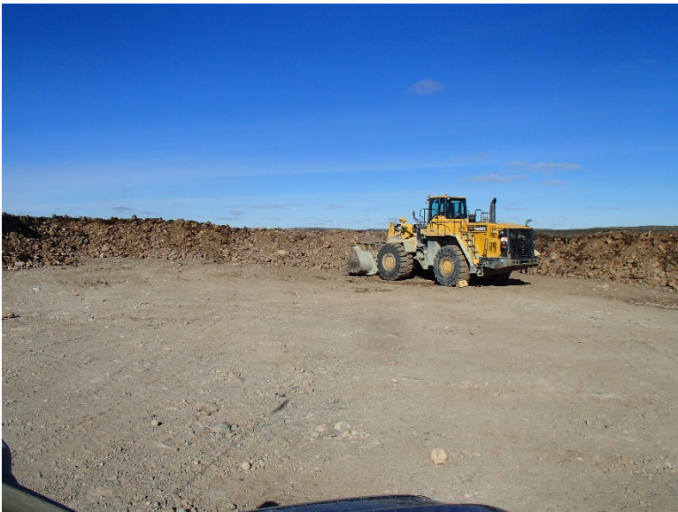
Photograph F2-14 Eskers and Quarries 6 – km 62+000
