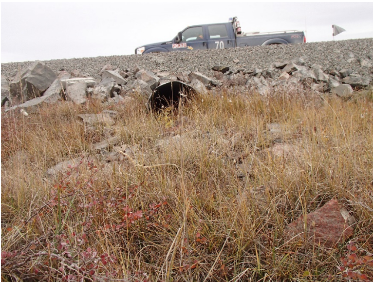
Photograph D1-22: PC-13 km 12+745
