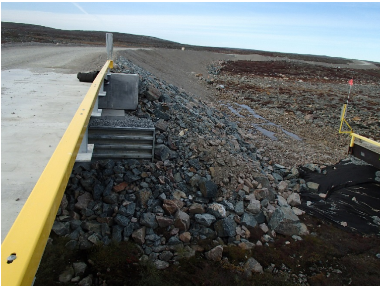
Photograph E2-30 Bridges 8 – km 43+500
