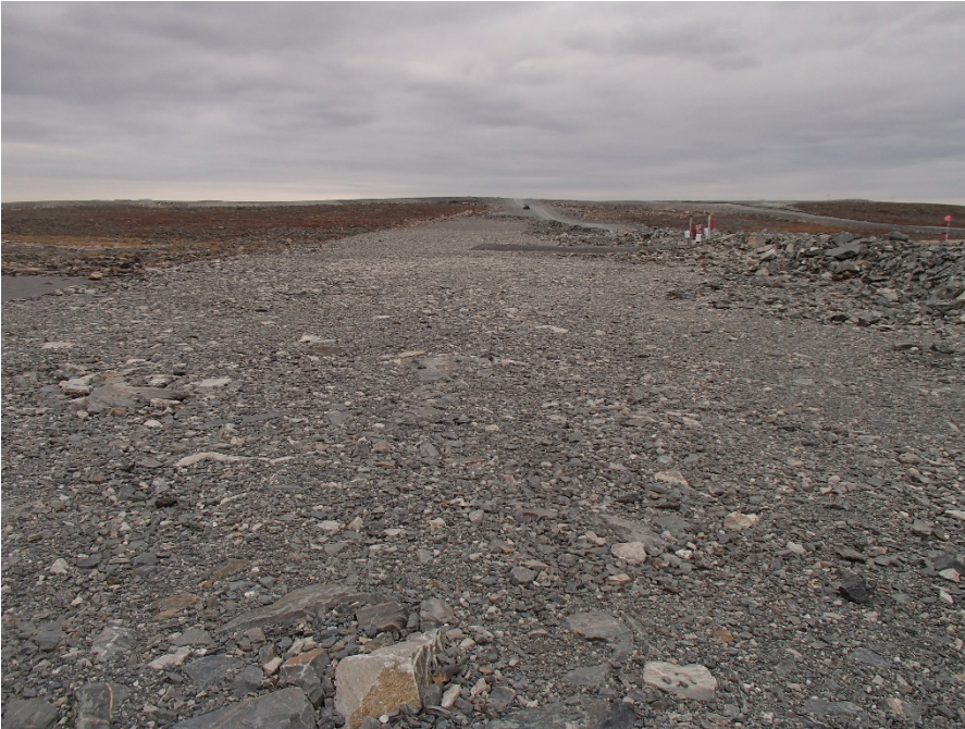
Photograph A4-5 Vault Dike
