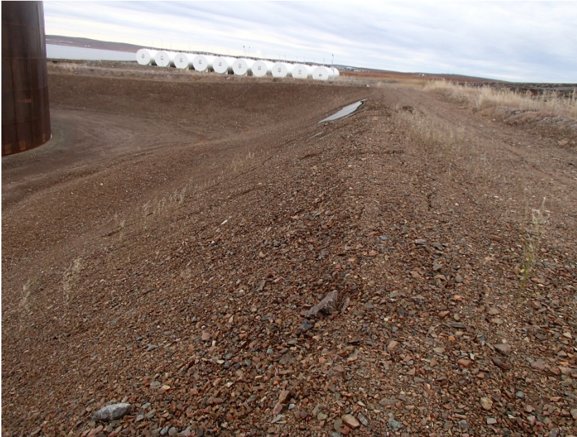
Photograph G1-23 Baker Lake Tank Farm
