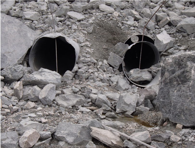
Photograph H1-5 Vault Road Culverts
