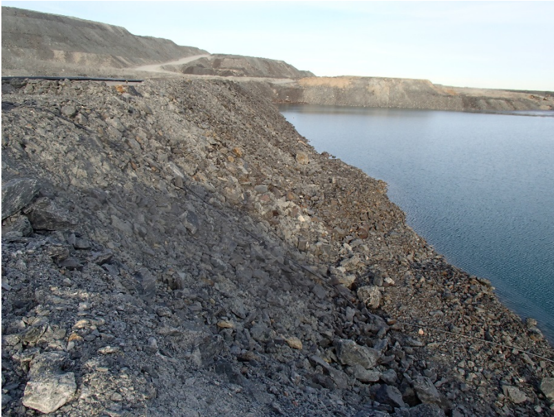
Photograph B7-9 Stormwater Dike
