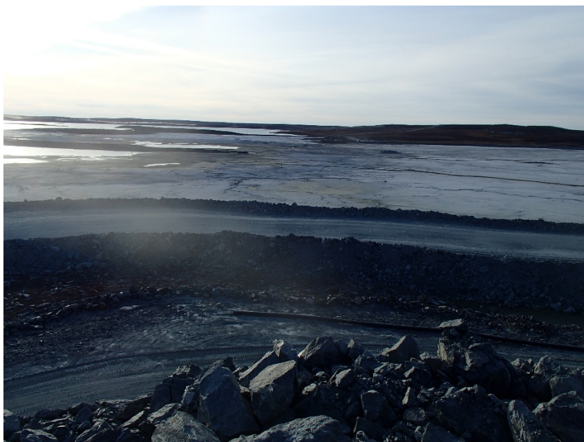
Photograph B1-11 Tailings Storage Facility
