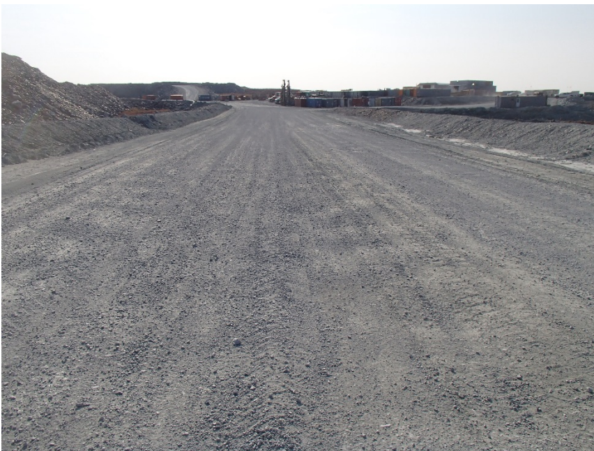
Photograph A2-4 South Camp Dike
