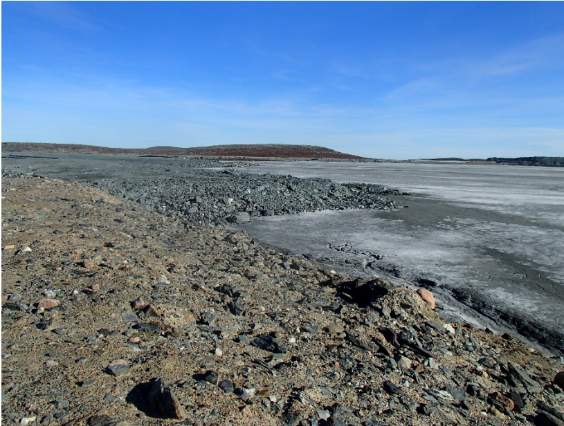
Photograph B1-5 Tailings Storage Facility
