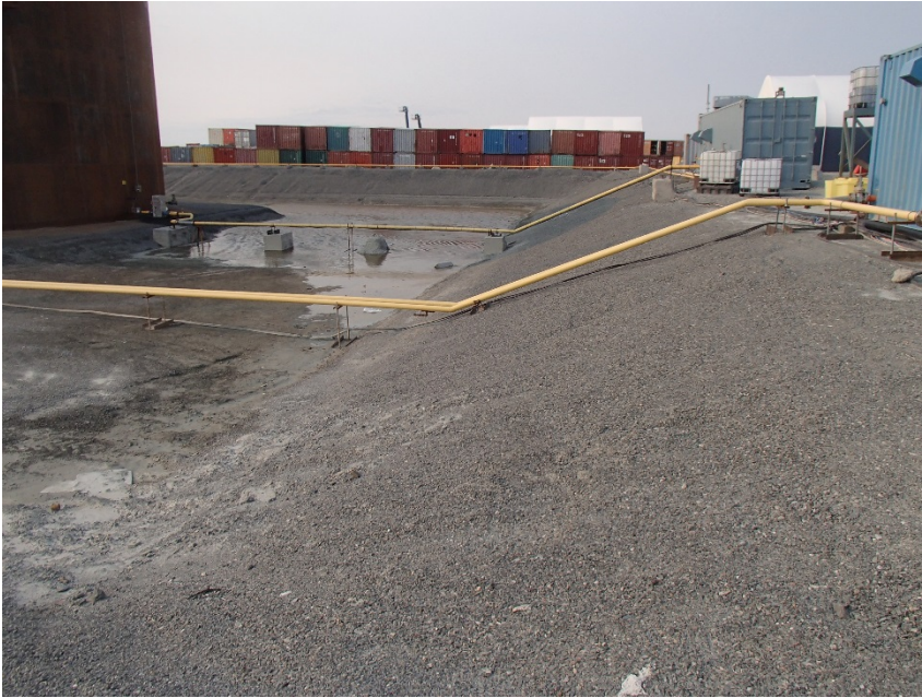
Photograph G2-5 Meadowbank Tank Farm
