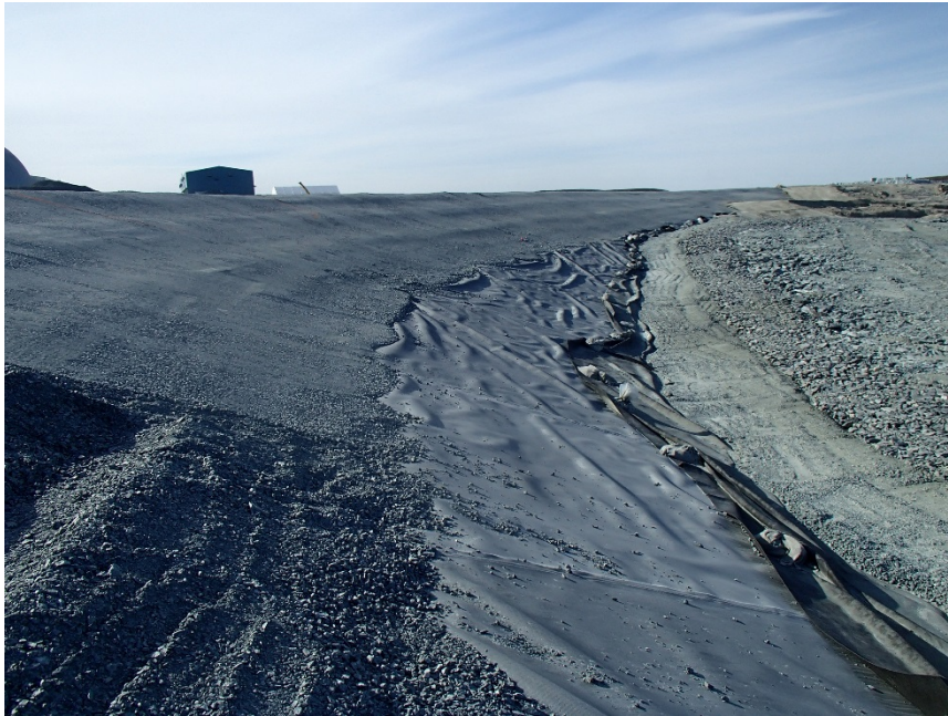
Photograph B7-17 Central Dike and Saddle Dam 5
