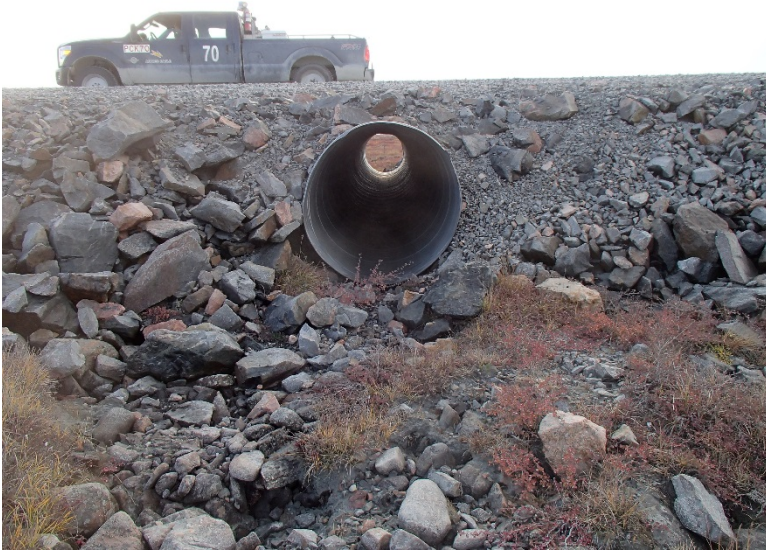
Photograph D1-57: R-17 km 77+440
