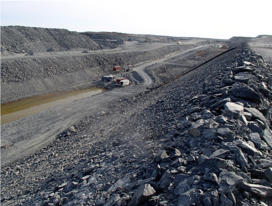
Photograph B7-9 Central Dike and Saddle Dam 5
