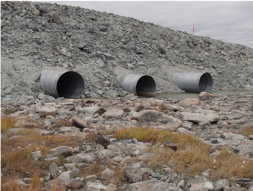
Photograph H1-1 Vault Road Culverts
