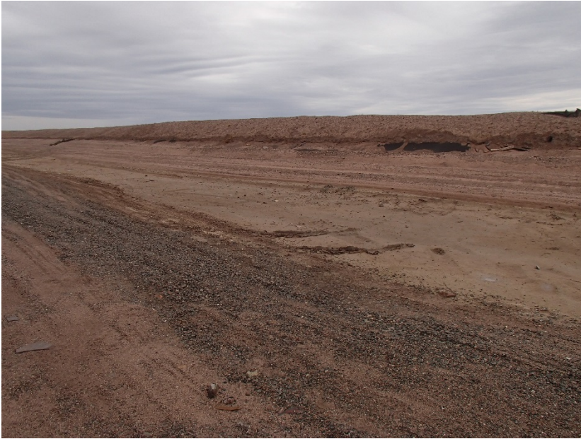
Photograph G1-7 Baker Lake Tank Farm
