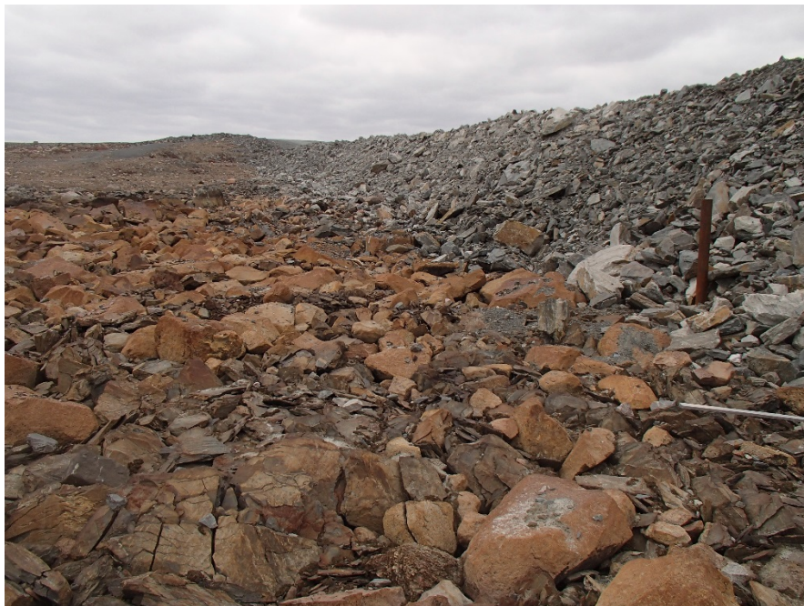
Photograph A4-3 Vault Dike
