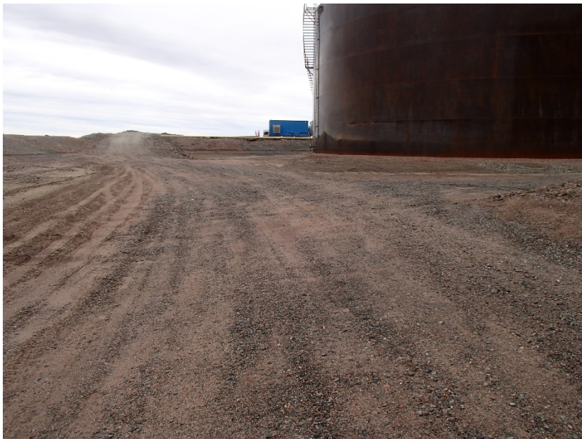
Photograph G1-4 Baker Lake Tank Farm
