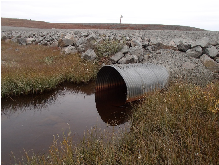
Photograph D1-32: R-05A km 15+745
