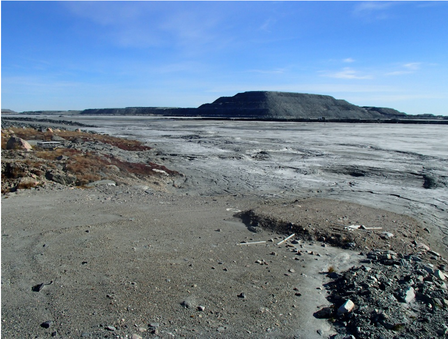
Photograph B1-3 Tailings Storage Facility
