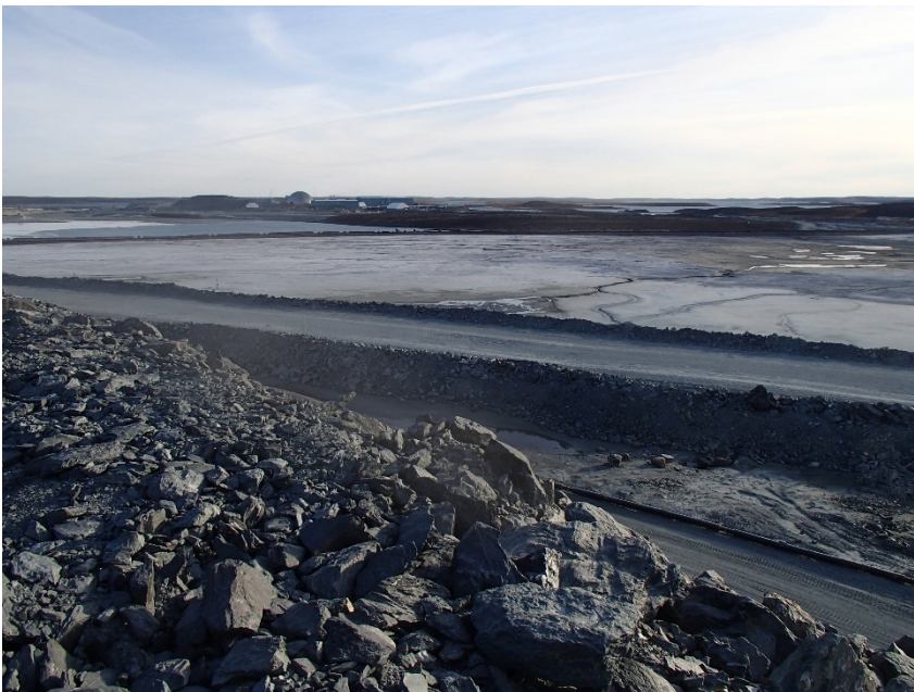
Photograph B1-10 Tailings Storage Facility
