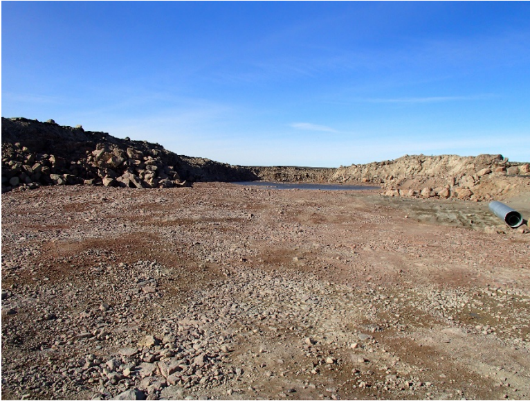
Photograph F2-13 Eskers and Quarries 5 – km 52+000
