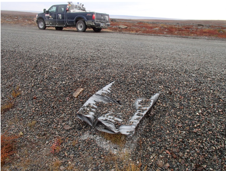
Photograph D1-8: R-00A km 2+550
