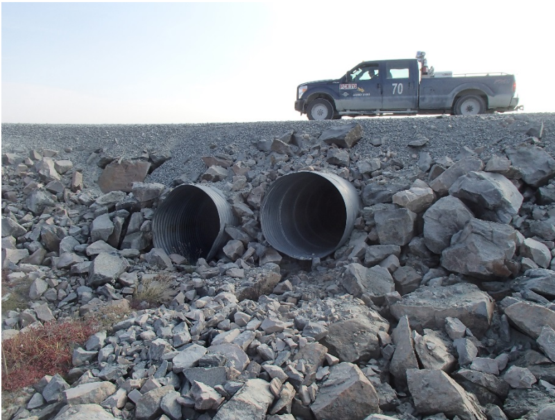
Photograph D1-68: R-24 km 98+100
