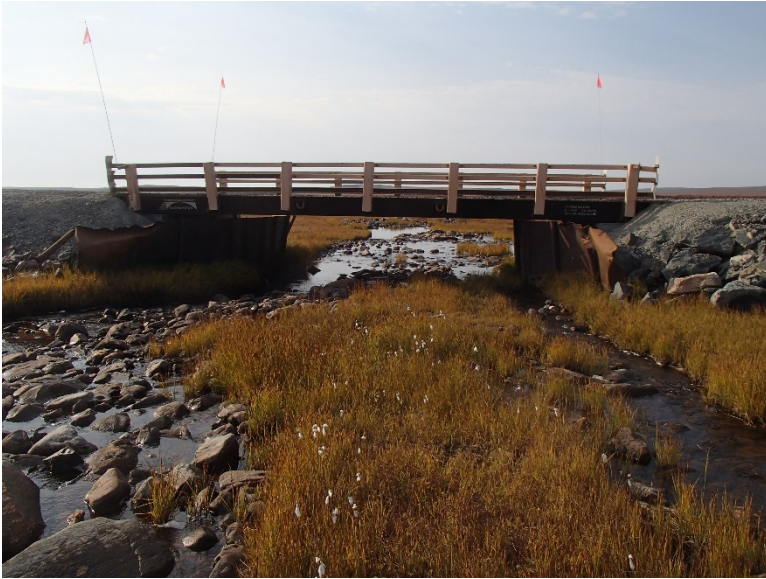
Photograph D2-27 Bridges 9 – R19 km 83+150
