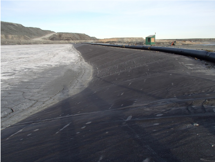
Photograph B4-3 Stormwater Dike
