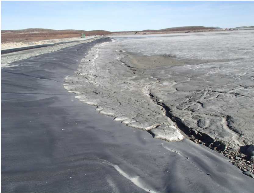
Photograph B1-1 Tailings Storage Facility
