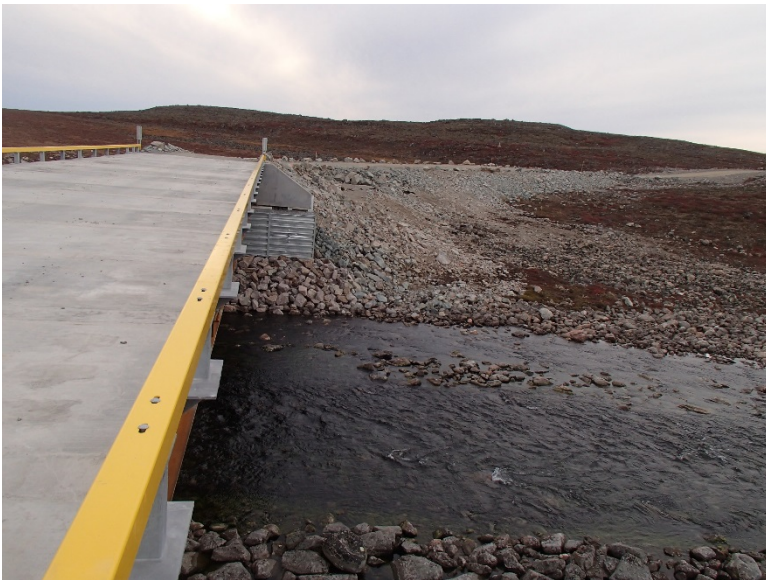
Photograph E2-26 Bridges 7 – km 32+300
