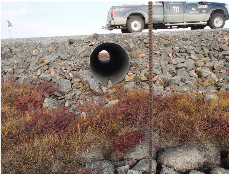
Photograph D1-56: R-17 km 77+440
