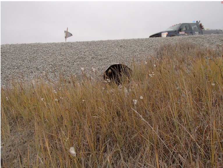
Photograph D1-36: PC-6 km 18+900
