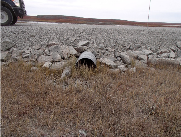
Photograph D1-35: PC-6 km 18+900
