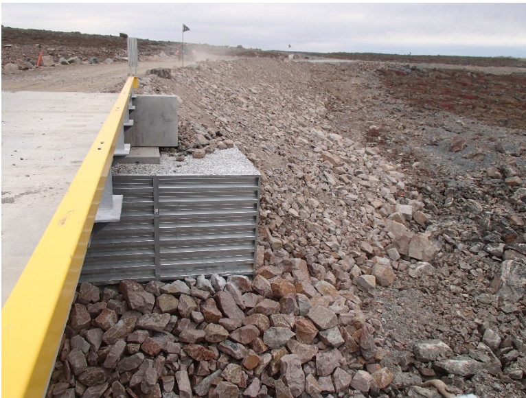
Photograph E2-24 Bridges 6 – km 26+100
