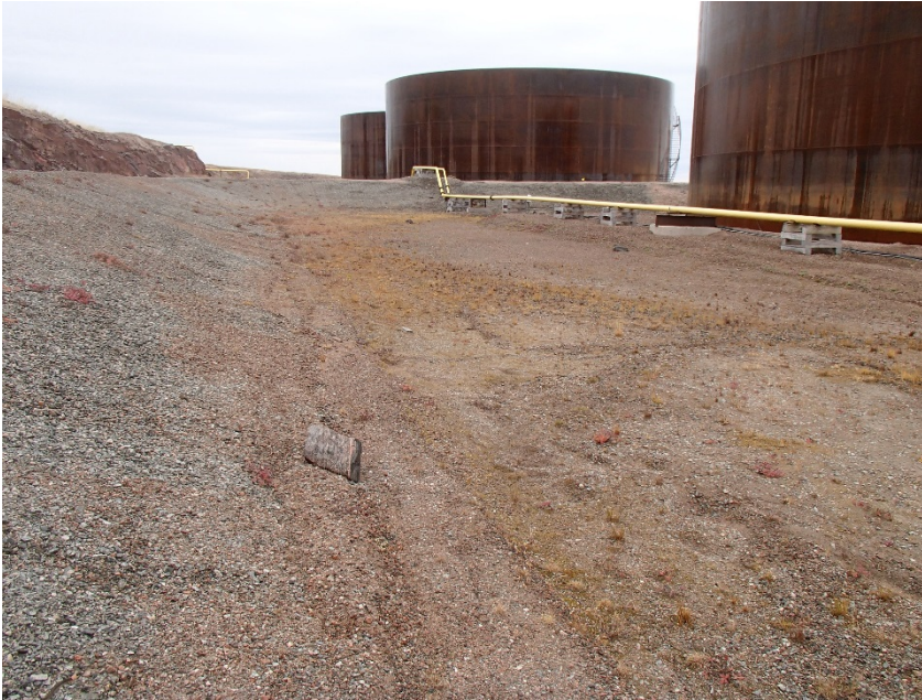
Photograph G1-15 Baker Lake Tank Farm
