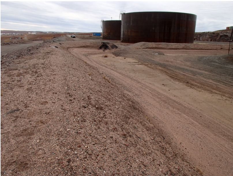
Photograph G1-8 Baker Lake Tank Farm
