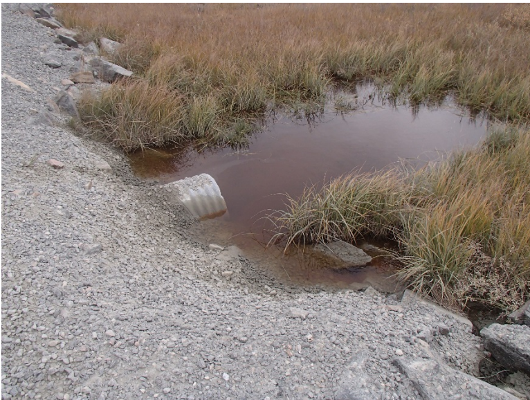
Photograph D1-52: PC-12 km 41+300
