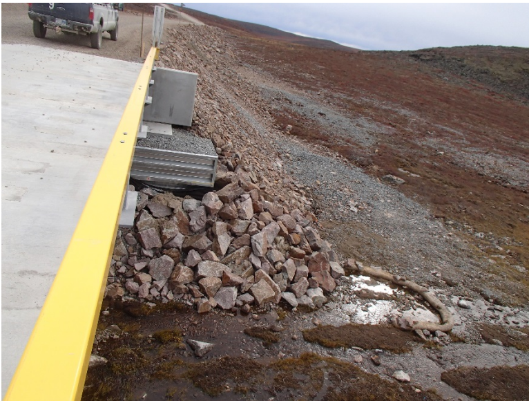
Photograph E2-16 Bridges 4 – km 20+000
