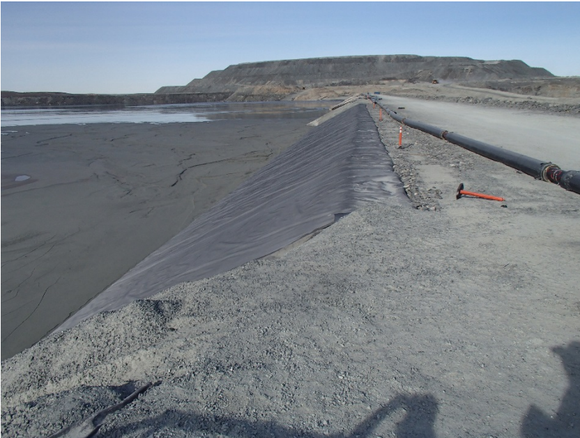
Photograph B7-13 Central Dike and Saddle Dam 5
