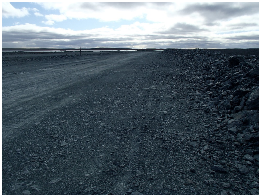
Photograph A3-23 Bay Goose Dike
