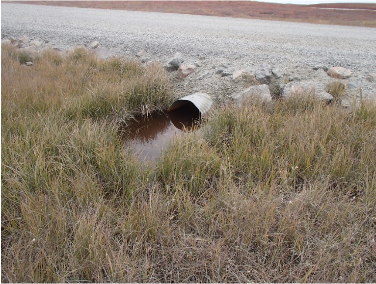
Photograph D1-51: PC-12 km 41+300
