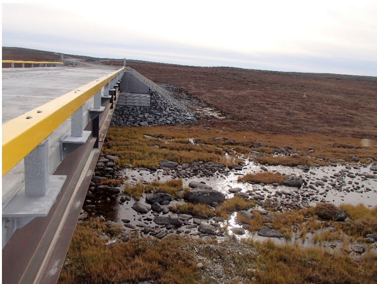
Photograph E2-36 Bridges 9 – km 44+800
