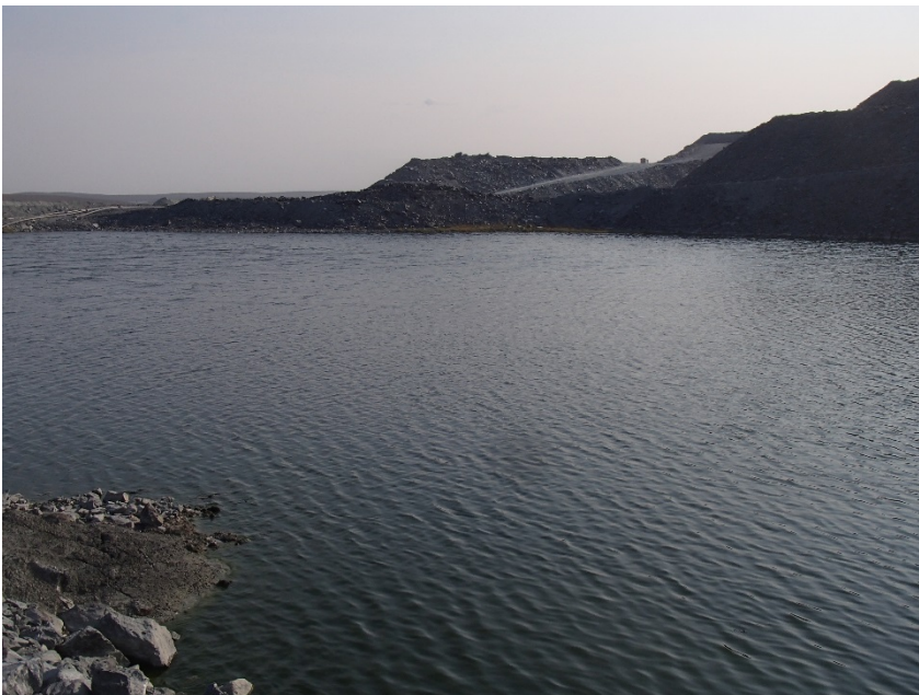
Photograph H7-2 Stormwater Pond
