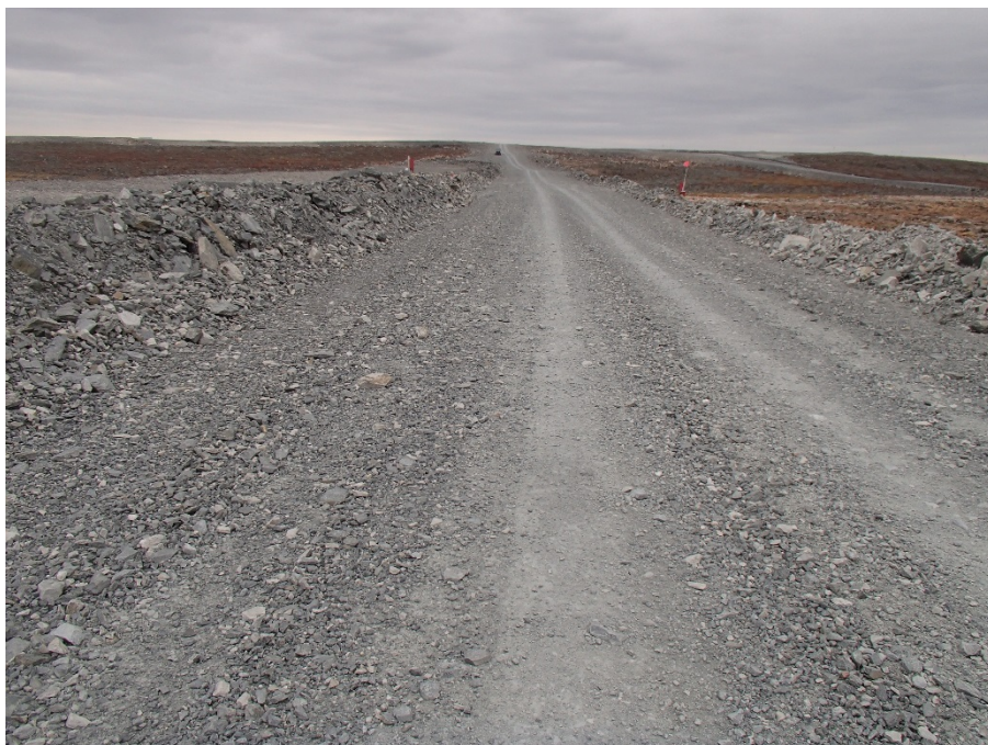
Photograph A4-4 Vault Dike
