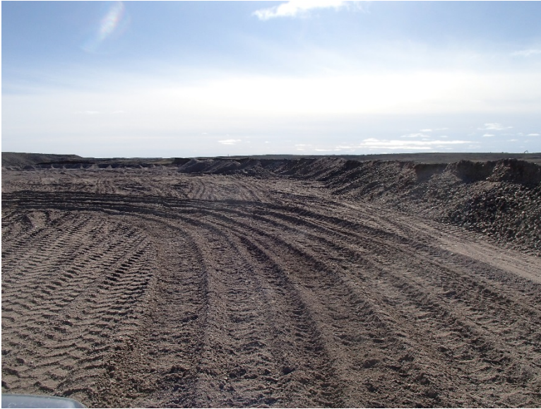
Photograph F2-17 Eskers and Quarries 6 – km 62+000
