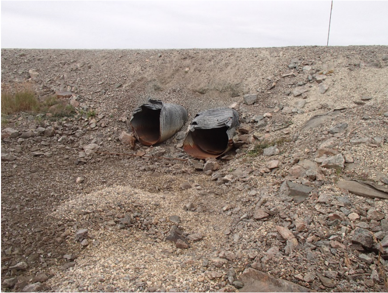
Photograph D1-13: PC-17 km 8+850
