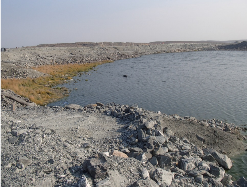
Photograph H7-3 Stormwater Pond
