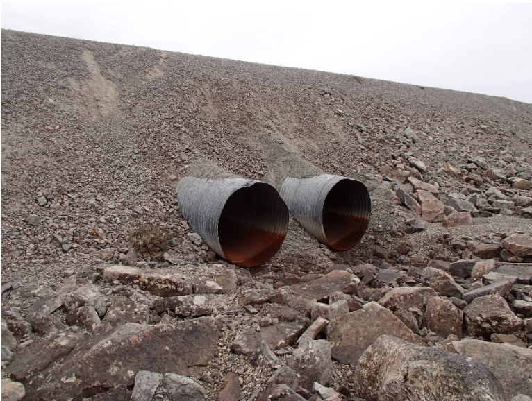
Photograph D1-14: PC-17 km 8+850
