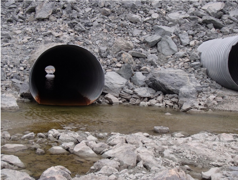
Photograph H1-3 Vault Road Culverts
