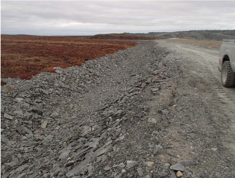
Photograph H2-9 Diversion Ditch and its Sediment and Erosion Protection Structure
