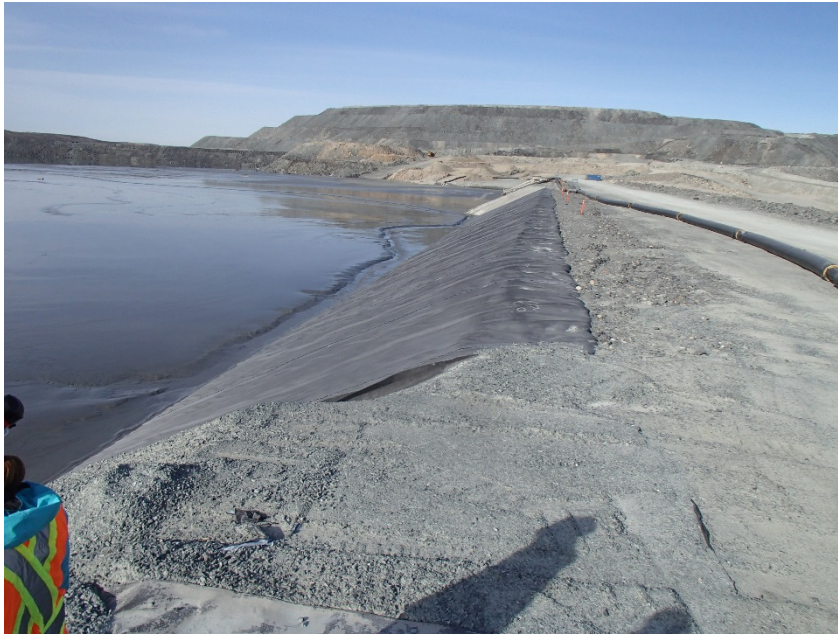
Photograph B7-5 Central Dike and Saddle Dam 5
