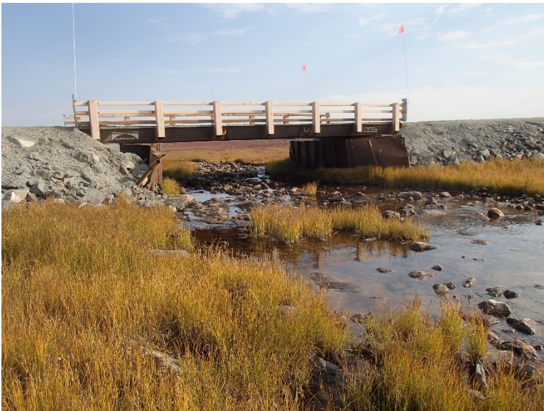
Photograph D2-28 Bridges 9 – R19 km 83+150
