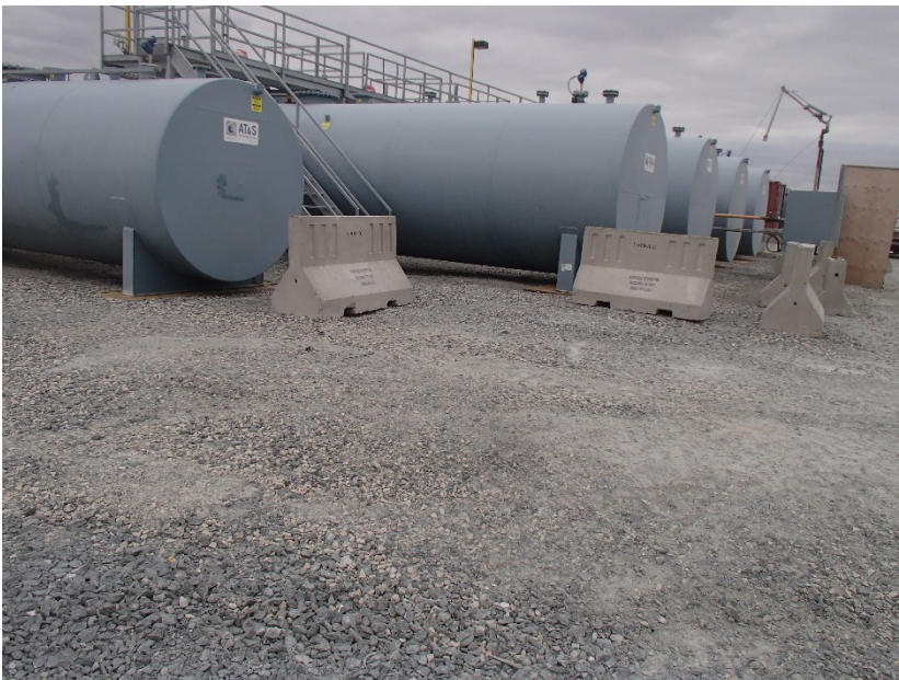
Photograph G3-4 Vault Tank Farm
