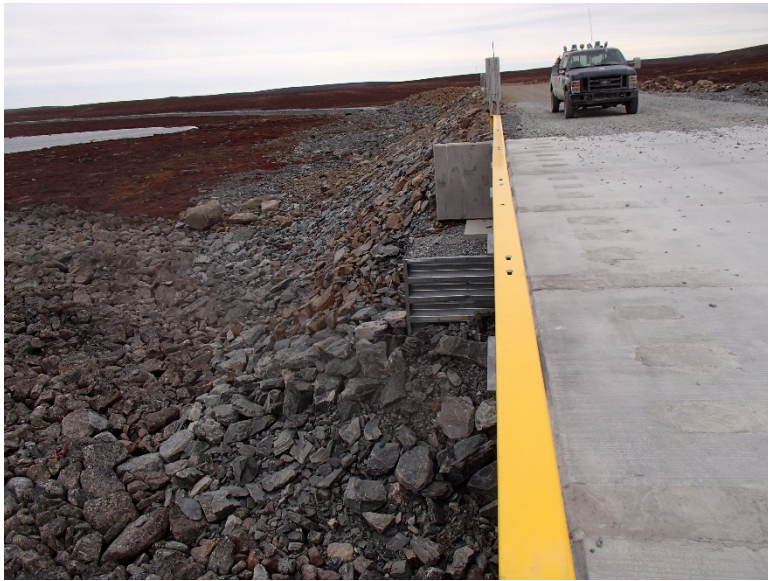
Photograph E2-5 Bridges 2 – km 10+700
