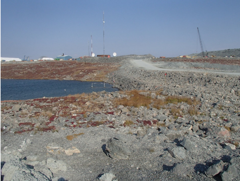
Photograph A2-1 South Camp Dike
