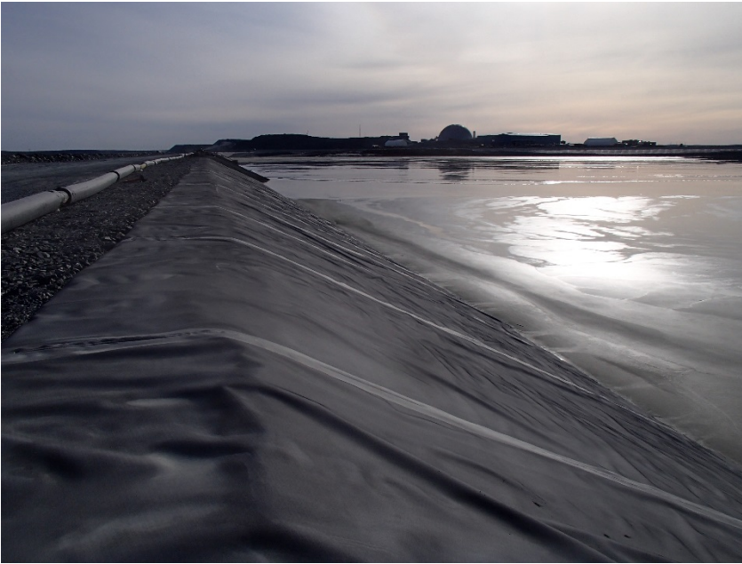
Photograph B7-1 Central Dike and Saddle Dam 5
