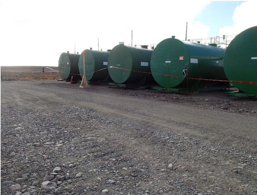
Photograph G4-1 Amaruq Tank Farm
