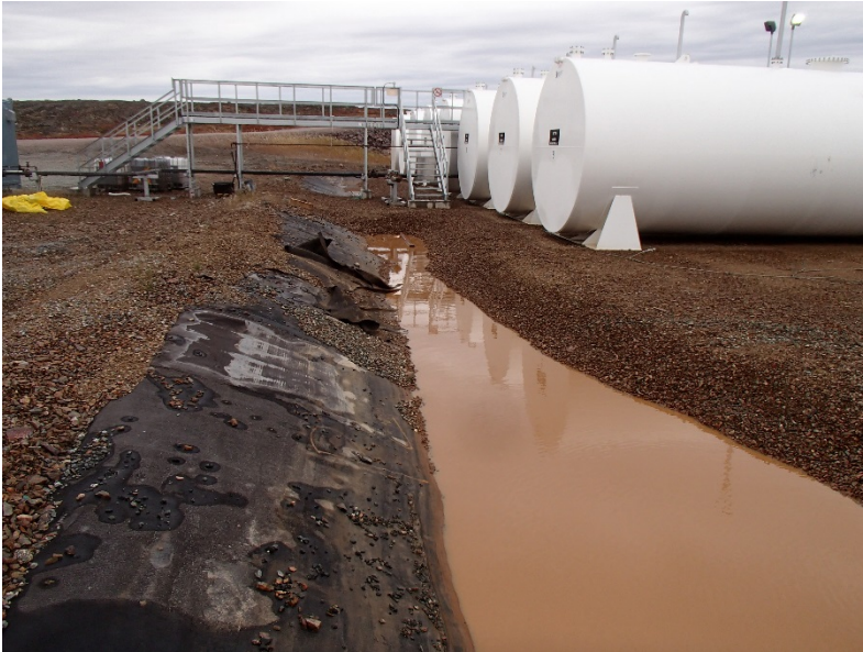
Photograph G1-27 Baker Lake Tank Farm
