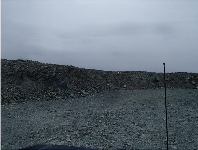
Photograph F1-17: Quarry 9 – km 44+600
