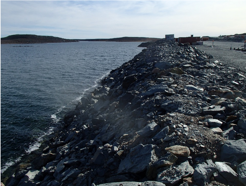
Photograph A1-5 East Dike
