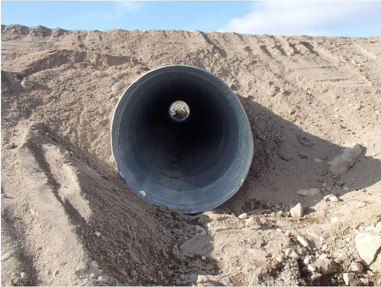
Photograph E1-9: Culvert #278 km 61+870
