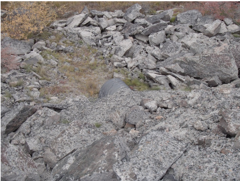
Photograph D1-46: PC-9 km 35+690
