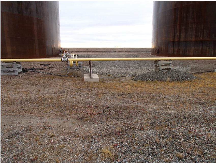
Photograph G1-14 Baker Lake Tank Farm
