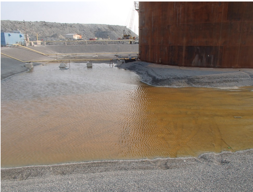
Photograph G2-4 Meadowbank Tank Farm
