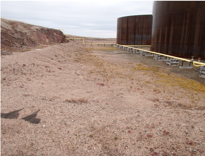
Photograph G1-17 Baker Lake Tank Farm
