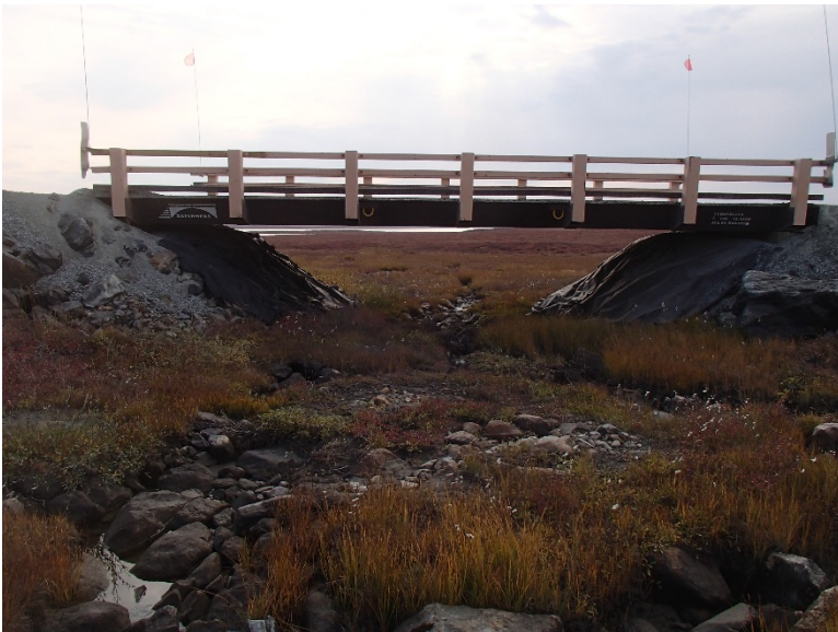
Photograph D2-24 Bridges 7 – R16 km 73+800
