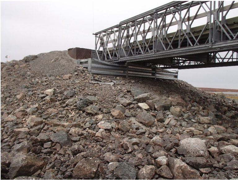
Photograph D2-3 Bridges 1 – R02 km 8+750
