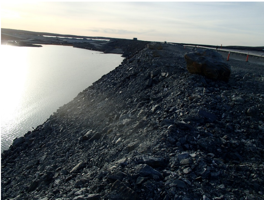
Photograph B7-10 Stormwater Dike
