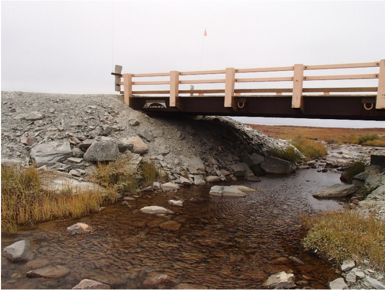
Photograph D2-13 Bridges 4 – R09 km 48+500
