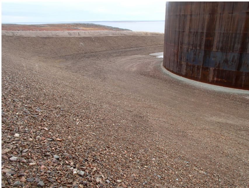
Photograph G1-21 Baker Lake Tank Farm
