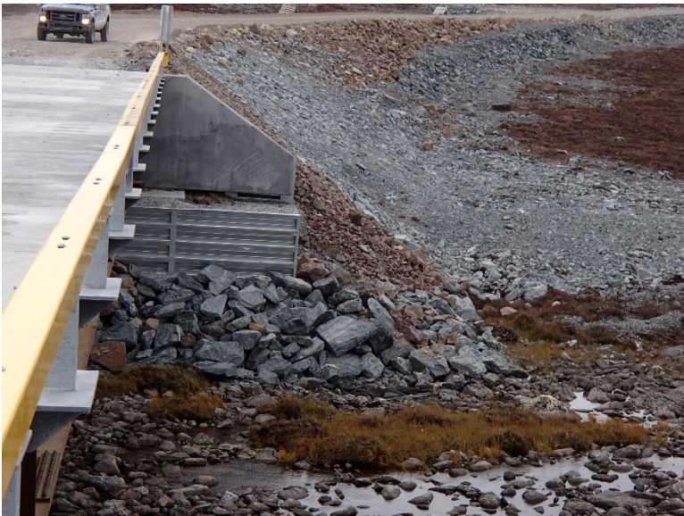
Photograph E2-10 Bridges 3 – km 16+000
