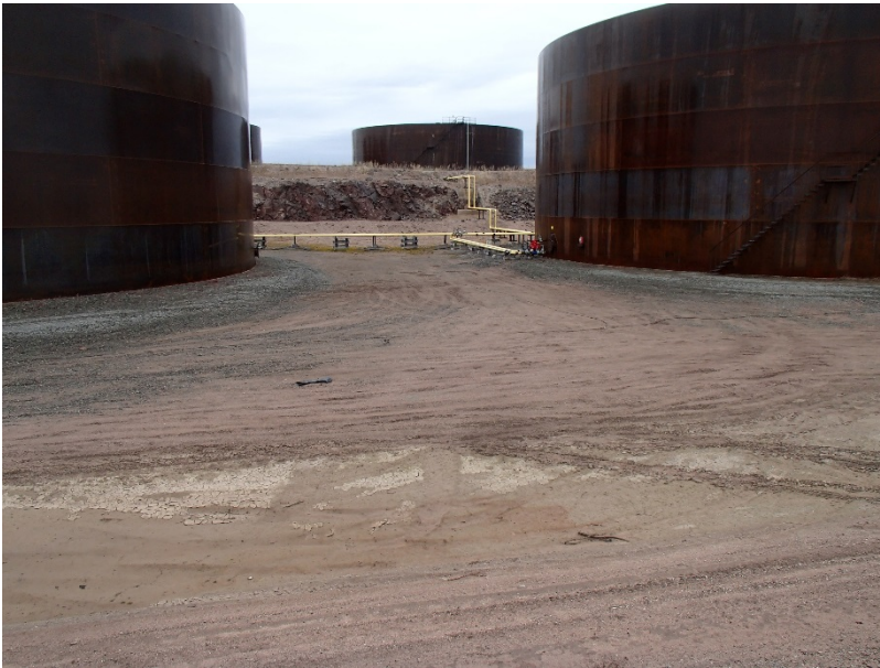
Photograph G1-9 Baker Lake Tank Farm
