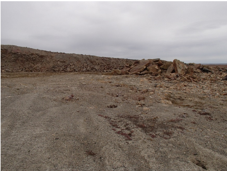
Photograph F1-14: Quarry 7 – km 39+800
