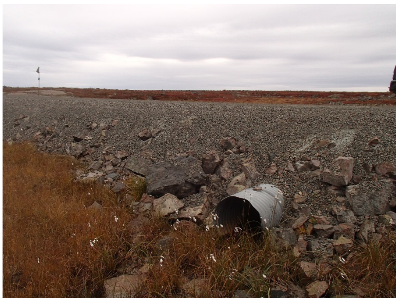
Photograph D1-18: R-03 km 10+580
