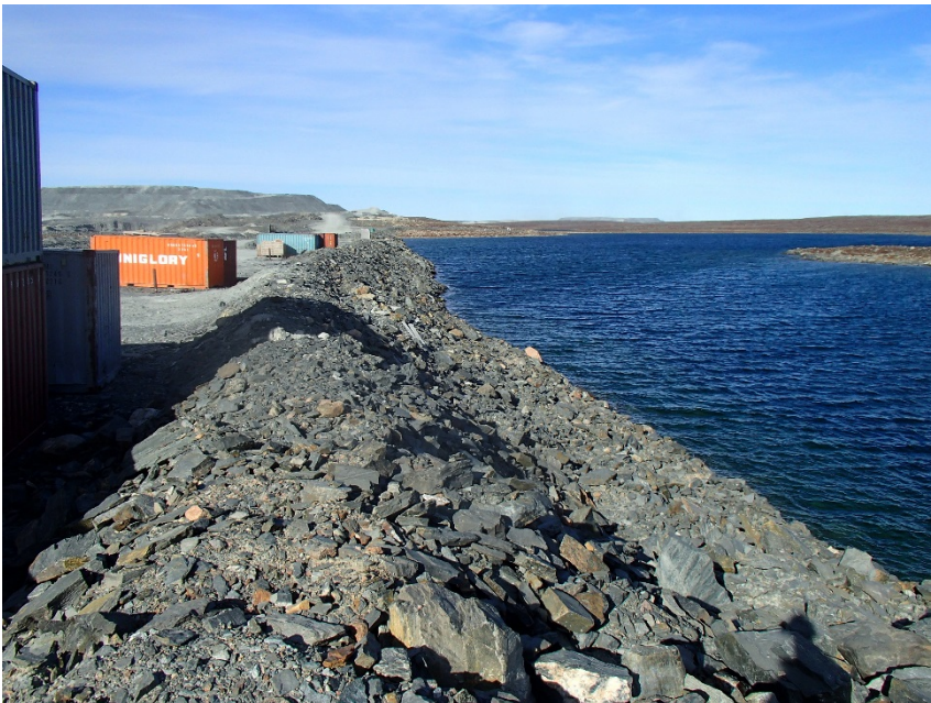
Photograph A1-8 East Dike
