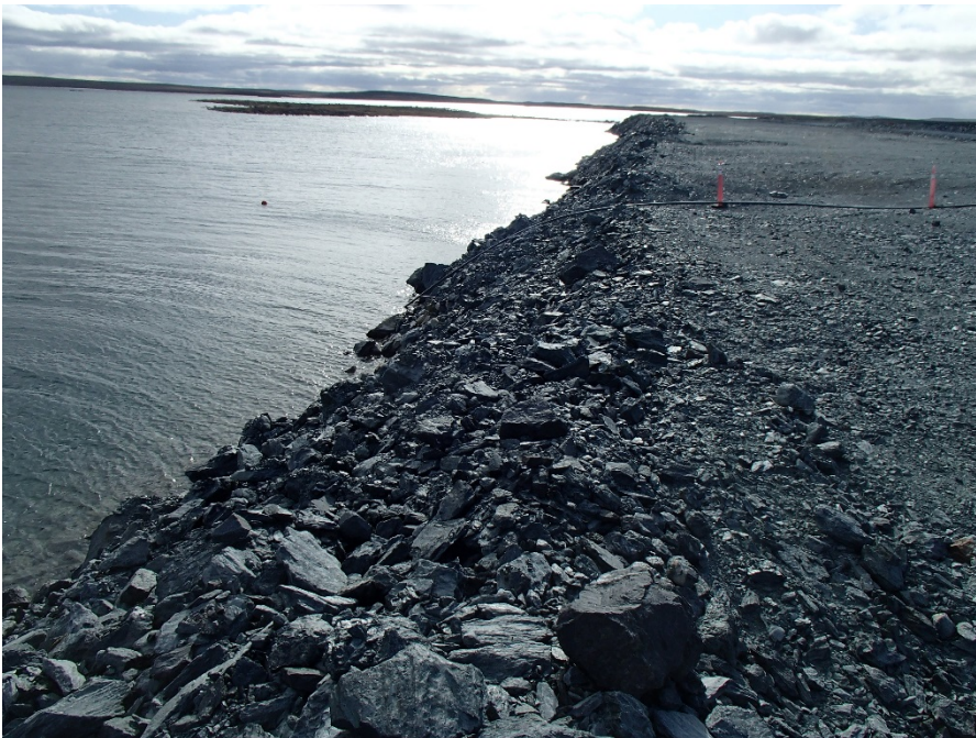
Photograph A3-14 Bay Goose Dike
