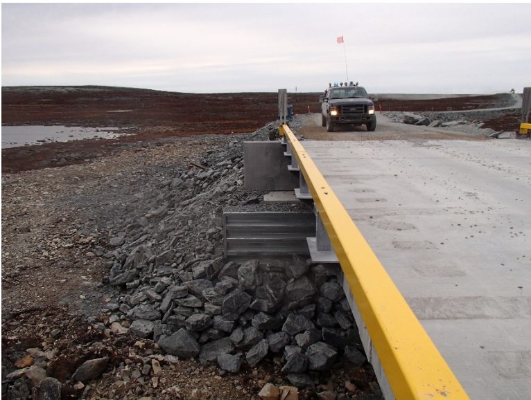
Photograph E2-2 Bridges 1 – km 3+400
