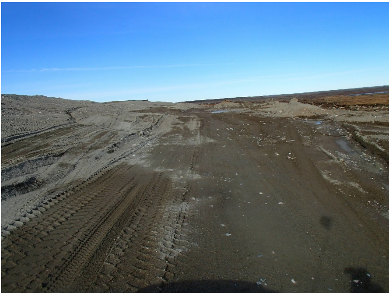
Photograph F2-8 Eskers and Quarries 4 – km 46+000
