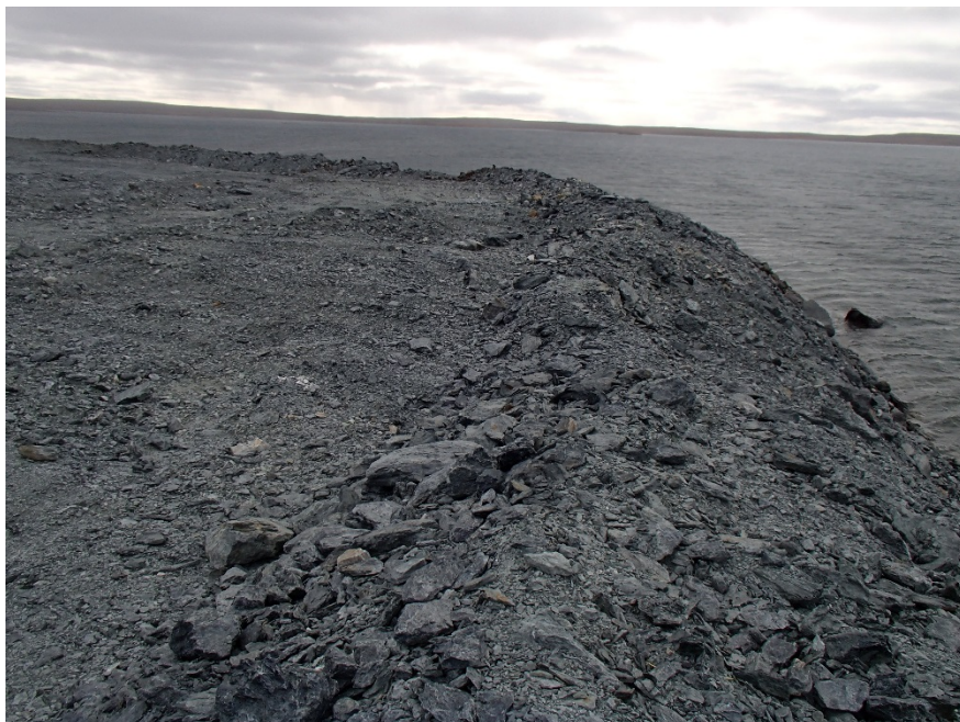
Photograph A3-31 Bay Goose Dike
