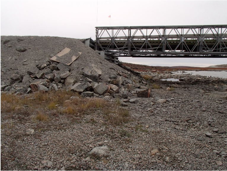
Photograph D2-9 Bridges 3 – R06 km 23+100
