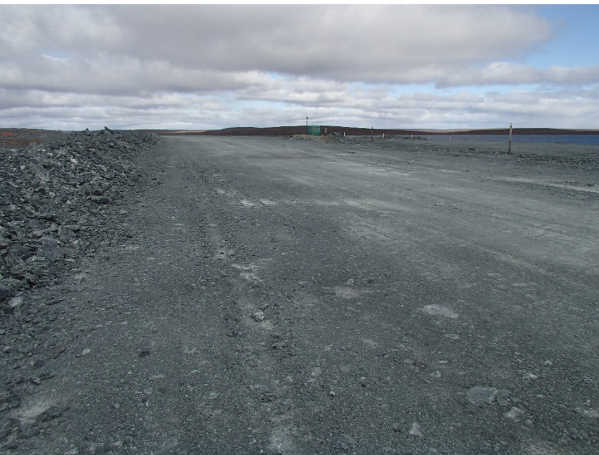
Photograph A3-22 Bay Goose Dike
