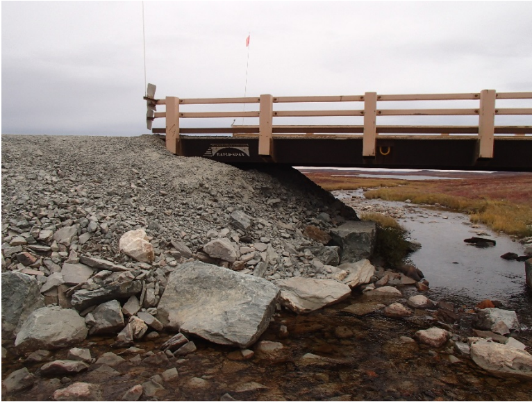
Photograph D2-15 Bridges 4 – R09 km 48+500
