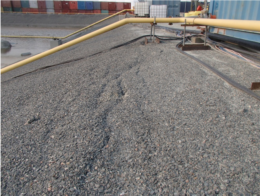
Photograph G2-7 Meadowbank Tank Farm
