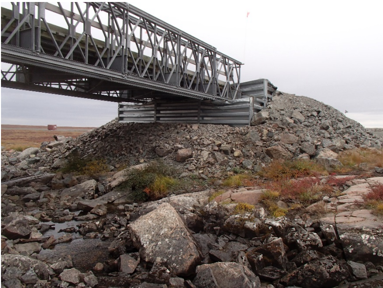
Photograph D2-4 Bridges 1 – R02 km 8+750
