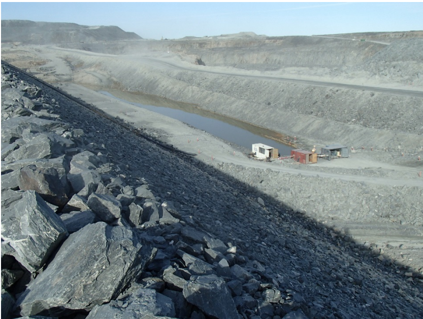
Photograph B7-18 Central Dike and Saddle Dam 5
