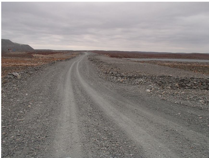
Photograph A4-1 Vault Dike
