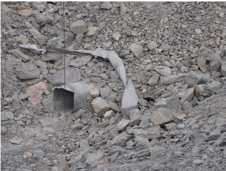
Photograph H1-6 Vault Road Culverts
