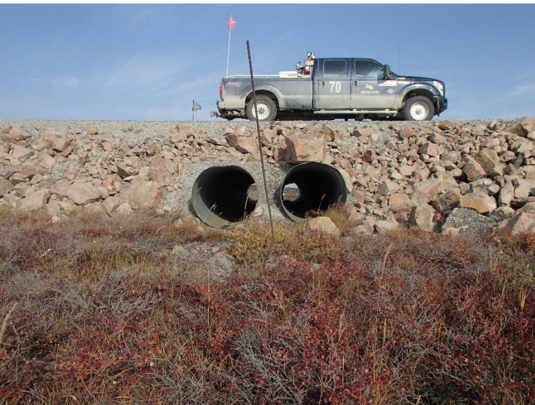
Photograph D1-64: R-21 km 87+300
