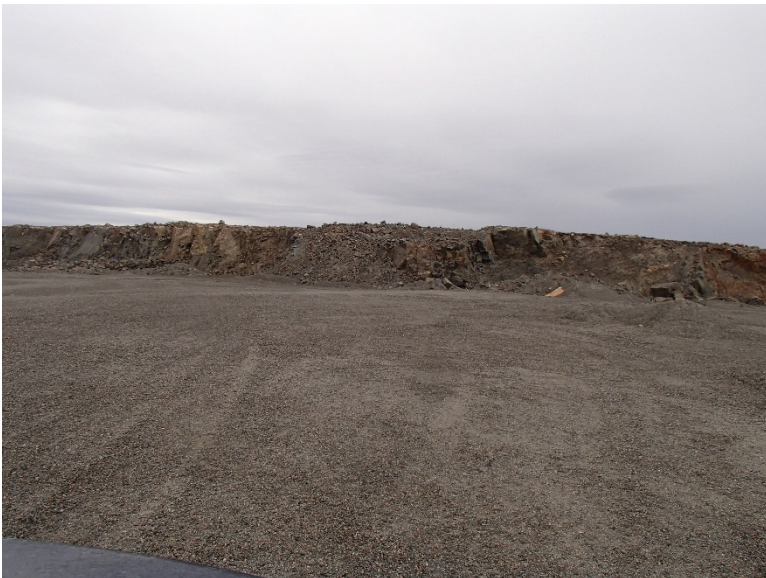
Photograph F1-4: Quarry 2 – km 13+250
