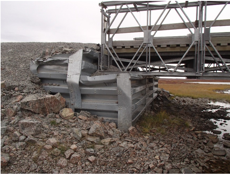
Photograph D2-7 Bridges 2 – R05 km 17+600
