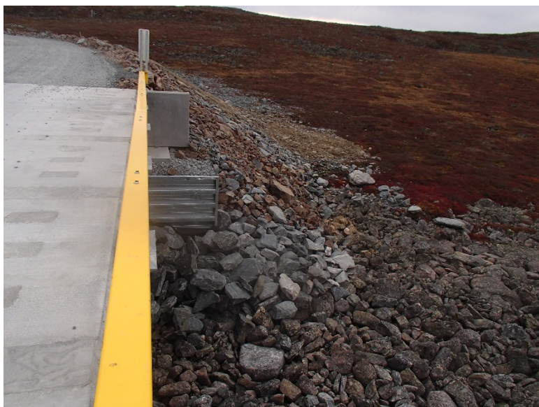
Photograph E2-8 Bridges 2 – km 10+700
