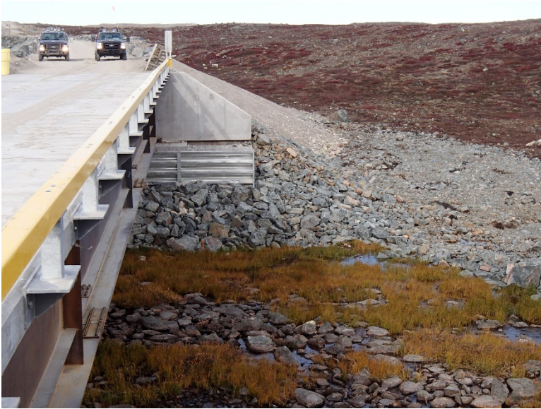
Photograph E2-33 Bridges 9 – km 44+800
