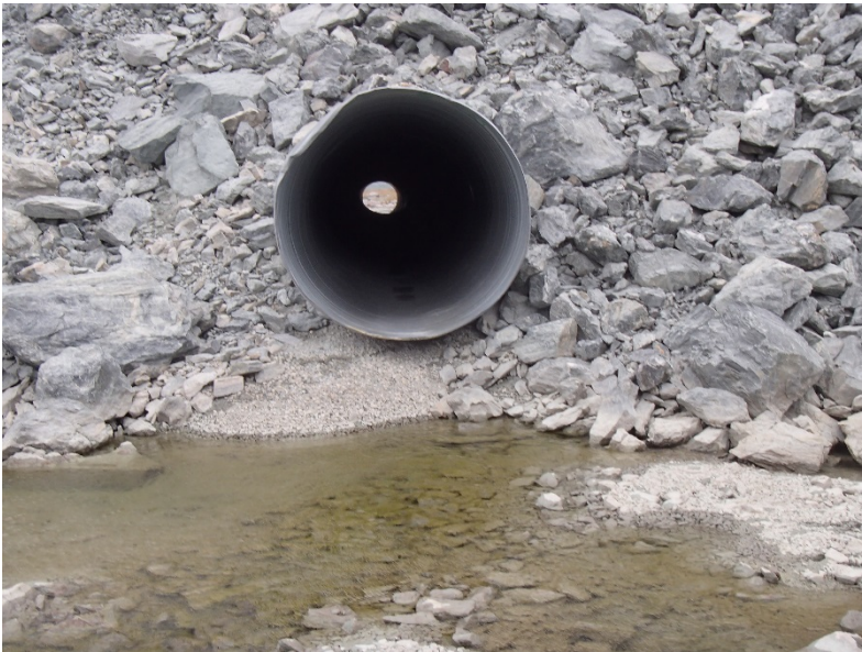
Photograph H1-4 Vault Road Culverts
