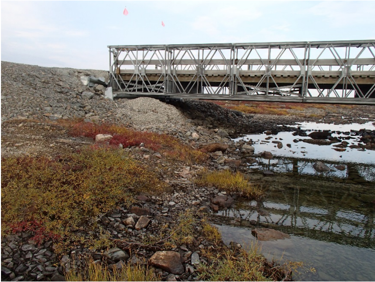
Photograph D2-19 Bridges 6 – R15 km 69+200
