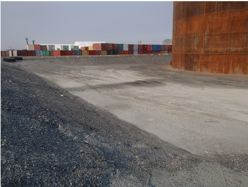
Photograph G2-2 Meadowbank Tank Farm
