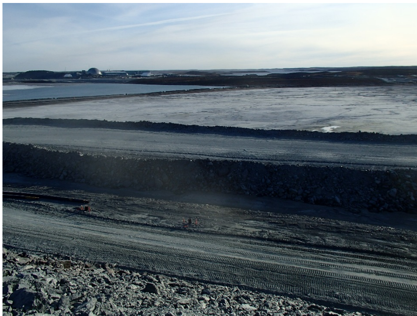
Photograph B1-8 Tailings Storage Facility
