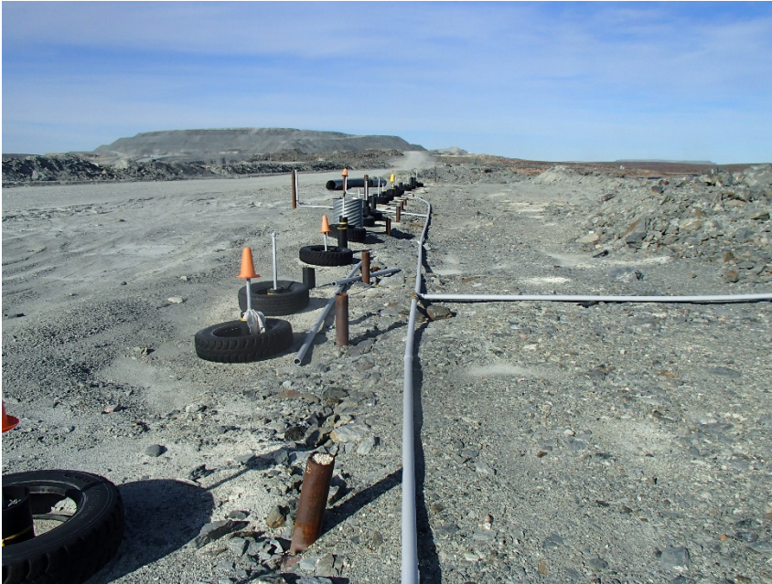
Photograph A1-3 East Dike
