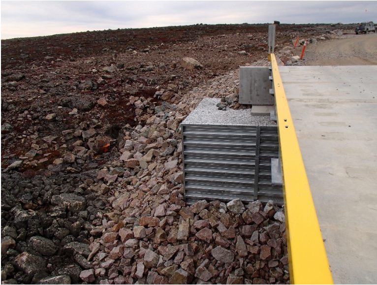
Photograph E2-23 Bridges 6 – km 26+100
