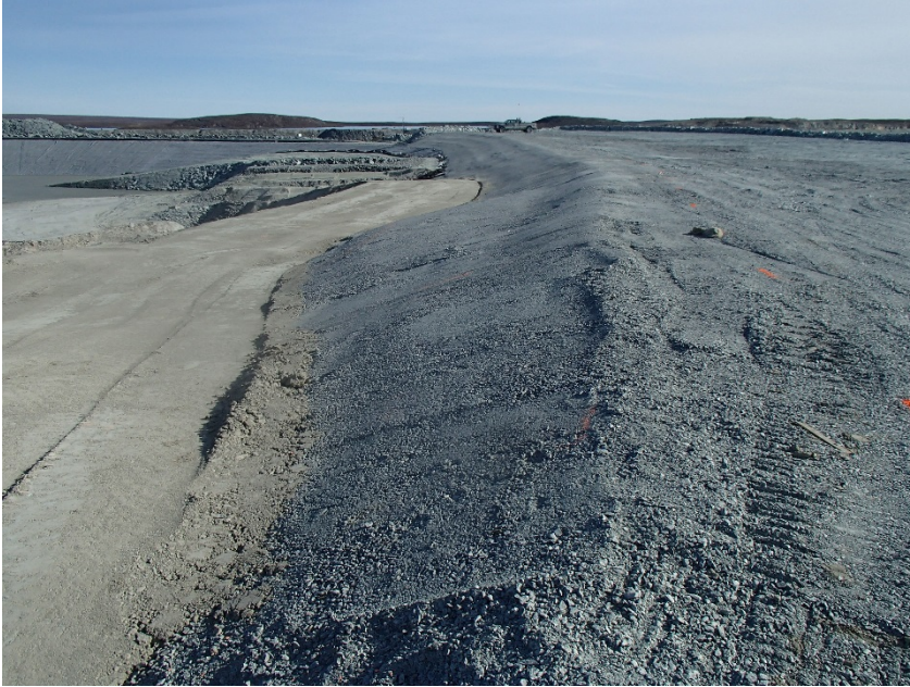
Photograph B7-19 Central Dike and Saddle Dam 5
