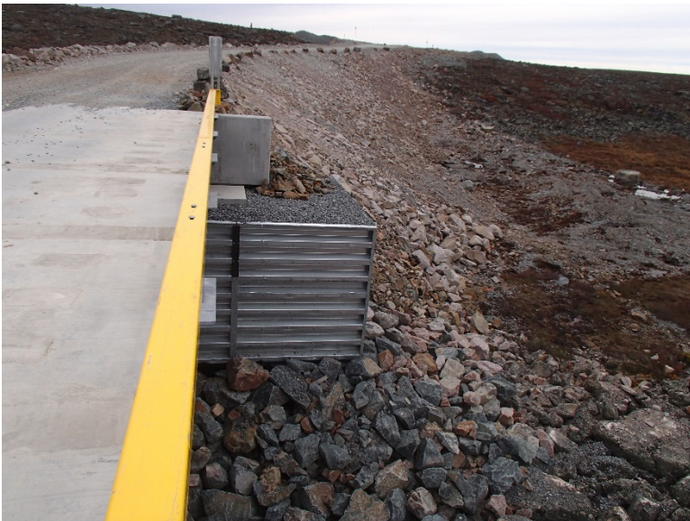
Photograph E2-22 Bridges 6 – km 26+100
