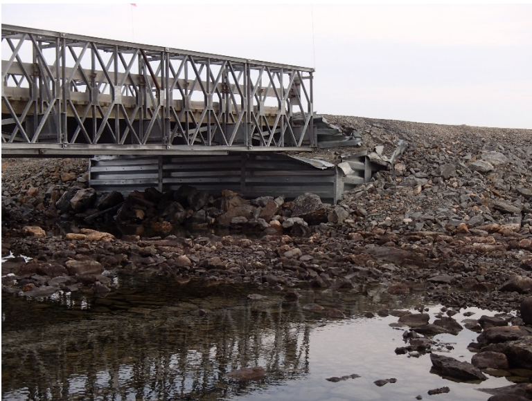
Photograph D2-20 Bridges 6 – R15 km 69+200
