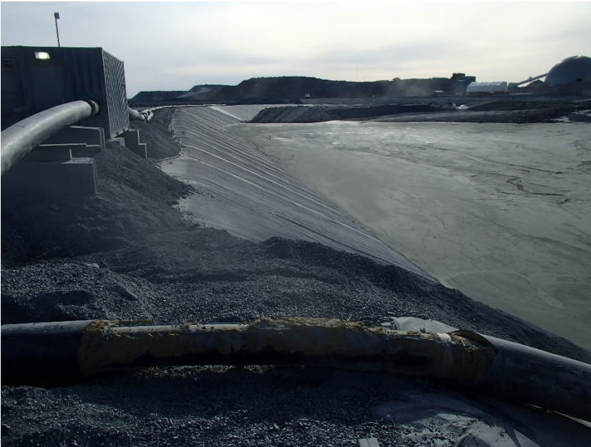
Photograph B7-15 Central Dike and Saddle Dam 5
