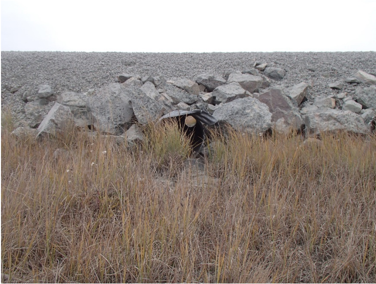
Photograph D1-33: PC-5 km 18+280
