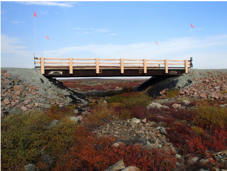
Photograph D2-26 Bridges 8 – R18 km 79+500
