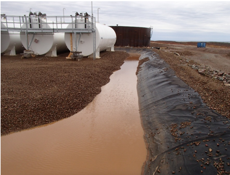
Photograph G1-28 Baker Lake Tank Farm
