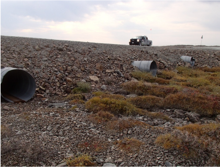
Photograph D1-55: R-14 km 67+840
