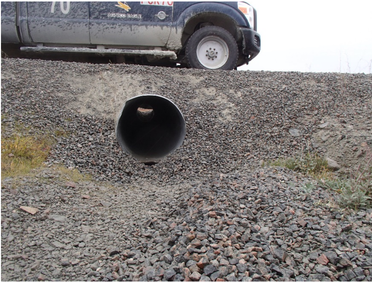
Photograph D1-9: unnamed km 5+700
