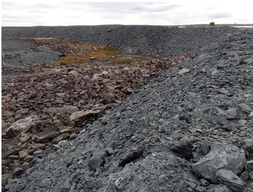
Photograph A3-32 Bay Goose Dike
