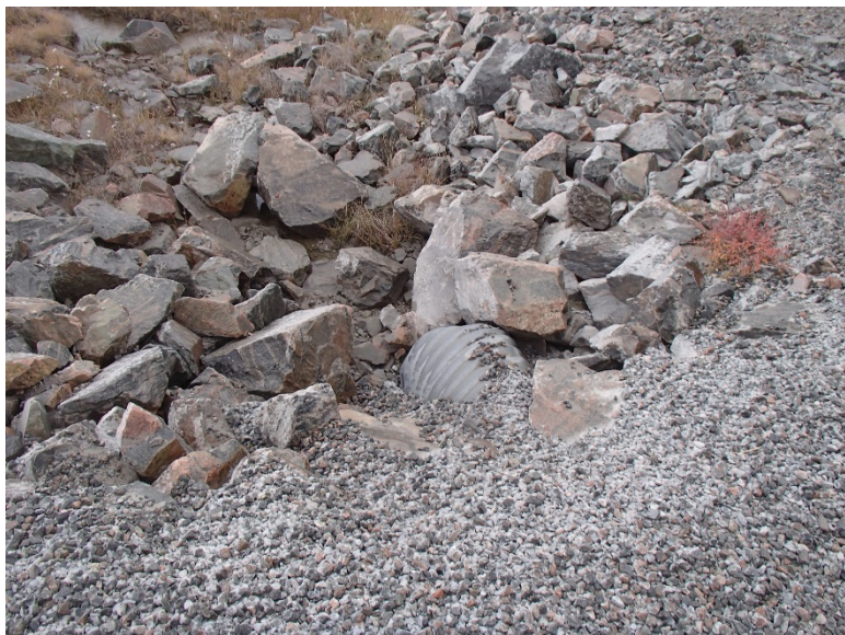
Photograph D1-30: PC-4 km 14+910
