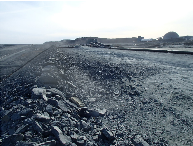
Photograph B7-11 Central Dike and Saddle Dam 5
