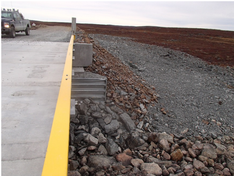
Photograph E2-6 Bridges 2 – km 10+700
