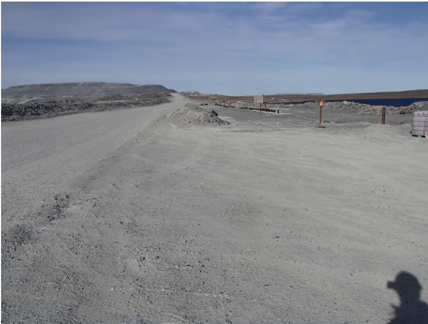
Photograph A1-2 East Dike
