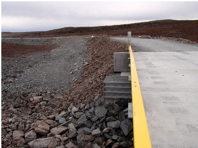
Photograph E2-7 Bridges 2 – km 10+700
