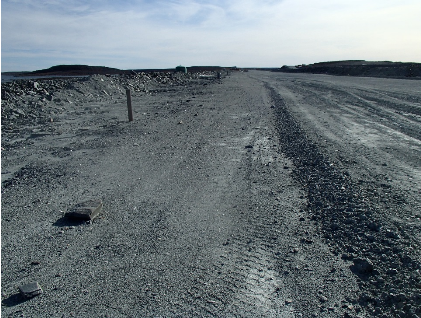
Photograph A1-7 East Dike
