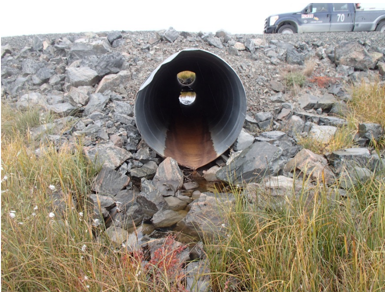
Photograph D1-20: R-04 km 12+050
