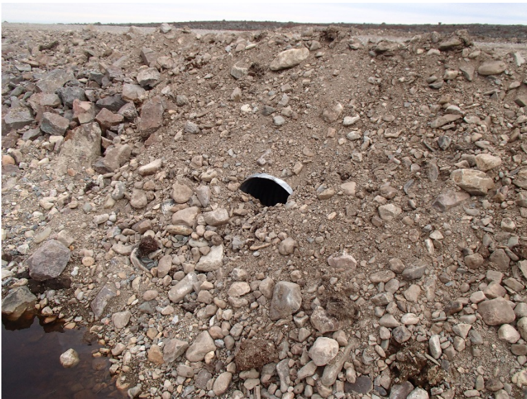
Photograph E1-4: Culvert #86 km 20+740
