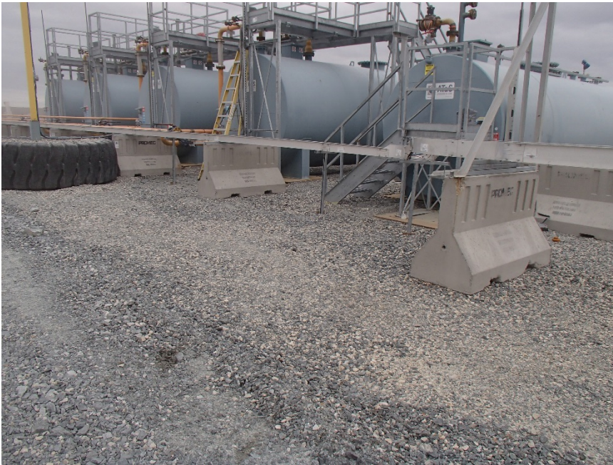
Photograph G3-1 Vault Tank Farm
