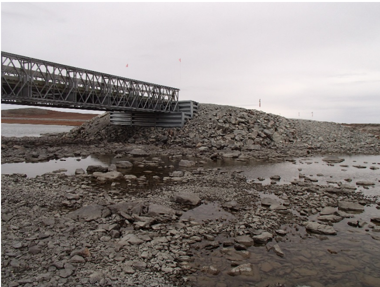
Photograph D2-10 Bridges 3 – R06 km 23+100
