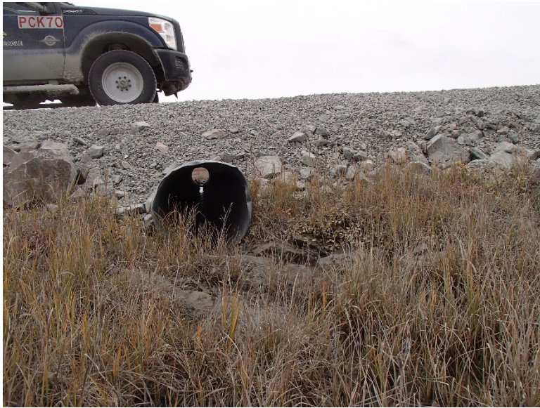
Photograph D1-39: PC-7 km 20+250
