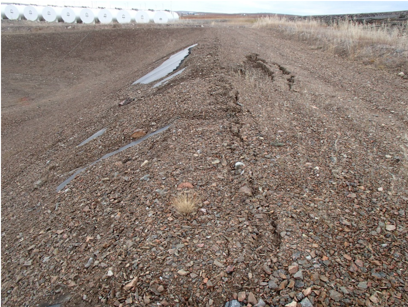
Photograph G1-24 Baker Lake Tank Farm
