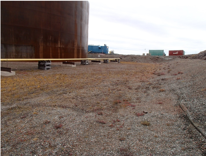
Photograph G1-13 Baker Lake Tank Farm
