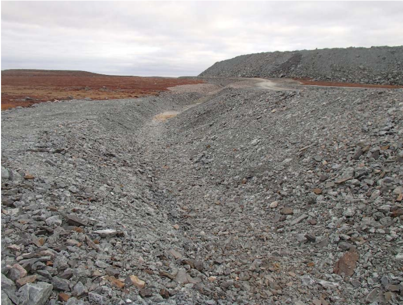
Photograph H2-7 Diversion Ditch and its Sediment and Erosion Protection Structure
