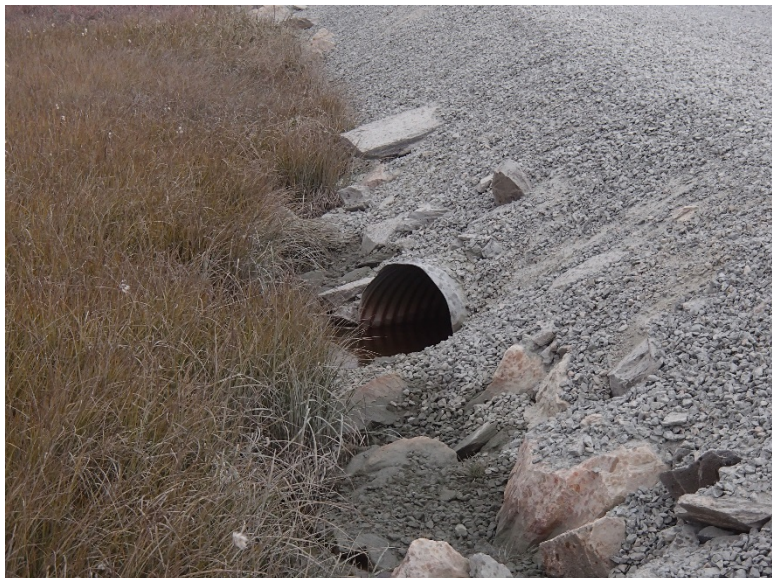
Photograph D1-47: PC-10 km 36+865
