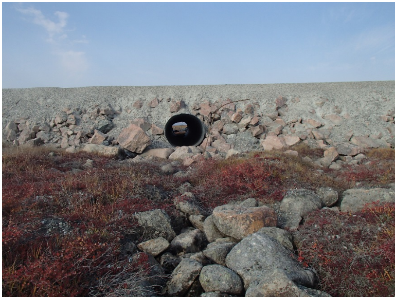
Photograph D1-62: R-20 km 85+490
