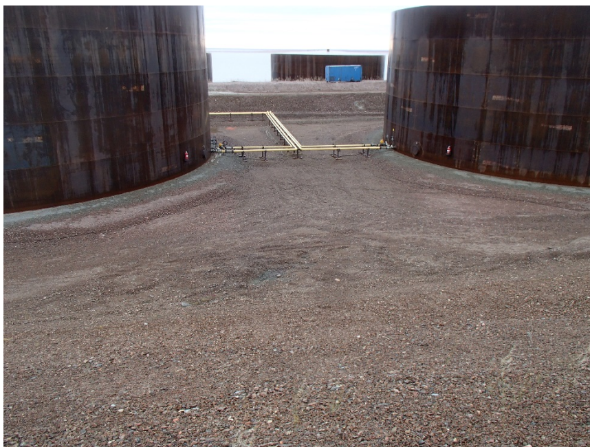
Photograph G1-22 Baker Lake Tank Farm
