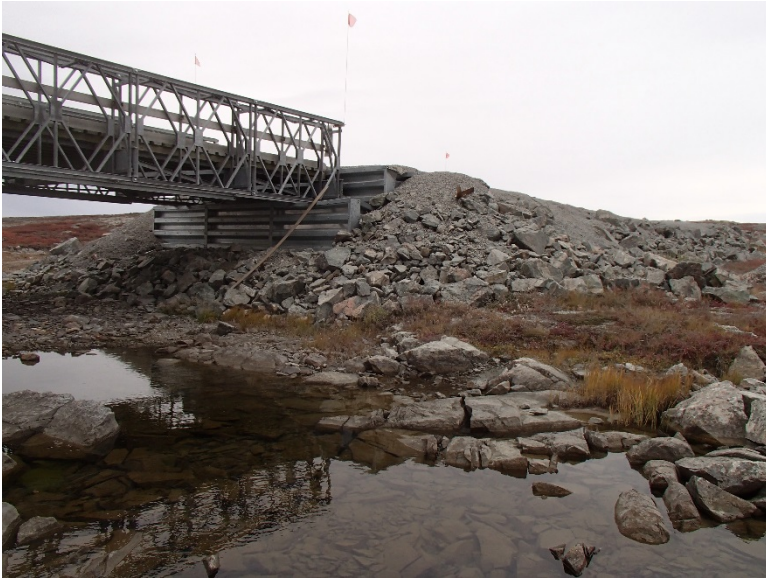
Photograph D2-11 Bridges 3 – R06 km 23+100
