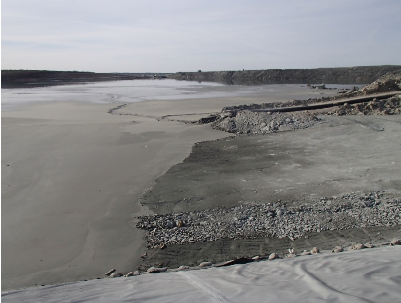
Photograph B1-15 Tailings Storage Facility
