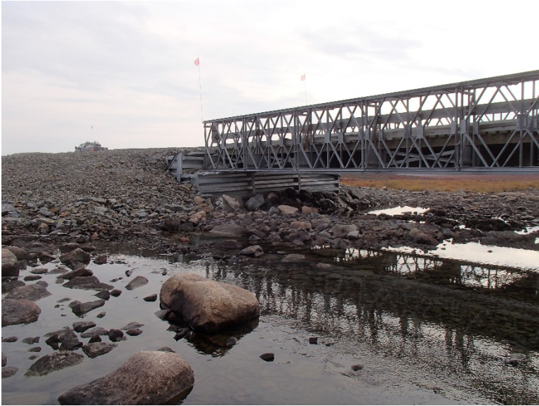
Photograph D2-21 Bridges 6 – R15 km 69+200
