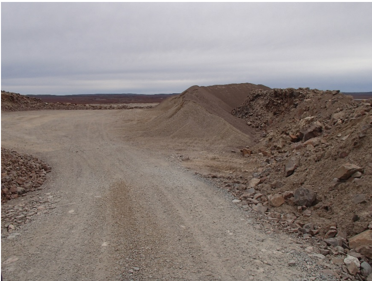
Photograph F2-2 Eskers and Quarries 1 – km 15+000
