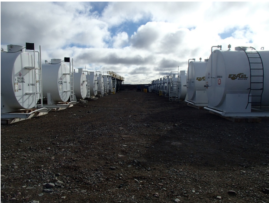
Photograph G4-6 Amaruq Tank Farm
