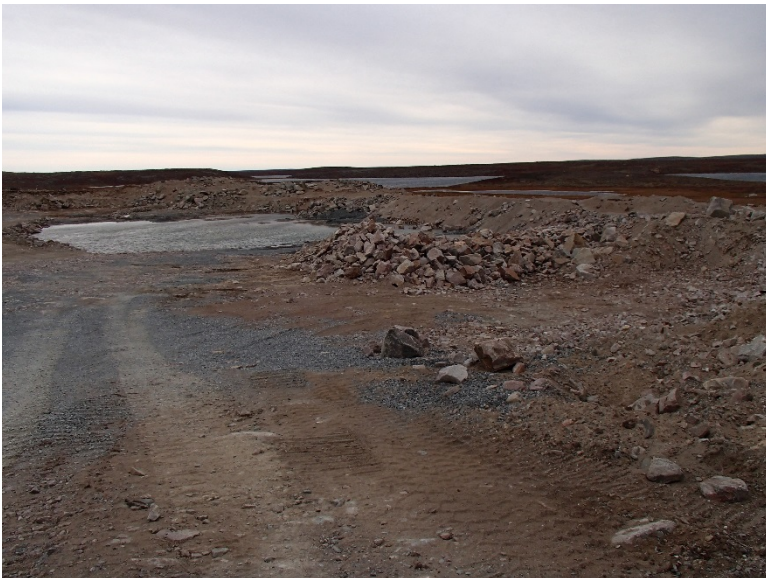
Photograph F2-4 Eskers and Quarries 2 – km 25+000
