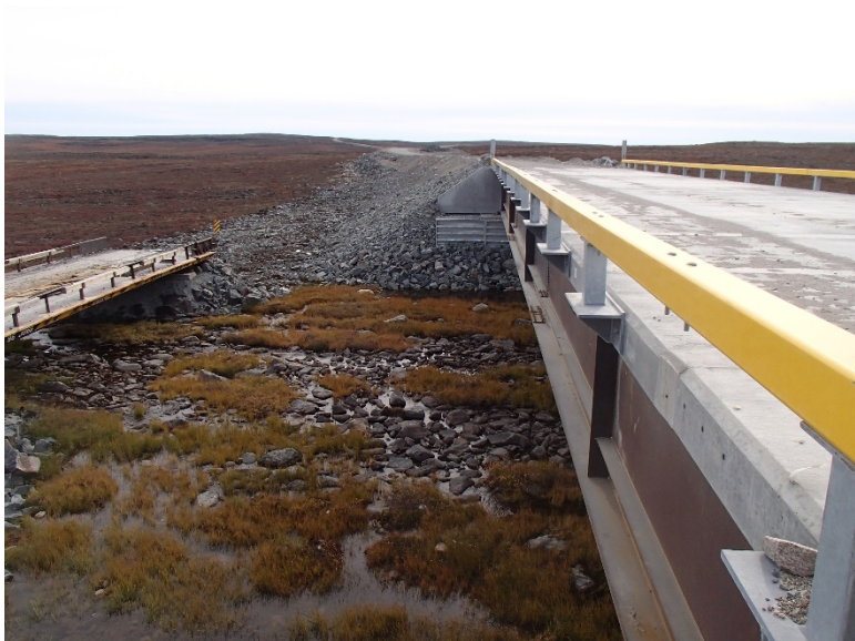
Photograph E2-35 Bridges 9 – km 44+800
