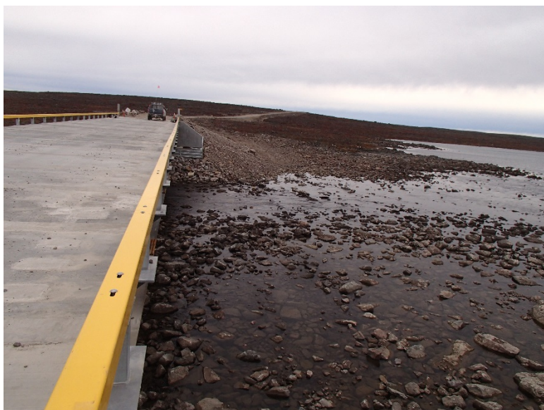
Photograph E2-20 Bridges 5 – km 23+900
