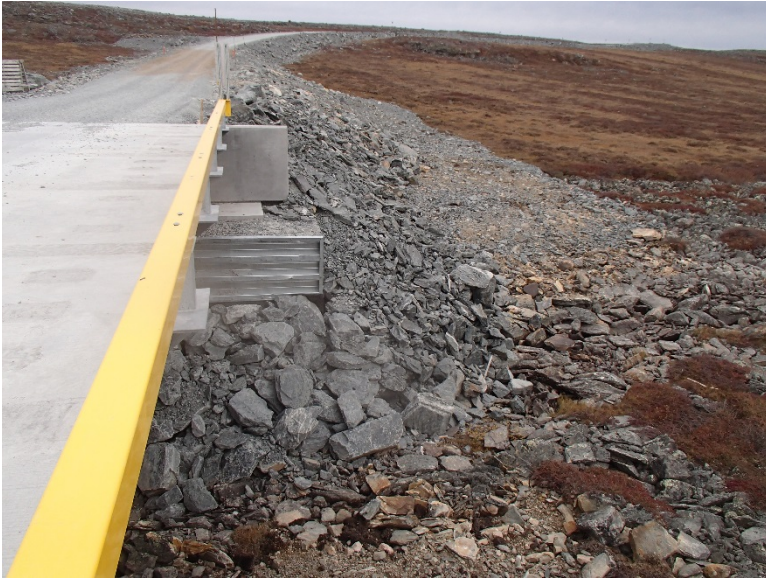
Photograph E2-3 Bridges 1 – km 3+400
