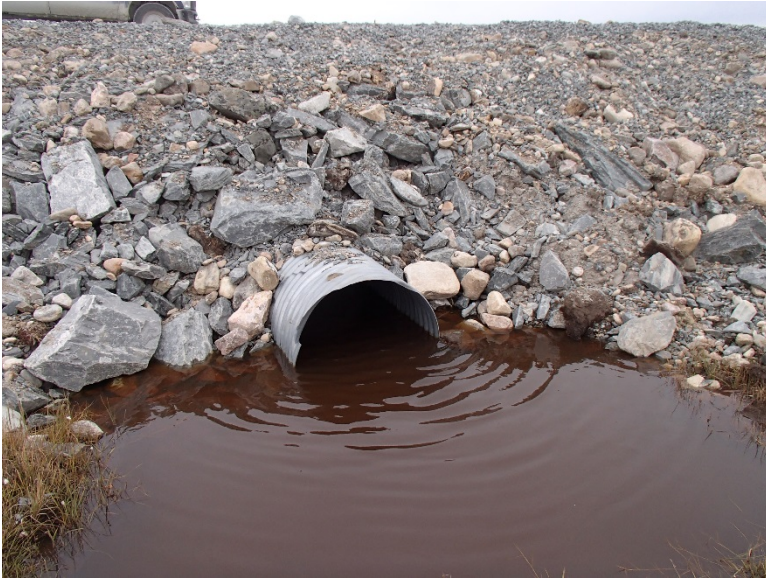
Photograph E1-3: Culvert #60 km 12+775
