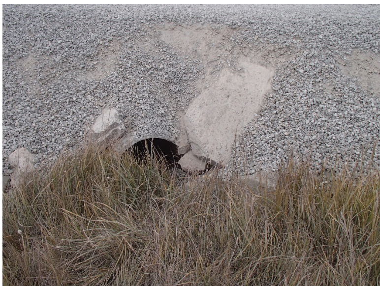
Photograph D1-48: PC-10 km 36+865
