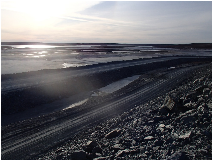
Photograph B1-9 Tailings Storage Facility
