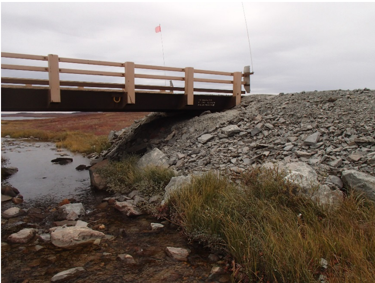
Photograph D2-16 Bridges 4 – R09 km 48+500
