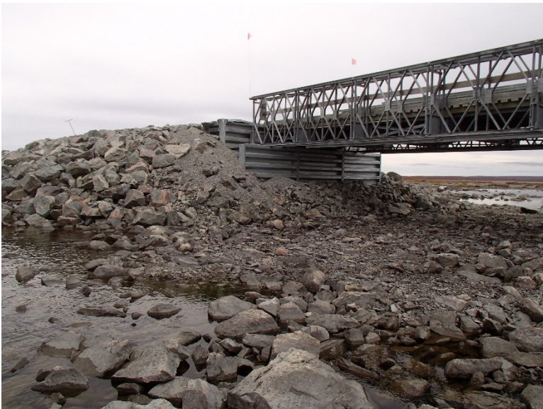
Photograph D2-12 Bridges 3 – R06 km 23+100
