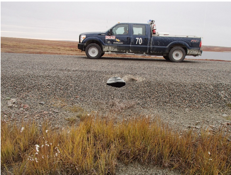
Photograph D1-10: unnamed km 5+700
