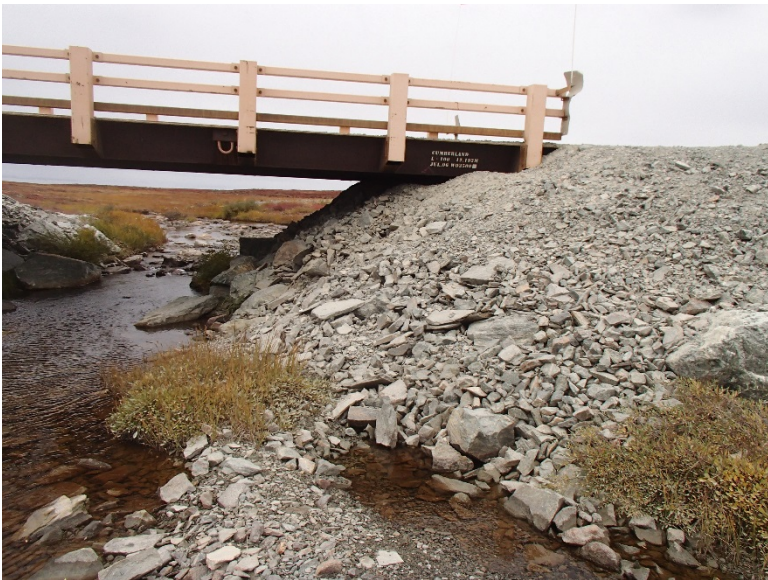
Photograph D2-14 Bridges 4 – R09 km 48+500
