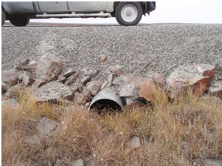
Photograph D1-15: PC-1 km 9+952
