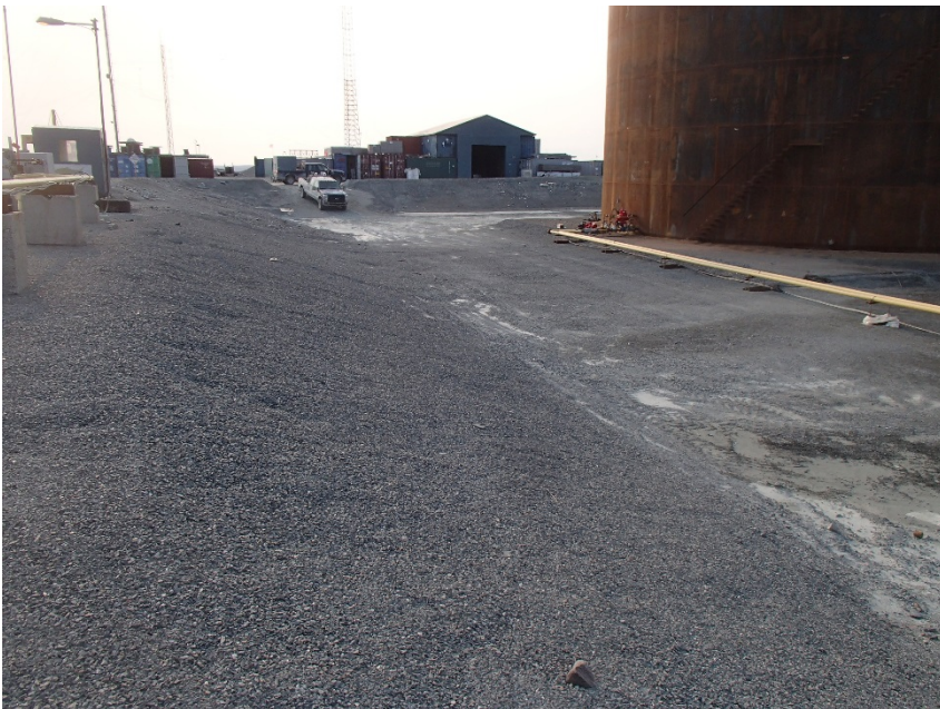
Photograph G2-6 Meadowbank Tank Farm
