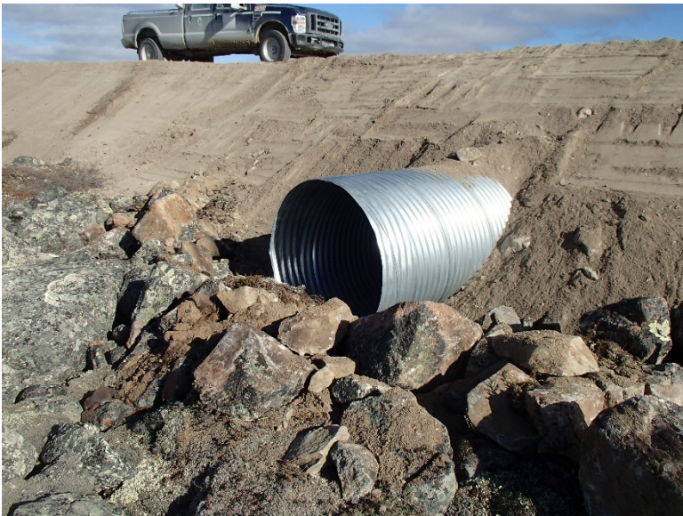
Photograph E1-10: Culvert #278 km 61+870
