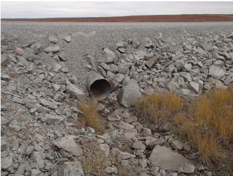
Photograph D1-34: PC-5 km 18+280
