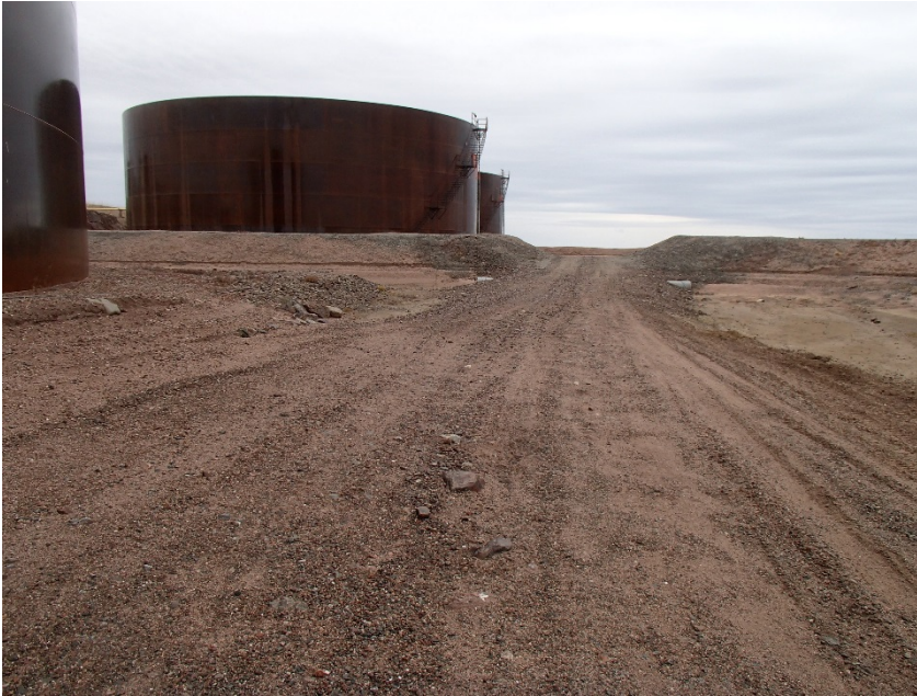
Photograph G1-5 Baker Lake Tank Farm
