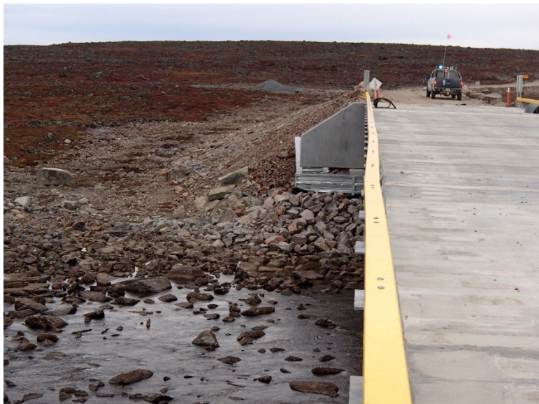
Photograph E2-19 Bridges 5 – km 23+900
