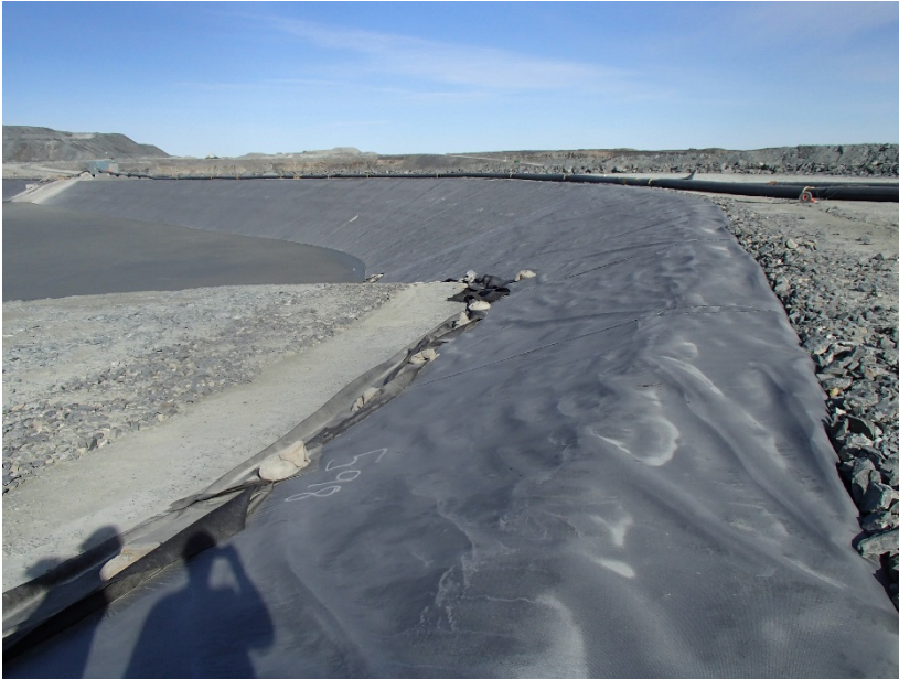
Photograph B1-19 Tailings Storage Facility
