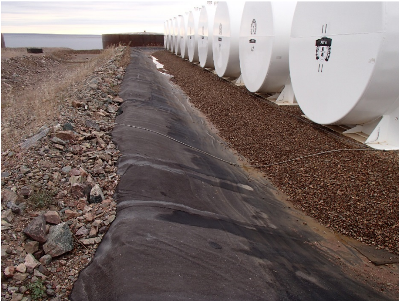
Photograph G1-25 Baker Lake Tank Farm
