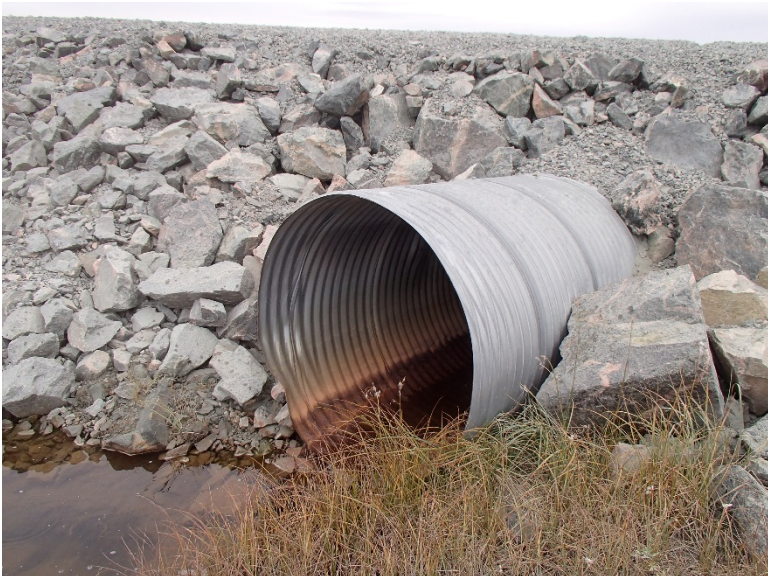
Photograph D1-42: R-07 km 25+900
