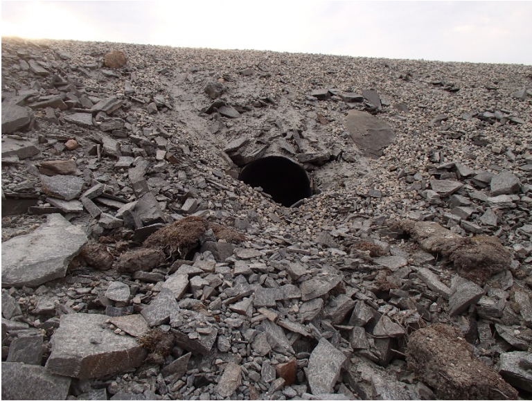
Photograph D1-53: PC-16 km 41+300
