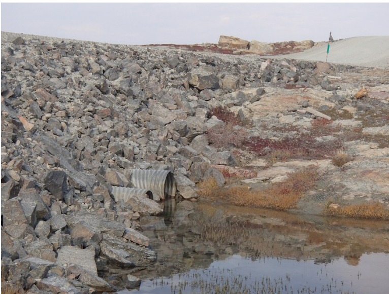
Photograph D1-70: R-25 km 101+950
