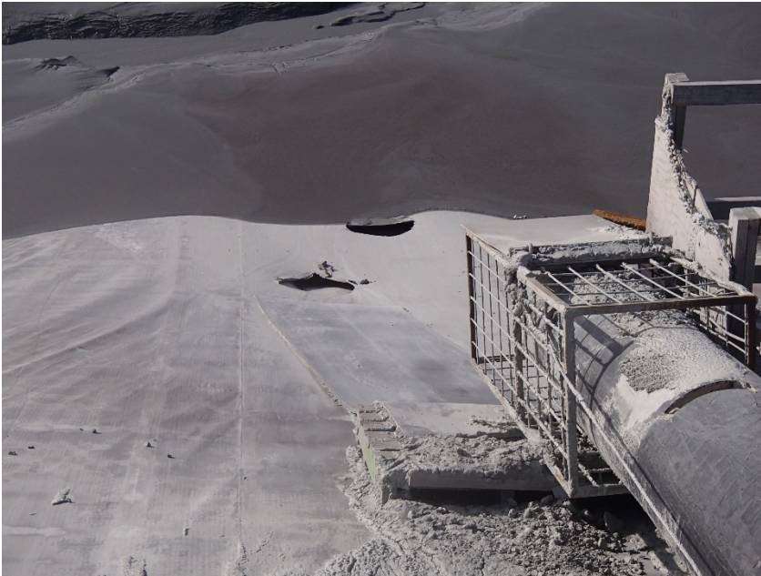
Photograph B7-3 Central Dike and Saddle Dam 5
