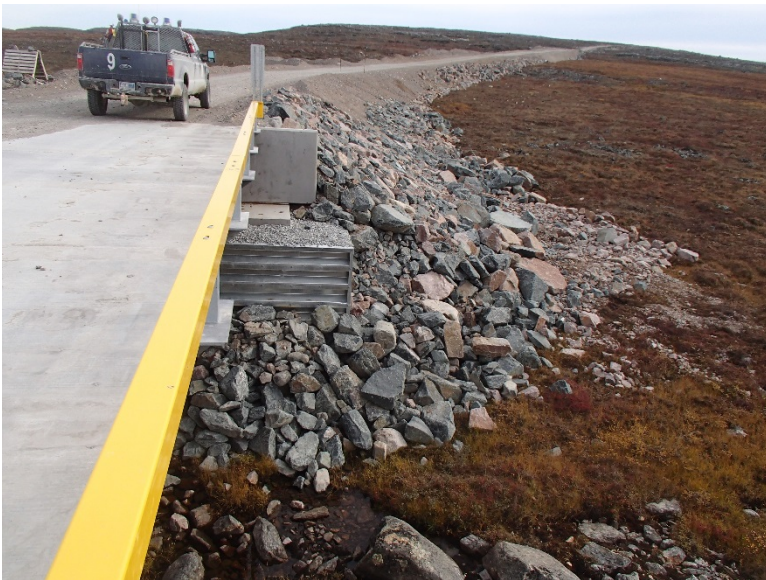
Photograph E2-32 Bridges 8 – km 43+500
