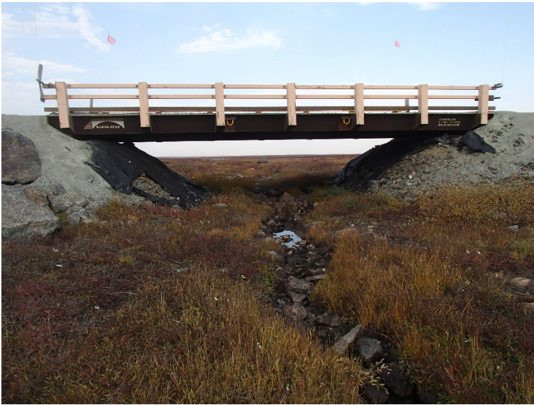
Photograph D2-23 Bridges 7 – R16 km 73+800
