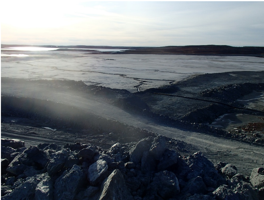
Photograph B1-13 Tailings Storage Facility
