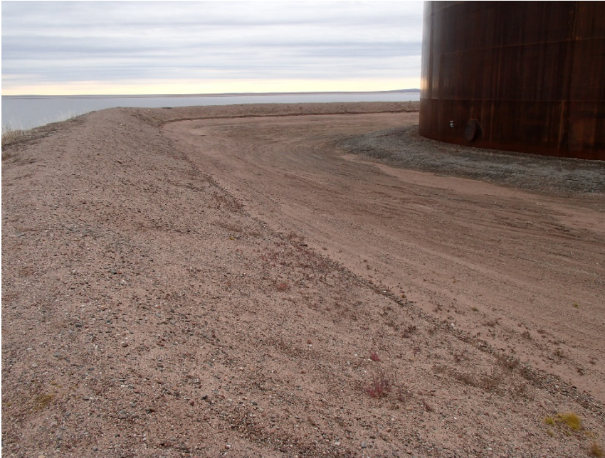
Photograph G1-11 Baker Lake Tank Farm
