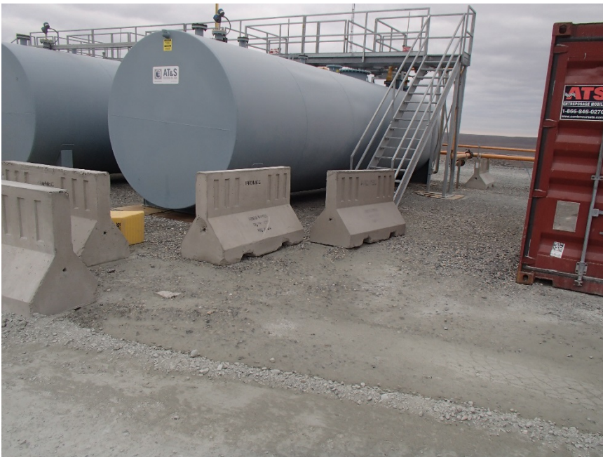
Photograph G3-2 Vault Tank Farm
