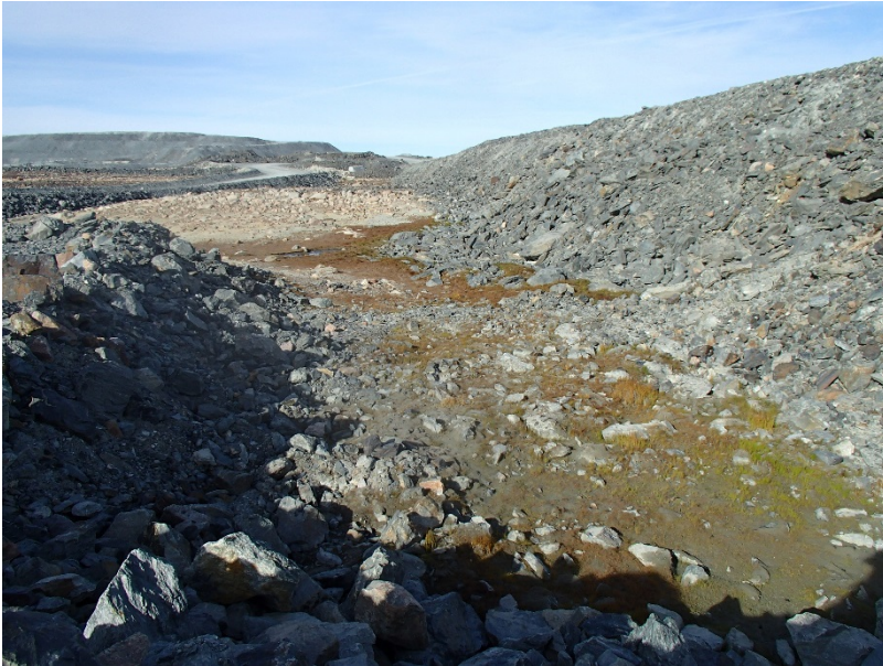
Photograph A1-13 East Dike
