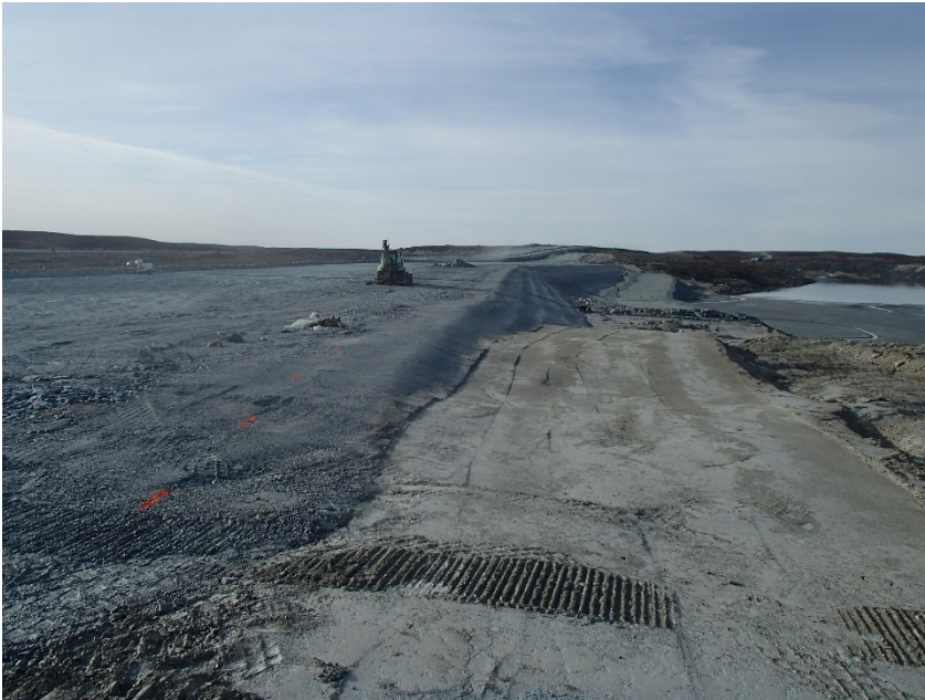
Photograph B6-1 Saddle Dam 4
