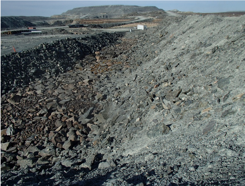
Photograph A1-11 East Dike
