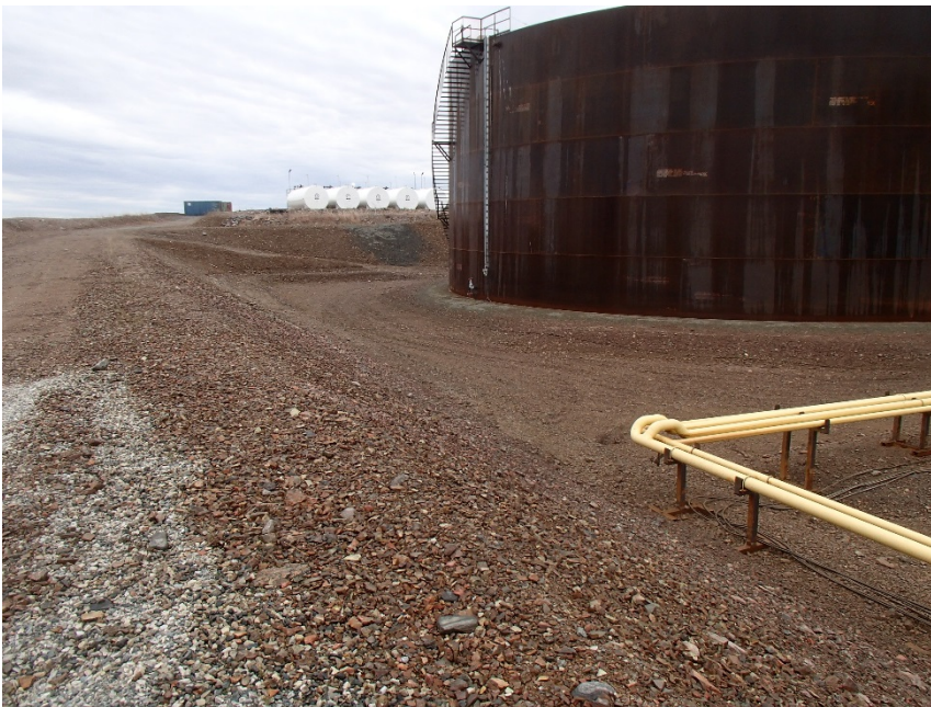
Photograph G1-18 Baker Lake Tank Farm
