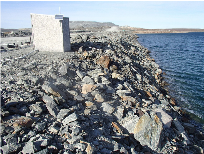
Photograph A1-6 East Dike
