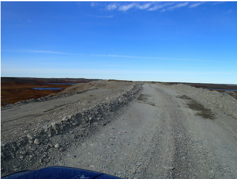
Photograph F2-10 Eskers and Quarries 4 – km 46+000
