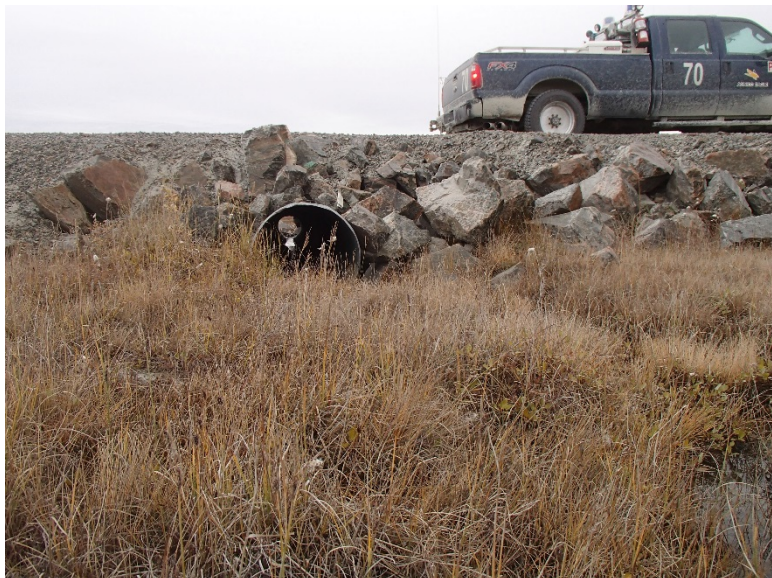
Photograph D1-29: PC-4 km 14+910
