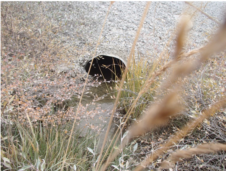
Photograph D1-50: PC-11 km 39+552
