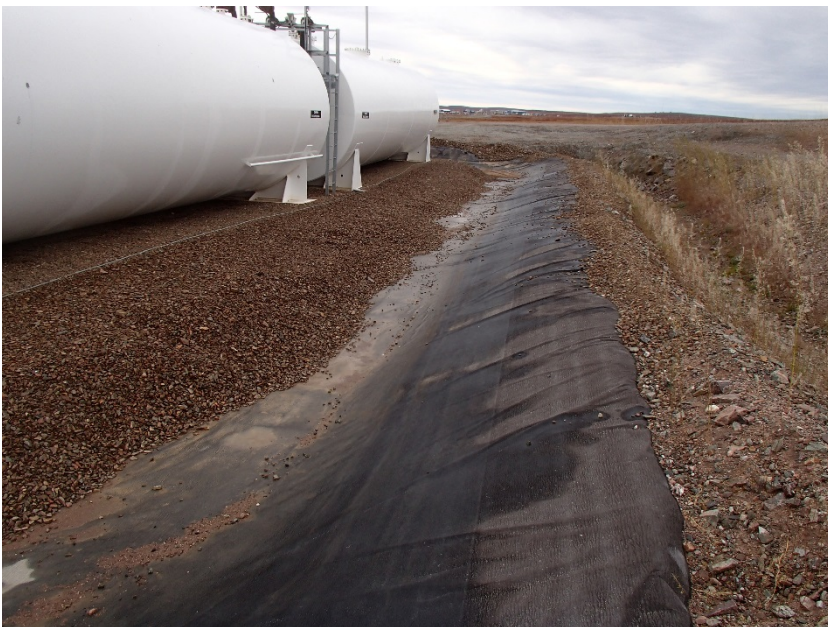
Photograph G1-26 Baker Lake Tank Farm
