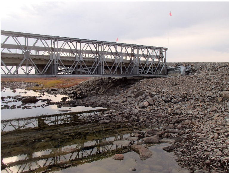
Photograph D2-22 Bridges 6 – R15 km 69+200
