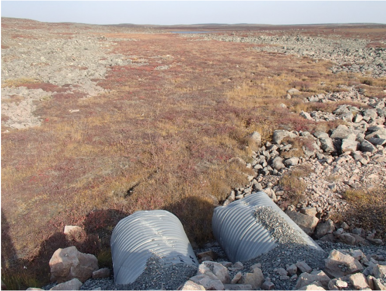
Photograph D1-65: R-21 km 87+300
