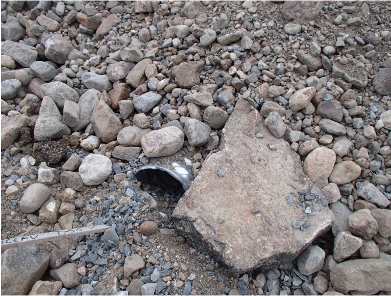
Photograph E1-5: Culvert #115 km 26+865
