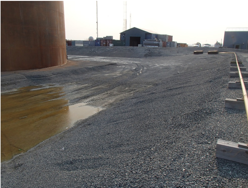
Photograph G2-3 Meadowbank Tank Farm
