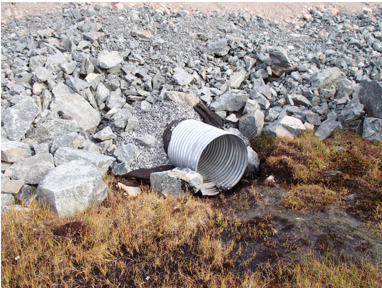
Photograph E1-6: Culvert #167 km 41+843
