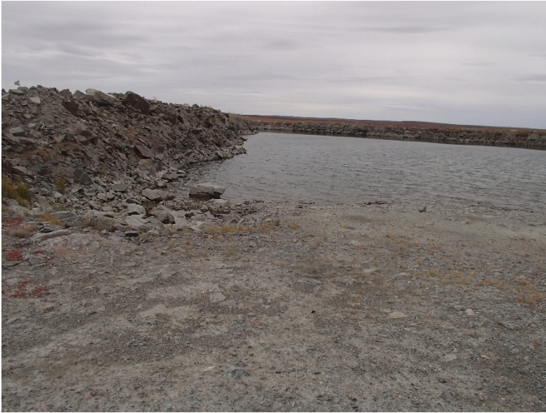
Photograph F1-7: Quarry 4 – km 31+300
