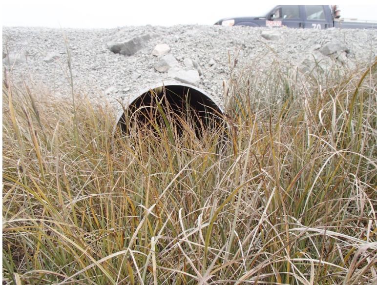
Photograph D1-44: PC-8 km 29+420
