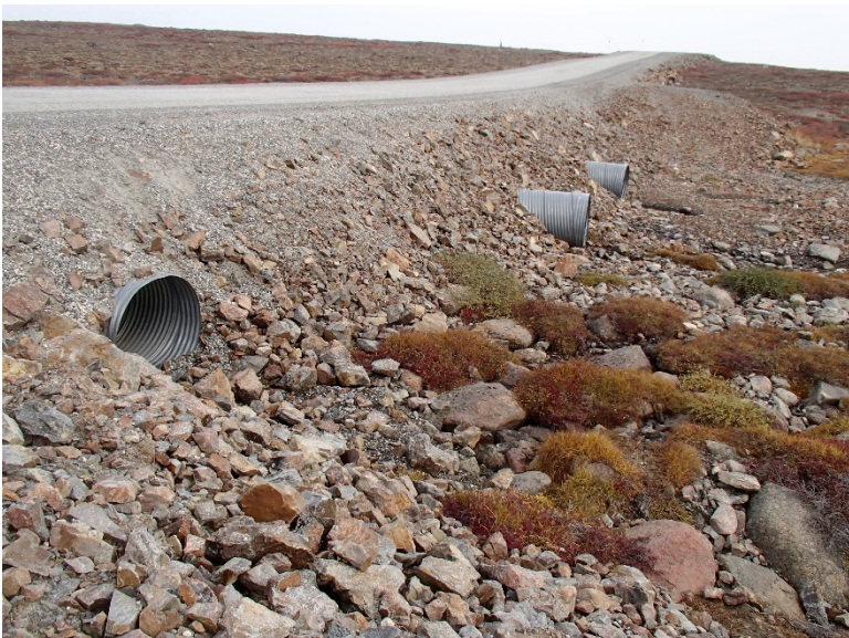
Photograph D1-54: R-14 km 67+840
