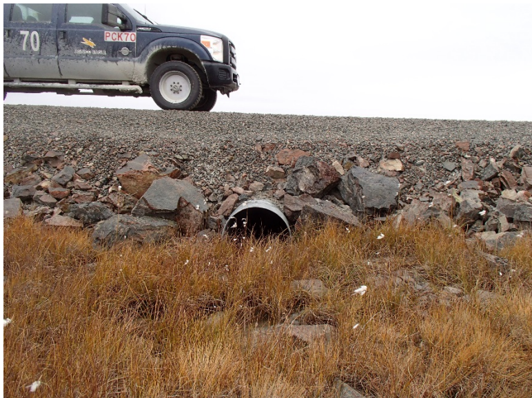
Photograph D1-17: R-03 km 10+580
