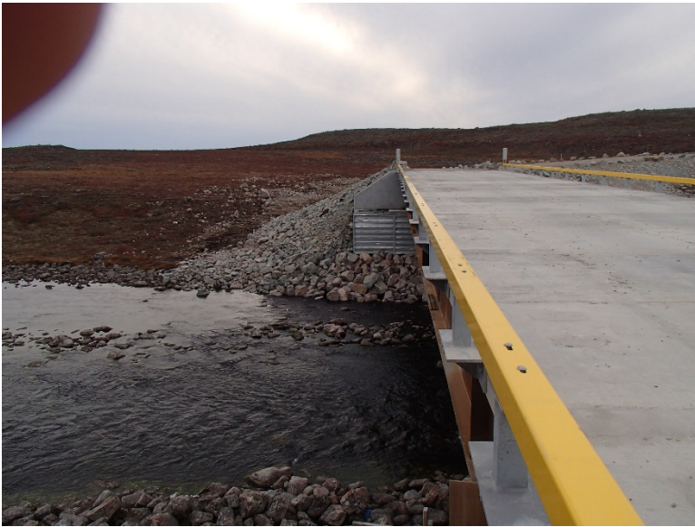
Photograph E2-25 Bridges 7 – km 32+300
