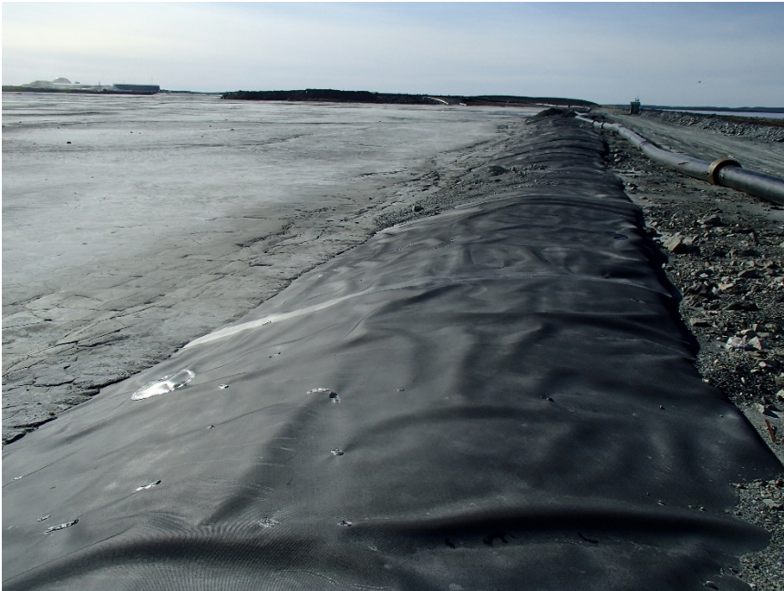
Photograph B1-2 Tailings Storage Facility
