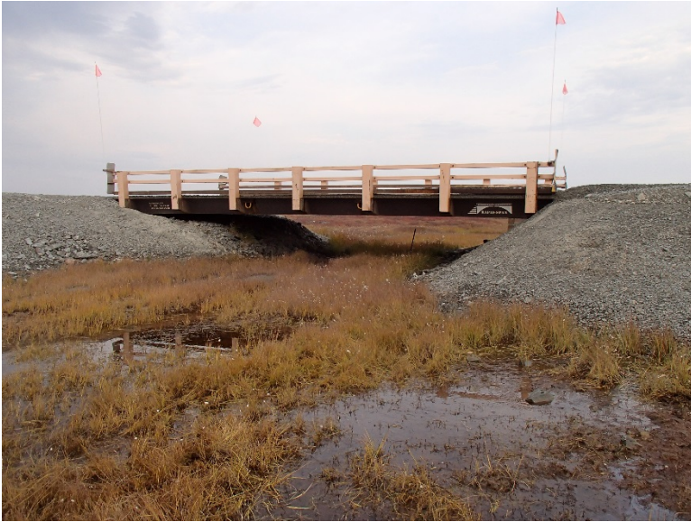
Photograph D2-17 Bridges 5 – R13 km 62+060
