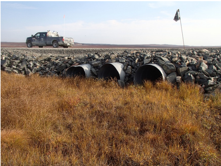
Photograph D1-58: R-18A km 80+950
