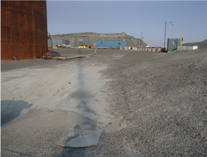
Photograph G2-1 Meadowbank Tank Farm
