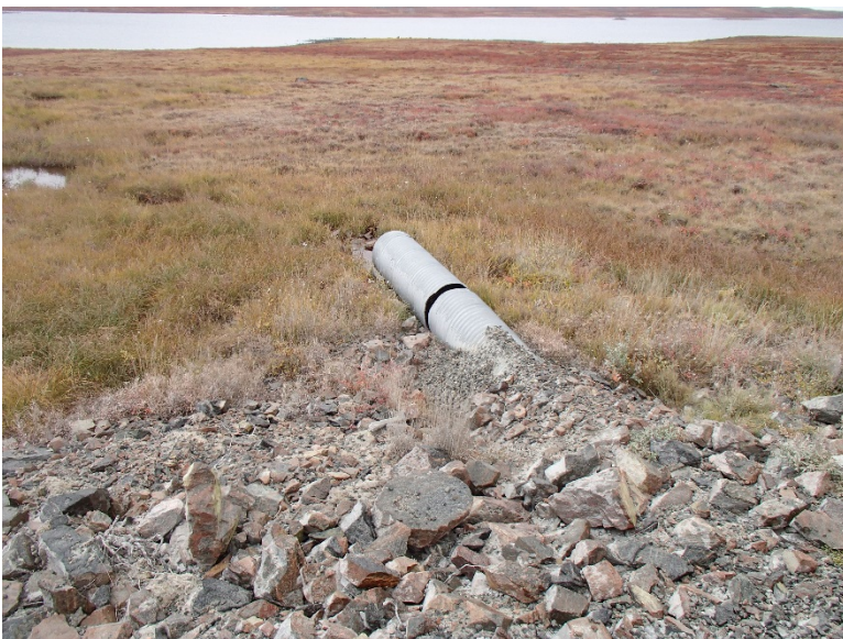
Photograph D1-26: PC-3 km 13+685
