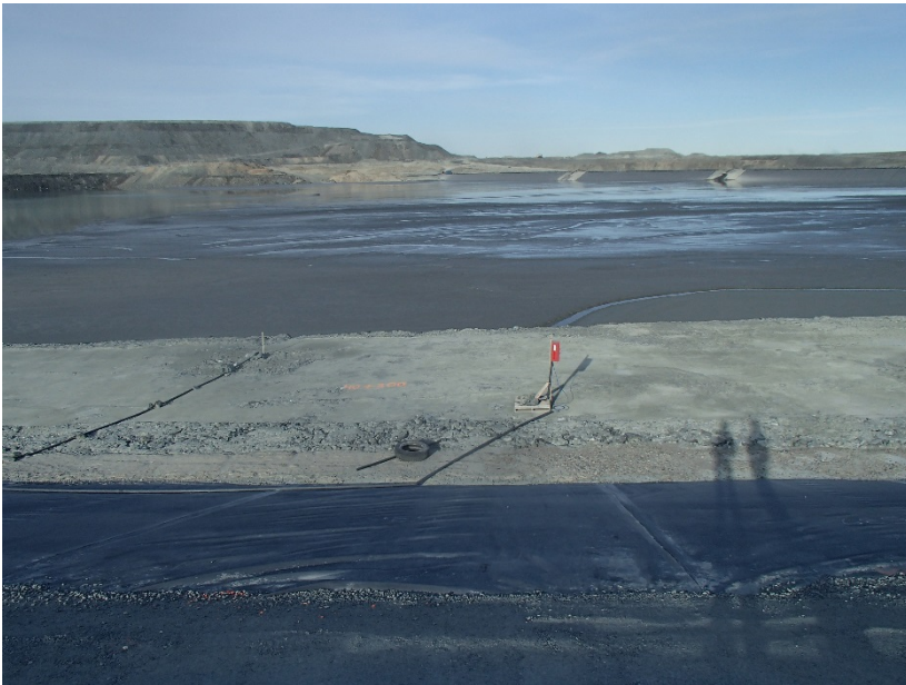
Photograph B1-20 Tailings Storage Facility
