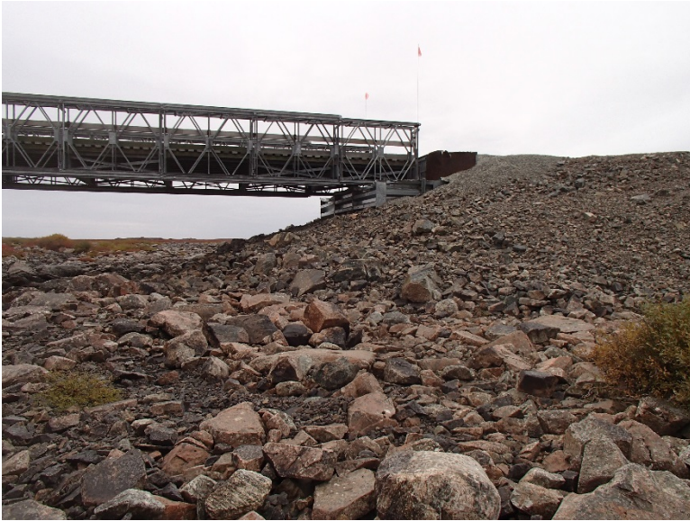
Photograph D2-1 Bridges 1 – R02 km 8+750
