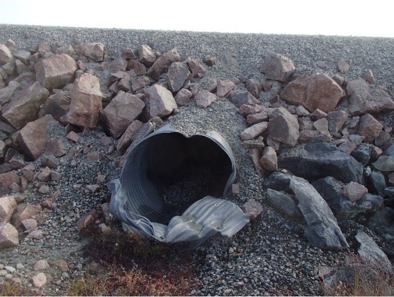
Photograph D1-63: R-20 km 85+490
