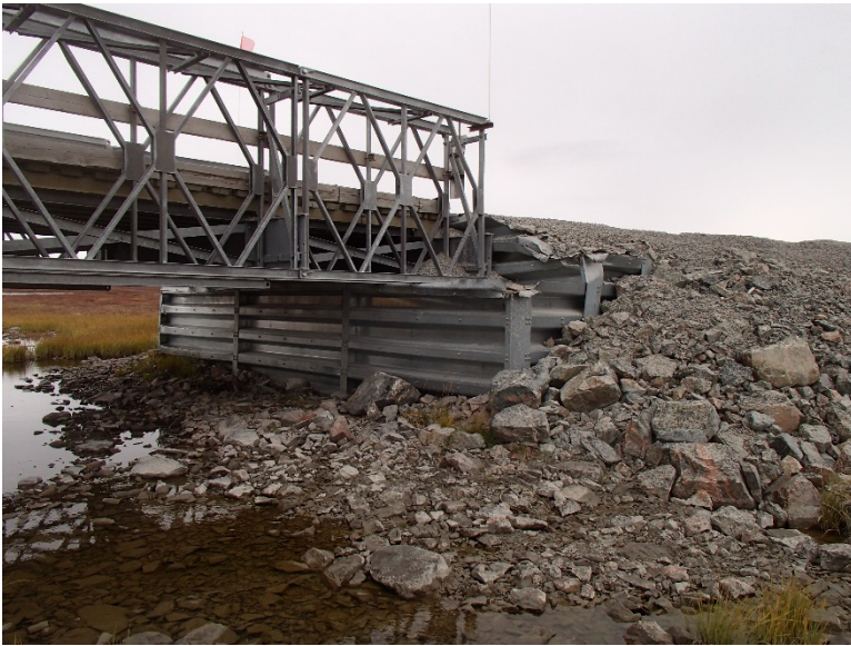
Photograph D2-5 Bridges 2 – R05 km 17+600
