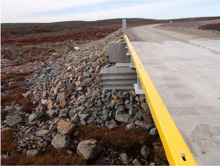
Photograph E2-29 Bridges 8 – km 43+500
