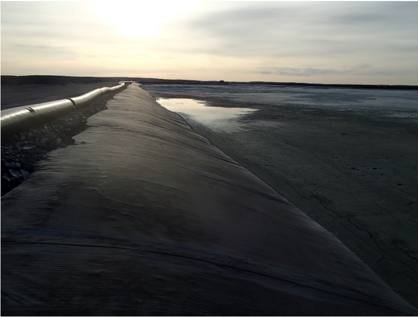
Photograph B4-1 Stormwater Dike
