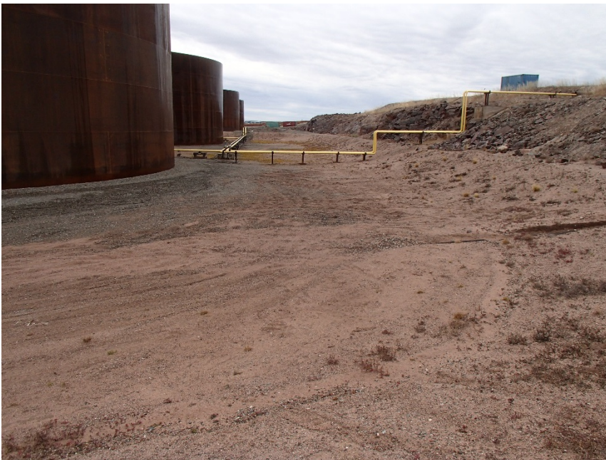
Photograph G1-12 Baker Lake Tank Farm
