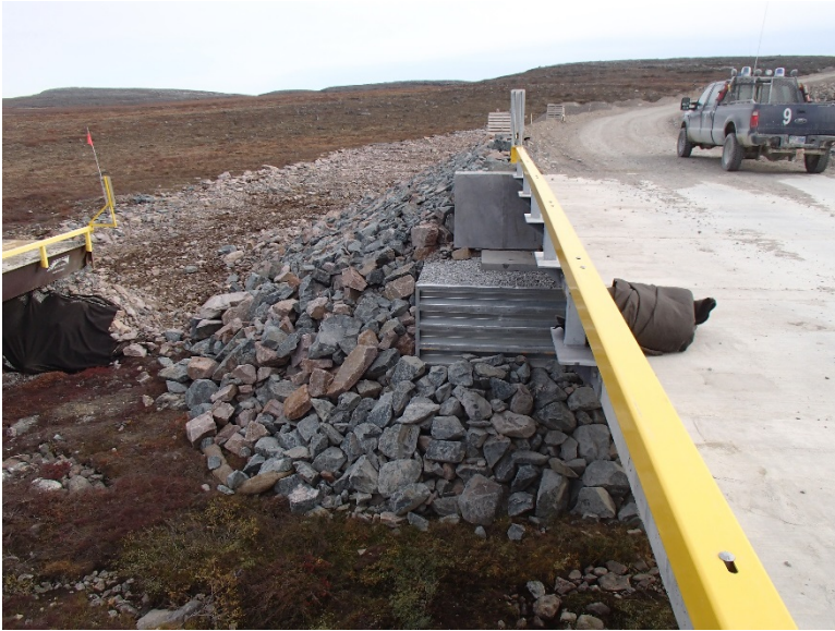
Photograph E2-31 Bridges 8 – km 43+500
