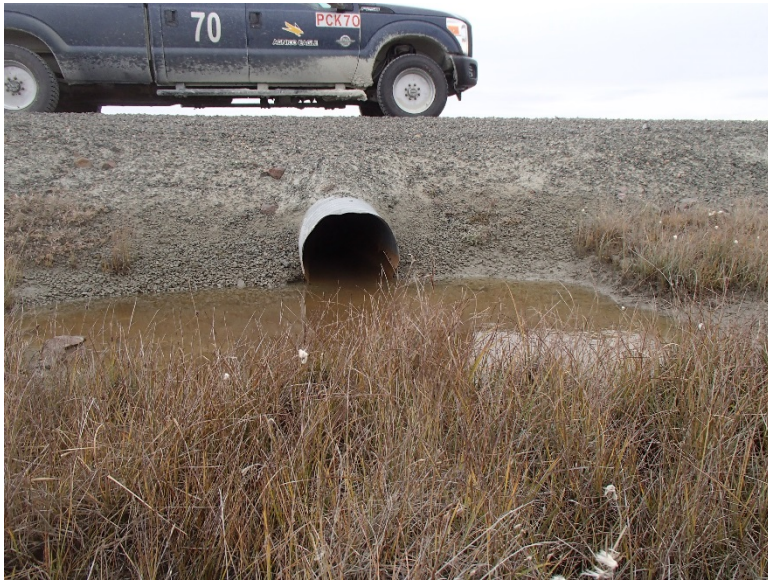
Photograph D1-27: unnamed km 13+950
