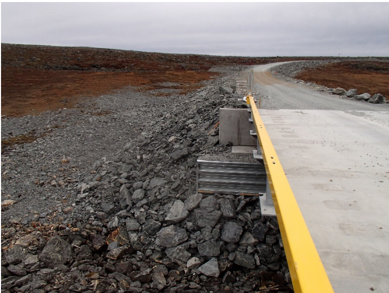
Photograph E2-4 Bridges 1 – km 3+400
