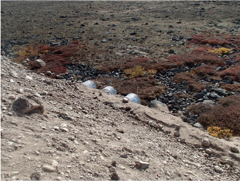
Photograph E1-11: Culvert #284 km 63+070
