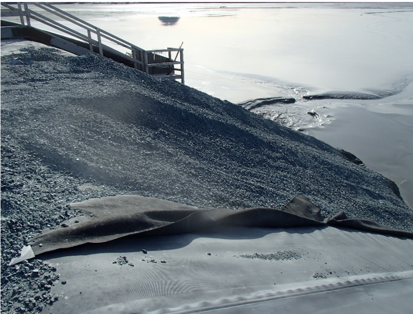
Photograph B7-8 Central Dike and Saddle Dam 5
