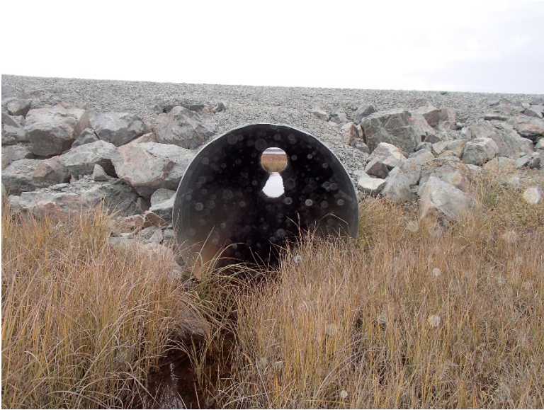
Photograph D1-41: R-07 km 25+900
