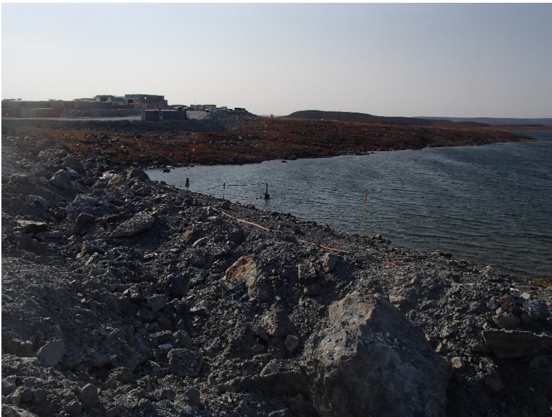
Photograph A2-2 South Camp Dike
