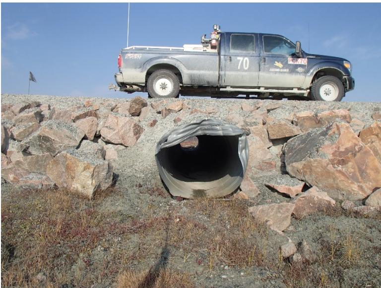
Photograph D1-66: R-23 km 93+600
