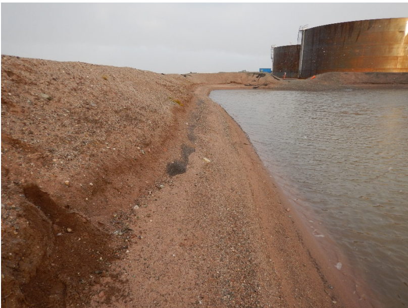
Photograph F1-8 Baker Lake Tank Farm
