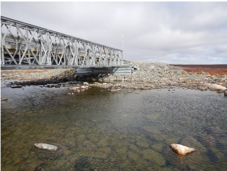
Photograph D2-16 Bridges 6 – R15 km 69+200
