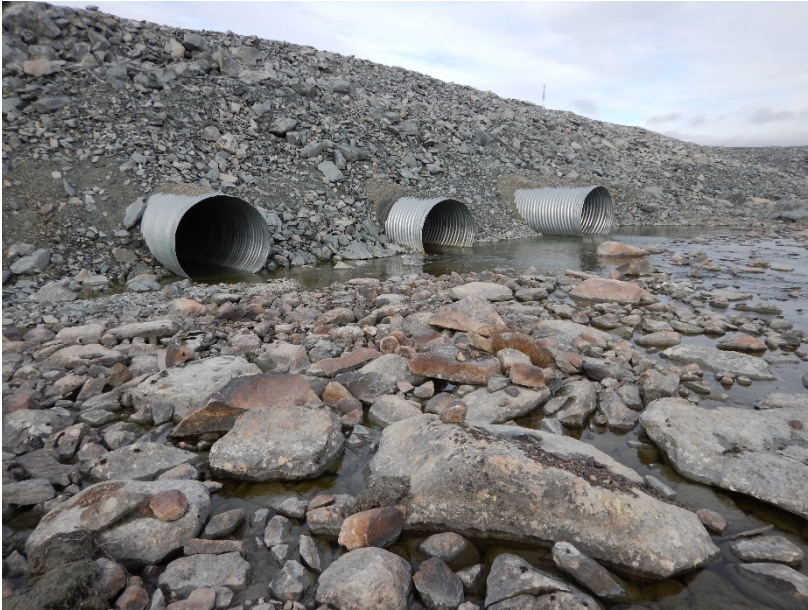
Photograph G1-1 Vault Road Culverts
