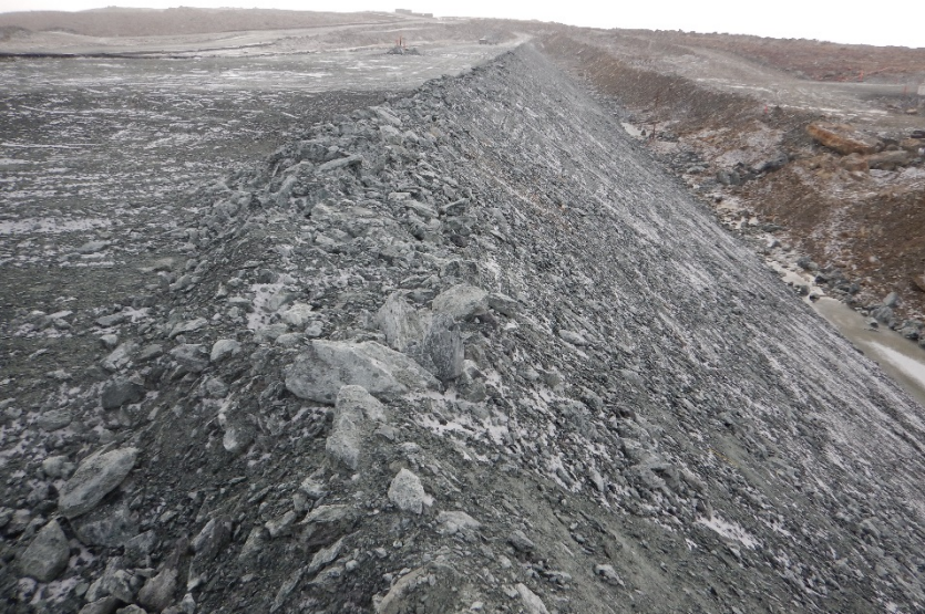
Photograph B5-2 Saddle Dam 3
