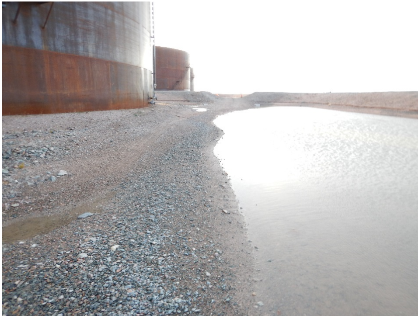
Photograph F1-5 Baker Lake Tank Farm
