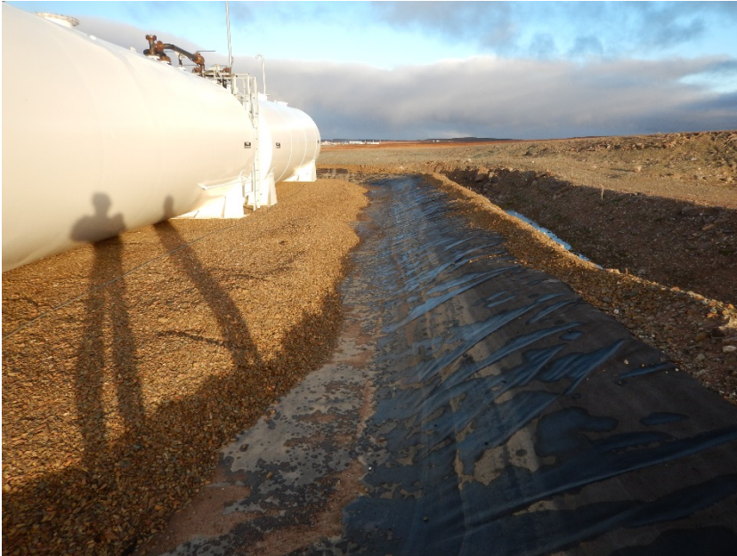
Photograph F1-23 Baker Lake Tank Farm
