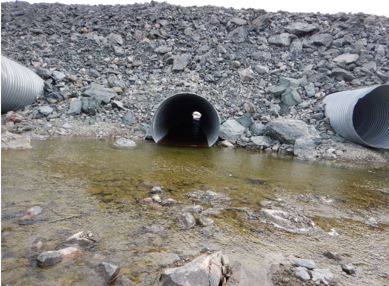
Photograph G1-3 Vault Road Culverts
