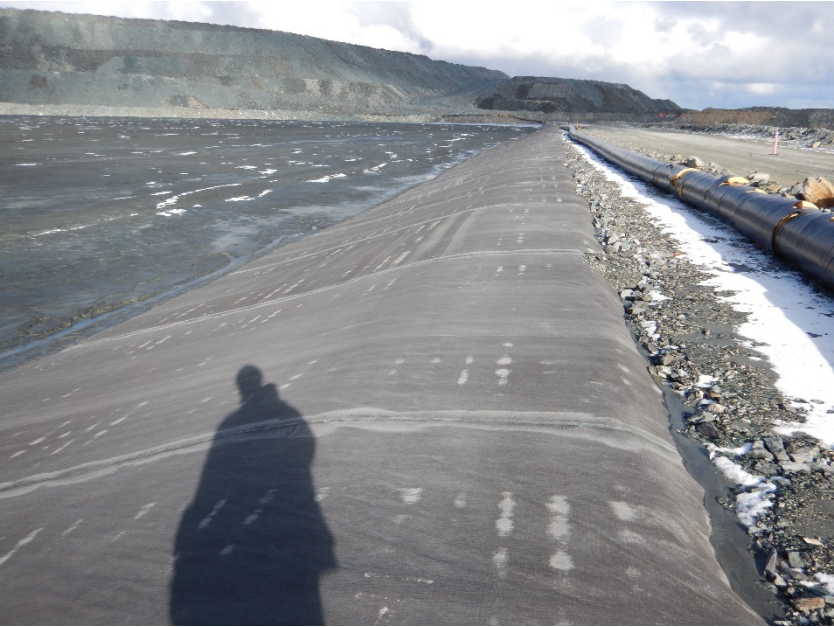
Photograph B4-2 Stormwater Dike
