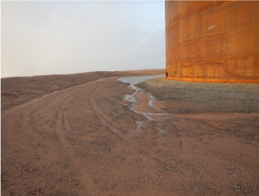
Photograph F1-11 Baker Lake Tank Farm
