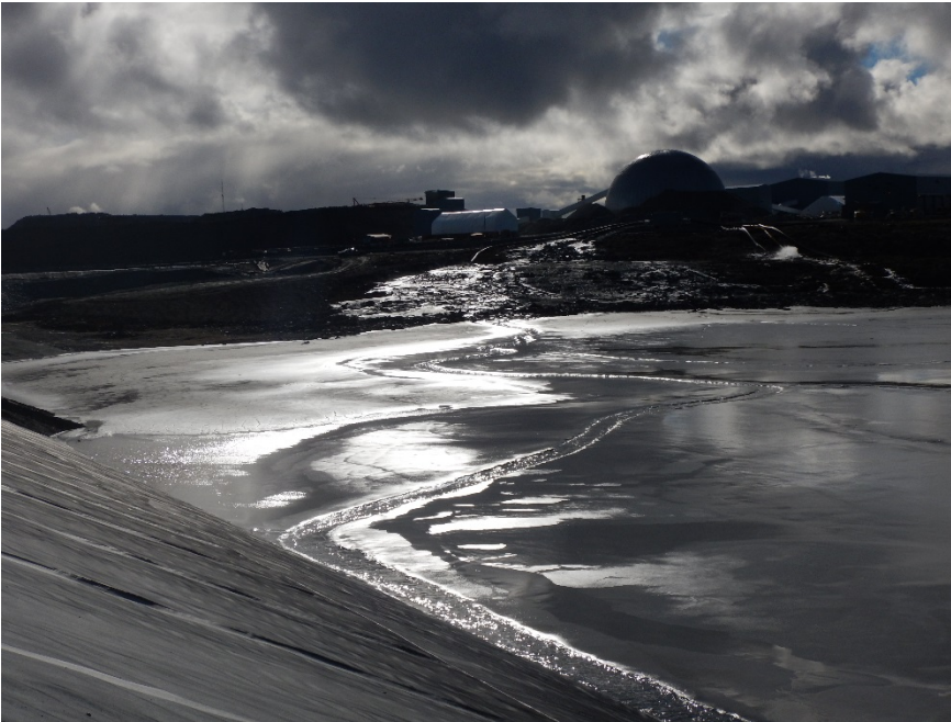
Photograph B7-3 Central Dike
