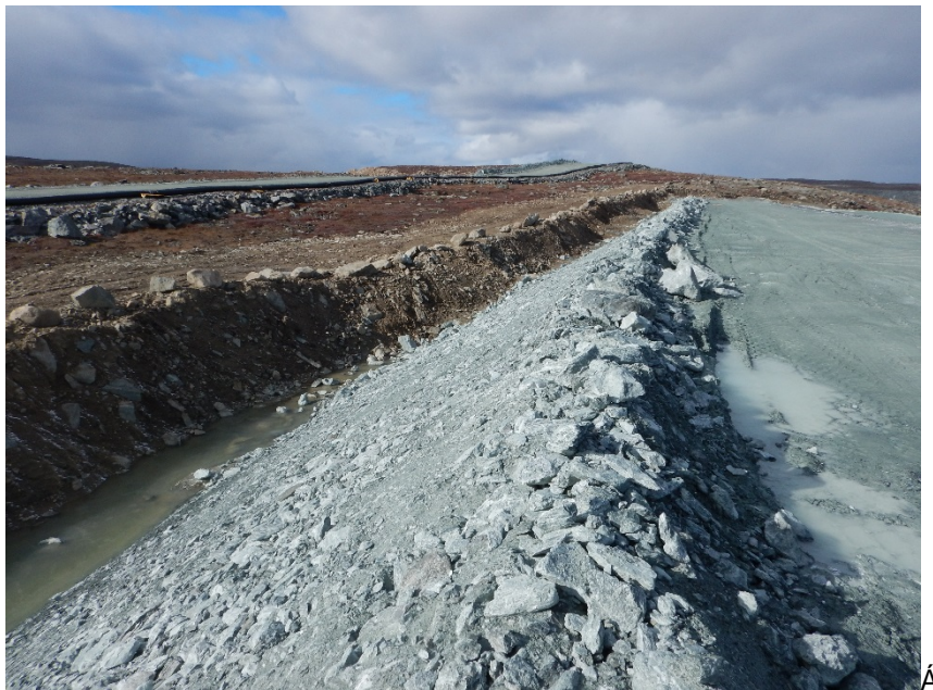
Photograph B6-4 Saddle Dam 4
