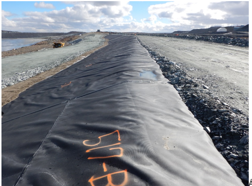
Photograph B6-3 Saddle Dam 4
