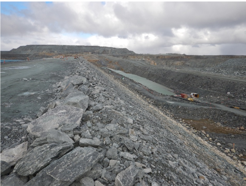
Photograph B7-6 Central Dike
