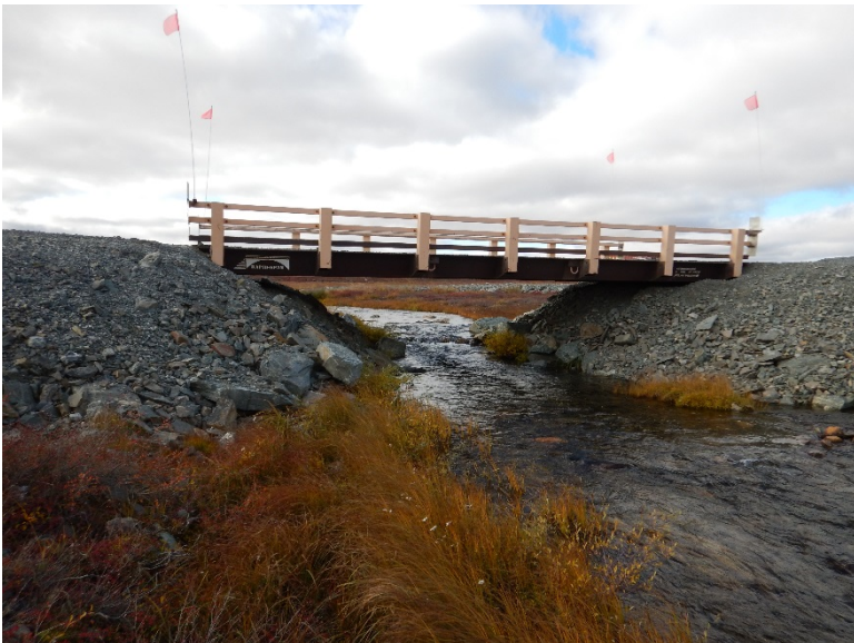
Photograph D2-12 Bridges 4 – R09 km 48+500
