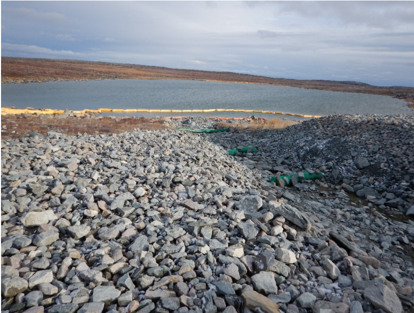
Photograph G2-1 Diversion Ditch and its Sediment and Erosion Protection Structure
