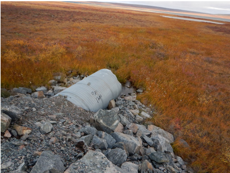
Photograph D1-22: R-04 km 12+050
