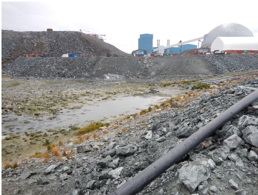
Photograph G7-1 Stormwater Pond
