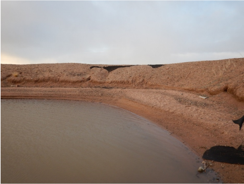
Photograph F1-7 Baker Lake Tank Farm
