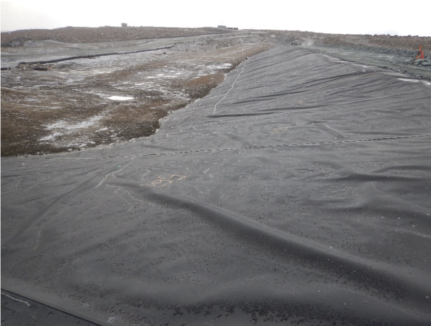
Photograph B5-1 Saddle Dam 3
