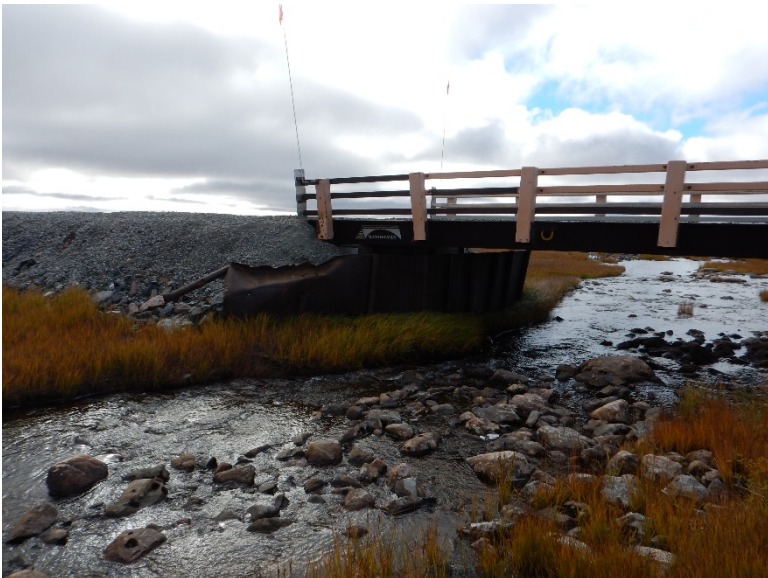
Photograph D2-26 Bridges 9 – R19 km 83+150
