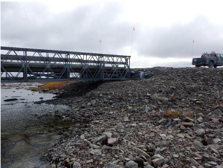
Photograph D2-18 Bridges 6 – R15 km 69+200
