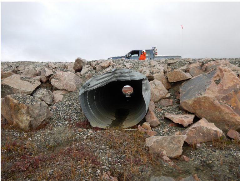
Photograph D1-68: R-23 km 93+600
