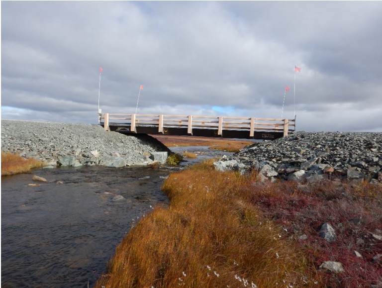
Photograph D2-11 Bridges 4 – R09 km 48+500
