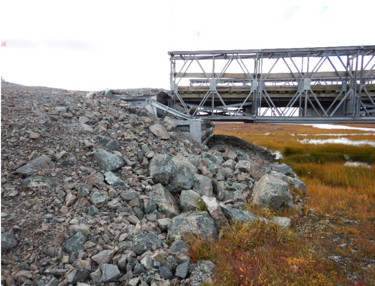
Photograph D2-6 Bridges 2 – R05 km 17+600
