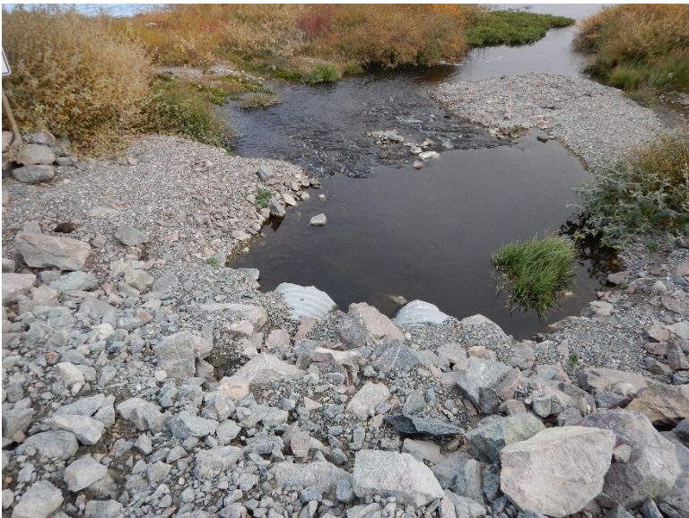
Photograph D1-4: PRC2 km 0+470
