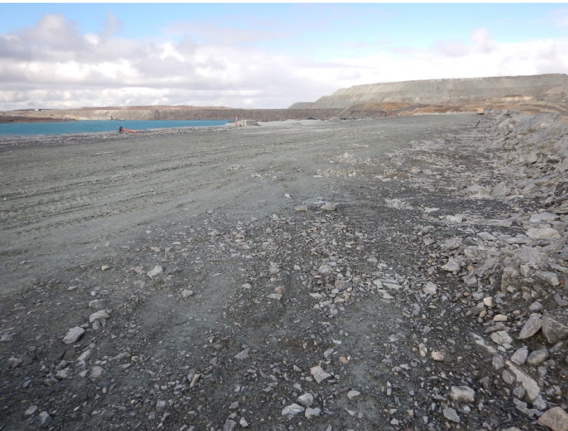
Photograph B7-10 Central Dike
