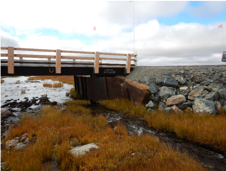
Photograph D2-25 Bridges 9 – R19 km 83+150
