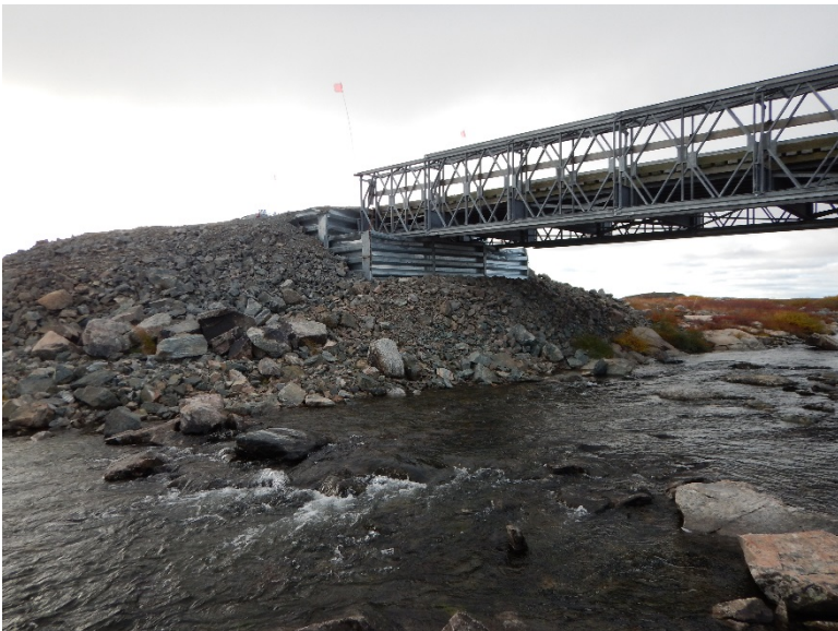
Photograph D2-2 Bridges 1 – R02 km 8+750
