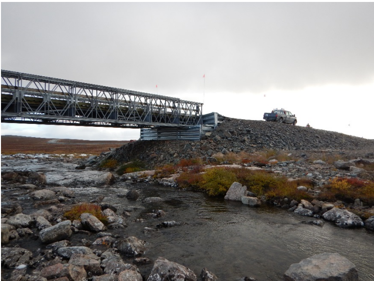
Photograph D2-4 Bridges 1 – R02 km 8+750
