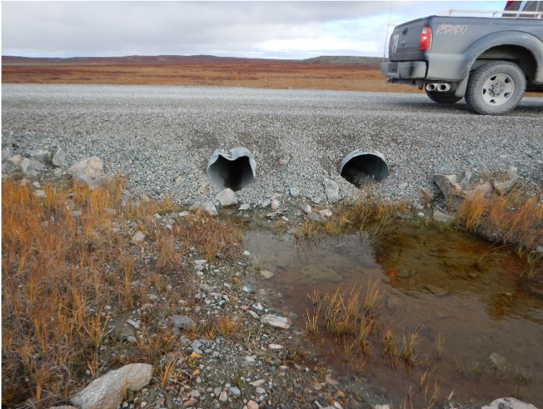
Photograph D1-39: PC-7A km 20+240
