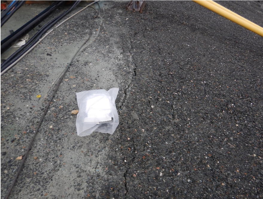
Photograph F2-9 Meadowbank Tank Farm
