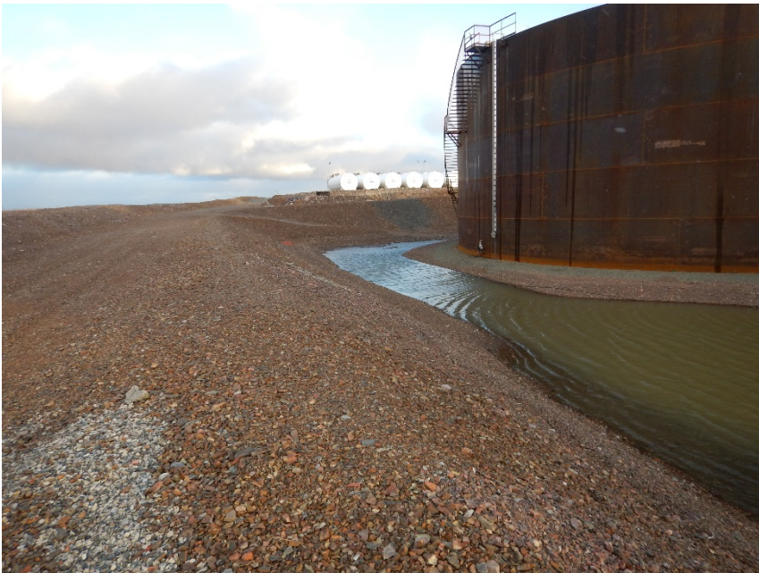
Photograph F1-16 Baker Lake Tank Farm
