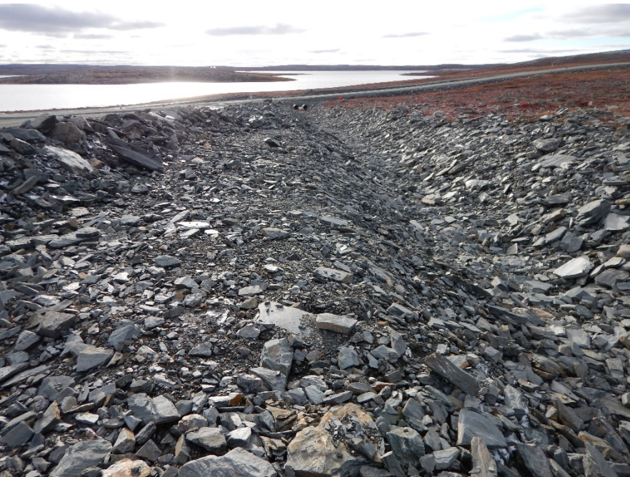
Photograph G2-12 Diversion Ditch and its Sediment and Erosion Protection Structure
