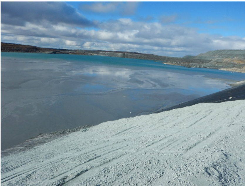
Photograph B7-2 Central Dike
