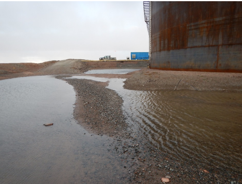
Photograph F1-4 Baker Lake Tank Farm
