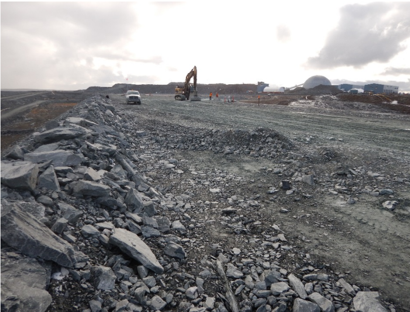
Photograph B7-9 Central Dike
