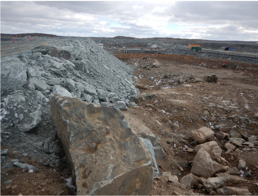
Photograph B7-11 Saddle Dam 5
