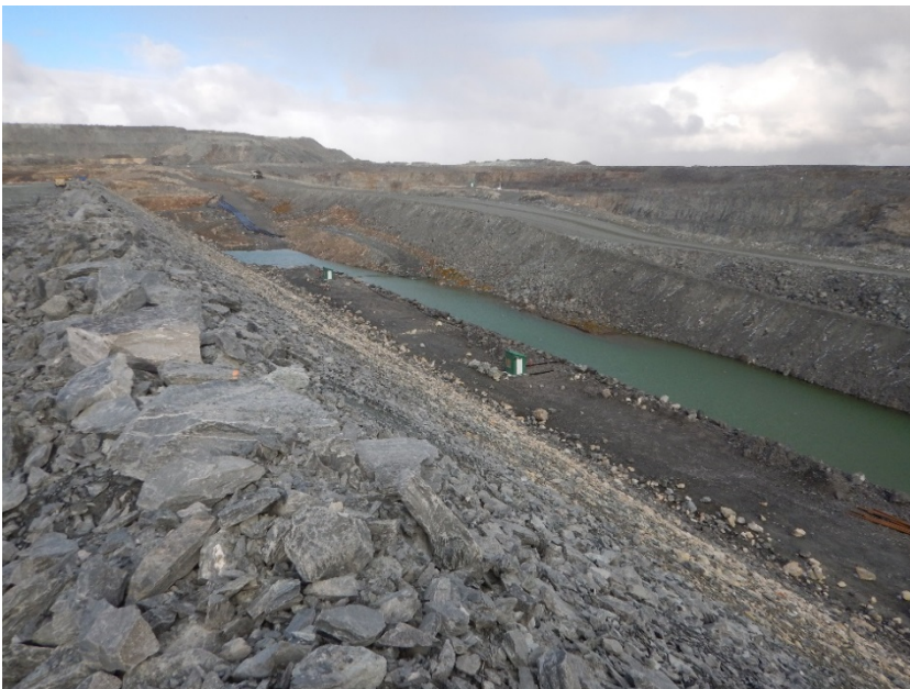
Photograph B7-8 Central Dike
