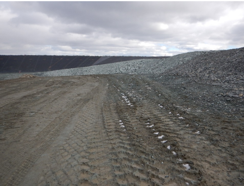
Photograph B7-12 Saddle Dam 5
