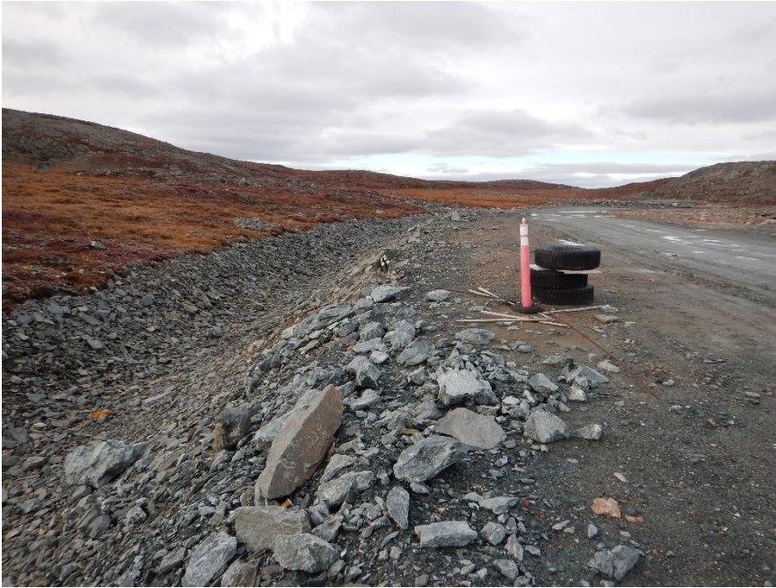
Photograph G2-7 Diversion Ditch and its Sediment and Erosion Protection Structure
