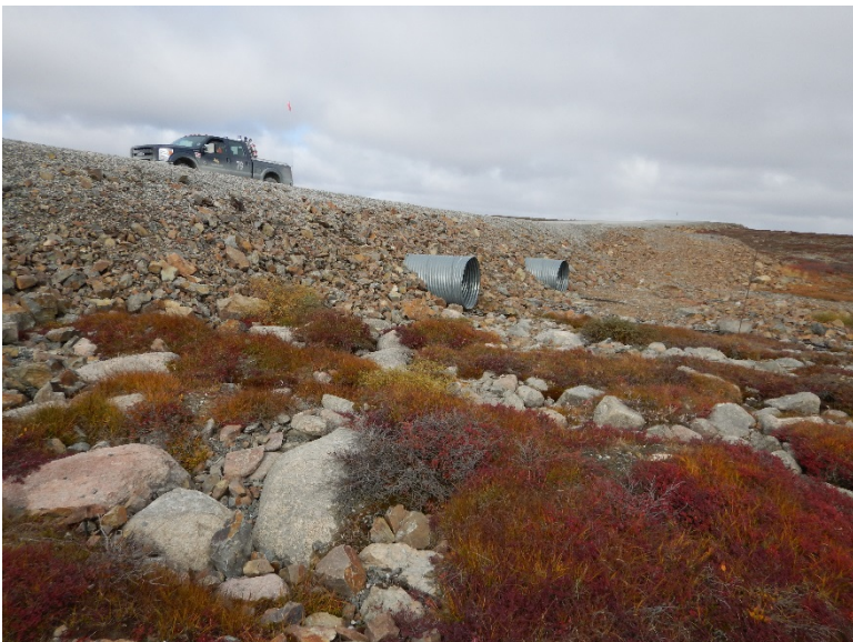
Photograph D1-56: R-14 km 67+840
