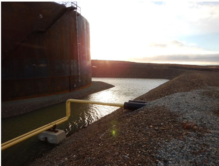
Photograph F1-18 Baker Lake Tank Farm
