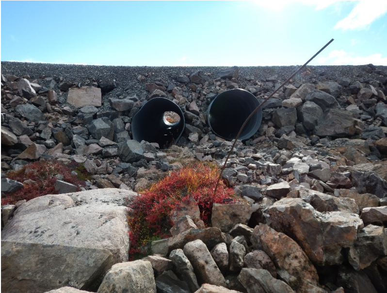
Photograph D1-69: R-24 km 98+100
