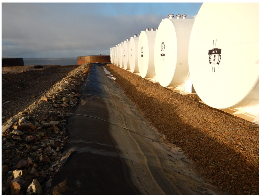
Photograph F1-22 Baker Lake Tank Farm
