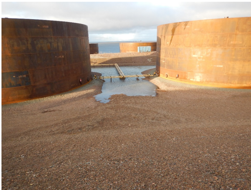
Photograph F1-20 Baker Lake Tank Farm
