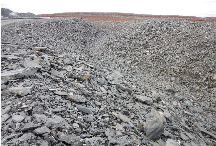
Photograph G2-4 Diversion Ditch and its Sediment and Erosion Protection Structure
