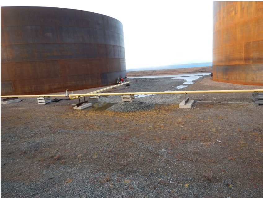
Photograph F1-14 Baker Lake Tank Farm
