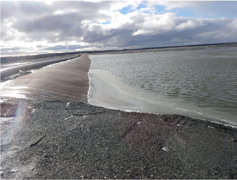
Photograph B4-1 Stormwater Dike
