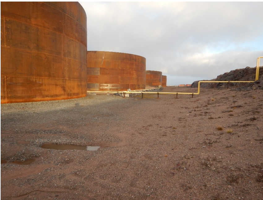
Photograph F1-12 Baker Lake Tank Farm
