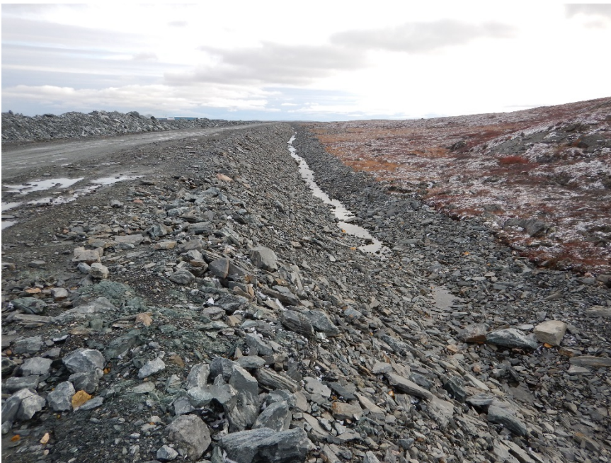
Photograph G2-8 Diversion Ditch and its Sediment and Erosion Protection Structure
