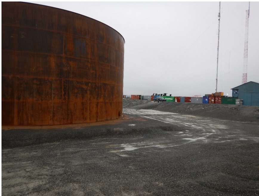
Photograph F2-3 Meadowbank Tank Farm
