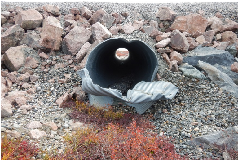
Photograph D1-64: R-20 km 85+490
