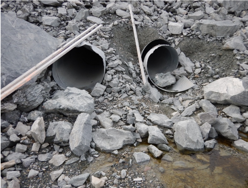
Photograph G1-5 Vault Road Culverts
