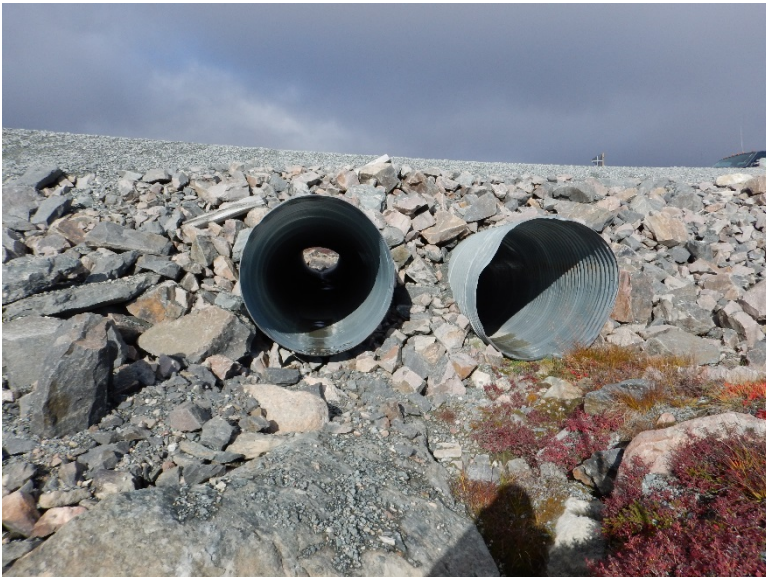
Photograph D1-70: R-24 km 98+100
