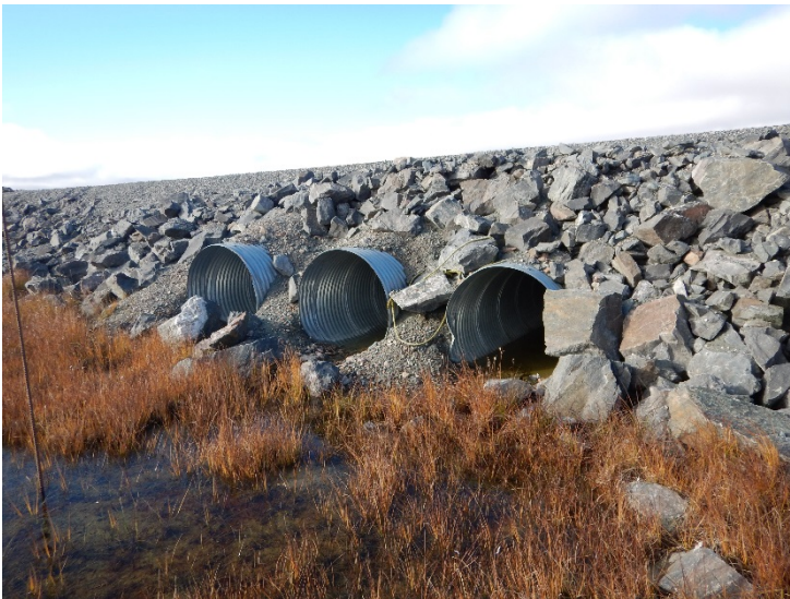
Photograph D1-74: R-26 km 104+400
