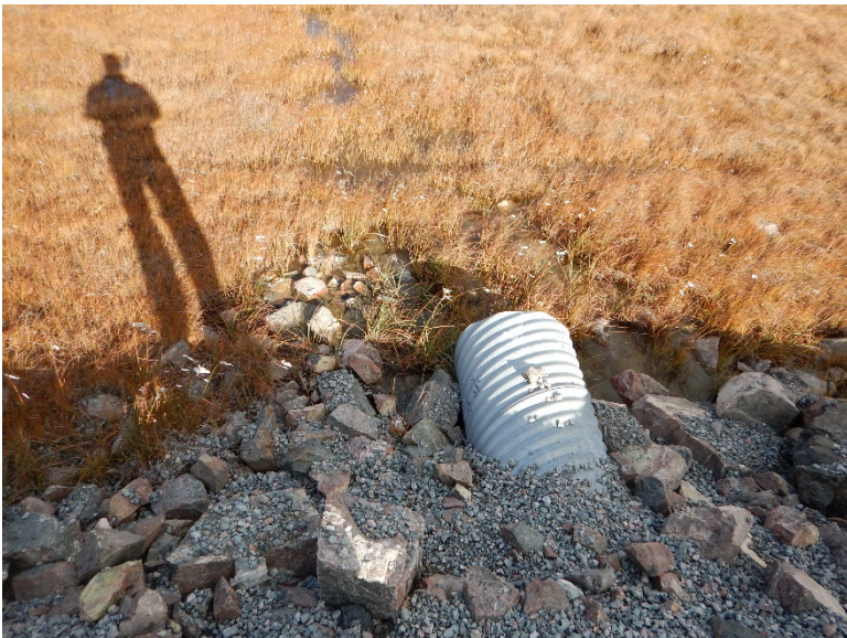
Photograph D1-20: R-03 km 10+580
