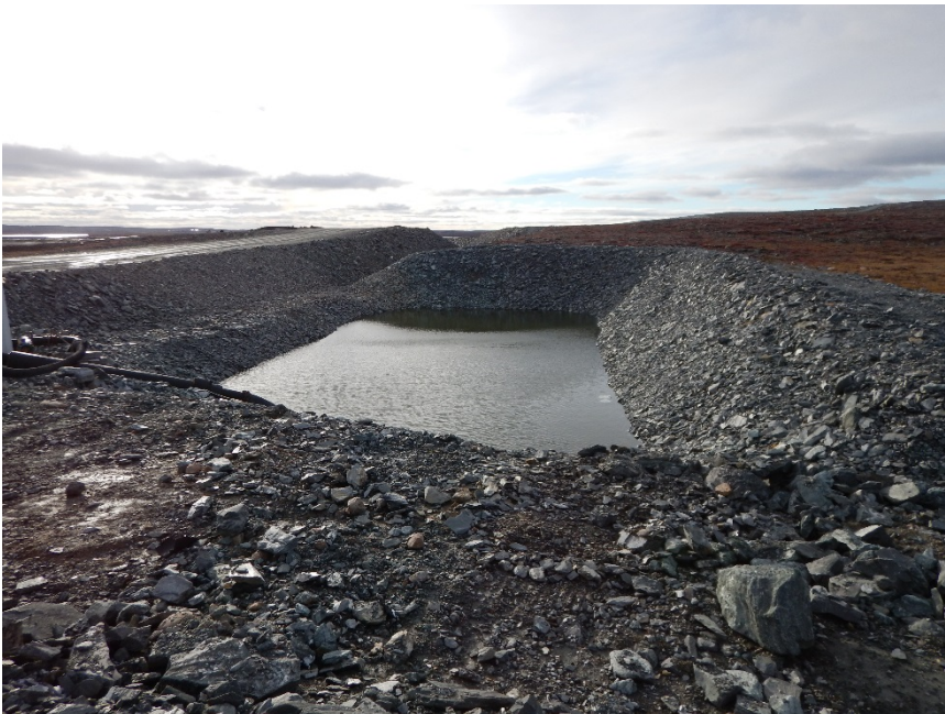
Photograph G2-10 Diversion Ditch and its Sediment and Erosion Protection Structure
