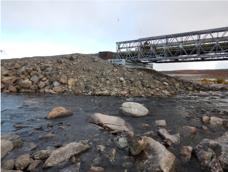
Photograph D2-3 Bridges 1 – R02 km 8+750
