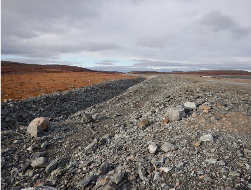
Photograph G2-9 Diversion Ditch and its Sediment and Erosion Protection Structure
