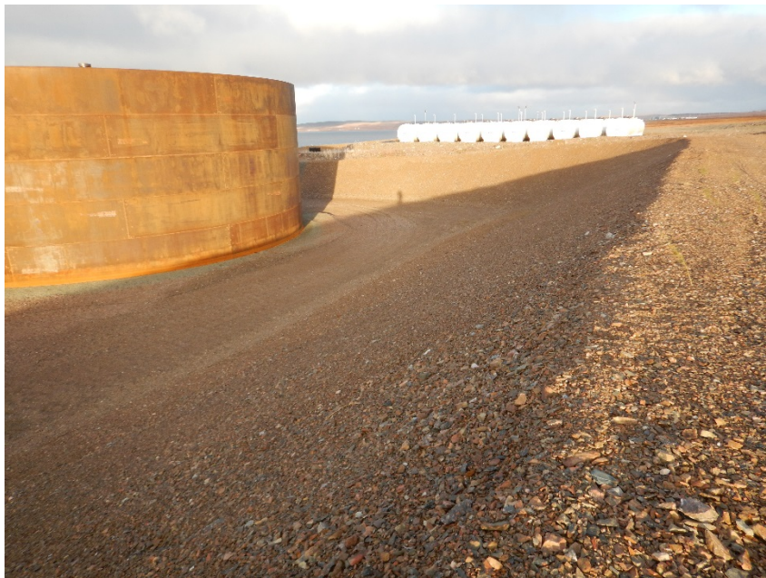
Photograph F1-21 Baker Lake Tank Farm
