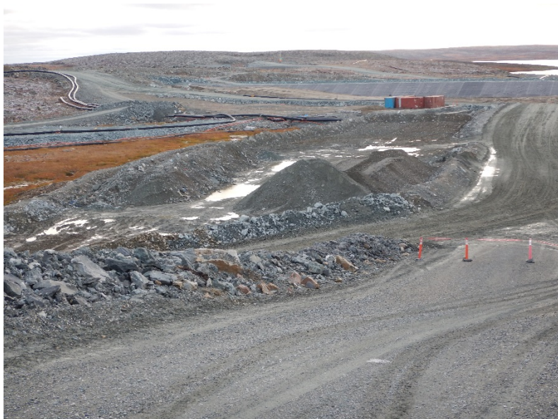
Photograph G6-1 Contaminated Soil Storage and Bioremediation Landfarm Facility
