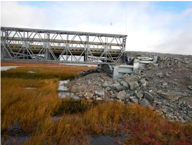
Photograph D2-8 Bridges 2 – R05 km 17+600
