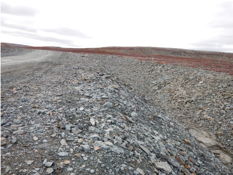
Photograph G2-6 Diversion Ditch and its Sediment and Erosion Protection Structure
