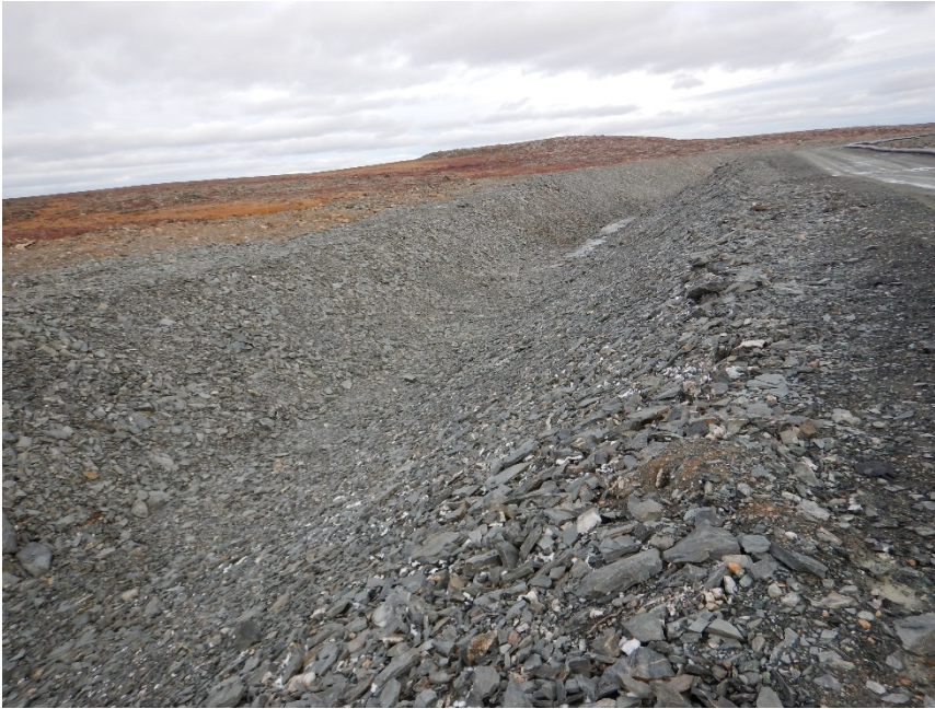
Photograph G2-3 Diversion Ditch and its Sediment and Erosion Protection Structure
