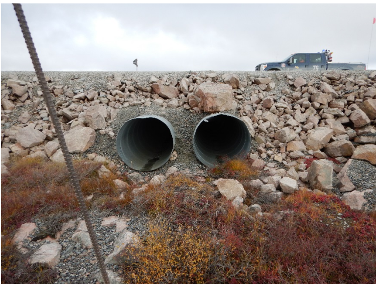
Photograph D1-66: R-21 km 87+300
