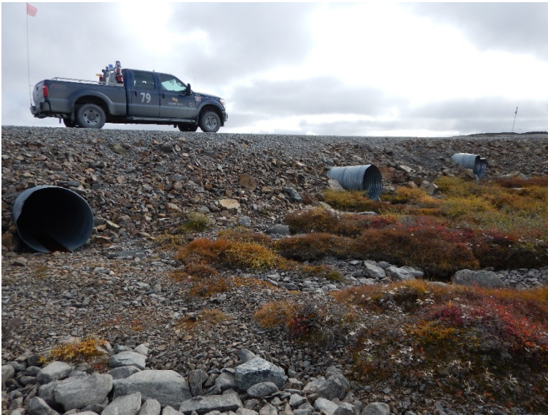
Photograph D1-55: R-14 km 67+840
