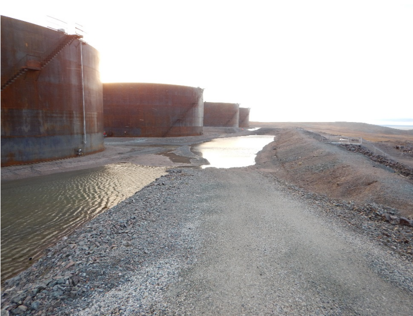
Photograph F1-1 Baker Lake Tank Farm
