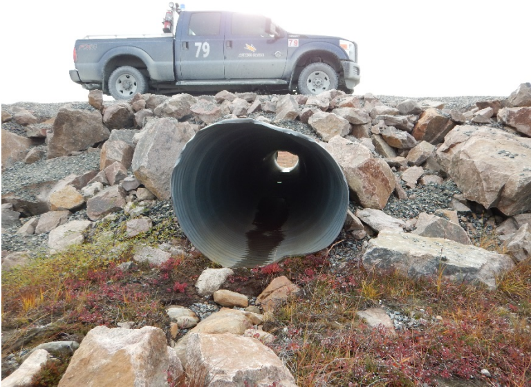
Photograph D1-67: R-23 km 93+600
