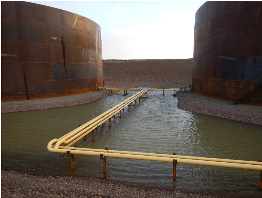
Photograph F1-17 Baker Lake Tank Farm
