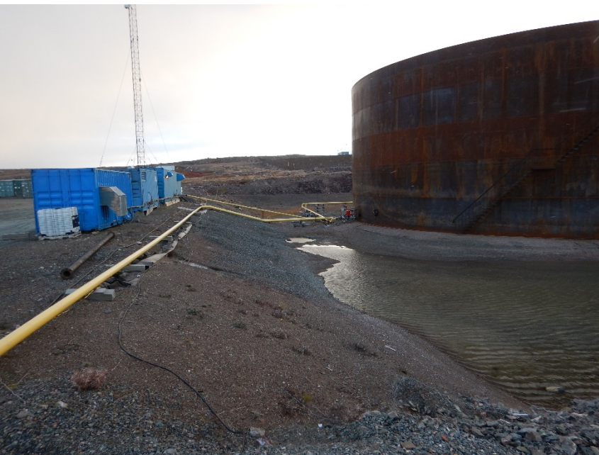
Photograph F1-2 Baker Lake Tank Farm
