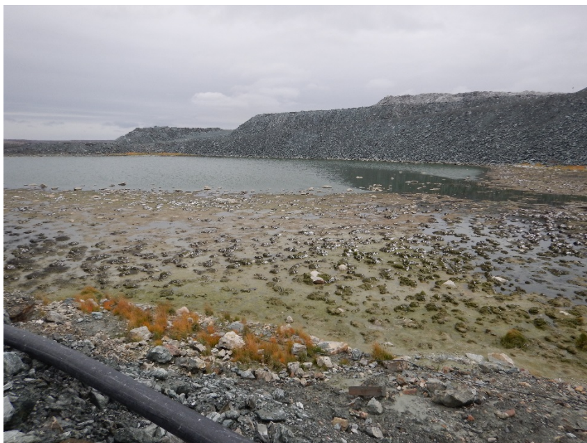
Photograph G7-2 Stormwater Pond
