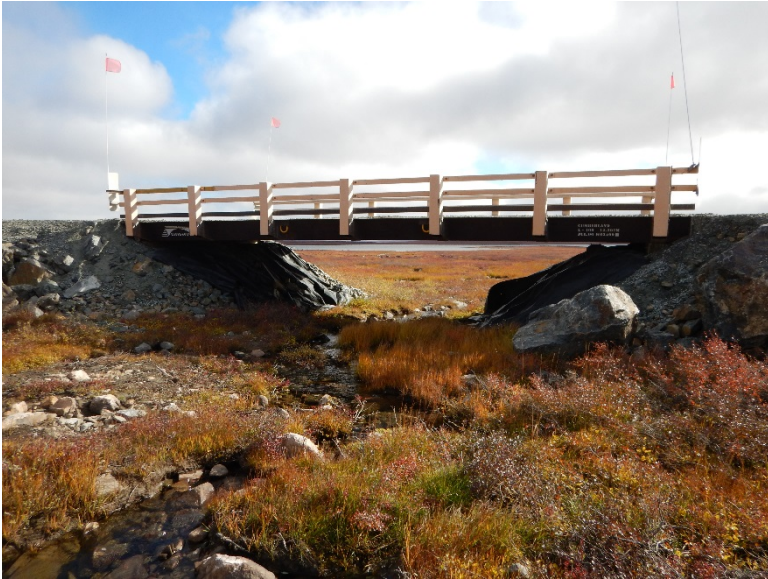
Photograph D2-19 Bridges 7 – R16 km 73+800
