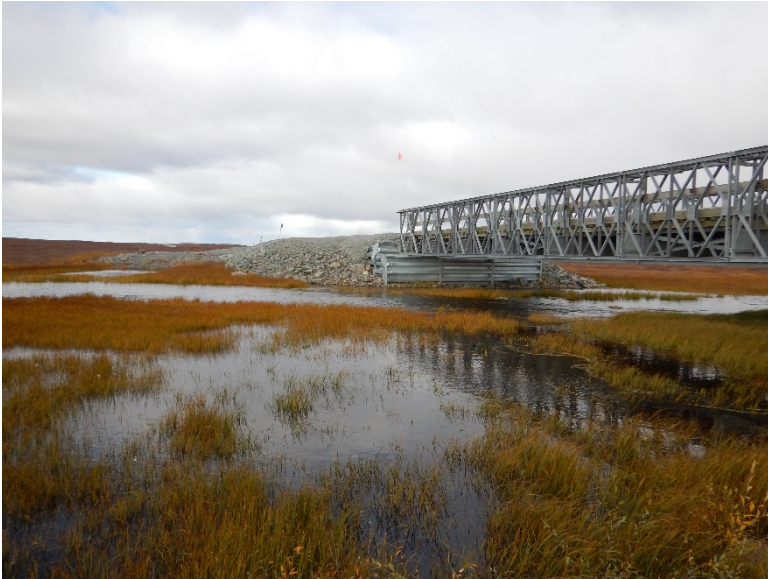
Photograph D2-7 Bridges 2 – R05 km 17+600
