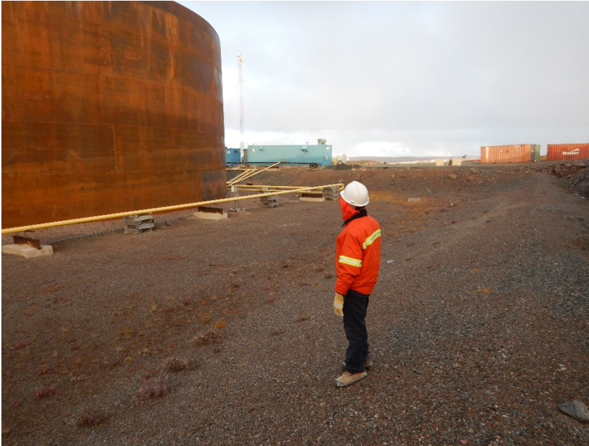
Photograph F1-13 Baker Lake Tank Farm
