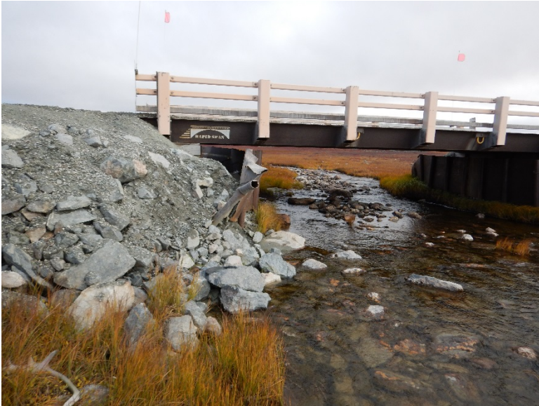
Photograph D2-23 Bridges 9 – R19 km 83+150
