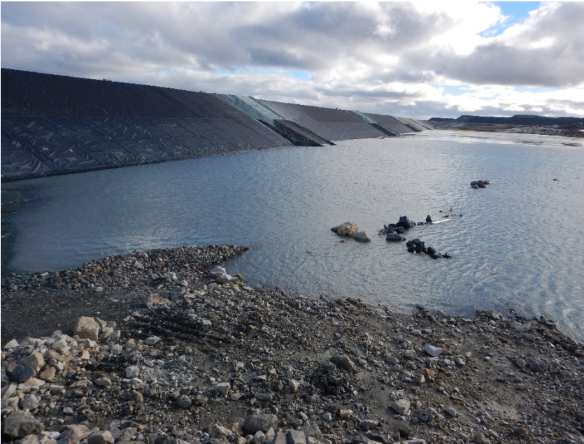
Photograph B7-1 Central Dike
