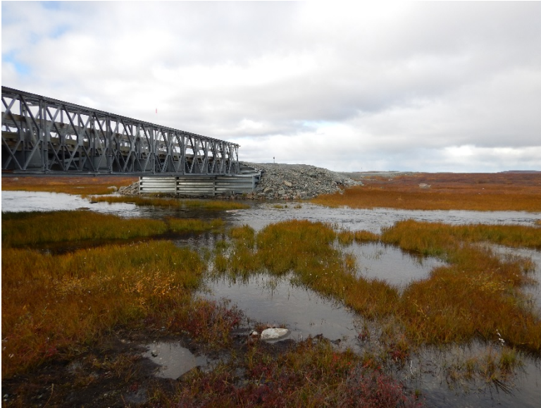
Photograph D2-5 Bridges 2 – R05 km 17+600
