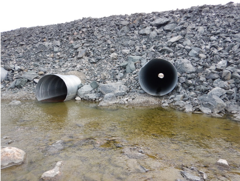
Photograph G1-2 Vault Road Culverts
