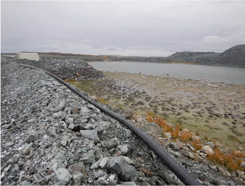
Photograph G7-3 Stormwater Pond
