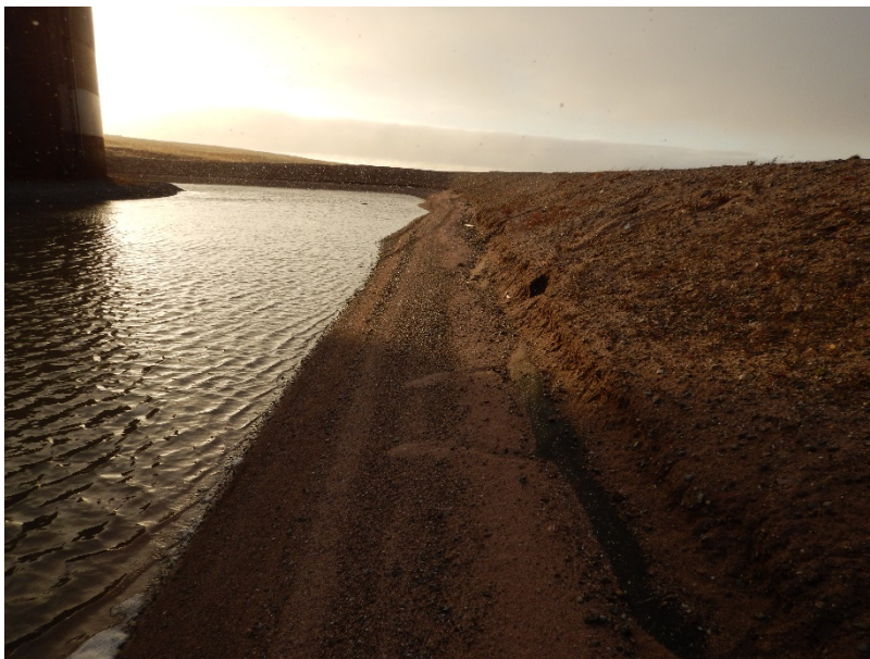
Photograph F1-10 Baker Lake Tank Farm
