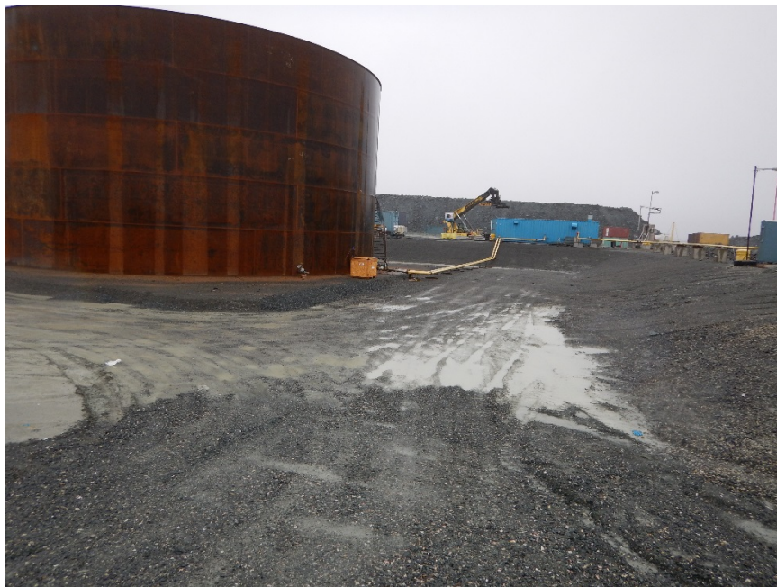
Photograph F2-1 Meadowbank Tank Farm
