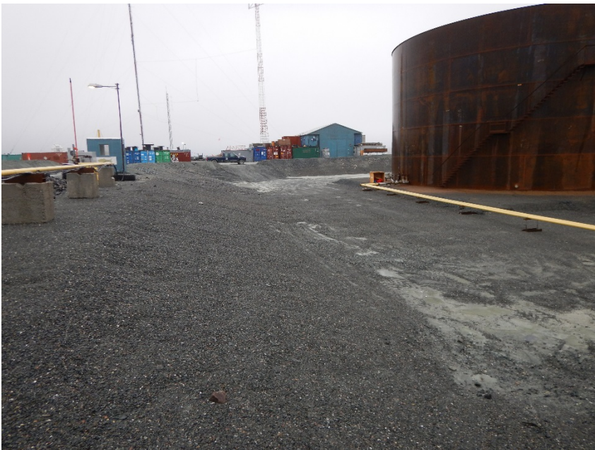
Photograph F2-6 Meadowbank Tank Farm
