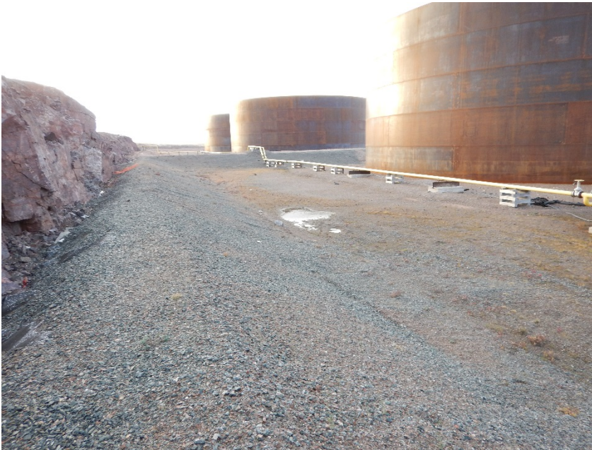
Photograph F1-15 Baker Lake Tank Farm
