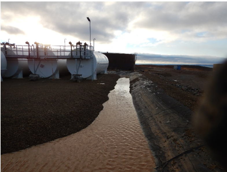
Photograph F1-24 Baker Lake Tank Farm
