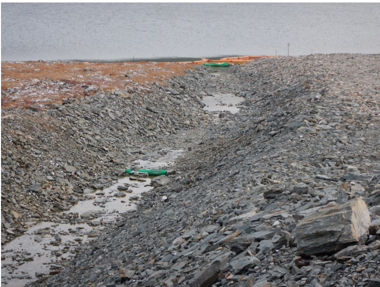
Photograph G2-2 Diversion Ditch and its Sediment and Erosion Protection Structure
