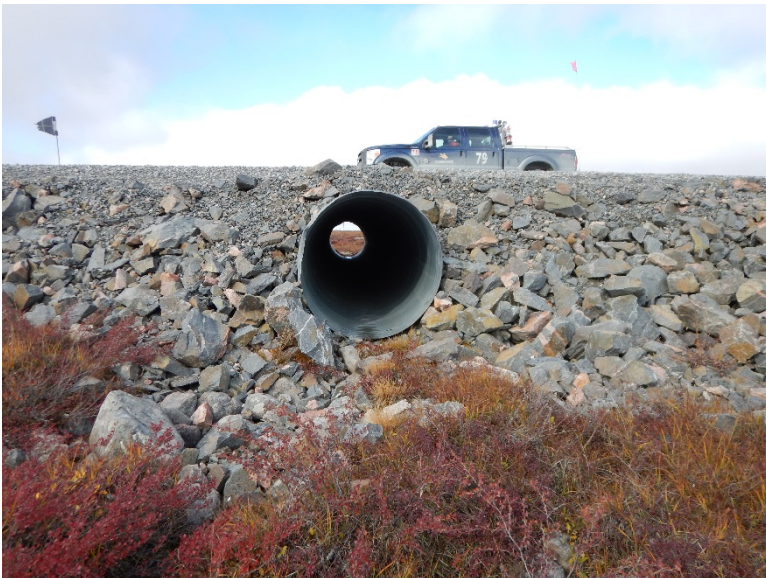
Photograph D1-58: R-17 km 77+440
