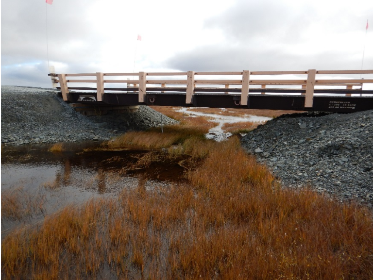
Photograph D2-13 Bridges 5 – R13 km 62+060
