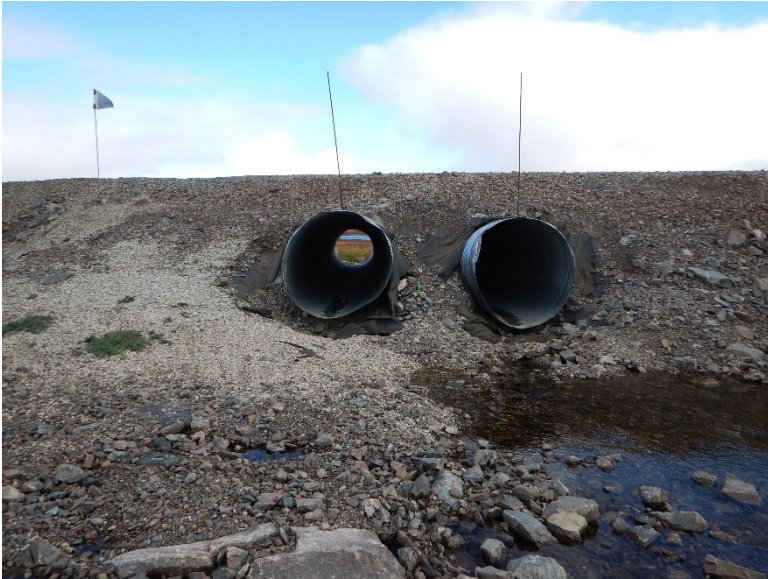
Photograph D1-13: PC-17A km 8+830
