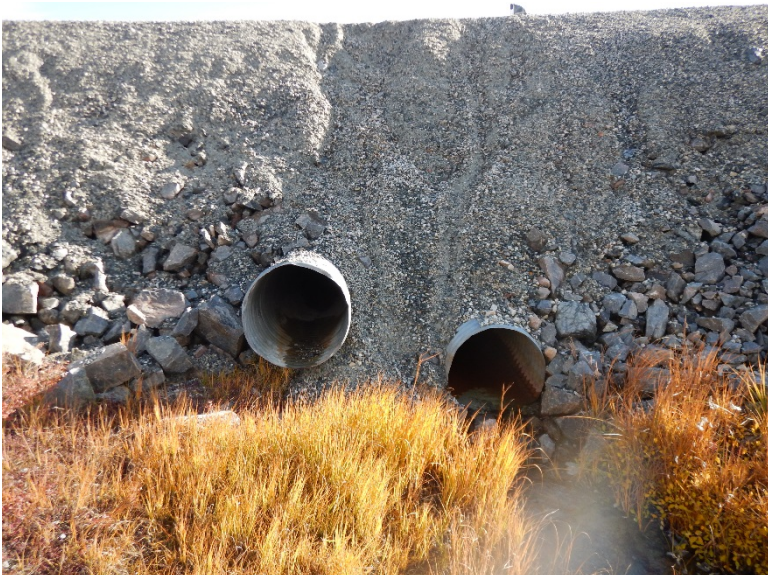
Photograph D1-72: R-25 km 101+950
