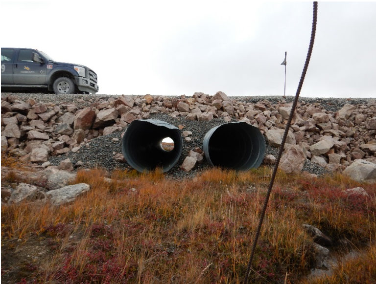
Photograph D1-65: R-21 km 87+300
