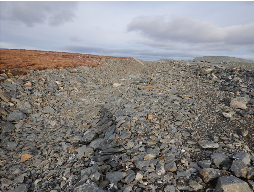
Photograph G2-11 Diversion Ditch and its Sediment and Erosion Protection Structure
