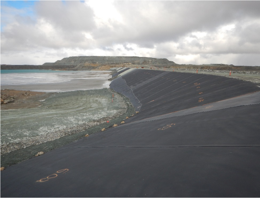
Photograph B7-5 Central Dike
