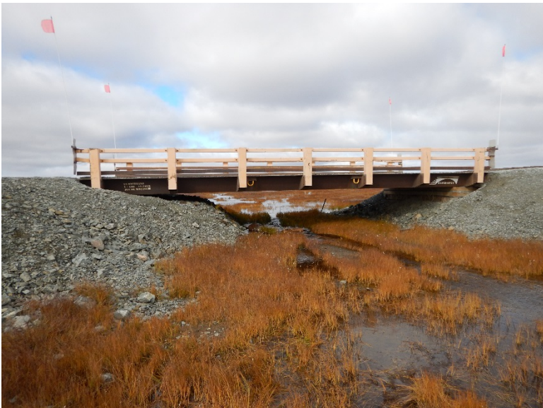
Photograph D2-14 Bridges 5 – R13 km 62+060
