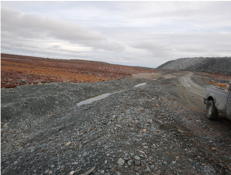
Photograph G2-5 Diversion Ditch and its Sediment and Erosion Protection Structure
