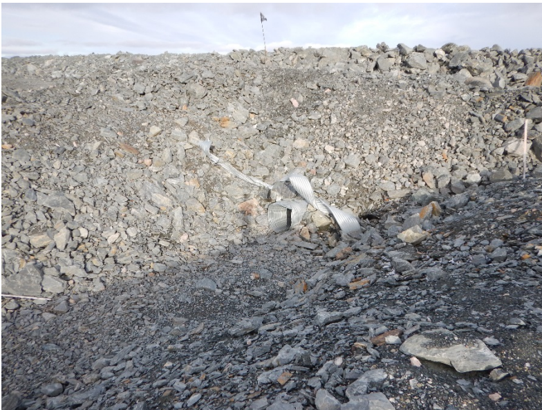
Photograph G1-6 Vault Road Culverts
