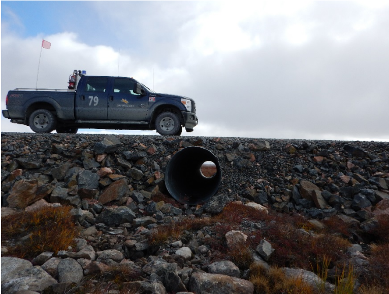
Photograph D1-57: R-17 km 77+440
