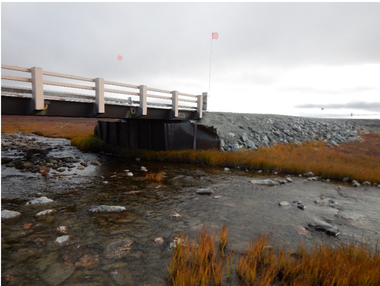
Photograph D2-24 Bridges 9 – R19 km 83+150
