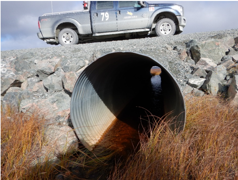
Photograph D1-43: R-07 km 25+900
