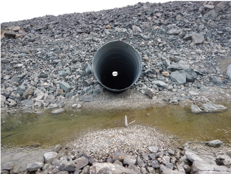
Photograph G1-4 Vault Road Culverts
