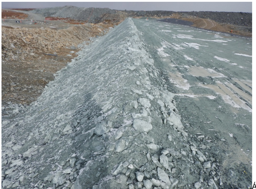
Photograph B5-3 Saddle Dam 3
