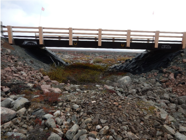
Photograph D2-21 Bridges 8 – R18 km 79+500
