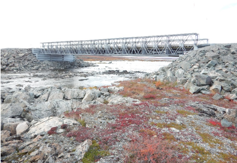
Photograph D2-10 Bridges 3 – R06 km 23+100
