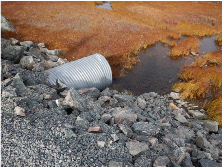
Photograph D1-44: R-07 km 25+900
