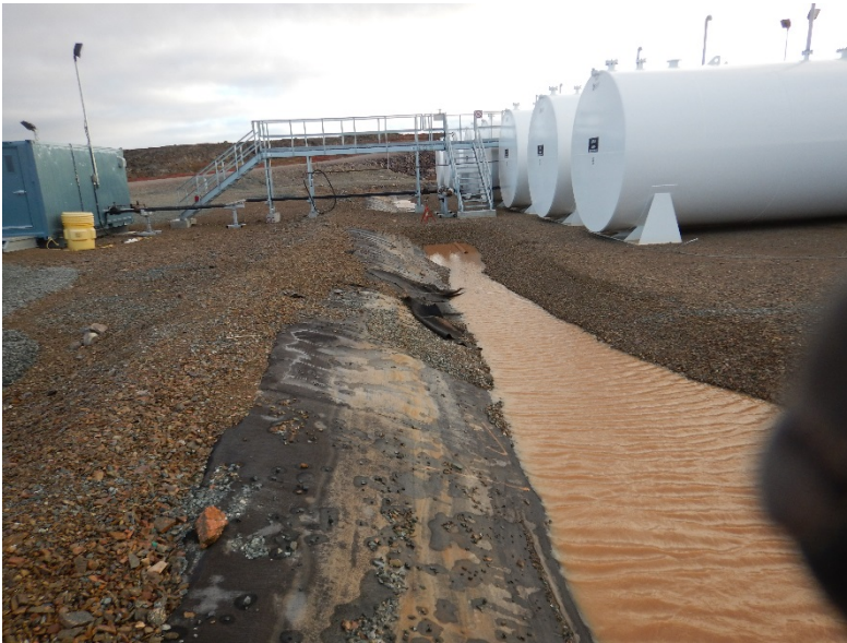
Photograph F1-25 Baker Lake Tank Farm
