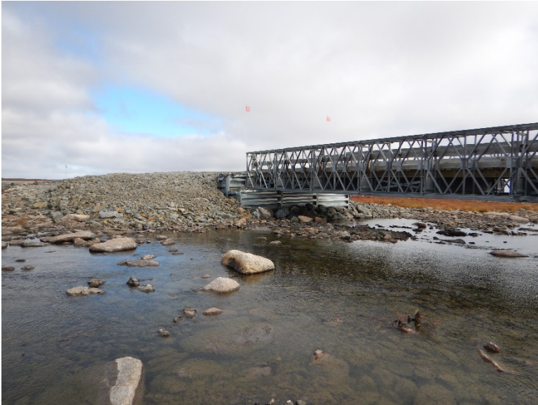
Photograph D2-17 Bridges 6 – R15 km 69+200
