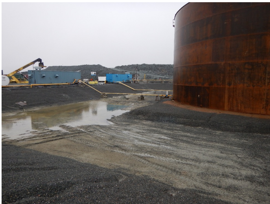
Photograph F2-4 Meadowbank Tank Farm
