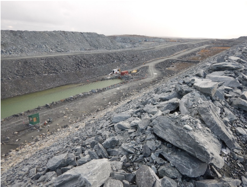
Photograph B7-7 Central Dike
