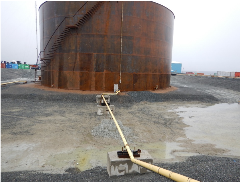
Photograph F2-7 Meadowbank Tank Farm
