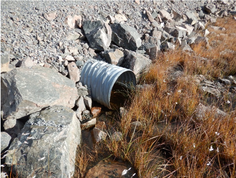
Photograph D1-19: R-03 km 10+580
