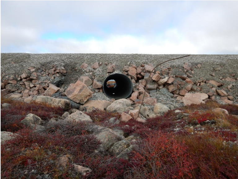
Photograph D1-63: R-20 km 85+490
