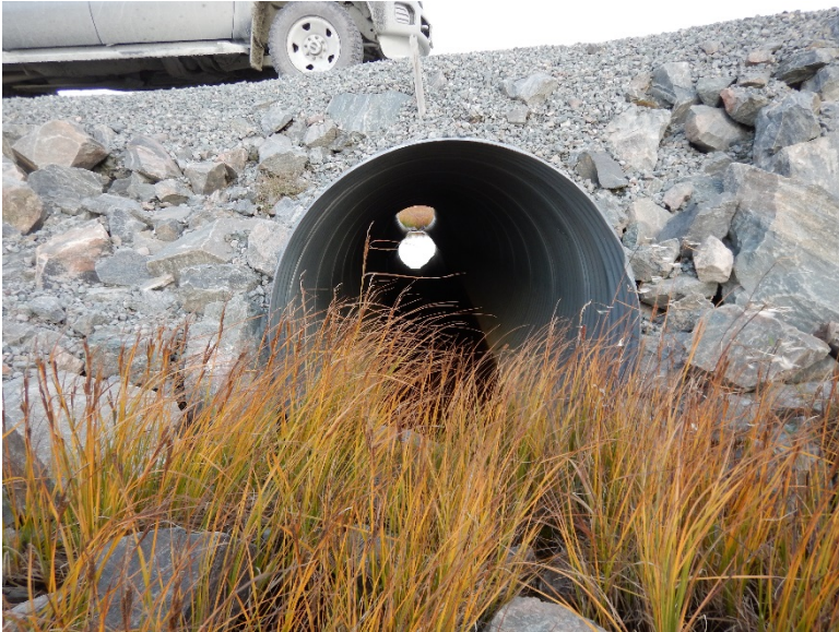
Photograph D1-21: R-04 km 12+050
