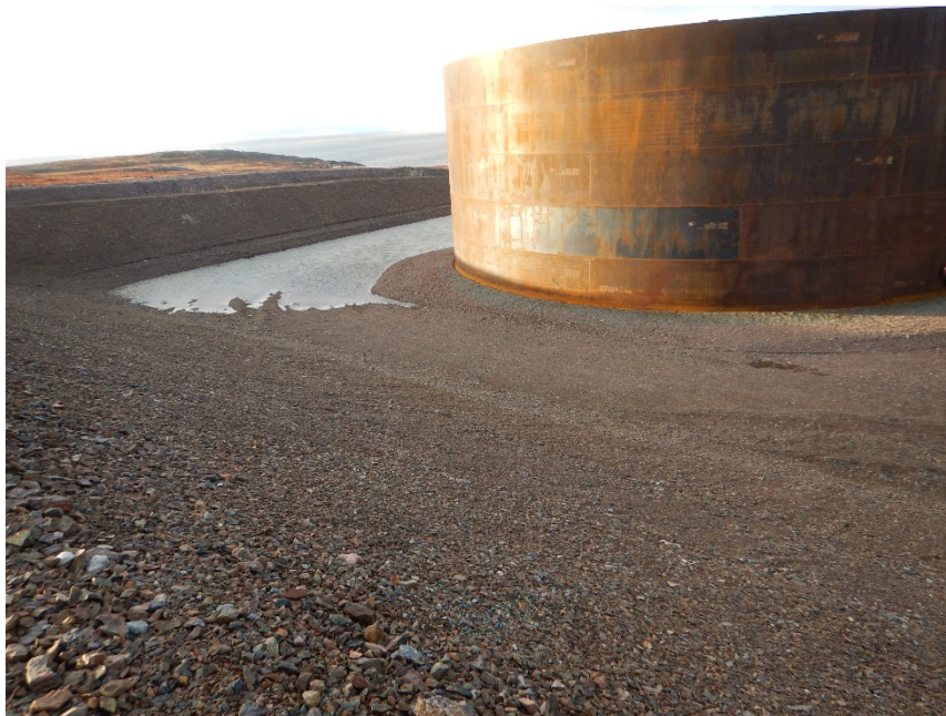
Photograph F1-19 Baker Lake Tank Farm
