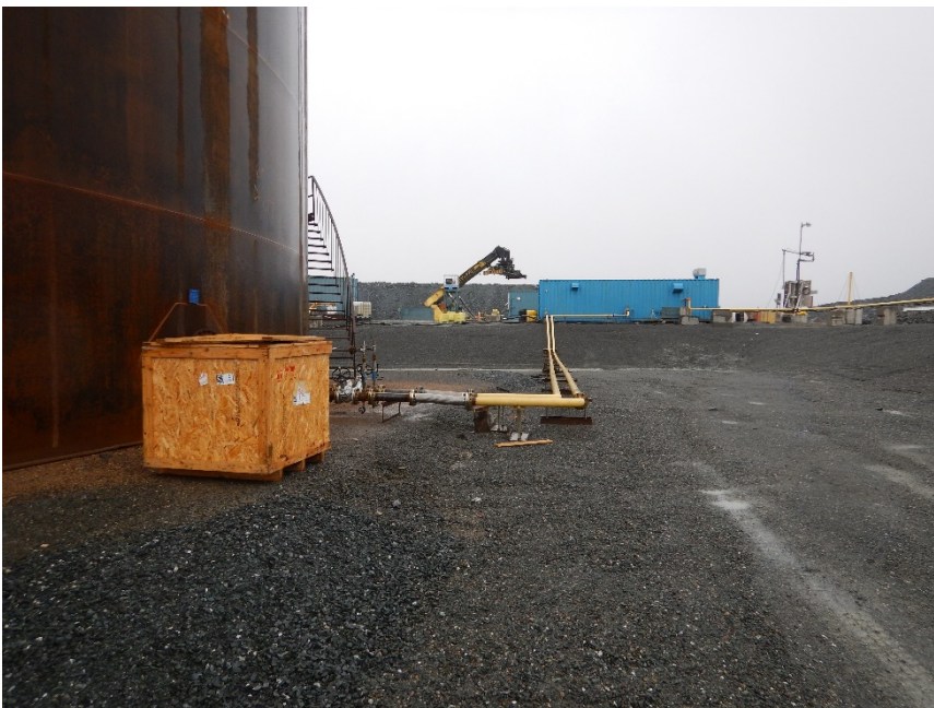
Photograph F2-8 Meadowbank Tank Farm
