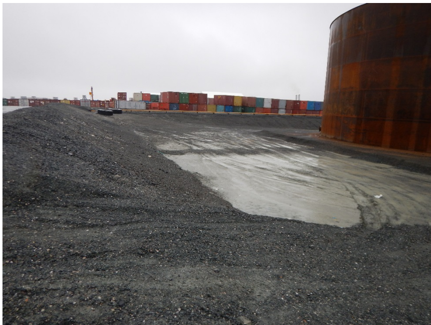
Photograph F2-2 Meadowbank Tank Farm
