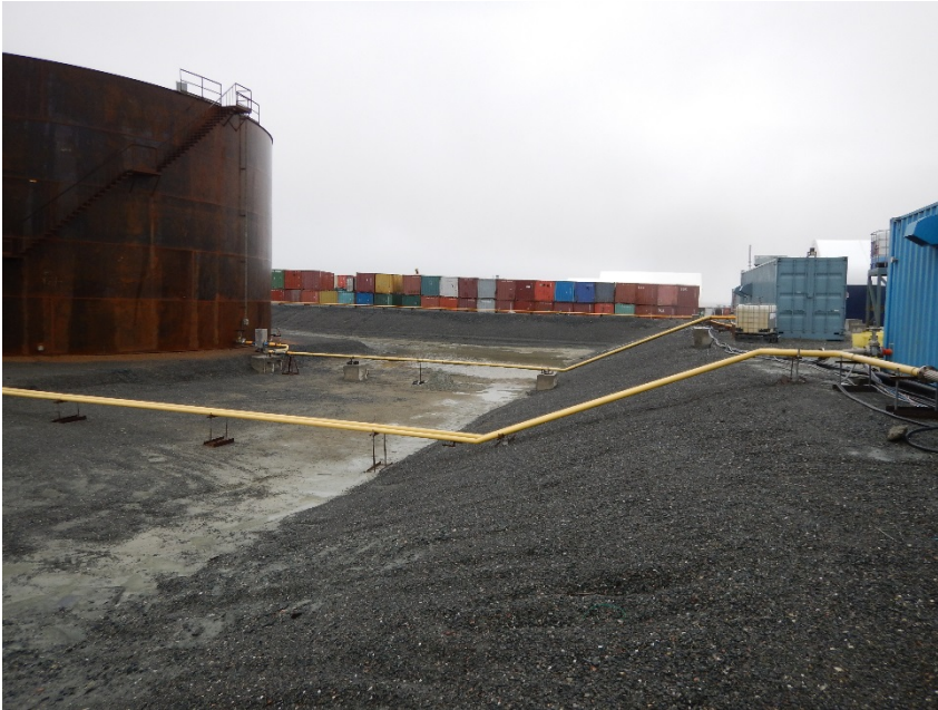
Photograph F2-5 Meadowbank Tank Farm
