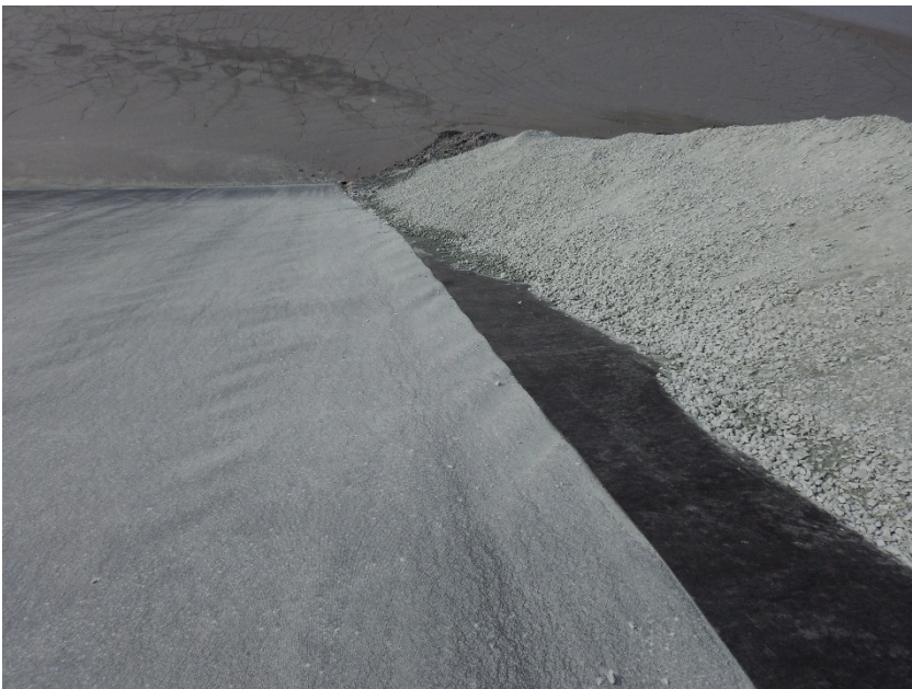
Photograph B7-4 Central Dike
