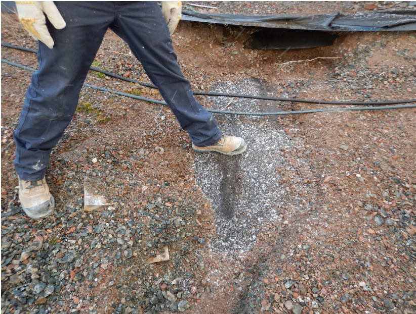
Photograph F1-3 Baker Lake Tank Farm
