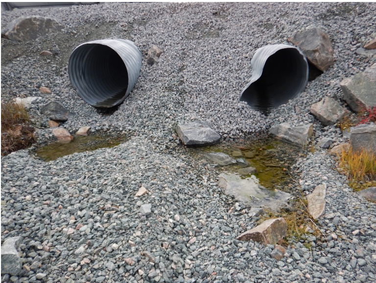
Photograph D1-40: PC-7A km 20+240
