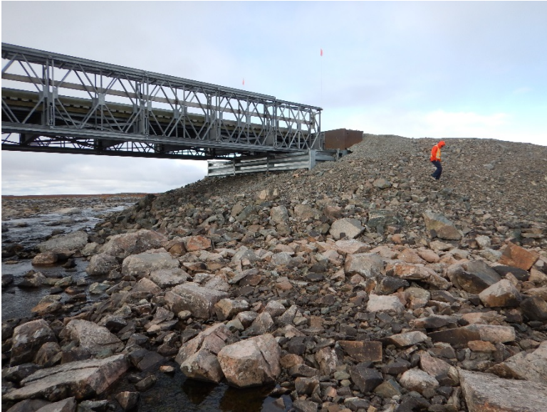
Photograph D2-1 Bridges 1 – R02 km 8+750
