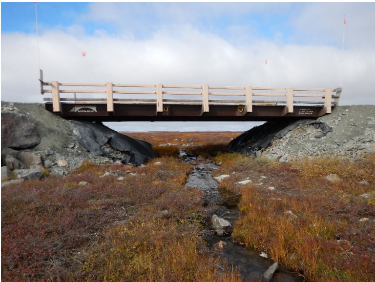
Photograph D2-20 Bridges 7 – R16 km 73+800
