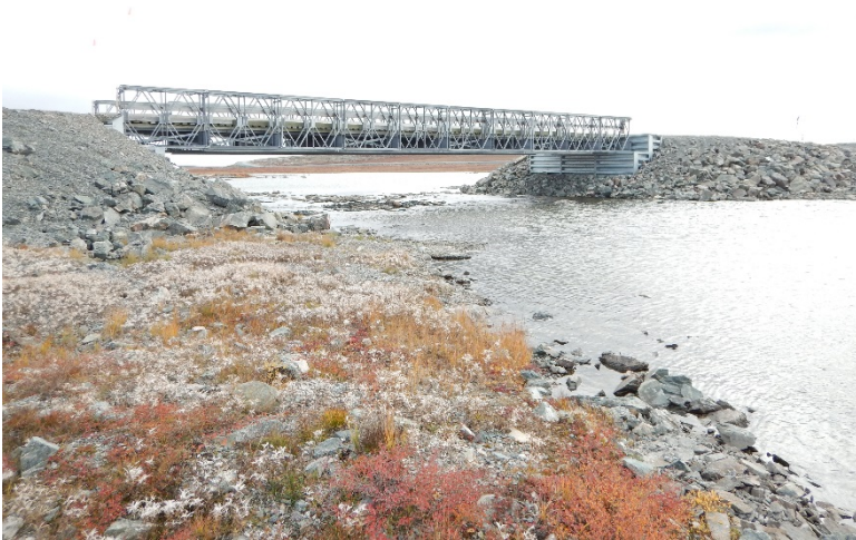
Photograph D2-9 Bridges 3 – R06 km 23+100
