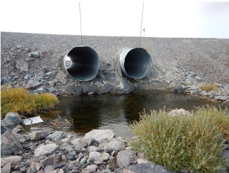
Photograph D1-14: PC-17A km 8+830
