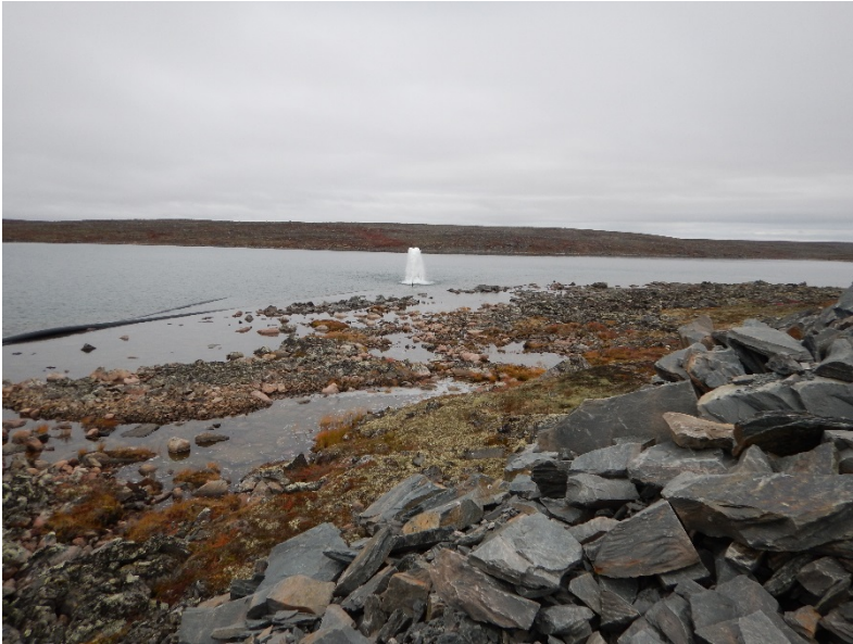
Photograph G4-1 Diffusers – Wally Lake Diffuser
