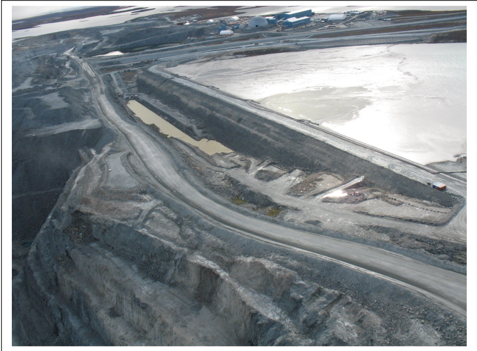
Photo #4 Central Dike. Portage Pit to the left of photo.
