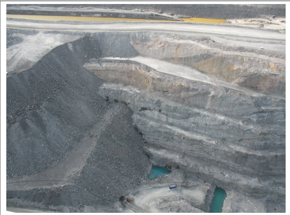
Photo #5 Wall of Portage Pit downstream of Central Dike
