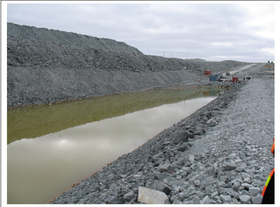
Photo #6 Seepage collection pond at toe of Central Dike
