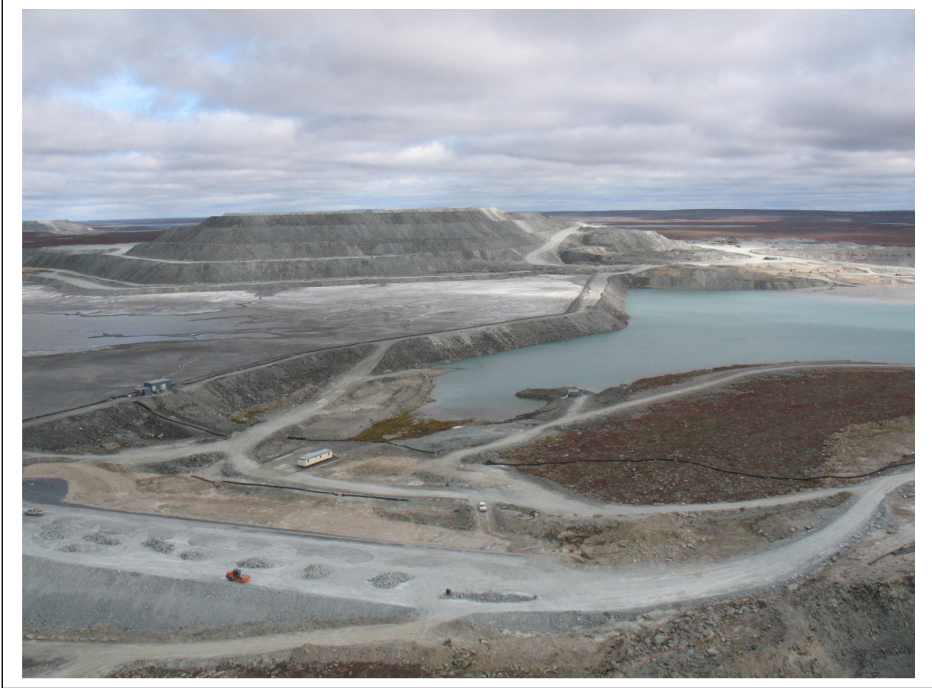
Photo #1 Stormwater dike
