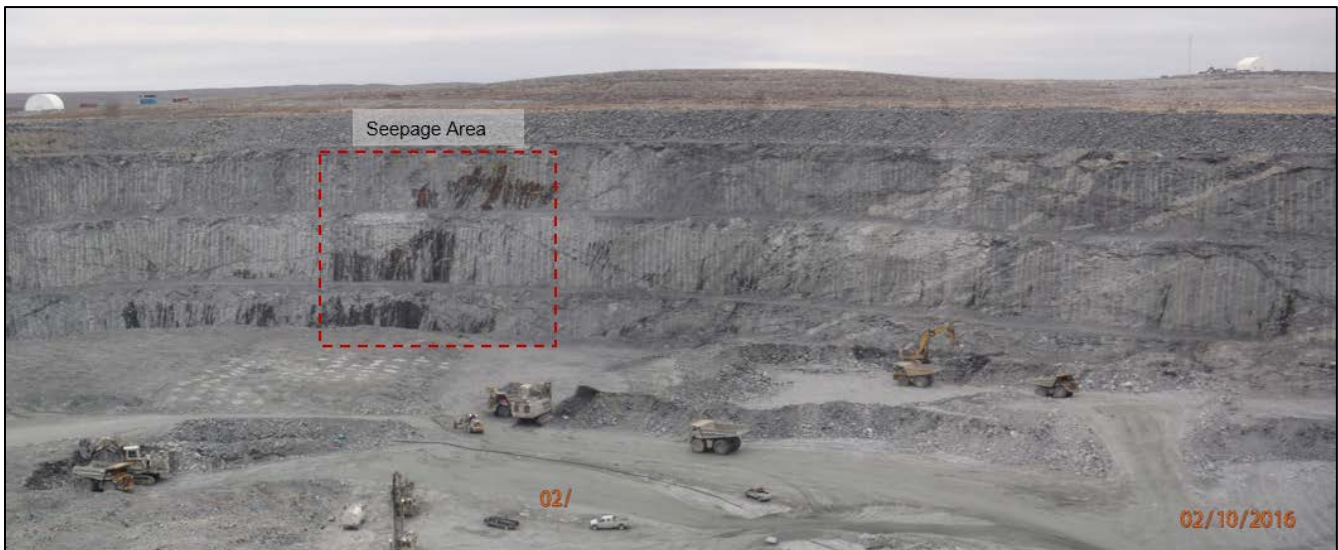
Photograph 8-10: Seepage from the southeast highwall near 2015 inflow
