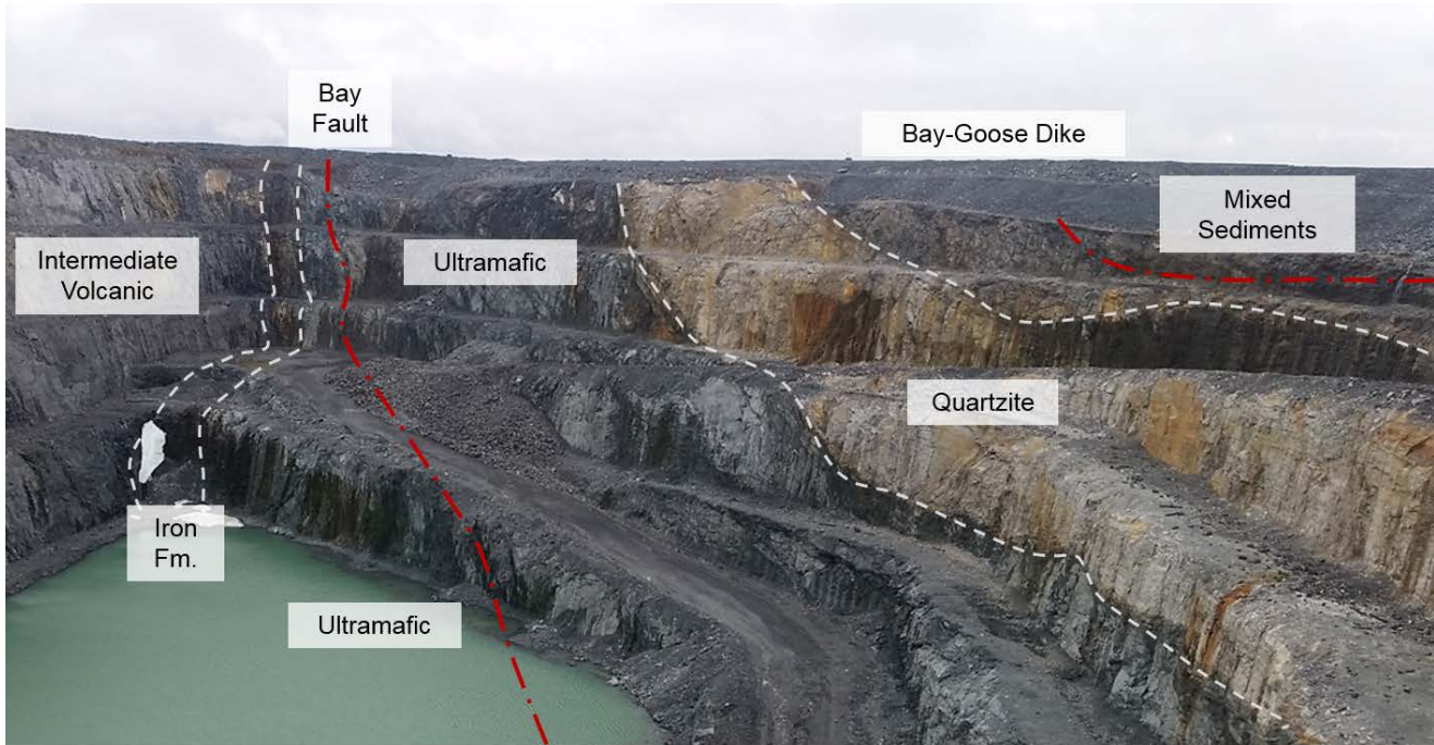
Photograph 7-2: Goose Pit south wall performance (September 2016)
