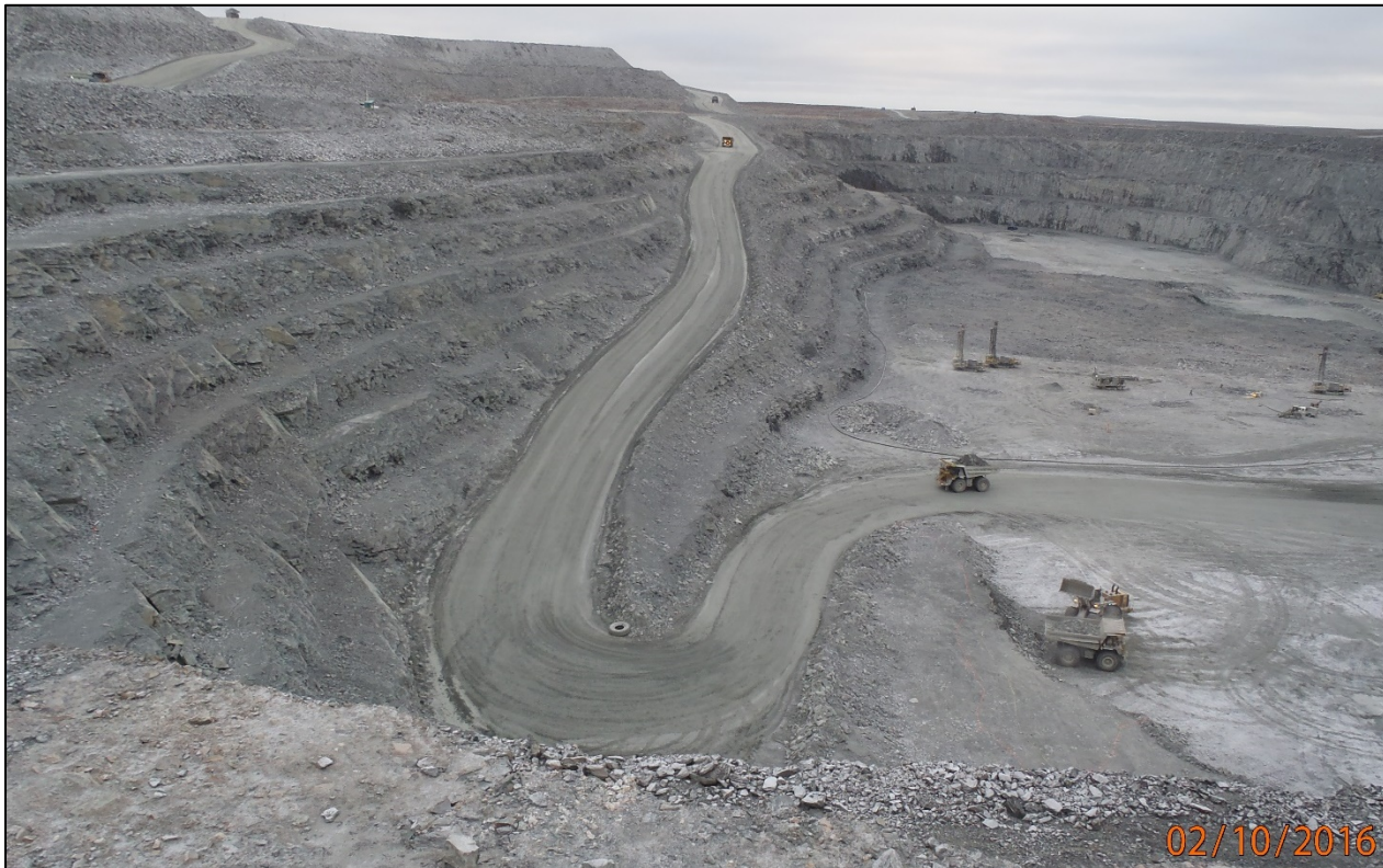
Photograph 8-1: Vault pit grid west footwall slope, south end of pit, looking north
