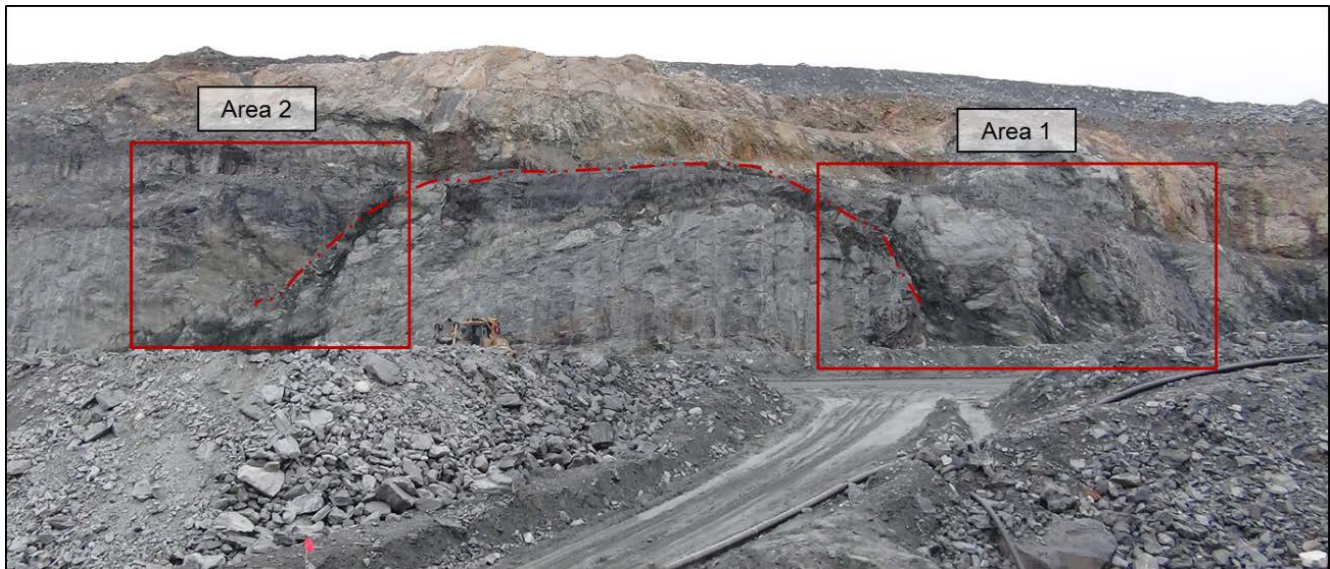
Photograph 6-9: Pit E3 Ramp Areas 1 and 2 - Bay Fault or splay (from 2015 inspection)
