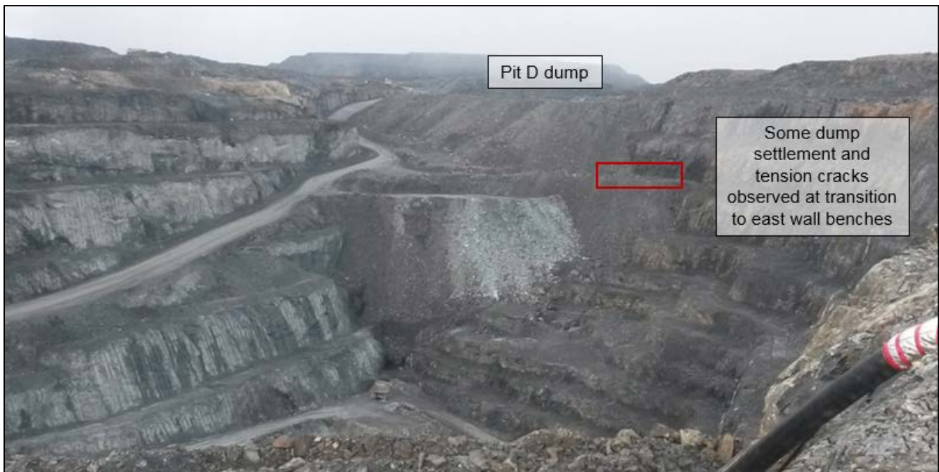
Photograph 5-2: Pit D dump, viewing north from crest of Pit E3 (2016)
