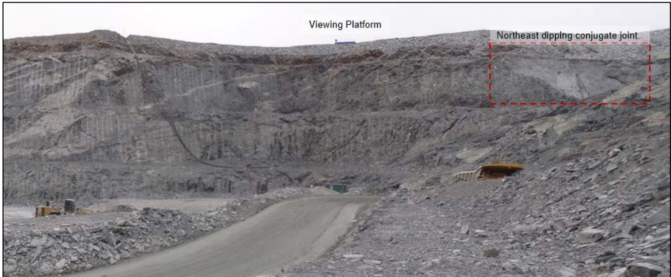
Photograph 8-5: Vault Pit grid south wall transition
