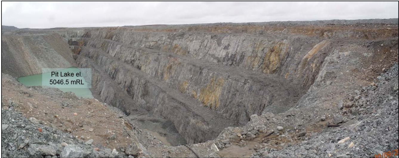
Photograph 7-1: Goose Pit east wall performance looking north (2016)
