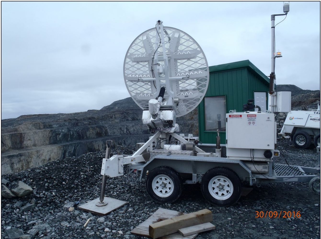
Photograph 4-10: GroundProbe radar monitoring the west wall of Pit A, from the east wall crest
