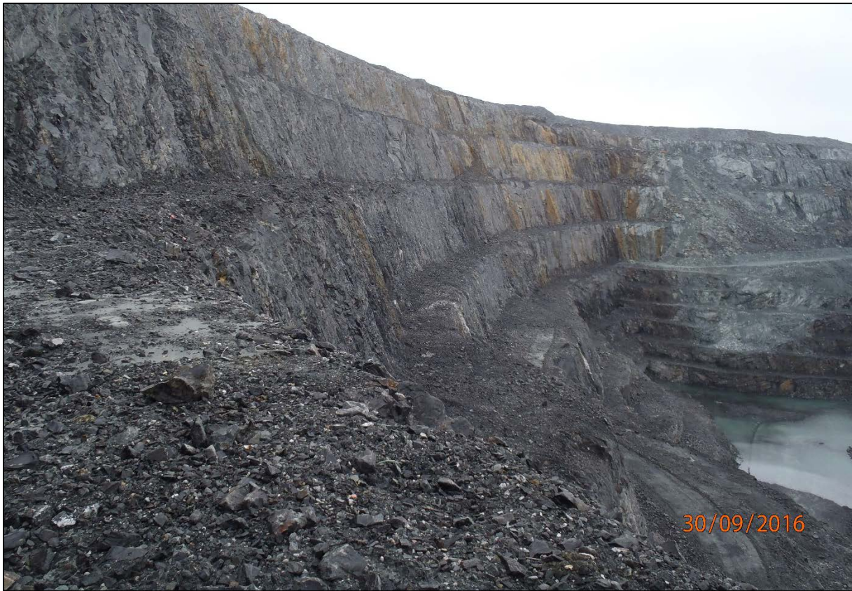
Figure 6-1: East wall showing good bench and wall performance (2016)
