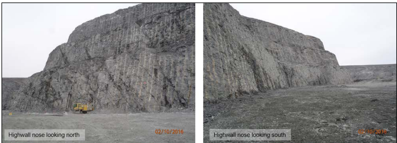
Photograph 8-12: Faults and widely spaced open joints dipping into nose of highwall
