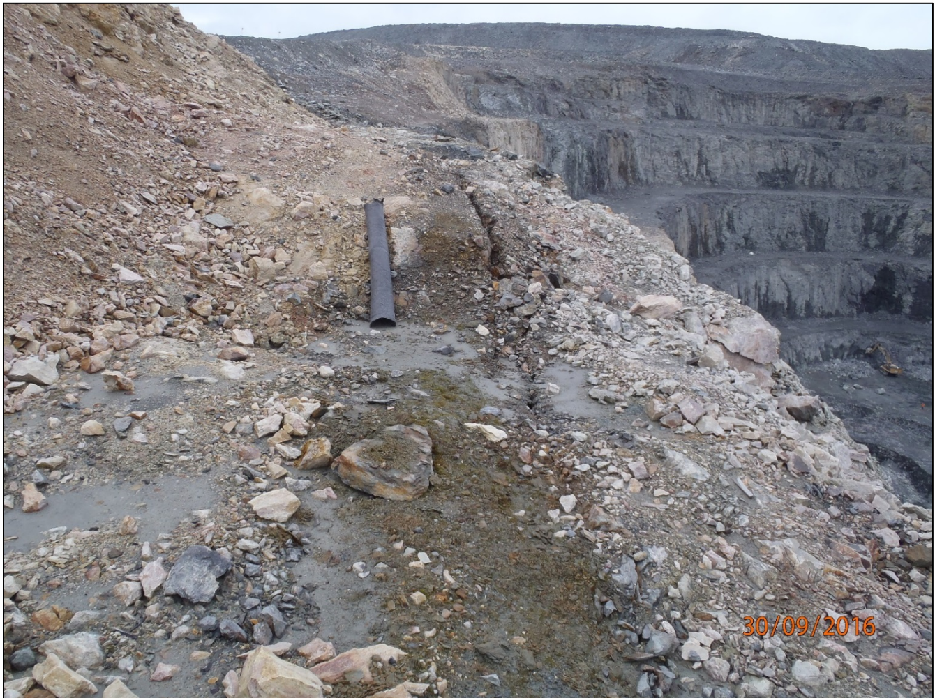
Photograph 4-9: Bench above Pit A 2016 rock fall showing formation of tension crack
