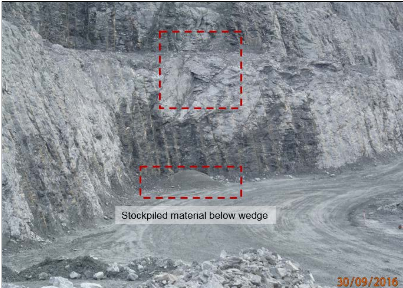
Photograph 4-15: Wedge above stockpiled material
