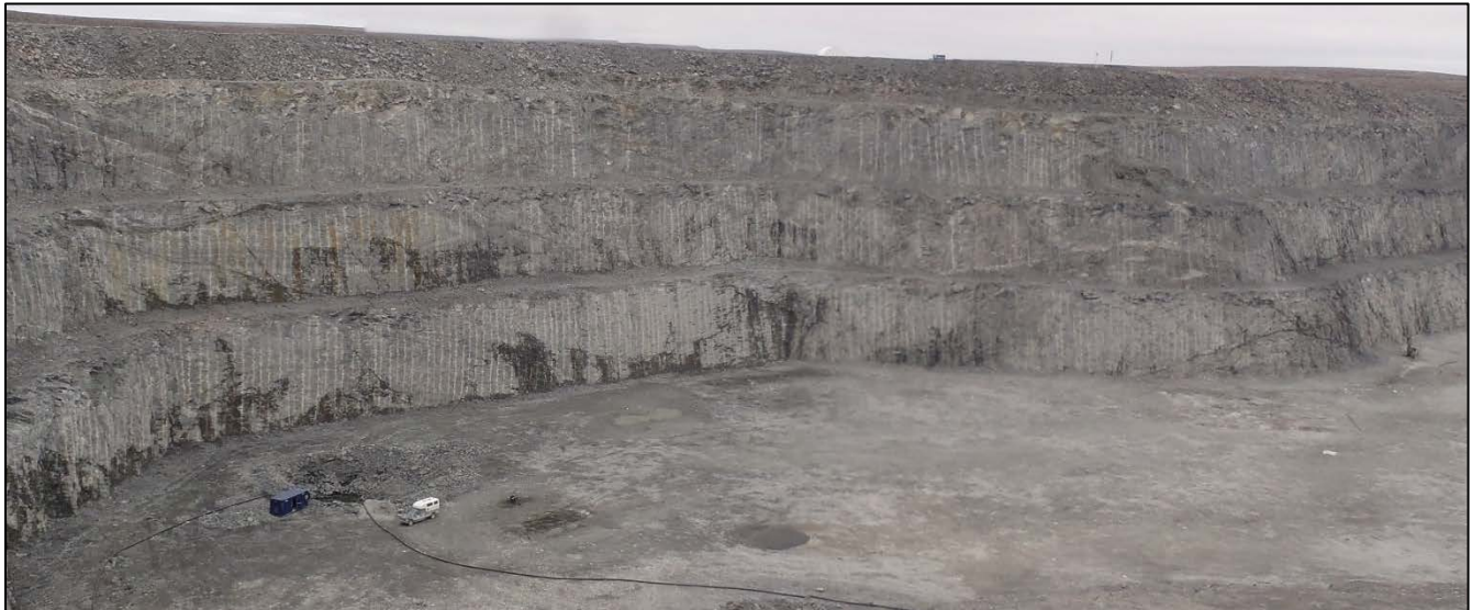
Photograph 8-13: Performance of northeast section of highwall
