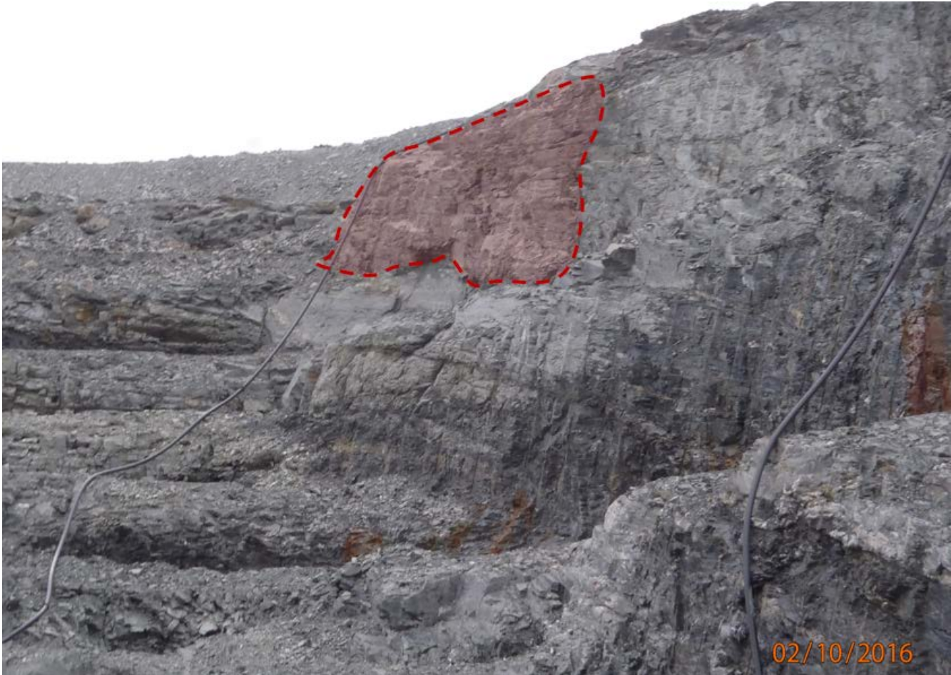
Photograph 8-24: Vault Pit north transition wall wedge
