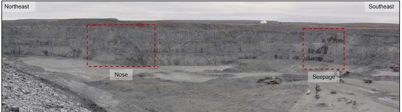
Photograph 8-7: Panaromic of highwall
