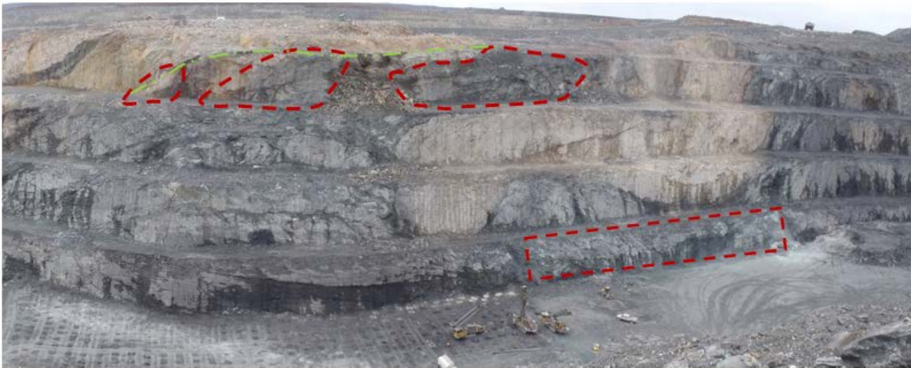
Photograph 4-11: Areas of potential bench-scale instability along the Pit A west wall
