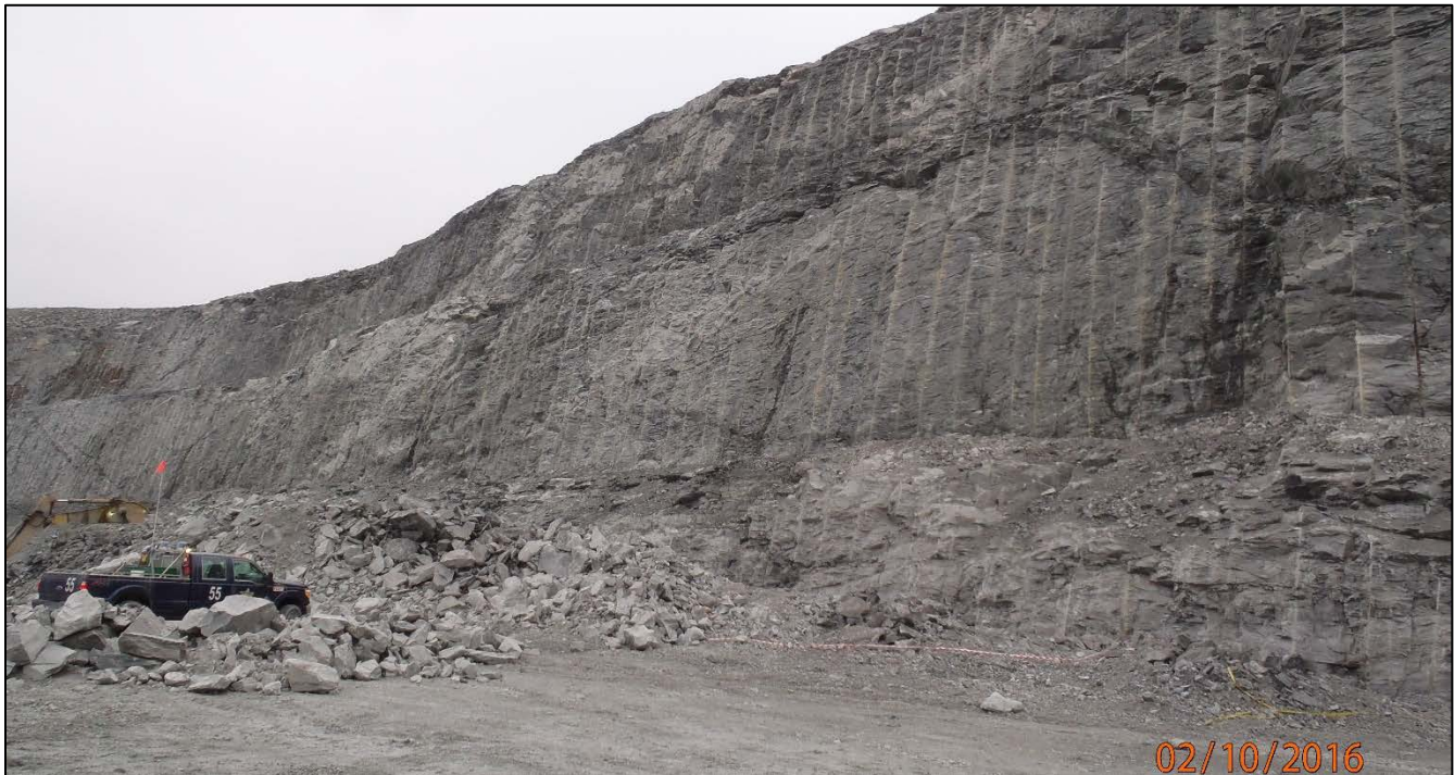
Photograph 8-9: Bench performance and visible half barrels on highwall
