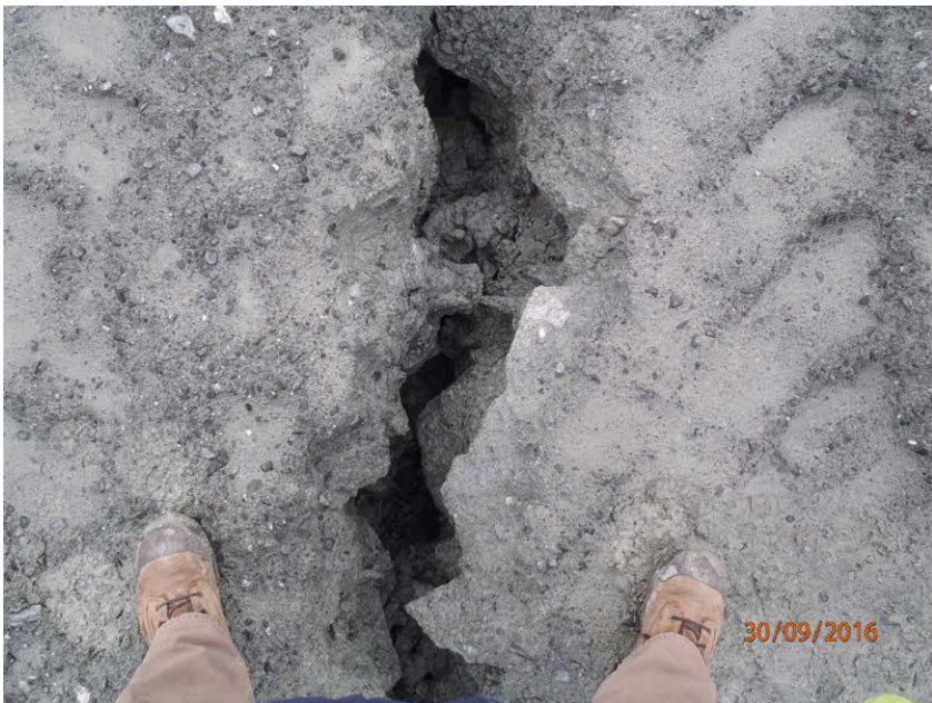
Photograph 7-6: Opening of tension cracks on dump platform (September 2016)
