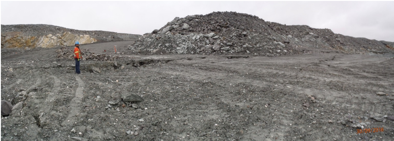
Photograph 7-5: Goose Pit dump crest and tension cracks, September 2016
