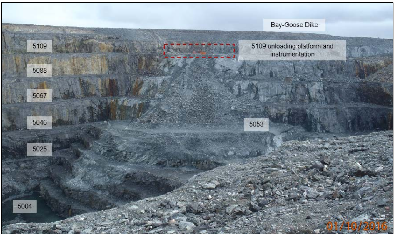
Photograph 6-3: Pit E3 south wall (2016)
