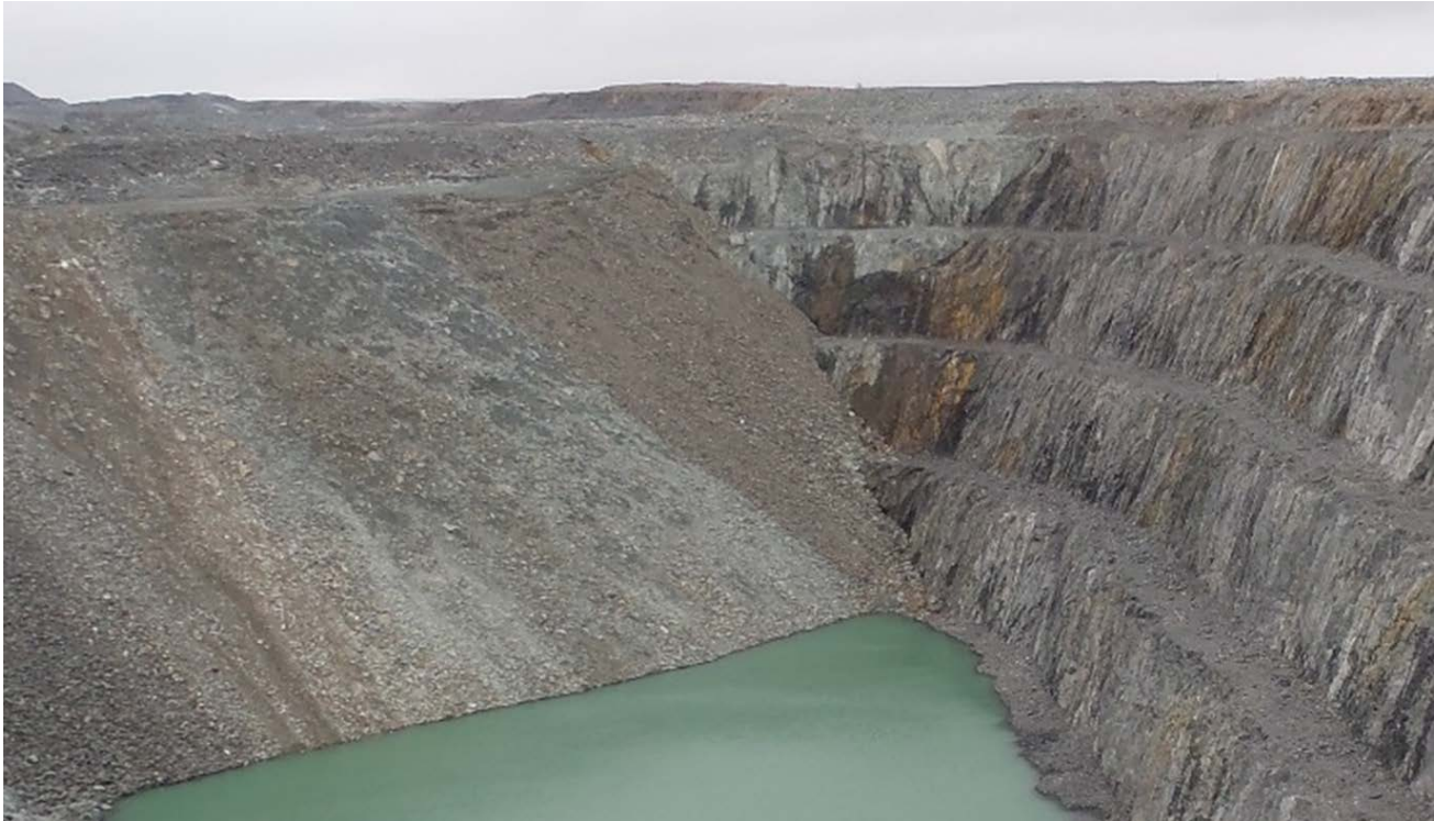
Photograph 7-7: Goose Pit north end wall (September 2016)
