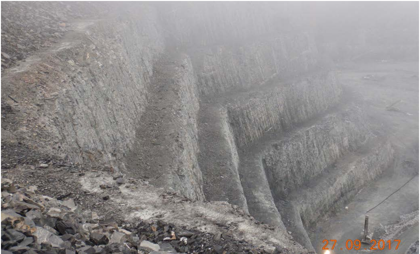
Photograph 8-9: Vault Pit east wall northeast end looking south (2017)
