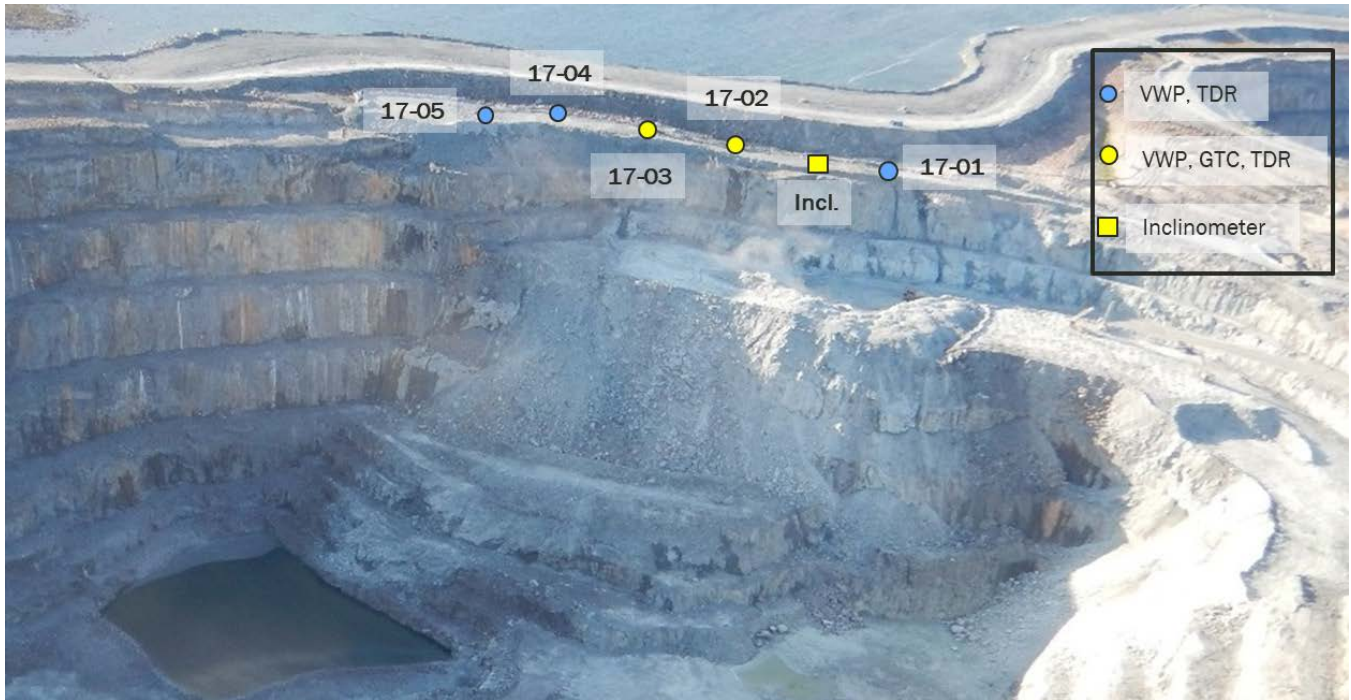
Photograph 6-10: Pit E south wall instrumentation locations
