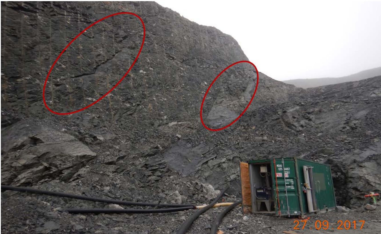
Photograph 8-6: Vault Pit sump and out-dipping planes
