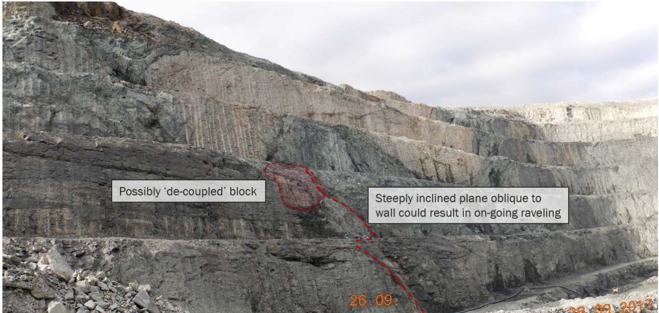
Photograph 4-4: Pit A lower west wall bench performance in iron formation
