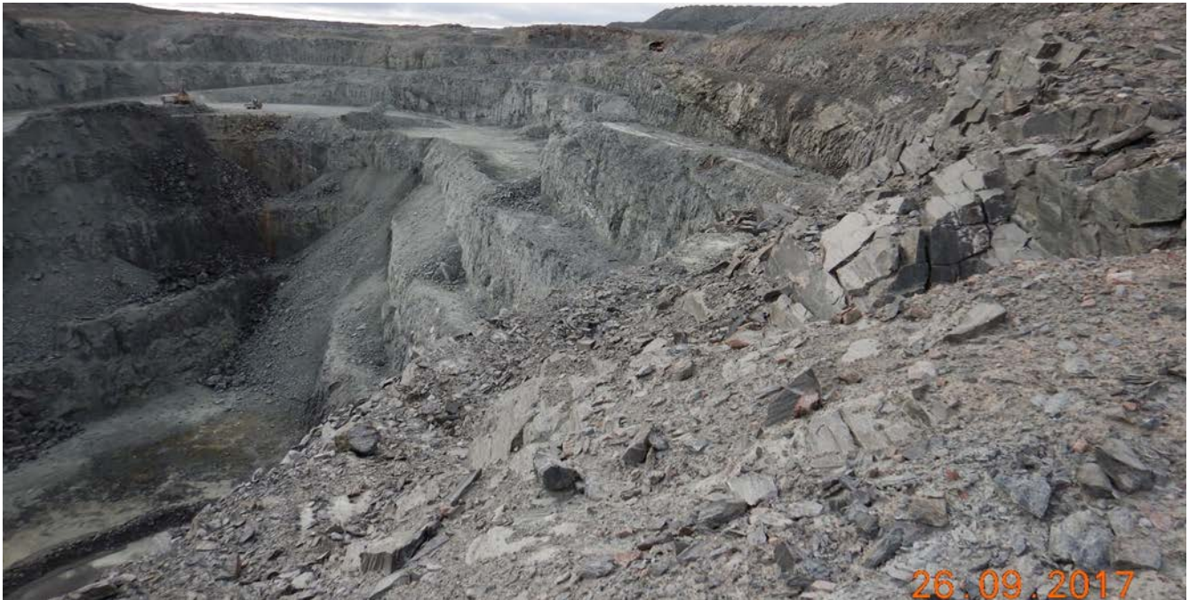
Photograph 6-12: Pit E west wall south end upper benches (2017)
