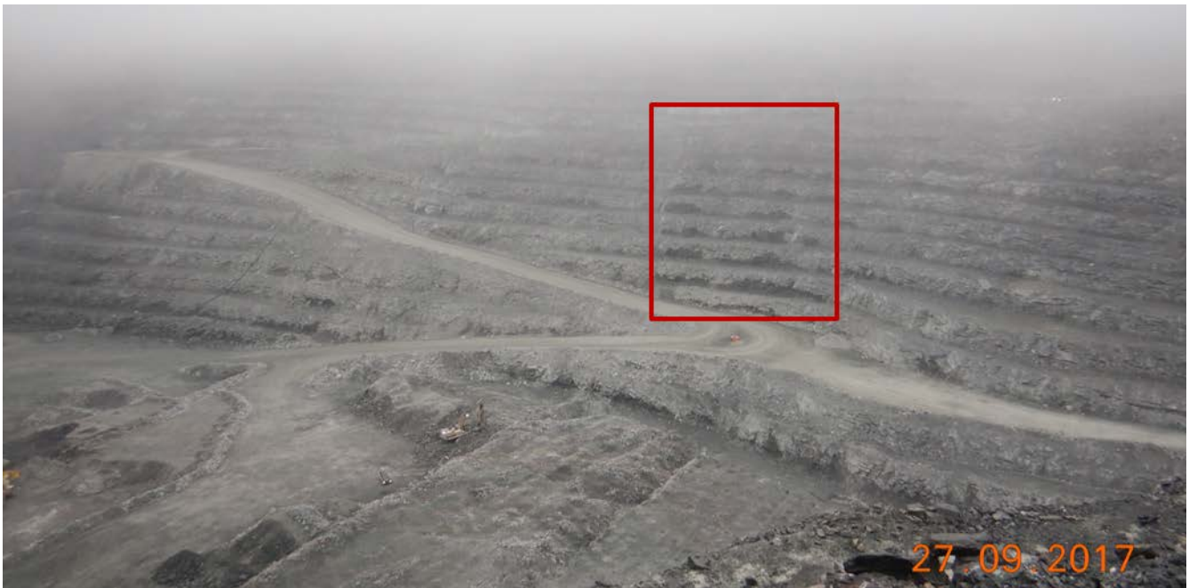
Photograph 8-3: Vault Pit west wall seepage
