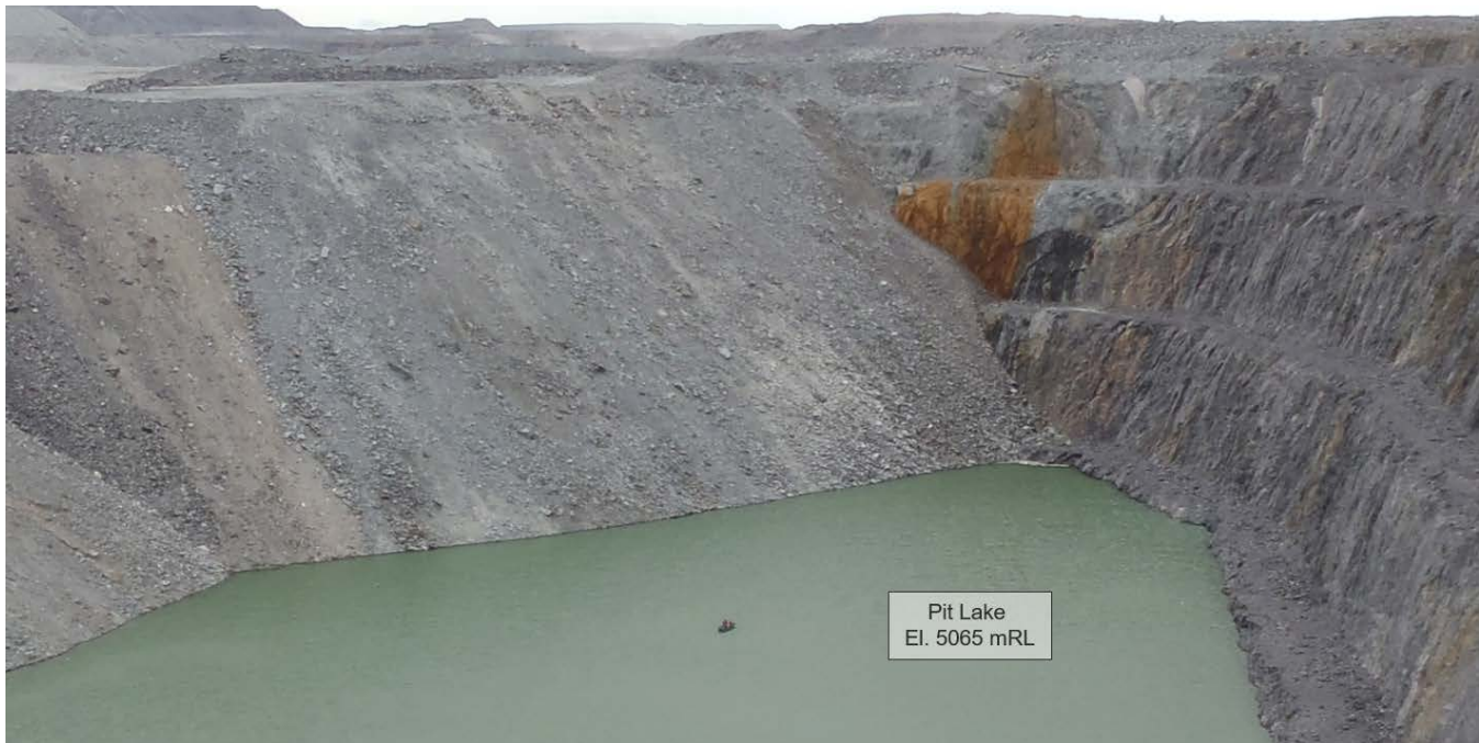
Photograph 7-5: Goose Pit northwest through northeast wall (north end wall 2017)
