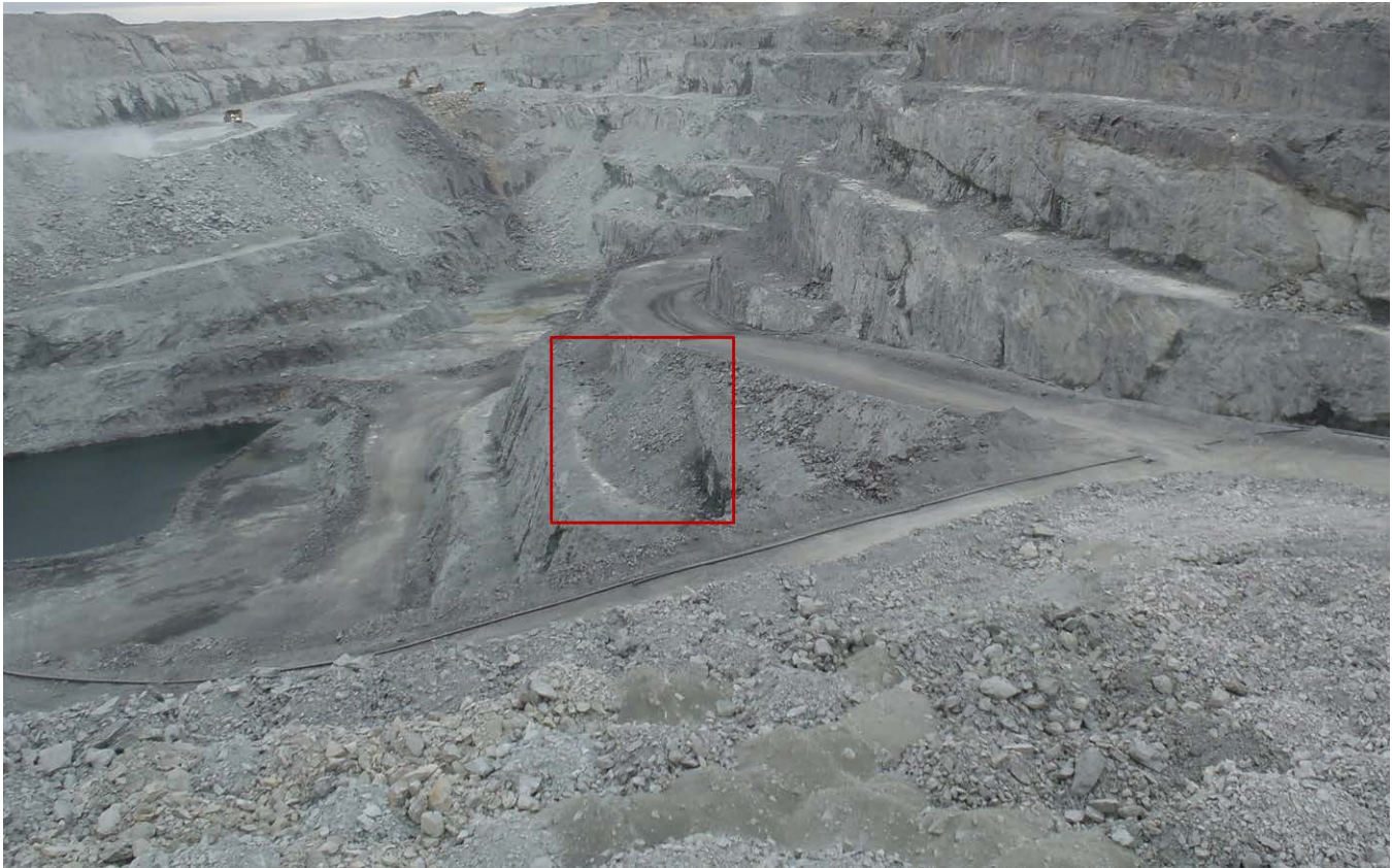
Photograph 6-21: Pit E west wall ramp buttress and step-in (2017)
