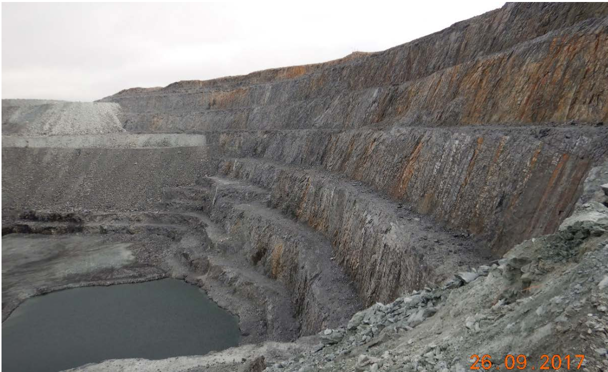
Photograph 6-3: Pit E east wall performance (2017)
