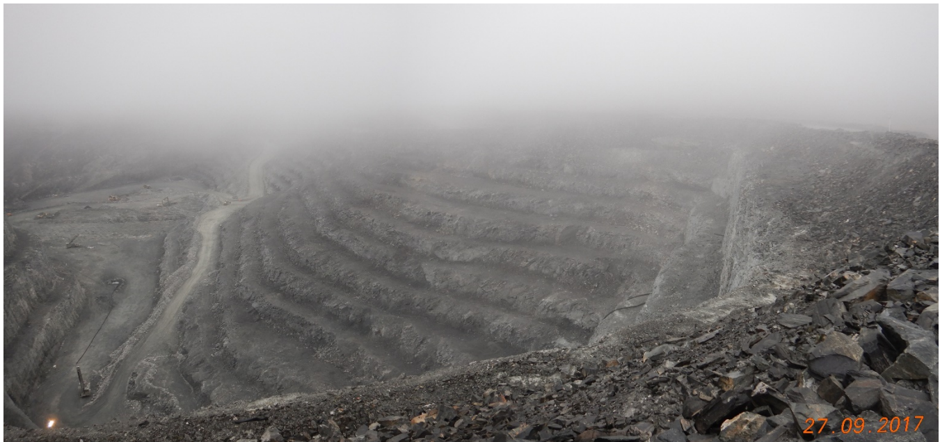
Photograph 8-2: Vault Pit west wall looking south (2017)
