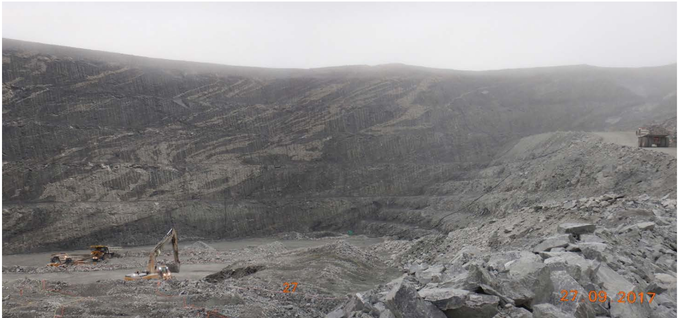
Photograph 8-4: Vault Pit grid south wall (2017)
