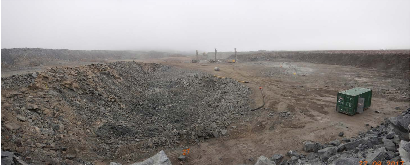
Photograph 8-18: Phaser Pit stripping (September 2017)
