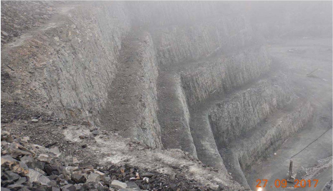
Photograph 8-14: Vault Pit northeast wall bench performance (2017)
