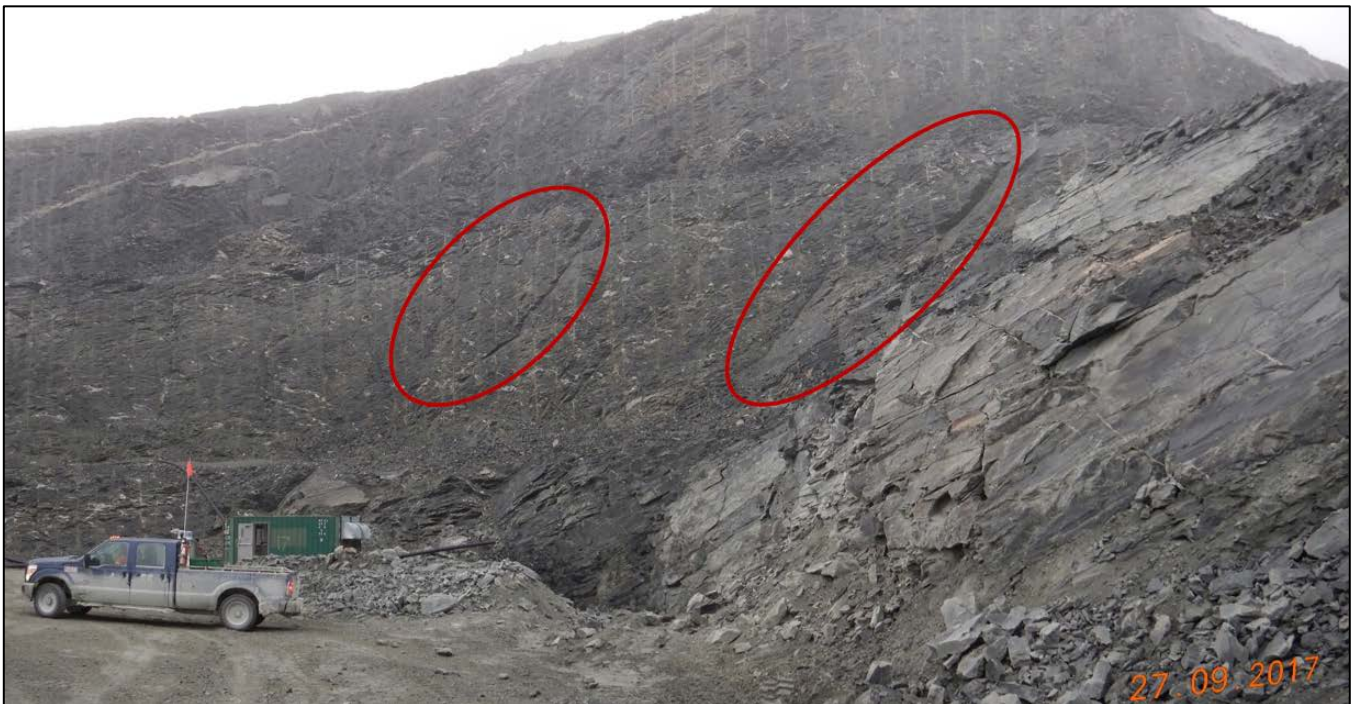
Photograph 8-5: Vault Pit south ramp sump and out dipping planes
