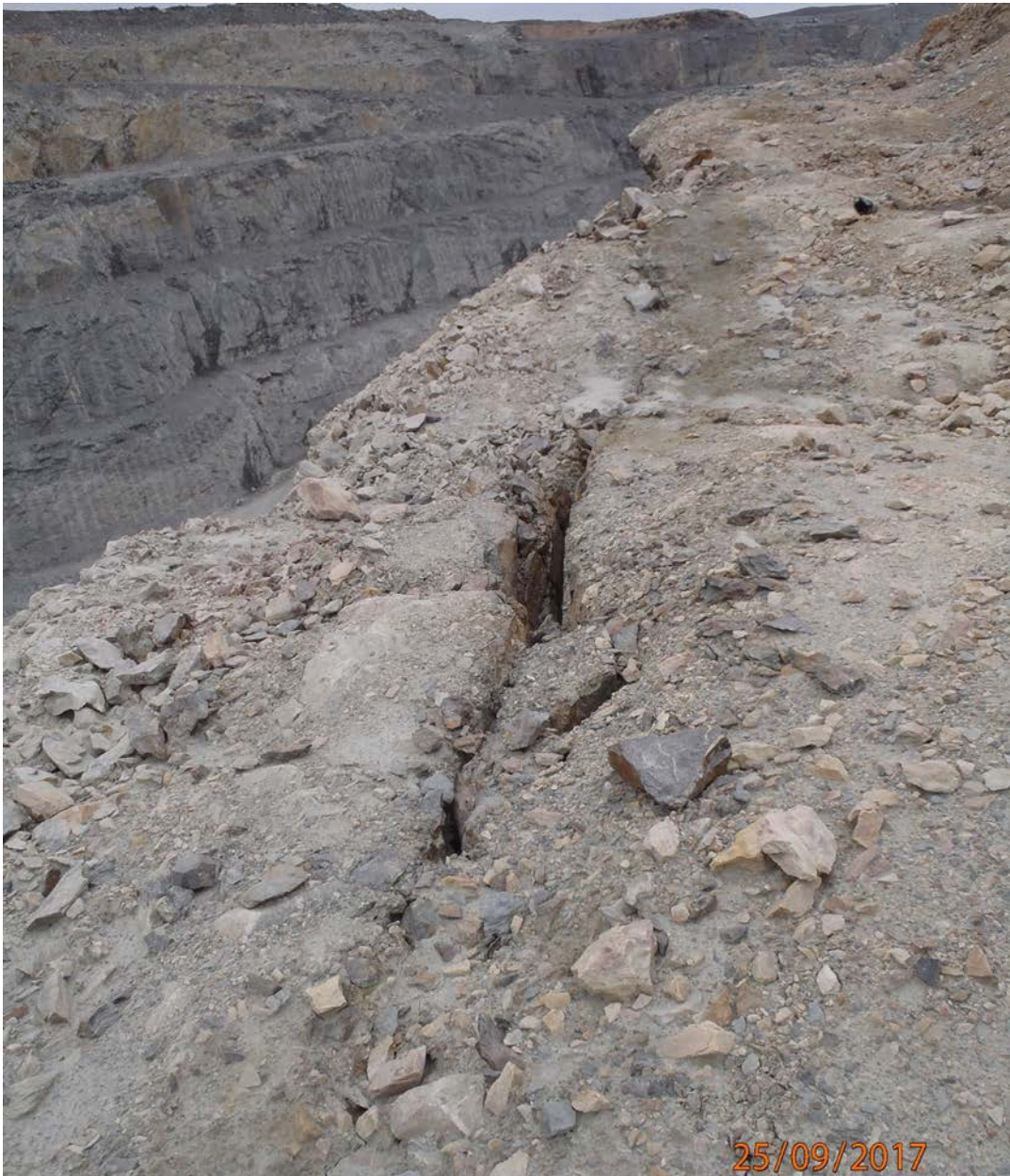
Photograph 4-6: Bench above 2016 rock fall showing tension crack
