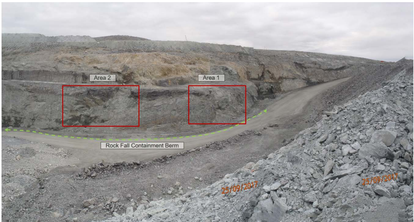
Photograph 6-13: Pit E west wall ramp areas of potential instability (2017)
