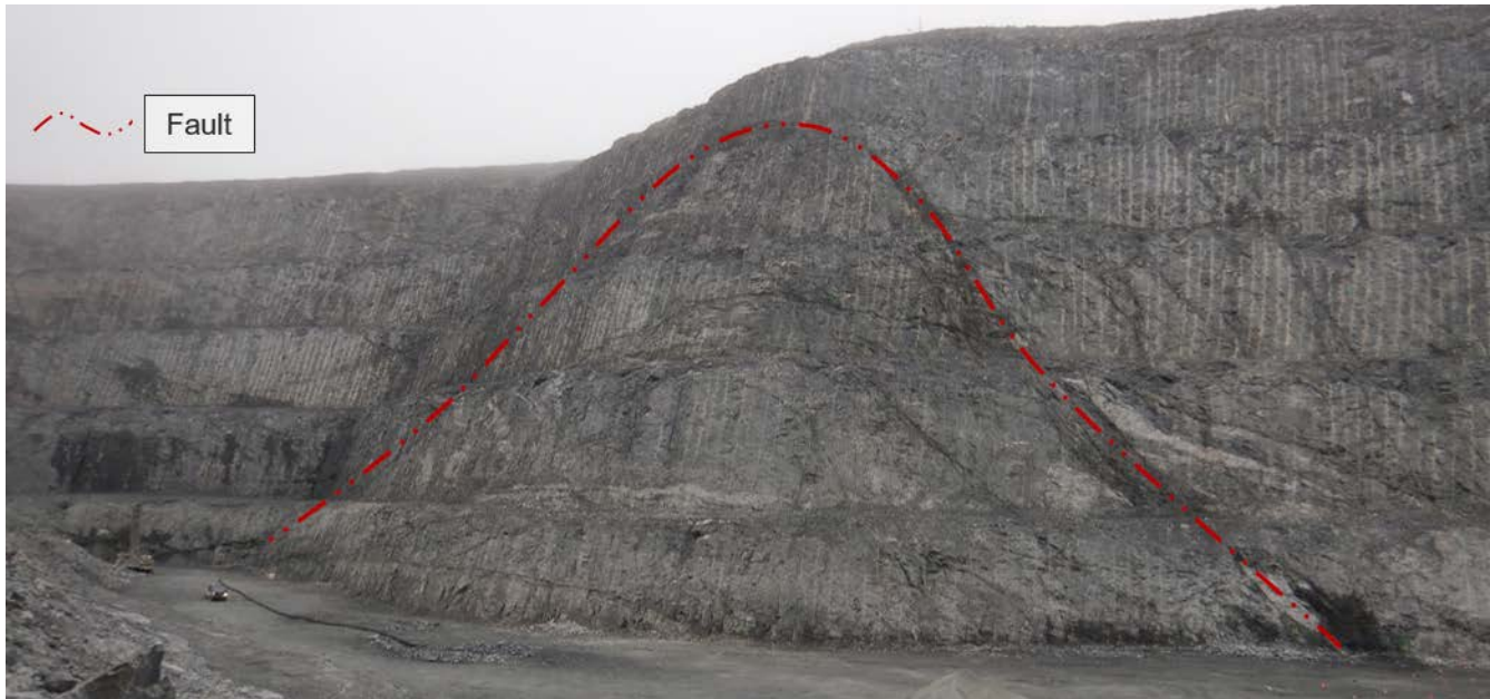
Photograph 8-13: Vault Pit east highwall nose, fault, and widely spaced open joints
