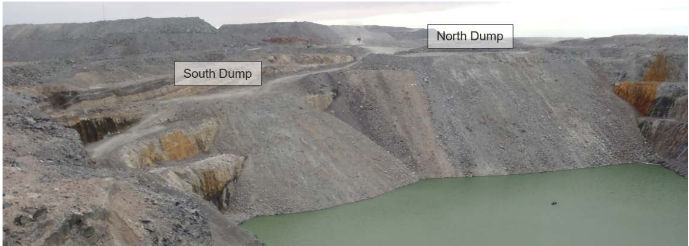
Photograph 7-4: Goose Pit waste rock dumps (2017)
