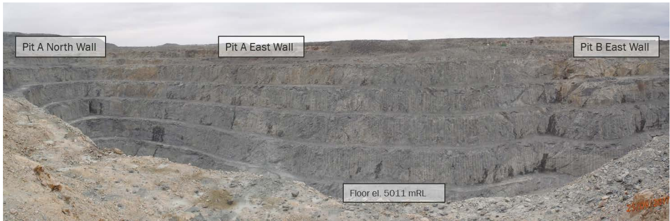
Photograph 4-2: Pits A and B looking north from west crest (2017)
