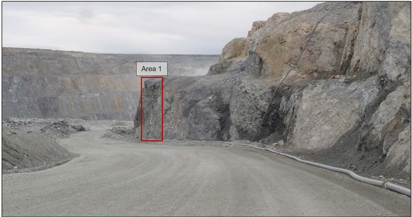
Photograph 6-15: Pit E Ramp Area 1 above ramp - Bay Fault or splay (2017)
