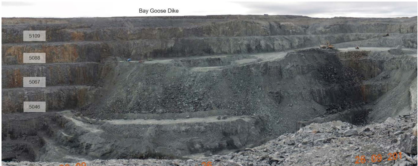
Photograph 6-4: Pit E south wall (2017)
