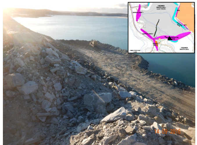
Figure 15: Buttress construction continues (September 14, 2016).
