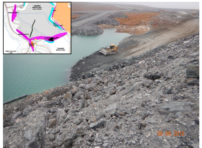
Figure 8: Advancement of the first lift of rockfill for the buttress (September 9, 2016).
