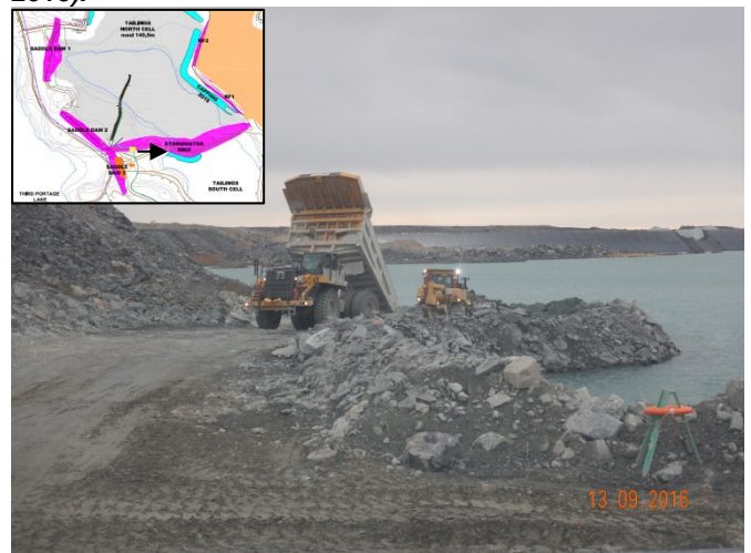
Figure 14: View of the buttress construction (September 13, 2016).
