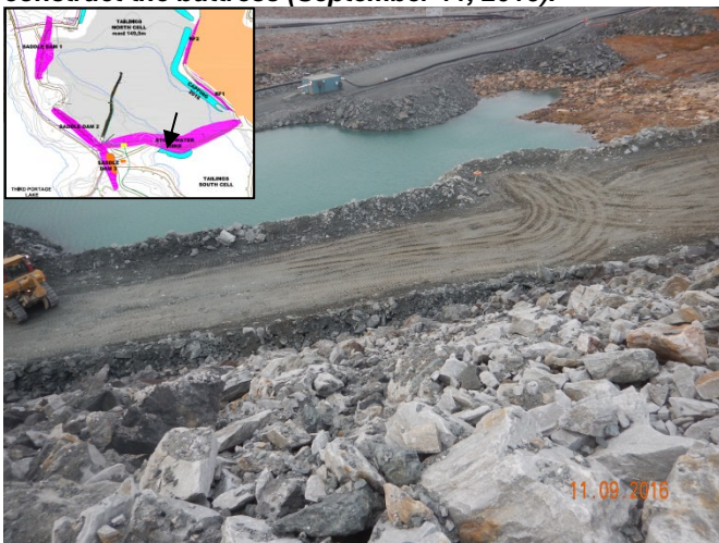
Figure 11: View of the buttress progress (September 11, 2016).
