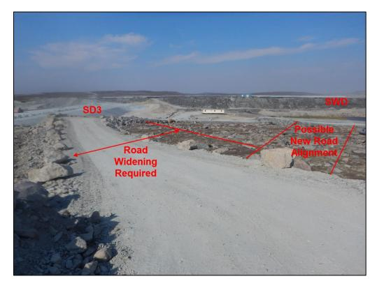
**Figure 3:** Road widening will be required on the Saddle Road as it turns toward Saddle Dam 3 since currently the road width is only enough for light vehicles. A new road could also be constructed to reduce the length of the hauling route, as seen on the right-hand side of the photo.
