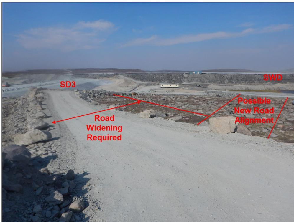
**Figure 3:** Road widening will be required on the Saddle Road as it turns toward Saddle Dam 3 since currently the road width is only enough for light vehicles. A new road could also be constructed to reduce the length of the hauling route, as seen on the right-hand side of the photo.
