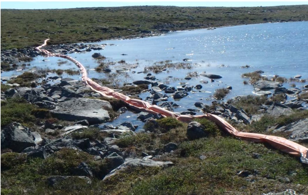
Figure 2-11: Turbidity barriers at the inlet of Dogleg Lake
