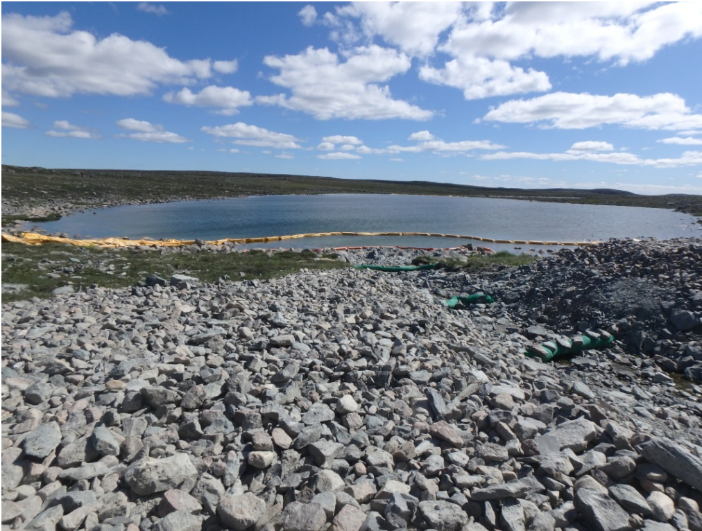
Figure 2-10: Turbidity barriers at inlet of NP1 installed in July 2016
