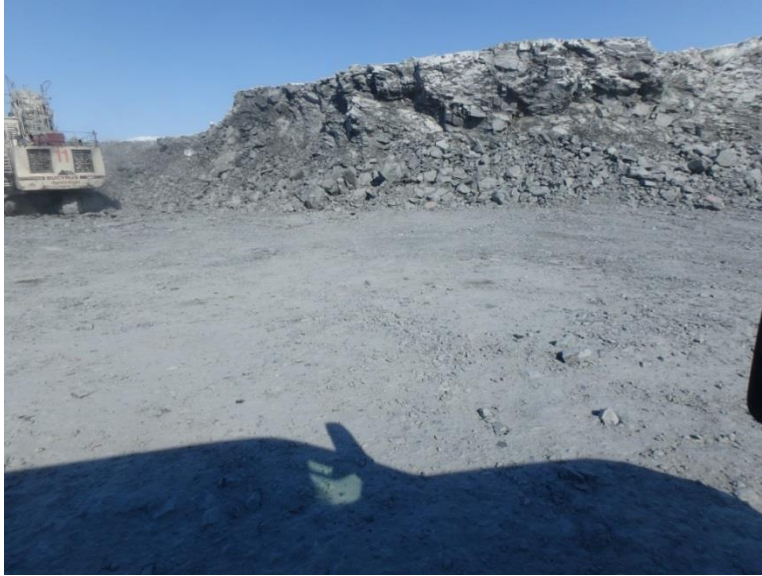
Area after clean-up
