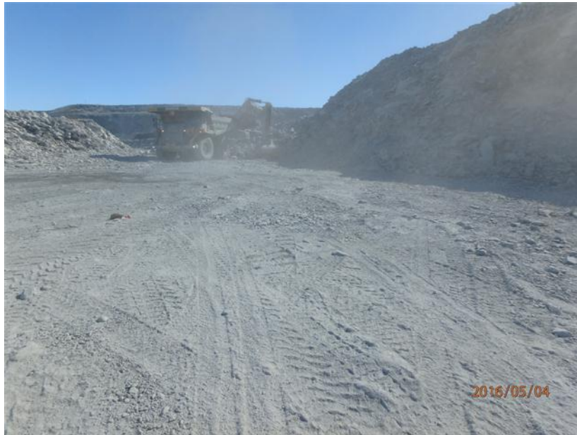
Area after clean-up
