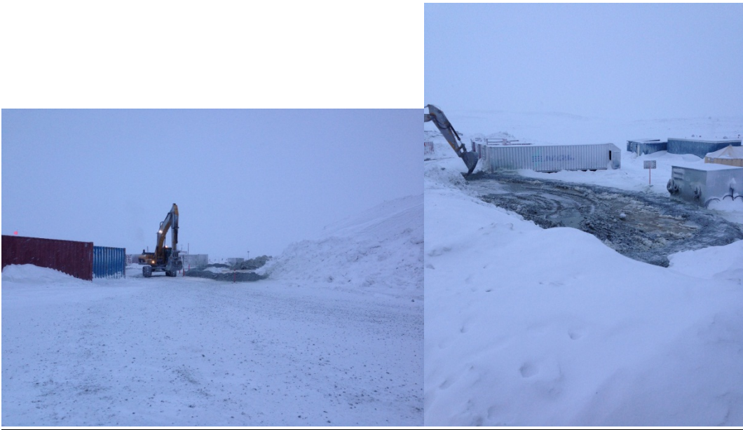
Photos 3-4- Berms constructed to contain the water/grease, 2 locations (January 4 th , 2016)
