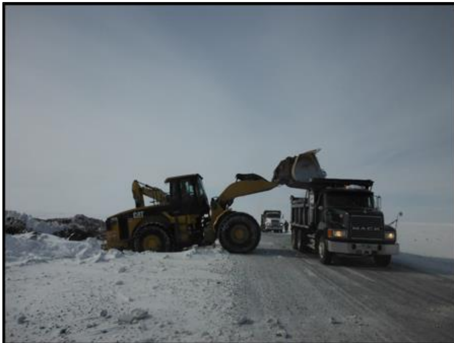
April 20: Loading trucks.
