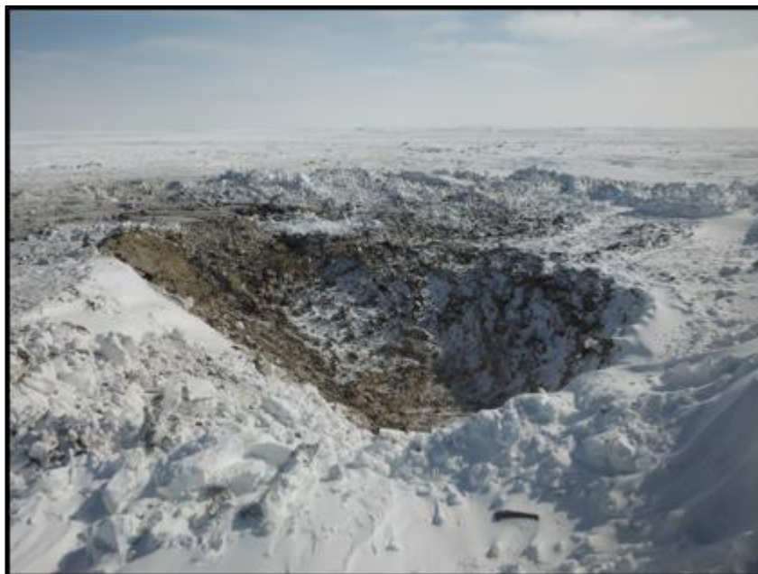
April 22: Final excavation boundary.
