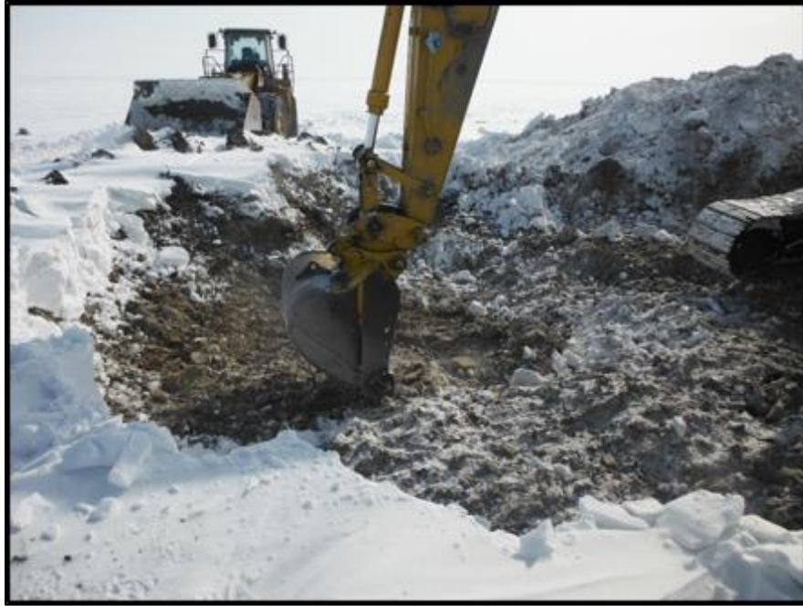
April 20: Excavation activities.
