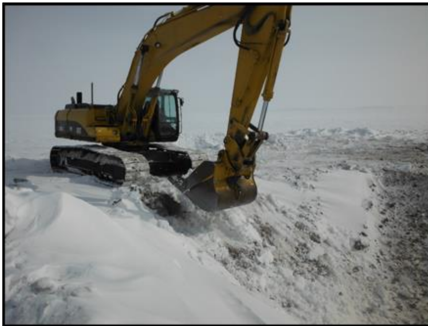
April 21: Removing snow from excavation for confirmatory sampling.
