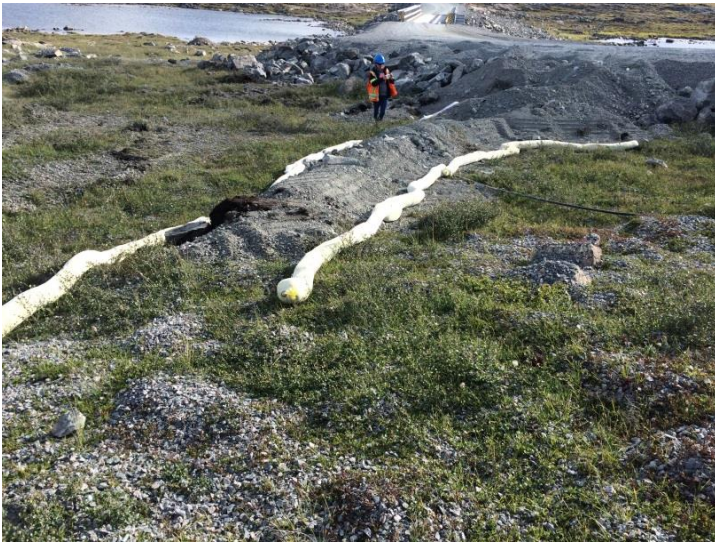
Berm and chemical booms
