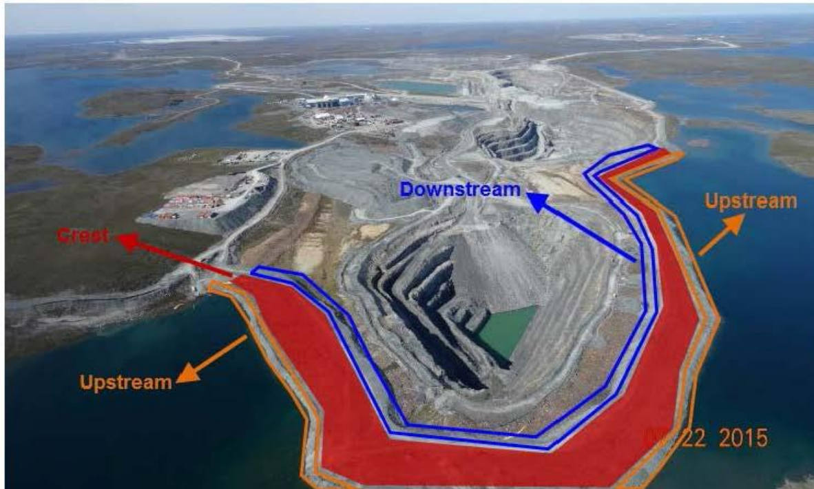
Aerial view of the Goose Bay Dike
