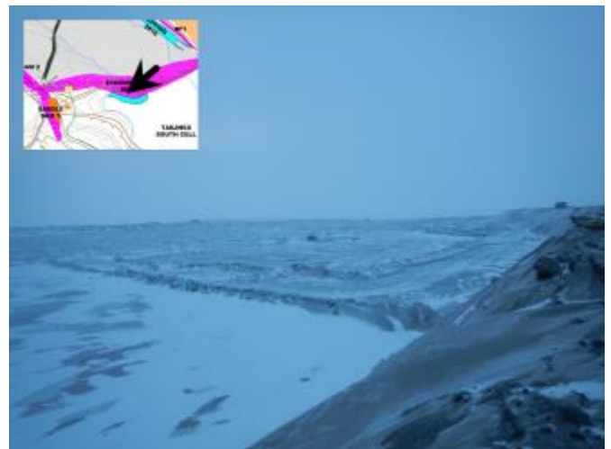
Photo 11: General view of the completed internal structure (November 10, 2017).
