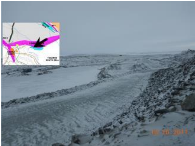
Photo 3: Access area of internal structures over Stormwater Dike 2016 buttress (October 18, 2017).
