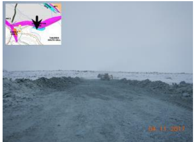
Photo 6: View on the platform towards the end of the structure (November 4, 2017).
