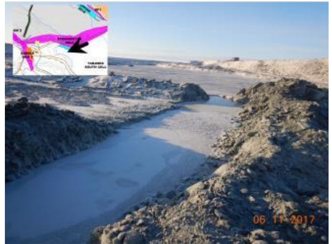
Photo 10: View of the completed trenching (November 6, 2017).
