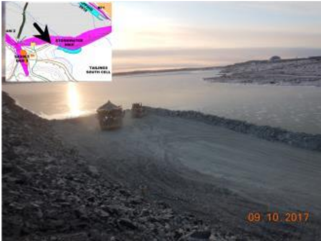
Photo 1: Placement of rockfill over 2016 Stormwater Dike buttress (October 9, 2017).
