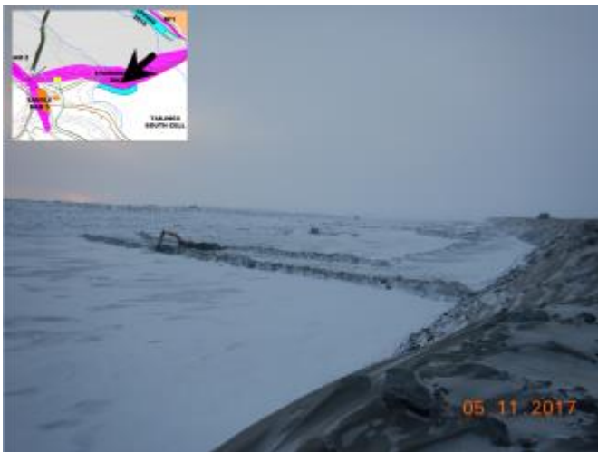
Photo 8: Backhoe working on the first trench (November 5, 2017).
