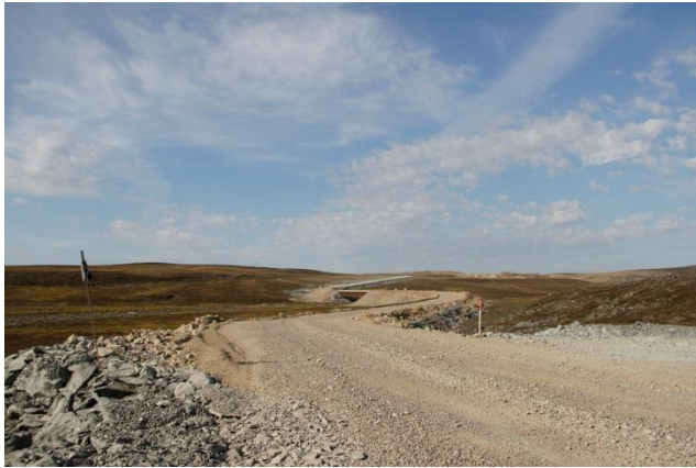
Photo 32: Bridge #2 along the Amaruq single-lane road
