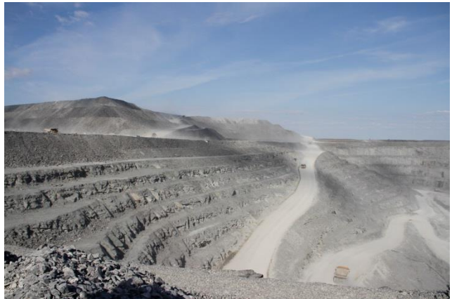
Photo 21: Vault Pit in 2017
