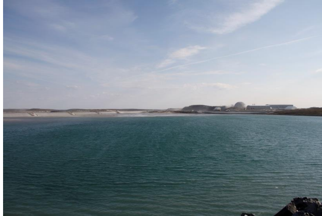
Photo 41: Tailings Storage Facility (South Cell)
