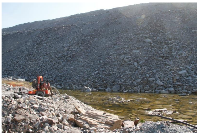
Photo 36: Seepage from the Portage waste rock storage facility
