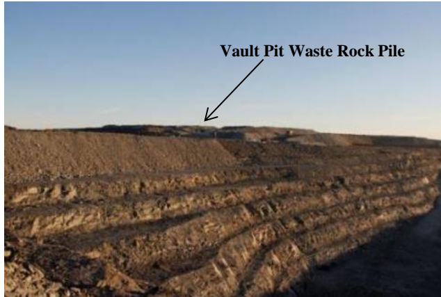
Photo 27: Vault Pit waste rock storage facility in 2015
