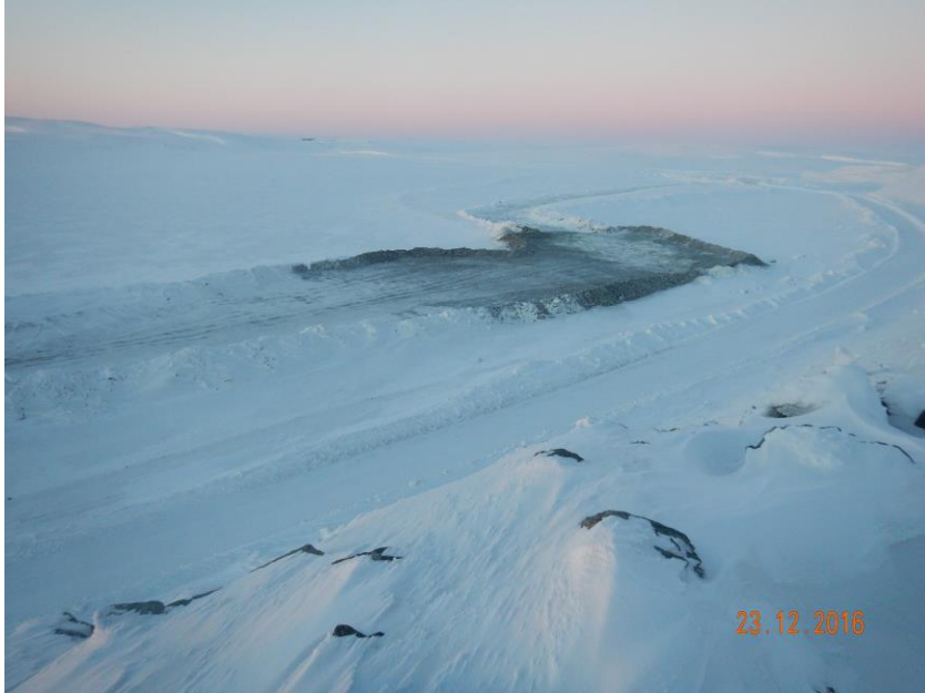
Photos 1: 2016 TSF Cover Construction
