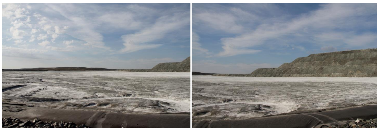
Photo 40: Tailings Storage Facility (North Cell)
