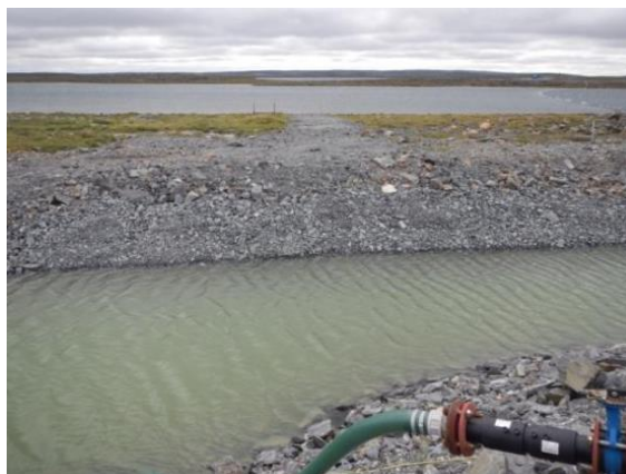
Photo 38: Trench below Assay Laboratory to prevent water from entering lake
