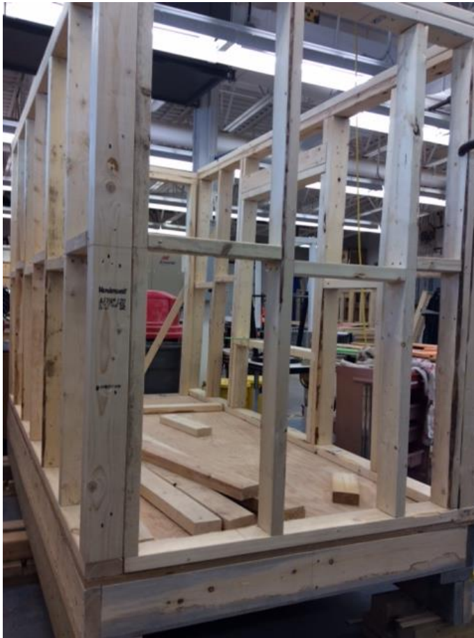
Figure 36. Cabin being built by carpentry students of Jonah Amitnaaq Secondary school with recycled wood.
