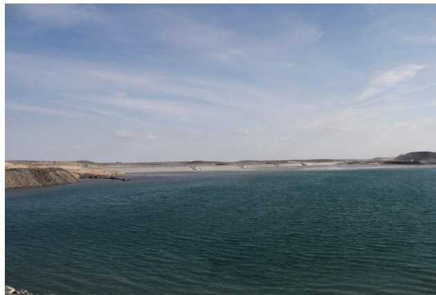
Photo 42: Raising the height of Saddle Dam
