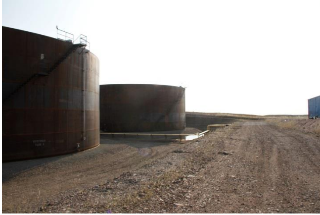
Photo 47: Baker Lake Fuel Tank Farm Facility
