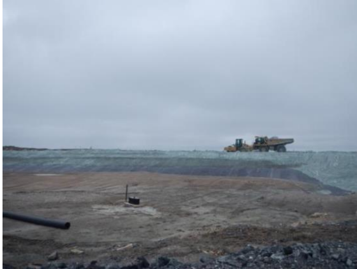
Photo 28: Raising the height of Saddle Dam 3
