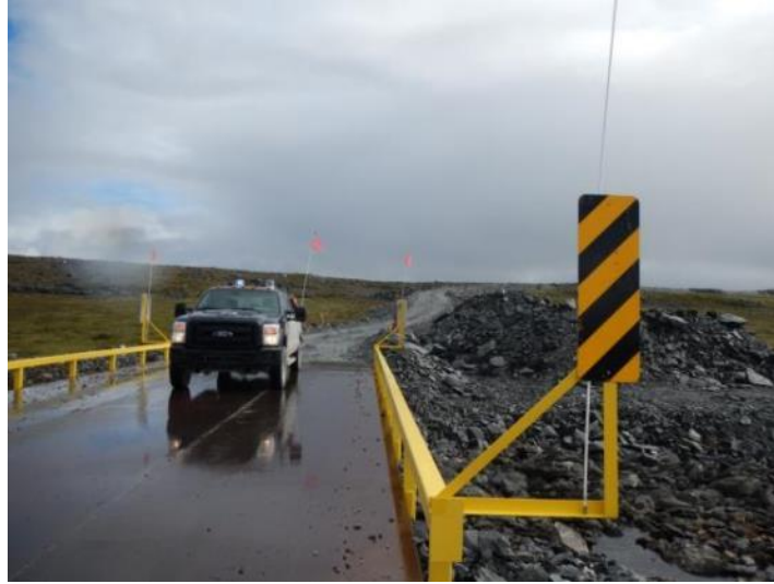
Photo 20: Bridge #1 along the Amaruq single-lane road
