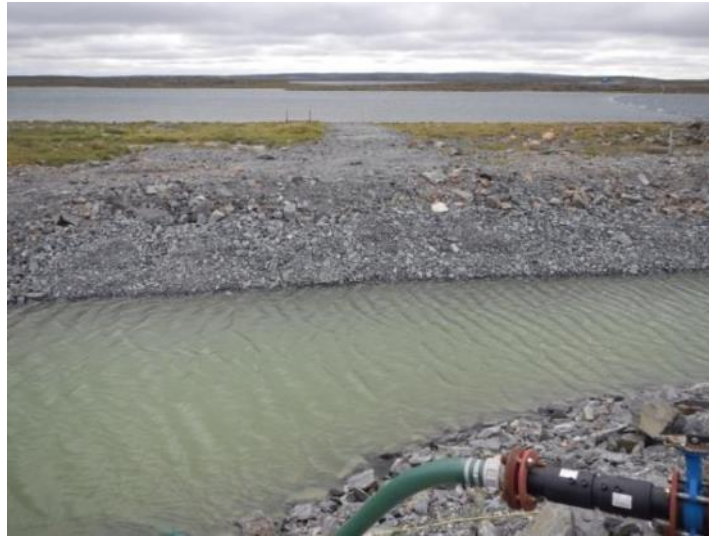
Photo 24: Trench below Assay Laboratory to prevent water from entering lake
