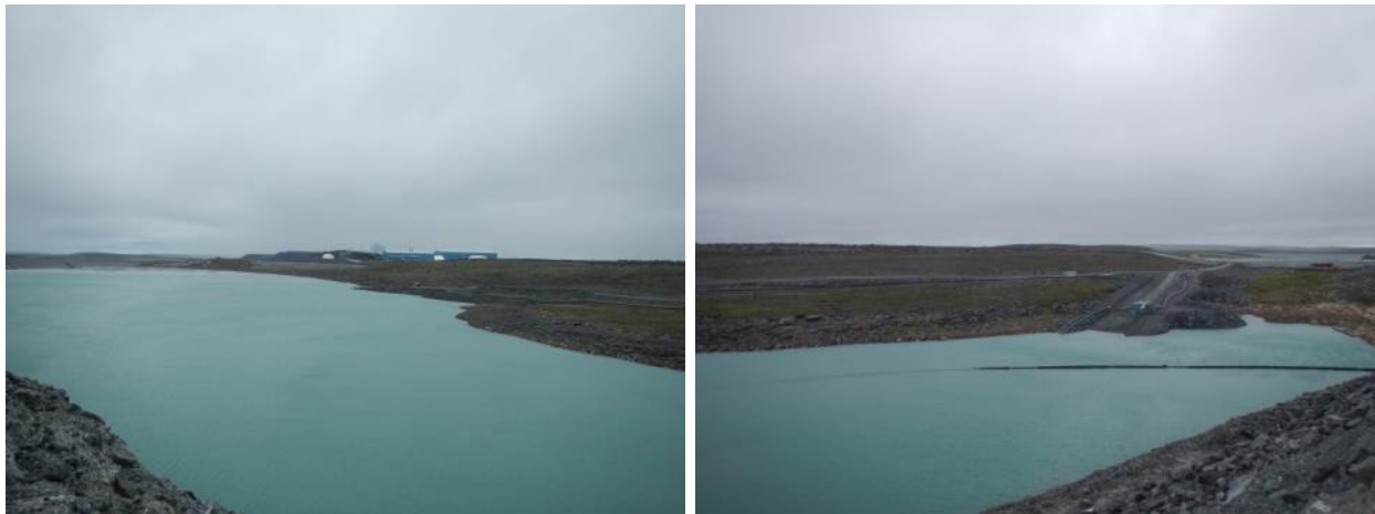
Photo 27: Tailings Storage Facility (South Cell)
