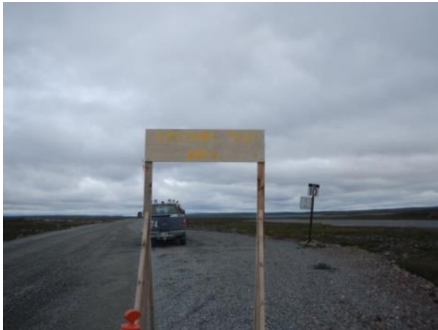
Photo 45: Dust test study area number one located near km 10: use of TETRA flakes
