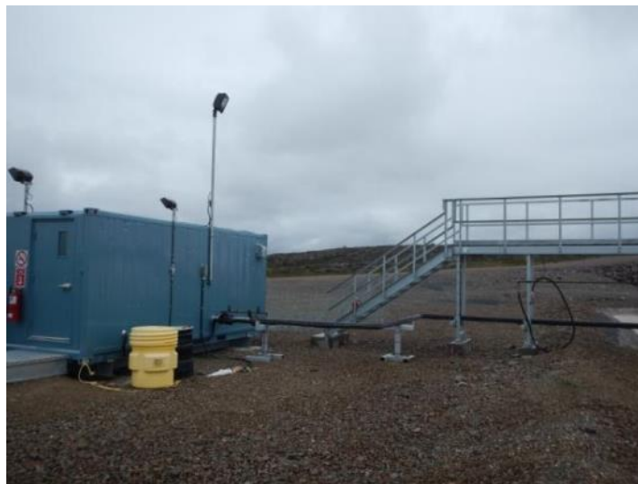
Photo 37: Refuelling station at the Baker Lake Fuel Tank Farm with Spill Containers in place
