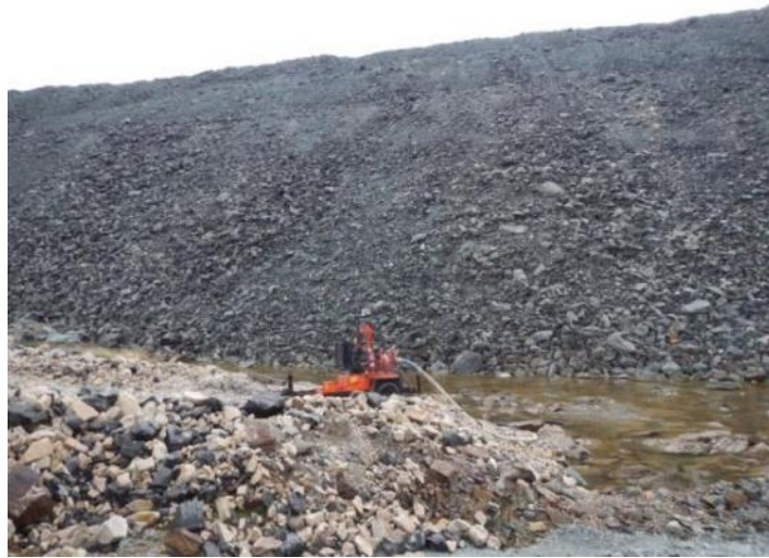
Photo 22: Seepage from the Portage waste rock storage facility
