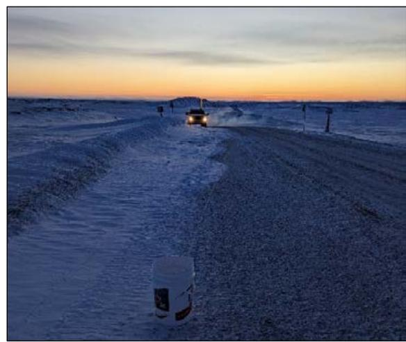
**Photo 2.4-1: Highest snowbanks measurements at Site SB3 indicating gentle slopes, December 9, 2022.**
