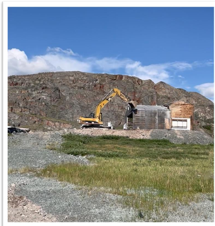
Figure 2-2: Excavator dismantling the Utility Building – July 14, 2022
