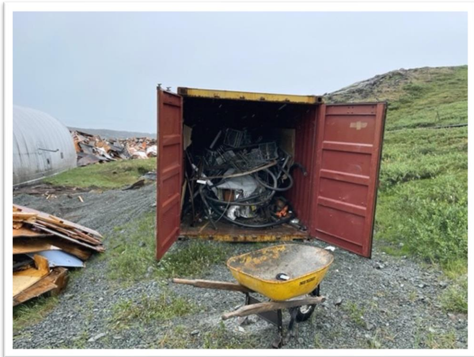
Figure 2-5: Material segregated – High value recyclable including Electrical fixtures and wires – July 18, 2022
