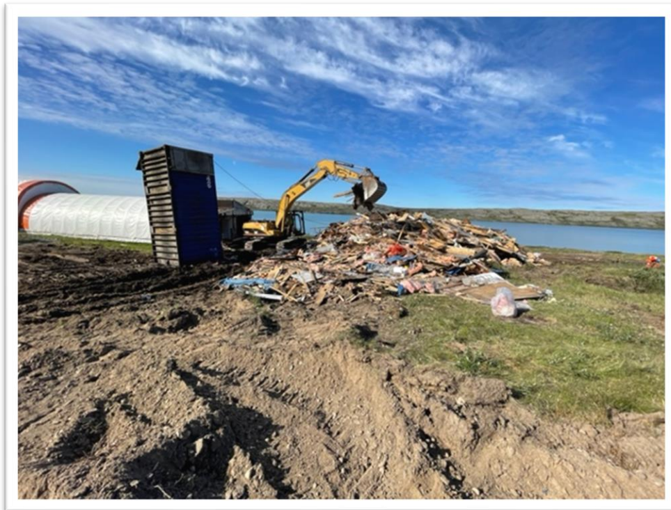
Figure 2-6: Construction debris loaded in sea containers for disposal down south – July 21, 2022
