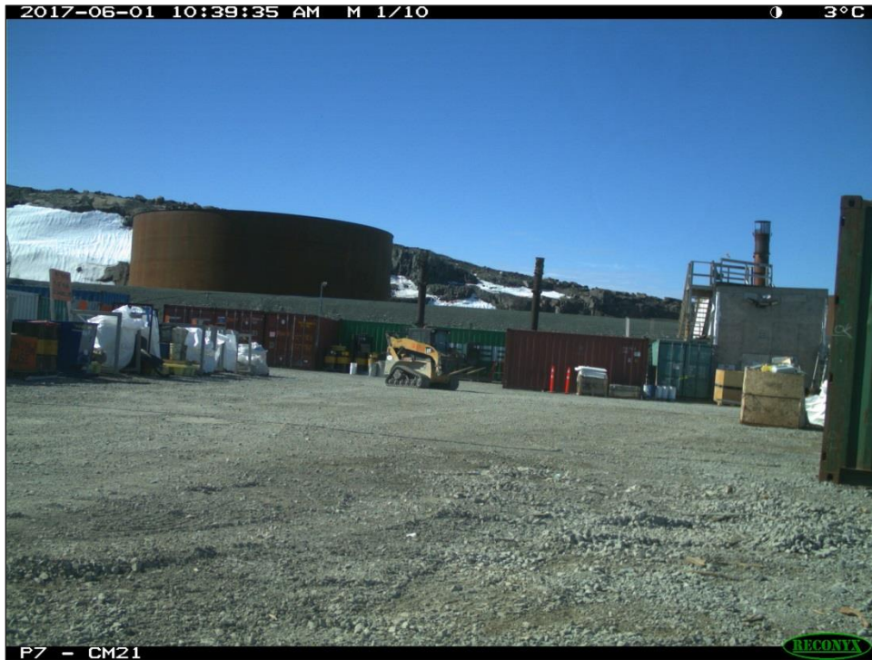
Photo 3.1-7 Example of the monitoring view of Camera 21 at the Roberts Bay Waste Management Facility.
