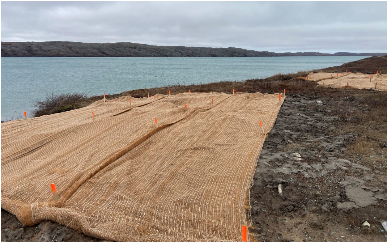
Figure 4 Erosion Blankets Along the Shoreline
