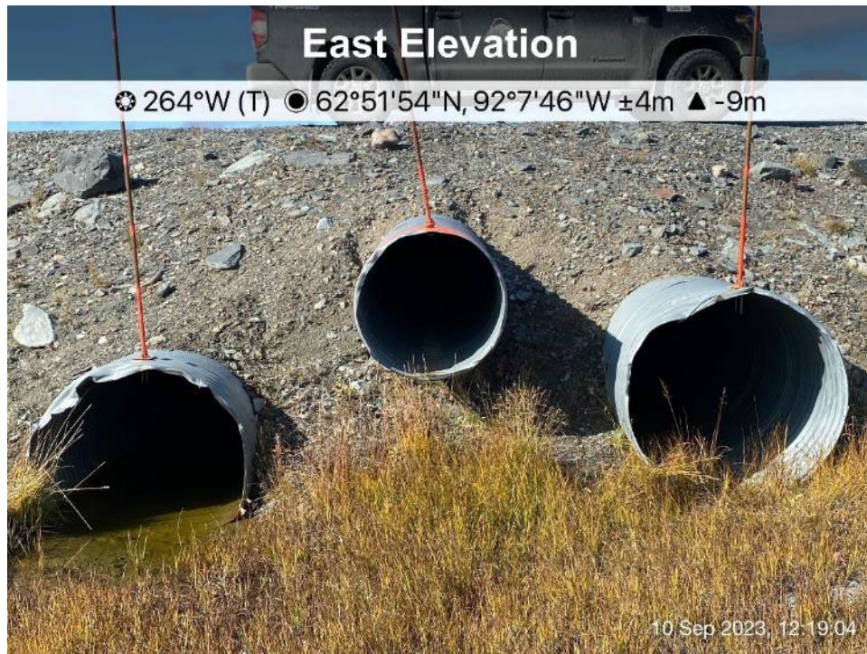
AWAR Road/Culvert - Photo 10: Culvert KM 7.0 - inlet.
