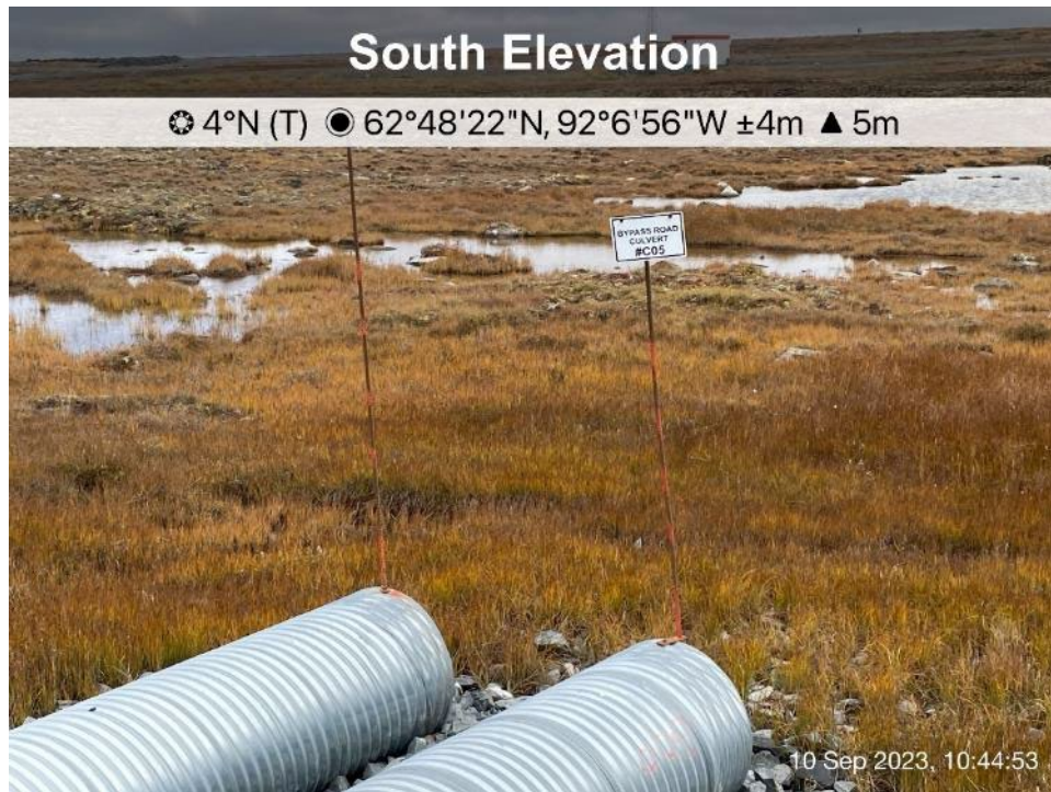
Itivia Bypass Road/Culvert - Photo 12: Culvert C05 inlet.
