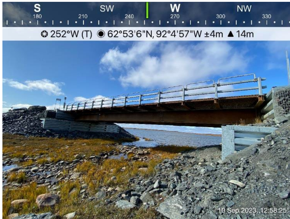
AWAR Road/Culvert - Photo 27: M-5 Bridge KM 10.5.
