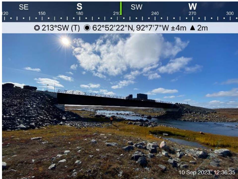
AWAR Road/Culvert - Photo 17: Meliadine River Bridge KM 8.0.
