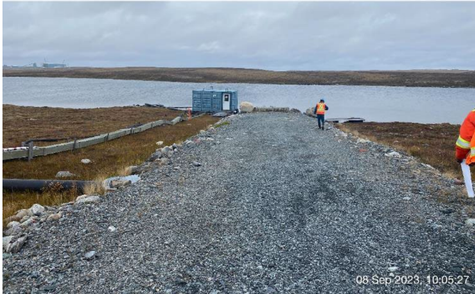
Site Road - Photo 9: Site Road - Exploration camp water intake access road.
