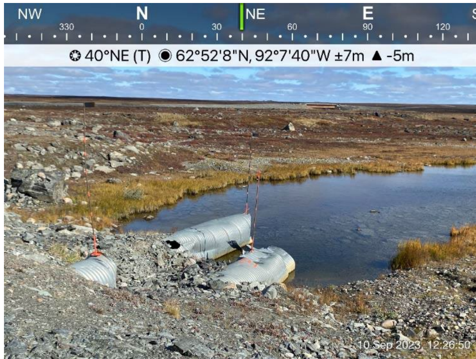
AWAR Road/Culvert - Photo 15: Culvert KM 7.4 – inlet.
