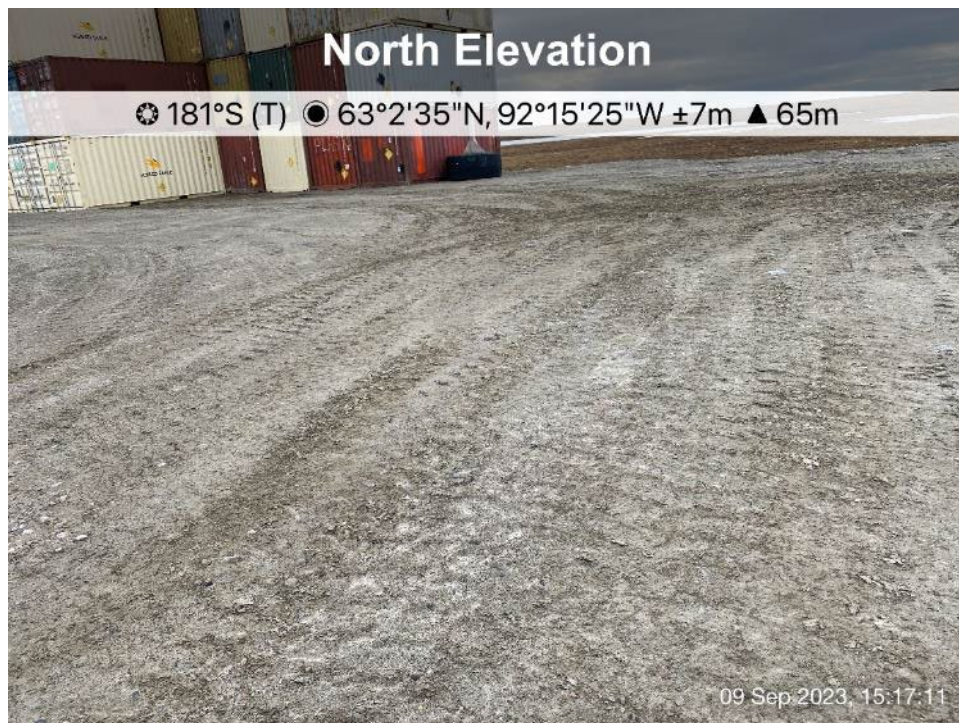
Emulsion Plant Pad - Photo 15: Emulsion Plant Pad - Overview, looking south.
