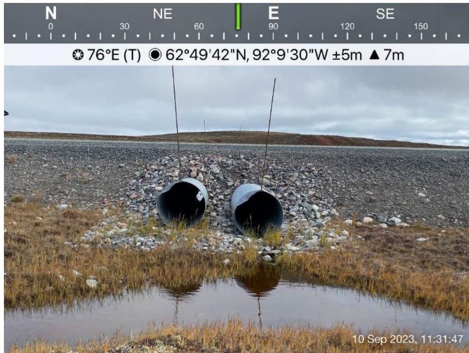
Itivia Bypass Road/Culvert - Photo 43: Culvert C15 outlet.
