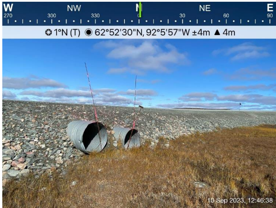
AWAR Road/Culvert - Photo 23: Culvert KM 9.1 – inlet.
