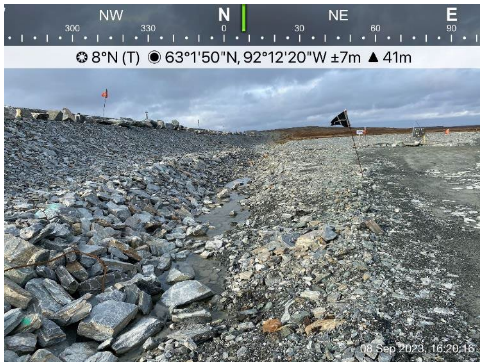
D-CP1 - Photo 8: Dike D-CP1: Dike downstream runoff/seepage collection south channel.
