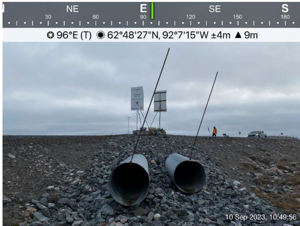
Itivia Bypass Road/Culvert - Photo 17: Culvert C06 outlet.
