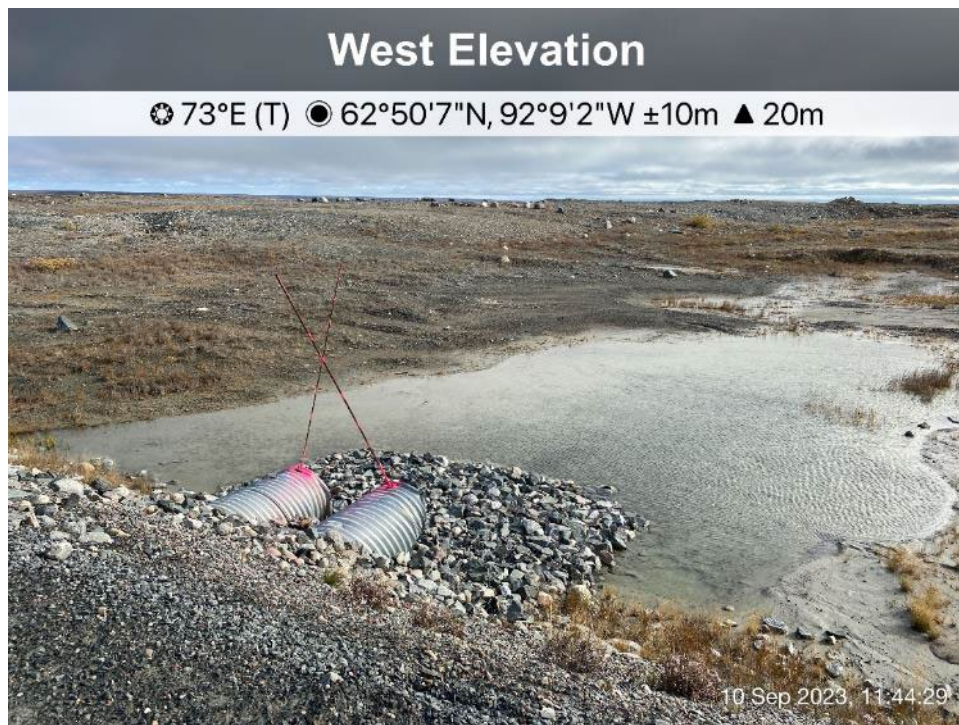
Itivia Bypass Road/Culvert - Photo 50: Culvert C18 inlet.
