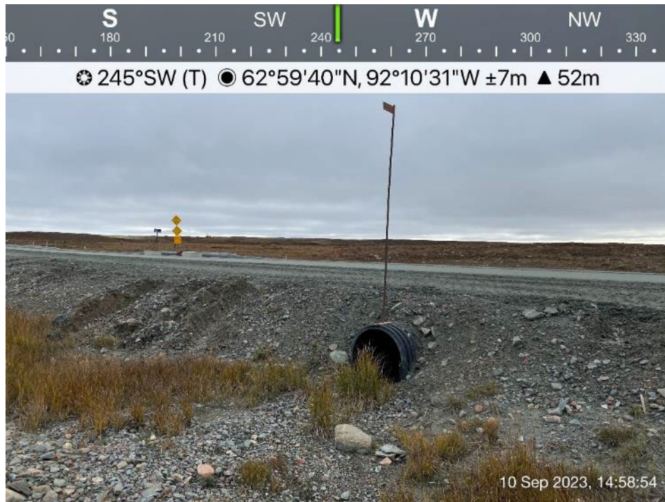
AWAR Road/Culvert - Photo 55: Culvert KM 25.8 - HDPE corrugated culvert – inlet.
