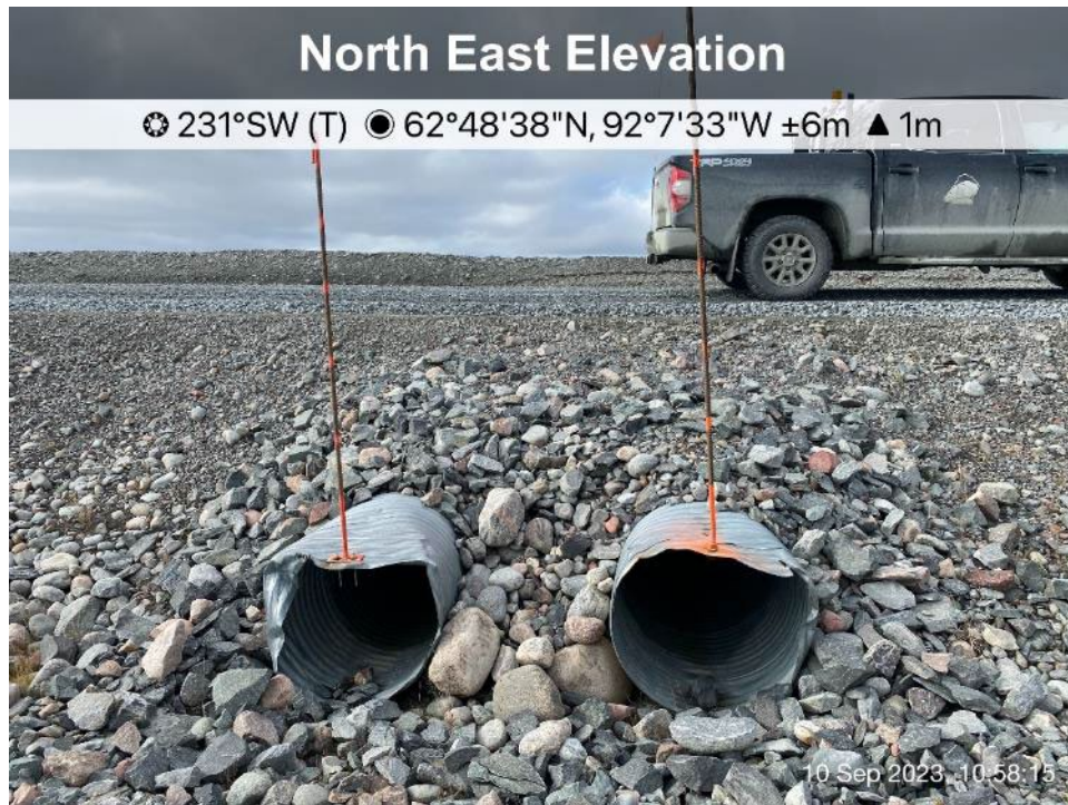
Itivia Bypass Road/Culvert - Photo 25: Culvert C09 inlet.
