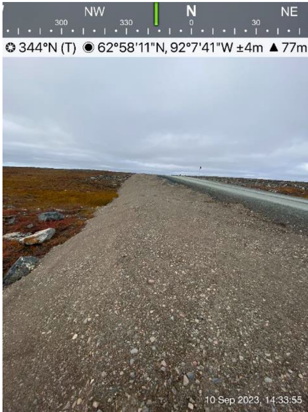
AWAR Road/Culvert - Photo 53:
