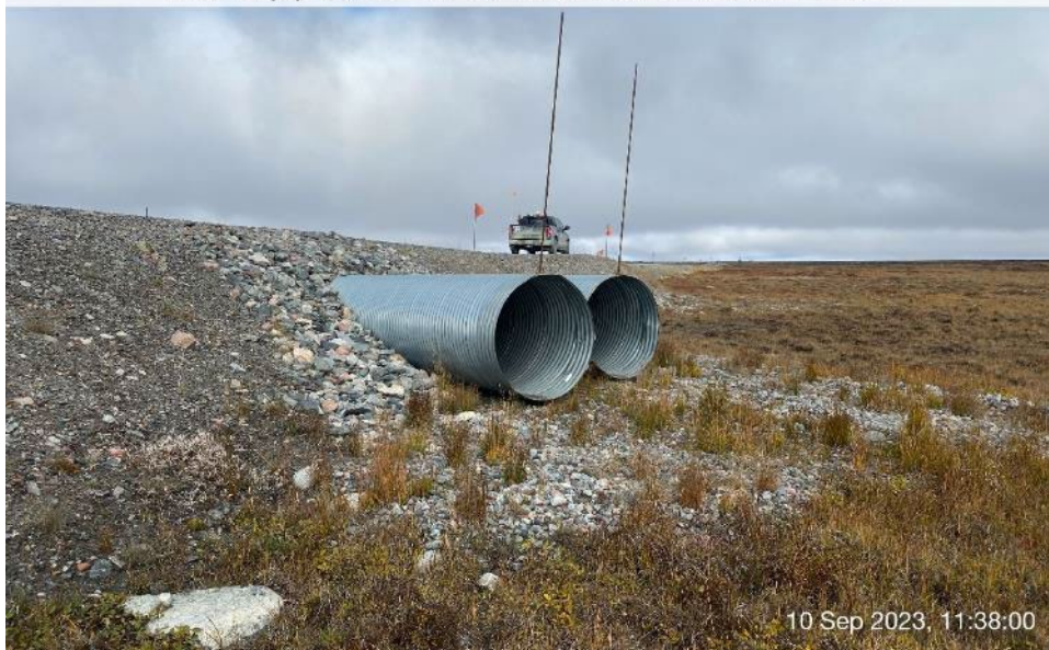
Itivia Bypass Road/Culvert - Photo 48: Culvert C17 inlet.
