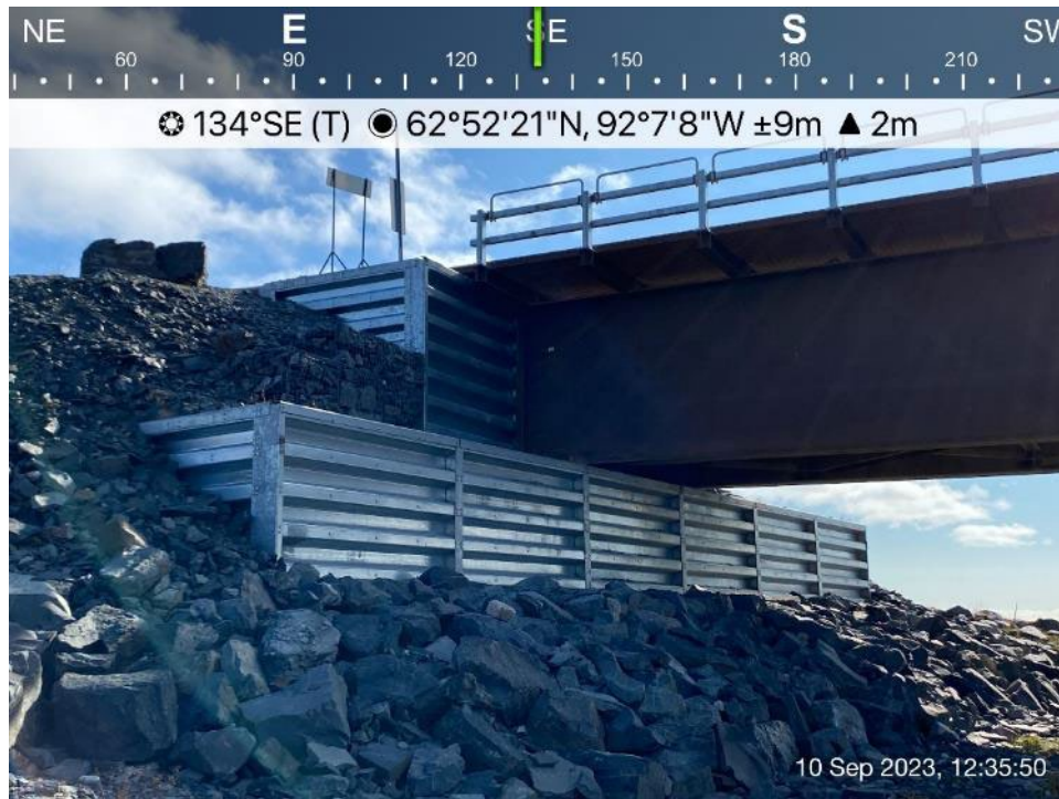
AWAR Road/Culvert - Photo 20: Meliadine River Bridge KM 8.0- west abutment.
