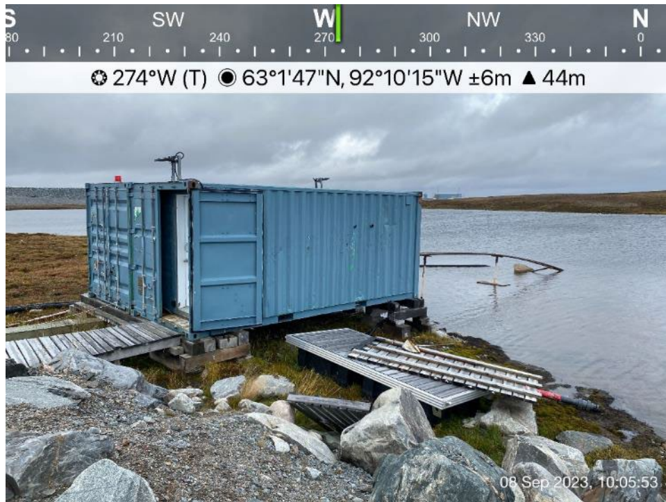
Exploration Camp - Photo 6: Exploration Camp - freshwater intake pump house, looking west.
