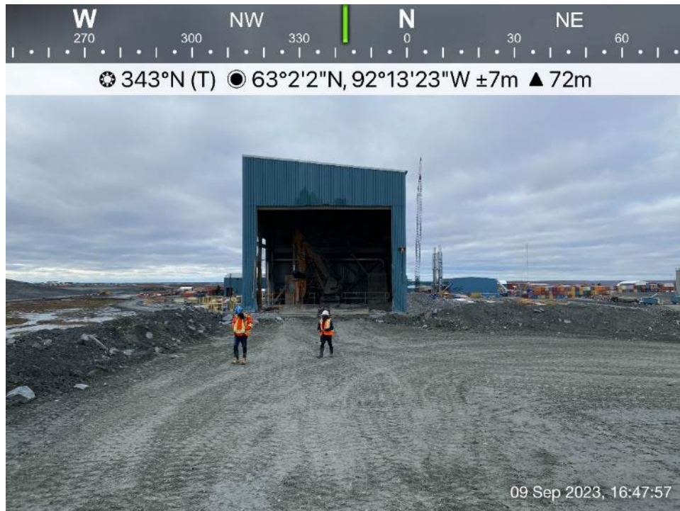
Crusher Pad - Photo 3: Crusher pad top view - looking north.
