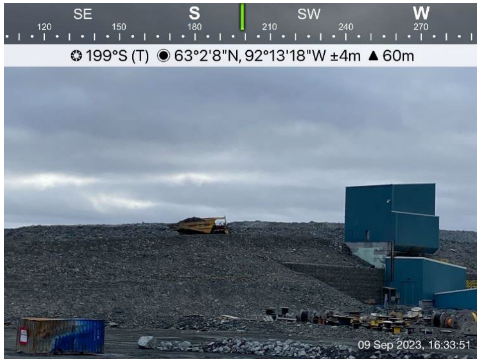
Crusher Pad - Photo 1: Crusher pad and ramp - Overview, looking south.
