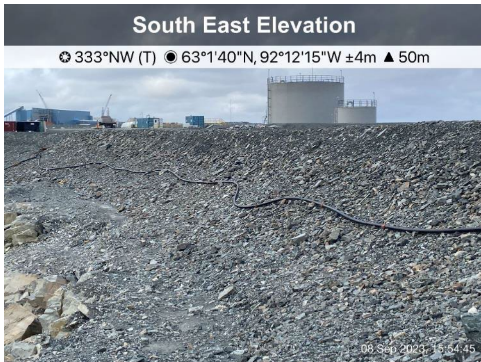
SP1 - Photo 2: SP1 Saline Pond - Perimeter berm side slope.
