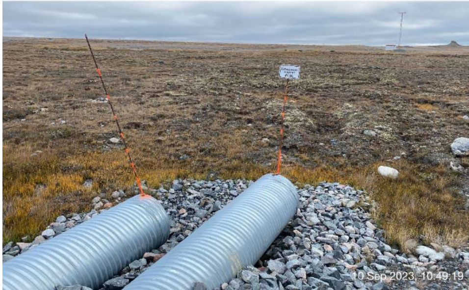
Itivia Bypass Road/Culvert - Photo 15: Culvert C06 inlet.
