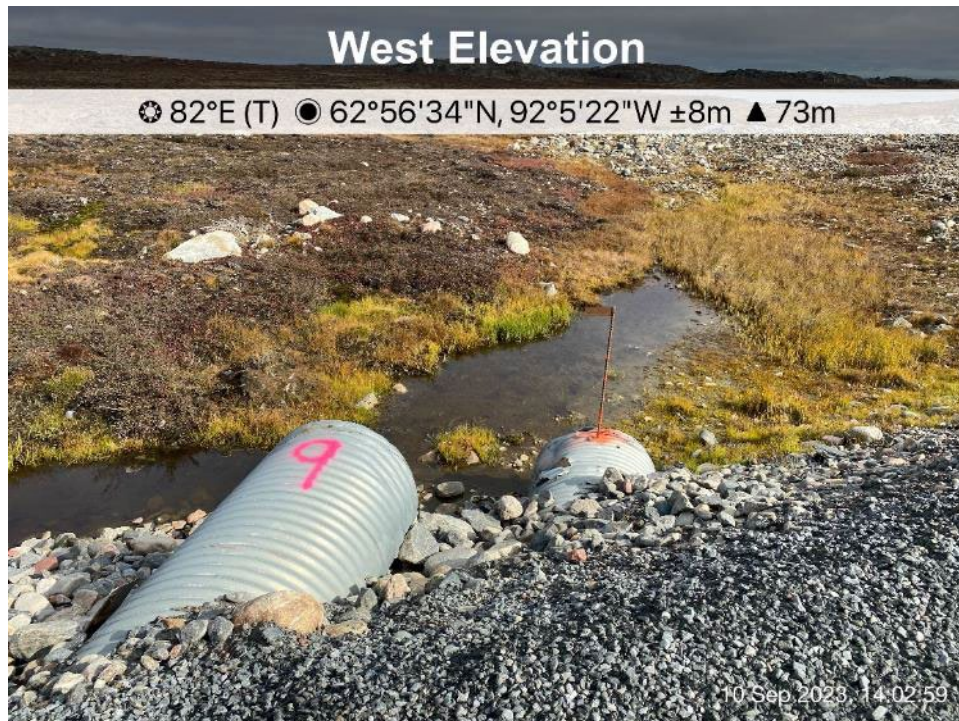
AWAR Road/Culvert - Photo 43: Culvert KM 18.1 – inlet.
