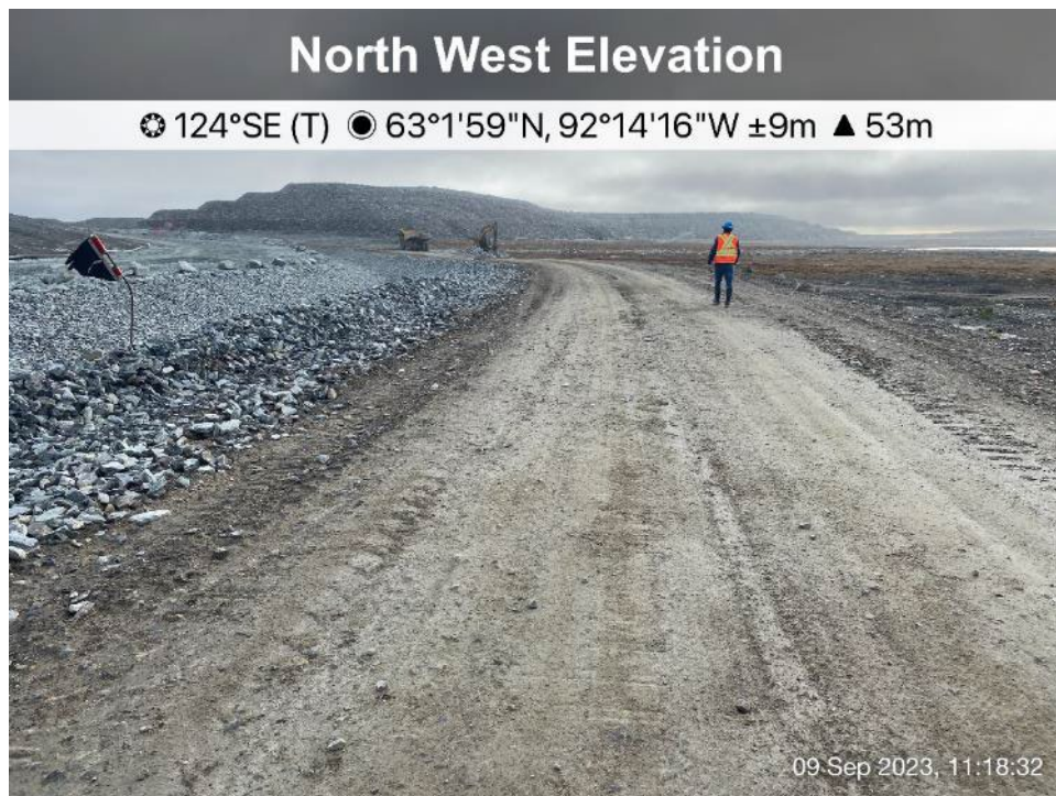
Site Road - Photo 2: Site Road - CP3 access road.
