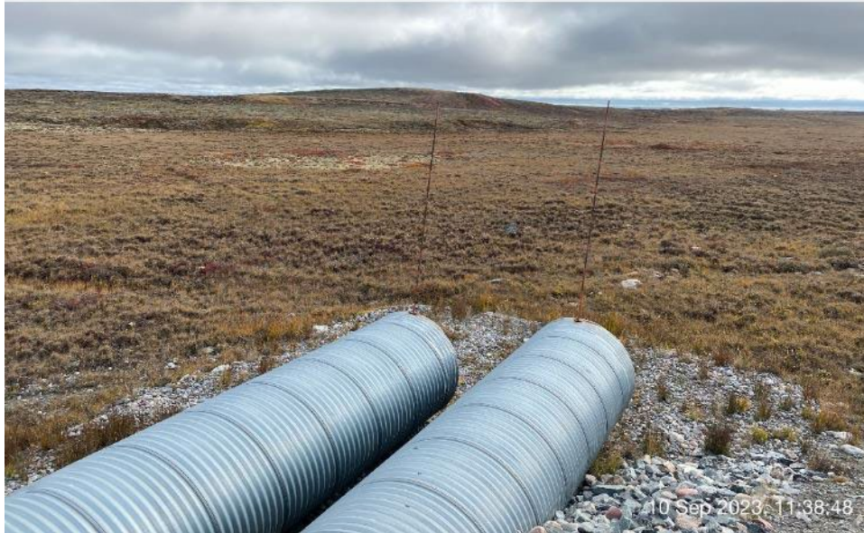
Itivia Bypass Road/Culvert - Photo 47: Culvert C17 inlet.
