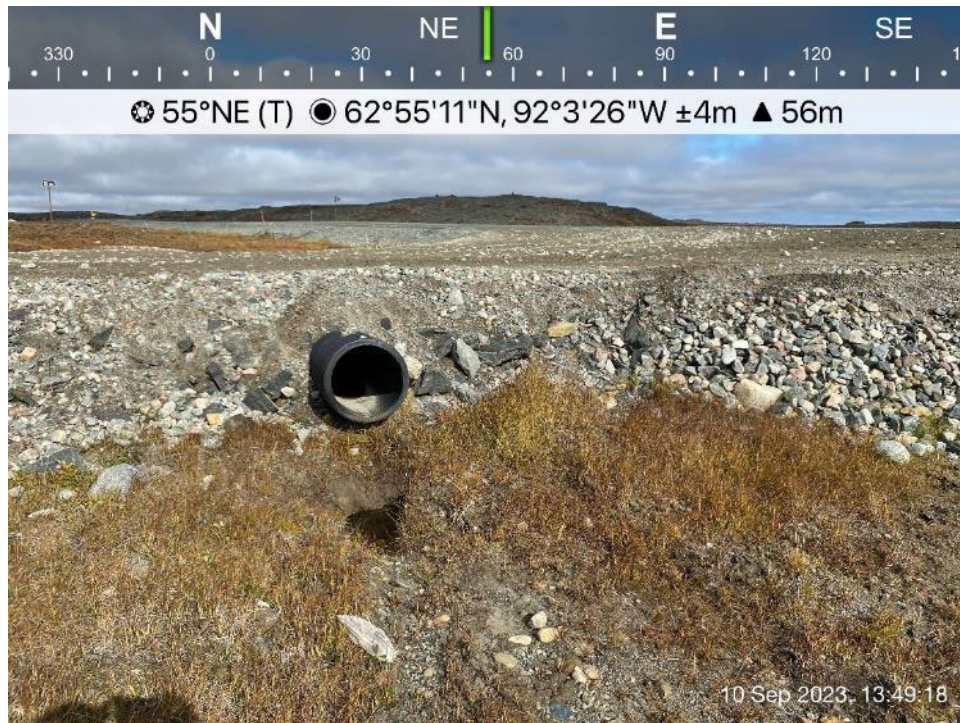
AWAR Road/Culvert - Photo 39: Culvert KM 14.7 - outlet- HDPE corrugated culvert.
