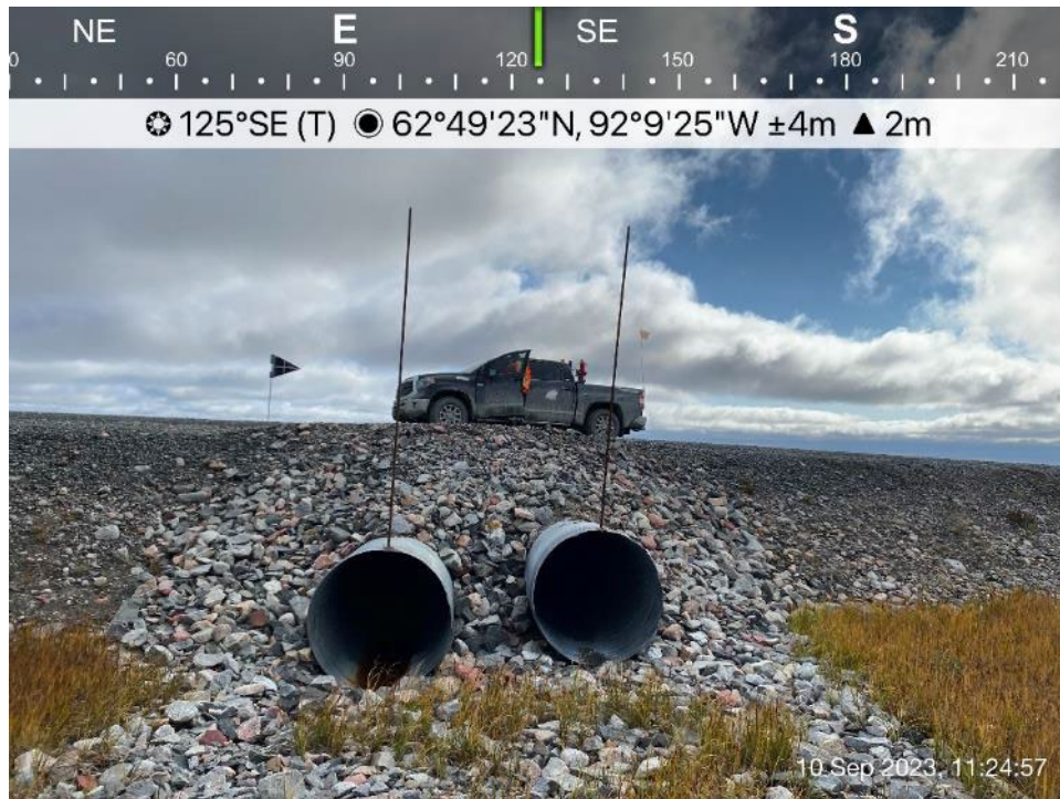
Itivia Bypass Road/Culvert - Photo 37: Culvert C13 outlet.
