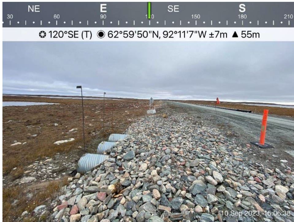
AWAR Road/Culvert - Photo 60: Culvert KM 26.5 – inlet.
