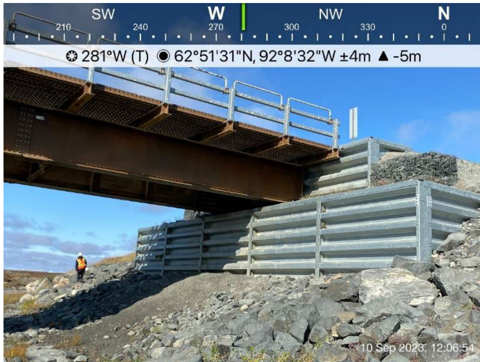
AWAR Road/Culvert - Photo 5: Char River Bridge KM 6.1 - south abutment.
