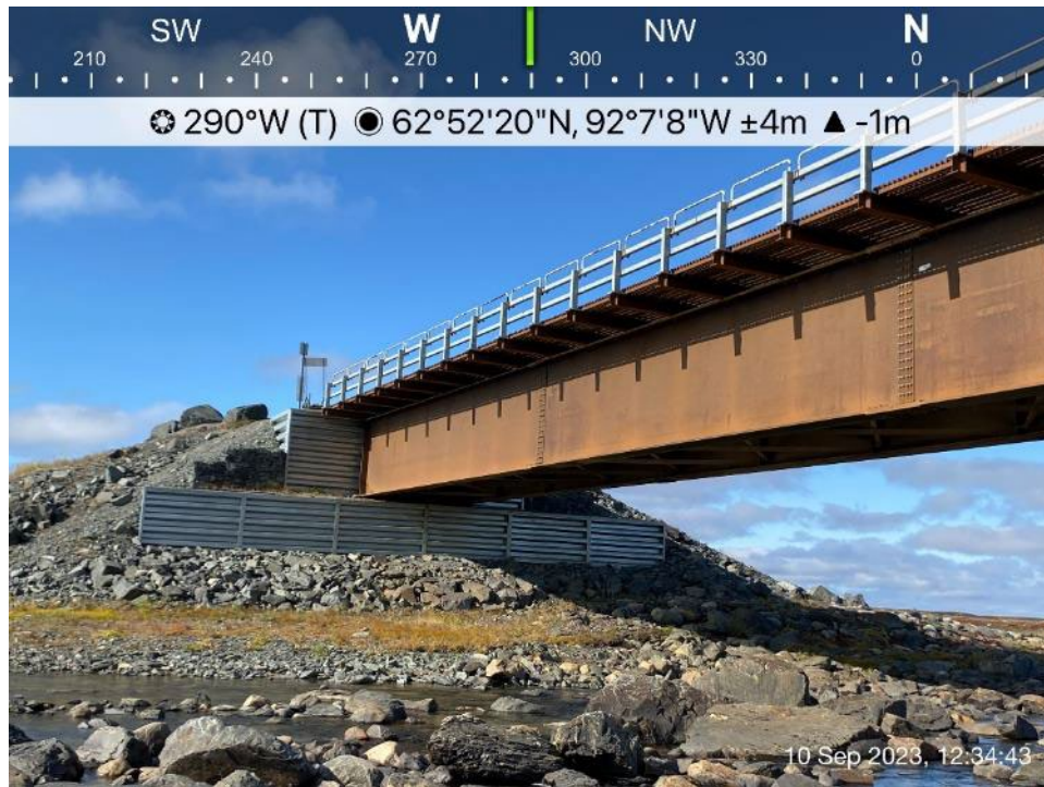
AWAR Road/Culvert - Photo 19: Meliadine River Bridge KM 8.0- east abutment.
