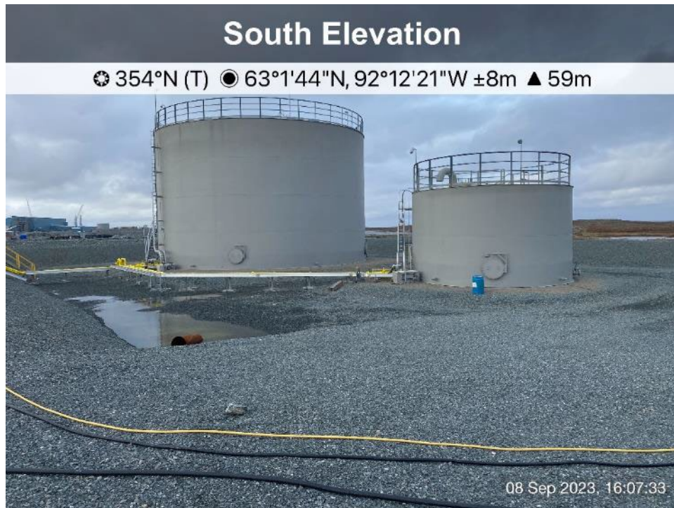
3M Fuel Tanks - Photo 30: 3M Fuel Tanks - Overview, looking north.
