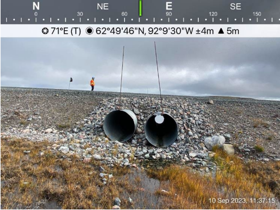
Itivia Bypass Road/Culvert - Photo 46: Culvert C16 outlet.
