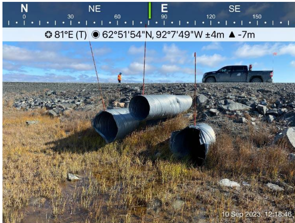
AWAR Road/Culvert - Photo 11: Culvert KM 7.0 - outlet.
