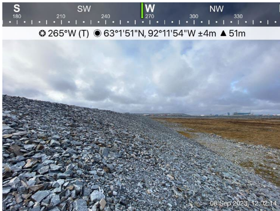
CP6 - Photo 6: CP6 Thermal Berm, looking west, upstream slope.
