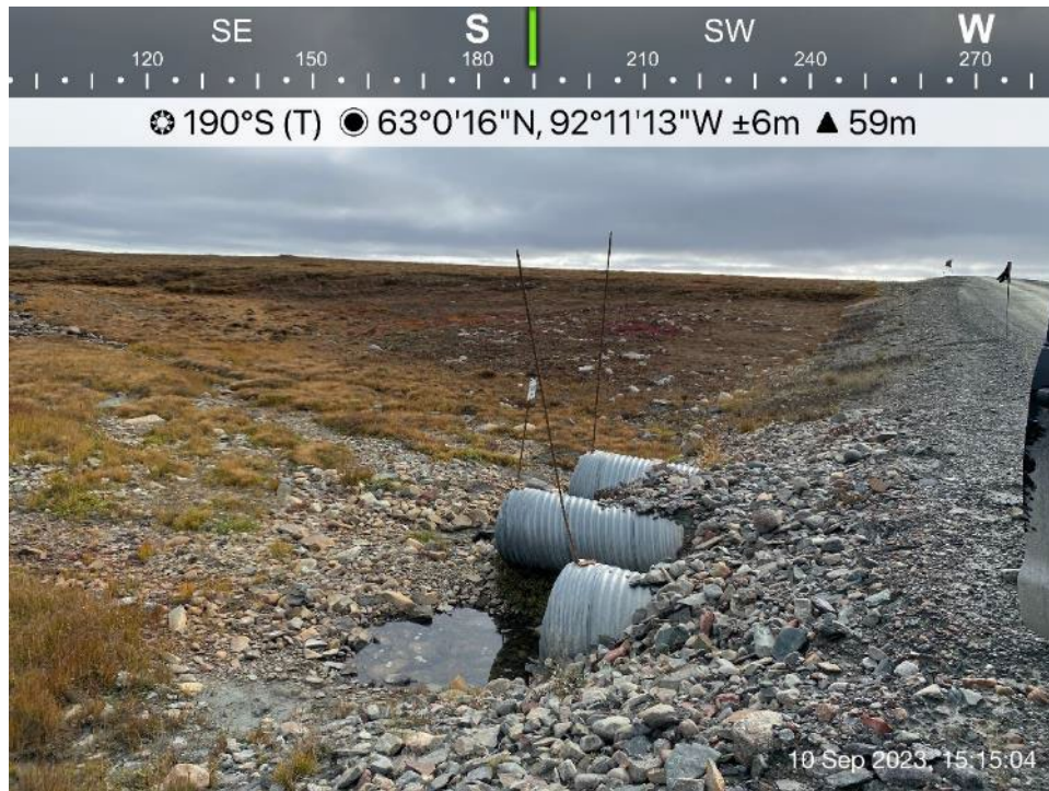
AWAR Road/Culvert - Photo 65: Culvert KM 27.1 – inlet.
