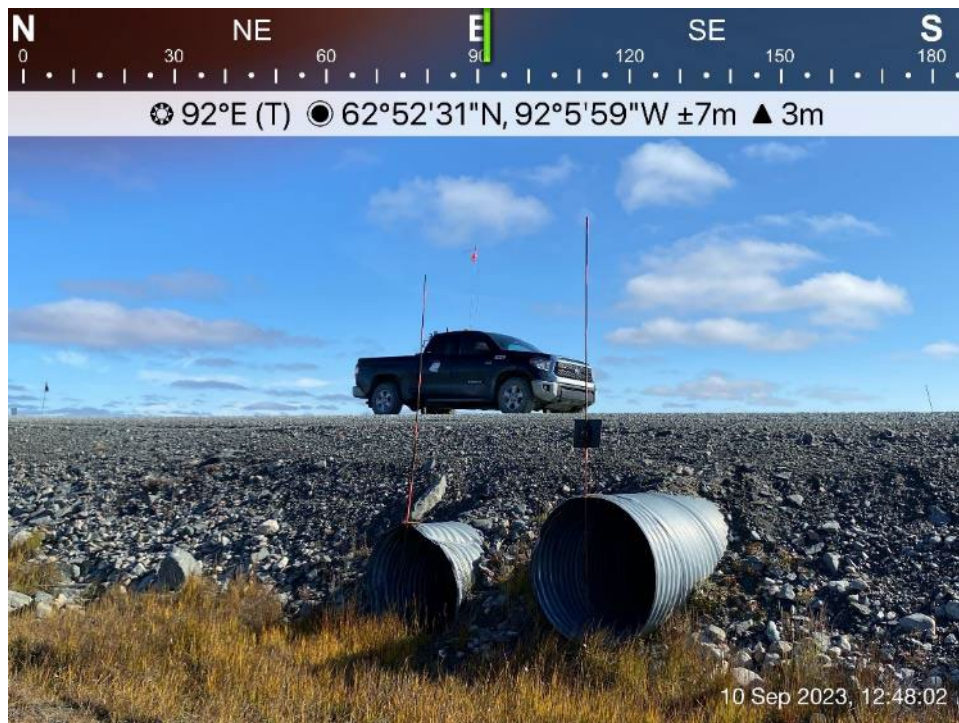
AWAR Road/Culvert - Photo 24: Culvert KM 9.1 – outlet.
