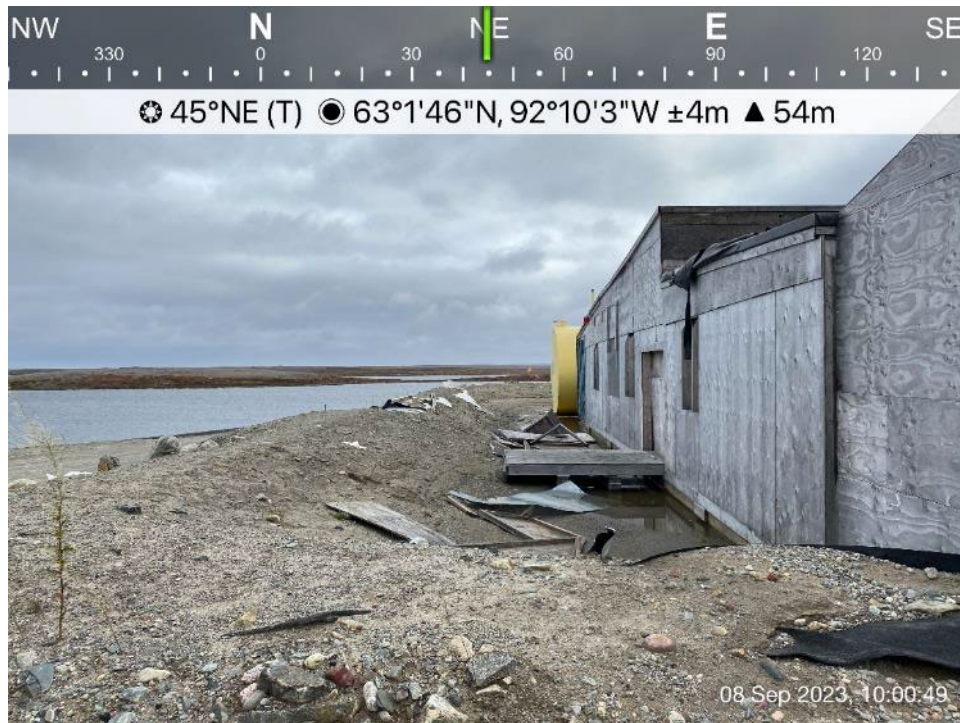
Exploration Camp - Photo 3: Exploration Camp - Fuel storage, looking northeast.
