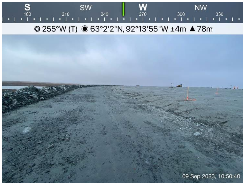
TSF - Photo 8: TSF - Crest of rockfill covered slope, and stack used for lift thickness control.
