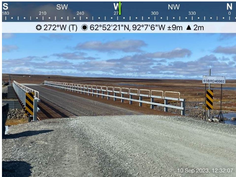
AWAR Road/Culvert - Photo 18: Meliadine River Bridge KM 8.0.
