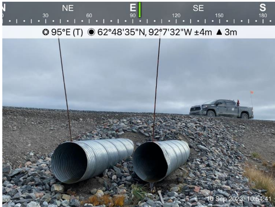
Itivia Bypass Road/Culvert - Photo 23: Culvert C08 outlet.
