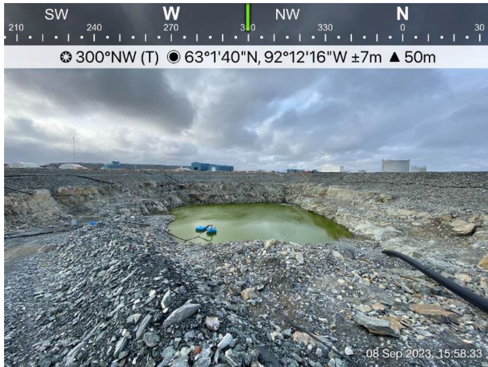
SP1 - Photo 1: SP1 Saline Pond - Looking west, overview of SP1, pond in bedrock, ROM covered overburden slopes.
