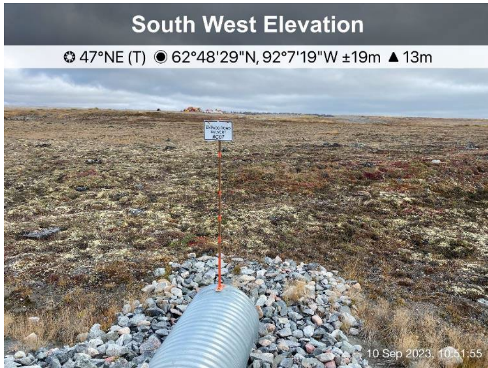
Itivia Bypass Road/Culvert - Photo 18: Culvert C07 inlet.
