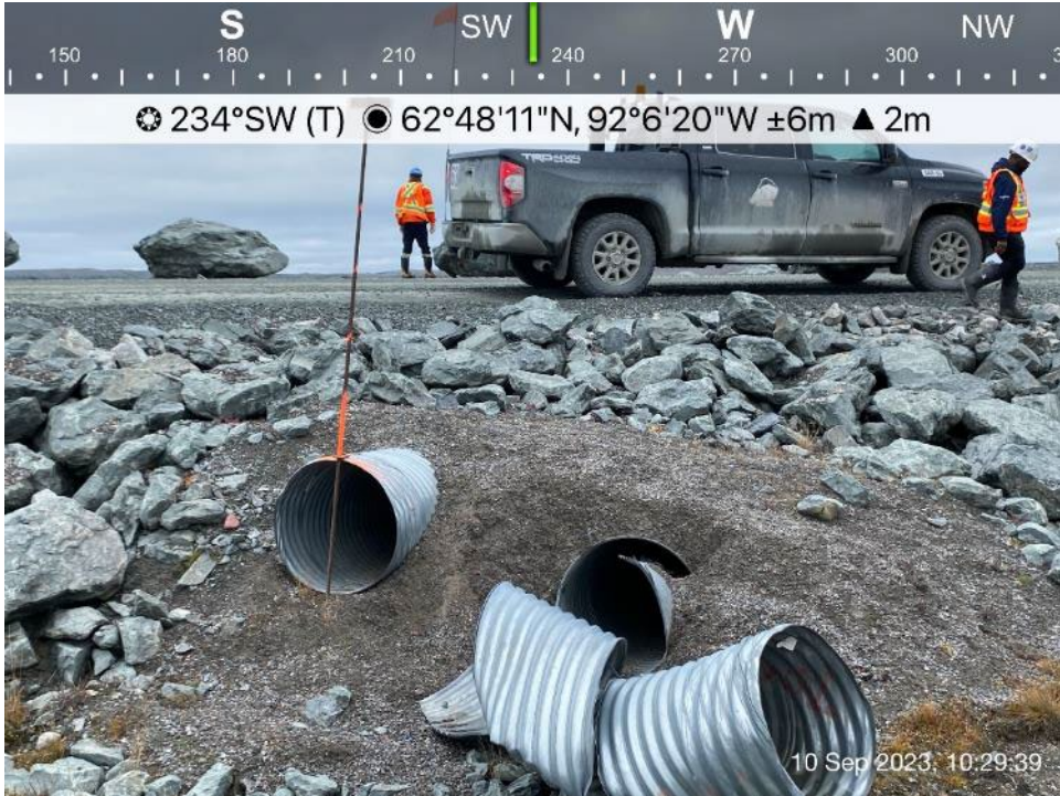
Itivia Bypass Road/Culvert - Photo 4: Culvert C02 Inlet.
