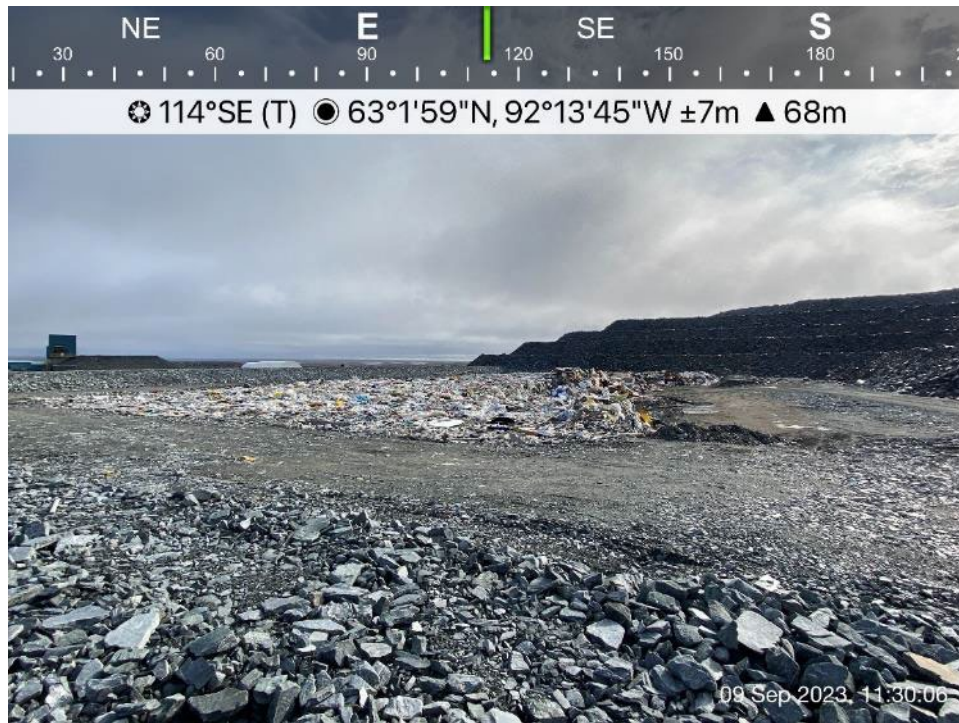
Landfill - Photo 8: WRSF1 Landfill - Overview of landfill, looking southeast.
