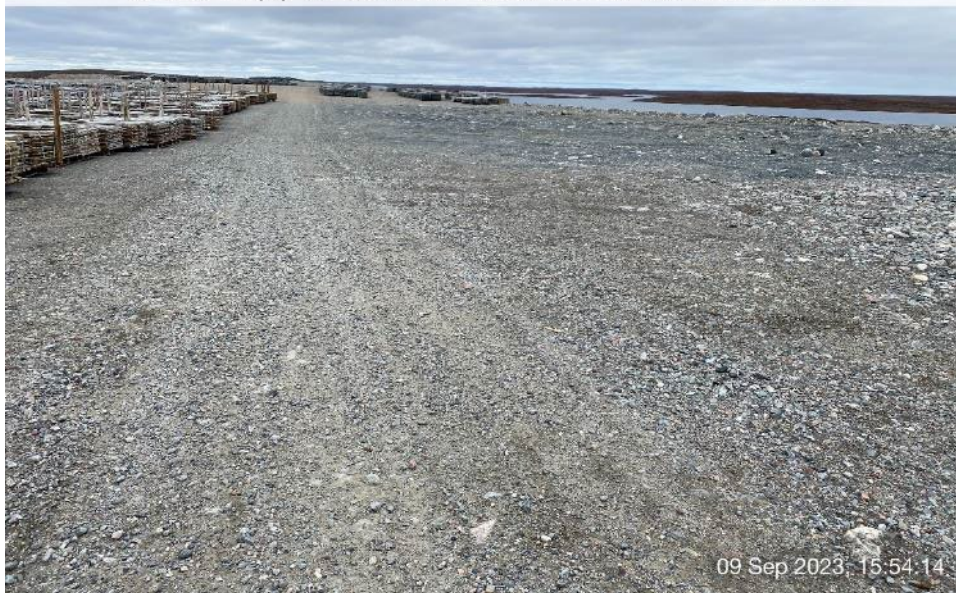
Site Road - Photo 10: Site Road - Meliadine North Esker access road.
