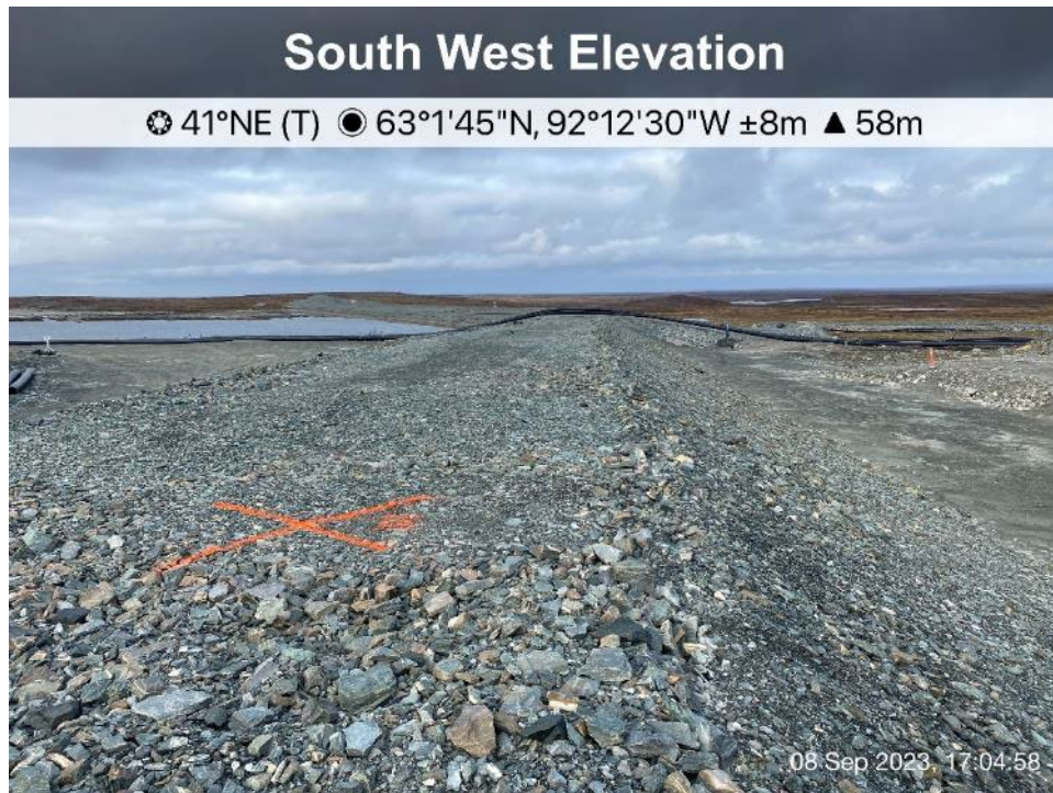
D-CP1 - Photo 15: Dike D-CP1: Pipelines crossing at Station 1+250 of Dike D-CP1.
