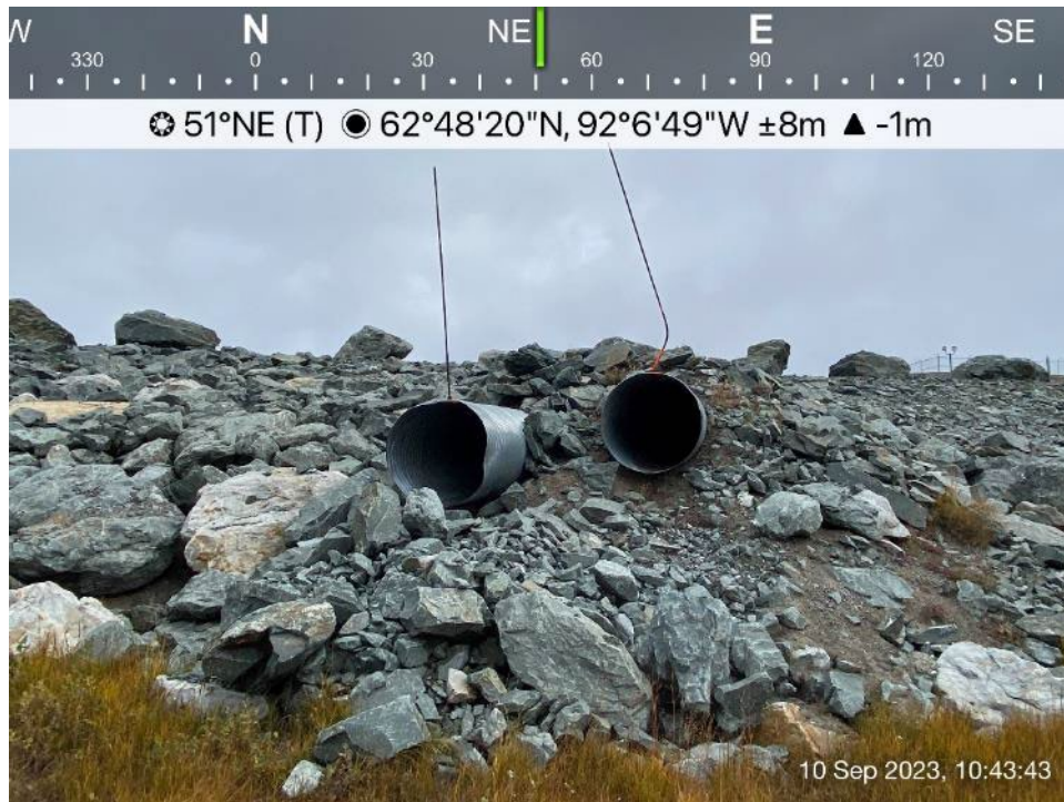
Itivia Bypass Road/Culvert - Photo 11: Culvert C04 outlet.
