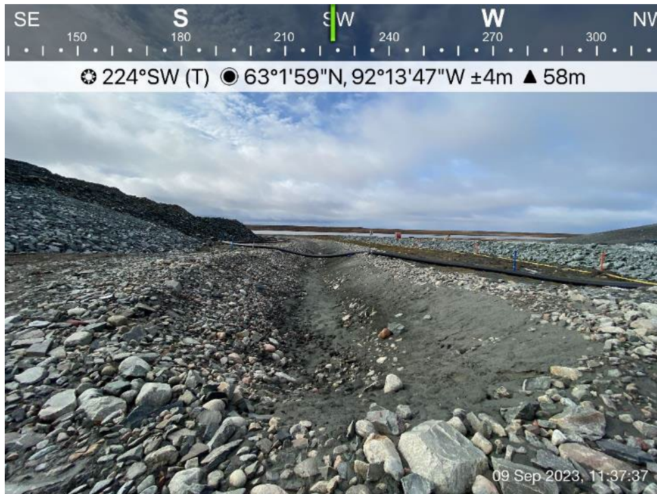
Channel 4 - Photo 9: Channel 4 - Upper reach of Channel 4, below landfill of WRSF1, infilling with sediments observed.
