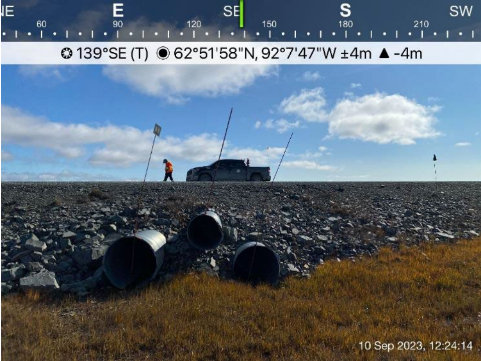
AWAR Road/Culvert - Photo 14: Culvert KM 7.1 – outlet.
