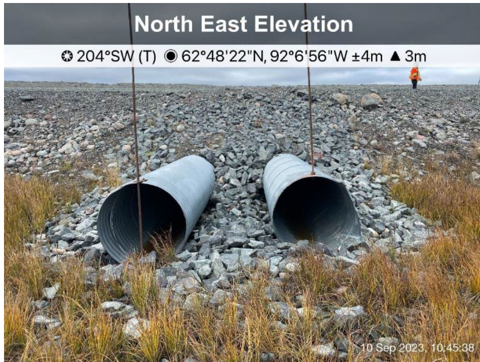
Itivia Bypass Road/Culvert - Photo 13: Culvert C05 inlet.
