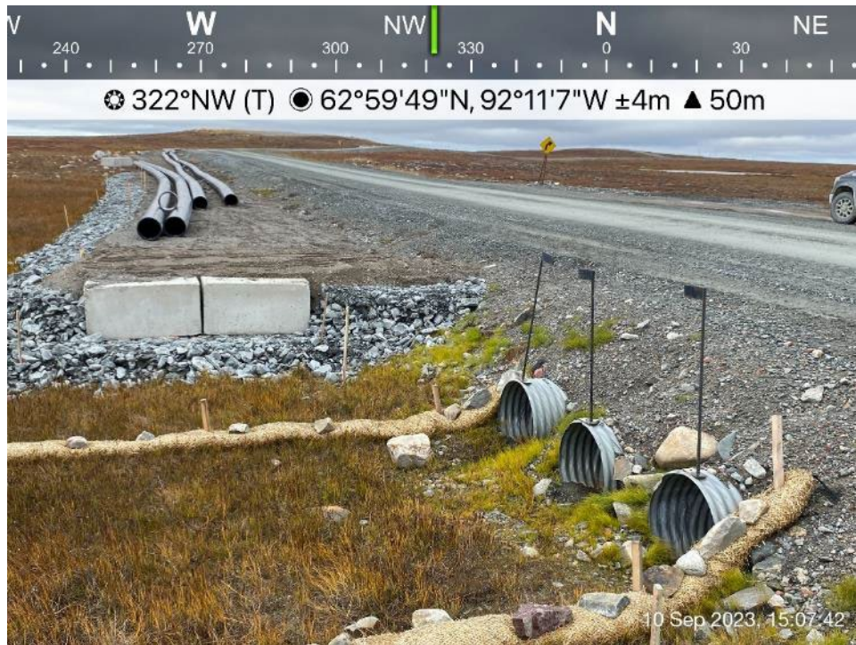
AWAR Road/Culvert - Photo 62: Culvert KM 26.5 – outlet.
