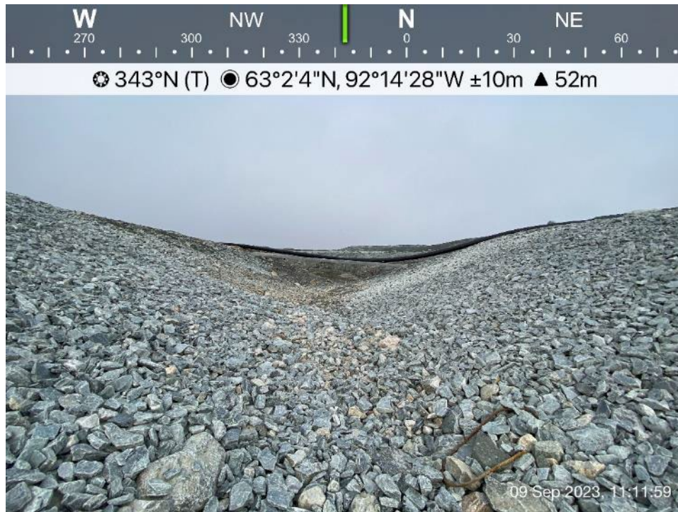
Channel 3 - Photo 6: Channel 3 - Channel 3 northwest end, entering CP3.
