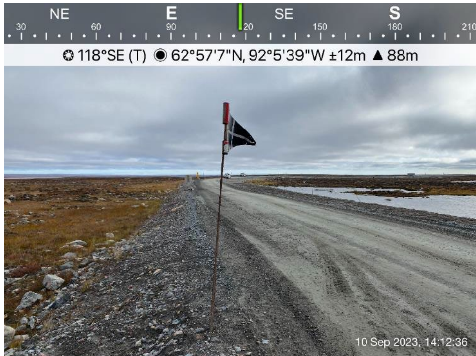
AWAR Road/Culvert - Photo 49: KM 19 - No culvert installed, ponded water upstream, no sign of overflow.
