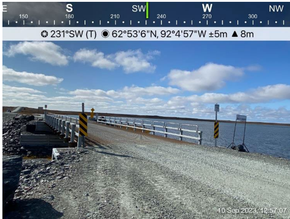
AWAR Road/Culvert - Photo 28: M-5 Bridge KM 10.5.
