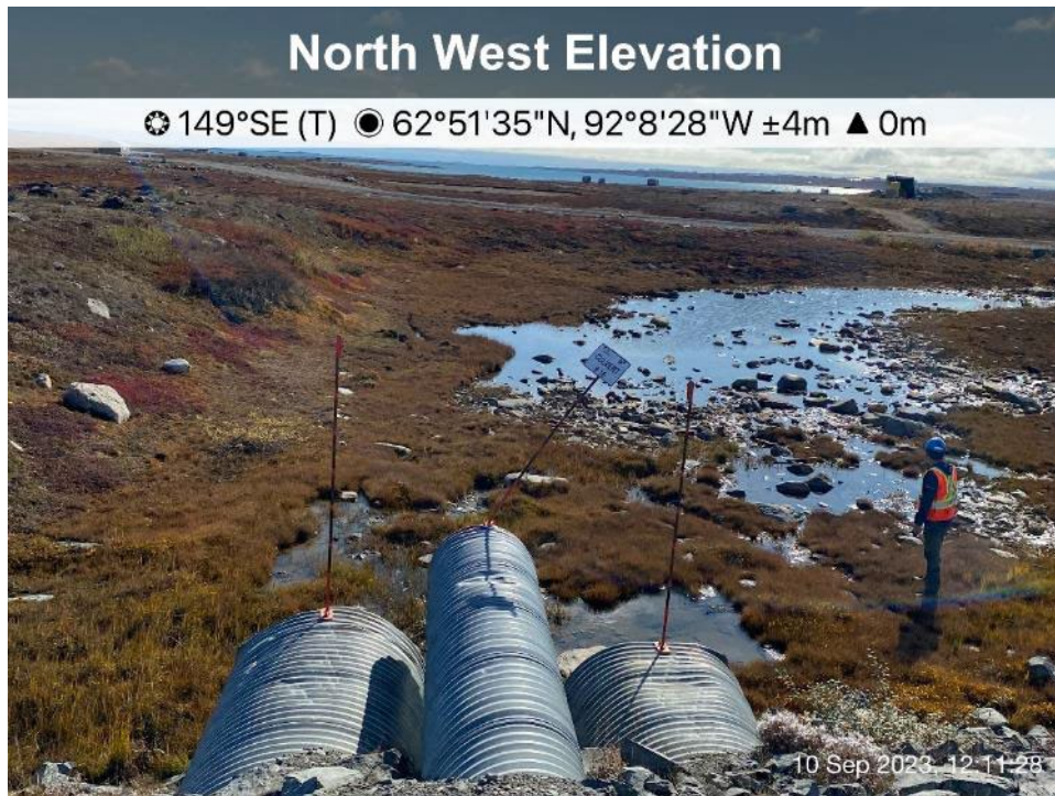
AWAR Road/Culvert - Photo 6: Culvert KM 6.2 - inlet.
