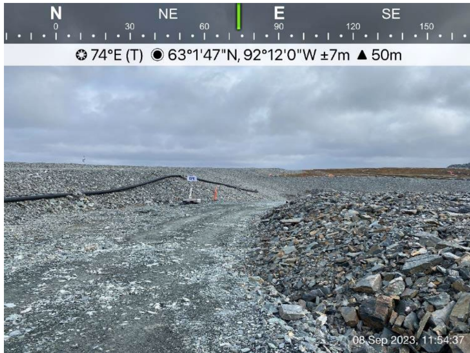
CP6 - Photo 1: CP6 - Looking east, ramp entering CP6.
