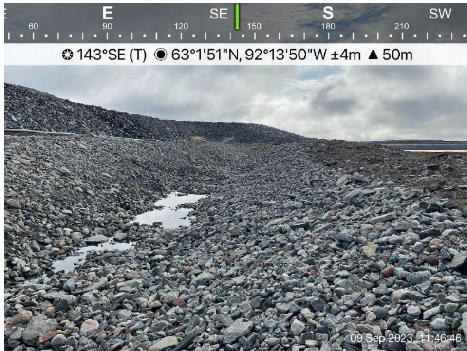
Channel 4 - Photo 11: Channel 4 - Settlement in base of channel resulting in minor ponding.
