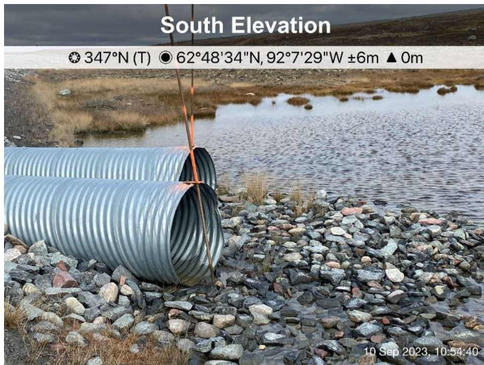
Itivia Bypass Road/Culvert - Photo 22: Culvert C08 inlet.
