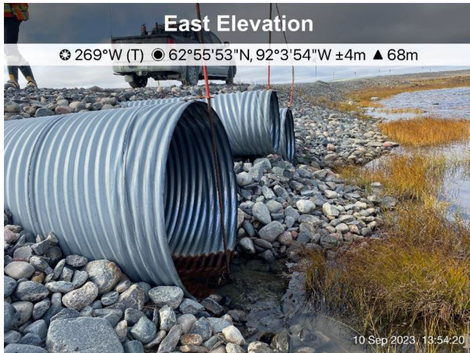
AWAR Road/Culvert - Photo 41: Culvert KM 16.3 – inlet.
