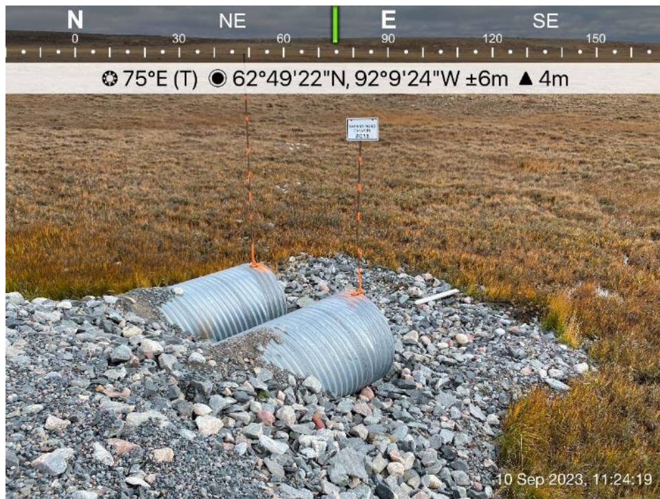
Itivia Bypass Road/Culvert - Photo 36: Culvert C13 inlet.
