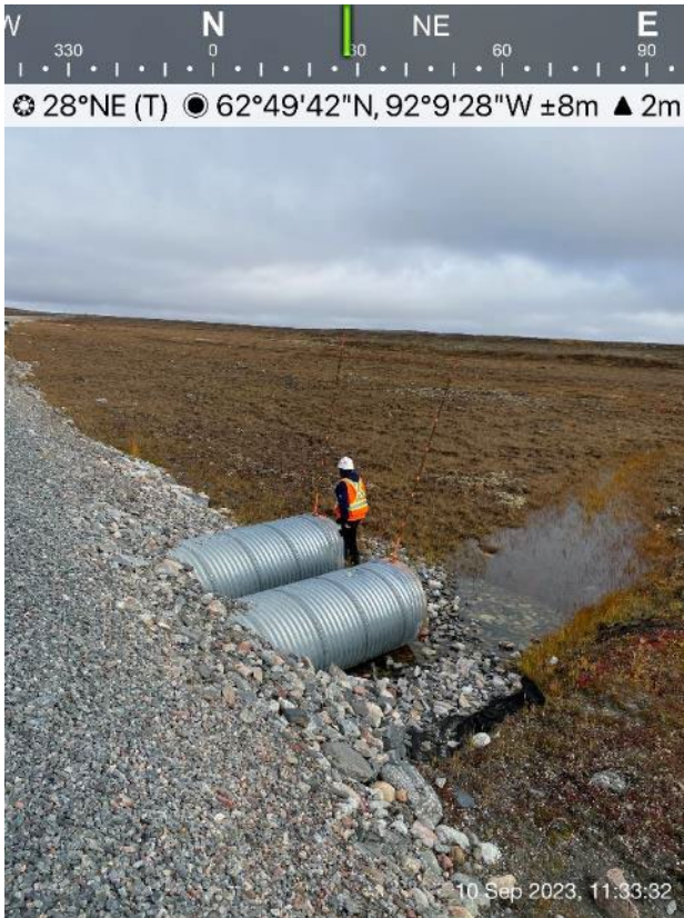
Itivia Bypass Road/Culvert Culvert C15 inlet. - Photo 41:
