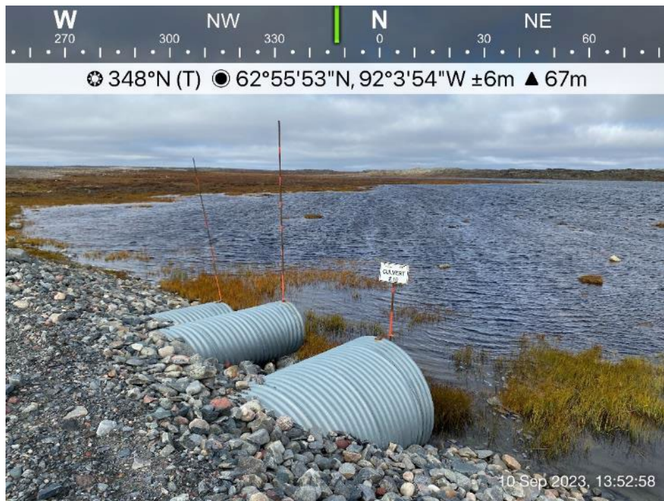
AWAR Road/Culvert - Photo 40: Culvert KM 16.3 – inlet.
