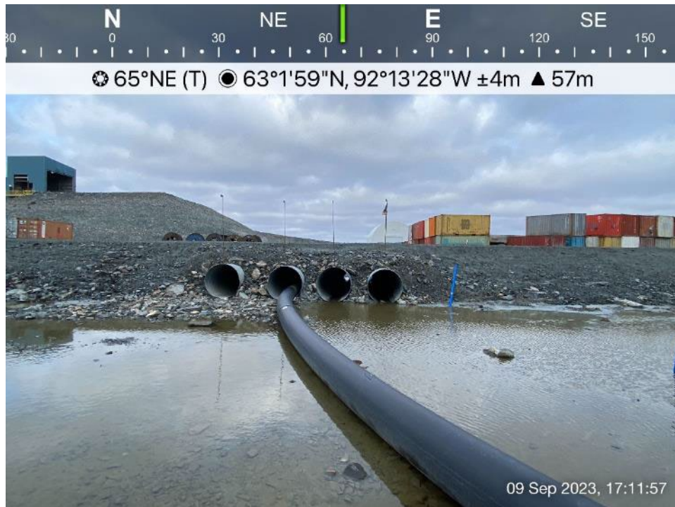
Channel 1 - Photo 1: Channel 1 - Upper reach, culverts divert water from Lake H13 to Channel 1.
