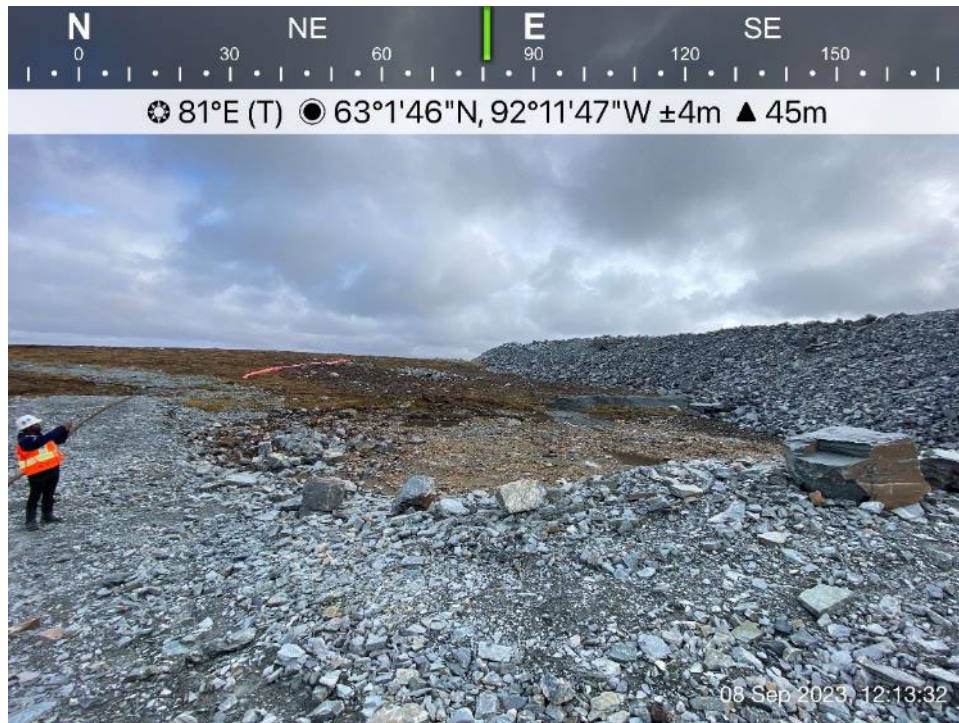
CP6 - Photo 11: CP6 - Ground between CP6 and WRSF3, not covered by rockfill, surface erosion observed.
