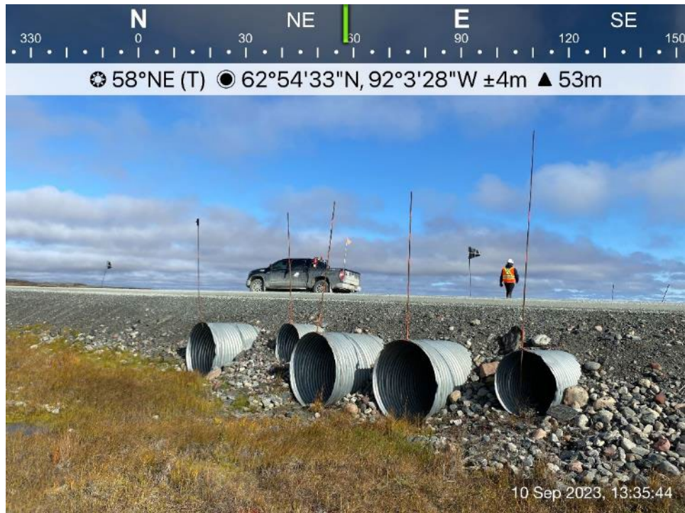
AWAR Road/Culvert - Photo 37: Culvert KM 13.5 – outlet.
