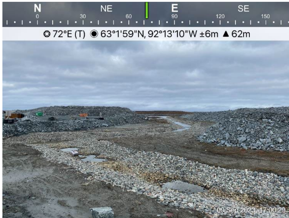
Ore Stockpile - Photo 3: Ore Stockpile - View from Channel 7, looking east.
