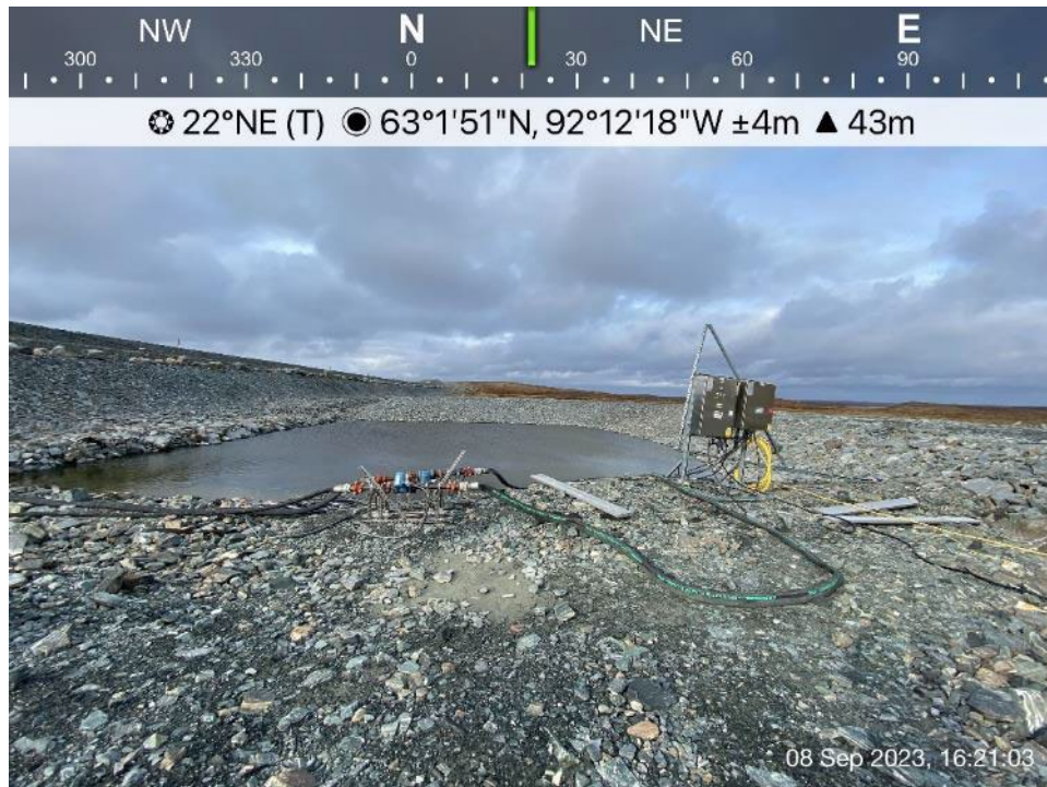
D-CP1 - Photo 9: Dike D-CP1: Dike downstream collection sump.
