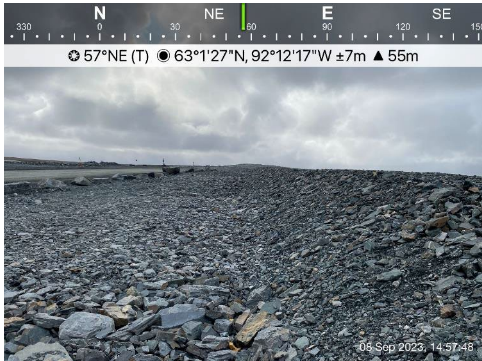
CP5 - Photo 1: Dike D-CP5 - Looking northeast, dike downstream side slope.
