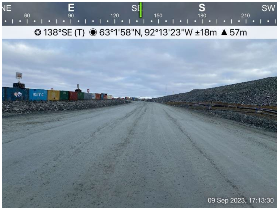
Site Road - Photo 7: Site Road - service road between WRSF1 and storage pad area.
