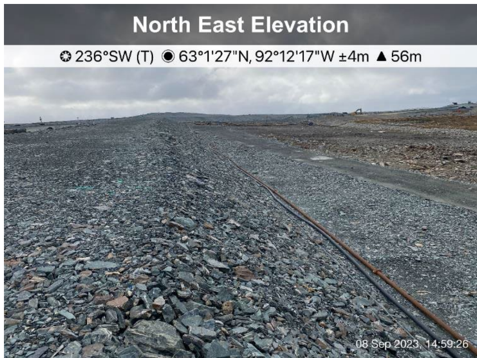
CP5 - Photo 2: Dike D-CP5 - Looking southwest, dike upstream side slope.
