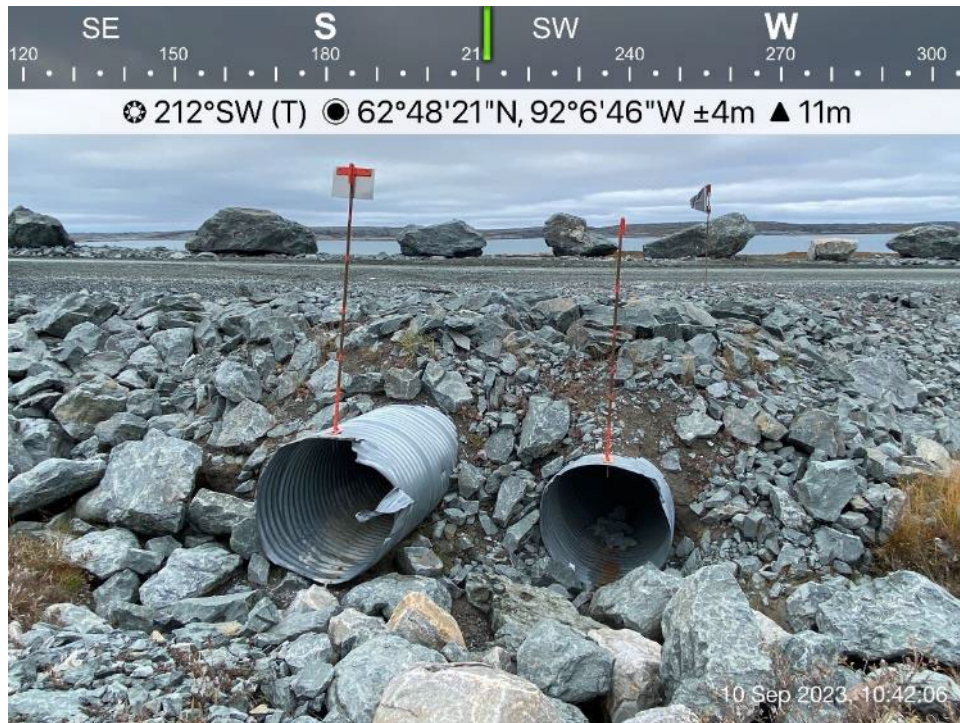
Itivia Bypass Road/Culvert - Photo 10: Culvert C04 inlet.
