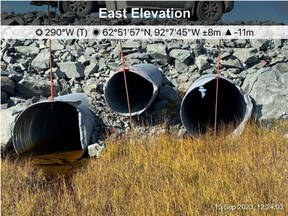
AWAR Road/Culvert - Photo 13: Culvert KM 7.1 – inlet.
