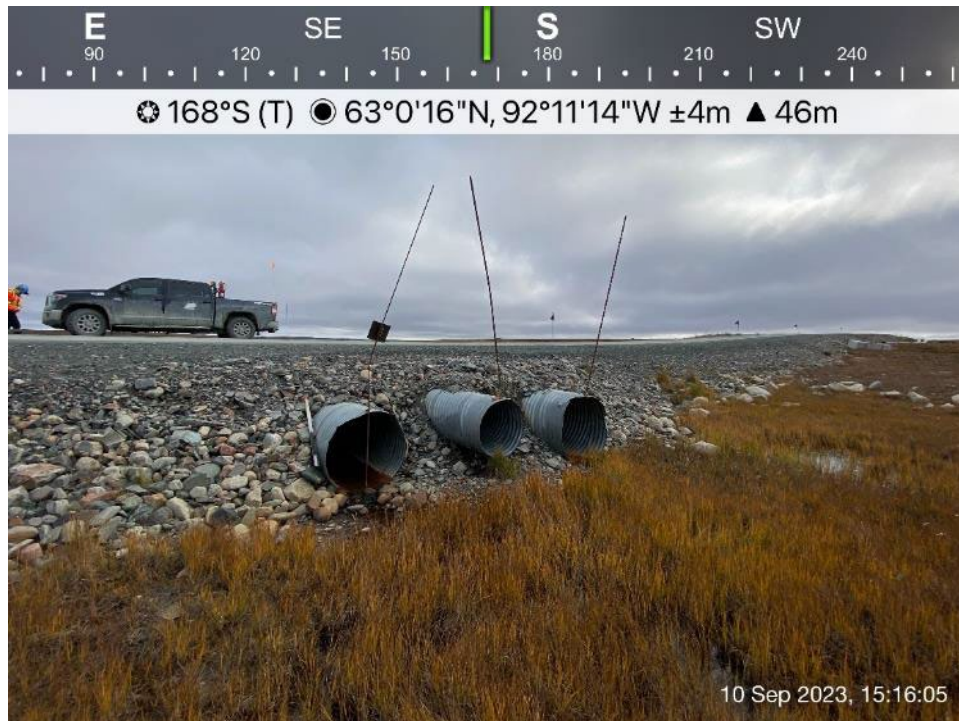
AWAR Road/Culvert - Photo 67: Culvert KM 27.1 – outlet.
