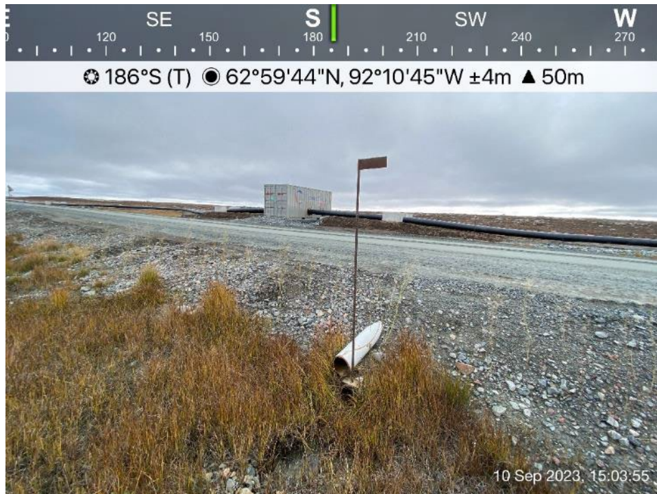
AWAR Road/Culvert - Photo 58: Culvert KM 26.2 - steel pipe as culvert, inlet.
