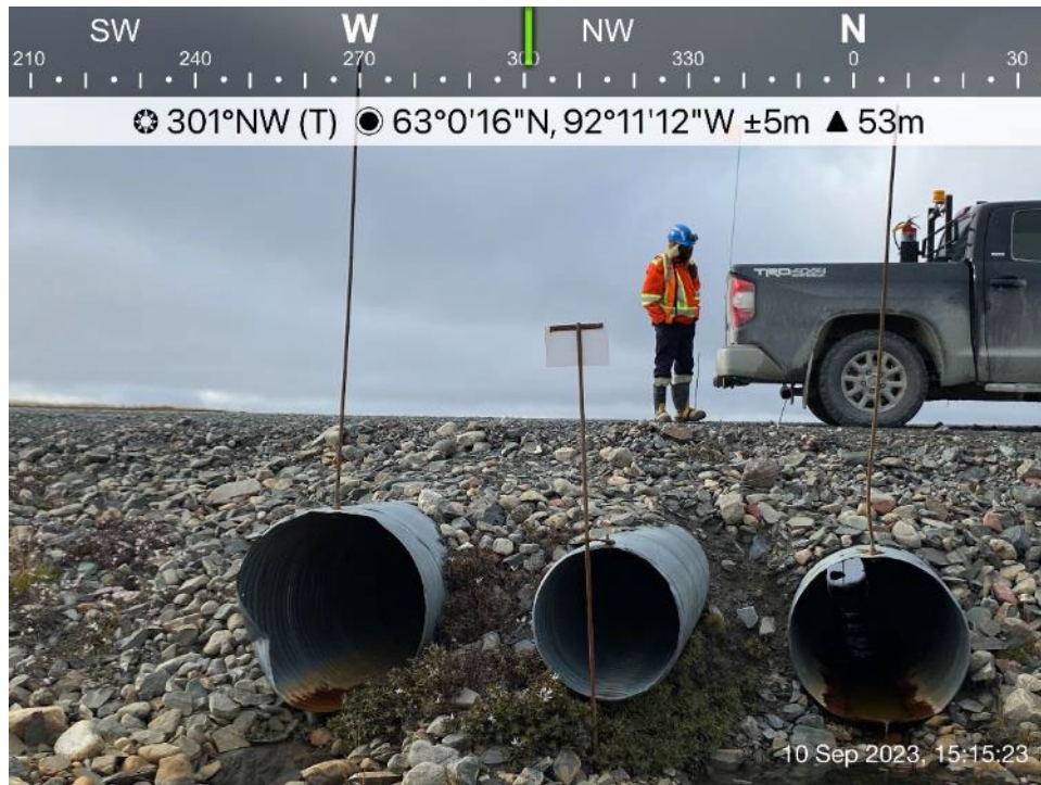
AWAR Road/Culvert - Photo 66: Culvert KM 27.1 – inlet.
