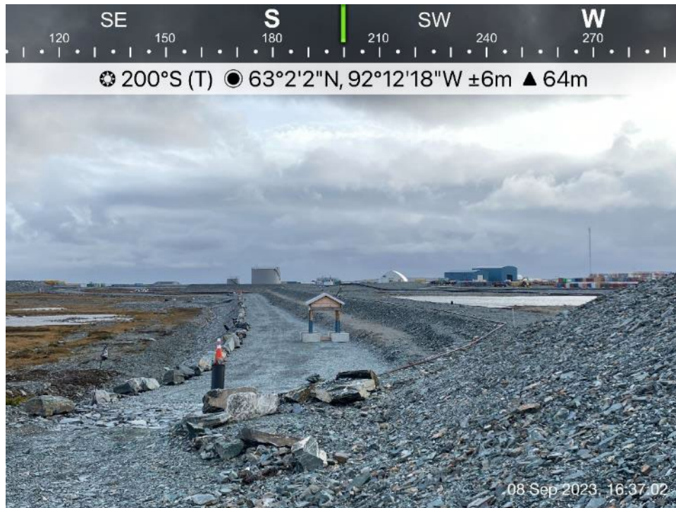
D-CP1 - Photo 7: Dike D-CP1: Dike downstream toe berm view.
