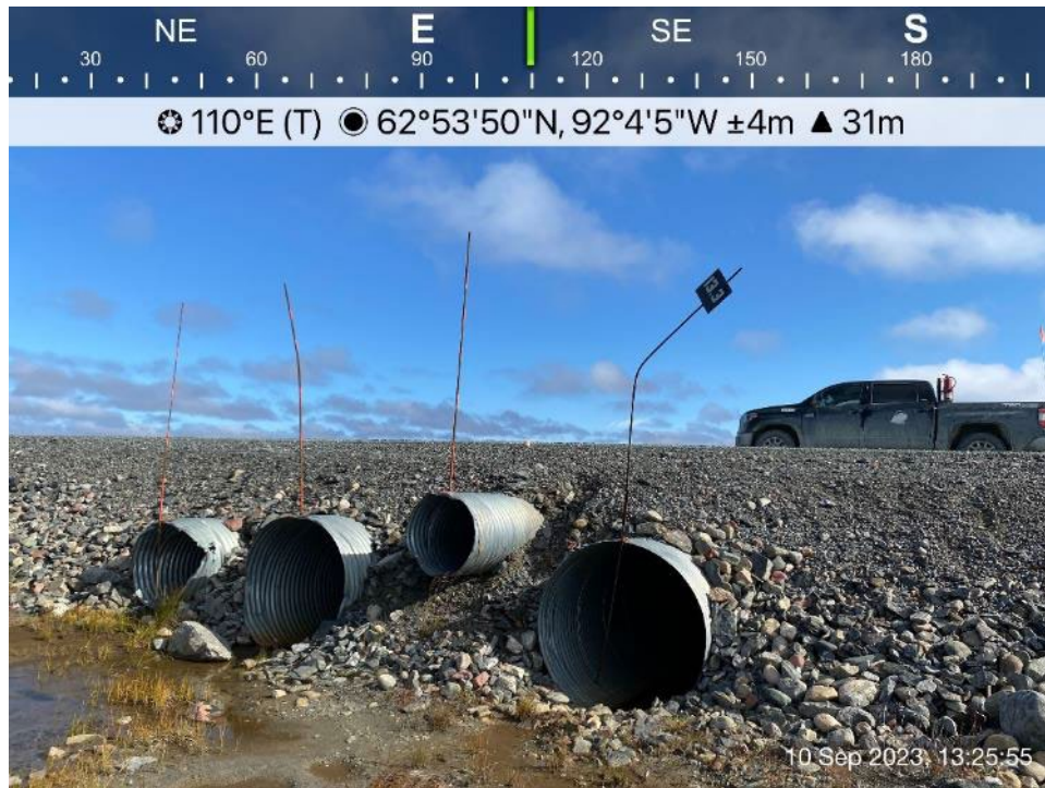
AWAR Road/Culvert - Photo 32: Culvert KM 12.1 – outlet.
