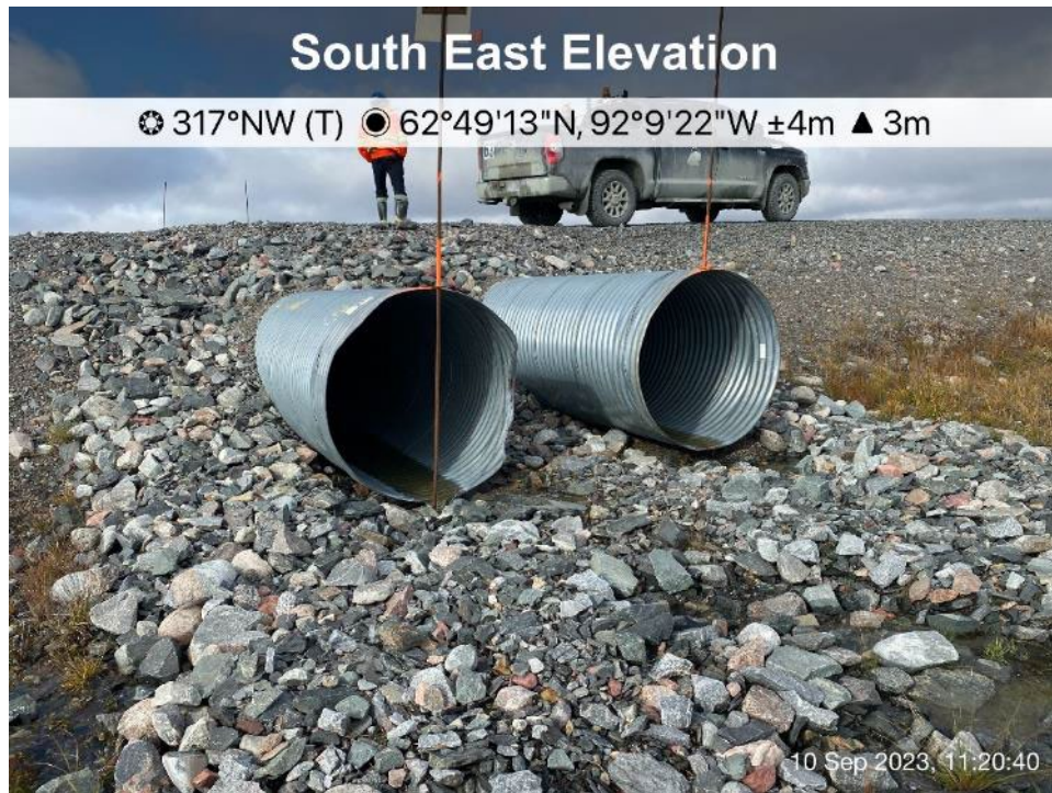
Itivia Bypass Road/Culvert - Photo 34: Culvert C12 inlet.
