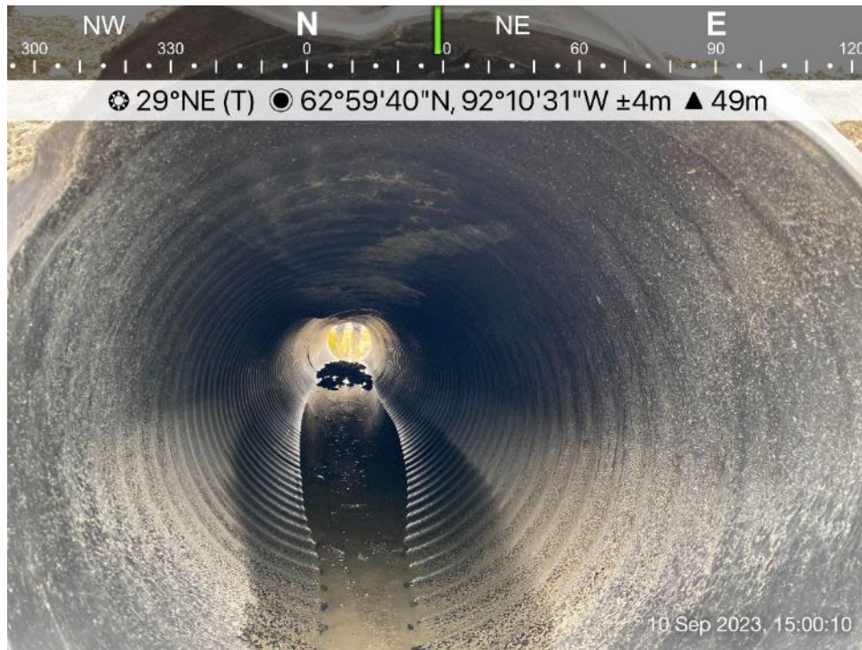
AWAR Road/Culvert - Photo 56: Culvert KM 25.8 - HDPE corrugated culvert – outlet.
