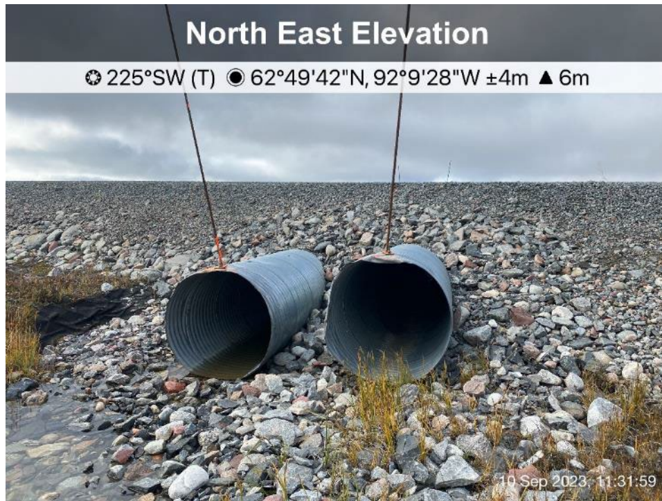
Itivia Bypass Road/Culvert - Photo 42: Culvert C15 inlet.
