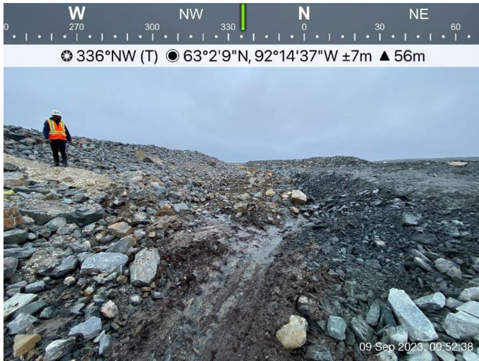
CP3 - Photo 4: CP3 - little water flow from snow stockpile melting to CP3.
