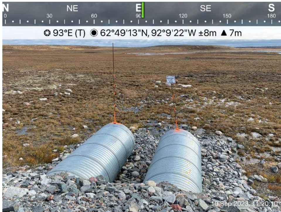
Itivia Bypass Road/Culvert - Photo 33: Culvert C12 inlet.
