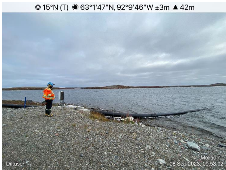
Exploration Camp - Photo 8: Exploration Camp - diffuer pipeline, looking north.
