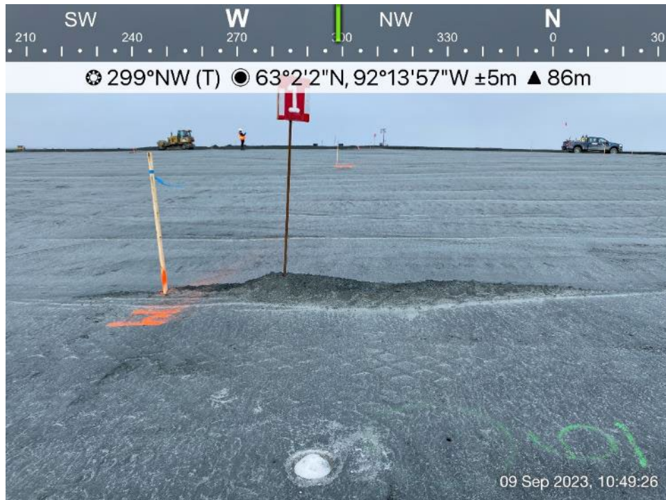
TSF - Photo 7: TSF - Sand cone and nuclear density testing locations.
