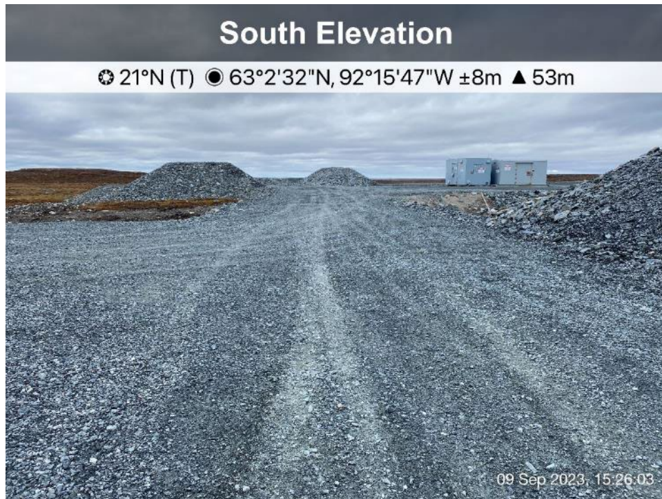
Emulsion Plant Pad - Photo 18: Emulsion Storage Pad - Overview, looking north.
