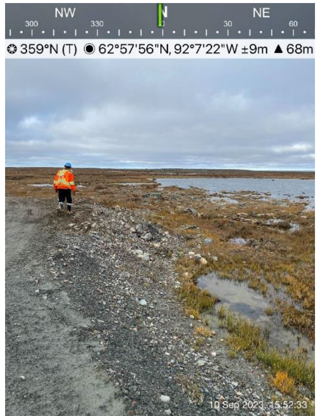
AWAR Road/Culvert - Photo 49: KM 19 - No culvert installed, ponded water upstream, no sign of overflow.
