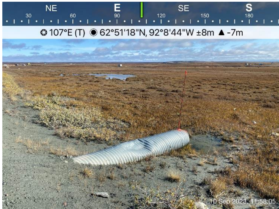
AWAR Road/Culvert - Photo 1: Culvert KM 5.5 - inlet.
