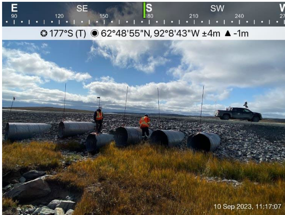
Itivia Bypass Road/Culvert - Photo 31: Culvert C11 inlet.
