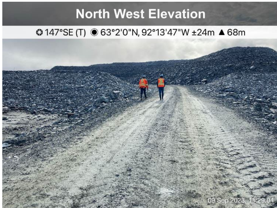
Site Road - Photo 3: Site Road - Landfill access road.
