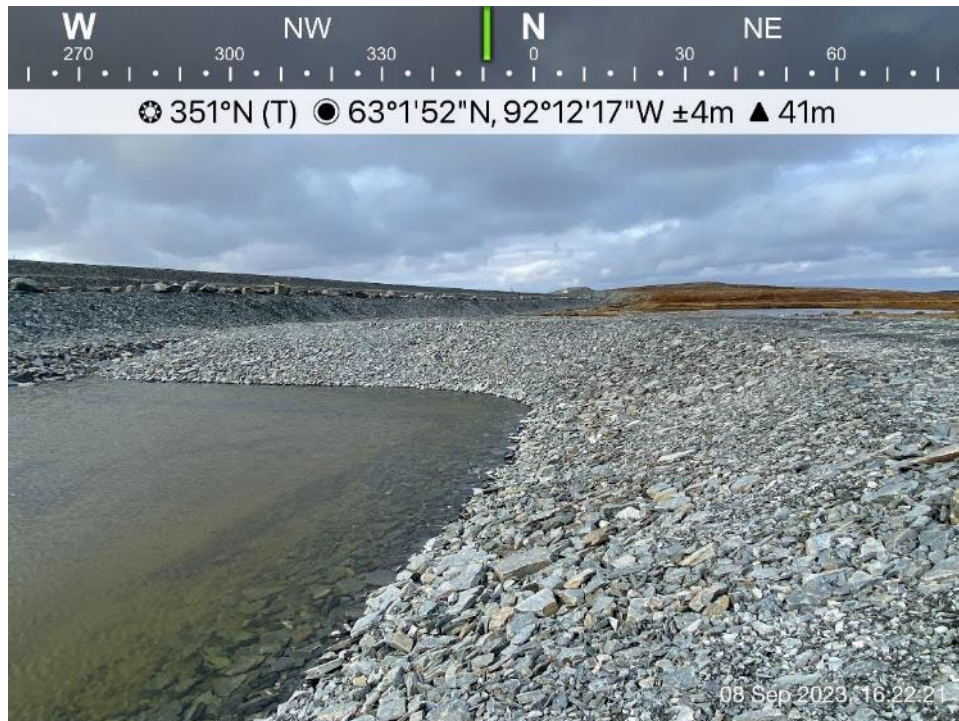
D-CP1 - Photo 10: Dike D-CP1: Dike downstream sump - rockfill berm.
