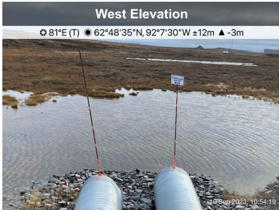
Itivia Bypass Road/Culvert - Photo 21: Culvert C08 inlet.
