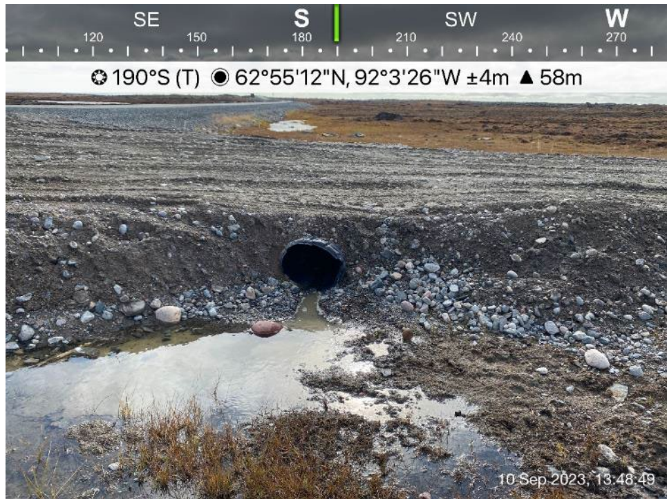
AWAR Road/Culvert - Photo 38: Culvert KM 14.7 - inlet - HDPE corrugated culvert.
