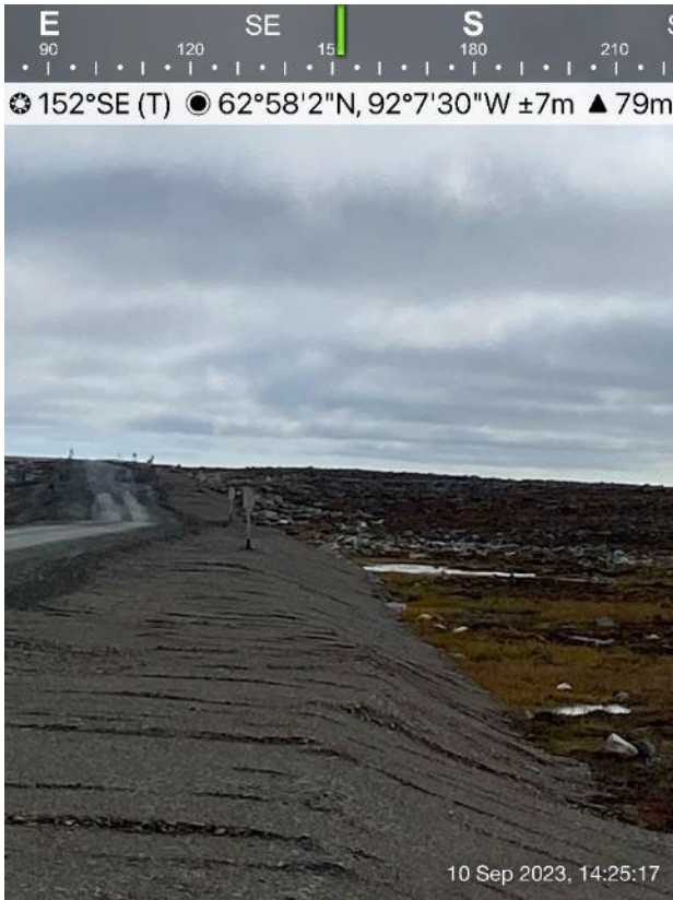
AWAR Road/Culvert - Photo 51:
