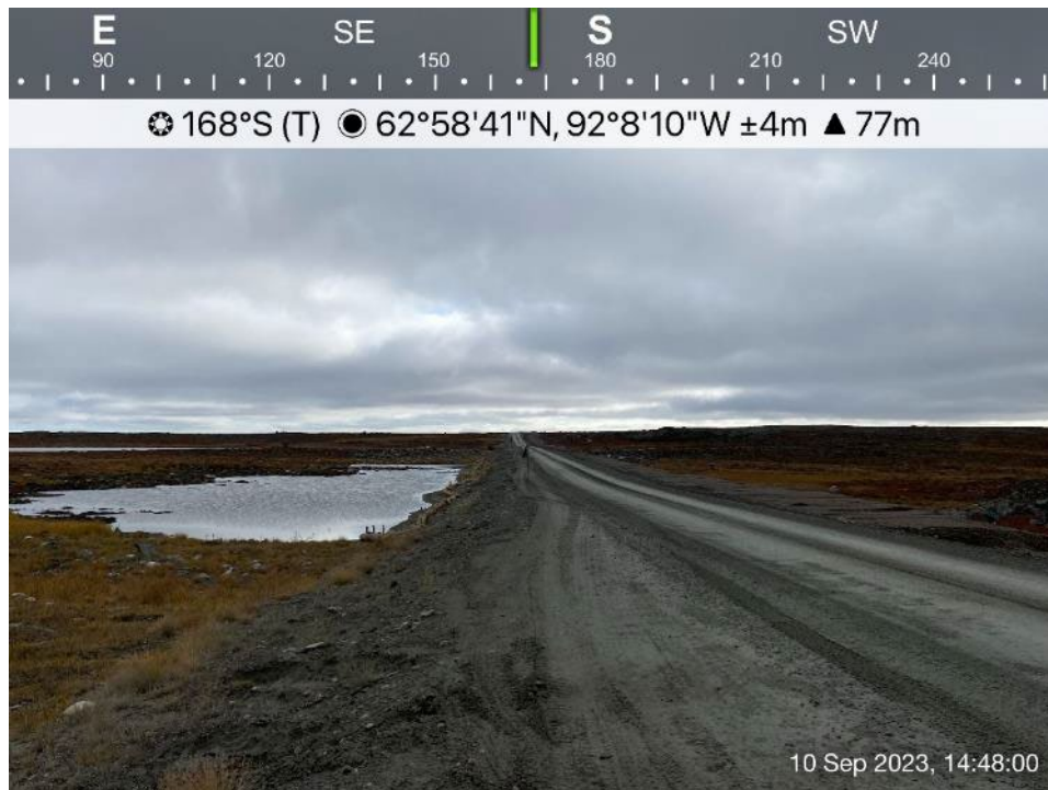
AWAR Road/Culvert - Photo 54:
