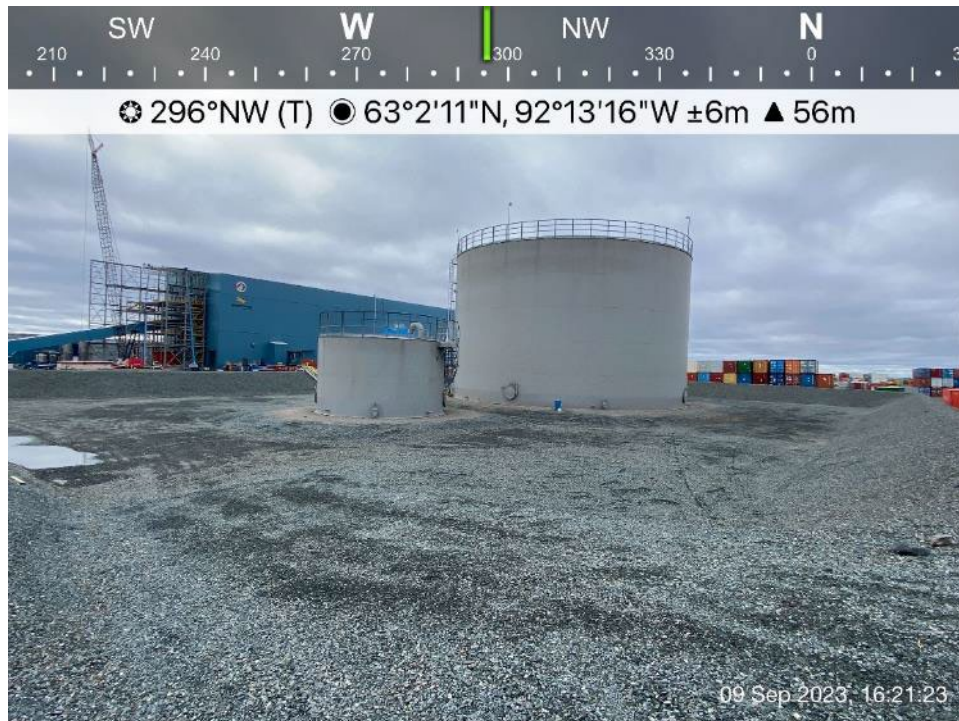
Industrial Fuel Tanks -Photo 23: Industrial Fuel Tanks - Overview, looking northwest.
