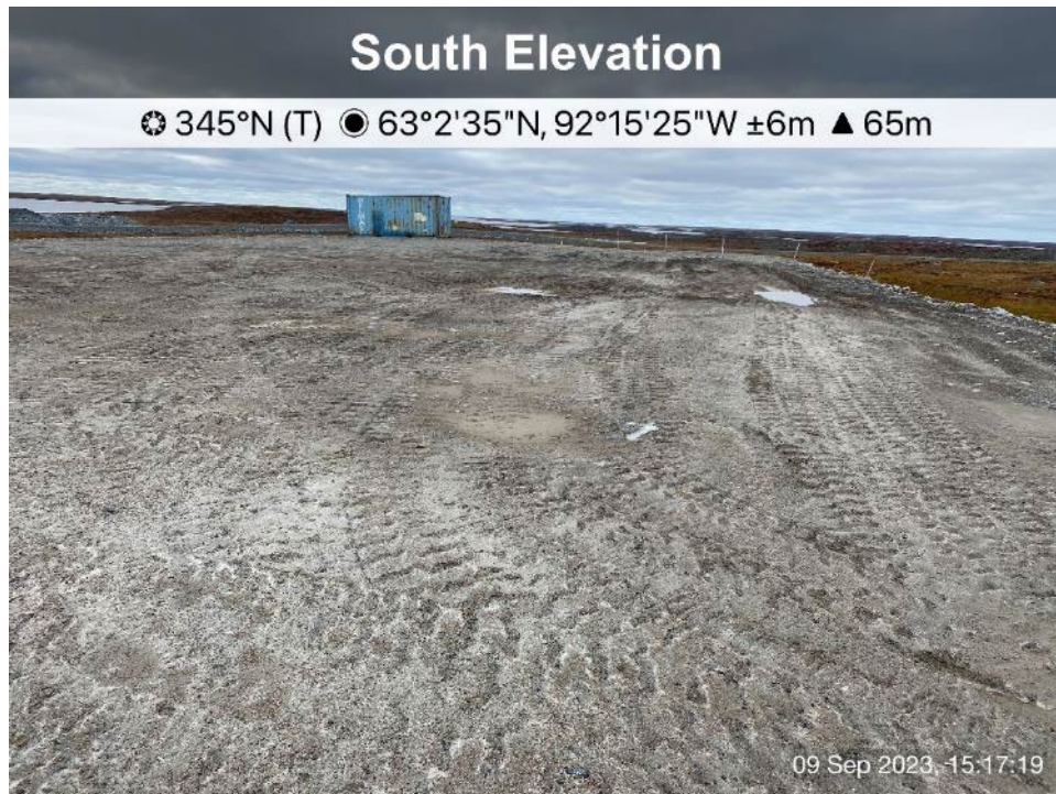
Emulsion Plant Pad - Photo 14: Emulsion Plant Pad - Overview, looking north.
