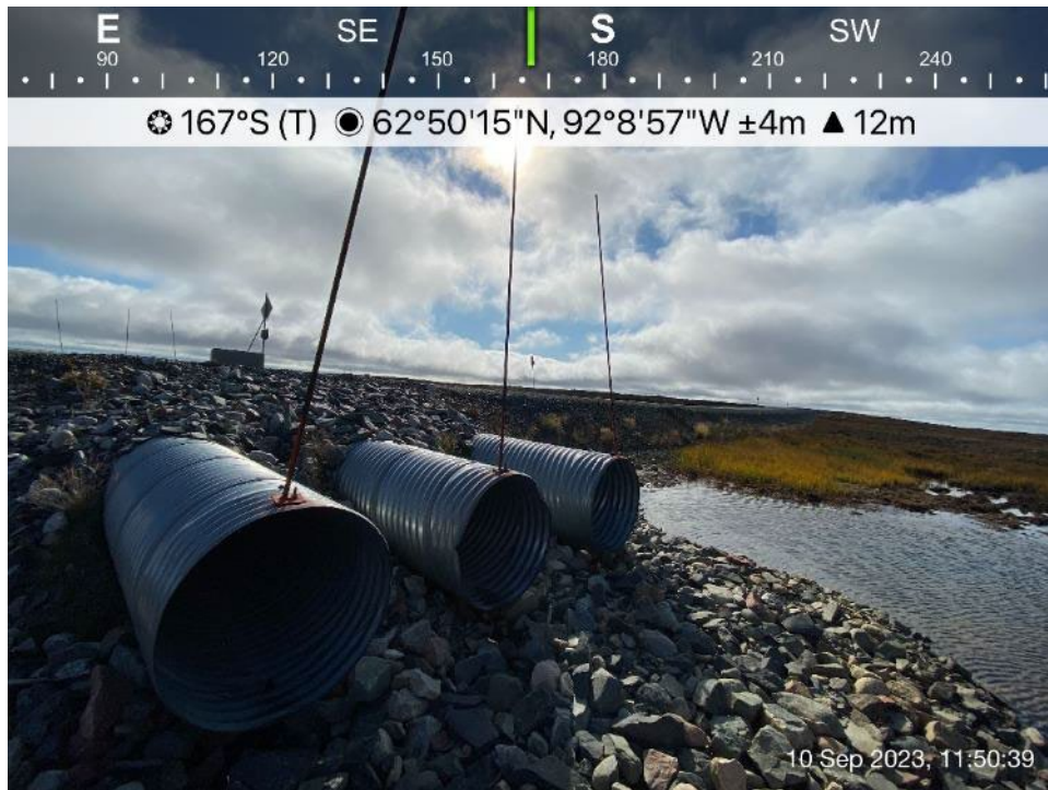
Itivia Bypass Road/Culvert - Photo 55: Culvert C19 outlet.
