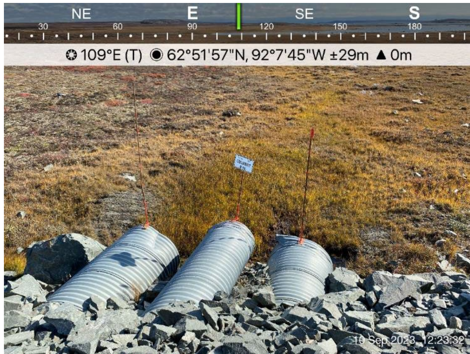
AWAR Road/Culvert - Photo 12: Culvert KM 7.1 - inlet.
