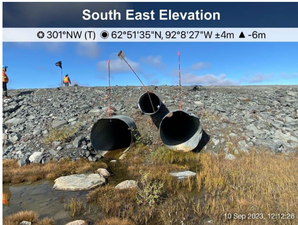
AWAR Road/Culvert - Photo 7: Culvert KM 6.2 - inlet.
