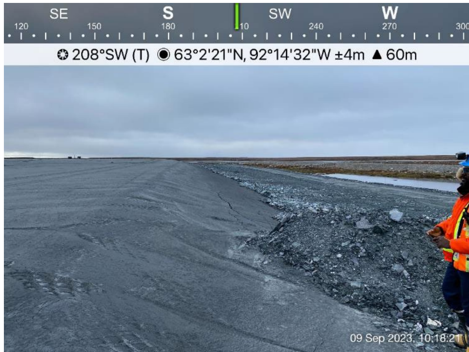
TSF - Photo 12: TSF - Rockfill cover and north slope of TSF Cell 2.
