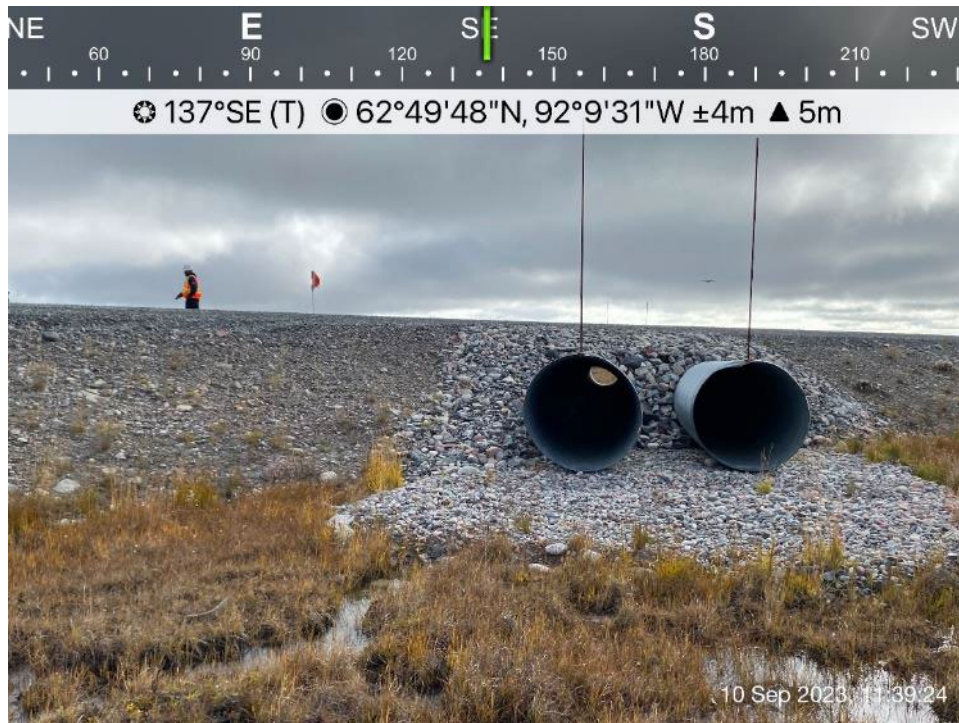
Itivia Bypass Road/Culvert - Photo 49: Culvert C17 outlet.
