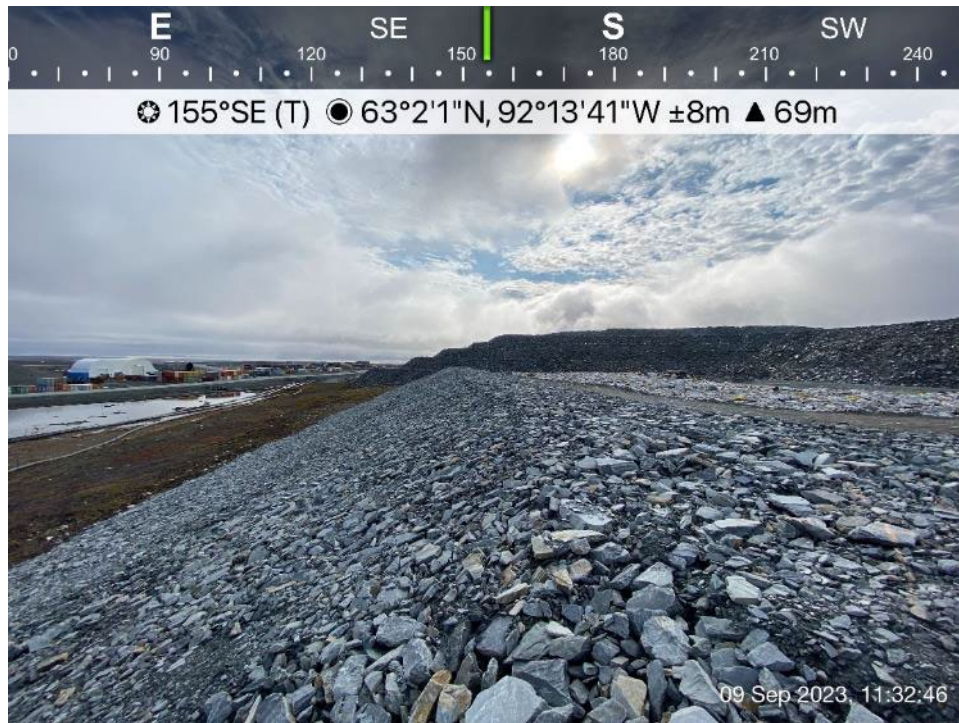
Landfill - Photo 10: WRSF1 Landfill- landfill west side slope, looking southeast.
