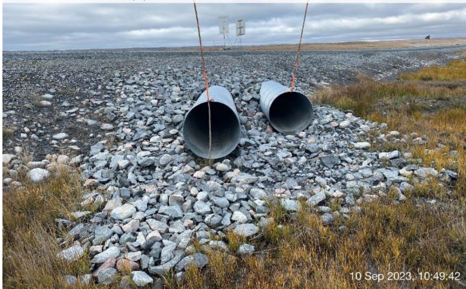
Itivia Bypass Road/Culvert - Photo 16: Culvert C06 inlet.
