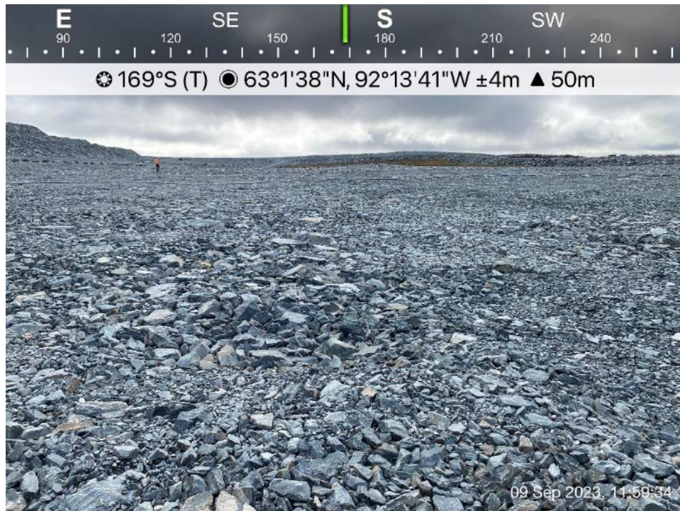
CP4 Thermal Berm - Photo 7: CP4 Thermal Berm - Looking south, even surface due to thaw settlement observed from the crest.
