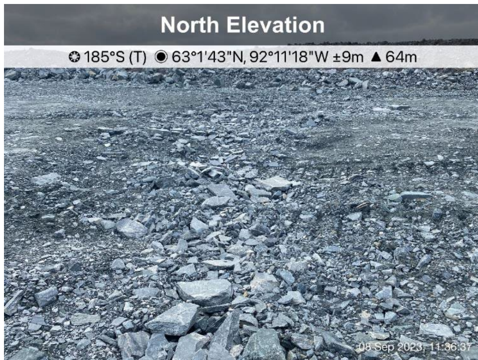
WRSF3- Photo 2: WRSF 3 - depression area observed on Bench 72 m.
