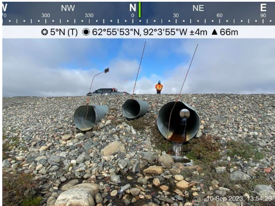
AWAR Road/Culvert - Photo 42: Culvert KM 16.3 – outlet.
