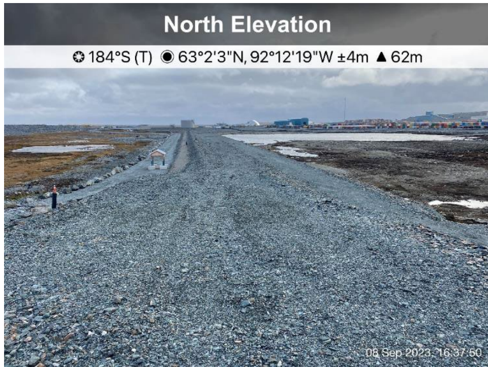
D-CP1 - Photo 4: Dike D-CP1: Dike crest view - downstream on left, upstream on right.
