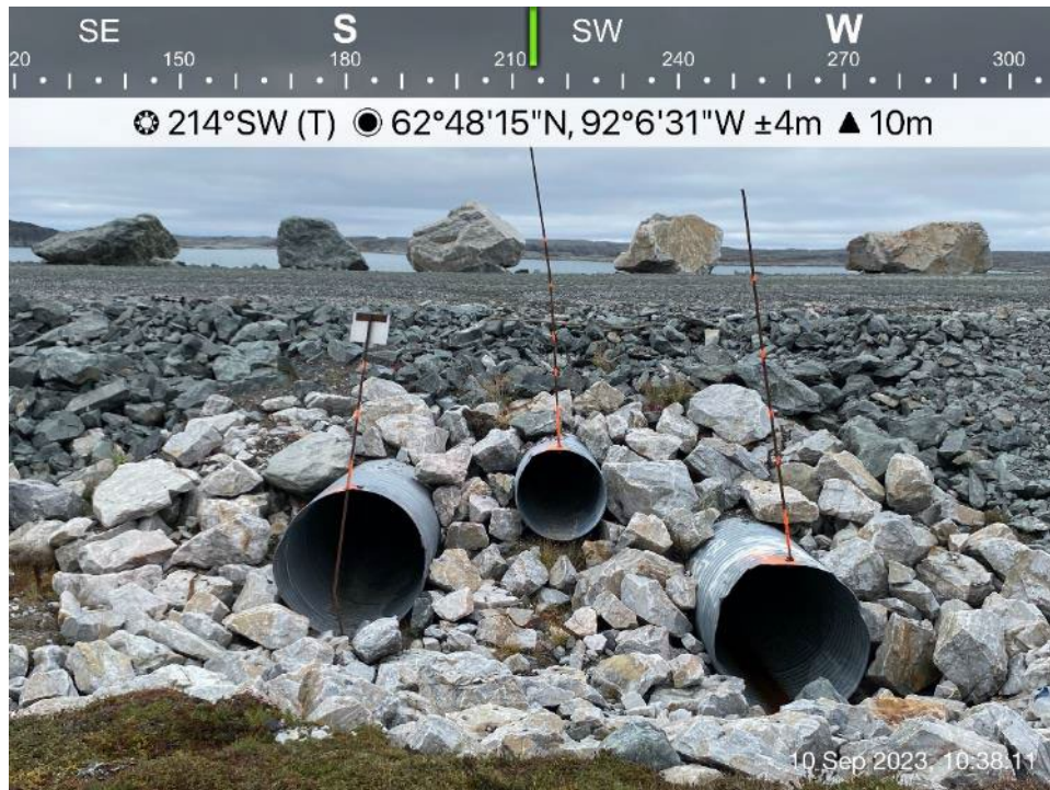
Itivia Bypass Road/Culvert - Photo 7: Culvert C03 inlet.
