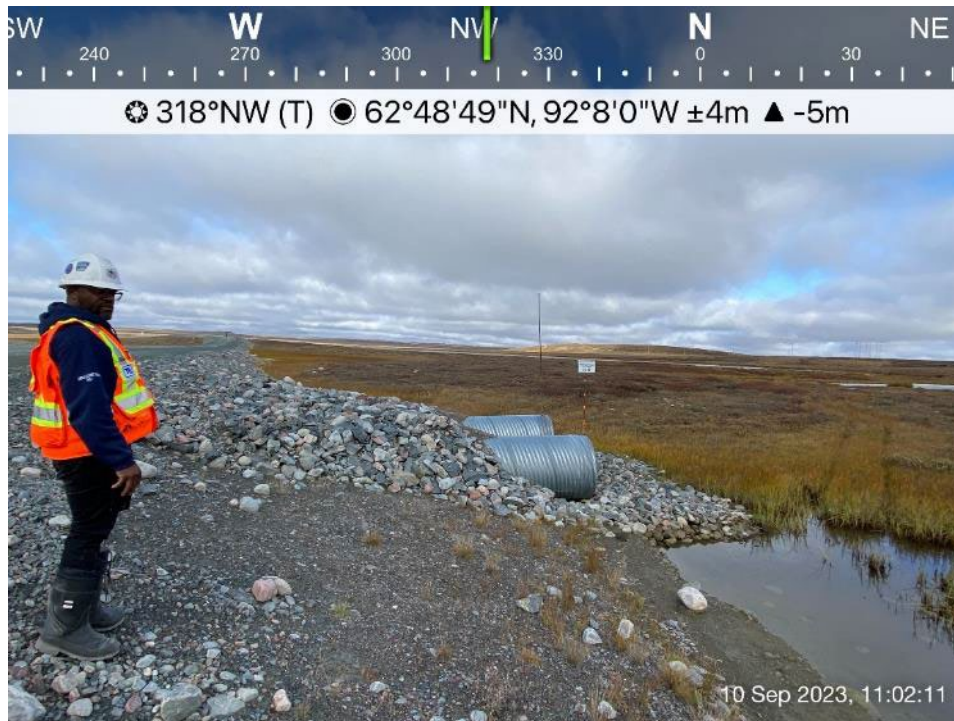
Itivia Bypass Road/Culvert - Photo 27: Culvert C10 inlet.
