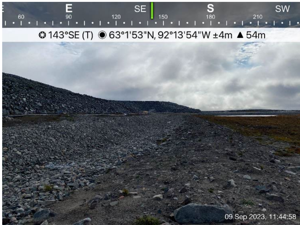
Channel 4 - Photo 10: Channel 4 - Looking southeast, WRSF1 in the background.
