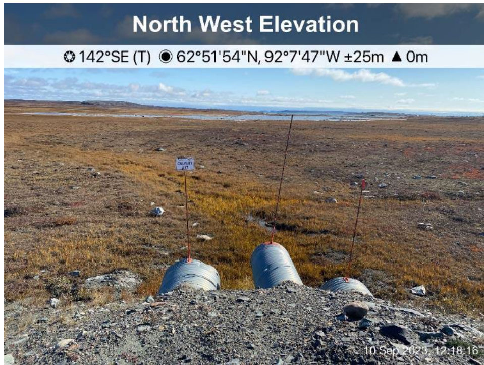
AWAR Road/Culvert - Photo 9: Culvert KM 7.0 - inlet.
