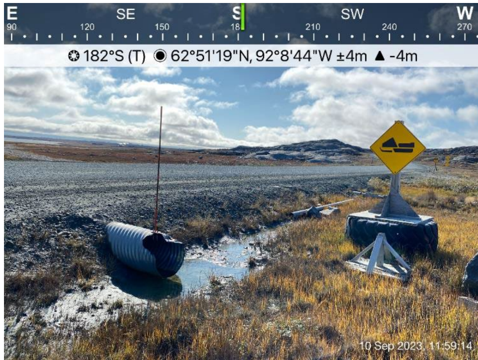
AWAR Road/Culvert - Photo 2: Culvert KM 5.5 - outlet.
