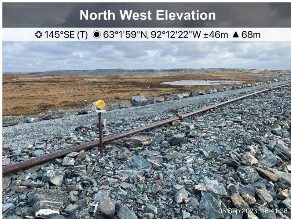
D-CP1 - Photo 14: Dike D-CP1: Dike survey control point.
