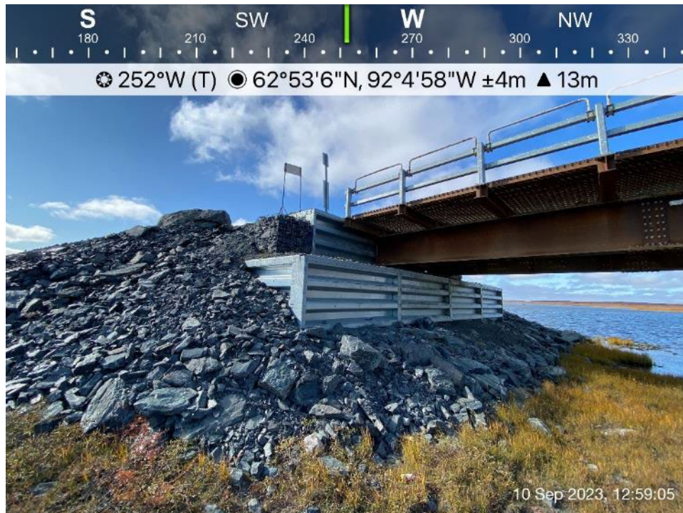
AWAR Road/Culvert - Photo 29: M-5 Bridge KM 10.5- south abutment.
