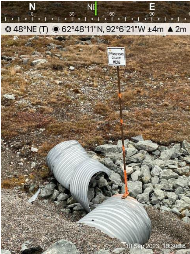
Itivia Bypass Road/Culvert Culvert C02 Inlet. - Photo 3:
