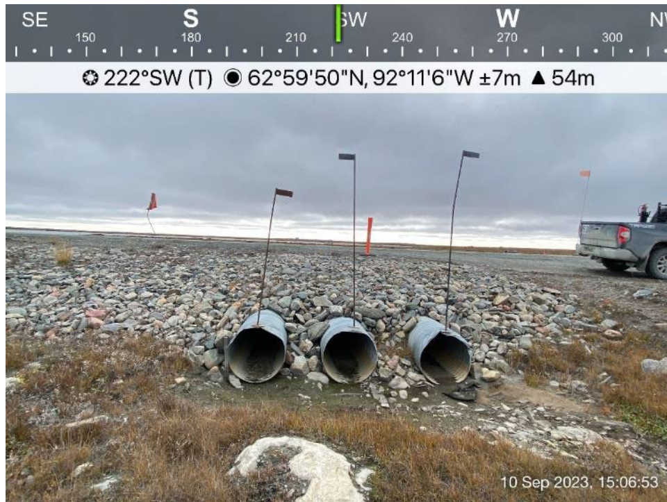
AWAR Road/Culvert - Photo 61: Culvert KM 26.5 – inlet.
