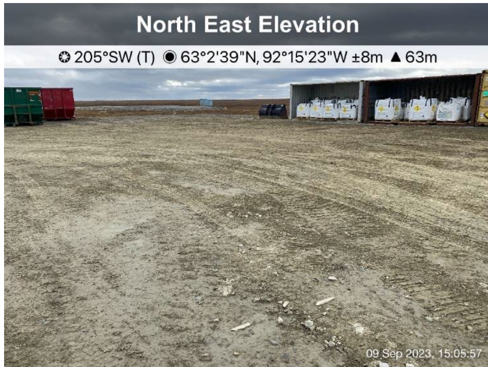
Emulsion Plant Pad - Photo 16: Emulsion Plant Pad - Overview, looking southwest.
