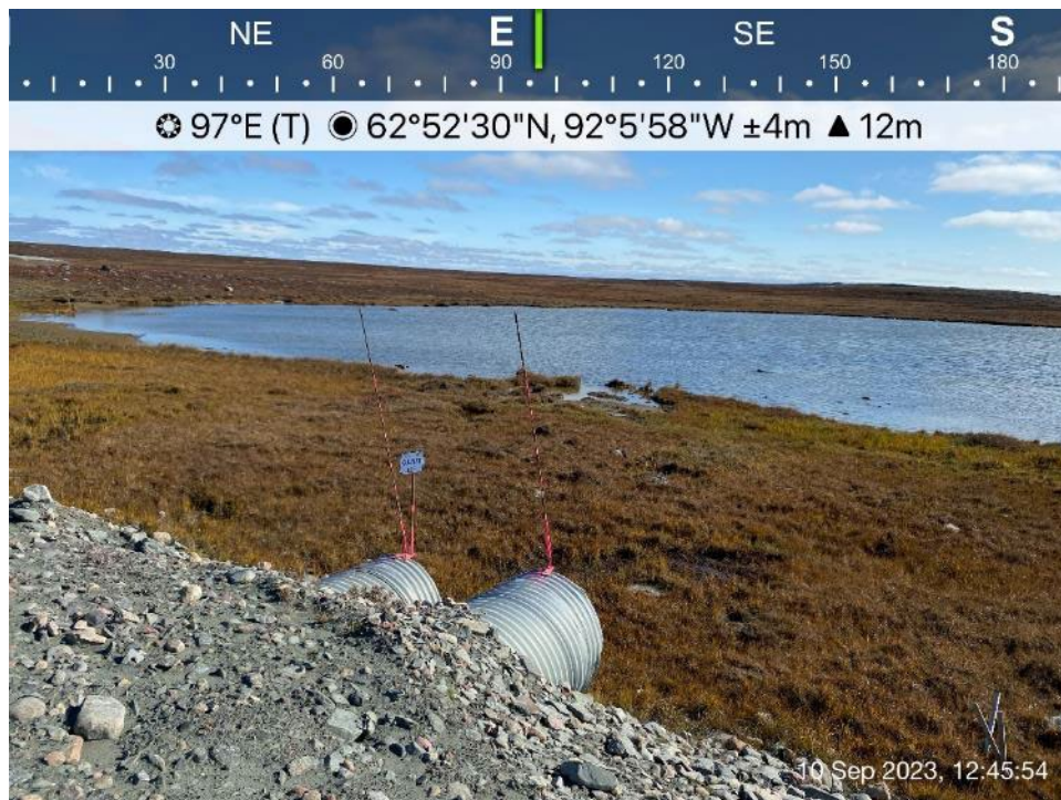
AWAR Road/Culvert - Photo 22: Culvert KM 9.1 – inlet.
