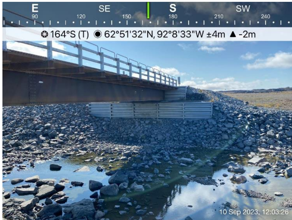
AWAR Road/Culvert - Photo 4: Char River Bridge KM 6.1 - north abutment.
