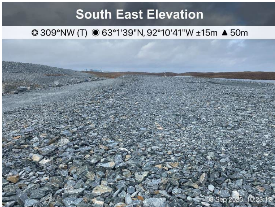
CP2 Thermal Berm - Photo 4:
