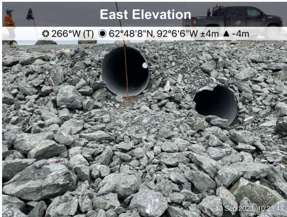
Itivia Bypass Road/Culvert - Photo 1: Culvert C01 Inlet.
