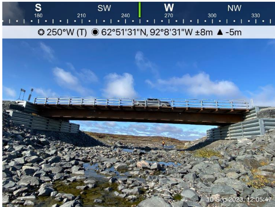
AWAR Road/Culvert - Photo 3: Char River Bridge KM 6.0.
