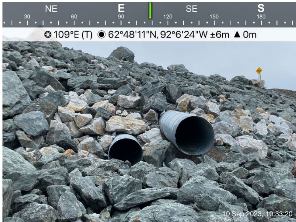
Itivia Bypass Road/Culvert - Photo 5: Culvert C02 outlet.
