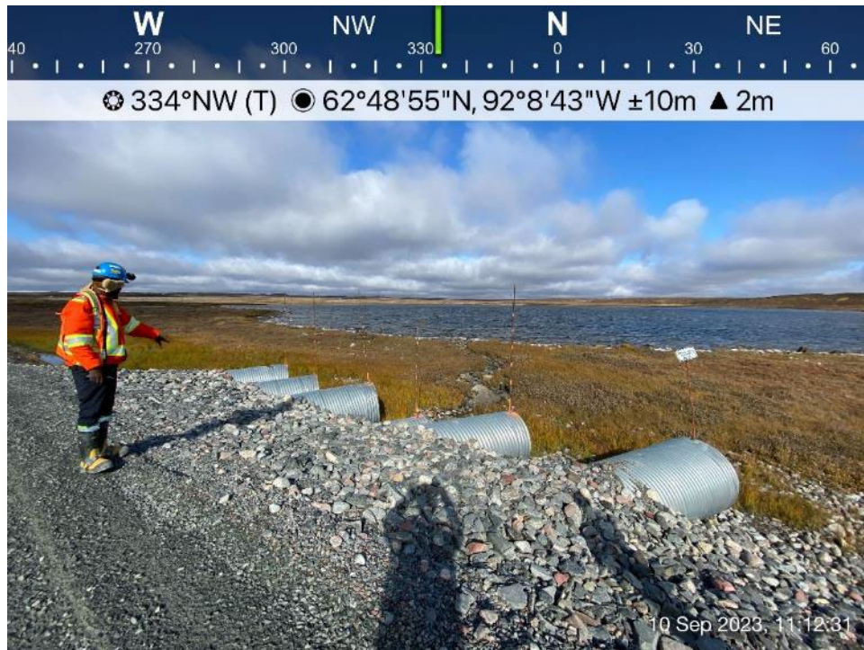
Itivia Bypass Road/Culvert - Photo 30: Culvert C11 inlet.
