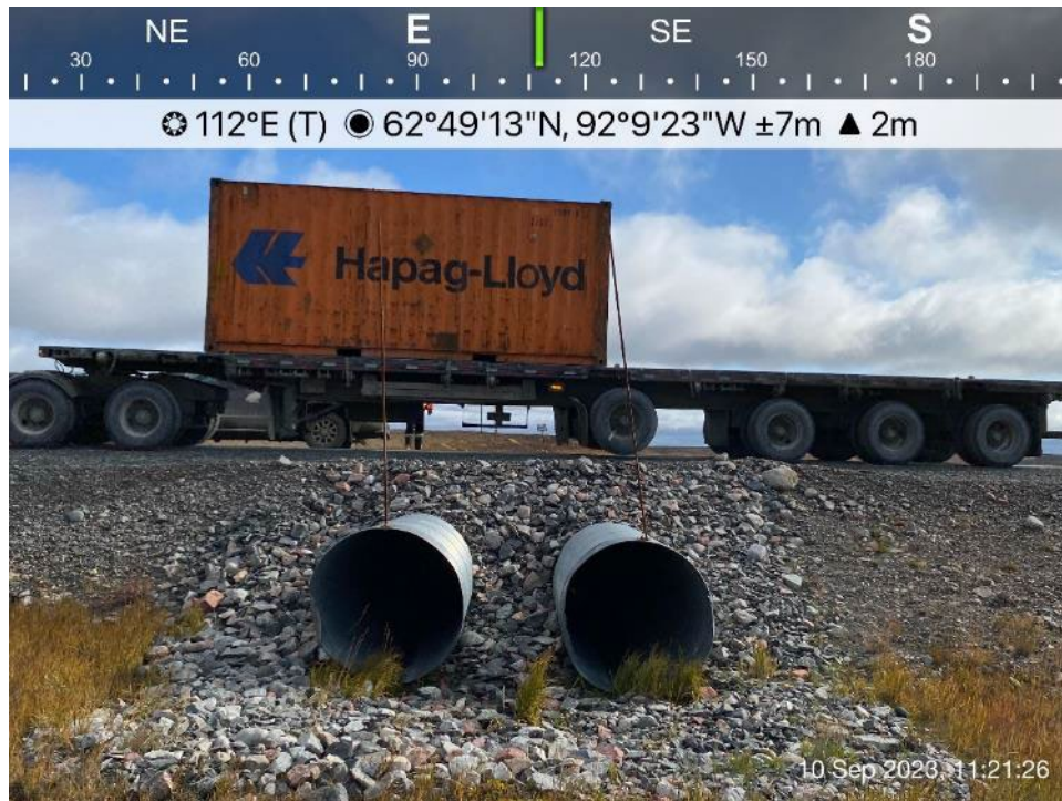
Itivia Bypass Road/Culvert - Photo 35: Culvert C12 outlet.
