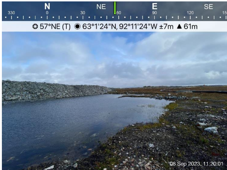
WRSF3- Photo 7: WRSF3 - Poned water observed at southwest corner of WRSF3, looking northeast.
