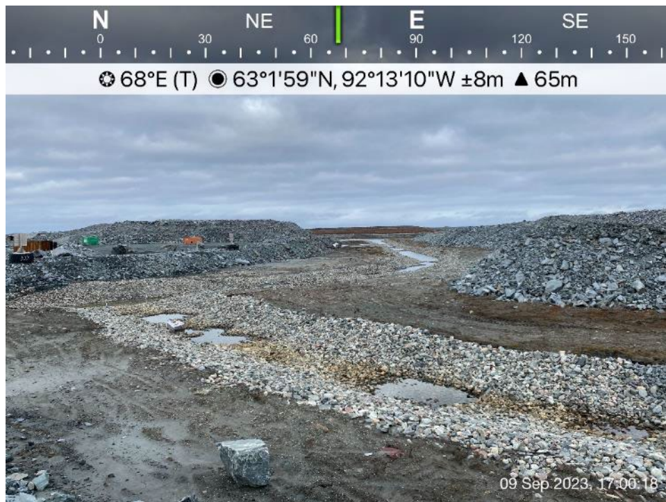
Channel 7 - Photo 16: Channel 7 -Outlet into Channel 1, minor water ponding and thaw subsidence, ore stockpiles in the background.
