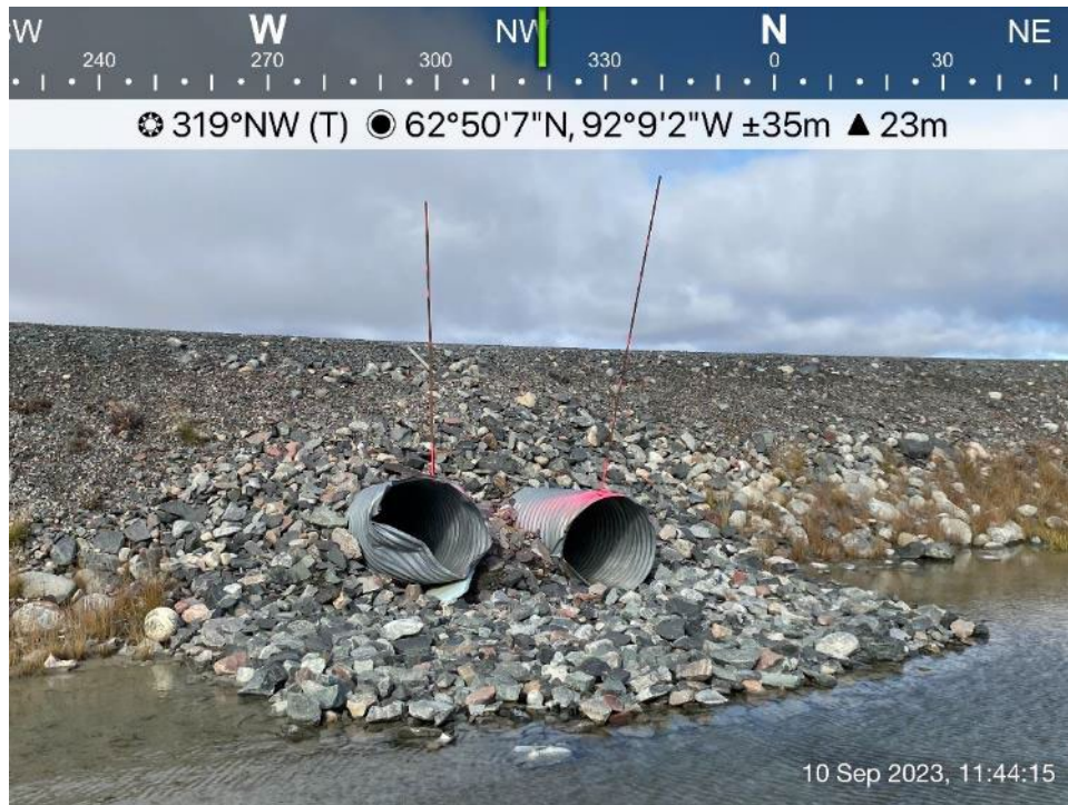
Itivia Bypass Road/Culvert - Photo 51: Culvert C18 inlet.
