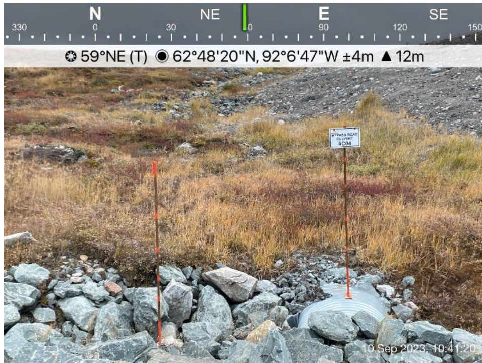
Itivia Bypass Road/Culvert - Photo 9: Culvert C04 inlet.
