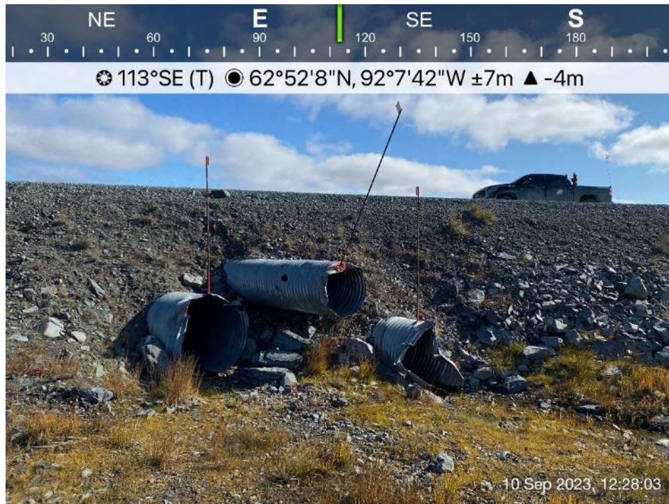
AWAR Road/Culvert - Photo 16: Culvert KM 7.4 – outlet.
