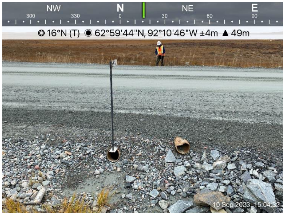
AWAR Road/Culvert - Photo 59: Culvert KM 26.2 - steel pipe as culvert, outlet.
