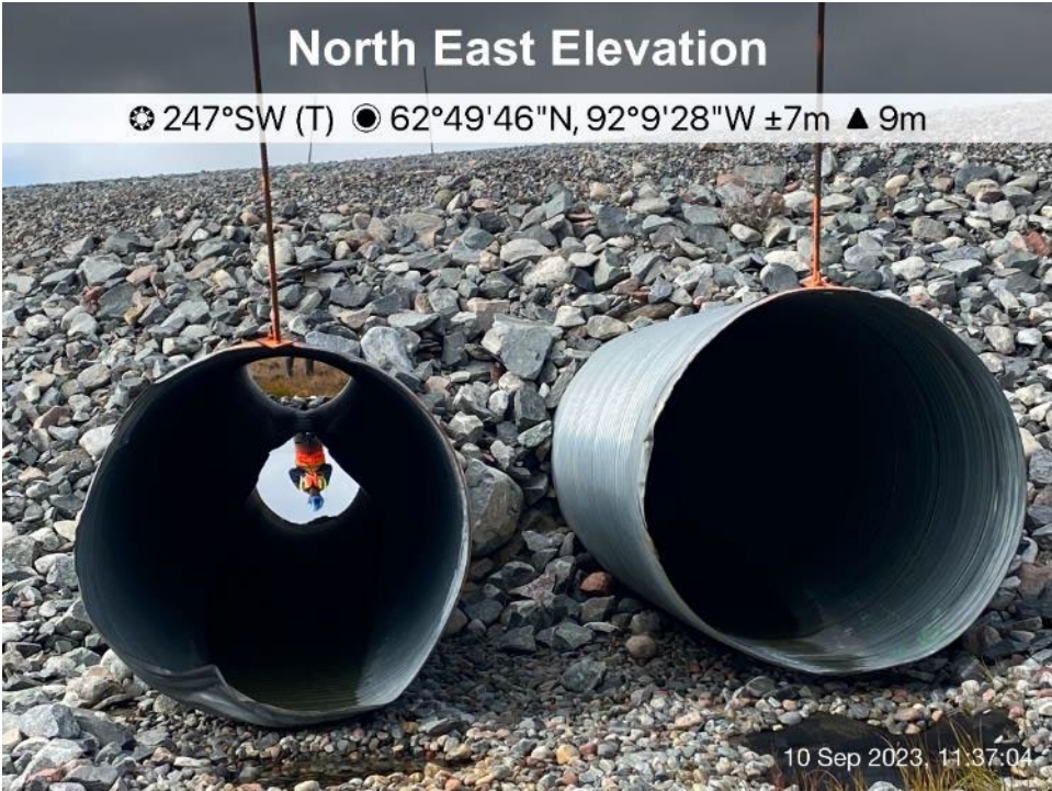
Itivia Bypass Road/Culvert - Photo 45: Culvert C16 inlet.
