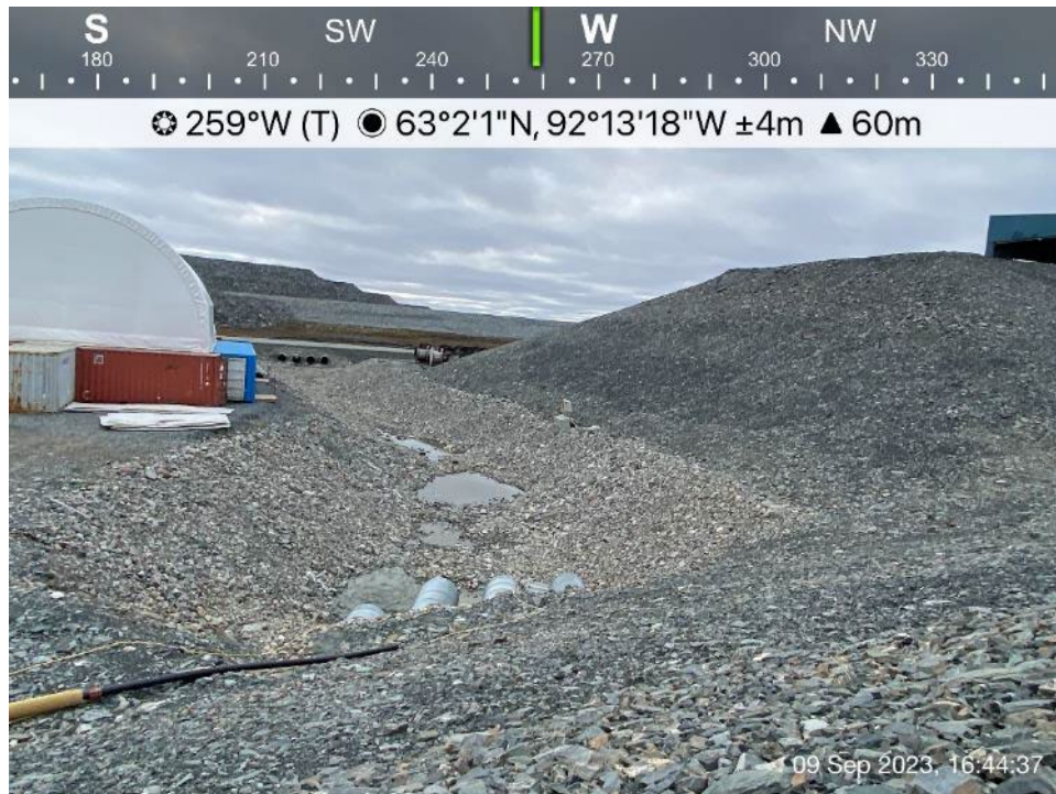
Channel 1 - Photo 2: Channel 1 - Crusher ramp embankment to the right, looking west.
