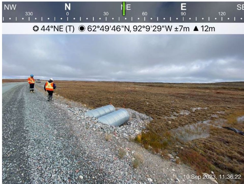
Itivia Bypass Road/Culvert - Photo 44: Culvert C16 inlet.
