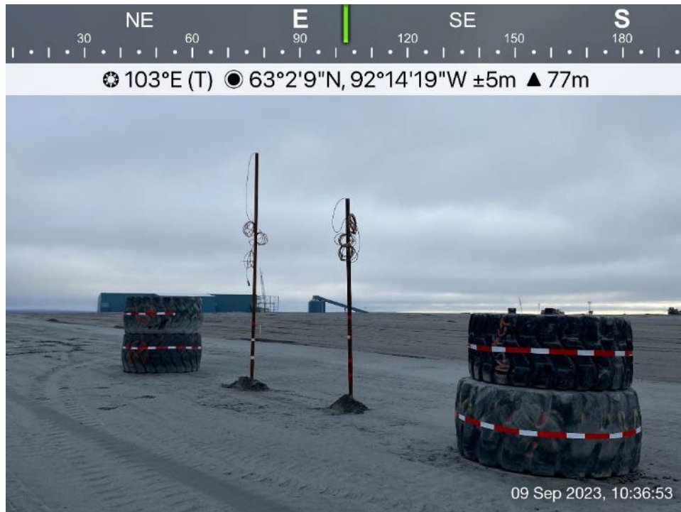
TSF - Photo 11: TSF - GTCs installed in the TSF.
