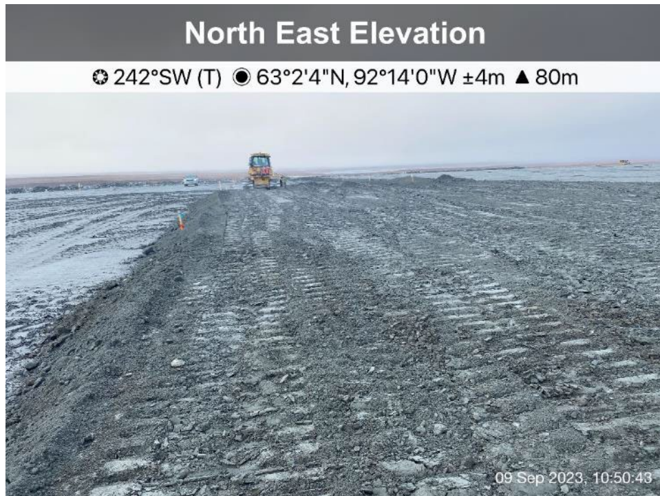
TSF - Photo 9: TSF - Spreading tailings following 0.3 m thick lift control.
