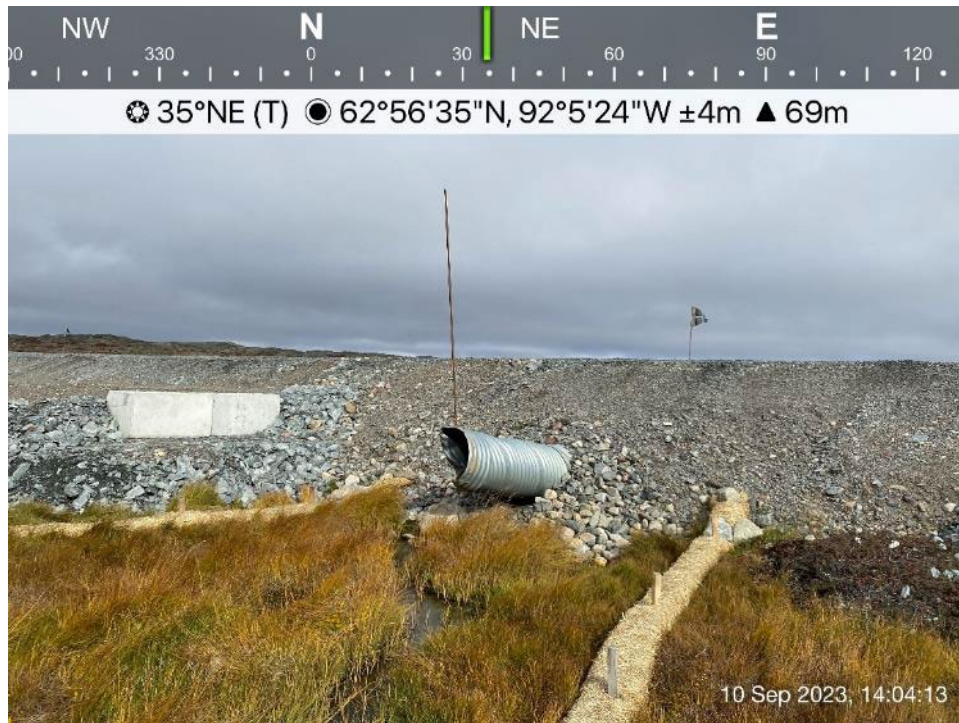
AWAR Road/Culvert - Photo 47: Culvert KM 18.15 – outlet.
