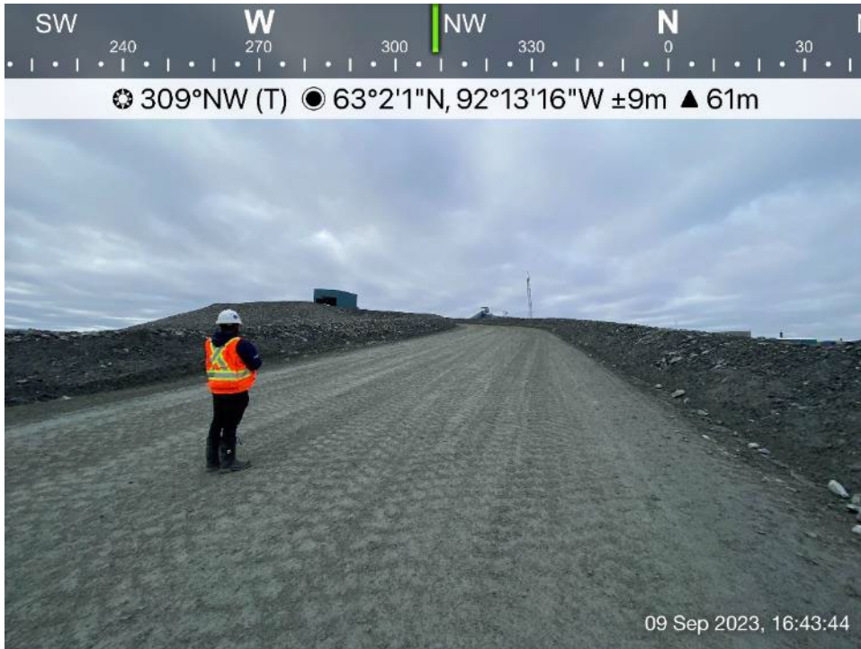
Site Road - Photo 6: Site Road - Crusher access ramp road.
