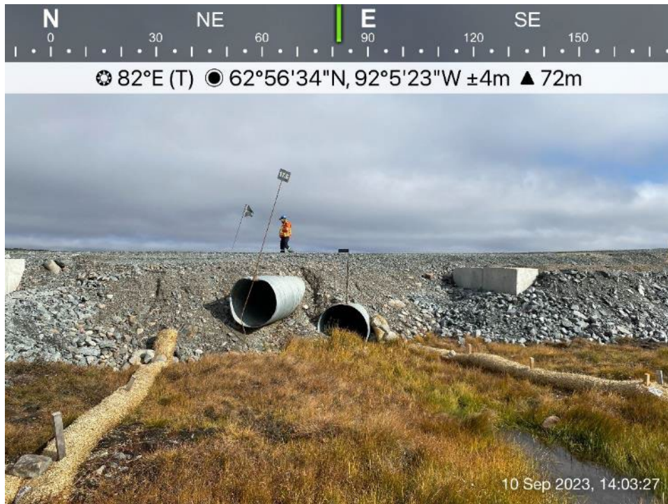
AWAR Road/Culvert - Photo 45: Culvert KM 18.1- outlet.
