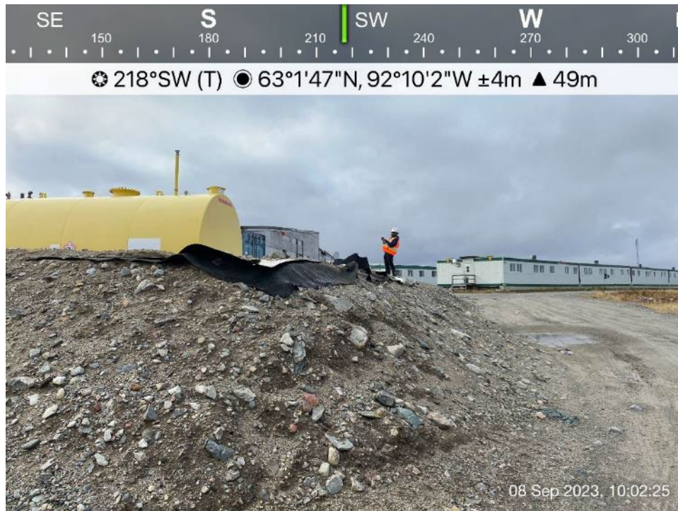
Exploration Camp - Photo 2: Exploration Camp - Fuel storage, looking southwest.
