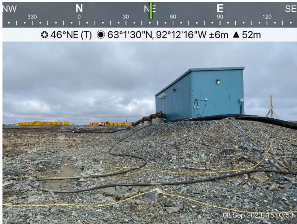
CP5 - Photo 7: CP5 - Jetty and pumping house.
