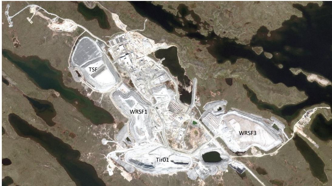
Figure 5: General site plan view with TIR01 open pit identified in addition to other site facilities.
