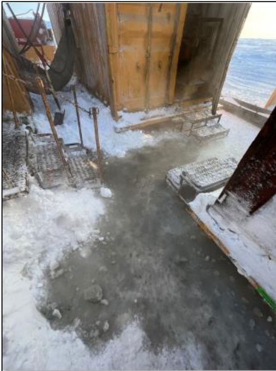
Photo 1: Drill cutting water spill.
