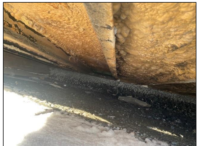
Photo 4: Spill remediation area.
