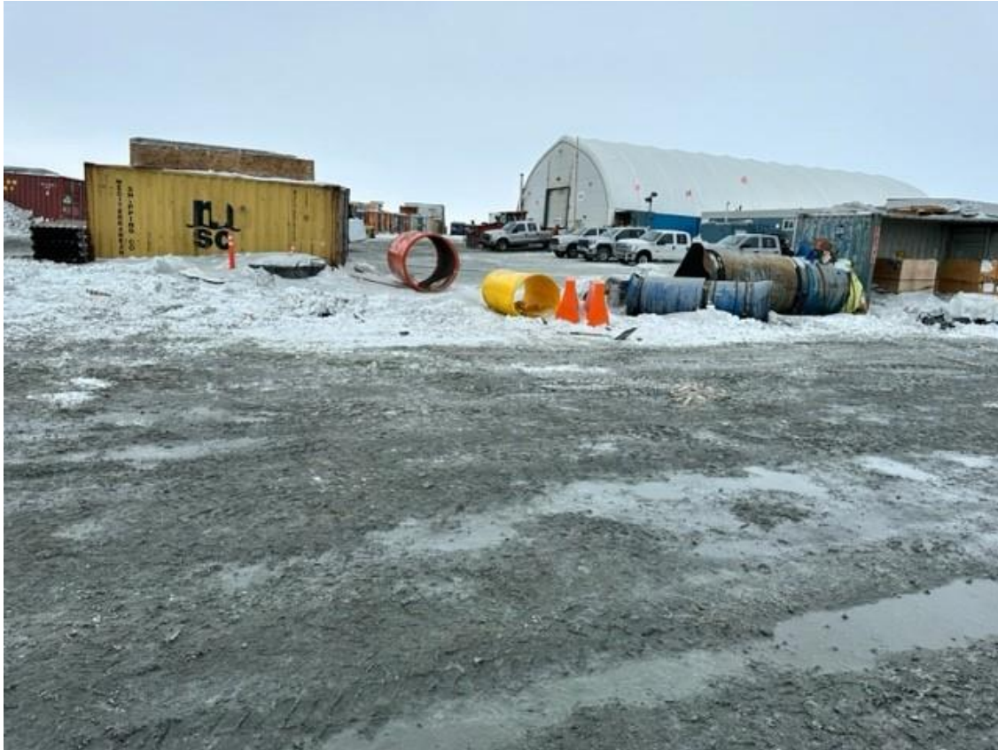
Photo 1: Post cleanup area
