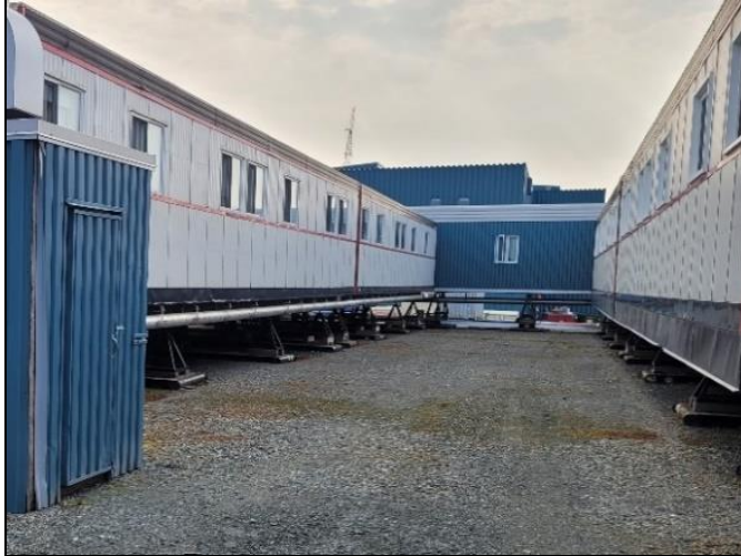
Photo 1: Sewage spill location.
