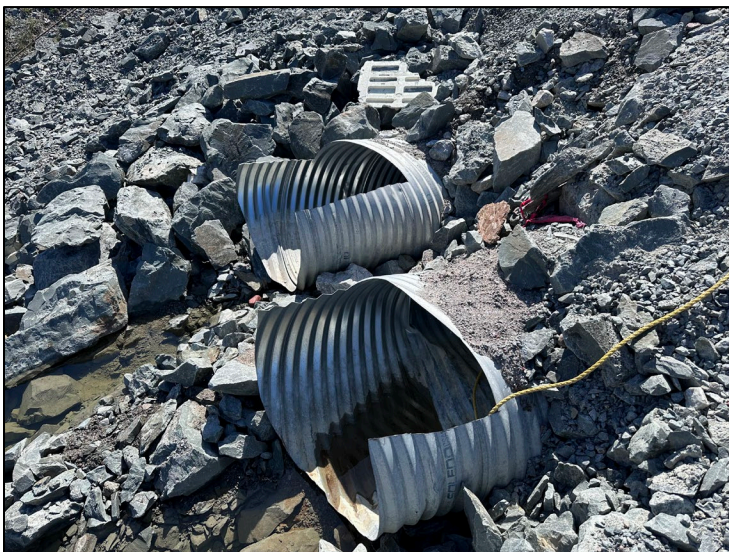
Photo 3 – Temporary repair to the culvert inlets.
