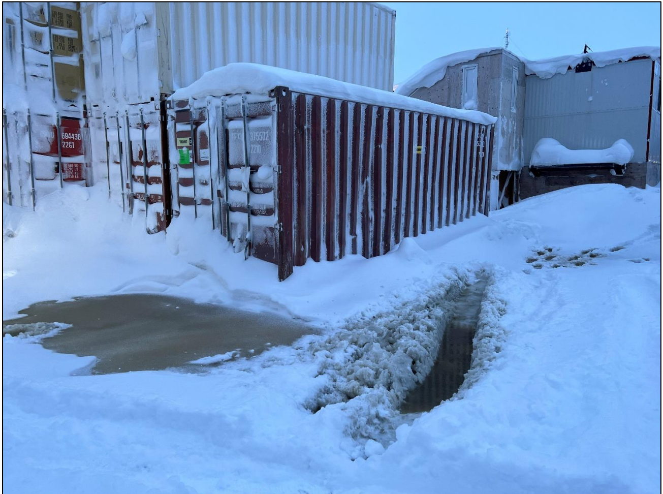
Photo 1: Sewage spill location.
