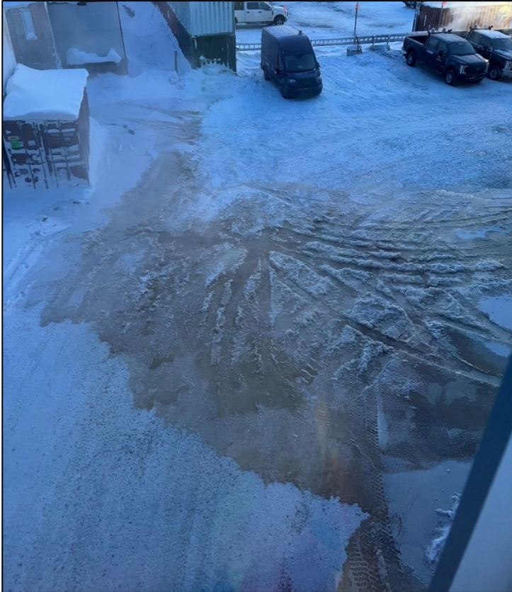
Photo 1: Sewage spill location.
