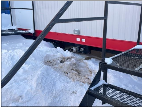
Photo 1: 20 L Sewage spill at powerplant washcar.
