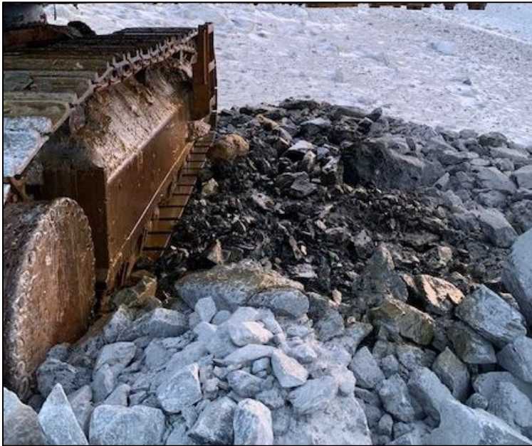
Photo 1: Hydraulic oil spill area.
