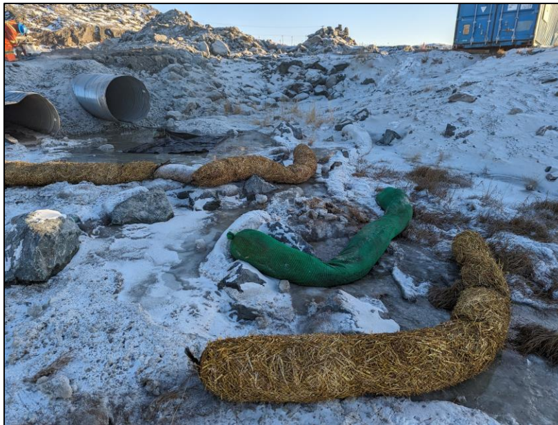
Figure 4: Sediment dewatering bag and straw/wood chip wattles installed downstream.
