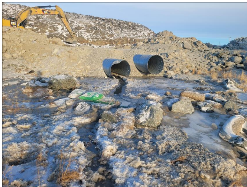
Figure 3: Discharge of pump dewatering downstream of Itivia culverts.
