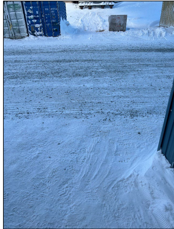
Photo 2: Sewage spill post remediation.
