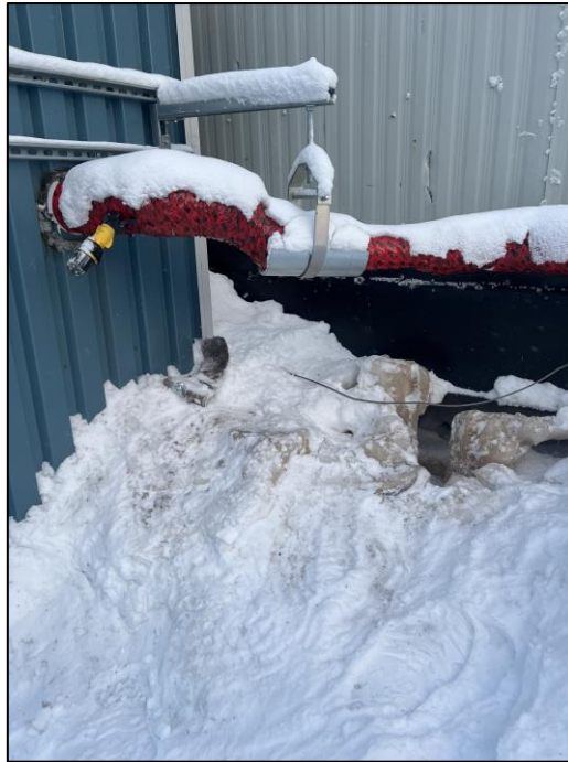
Photo 2: Spill location post snow removal.
