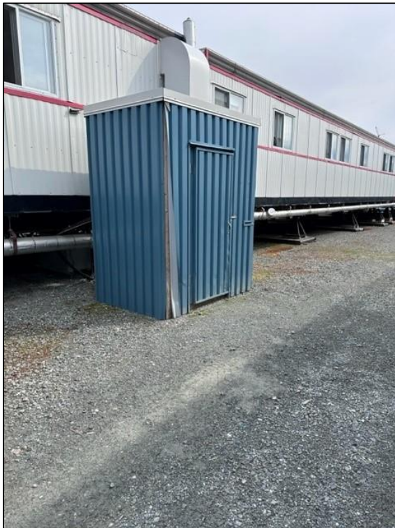
Photo 2: Sewage spill location post-remediation.
