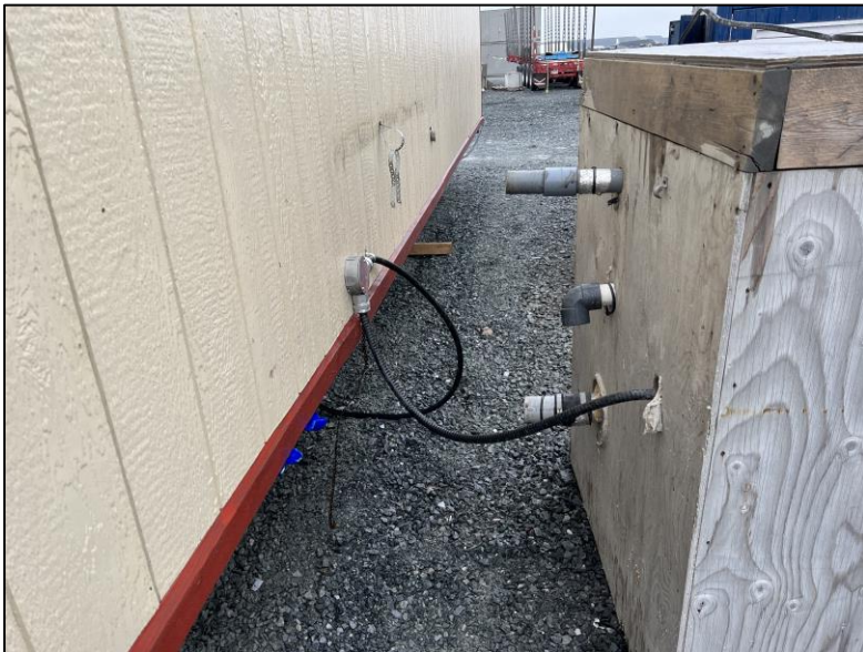
Photos 2: Spill location post remediation.
