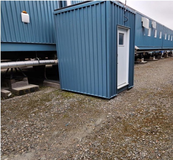
Photos 3 and 4: Spill location post remediation.
