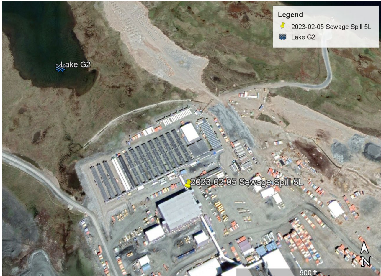
Figure 1: Location of the sewage spill and proximity to water bodies.
