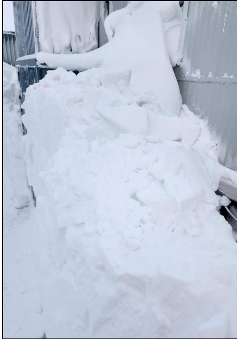
Photo 1: Sewage spill location.
