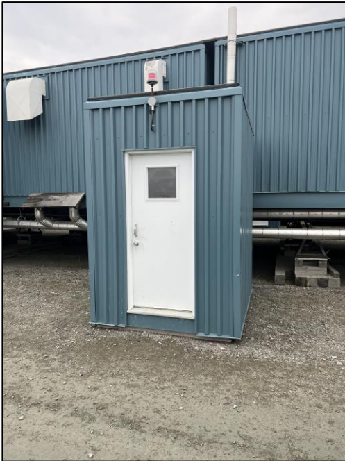
Photos 2: Spill location post remediation.
