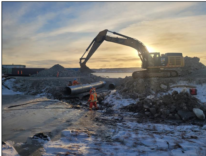
Figure 2: Dewatering of excavated area upstream of new Itivia culverts.
