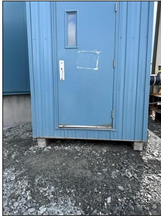
Photo 2: Sewage spill post remediation.
