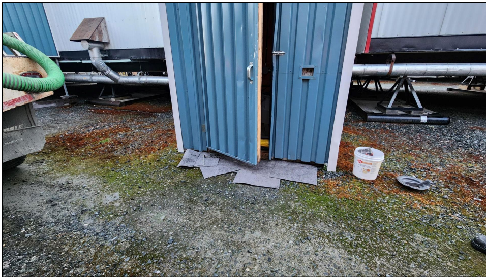
Photo 2: Sewage spill remediation.
