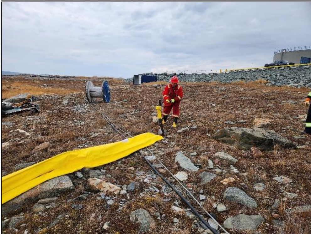
Photos 2 & 3: Assembly of marine booms
