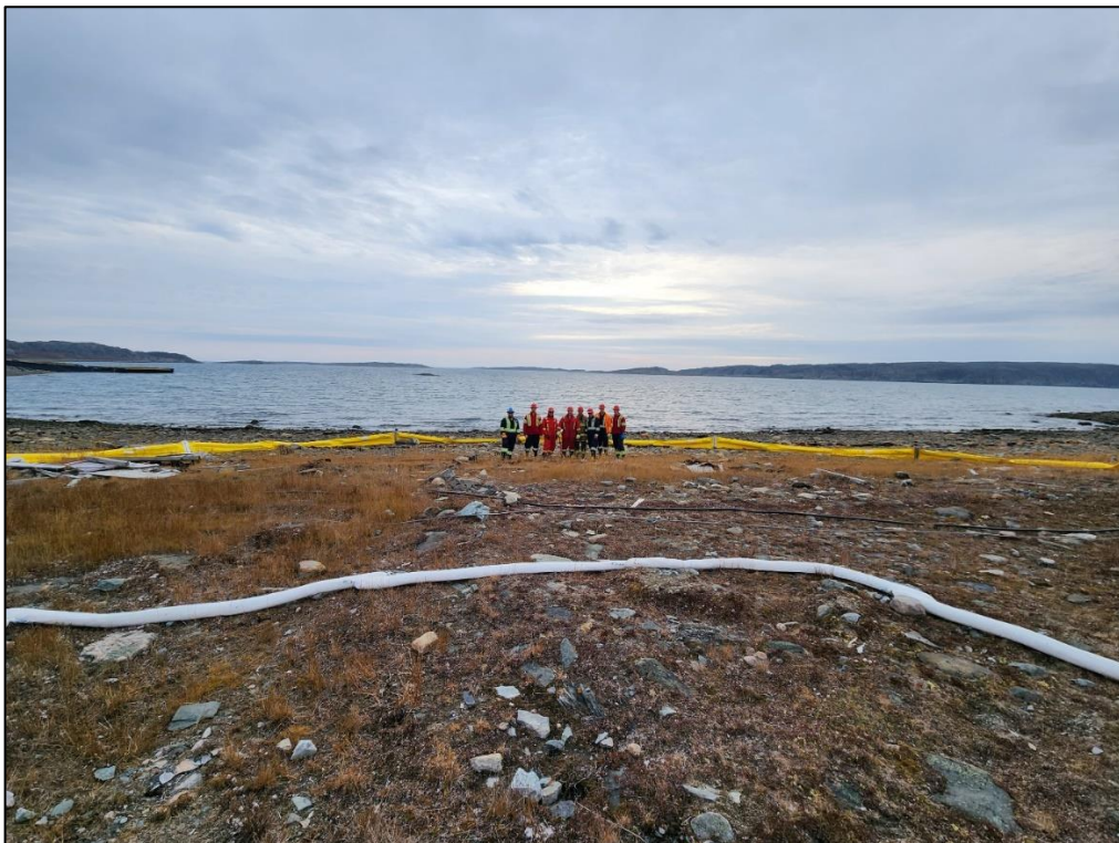
Photo 5: Final layout of the spill containment booms
