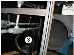
Secondary Chamber Blower Manual Slide Gate Open
