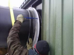
3. Once breech flanges are aligned and together bolt flanges together using the numerical order described in the pattern below using hardware provided.
