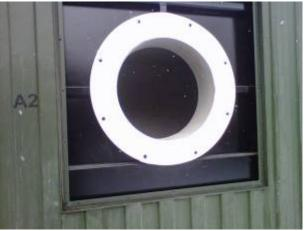
**Correctly Installed Gasket**
