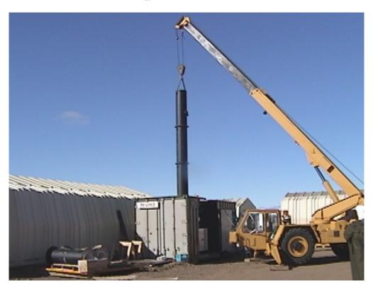
This is a Sample Photo only of Erection of the Stack Sections
