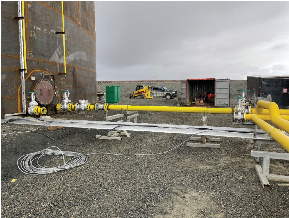
Tank #8 piping installation
