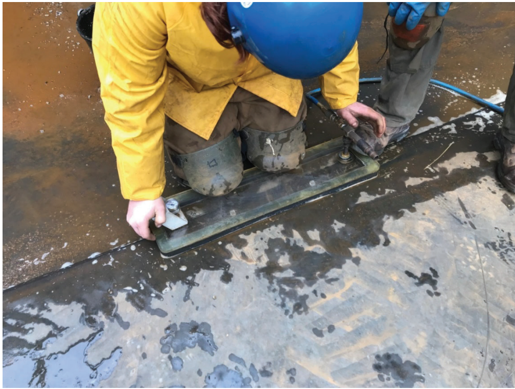
Weld testing with vacuum
