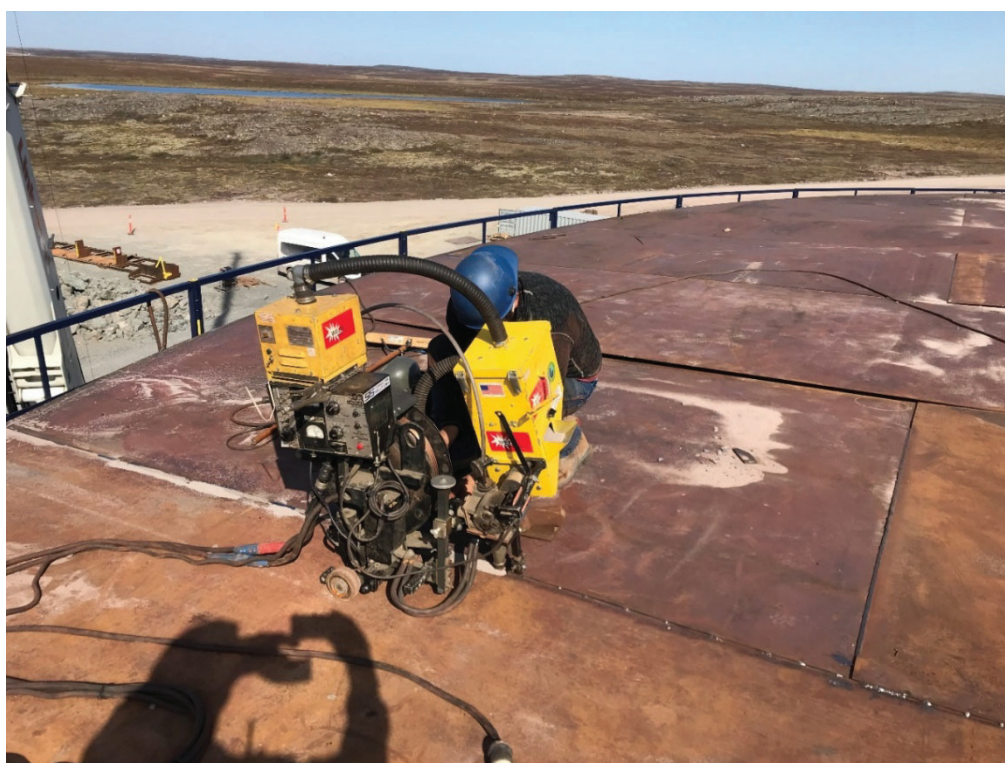
Tank roof plate welding
