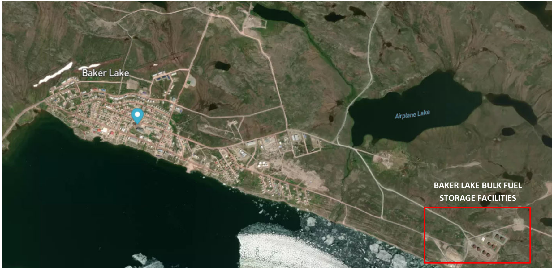
Figure 1-1: General Location of Baker Lake Bulk Fuel Storage Facilities
