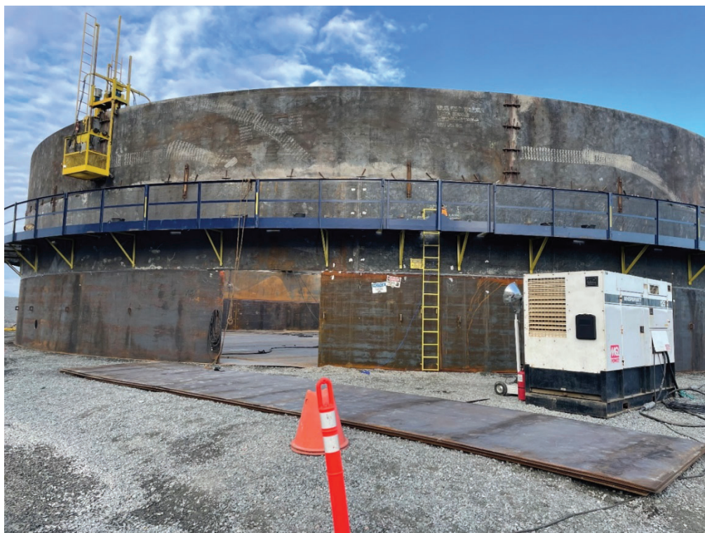
Tank wall third ring installation
