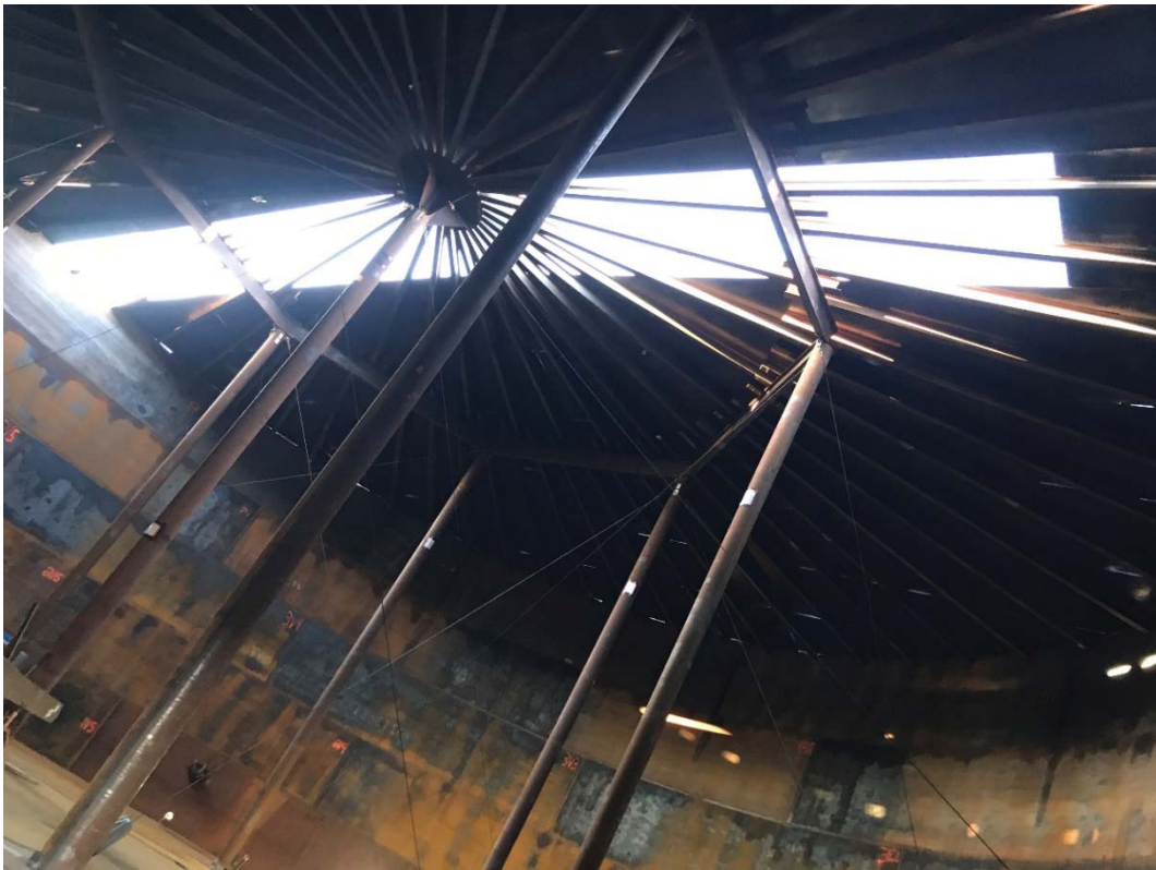
Tank roof structure
