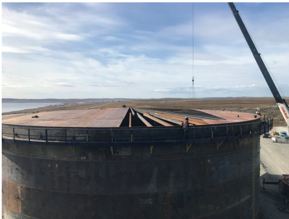
Tank roof structure
