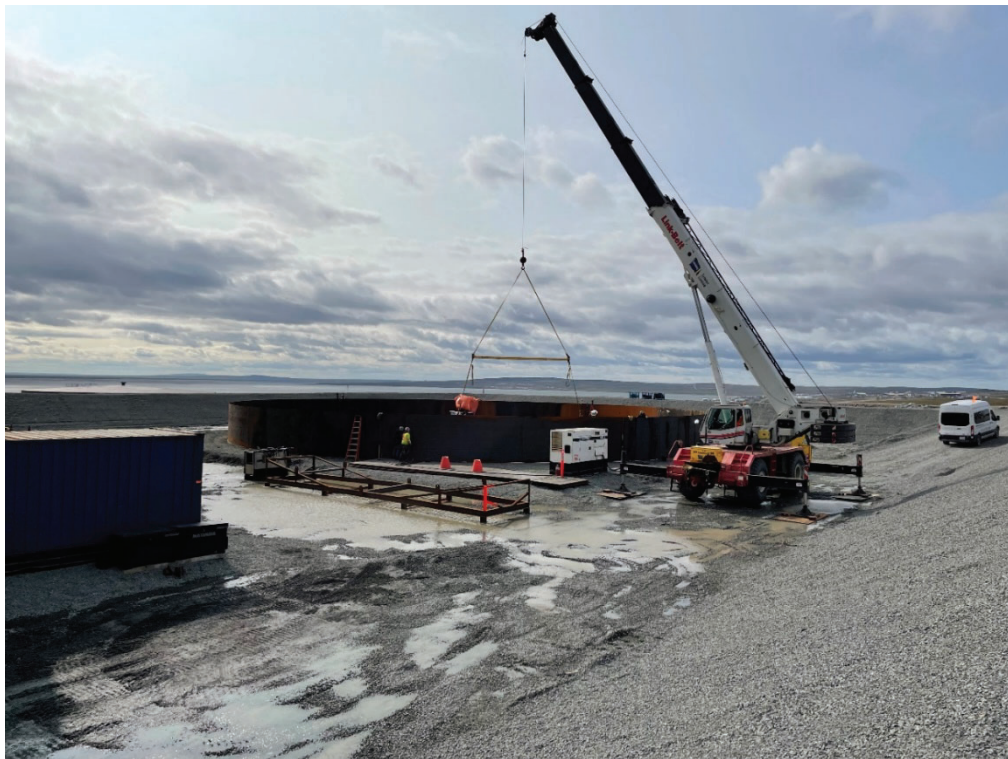
Tank wall welding
