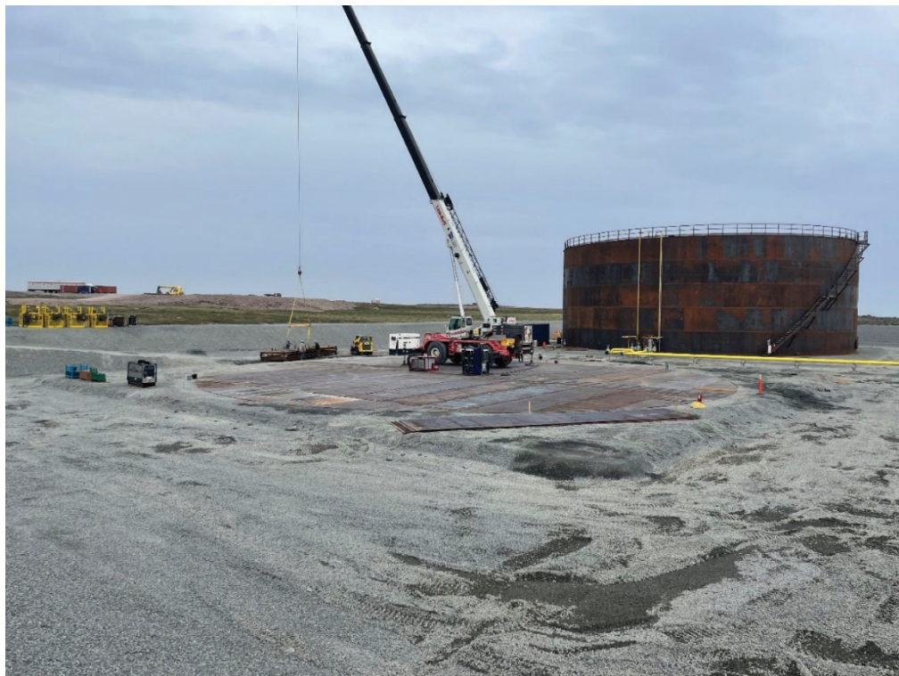
Tank floor construction
