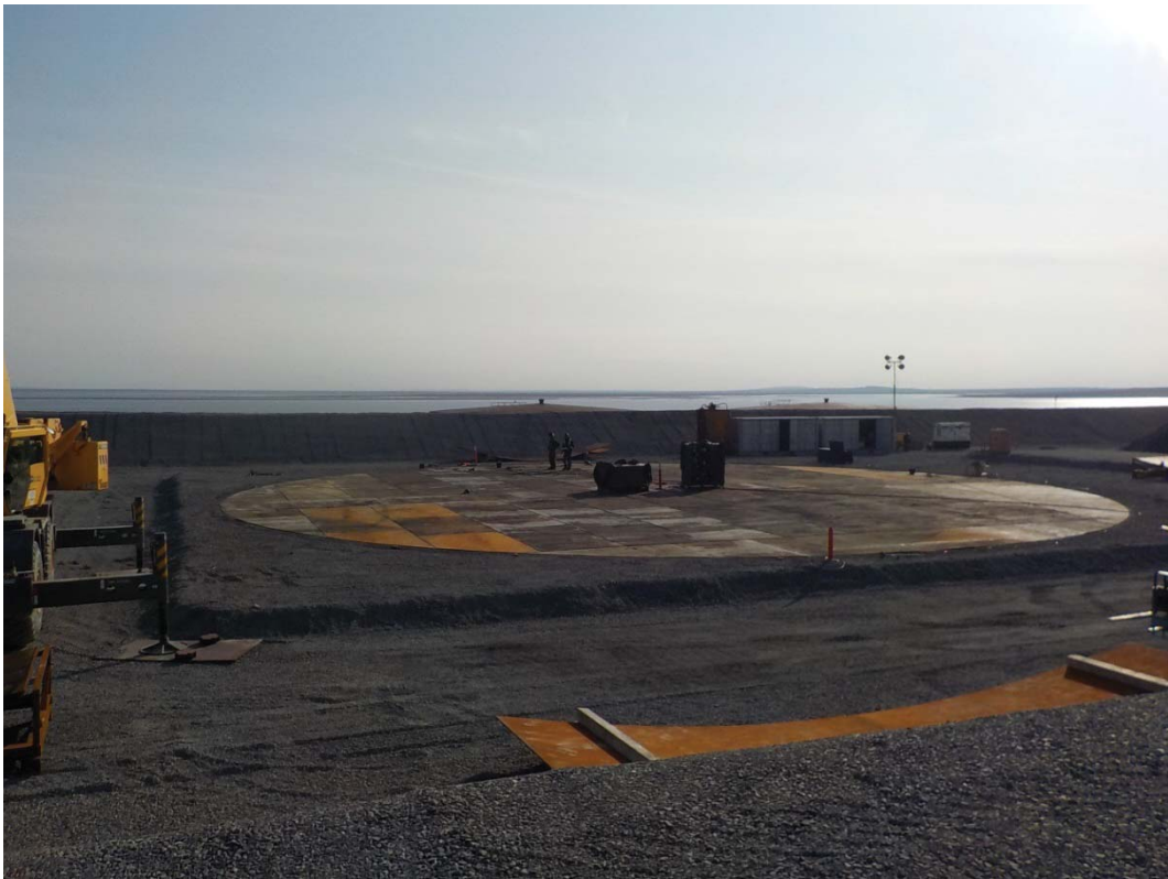
Tank floor construction
