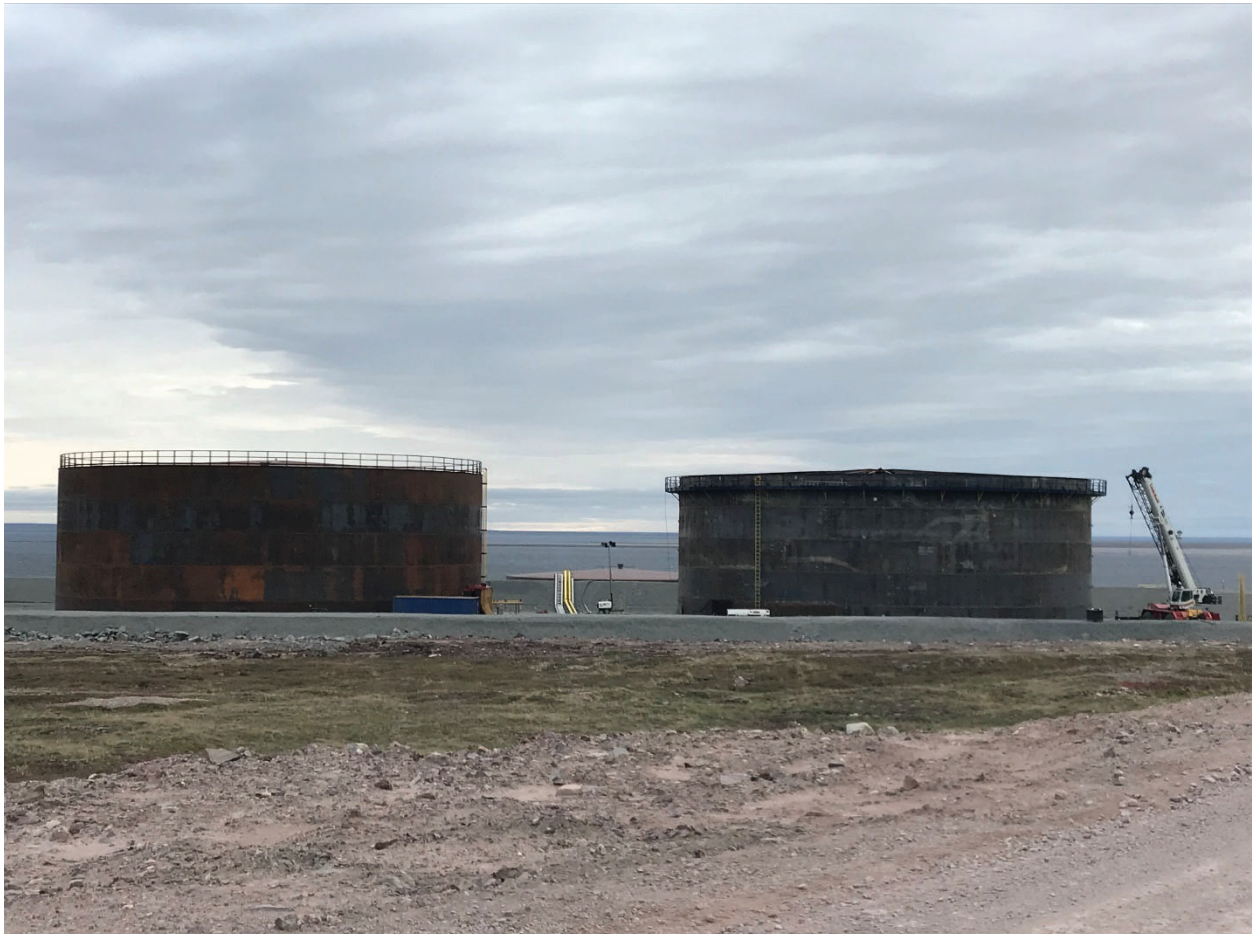
Figure 1 – Baker Lake Fuel Farm Site Overview (tank #7 and #8)
