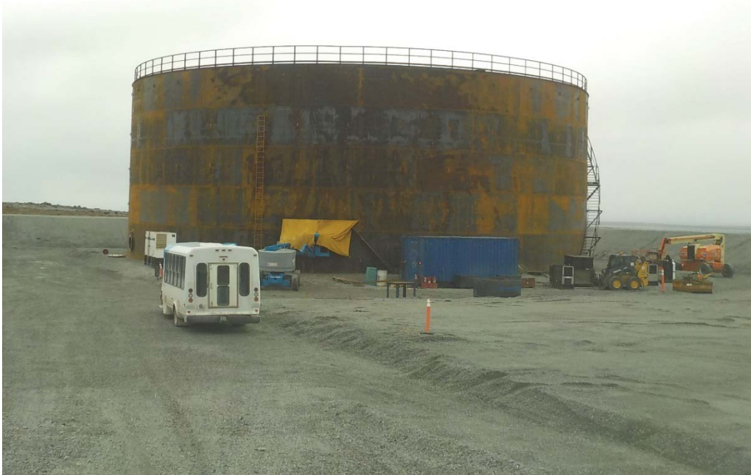
Tank general view
