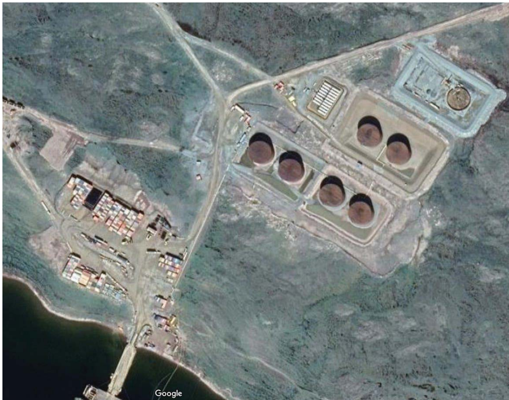
Figure 1 – Baker Lake Fuel Farm Site Overview (tank 7 in construction)
