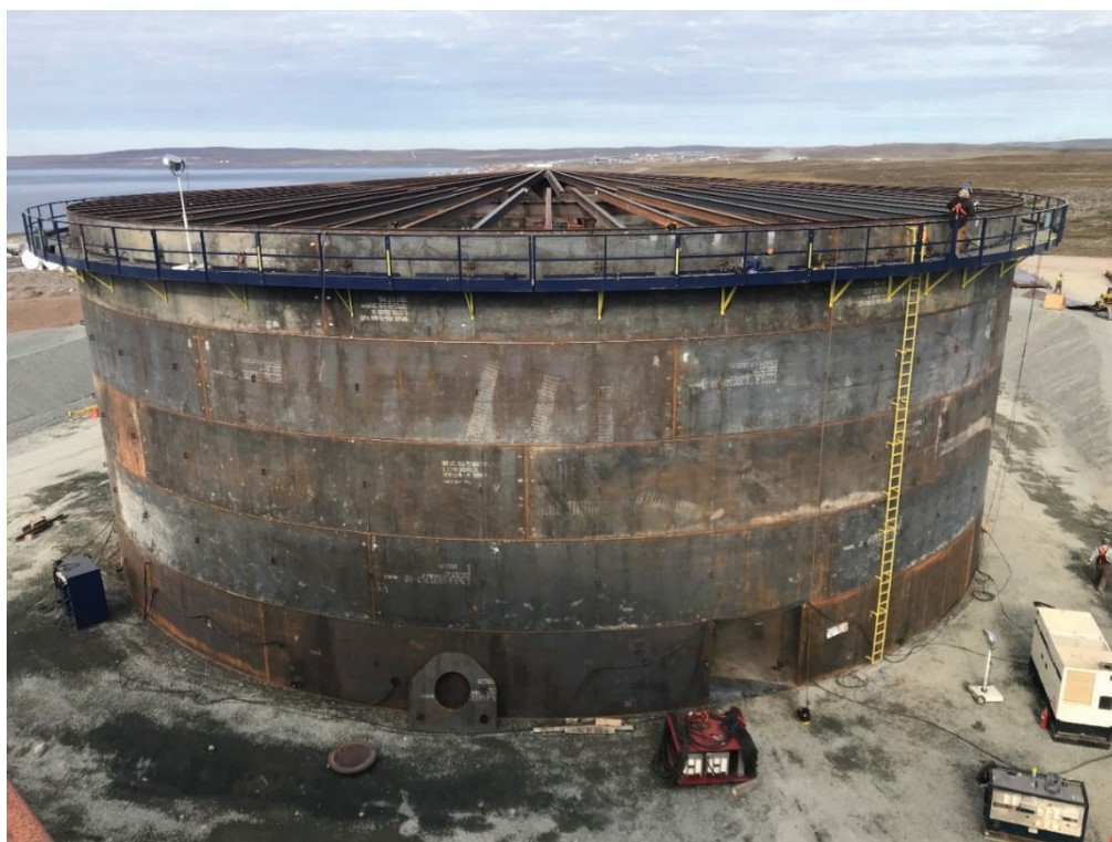
Tank general view
