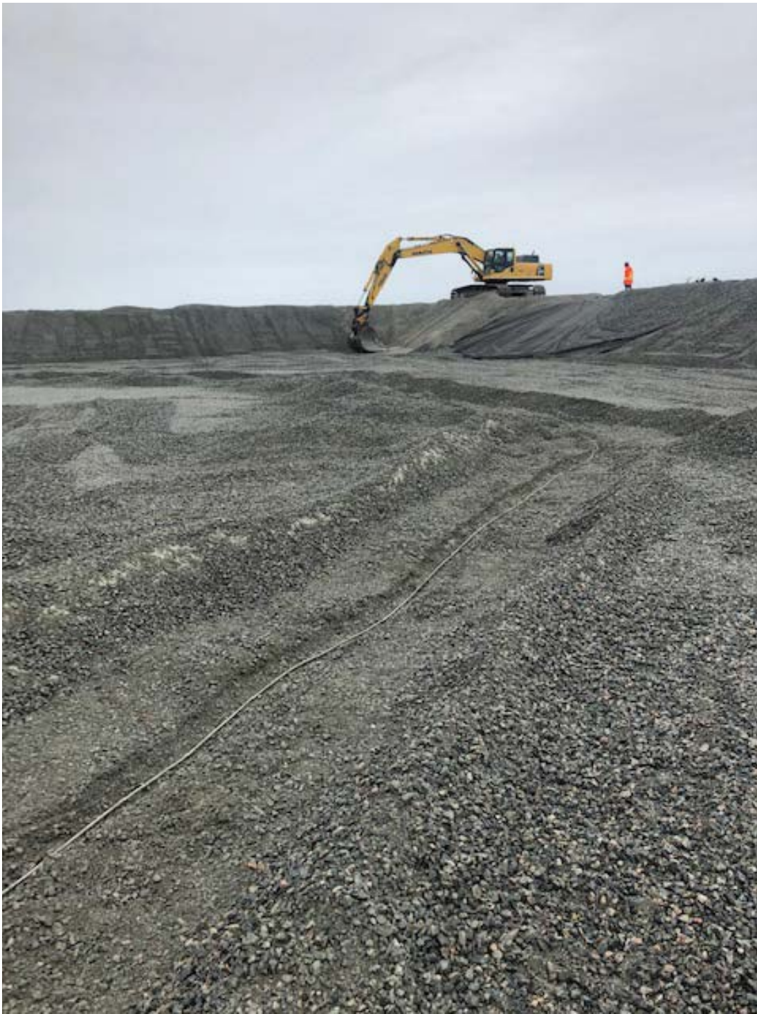
Pad and Berm construction
