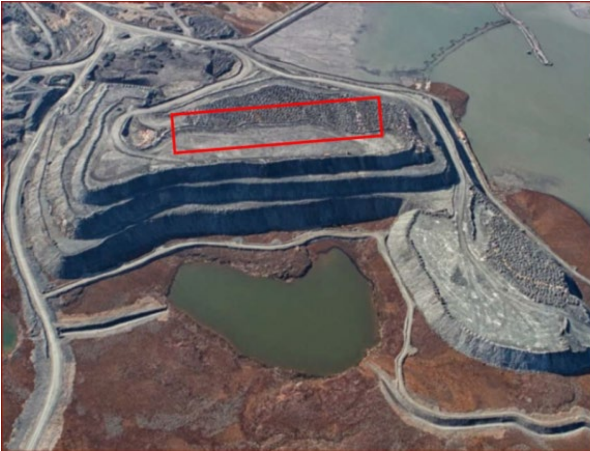
Figure 3: Approximate location of the Landfill #2 on top of Portage RSF
