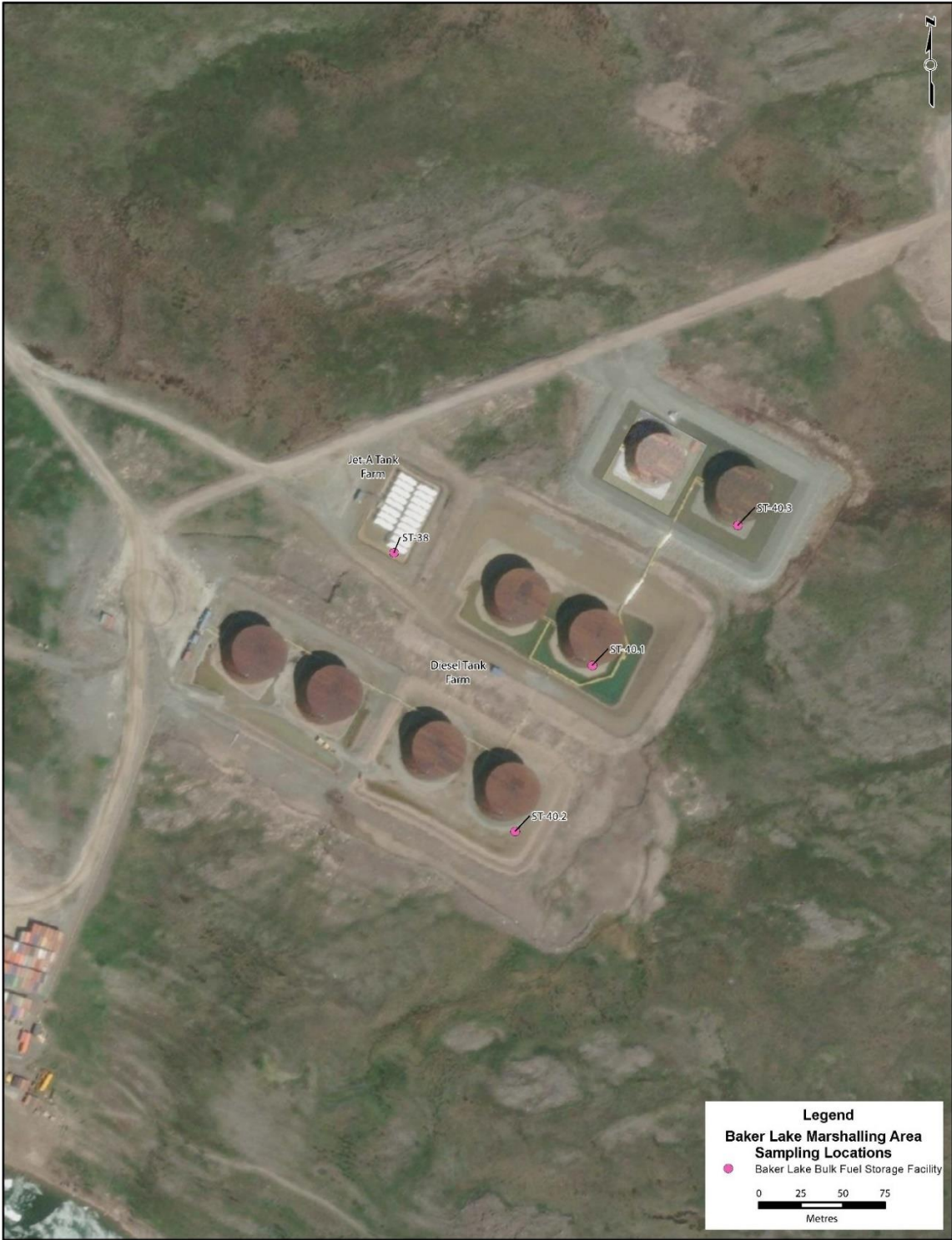
Figure 3 Baker Lake Marshalling Area: Diesel and Jet-A Tank
