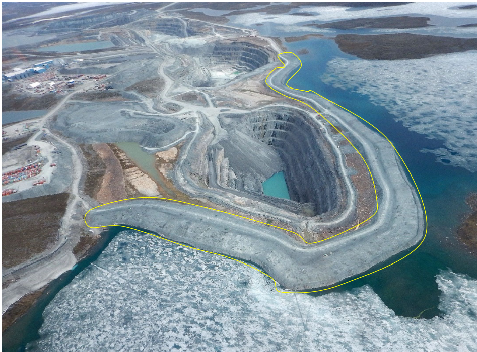
Figure 3-3 : Aerial View of Bay-Goose Dike
