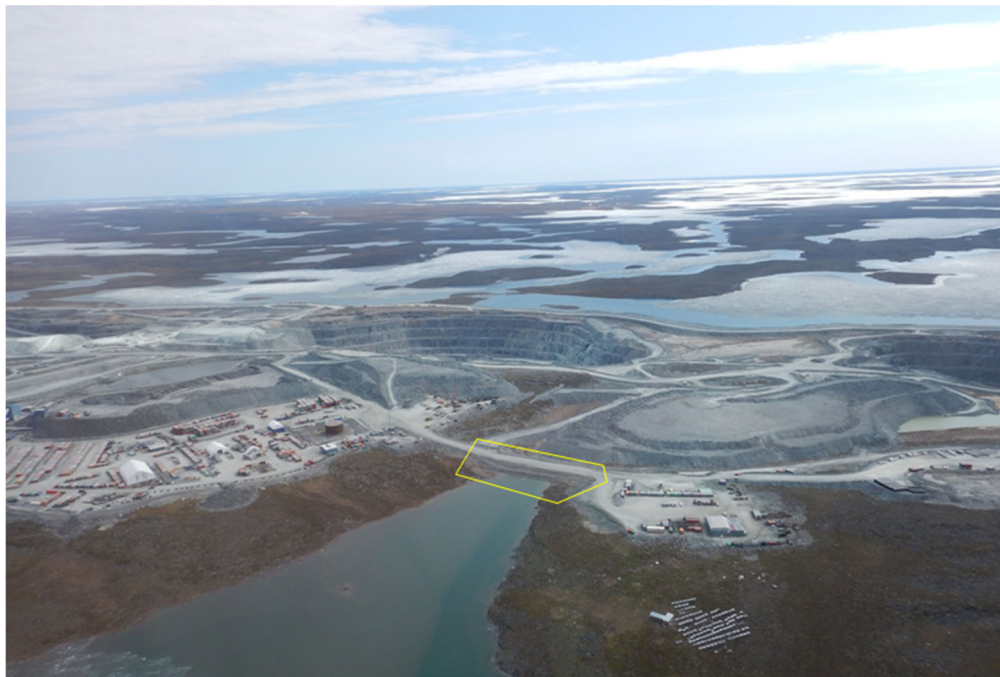
Figure 3-5 : Aerial View of South Camp Dike
