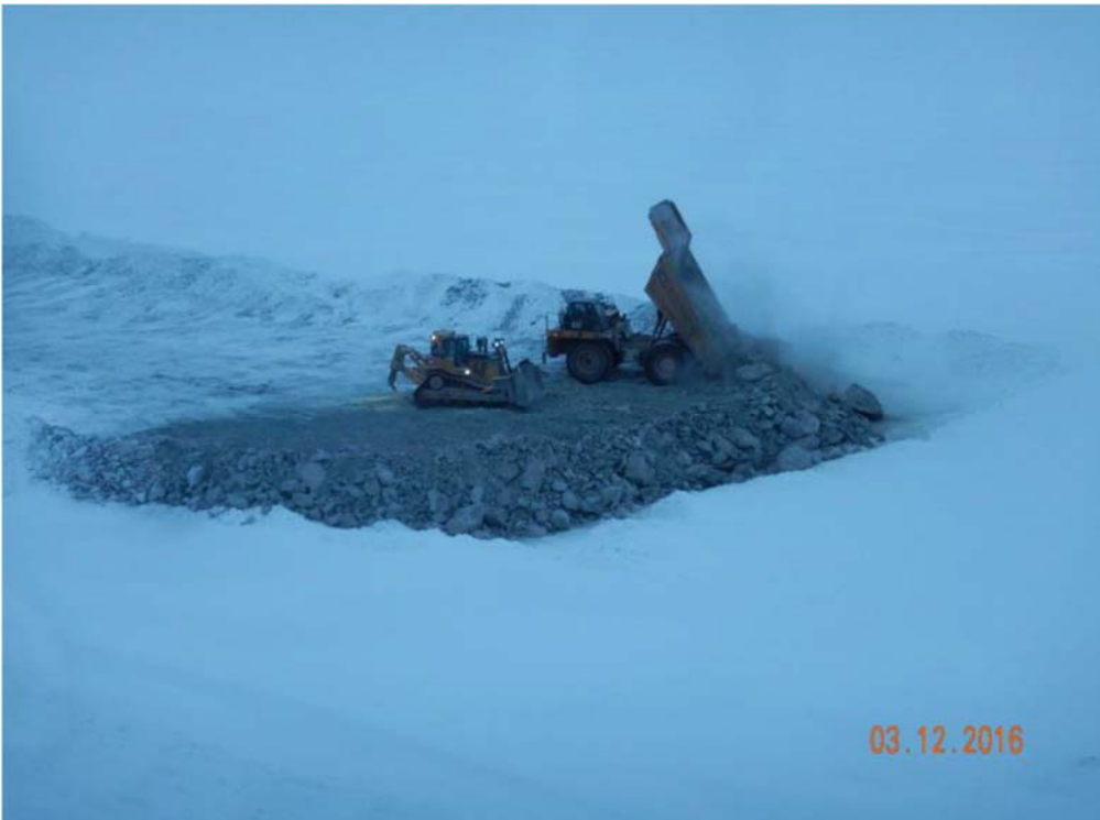
Photo 9: TSF North Cell, NPAG Cover construction, winter 2016
