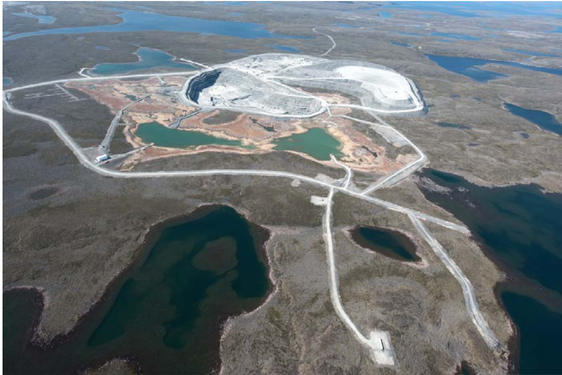
Photo 6 : Vault area, summer 2016
