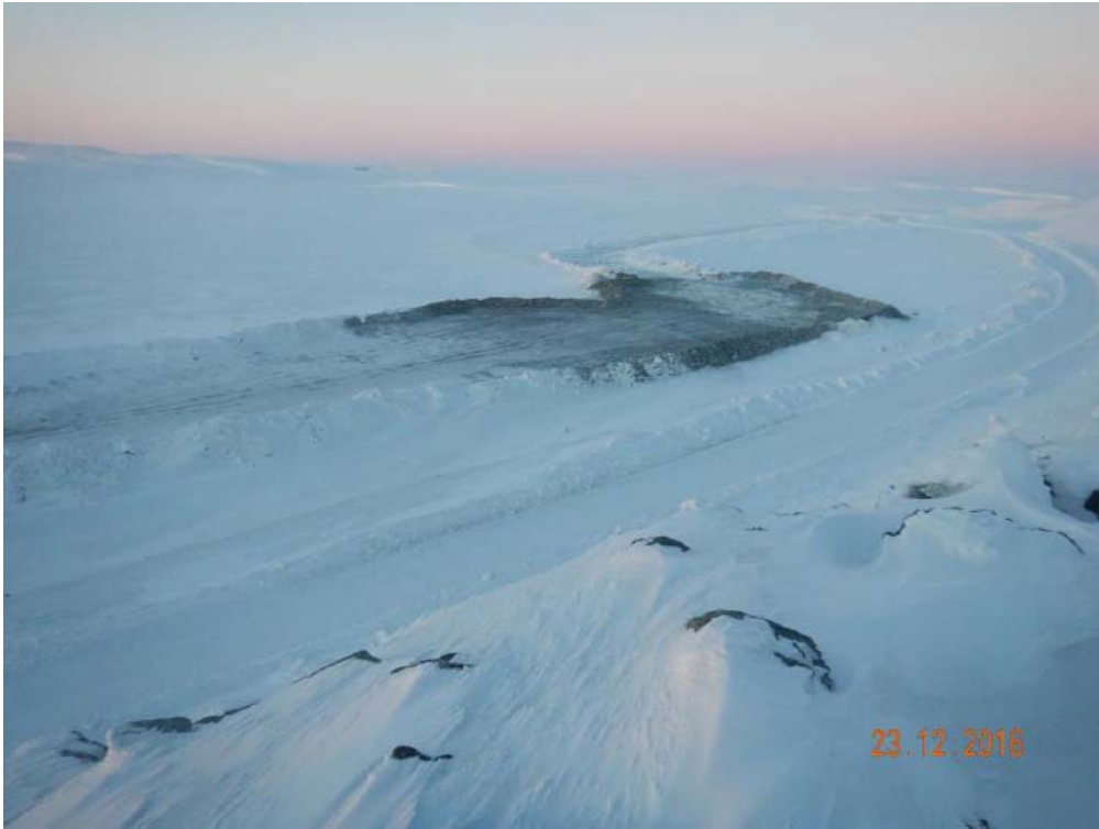
Photo 8: TSF North Cell, NPAG Cover construction, winter 2016
