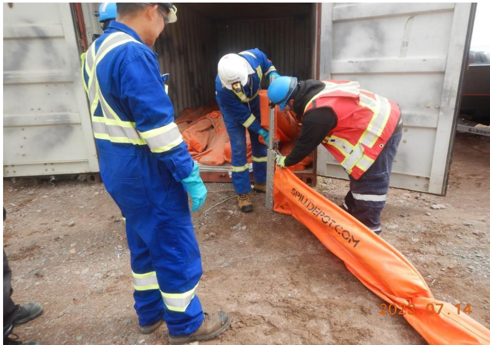
Assembly of marine barriers
