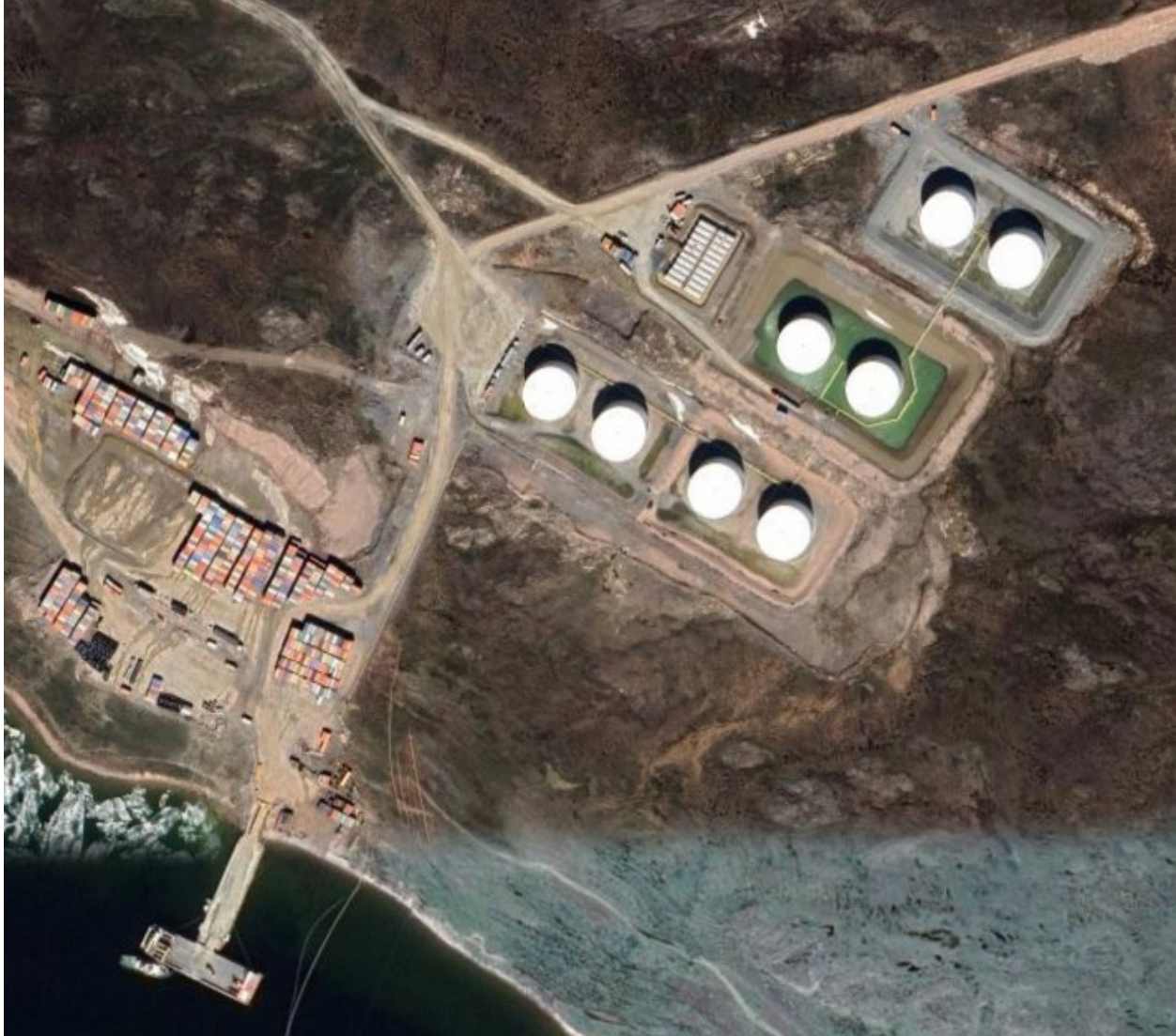
Figure 2-1 – Agnico Eagle’s Baker Lake Oil Handling Facility – Ship to Shore Transfer Area
