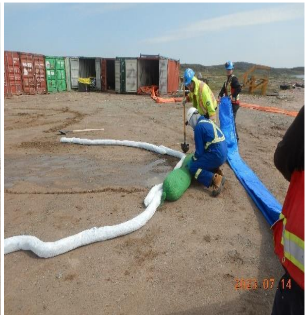
Utilizing shovel to construct a berm, collecting, and slowing the flow of diesel.
