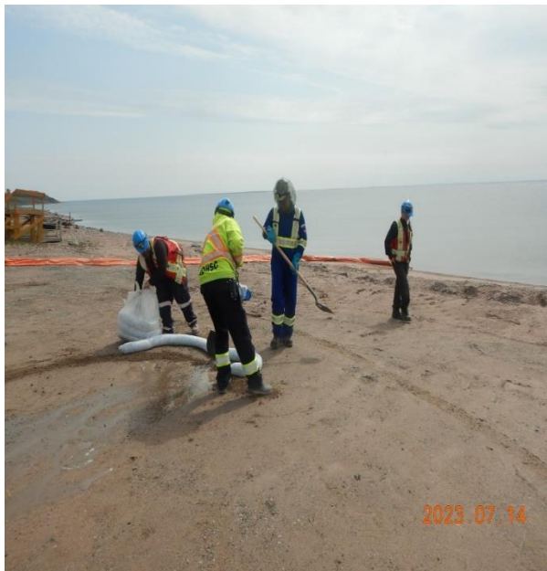
Utilizing shovel to construct a berm, collecting, and slowing the flow of diesel.
