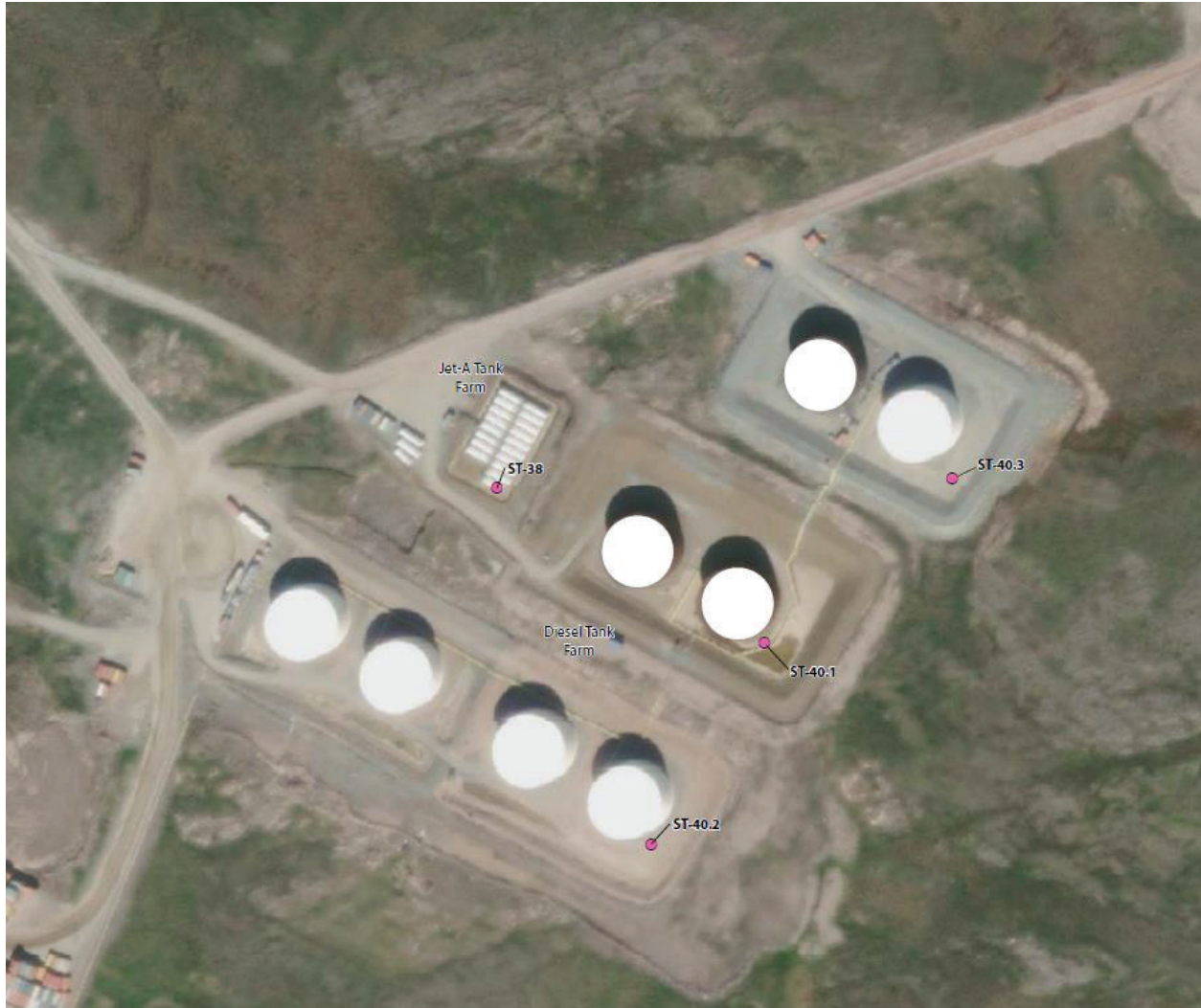
Figure 1: Agnico Eagle's Baker Lake Oil Handling Facility
