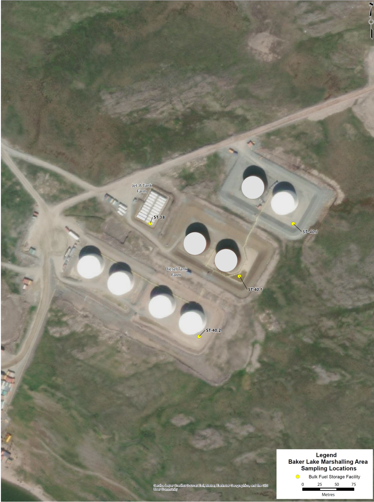
Figure 3: Baker Lake Diesel and Jet-A Fuel Tank Farm
