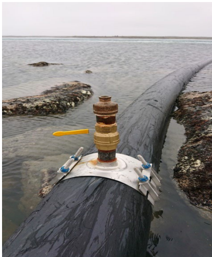
Photo 4. ST-MDMER-7 FDP before dismantling
