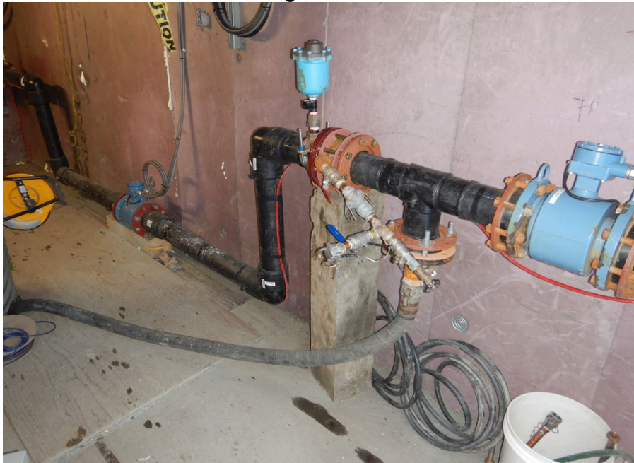
Photo 1. FDP East Dike Discharge Meadowbank
