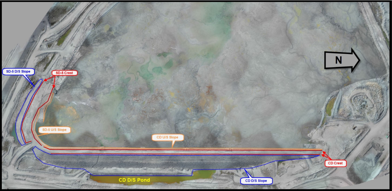
Figure 3-13: Aerial View of Central Dike and SD5
