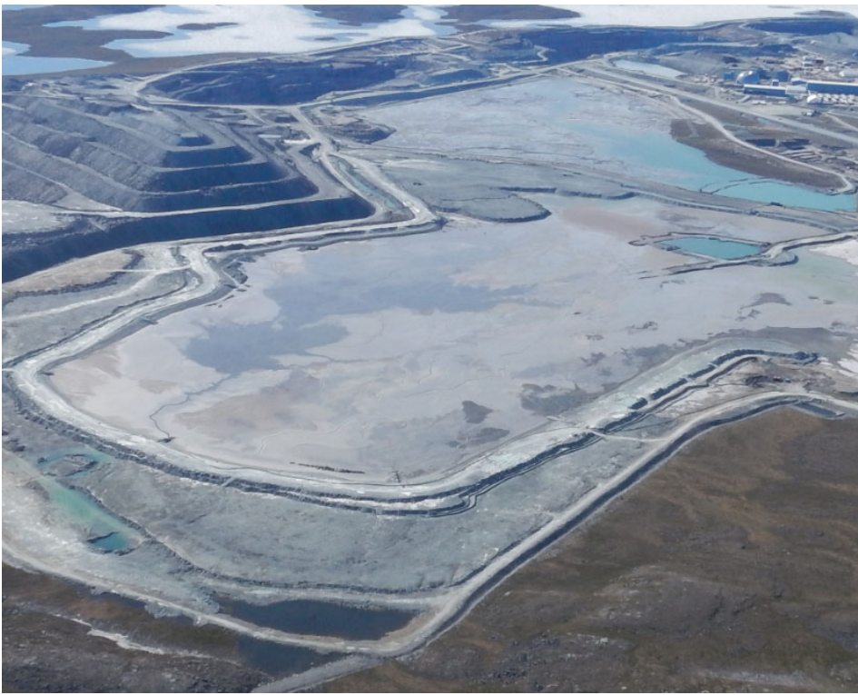
Figure 3-8: Aerial View of the North Cell Internal Structure
