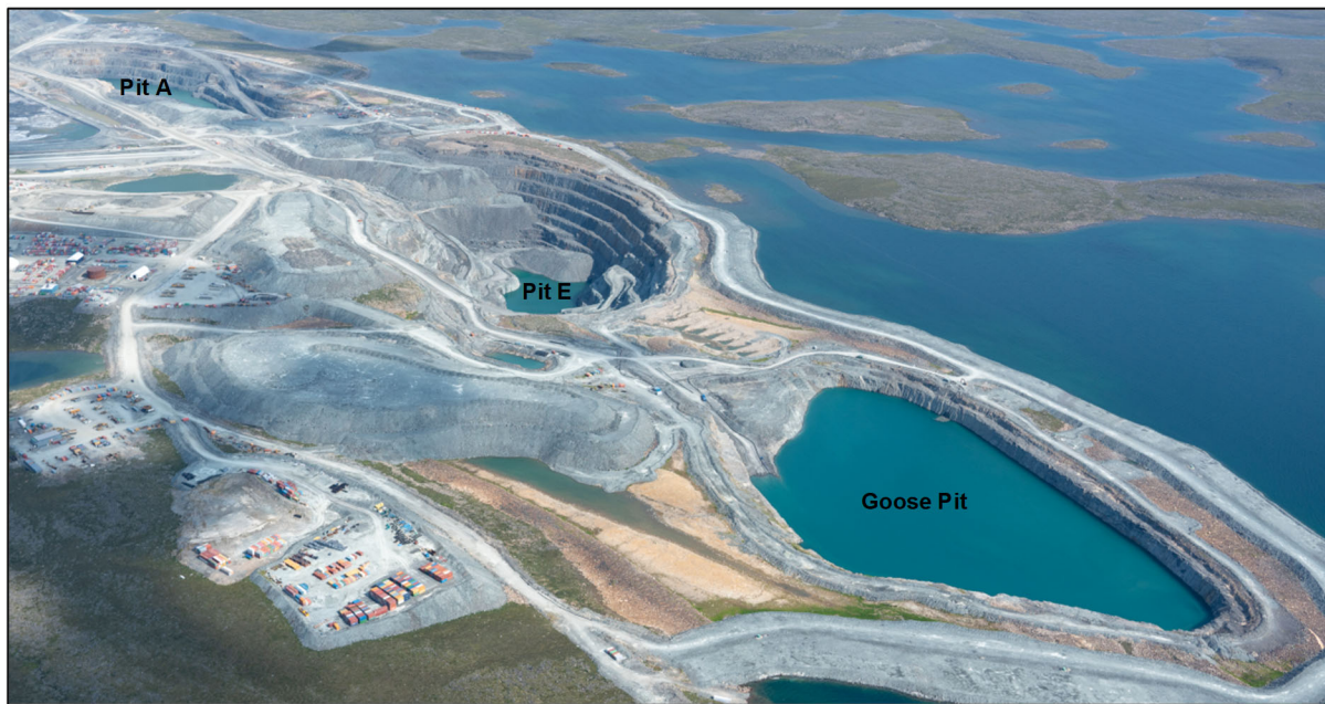
Figure 3-18: In-Pit Area for Tailings Management (Summer 2020)
