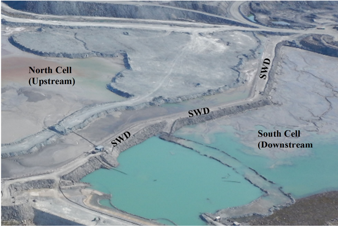
Figure 3-15: Aerial View of Stormwater Dike (2019)
