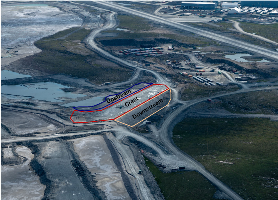
Figure 3-10: Aerial View of Saddle Dam 3
