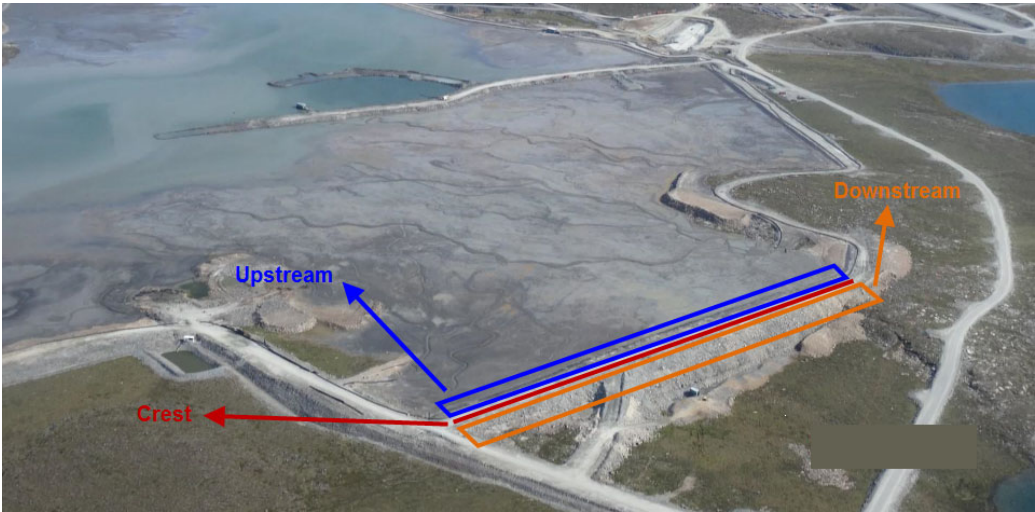
Figure 3-2: Aerial View of Saddle Dam 1
