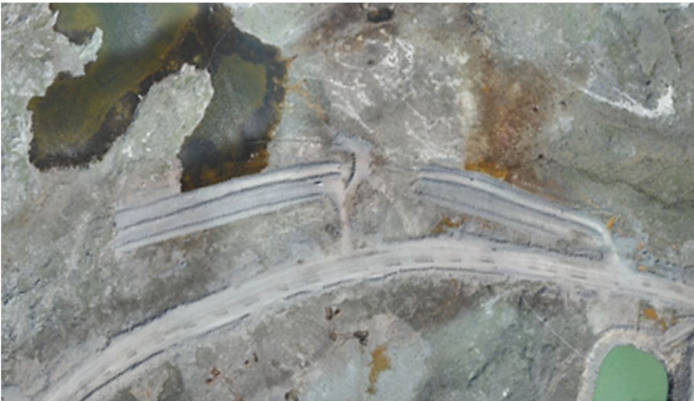
Figure 3-8 : Aerial View of North-East Dike (before dismantling)
