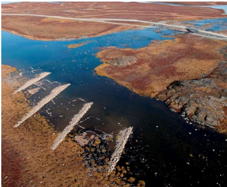
Figure 17 Arctic Grayling spawning pads constructed at Meadowbank all weather road crossing R02.
