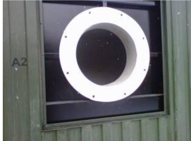
**Correctly Installed Gasket**
