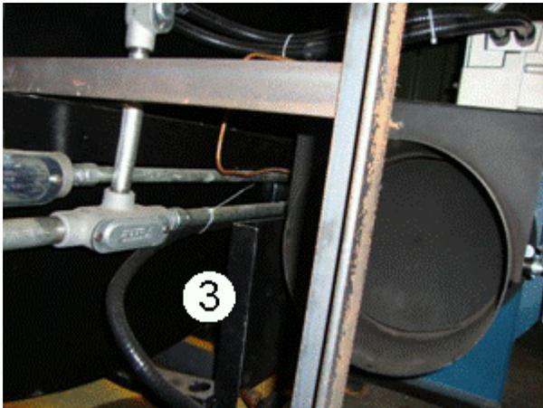
3. **Secondary Chamber Blower** Manual Slide Gate Open
