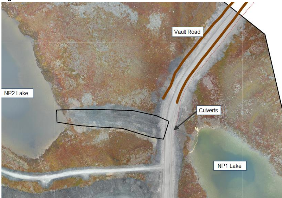
Figure 2-7: View of the diversion ditches at the Vault road area
