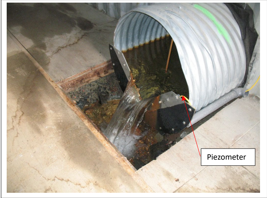
Photo #9 Main weir at Whale Tail Dike.
