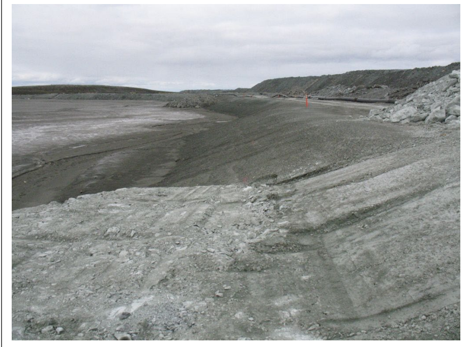
Photo #23 NCIS protective berm, looking north.
