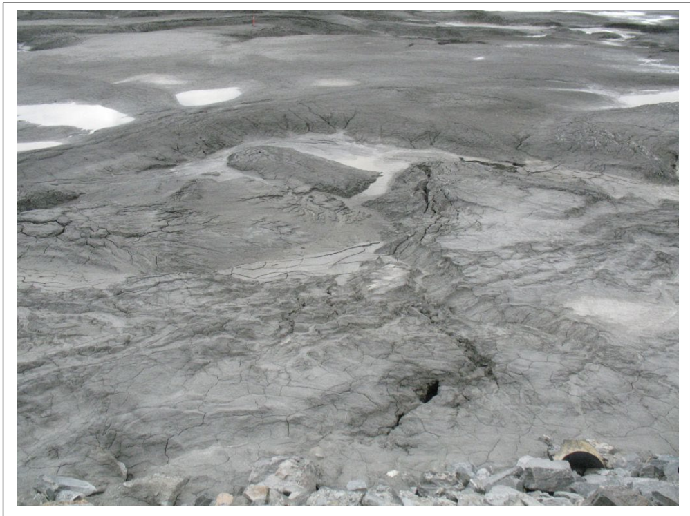
Photo #18 South Cell consolidation settlement and inflow areas that contribute to groundwater recharge.
