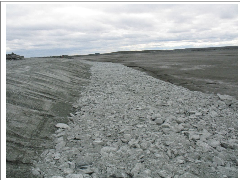
Photo #22 North Cell Internal Structure (NCIS). Protective toe berm, looking south.
