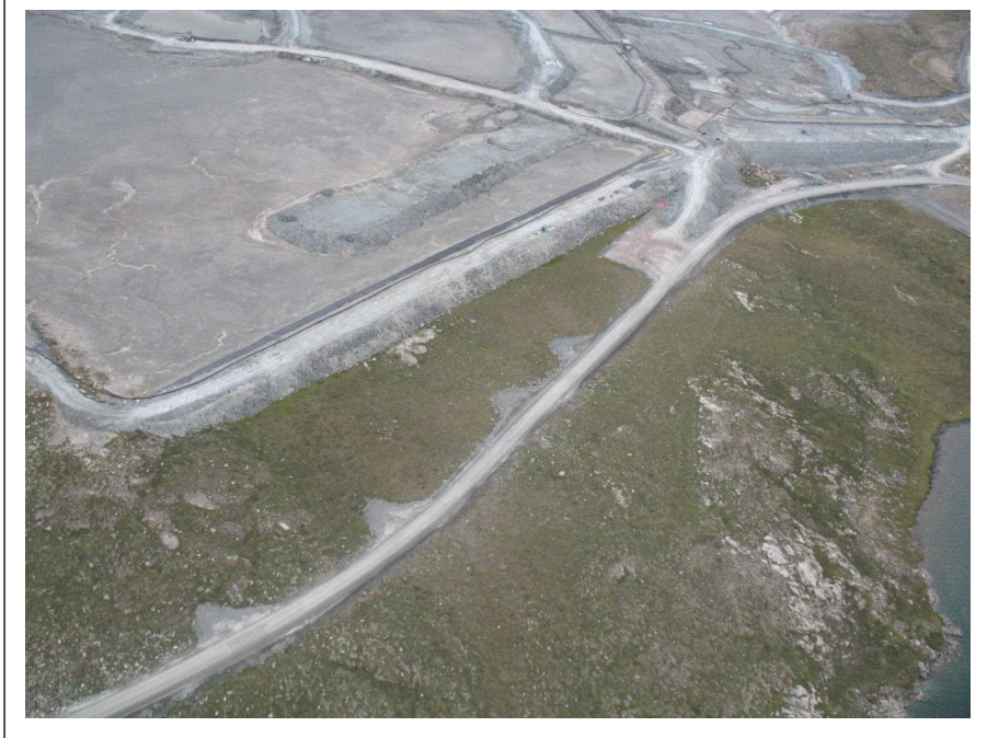
Photo #15 Saddle Dams SD2 and SD3.
