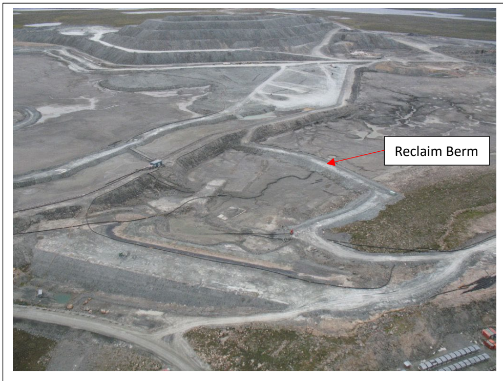
Photo #16 SD3, Stormwater Dike, and South Cell Reclaim Berm.
