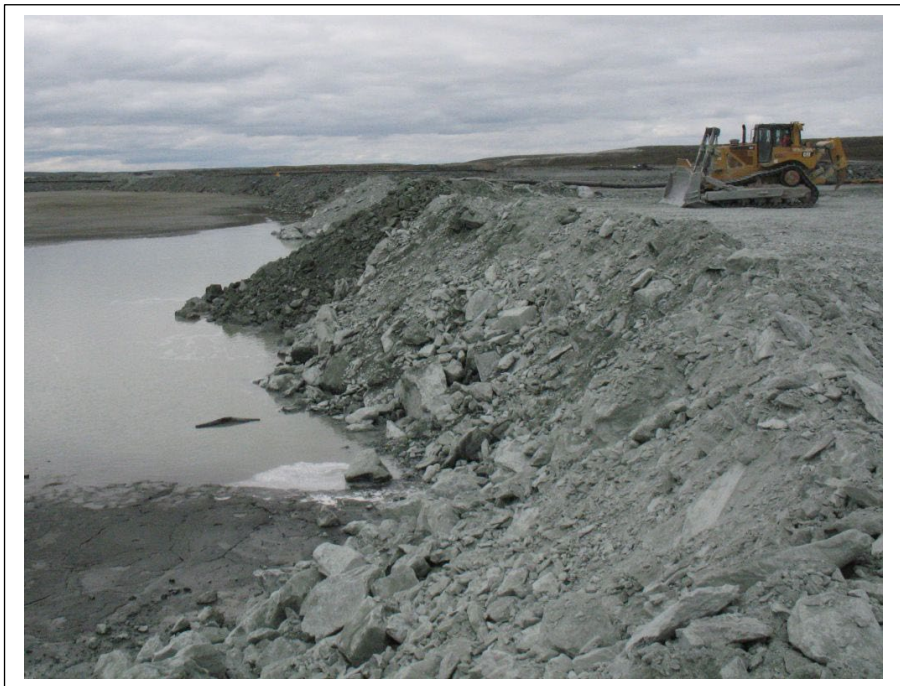
Photo #20 Progressive closure capping on North Cell of TSF.
