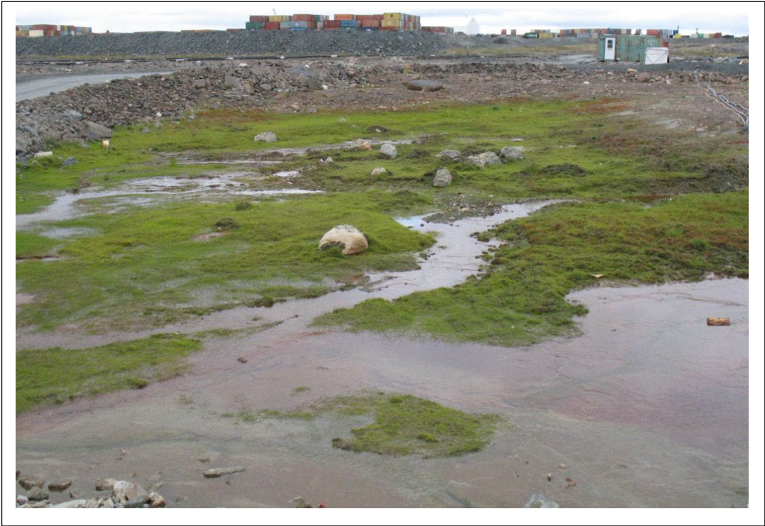
Photo #10 Whale Tail Dike area of seeps not accumulated at main weir.
