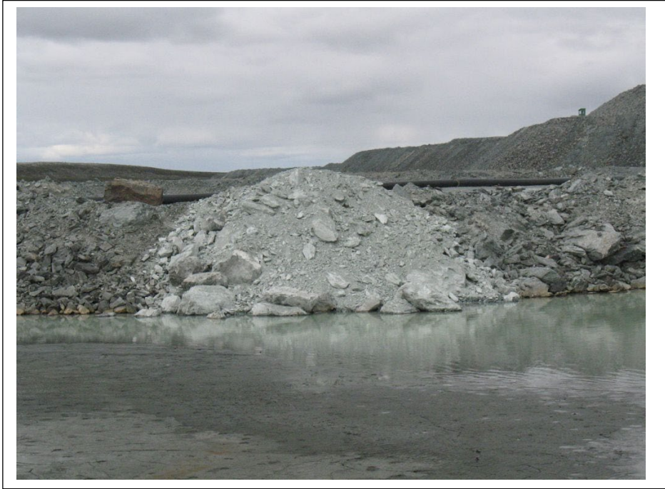
Photo #21 Segregation in dumped rockfill.
