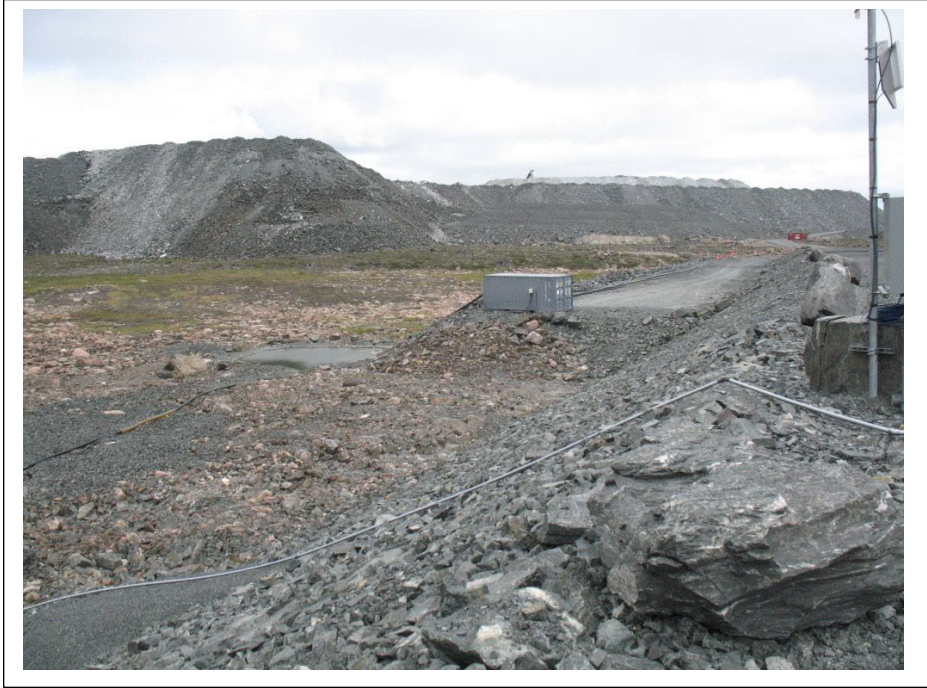
Photo #5 WRSF Dike. U/S area, little or no ponded water at time of visit.
