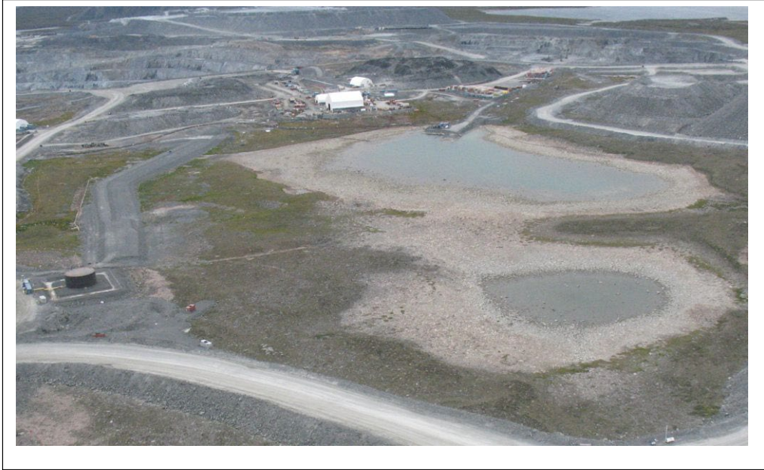
Photo #1 IVR Dike. Note low U/S pond level.
