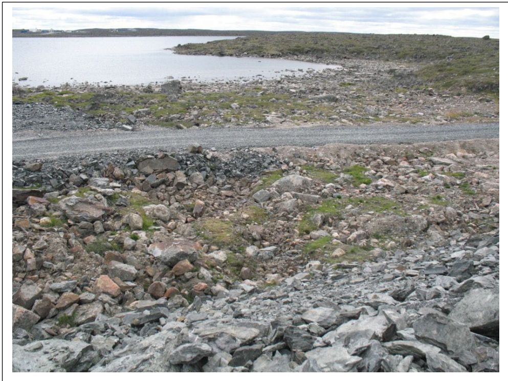
Photo #4 WRSF Dike. D/S area.
