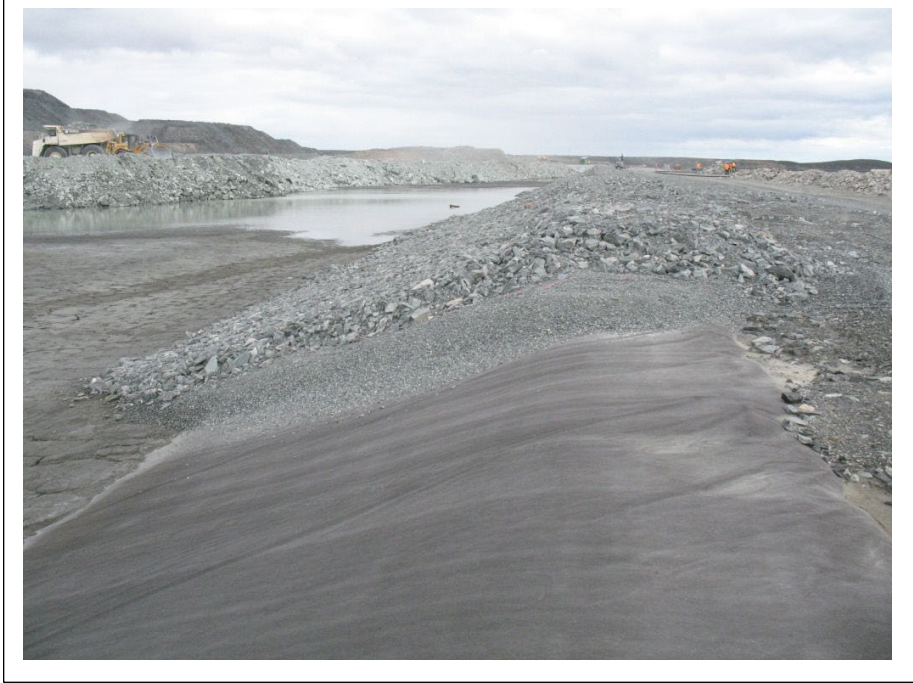
Photo #19 Fine and coarse filter protection of Stormwater Dike geomembrane.
