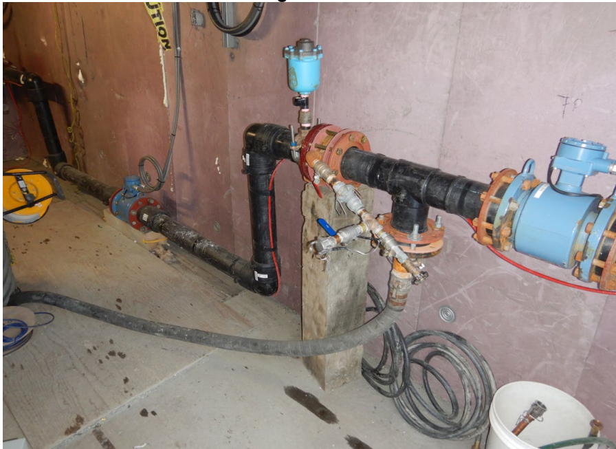
Photo 1. FDP East Dike Discharge Meadowbank
