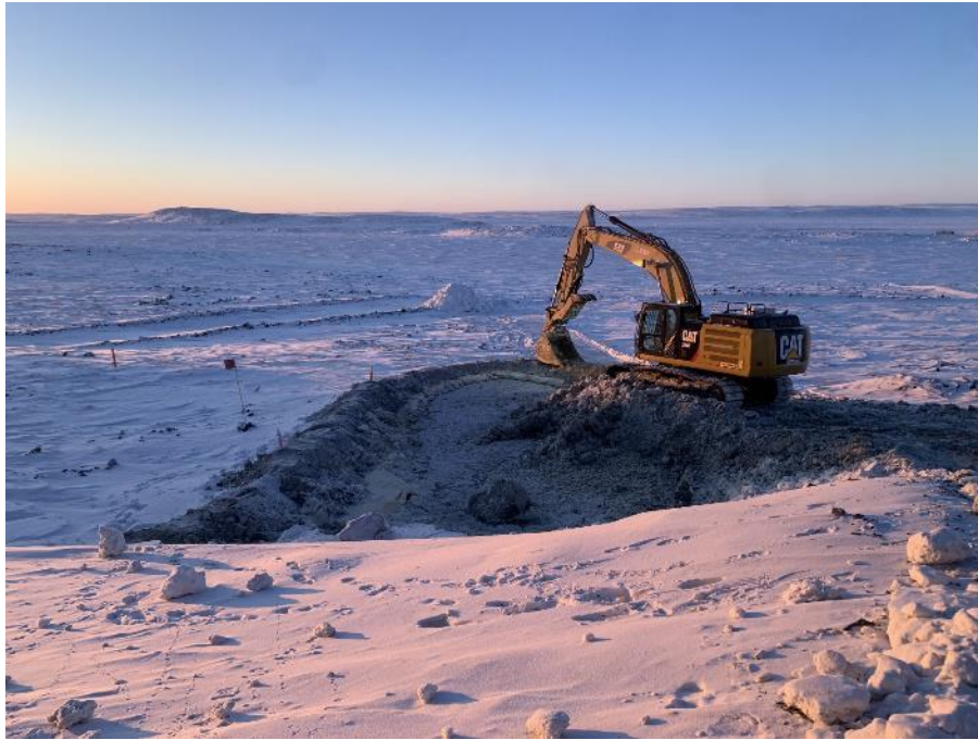
Figure 5. Continued berm repairs and excavation activities on Dec.19 th , 2023
