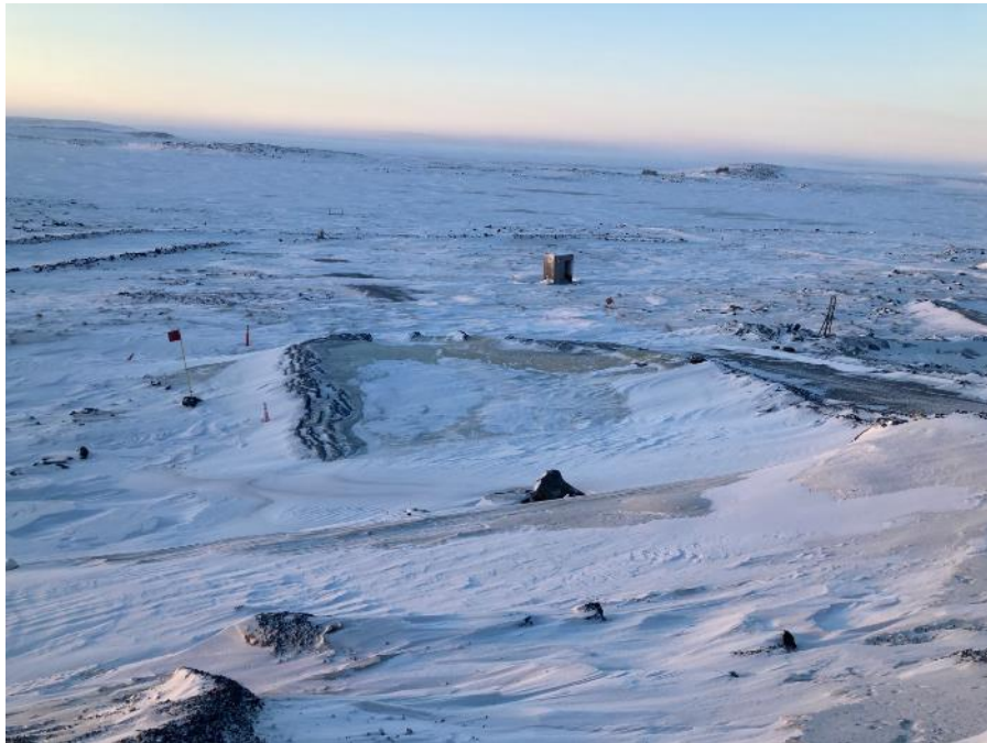
Figure 1. Water/Snow mixture contained upstream of the seepage collection trench.
