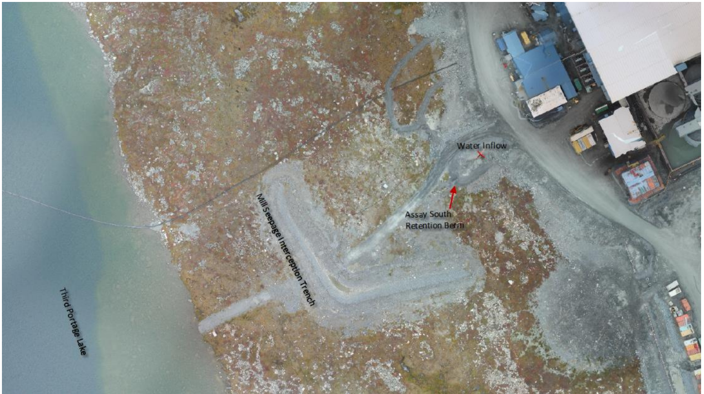
Figure 2. Site aerial image with water management infrastructure identified
