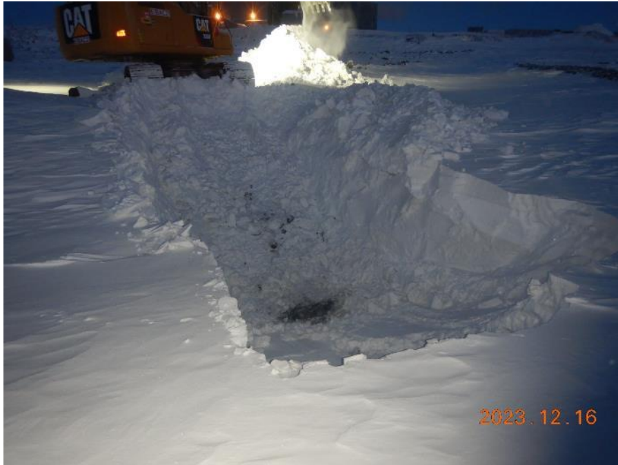
Figure 3. Snow removal from the Mill Seepage intercer trench Dec. 16 th , 2023
