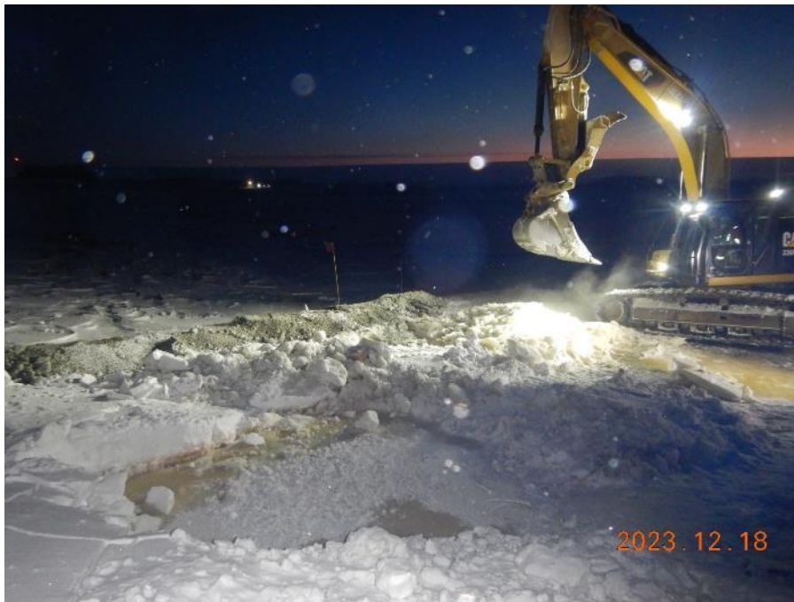
Figure 4. Containment berms being raised prior to excavation of snow/ice.
