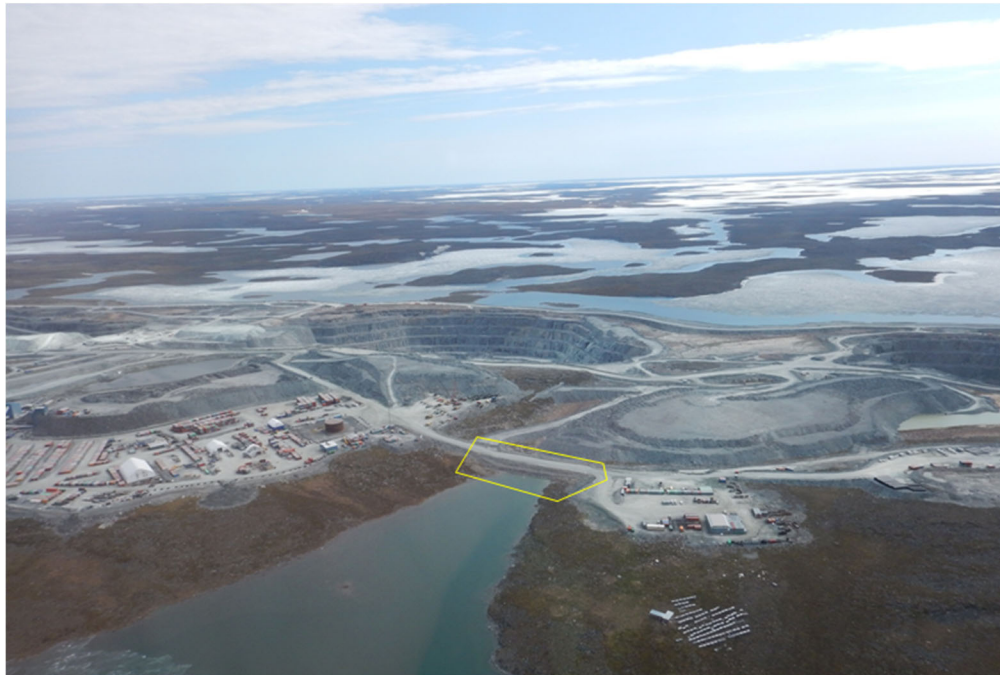
Figure 3-5 : Aerial View of South Camp Dike
