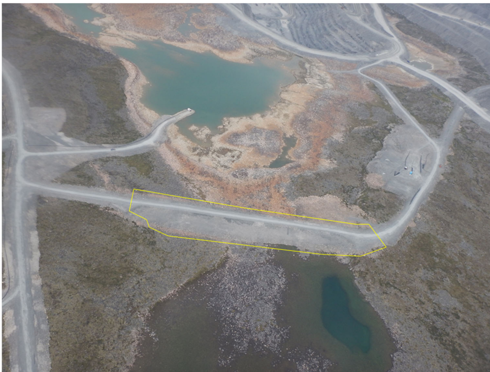
Figure 3-7 : Aerial View of Vault Dike
