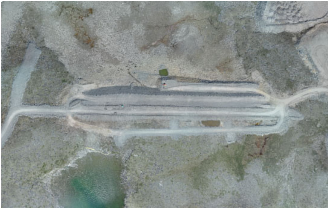
Figure 3-5 : Aerial View of WRSF Dike
