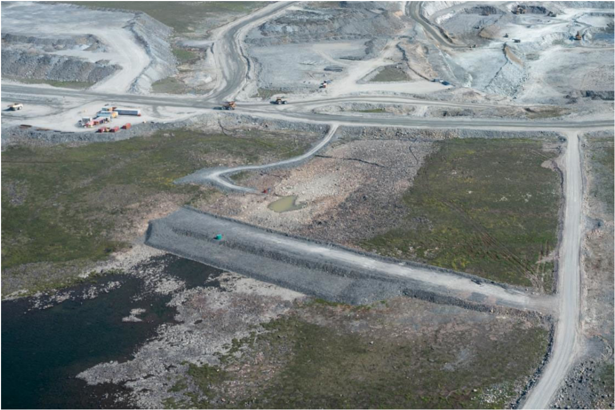
Figure 3-3 : Aerial View of Mammoth Dike
