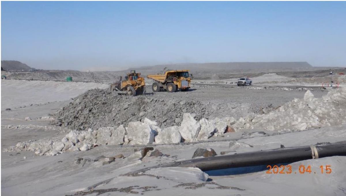
Figure 5. Final compaction of completed east abutment thermal capping (looking north).
