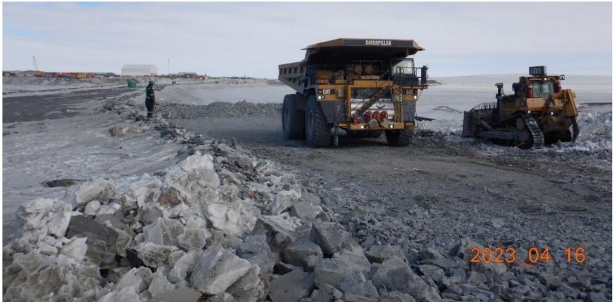
Figure 3. Compaction of completed lift # 2 at west abutment (April 16, 2023).
