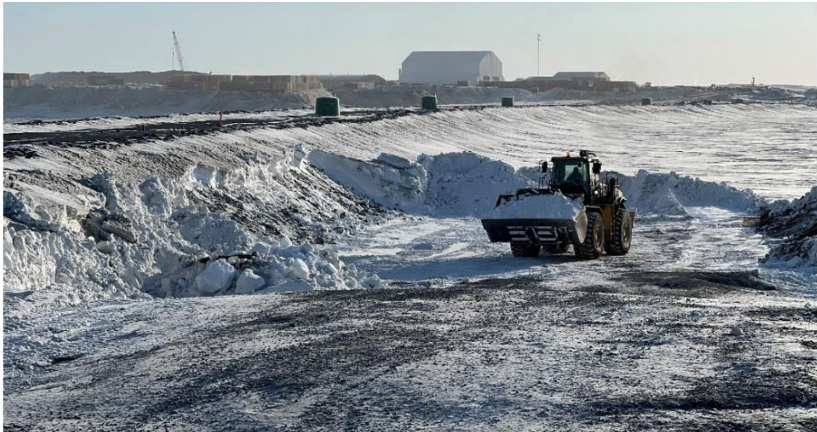
Figure 2. Snow removal on upstream slope at west abutment on April 13, 2023.
