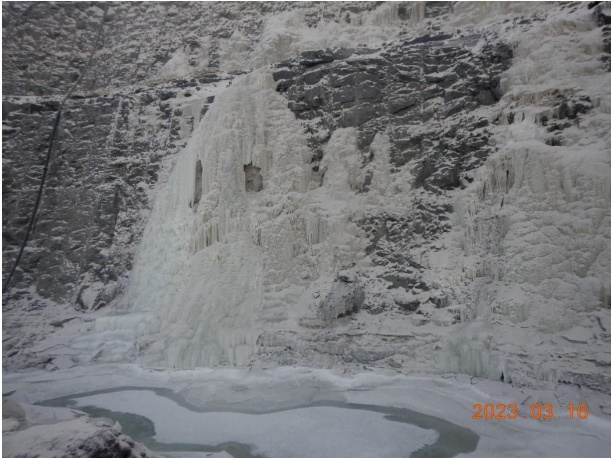
Photo 1: Seepage along Whale Tail Pit south wall, looking south toward pit 5081 mRL sump (ST-WT-4) on 16 March 2023.
