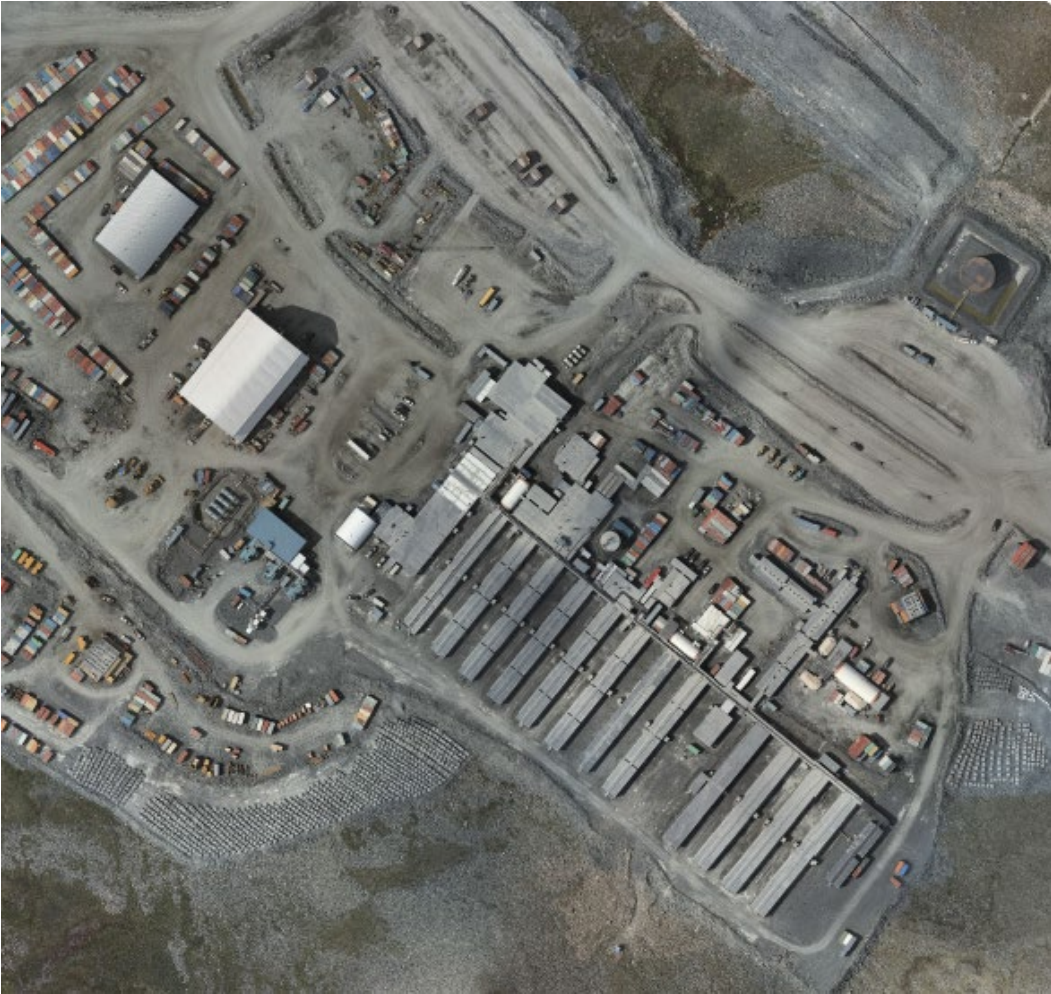
Figure 1-3 Aerial photo showing Whale Tail camp infrastructure (Summer 2023)
