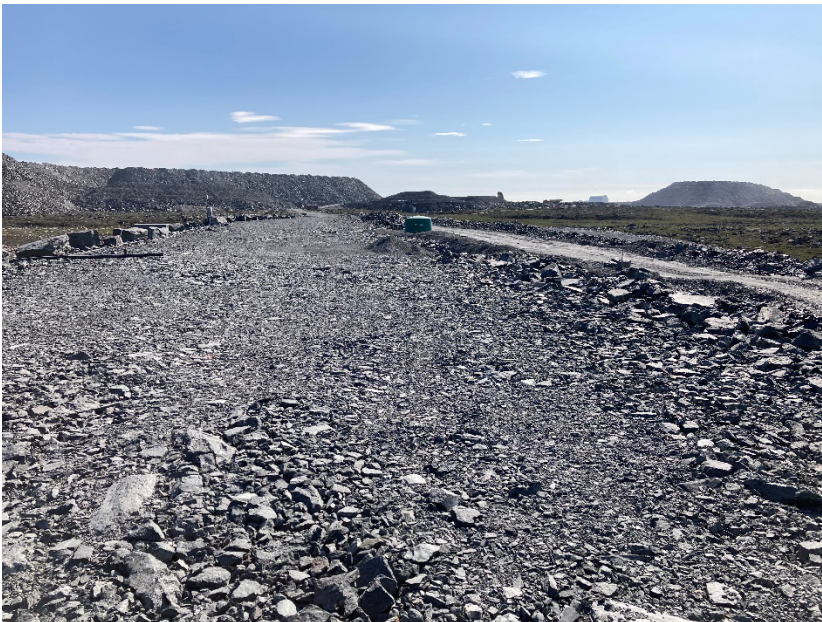
Photograph A7-8 WRSF Dike
