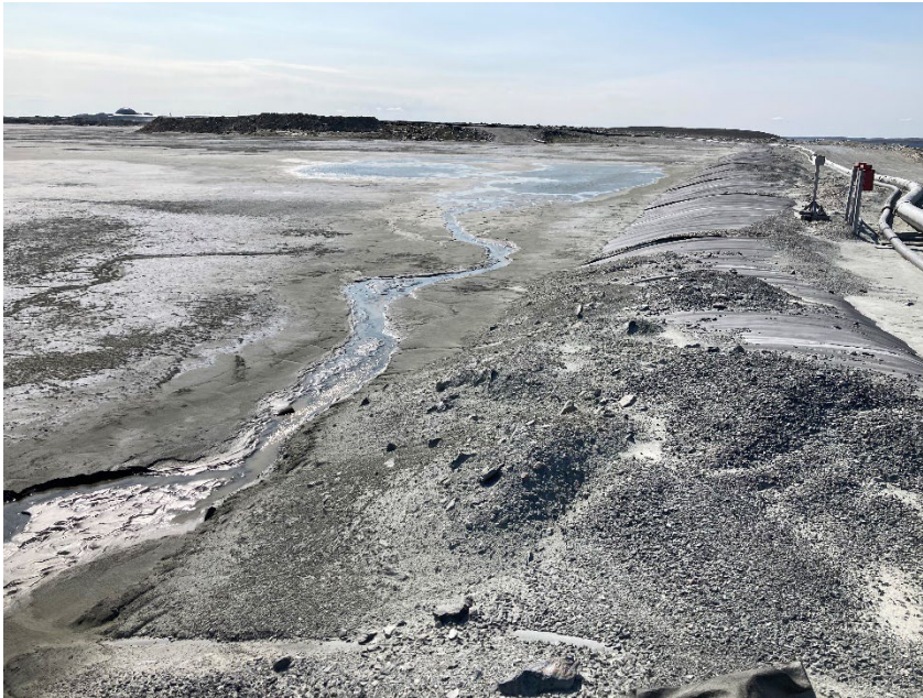
Photograph B2-5 Saddle Dam 1
