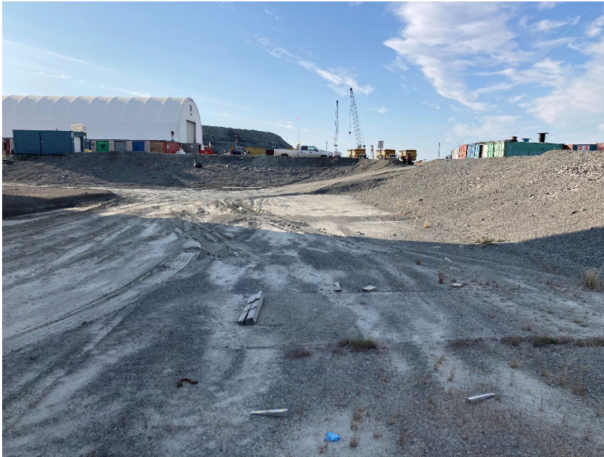
Photograph G2-1 Meadowbank Tank Farm
