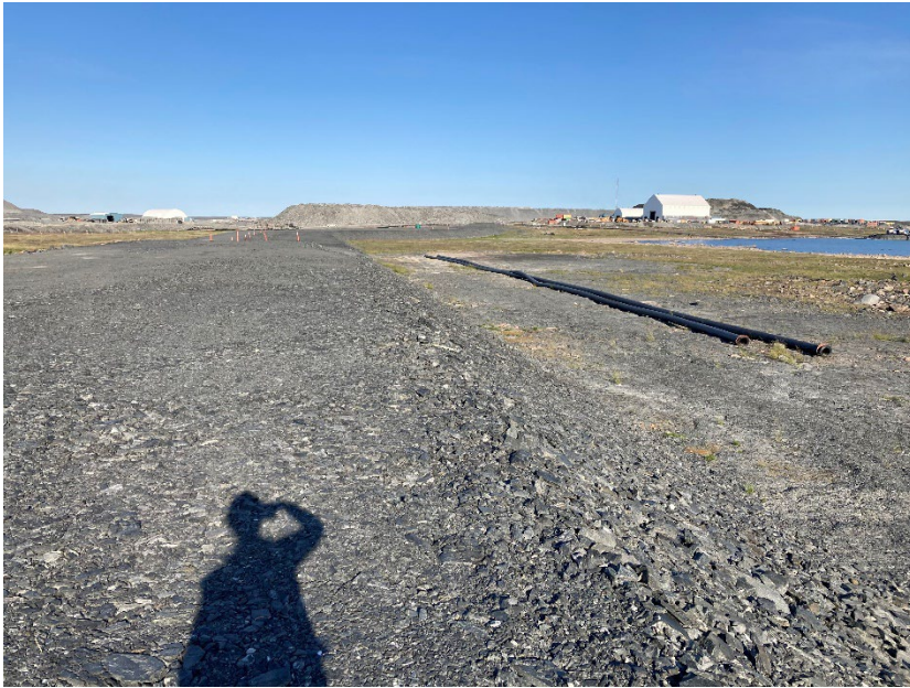
Photograph A6-1 IVR Dike D-1
