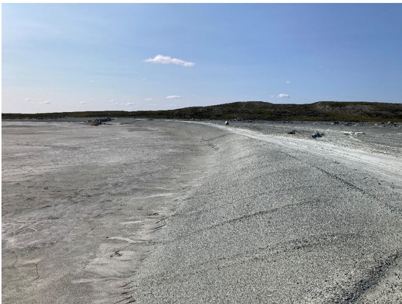
Photograph B1-4 Tailings Storage Facility
