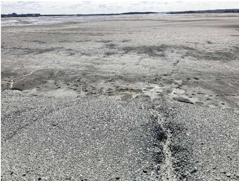
Photograph B1-6 Tailings Storage Facility
