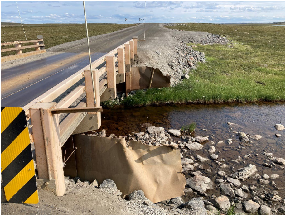
Photograph D3-17 Bridges 9 – R19 km 83+150
