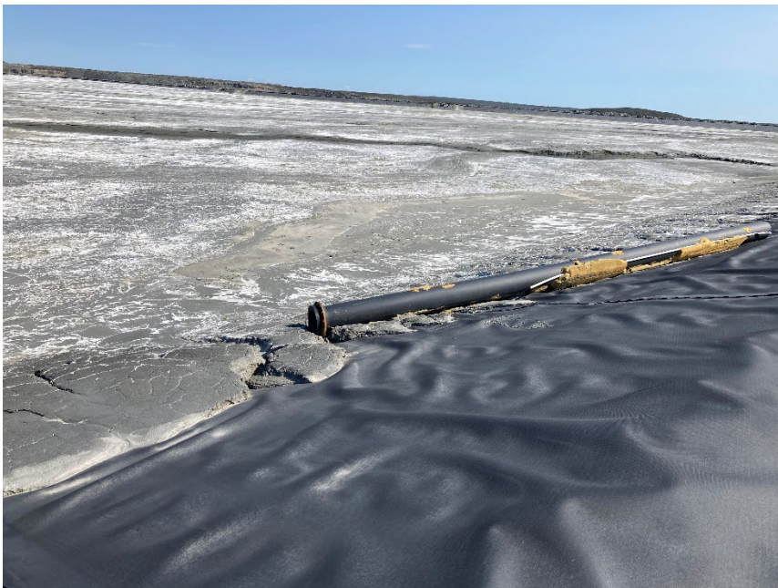
Photograph B6-6 Saddle Dam 4
