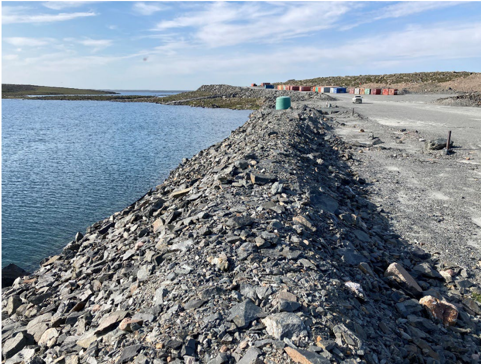
Photograph A1-7 East Dike
