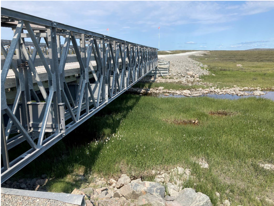
Photograph D3-3 Bridges 2 – R05 km 17+600
