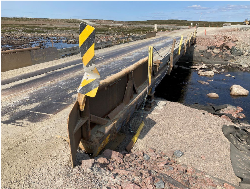
Photograph D3-11 Bridges 6 – R15 km 69+200
