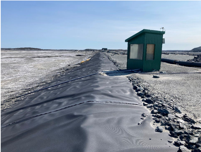
Photograph B6-5 Saddle Dam 4
