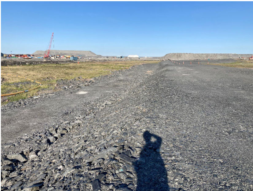
Photograph A6-2 IVR Dike D-1
