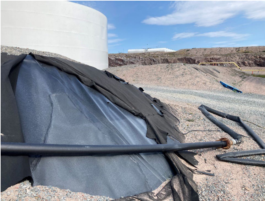
Photograph G1-7 Baker Lake Tank Farm
