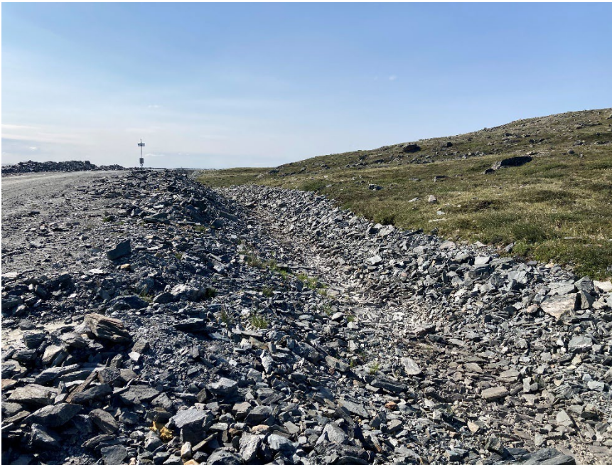
Photograph H2-14 Diversion Ditch and its Sediment and Erosion Protection Structure
