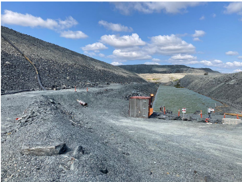
Photograph B7-10 Central Dike and Saddle Dam 5
