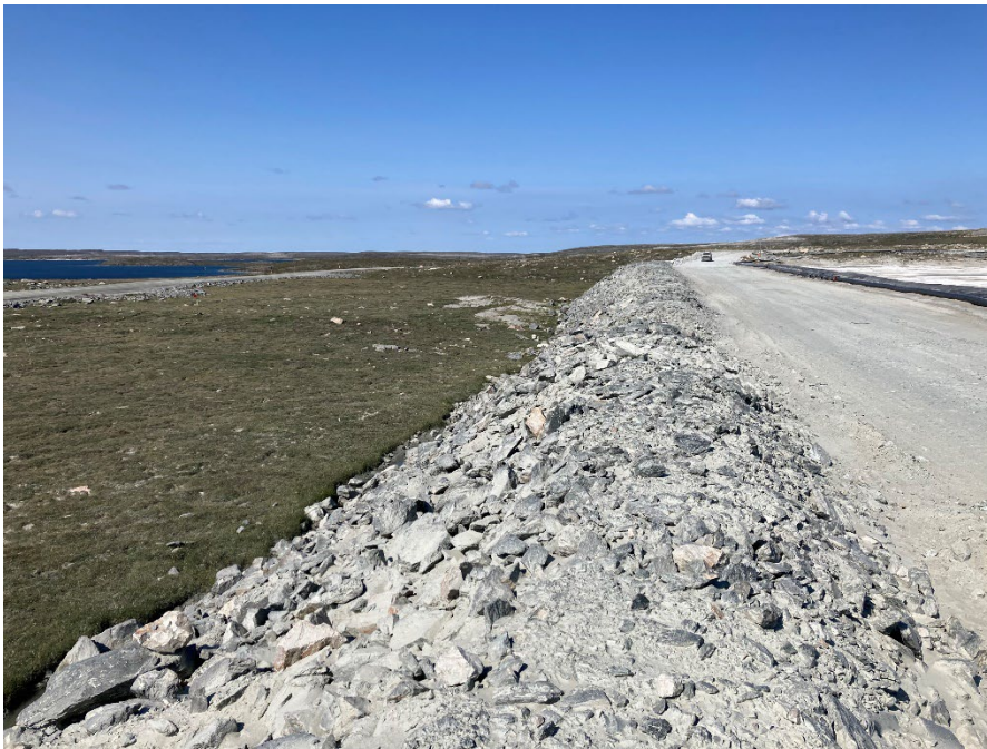
Photograph B3-4 Saddle Dam 2
