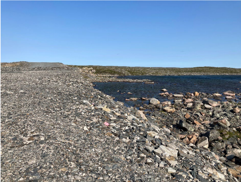
Photograph A4-5 Vault Dike
