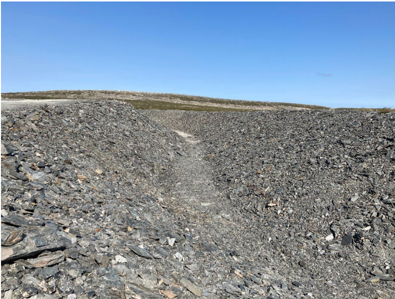
Photograph H2-6 Diversion Ditch and its Sediment and Erosion Protection Structure
