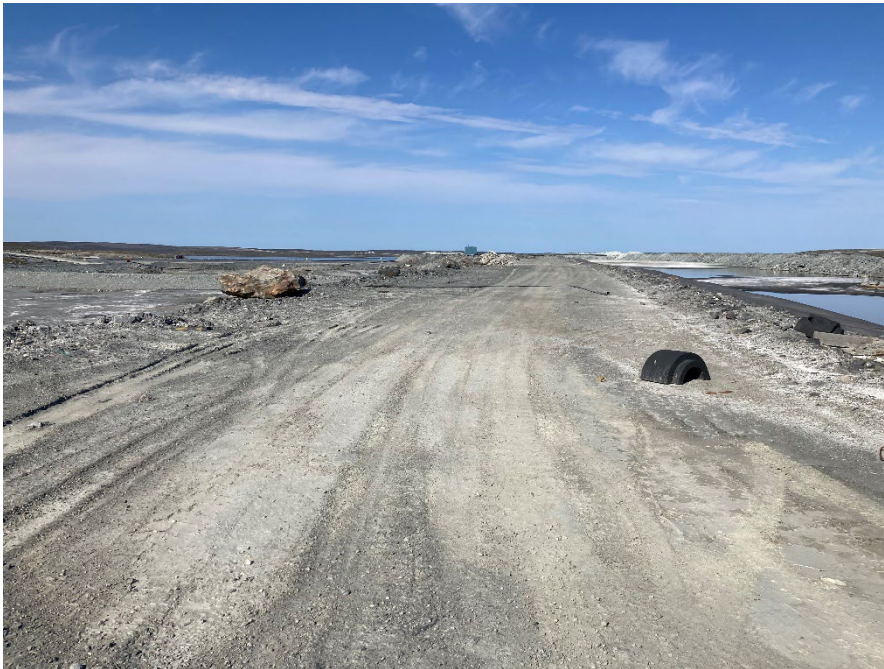
Photograph B4-6 Stormwater Dike
