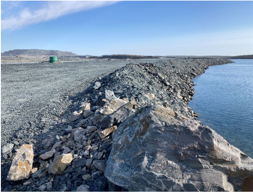
Photograph A3-5 Bay Goose Dike
