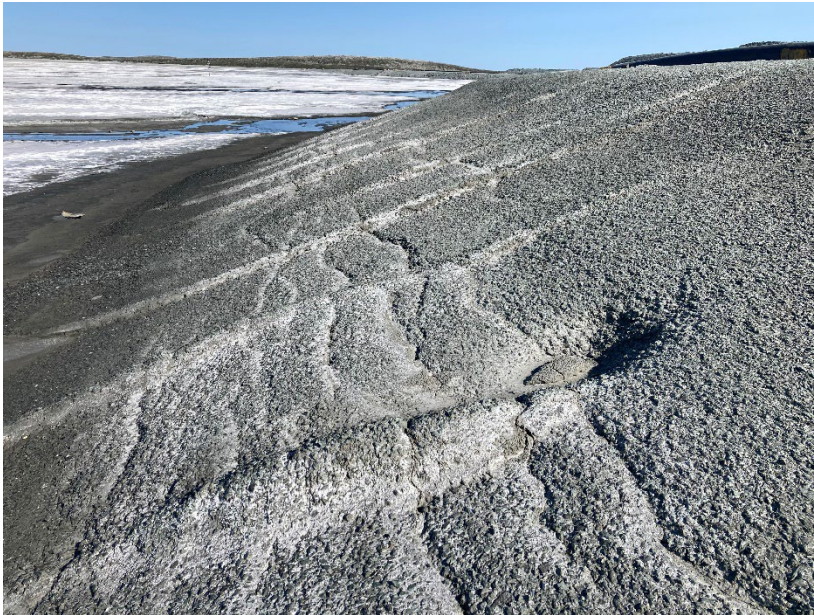
Photograph B1-15 Tailings Storage Facility
