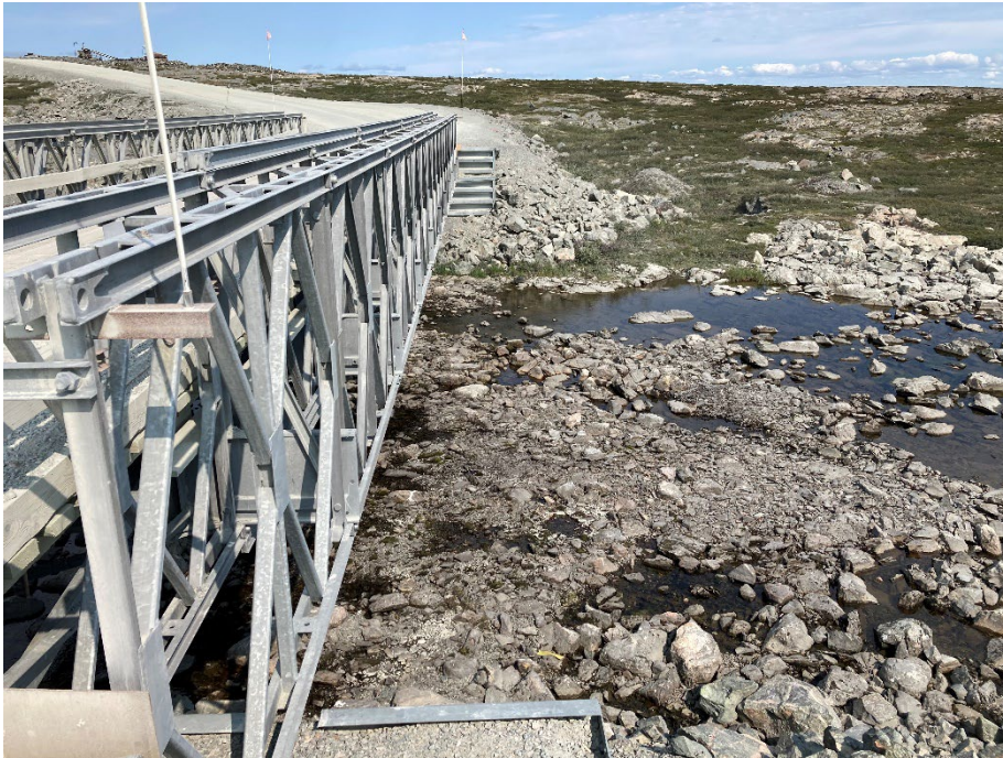
Photograph D3-5 Bridges 3 – R06 km 23+100
