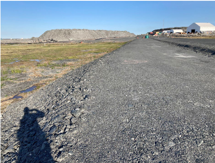
Photograph A6-8 IVR Dike D-1
