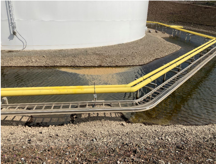
Photograph G1-15 Baker Lake Tank Farm
