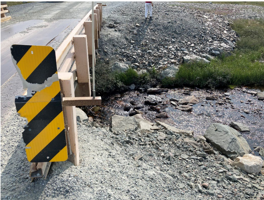
Photograph D3-8 Bridges 4 – R09 km 48+500
