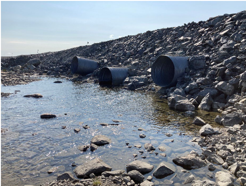
Photograph H1-2 Vault Road Culverts
