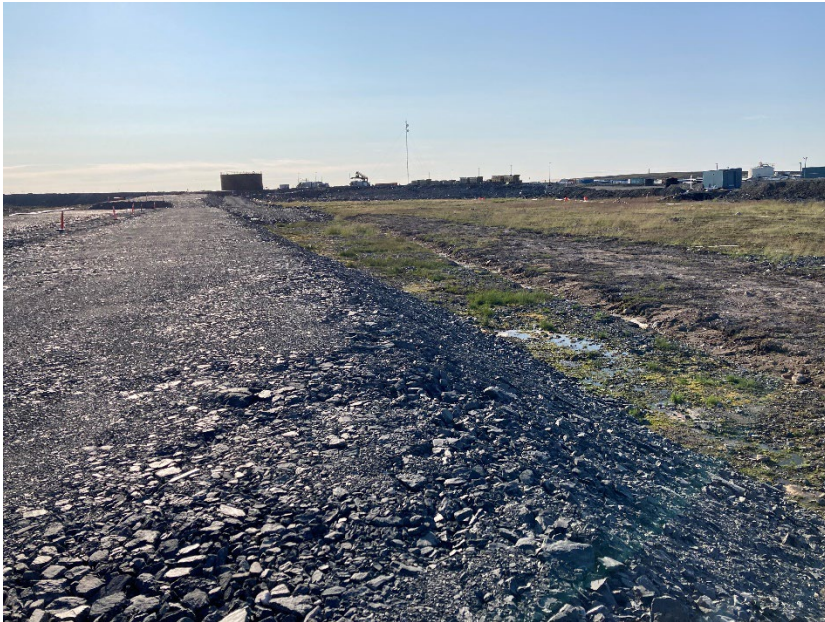
Photograph A6-9 IVR Dike D-1
