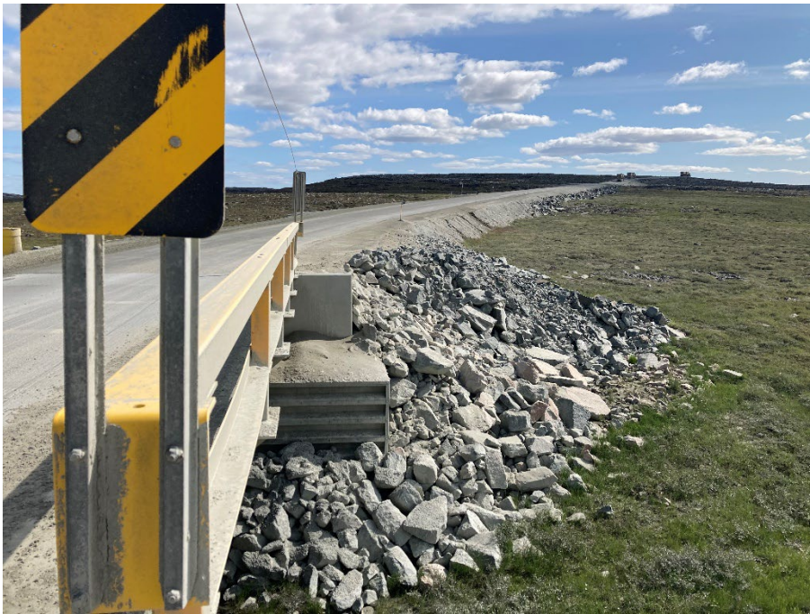
Photograph E2-17 Bridges 8 – km 159+500
