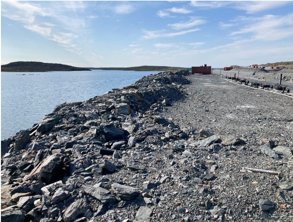
Photograph A1-3 East Dike
