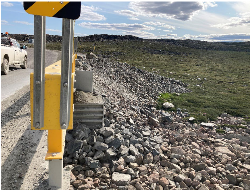
Photograph E2-4 Bridges 2 – km 126+700
