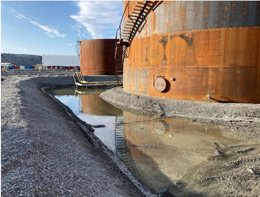
Photograph G2-9 Meadowbank Tank Farm
