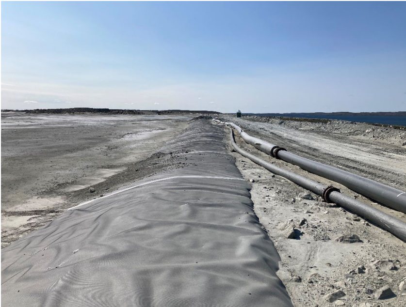
Photograph B2-3 Saddle Dam 1
