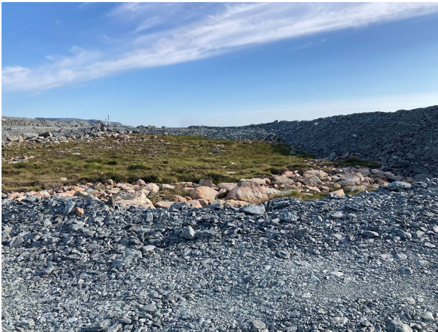
Photograph A3-10 Bay Goose Dike
