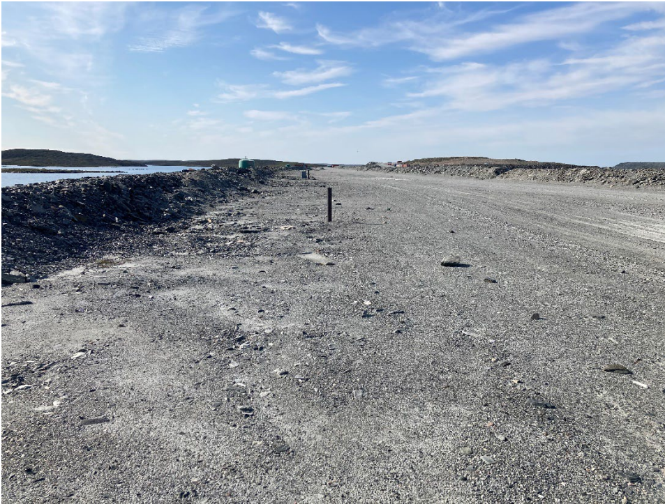
Photograph A1-5 East Dike
