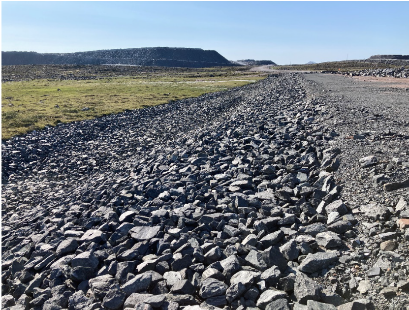
Photograph H13-3 IVR Diversion Channel
