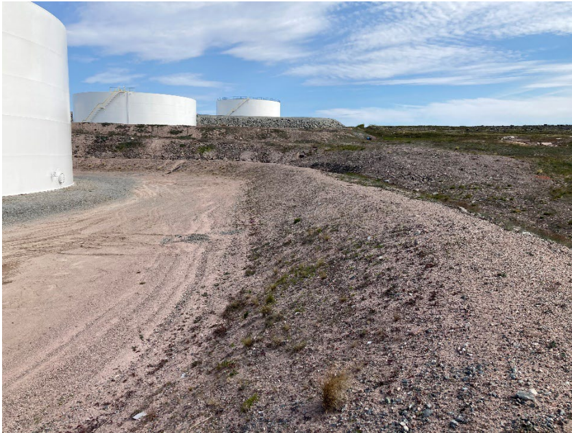
Photograph G1-9 Baker Lake Tank Farm
