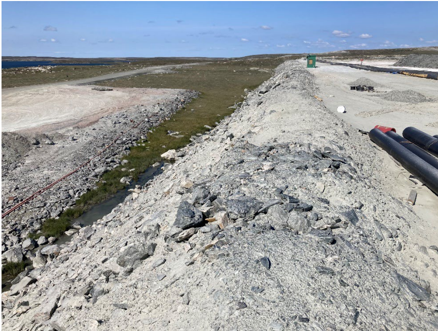
Photograph B3-7 Saddle Dam 2
