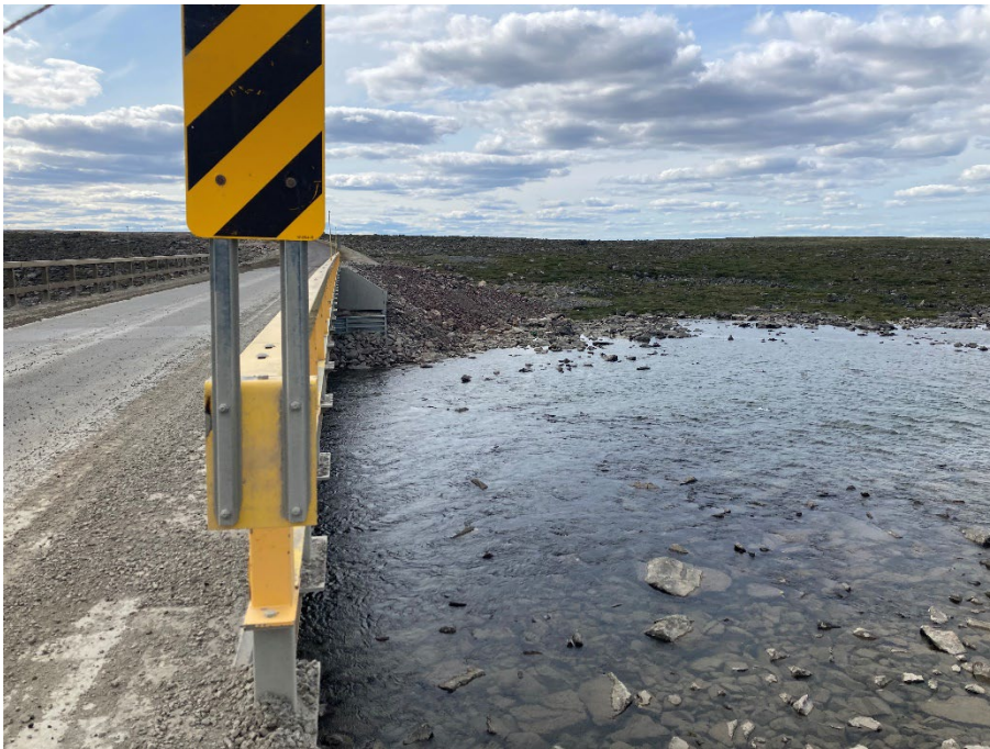
Photograph E2-10 Bridges 5 – km 139+900
