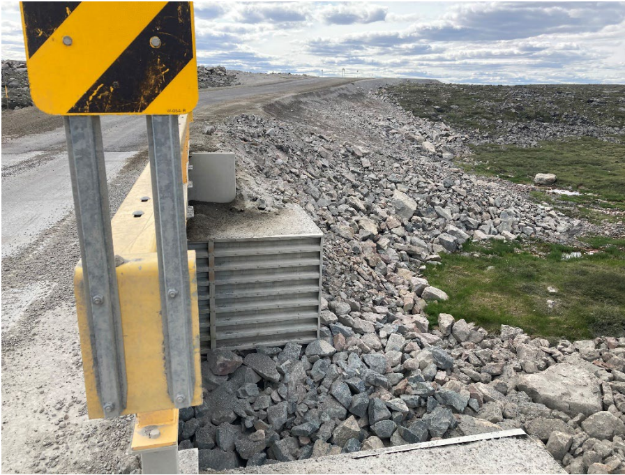
Photograph E2-13 Bridges 6 – km 142+100
