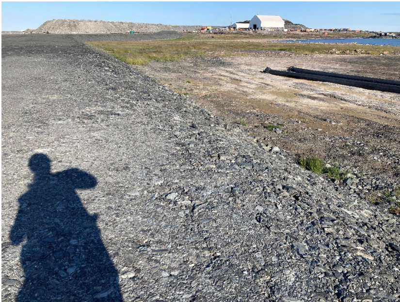
Photograph A6-4 IVR Dike D-1
