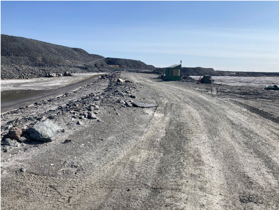
Photograph B4-7 Stormwater Dike
