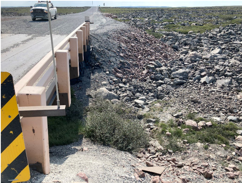
Photograph D3-16 Bridges 8 – R18 km 79+500
