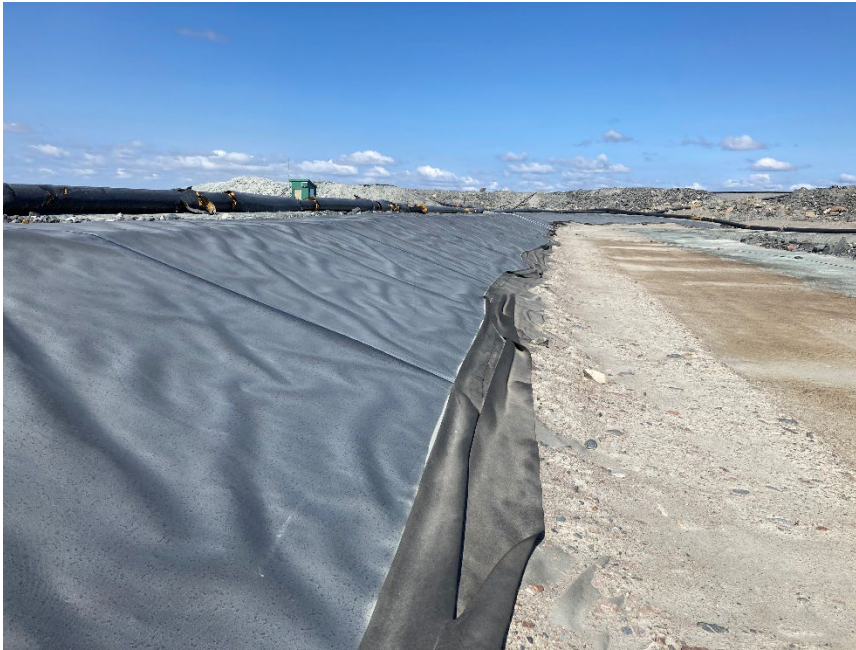
Photograph B5-3 Saddle Dam 3
