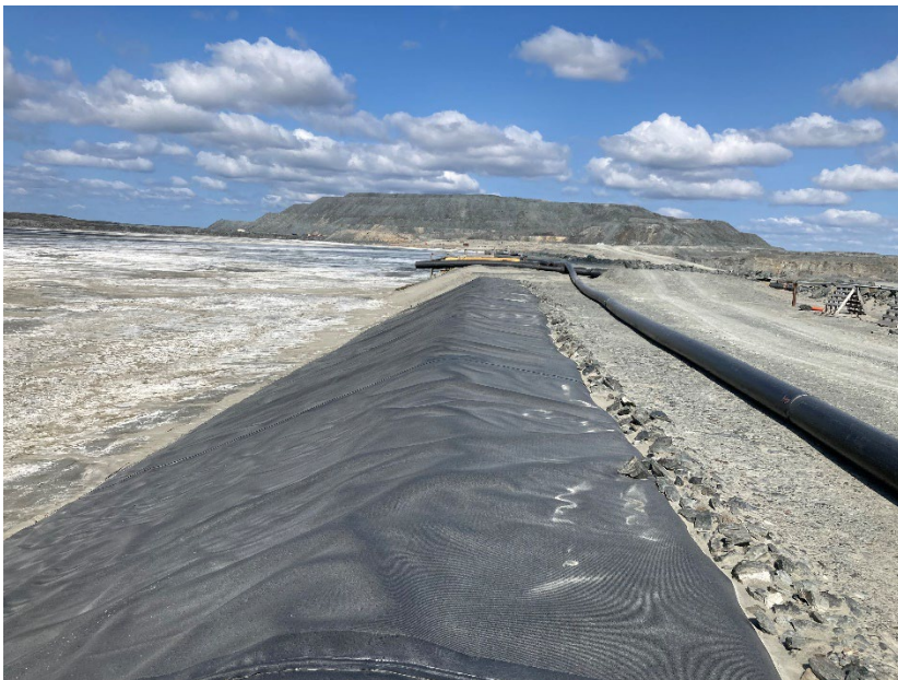
Photograph B7-6 Central Dike and Saddle Dam 5
