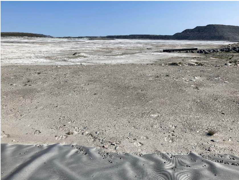
Photograph B2-8 Saddle Dam 1
