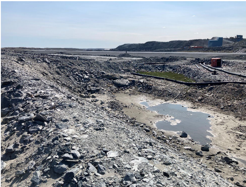
Photograph B6-8 Saddle Dam 4
