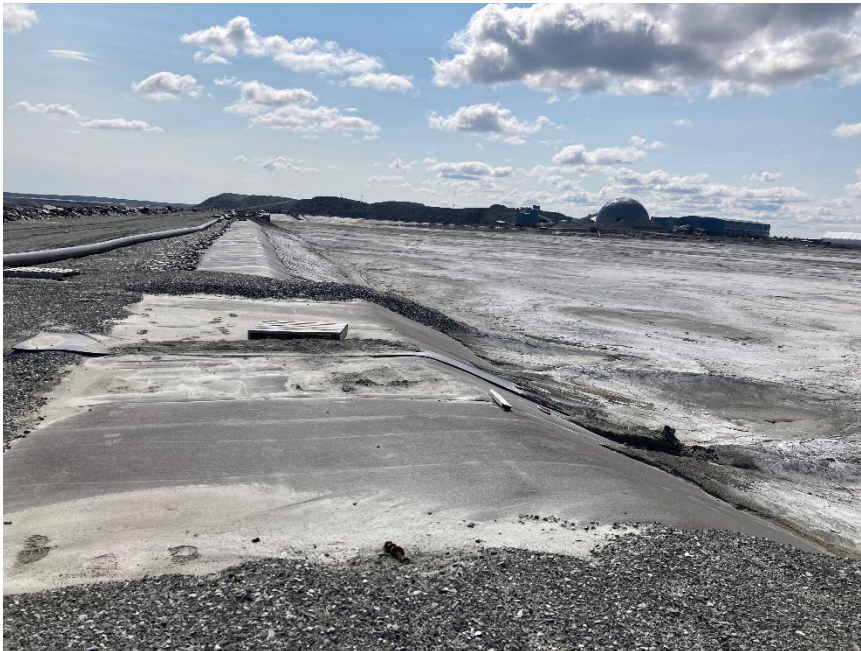
Photograph B7-2 Central Dike and Saddle Dam 5
