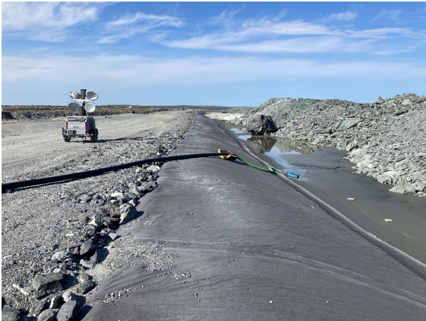
Photograph B4-2 Stormwater Dike
