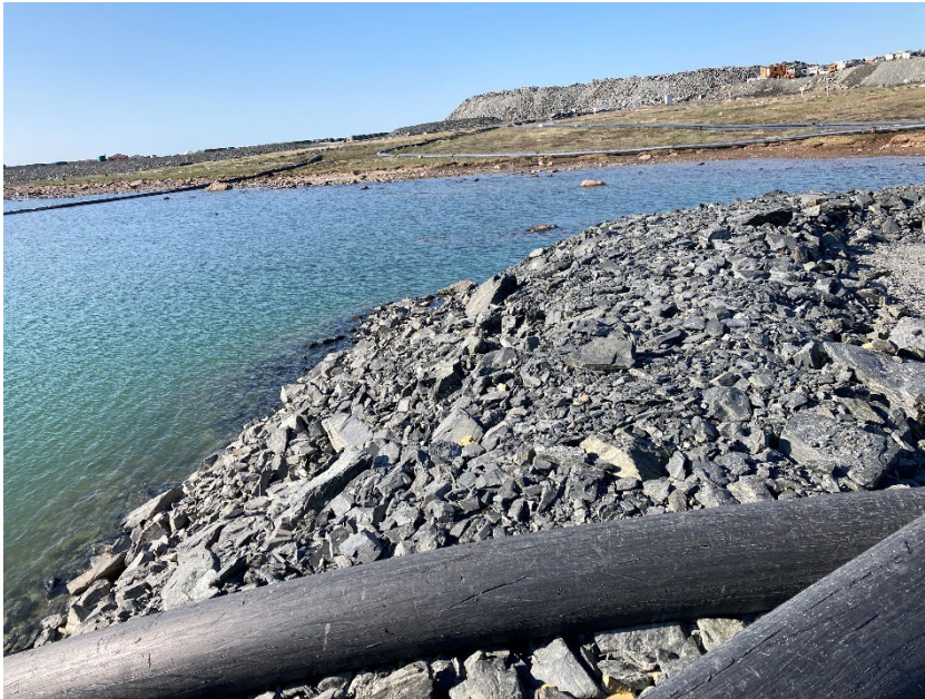
Photograph H8-1 IVR Attenuation Pond Jetty
