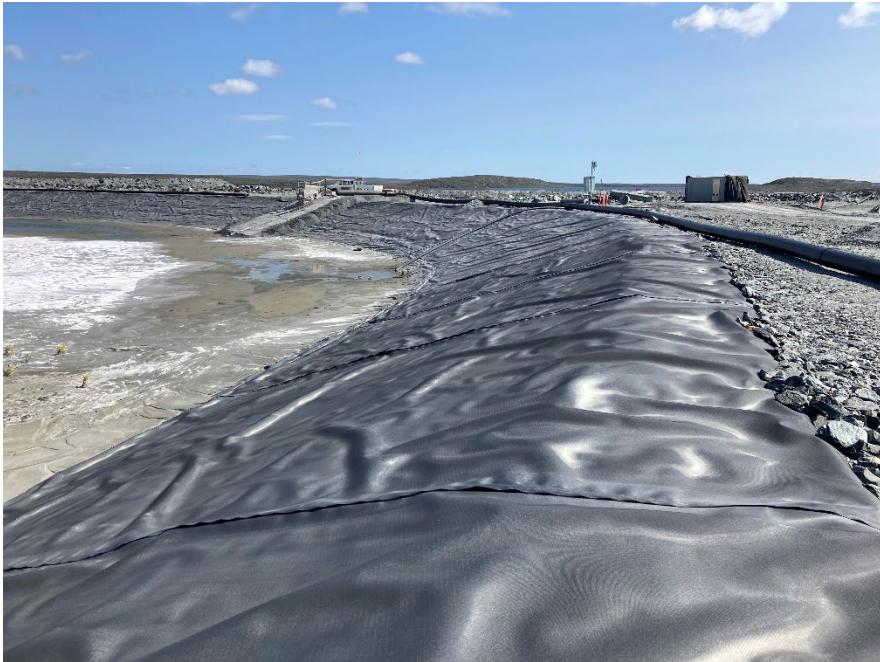
Photograph B7-13 Central Dike and Saddle Dam 5
