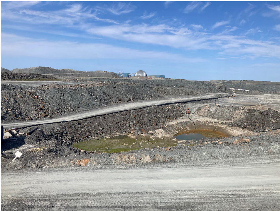
Photograph A1-8 East Dike
