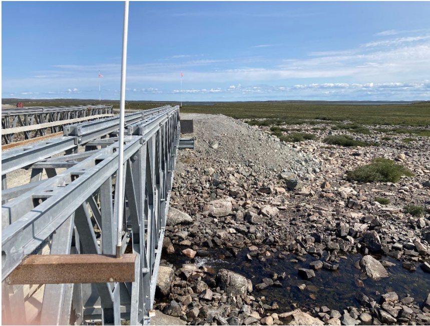
Photograph D3-1 Bridges 1 – R02 km 8+750
