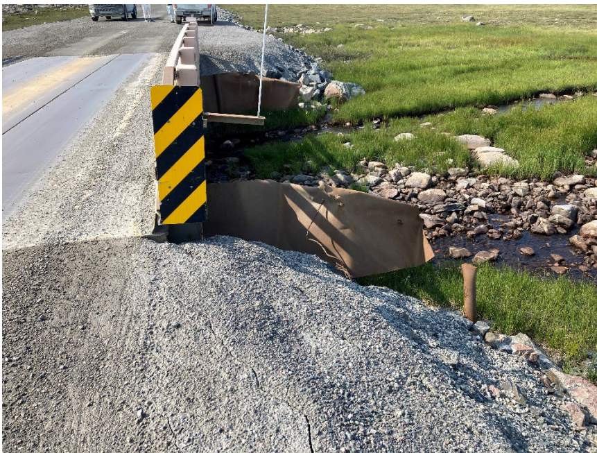
Photograph D3-18 Bridges 9 – R19 km 83+150
