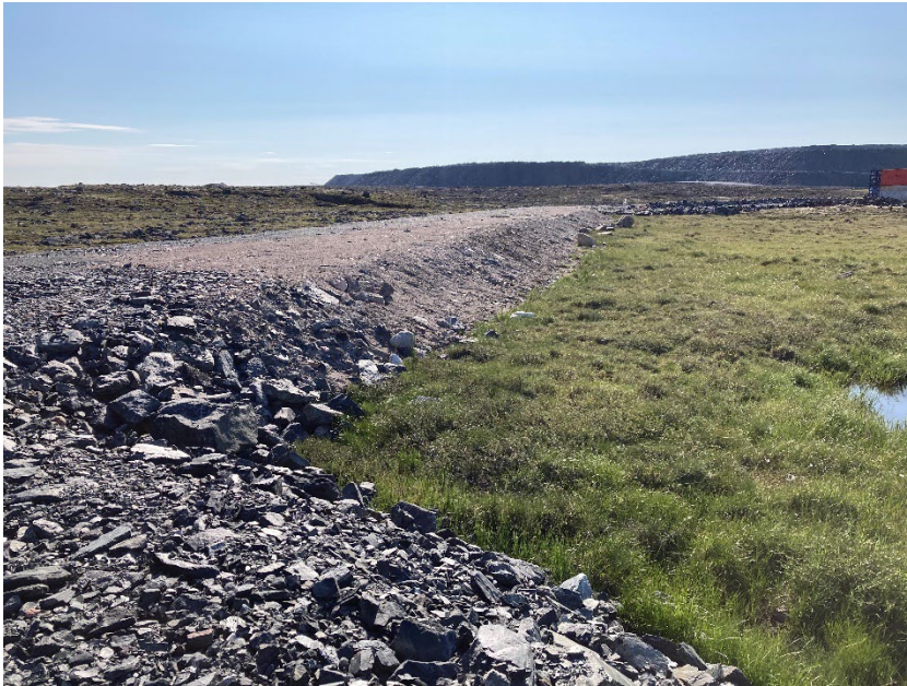
Photograph H13-7 IVR Diversion Channel
