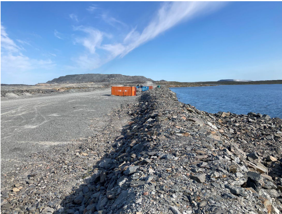
Photograph A1-6 East Dike
