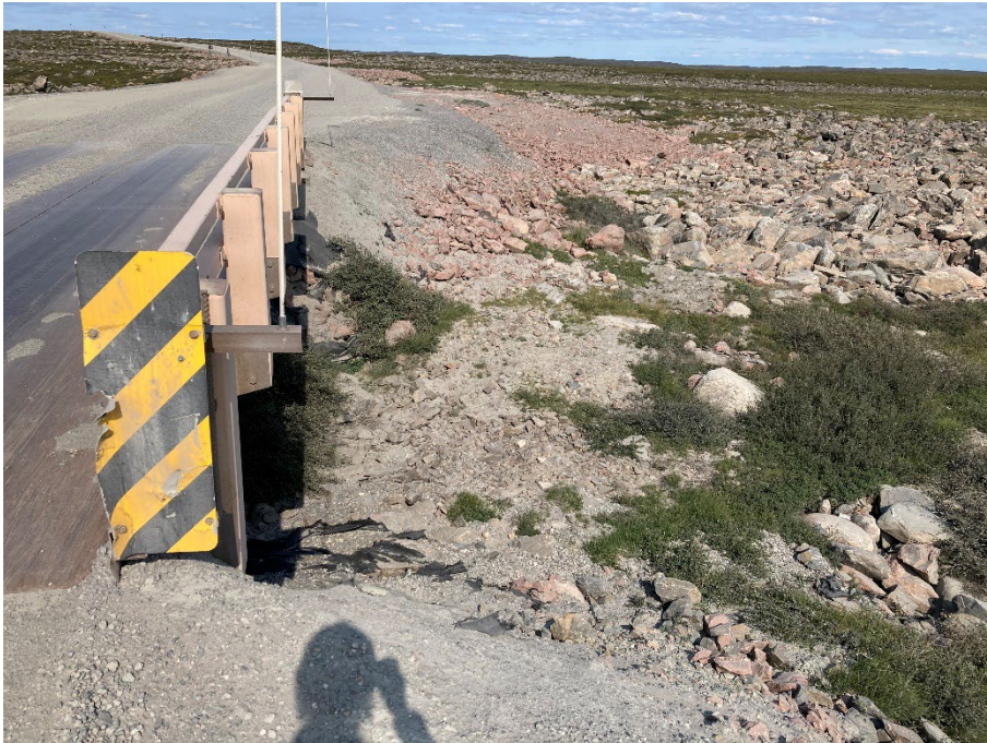
Photograph D3-15 Bridges 8 – R18 km 79+500
