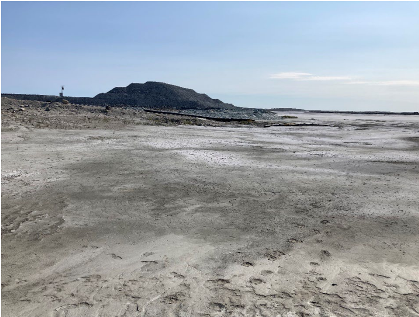
Photograph B2-9 Saddle Dam 1
