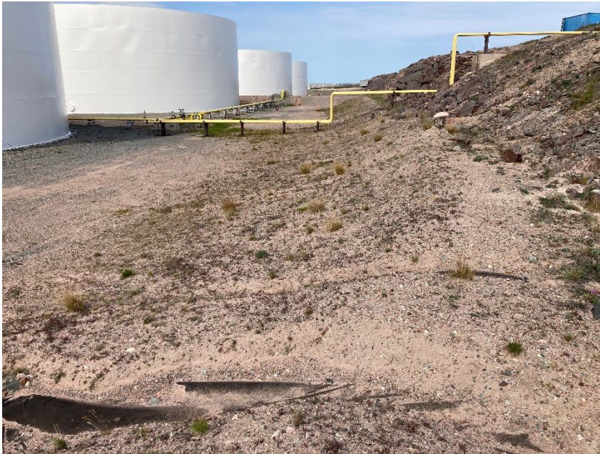
Photograph G1-11 Baker Lake Tank Farm
