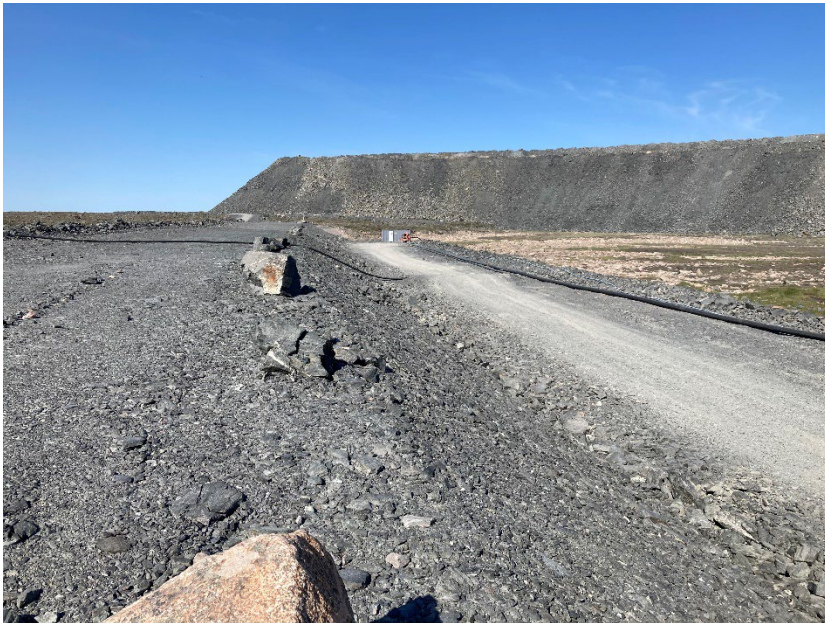
Photograph A7-4 WRSF Dike
