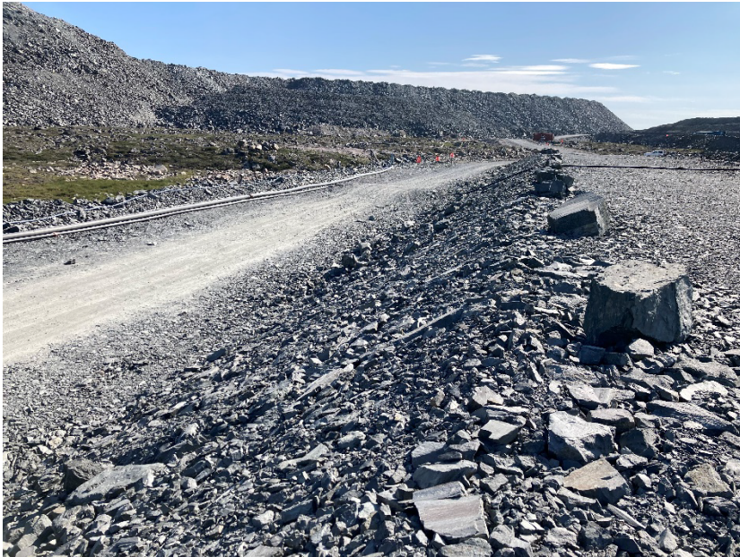
Photograph A7-5 WRSF Dike
