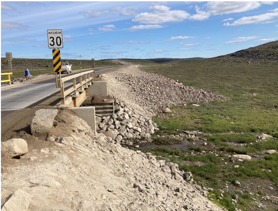
Photograph E2-8 Bridges 4 – km 136+000
