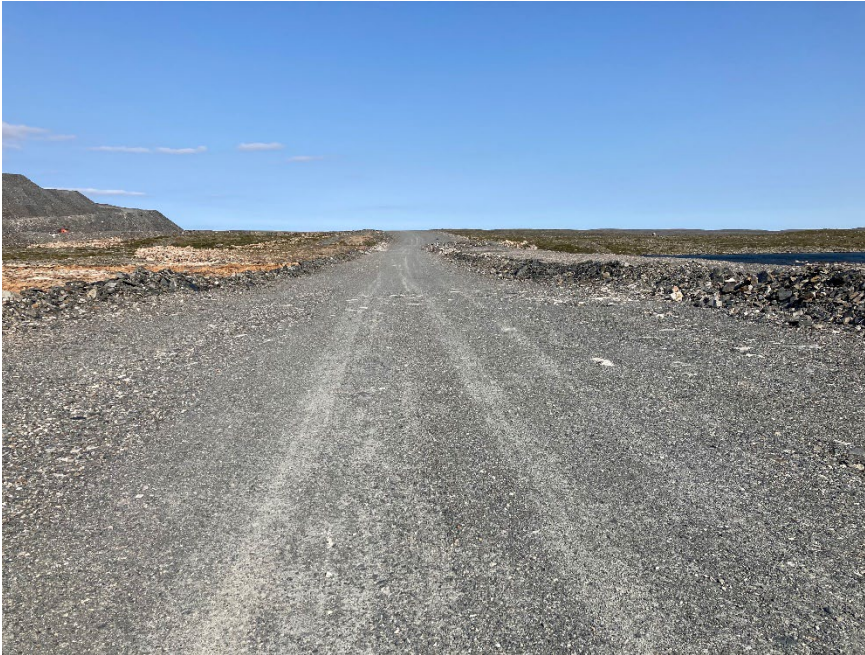
Photograph A4-1 Vault Dike
