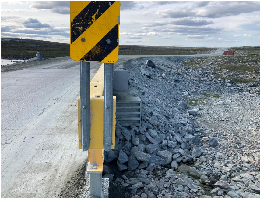
Photograph E2-1 Bridges 1 – km 119+400
