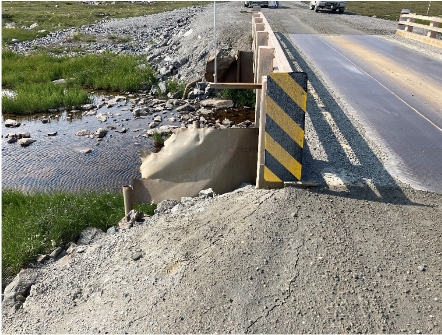
Photograph D3-19 Bridges 9 – R19 km 83+150
