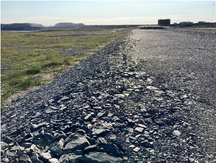
Photograph A6-7 IVR Dike D-1
