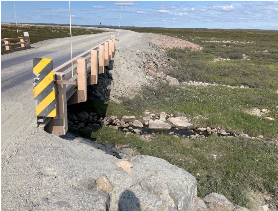
Photograph D3-13 Bridges 7 – R16 km 73+800
