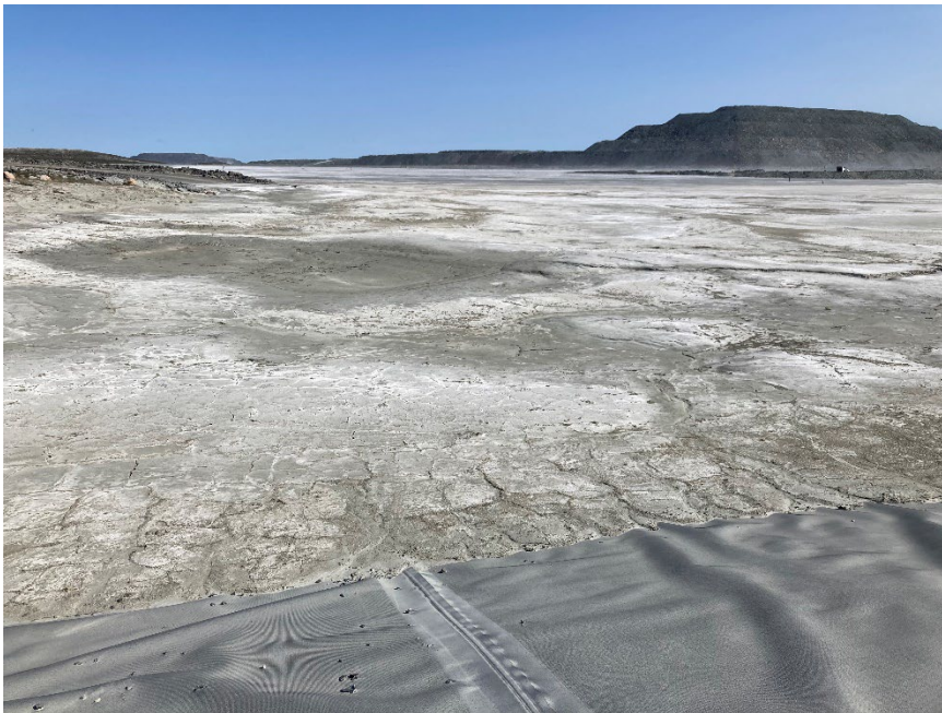
Photograph B3-2 Saddle Dam 2
