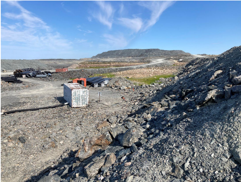
Photograph A1-11 East Dike
