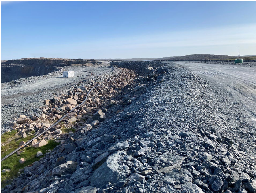
Photograph A3-3 Bay Goose Dike
