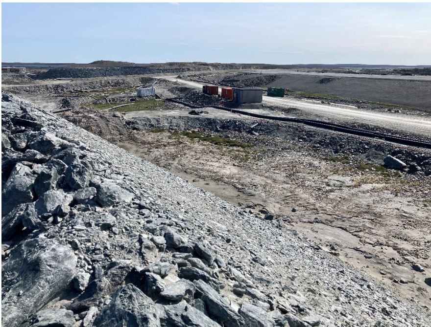
Photograph B7-14 Central Dike and Saddle Dam 5
