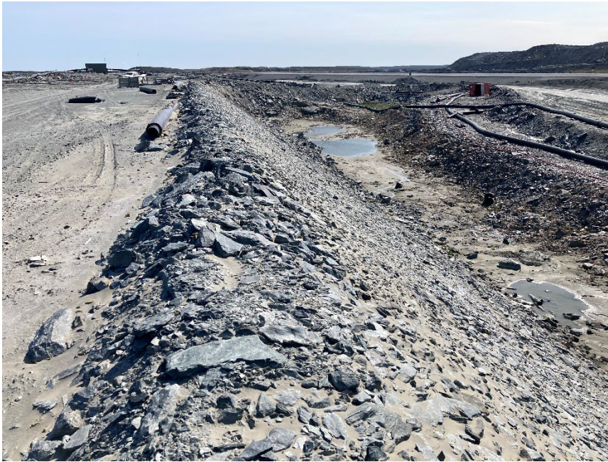
Photograph B6-7 Saddle Dam 4
