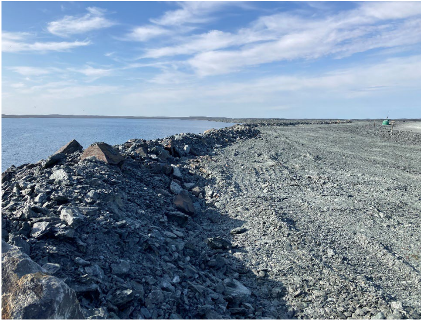
Photograph A3-1 Bay Goose Dike
