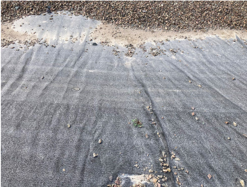
Photograph G1-23 Baker Lake Tank Farm
