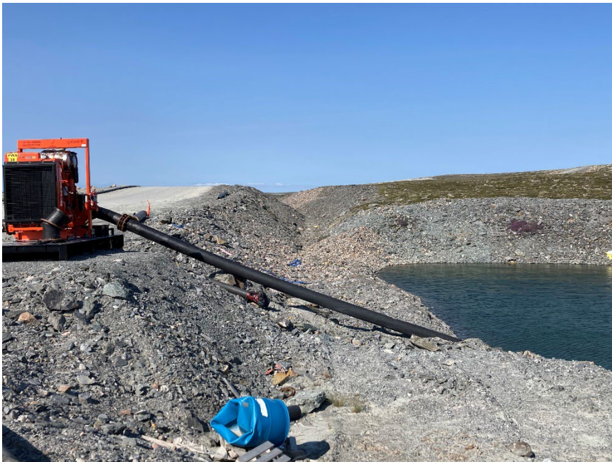
Photograph H2-16 Diversion Ditch and its Sediment and Erosion Protection Structure
