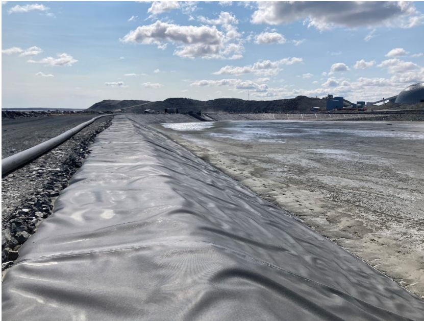
Photograph B7-5 Central Dike and Saddle Dam 5
