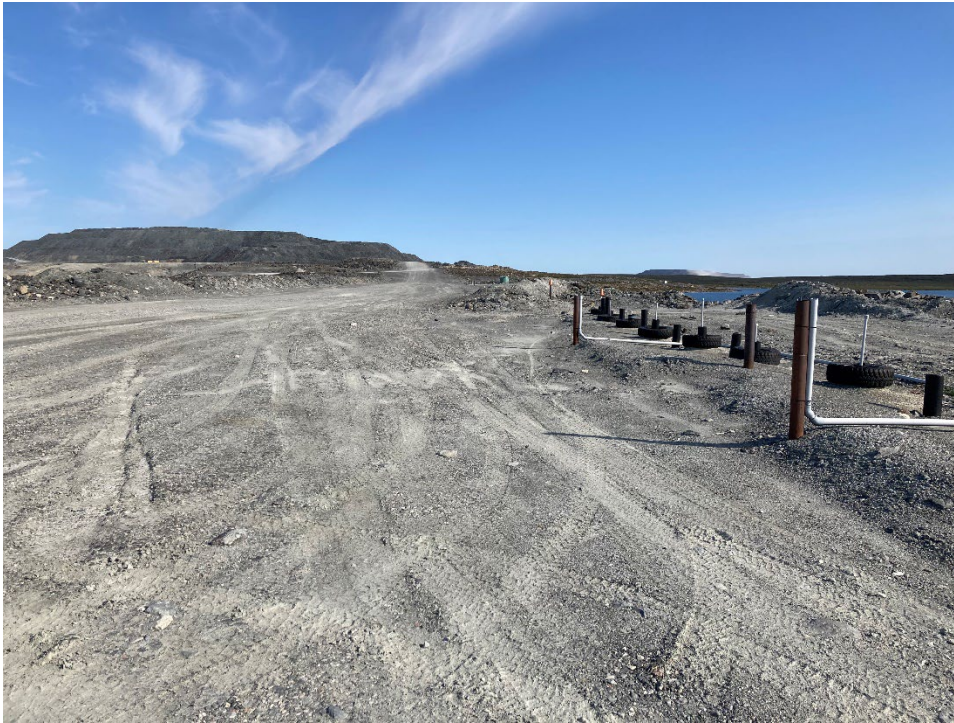
Photograph A1-1 East Dike
