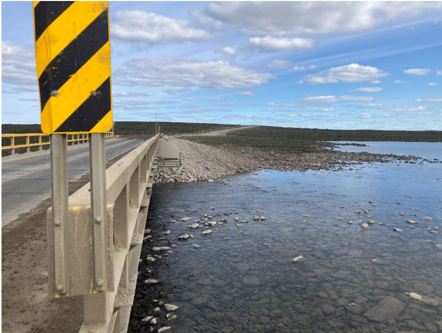
Photograph E2-11 Bridges 5 – km 139+900
