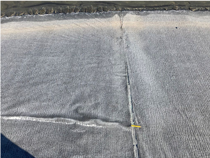
Photograph B4-8 Stormwater Dike
