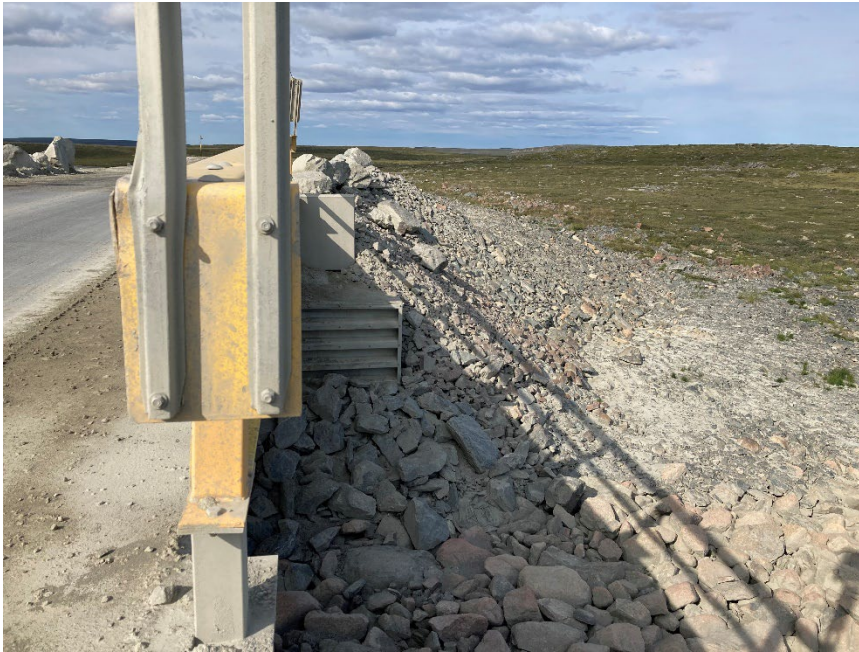
Photograph E2-3 Bridges 2 – km 126+700
