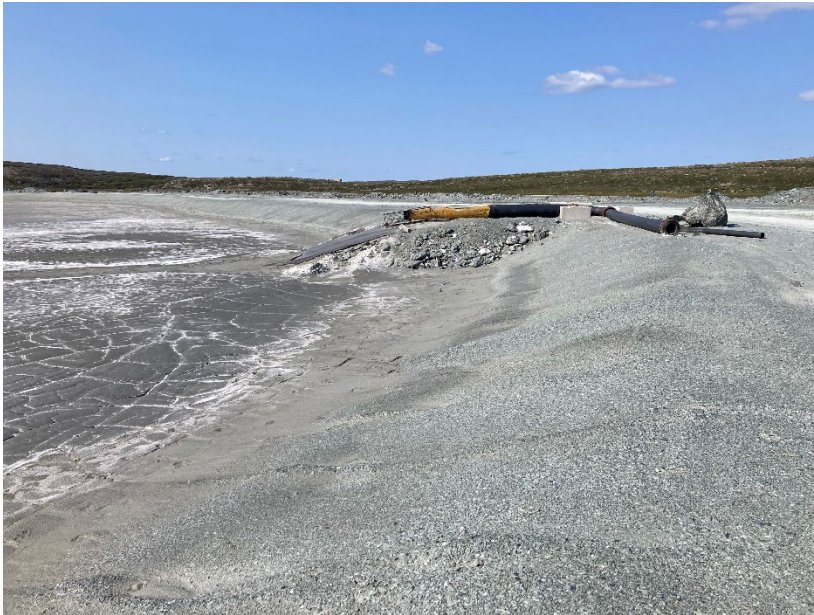
Photograph B1-7 Tailings Storage Facility
