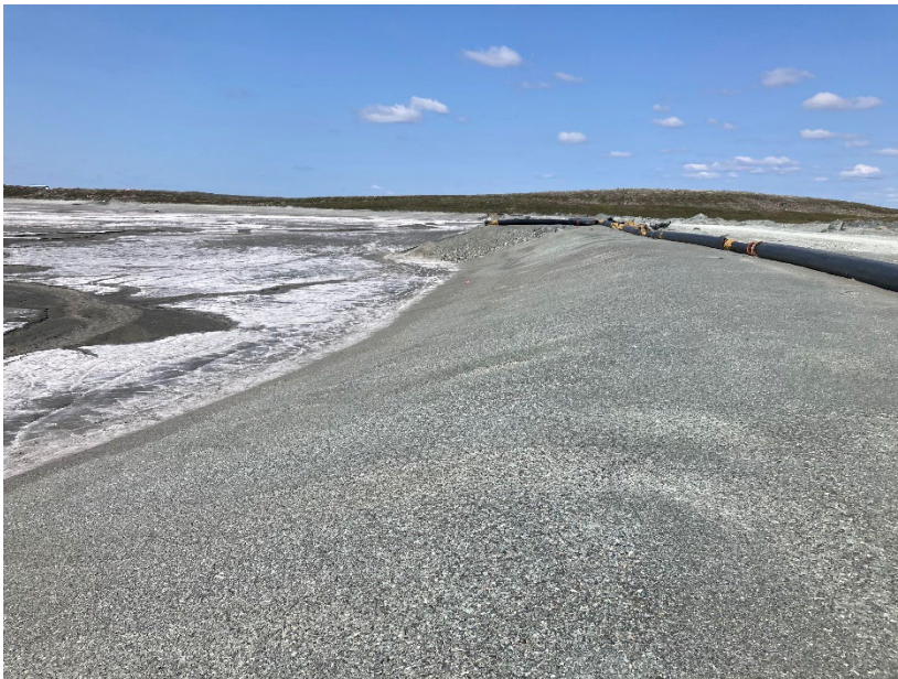
Photograph B1-8 Tailings Storage Facility
