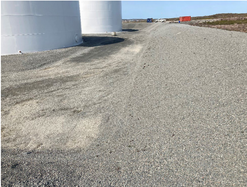
Photograph G1-19 Baker Lake Tank Farm
