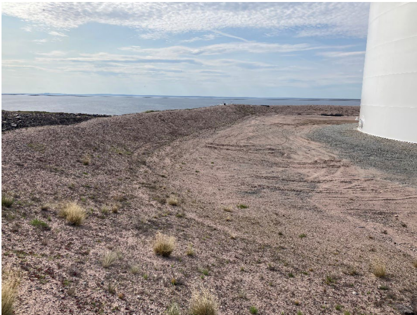
Photograph G1-10 Baker Lake Tank Farm
