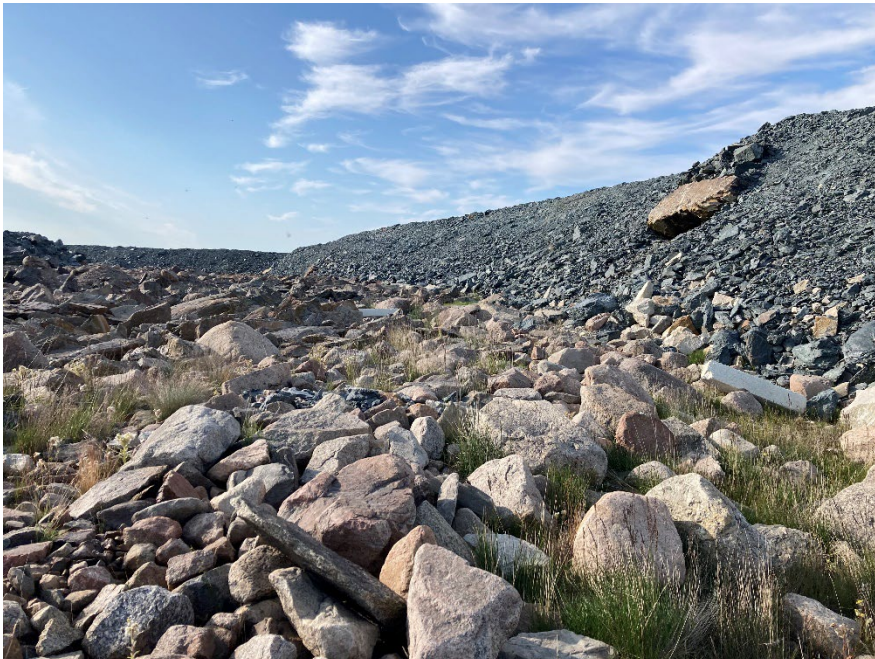
Photograph A3-32 Bay Goose Dike
