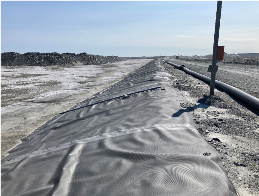
Photograph B3-5 Saddle Dam 2
