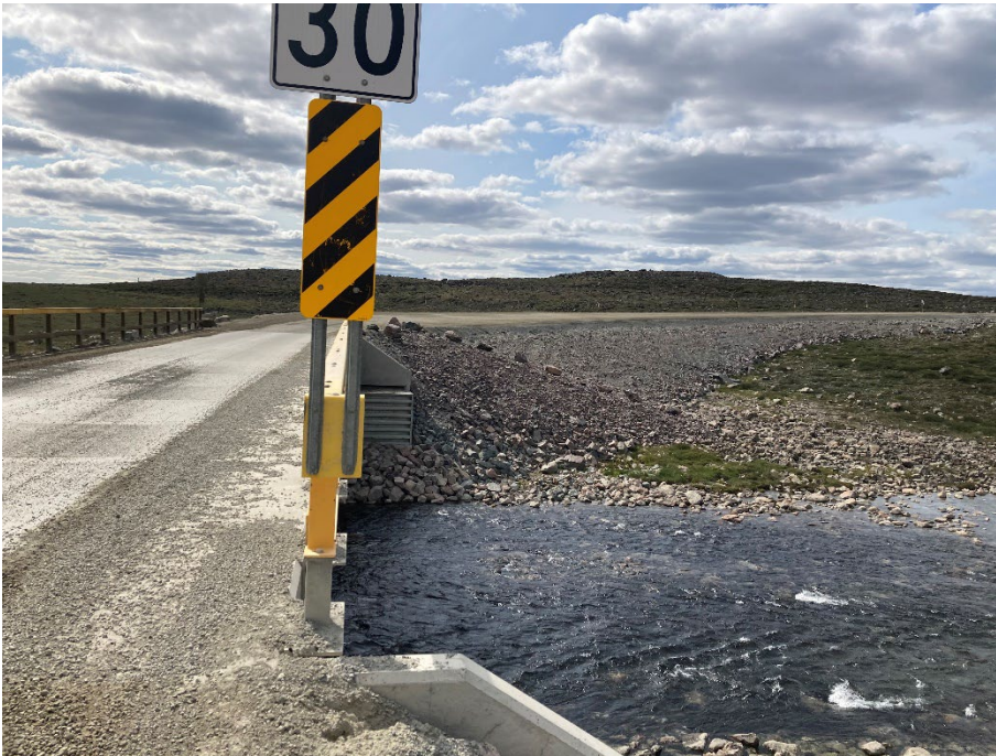
Photograph E2-14 Bridges 7 – km 148+300
