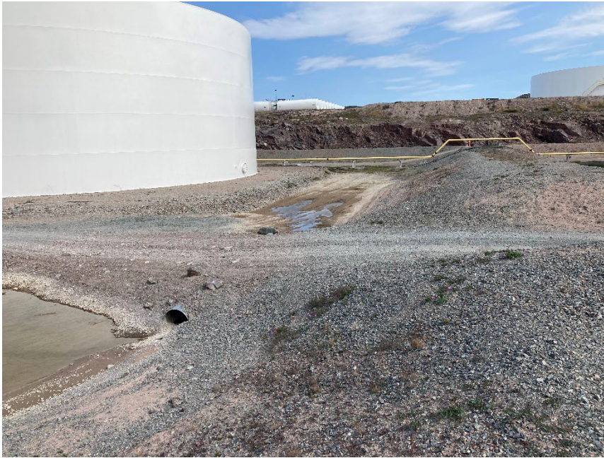
Photograph G1-3 Baker Lake Tank Farm
