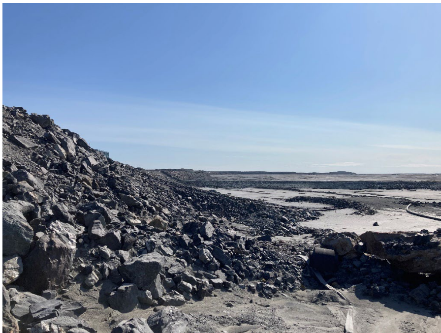
Photograph B4-11 Stormwater Dike
