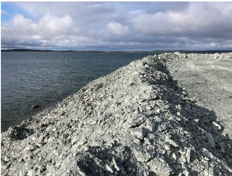
Photograph A3-18 Bay Goose Dike
