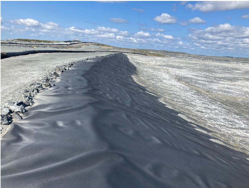
Photograph B6-2 Saddle Dam 4
