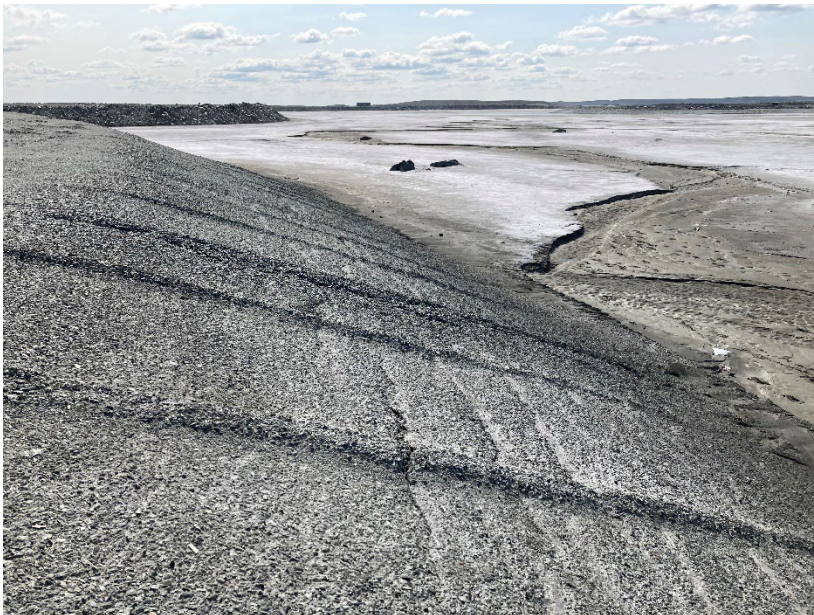
Photograph B1-12 Tailings Storage Facility
