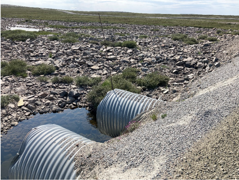
Photograph D2-1: PC-17A km 8+830
