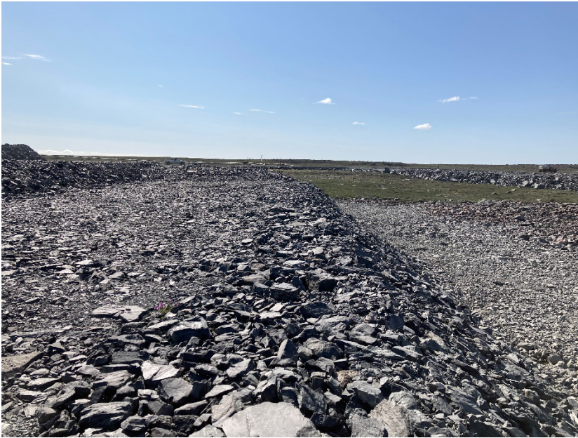
Photograph A8-7 Mammoth Dike
