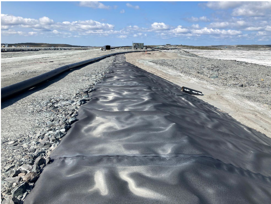
Photograph B7-12 Central Dike and Saddle Dam 5
