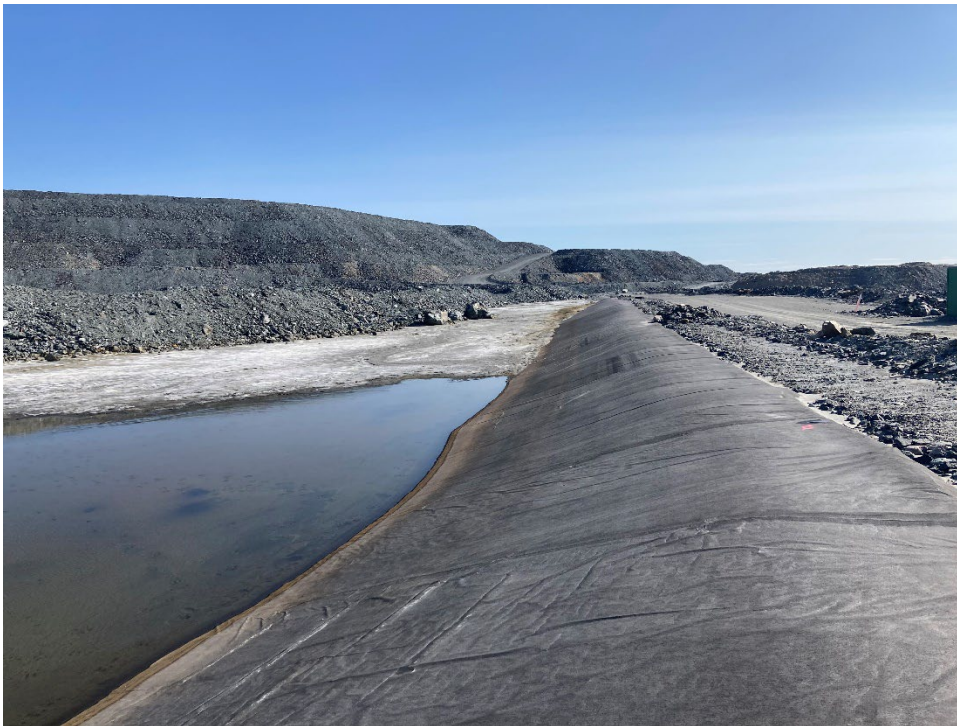
Photograph B4-4 Stormwater Dike
