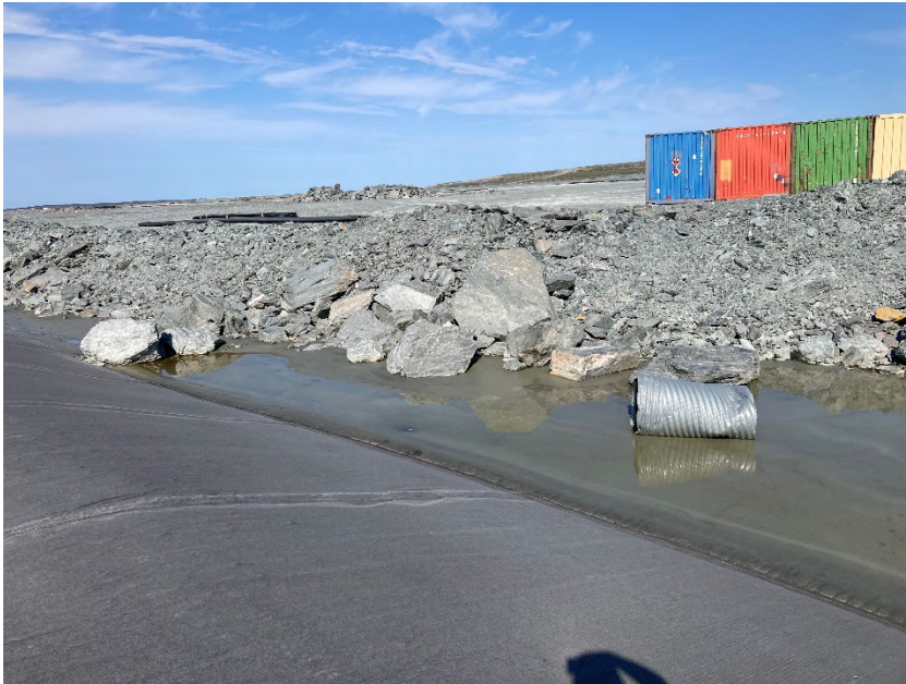
Photograph B4-1 Stormwater Dike
