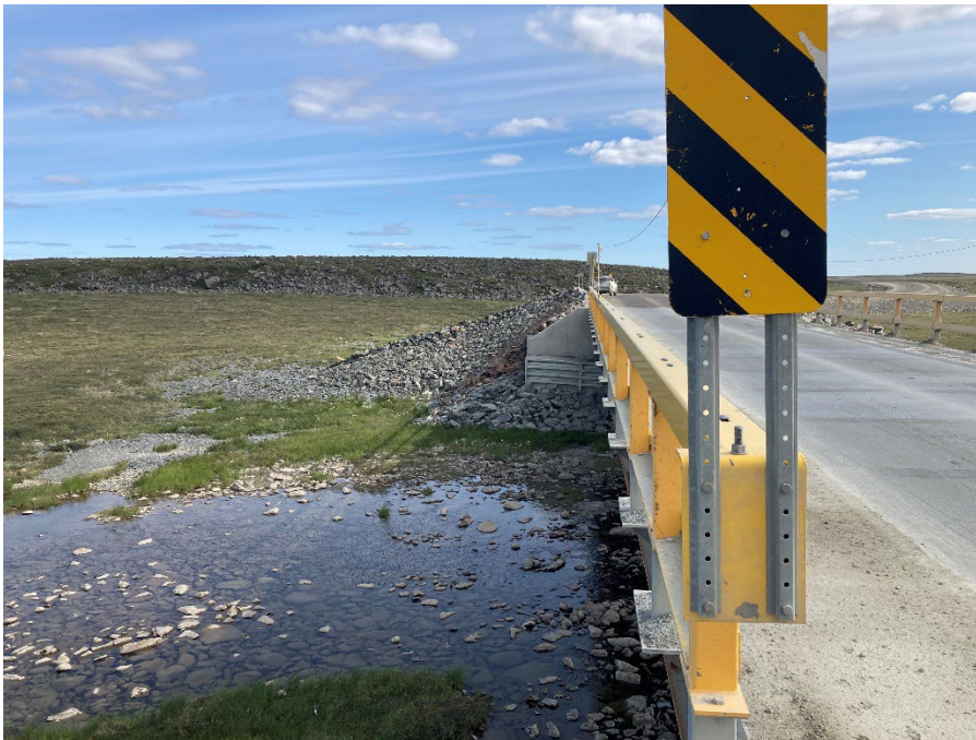
Photograph E2-6 Bridges 3 – km 132+000
