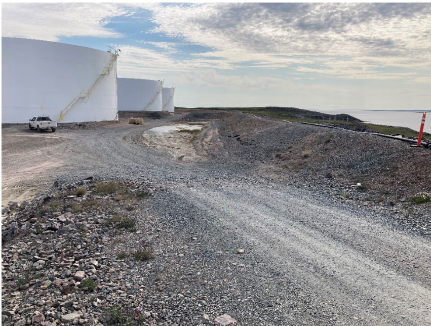
Photograph G1-2 Baker Lake Tank Farm
