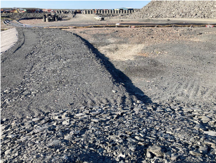
Photograph A6-15 IVR Dike D-1
