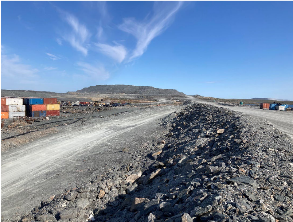
Photograph A1-9 East Dike
