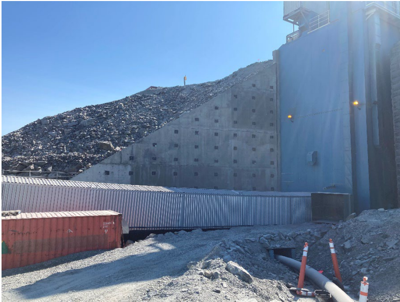
Photograph H6-1 Meadowbank Crusher Retaining Wall
