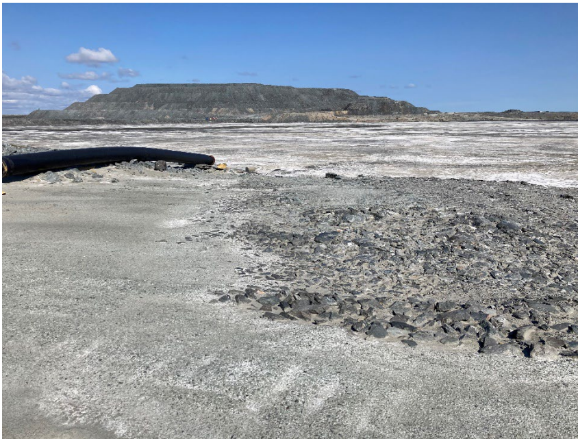
Photograph B6-4 Saddle Dam 4
