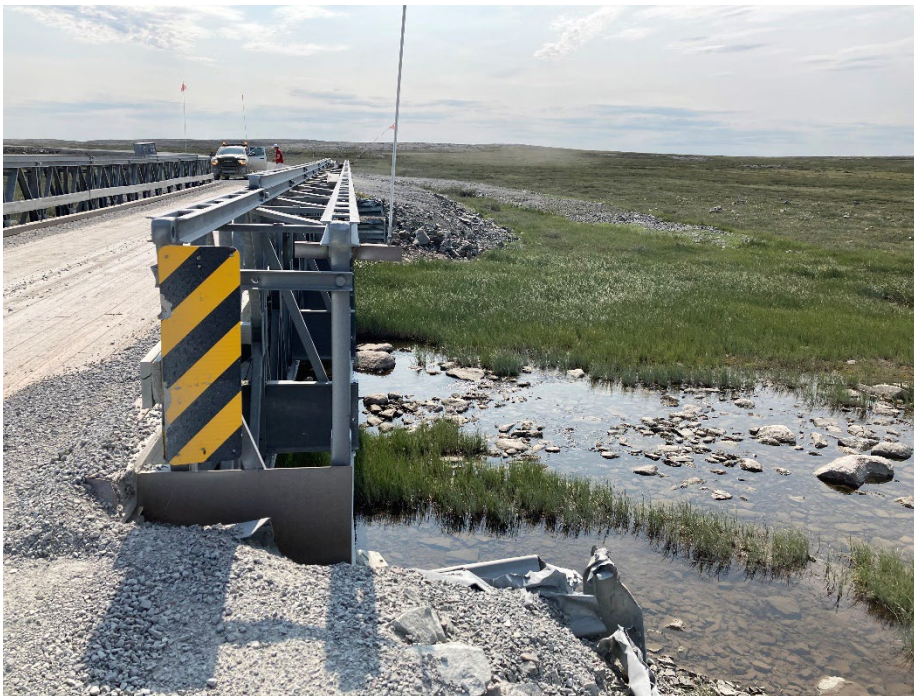
Photograph D3-4 Bridges 2 – R05 km 17+600
