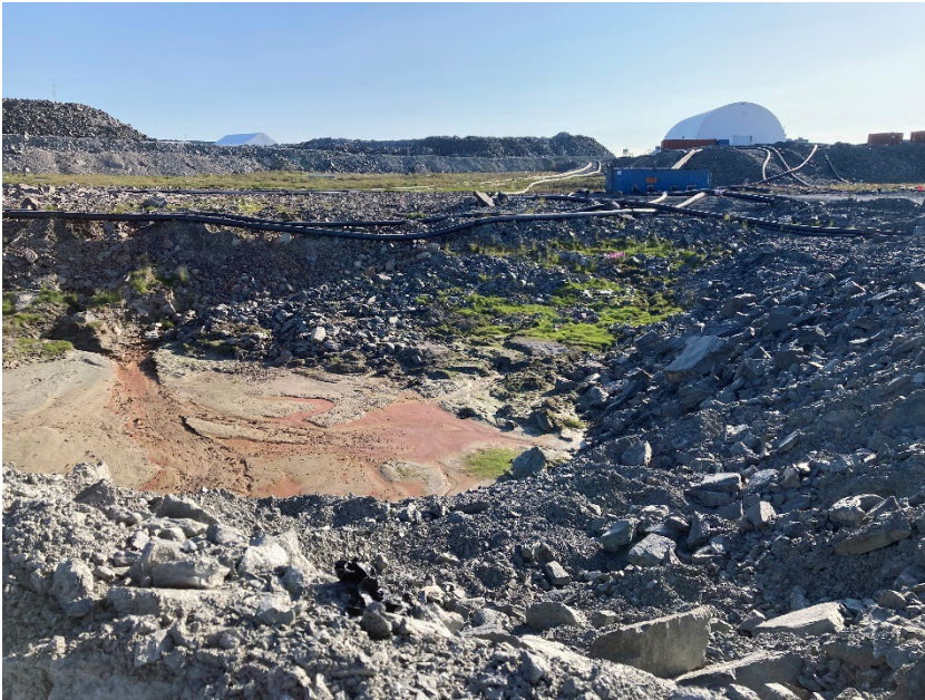
Photograph H7-1 Whale Tail Mine Site Attenuation Pond Jetty
