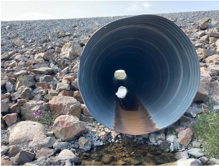
Photograph D2-3: R-14 km 67+840
