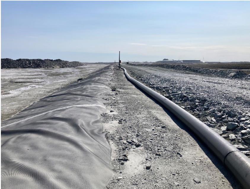
Photograph B3-1 Saddle Dam 2
