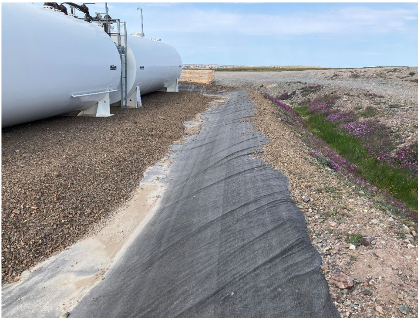
Photograph G1-24 Baker Lake Tank Farm
