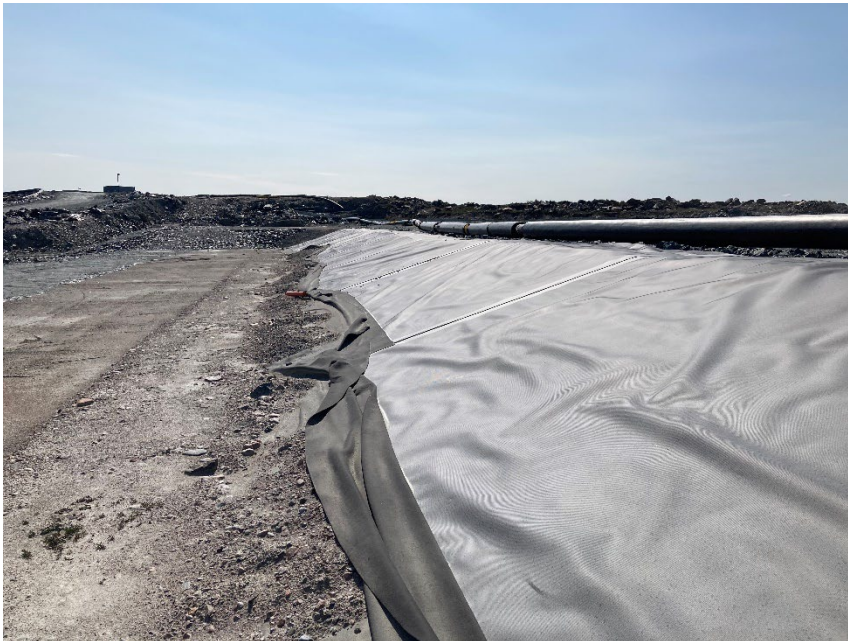
Photograph B5-2 Saddle Dam 3
