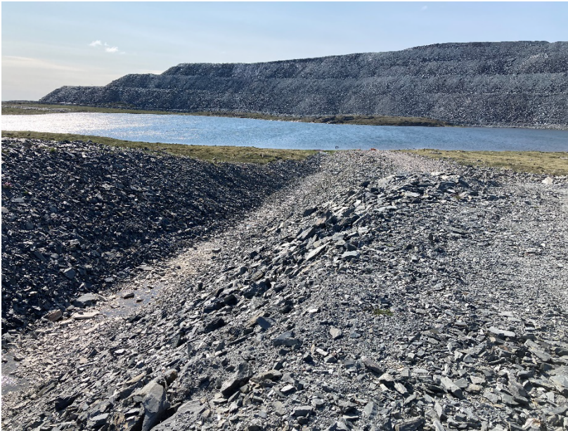
Photograph H2-3 Diversion Ditch and its Sediment and Erosion Protection Structure
