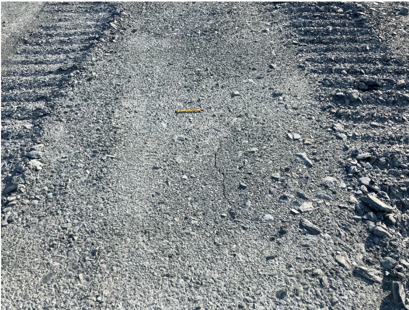
Photograph A3-38 Bay Goose Dike
