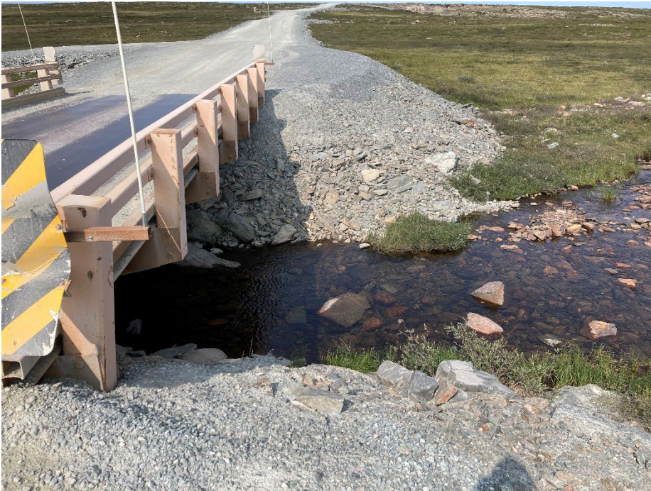
Photograph D3-7 Bridges 4 – R09 km 48+500
