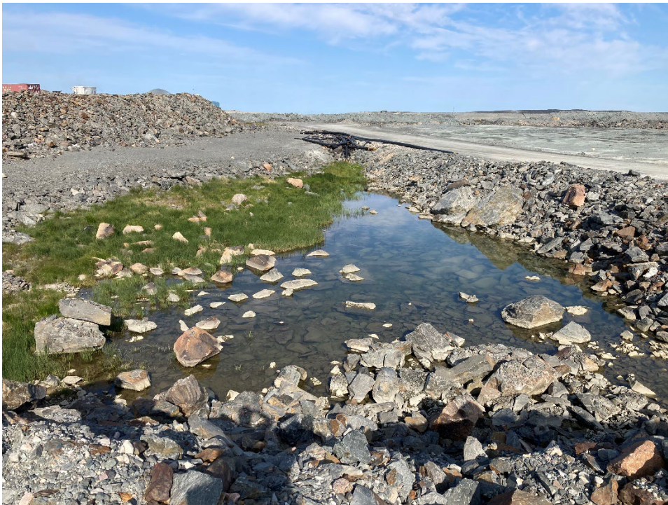
Photograph A1-14 East Dike
