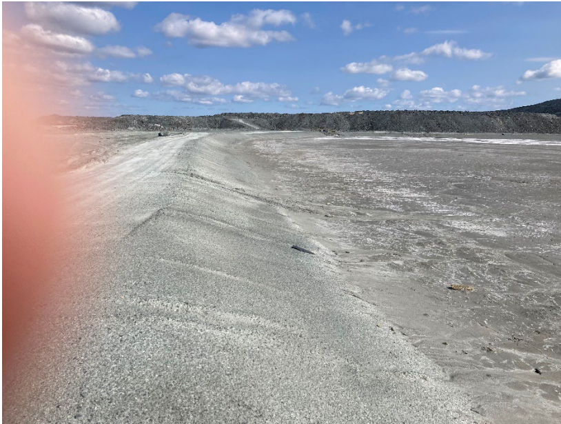
Photograph B1-5 Tailings Storage Facility
