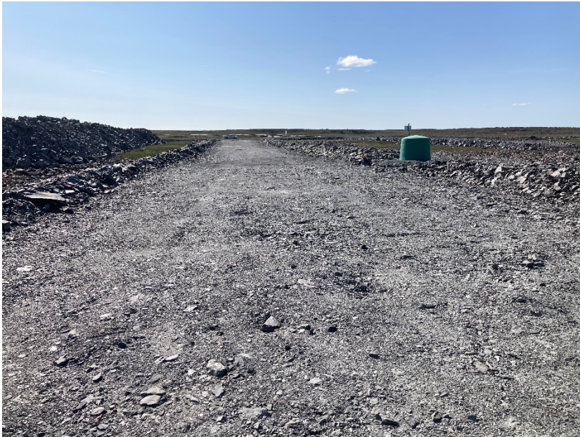
Photograph A8-3 Mammoth Dike
