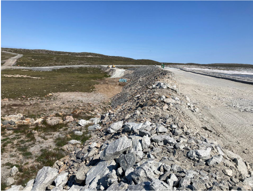
Photograph B2-1 Saddle Dam 1
