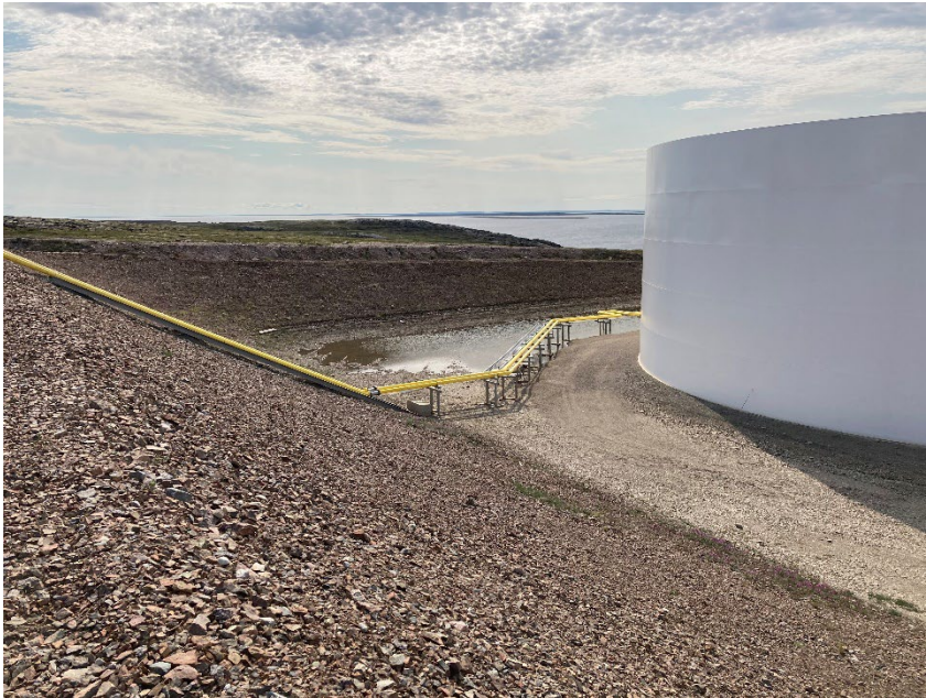
Photograph G1-17 Baker Lake Tank Farm
