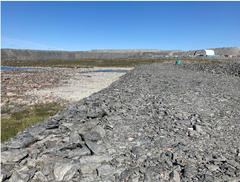
Photograph A8-8 Mammoth Dike
