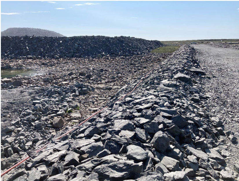
Photograph A8-4 Mammoth Dike
