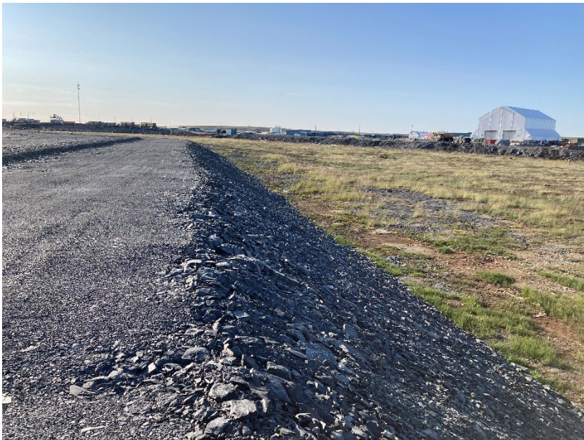
Photograph A6-10 IVR Dike D-1
