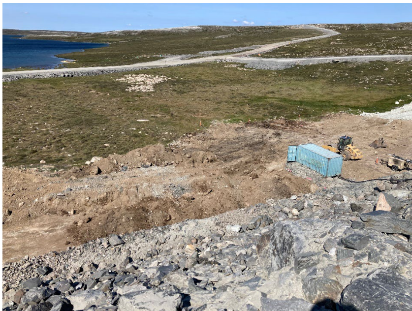
Photograph B2-2 Saddle Dam 1
