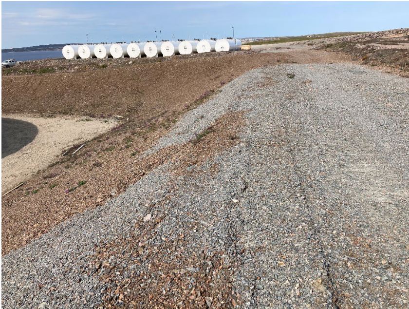
Photograph G1-18 Baker Lake Tank Farm
