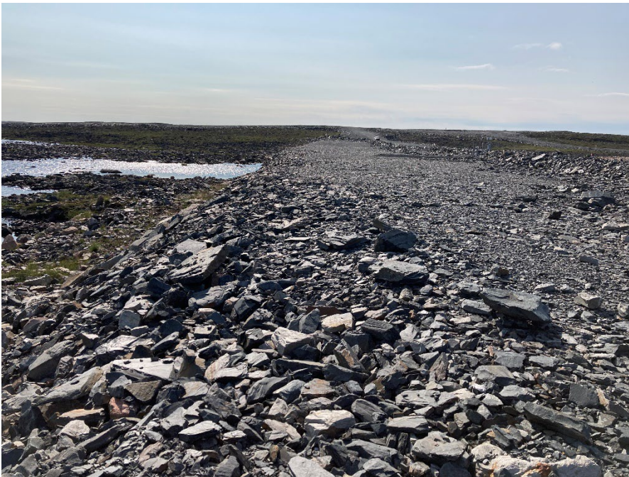
Photograph A4-4 Vault Dike
