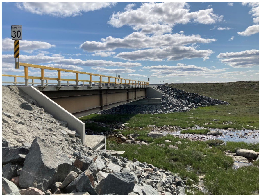
Photograph E2-19 Bridges 9 – km 160+800
