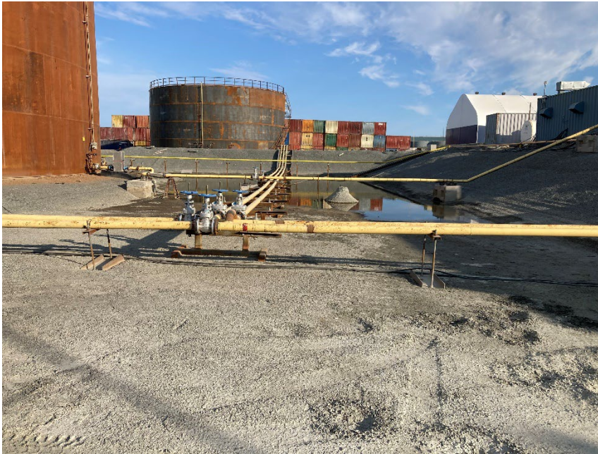
Photograph G2-5 Meadowbank Tank Farm
