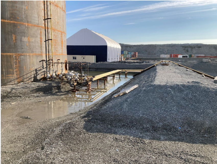
Photograph G2-7 Meadowbank Tank Farm
