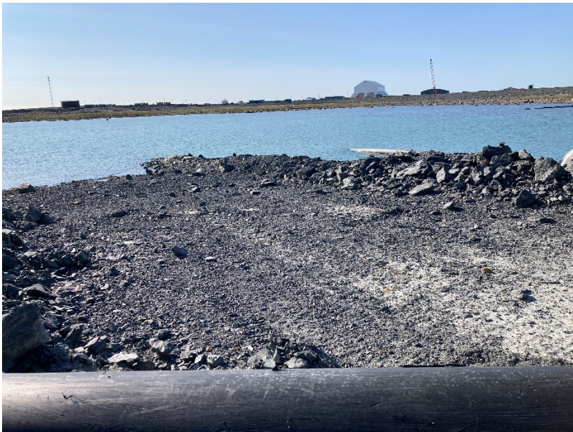
Photograph H8-2 IVR Attenuation Pond Jetty
