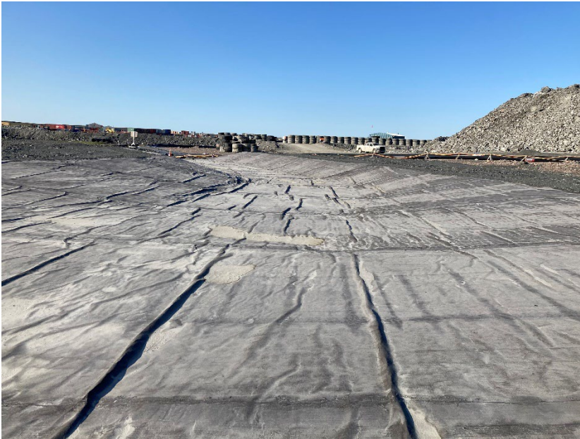
Photograph A6-13 IVR Dike D-1
