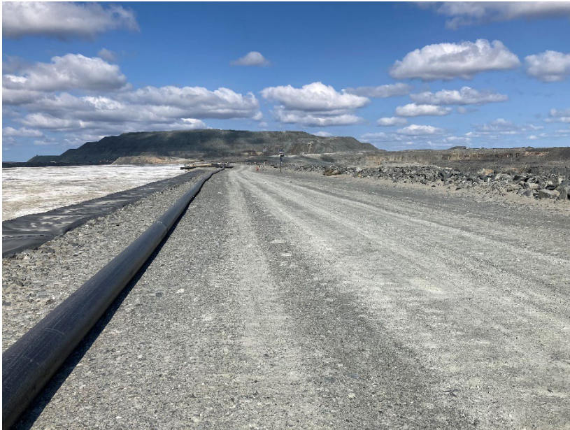
Photograph B7-9 Central Dike and Saddle Dam 5
