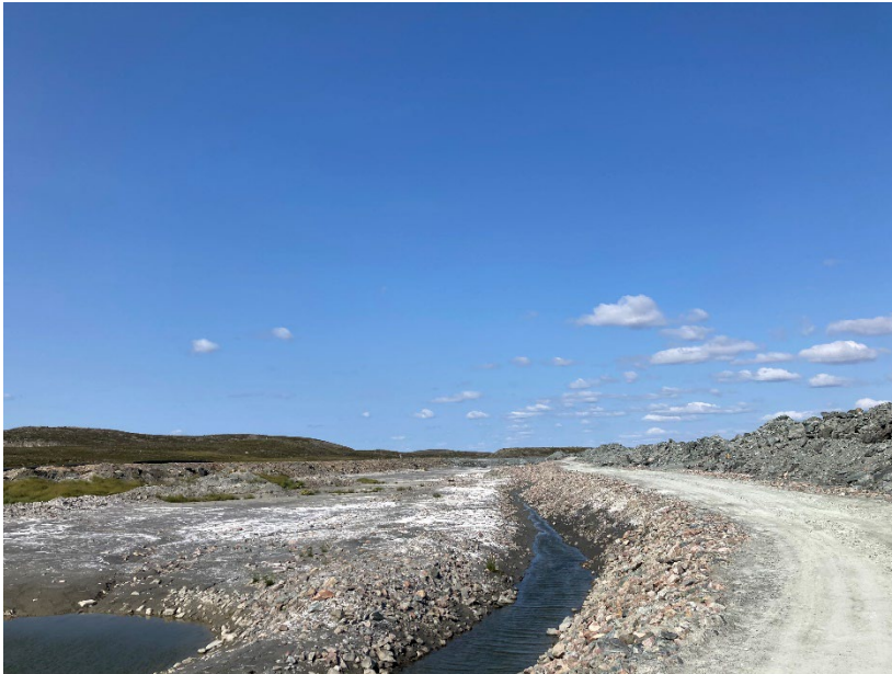
Photograph B1-3 Tailings Storage Facility
