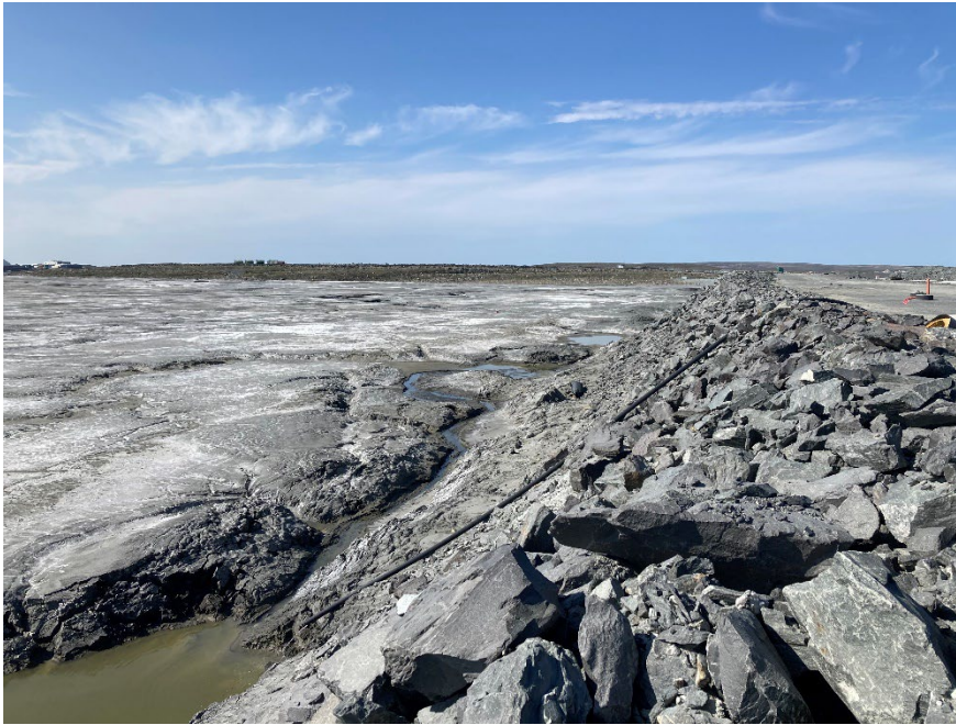
Photograph B4-3 Stormwater Dike
