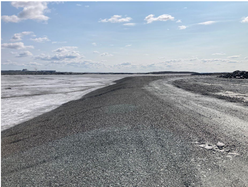
Photograph B1-2 Tailings Storage Facility
