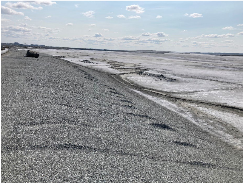
Photograph B1-9 Tailings Storage Facility
