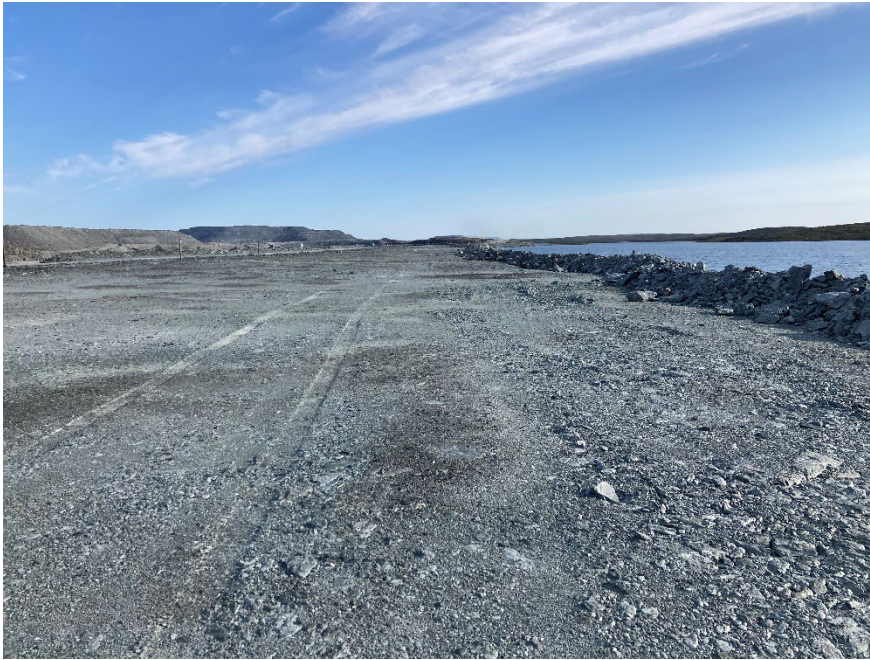
Photograph A3-13 Bay Goose Dike
