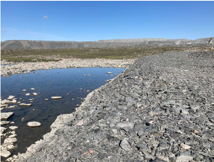
Photograph A8-6 Mammoth Dike
