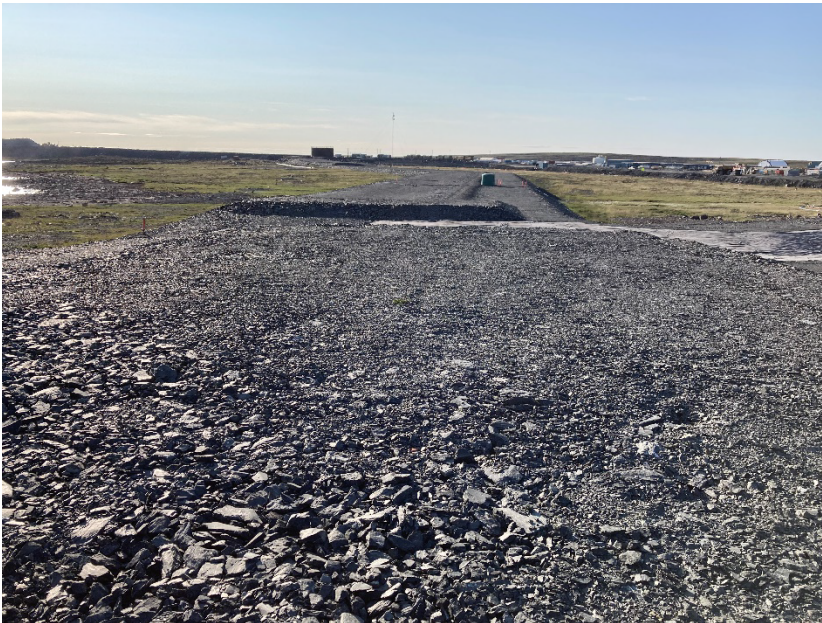
Photograph A6-14 IVR Dike D-1
