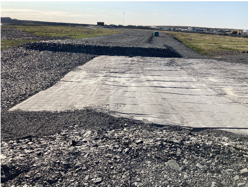
Photograph A6-16 IVR Dike D-1
