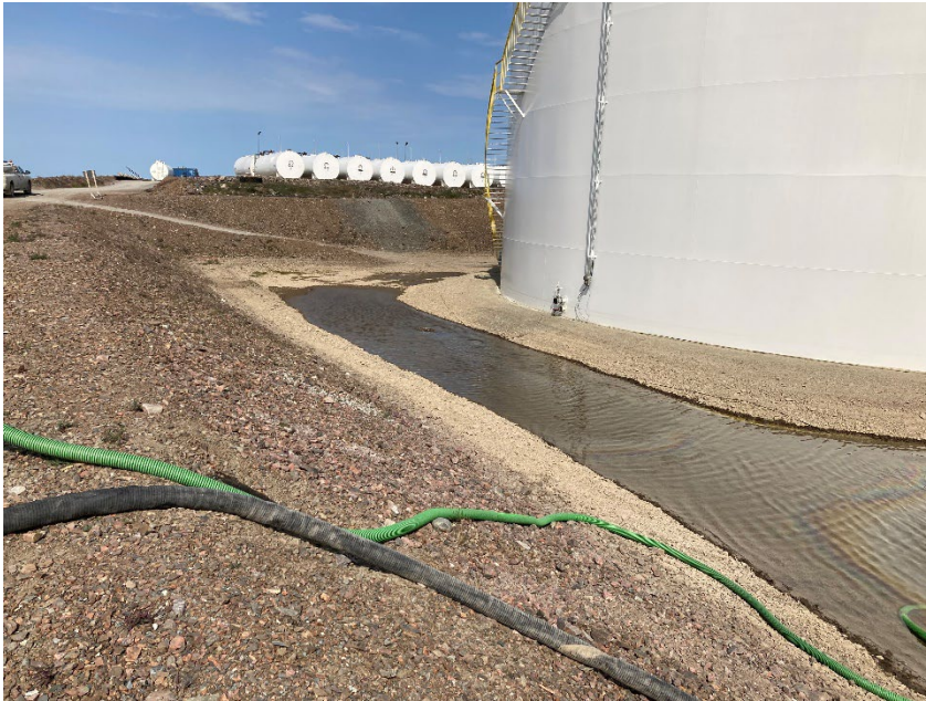
Photograph G1-13 Baker Lake Tank Farm
