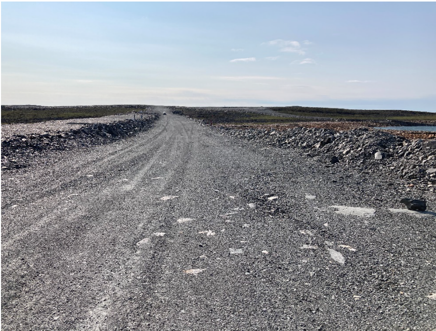
Photograph A4-3 Vault Dike
