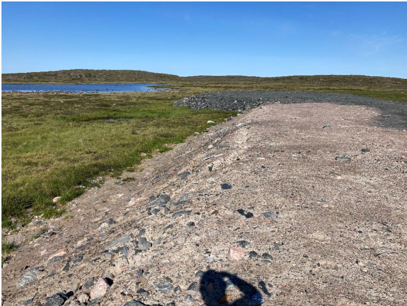
Photograph H13-8 IVR Diversion Channel
