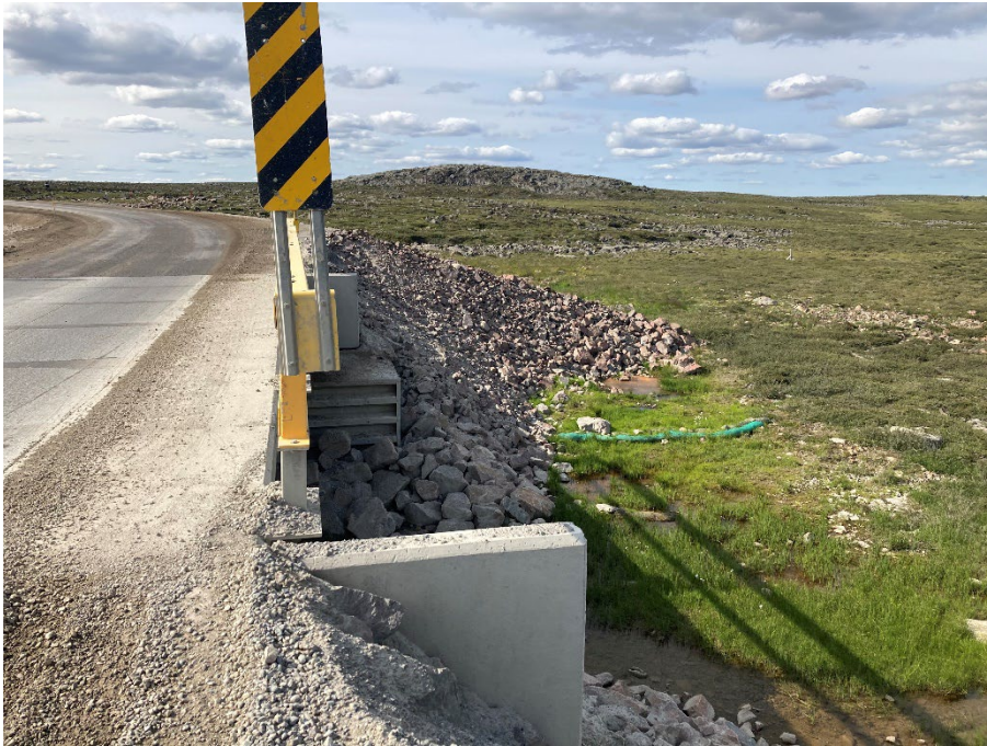
Photograph E2-9 Bridges 4 – km 136+000
