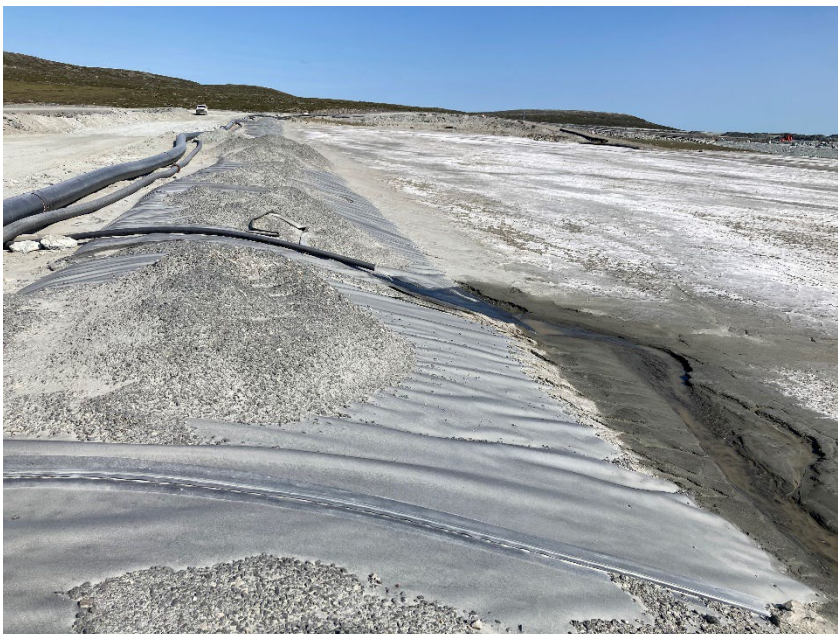
Photograph B2-6 Saddle Dam 1
