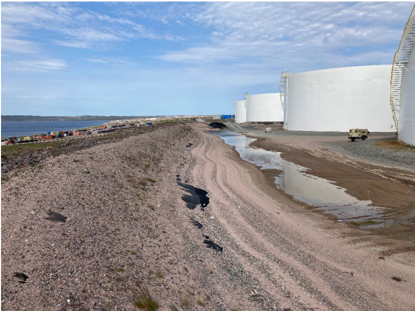
Photograph G1-8 Baker Lake Tank Farm
