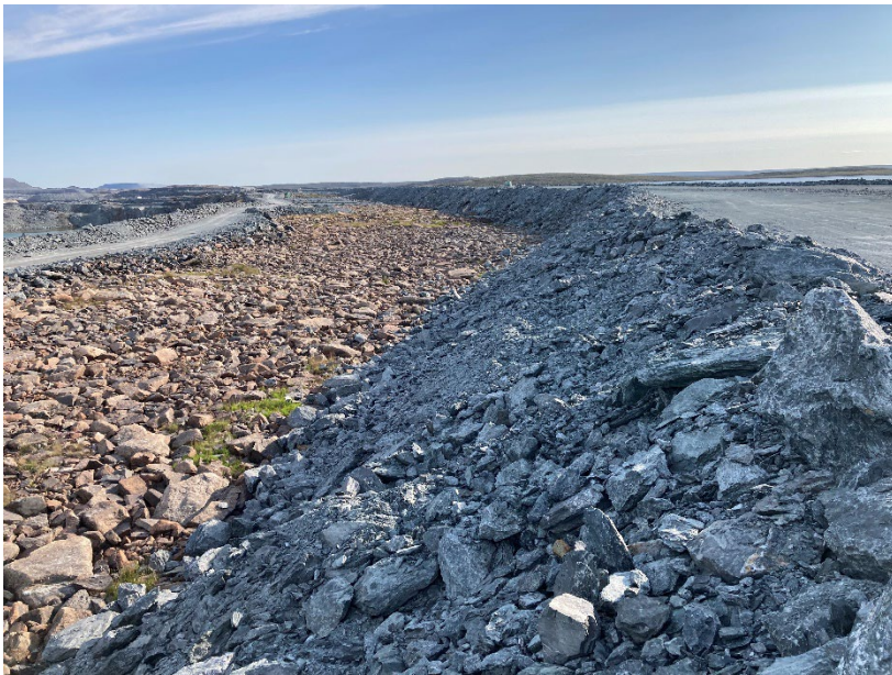
Photograph A3-20 Bay Goose Dike
