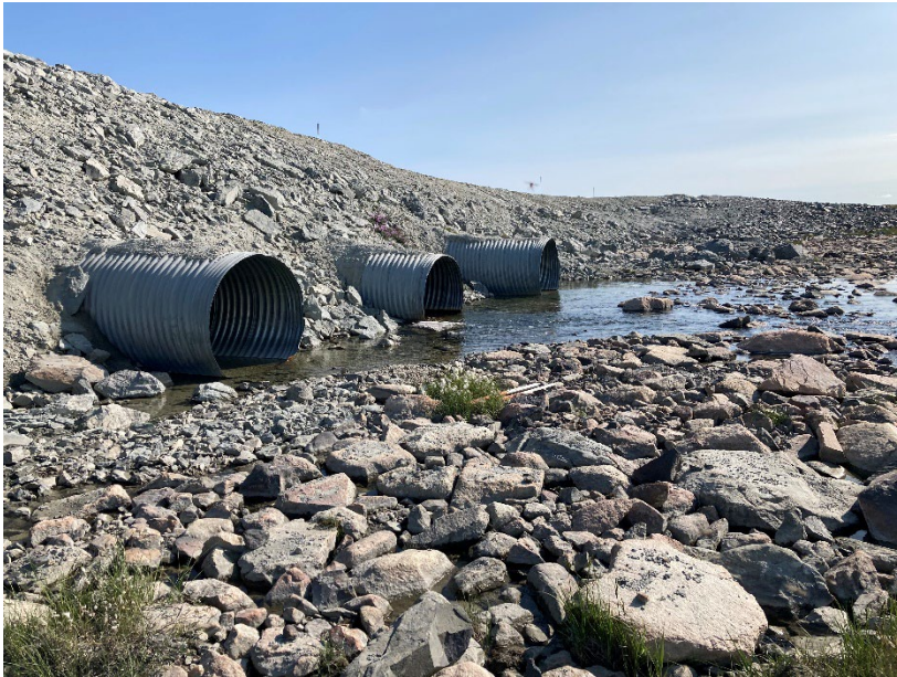
Photograph H1-1 Vault Road Culverts
