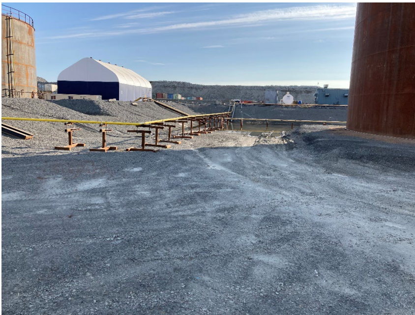
Photograph G2-2 Meadowbank Tank Farm
