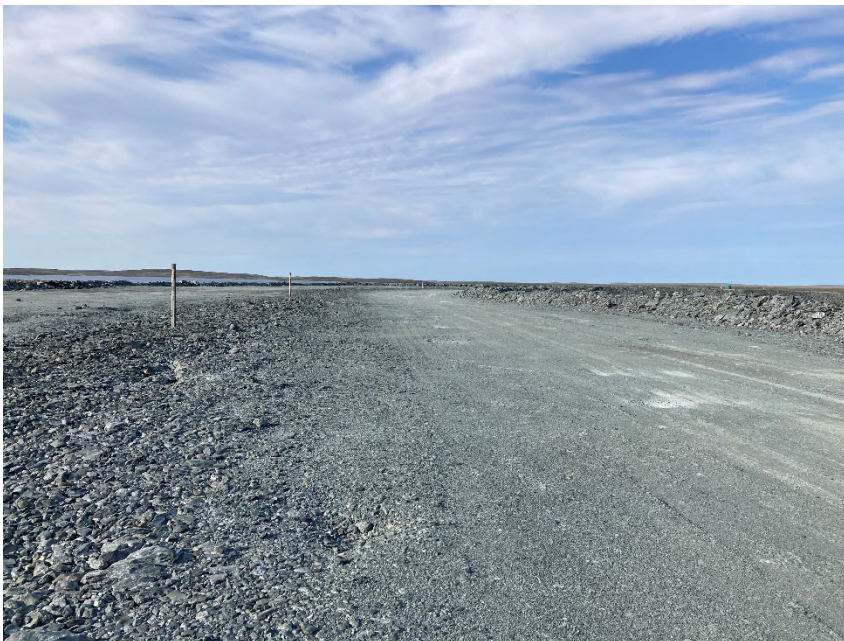
Photograph A3-16 Bay Goose Dike
