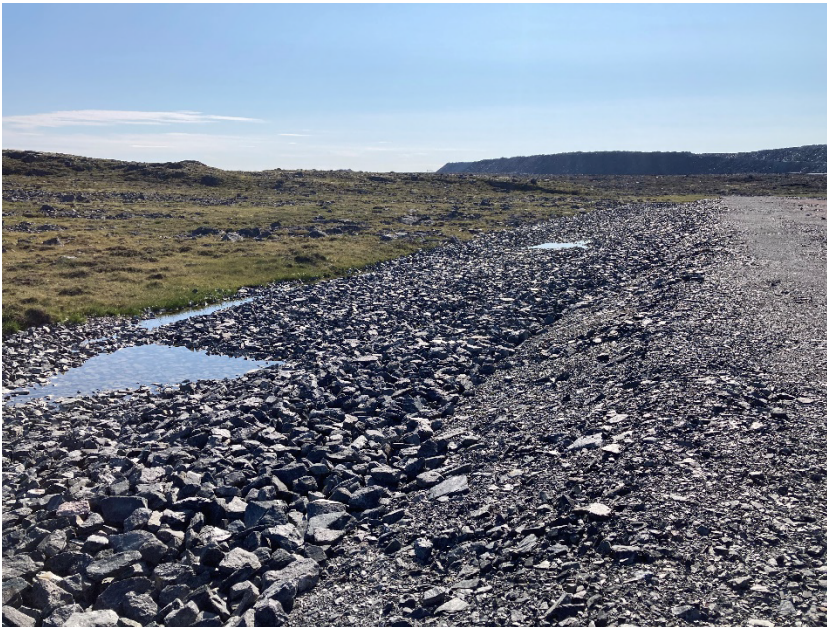
Photograph H13-6 IVR Diversion Channel
