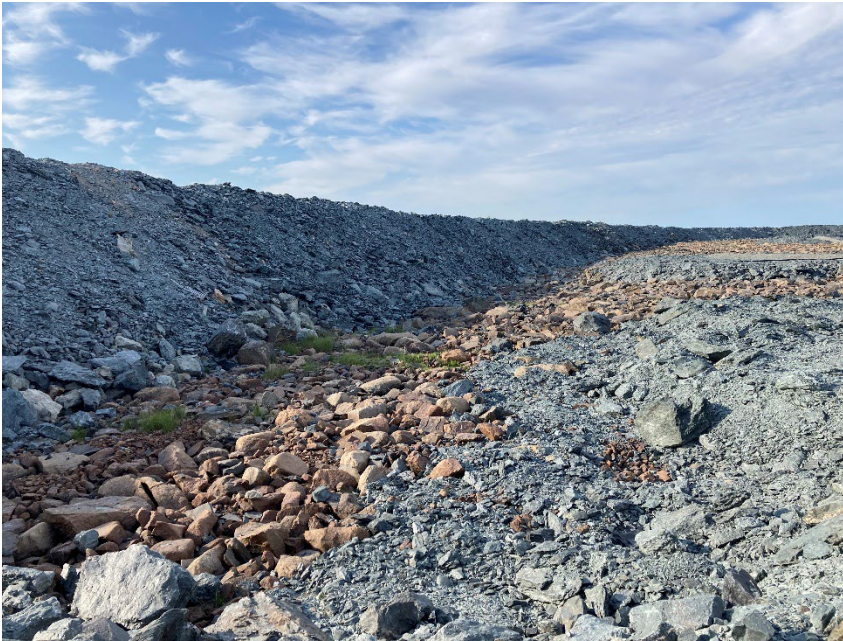
Photograph A3-11 Bay Goose Dike
