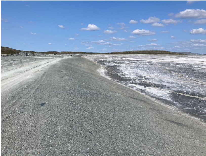
Photograph B1-1 Tailings Storage Facility
