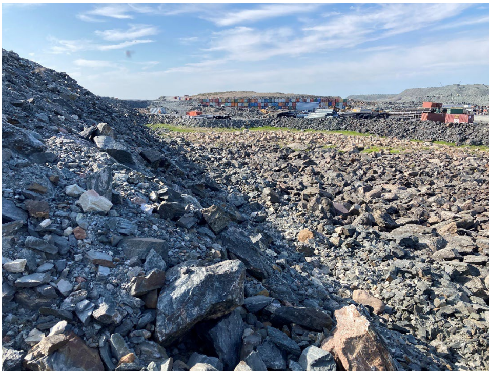
Photograph A1-12 East Dike
