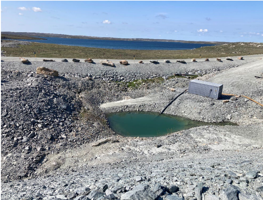
Photograph B5-5 Saddle Dam 3
