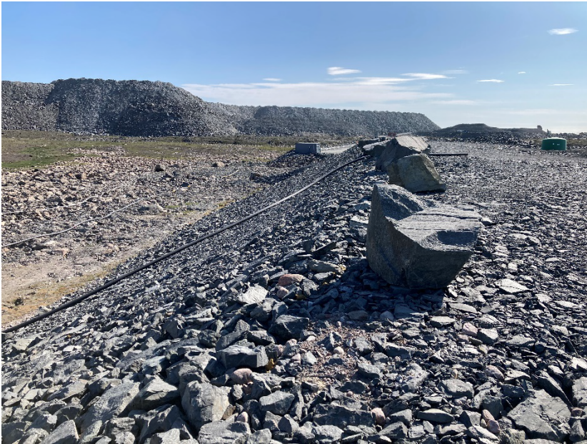
Photograph A7-7 WRSF Dike
