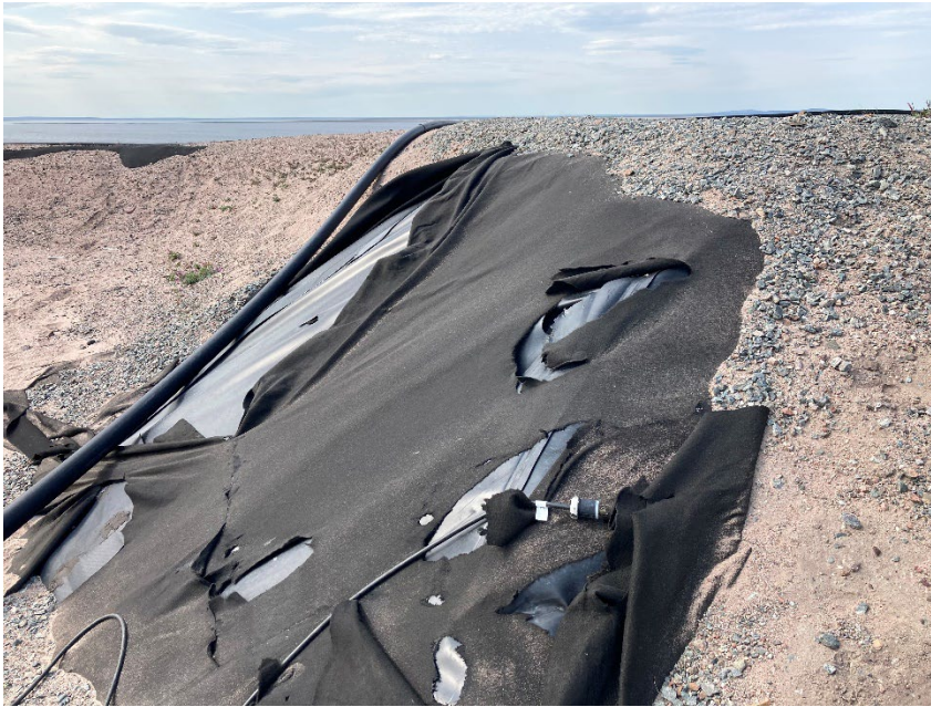
Photograph G1-5 Baker Lake Tank Farm
