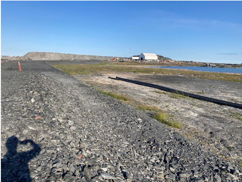
Photograph A6-3 IVR Dike D-1
