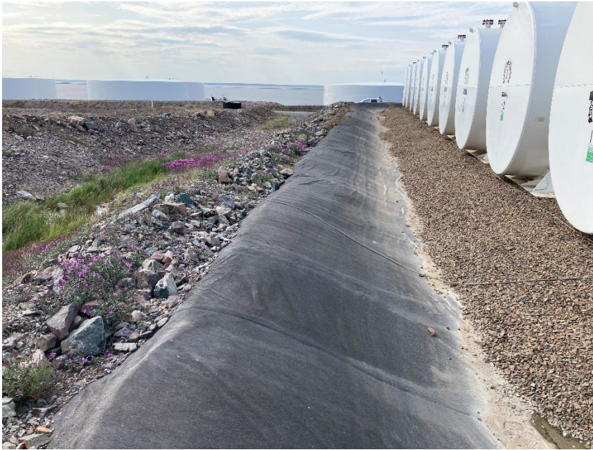
Photograph G1-25 Baker Lake Tank Farm
