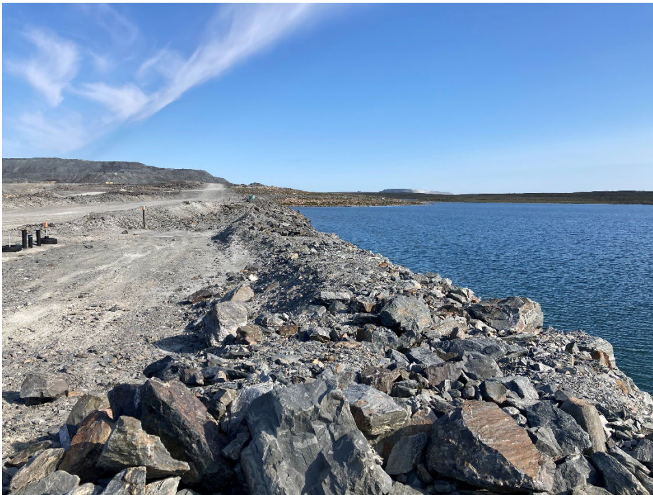
Photograph A1-4 East Dike
