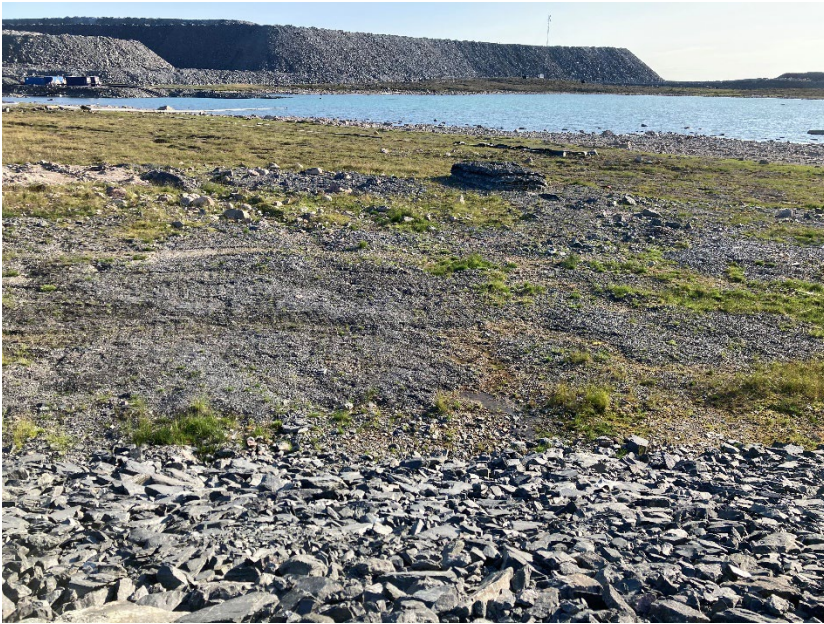
Photograph A6-11 IVR Dike D-1
