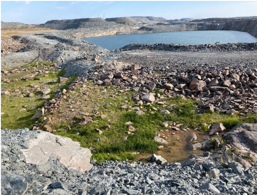
Photograph A3-22 Bay Goose Dike
