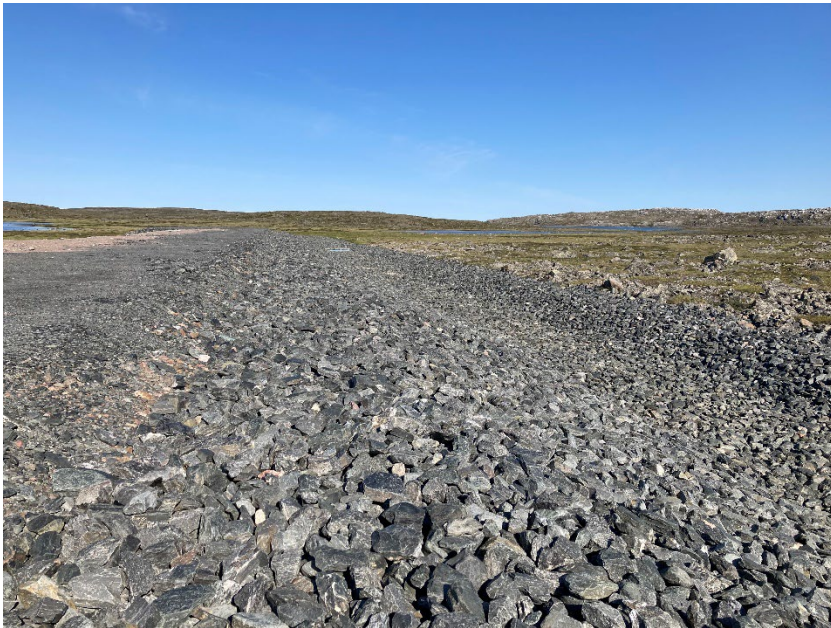
Photograph H13-4 IVR Diversion Channel
