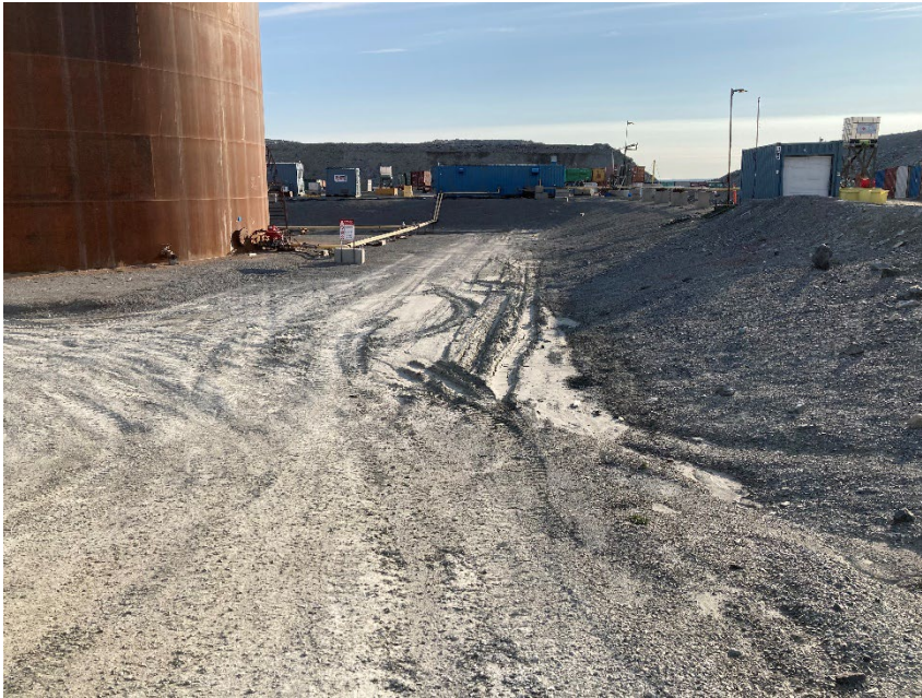
Photograph G2-3 Meadowbank Tank Farm
