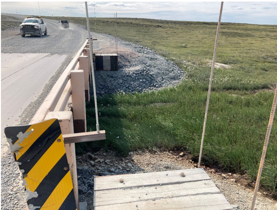
Photograph D3-10 Bridges 5 – R13 km 62+060
