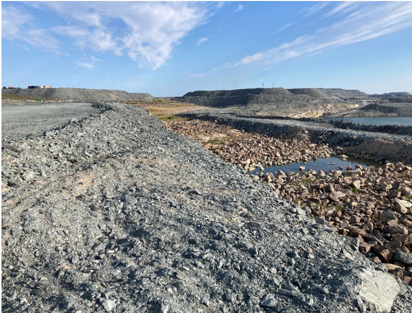
Photograph A3-27 Bay Goose Dike
