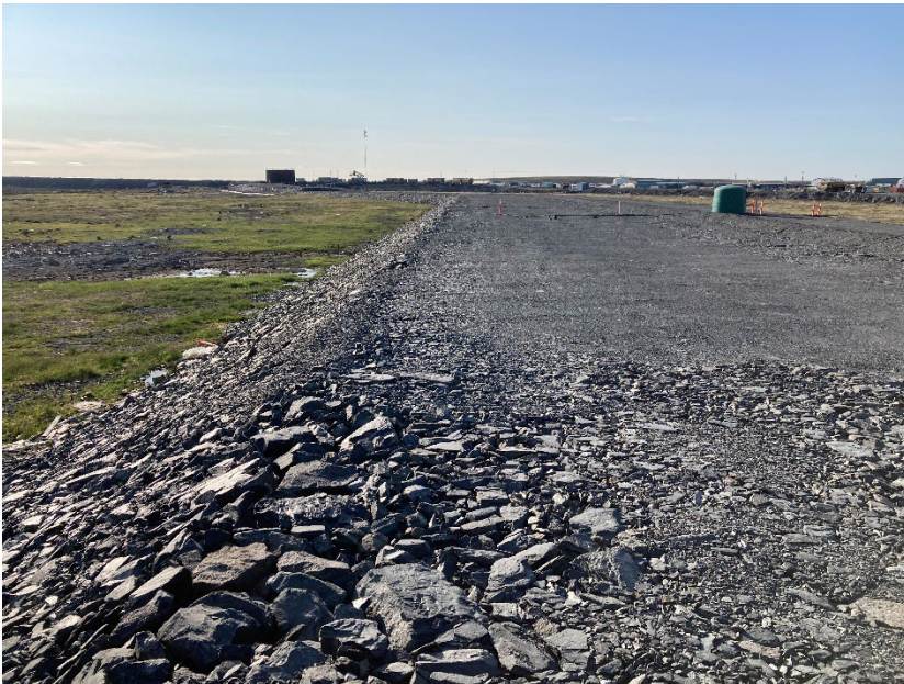
Photograph A6-12 IVR Dike D-1
