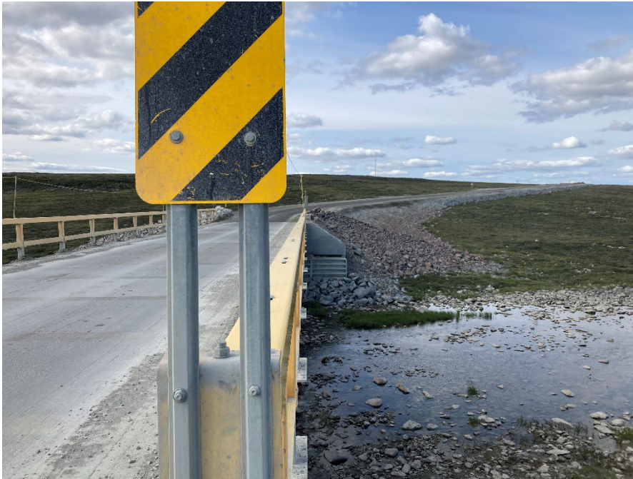
Photograph E2-5 Bridges 3 – km 132+000
