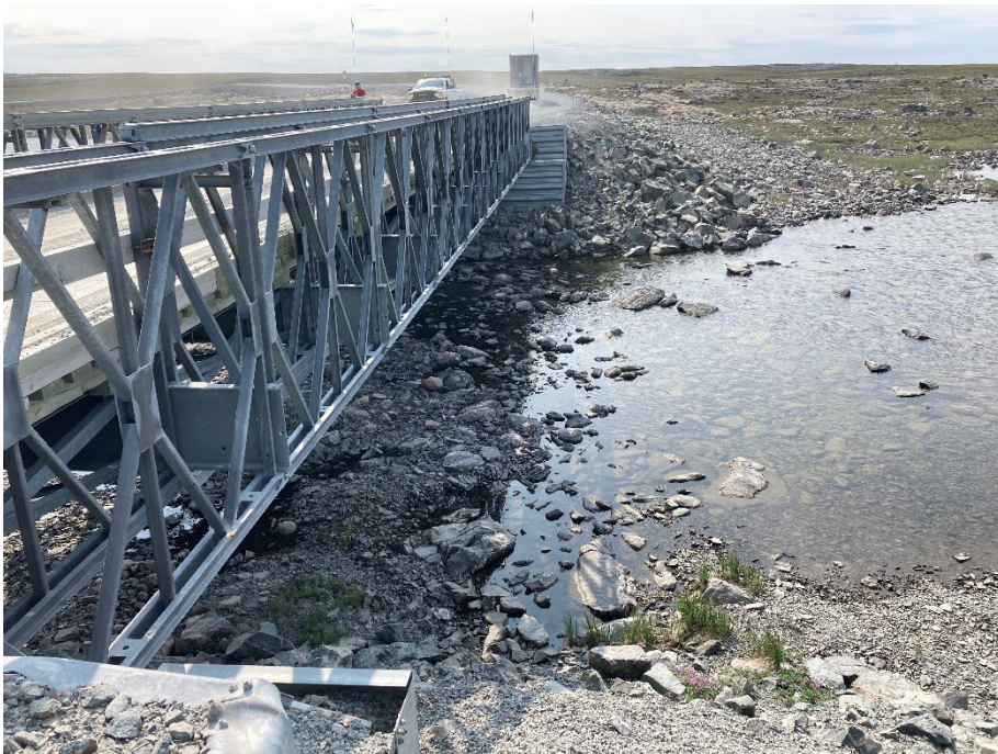
Photograph D3-6 Bridges 3 – R06 km 23+100
