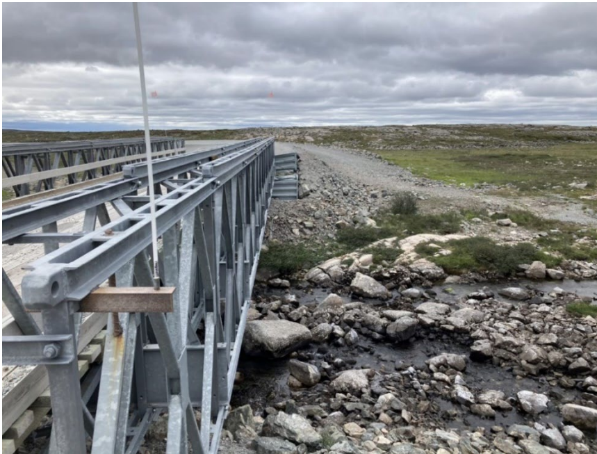
Photograph D3-2 Bridges 1 – R02 km 8+750
