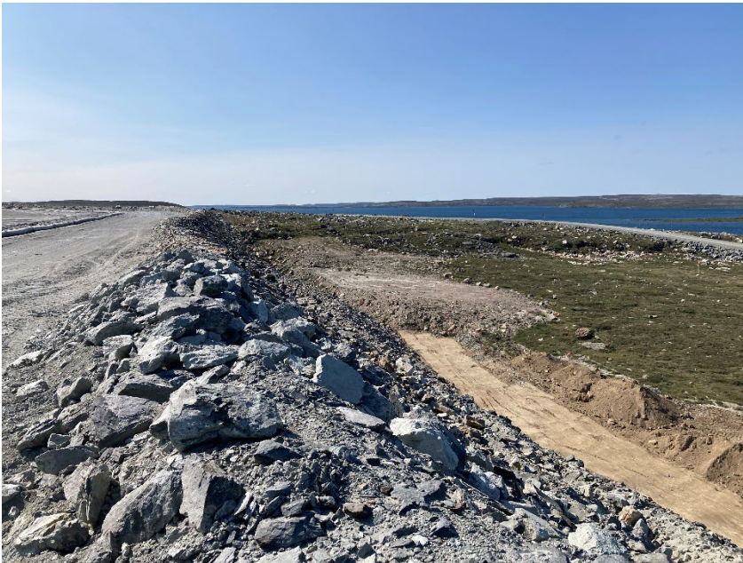
Photograph B2-10 Saddle Dam 1
