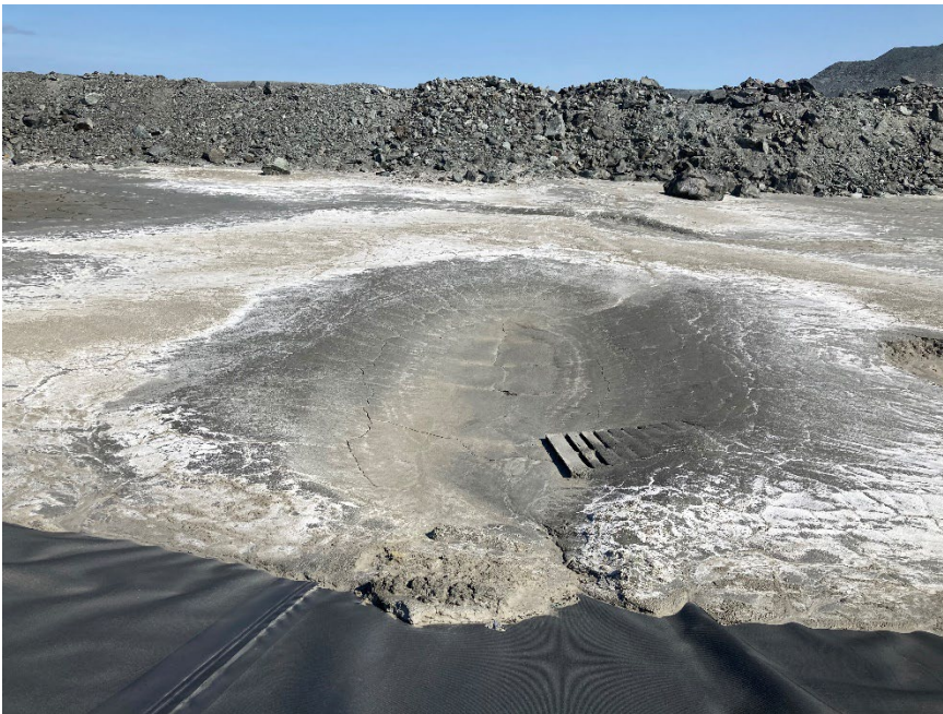
Photograph B3-6 Saddle Dam 2
