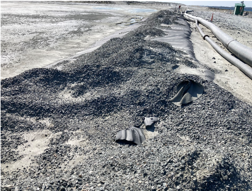
Photograph B2-4 Saddle Dam 1
