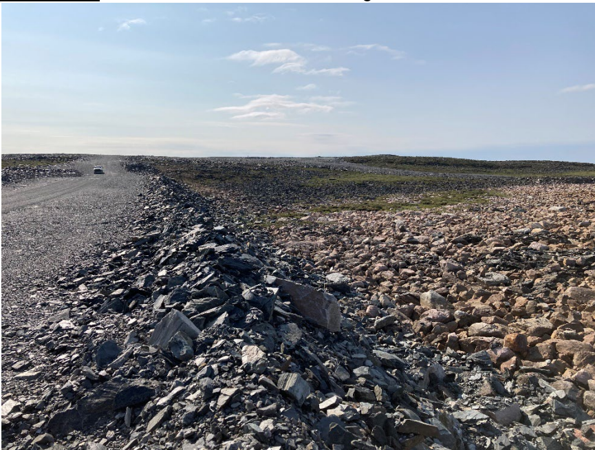
Photograph A4-2 Vault Dike
