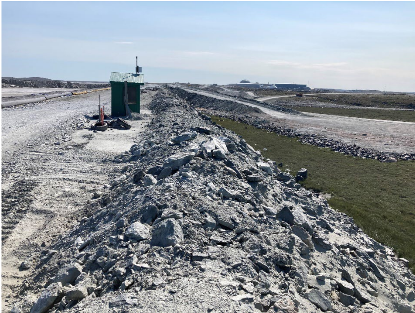
Photograph B3-3 Saddle Dam 2
