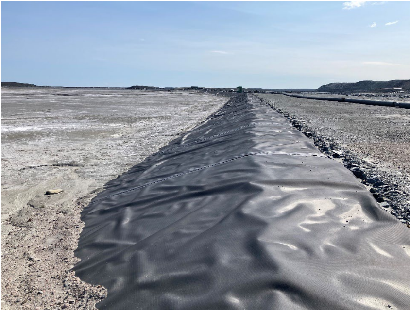
Photograph B6-3 Saddle Dam 4
