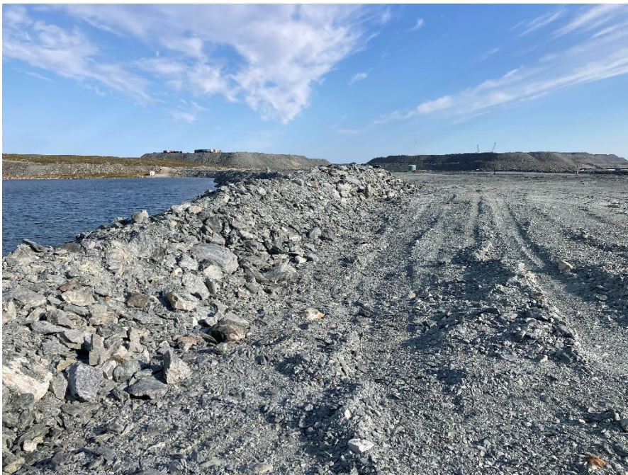
Photograph A3-24 Bay Goose Dike
