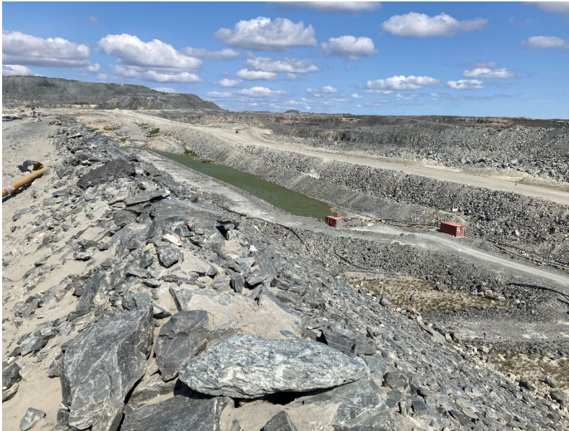
Photograph B7-7 Central Dike and Saddle Dam 5
