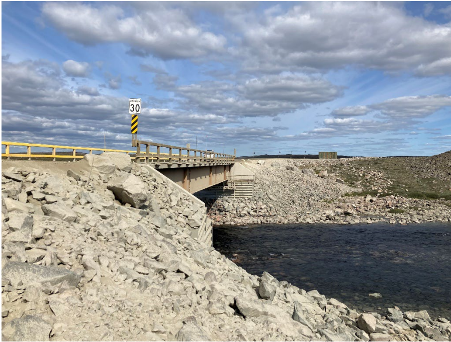
Photograph E2-15 Bridges 7 – km 148+300
