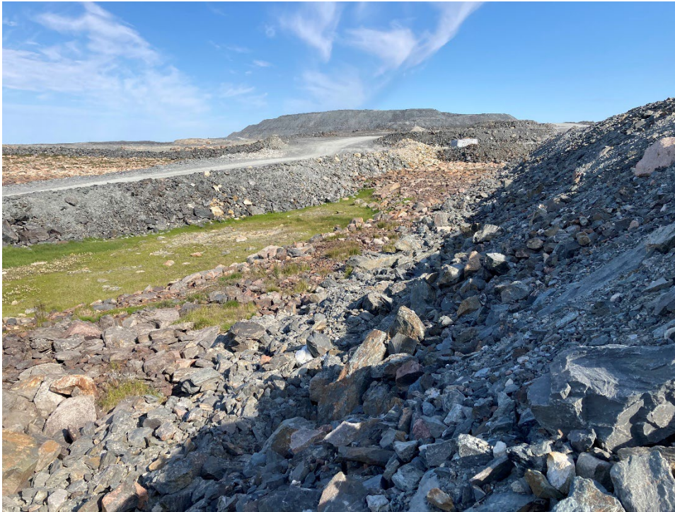
Photograph A1-13 East Dike
