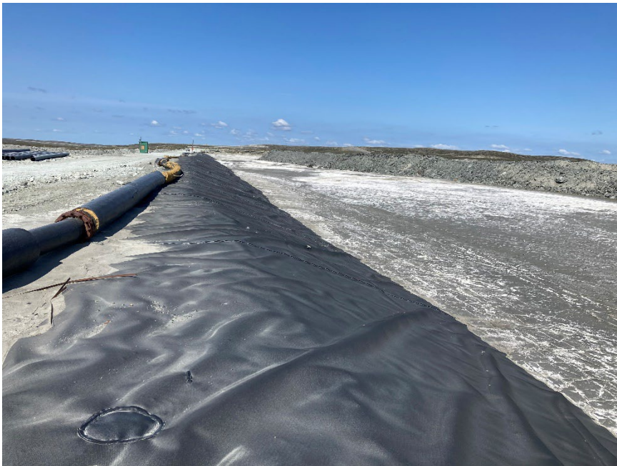
Photograph B3-8 Saddle Dam 2
