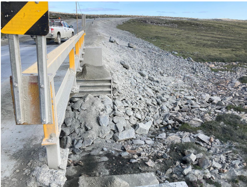
Photograph E2-2 Bridges 1 – km 119+400
