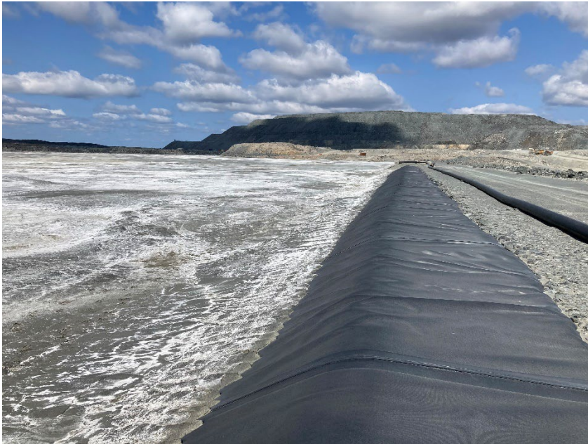
Photograph B7-1 Central Dike and Saddle Dam 5
