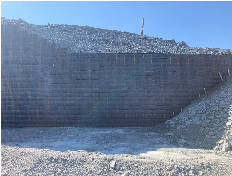
Photograph H6-2 Meadowbank Crusher Retaining Wall
