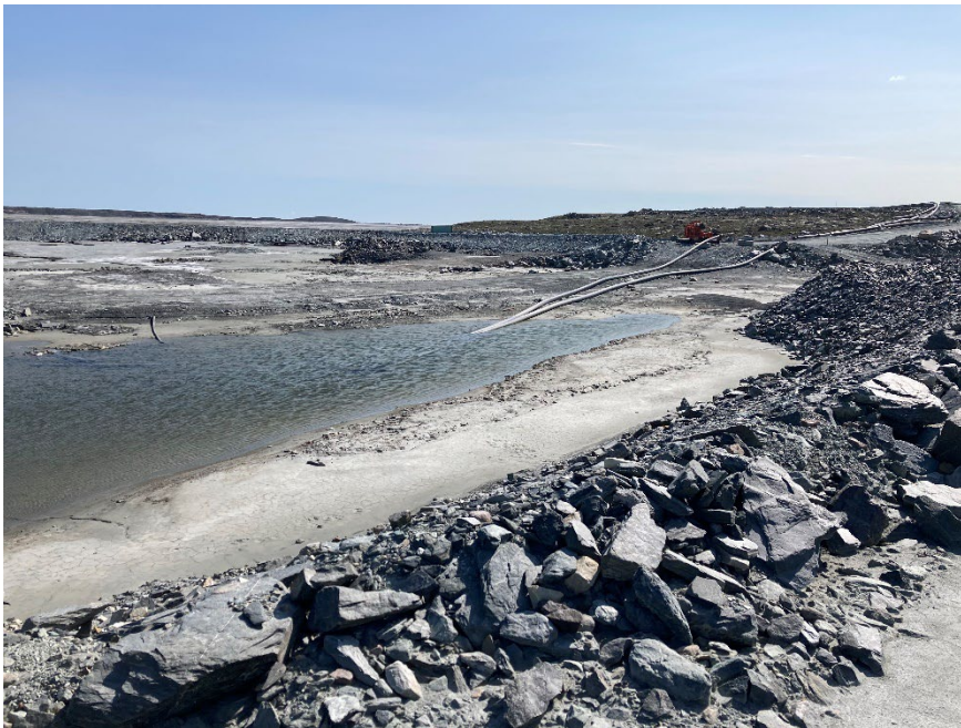
Photograph B5-4 Saddle Dam 3
