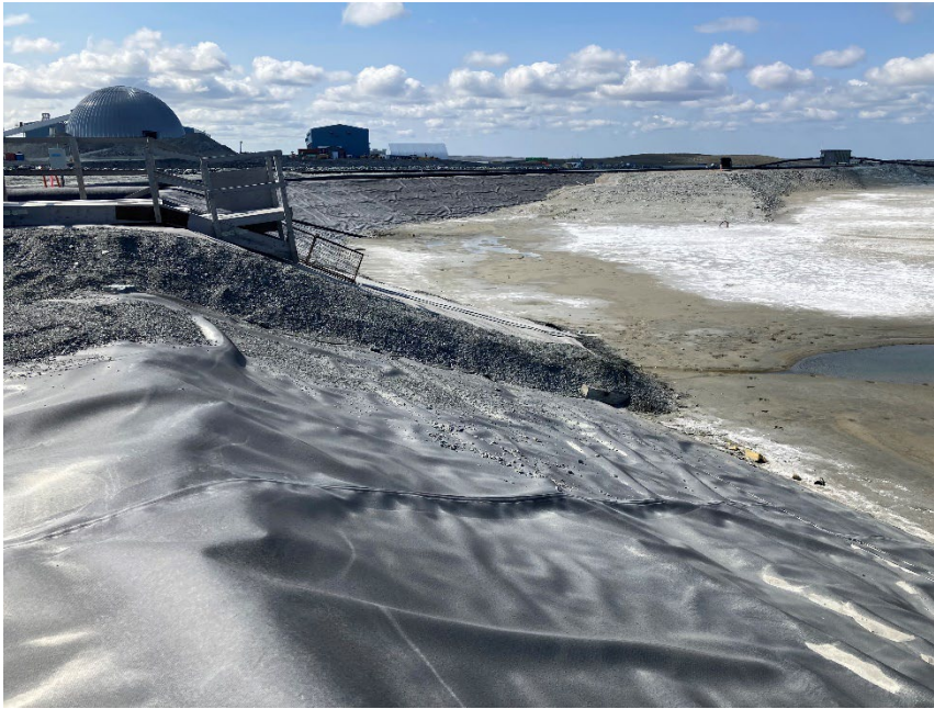
Photograph B7-11 Central Dike and Saddle Dam 5
