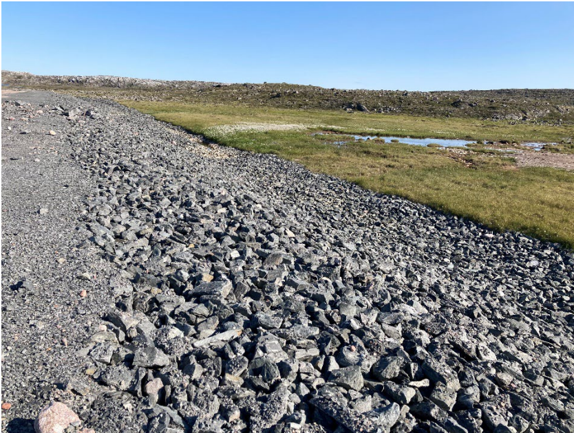
Photograph H13-1 IVR Diversion Channel
