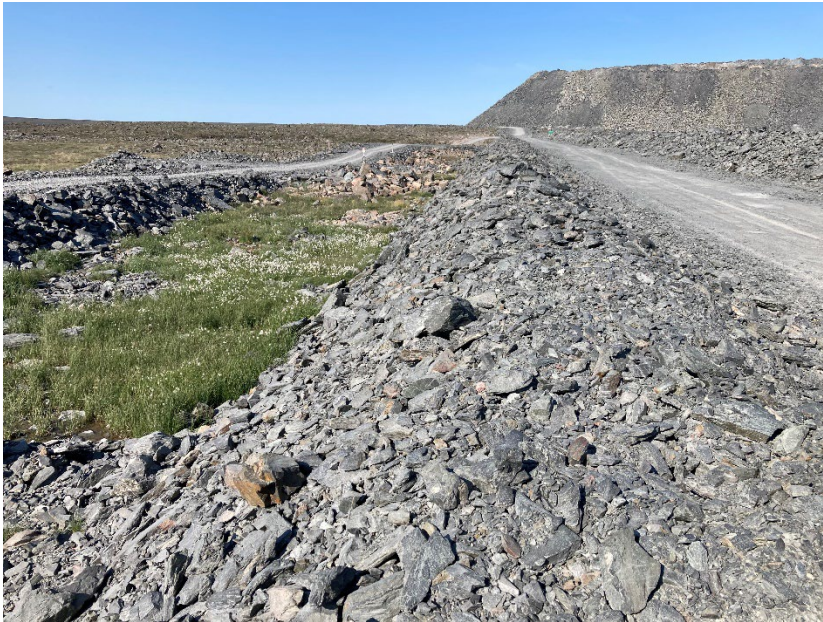
Photograph A7-1 WRSF Dike
