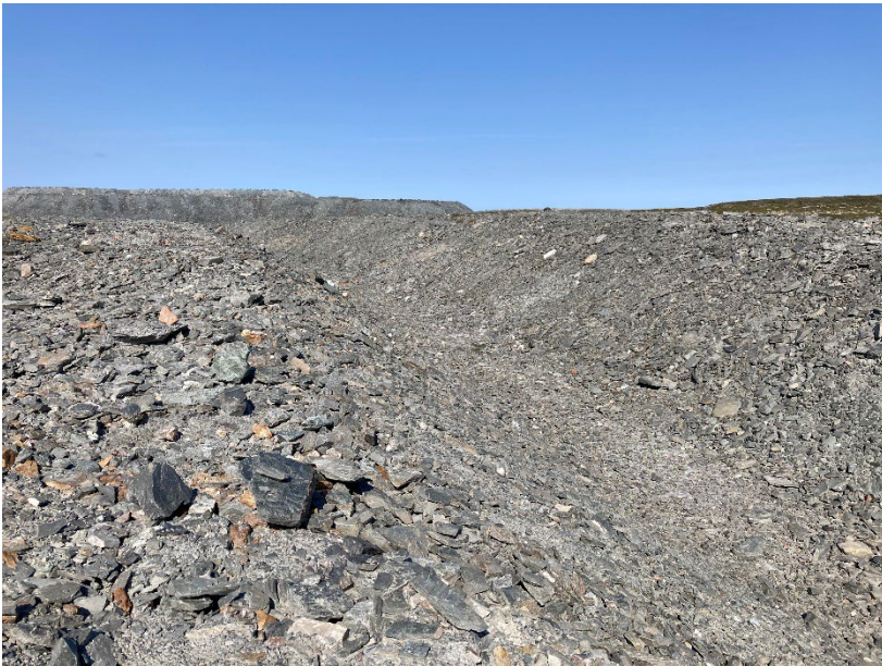
Photograph H2-2 Diversion Ditch and its Sediment and Erosion Protection Structure
