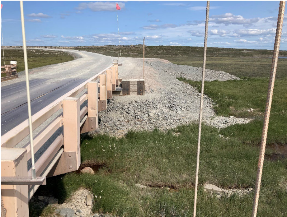
Photograph D3-9 Bridges 5 – R13 km 62+060
