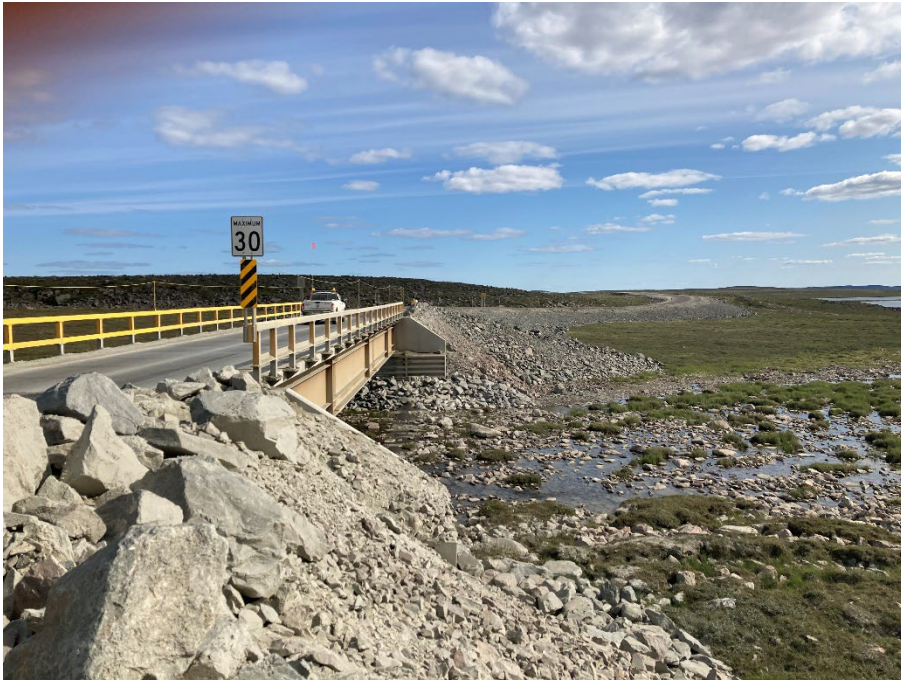
Photograph E2-7 Bridges 3 – km 132+000
