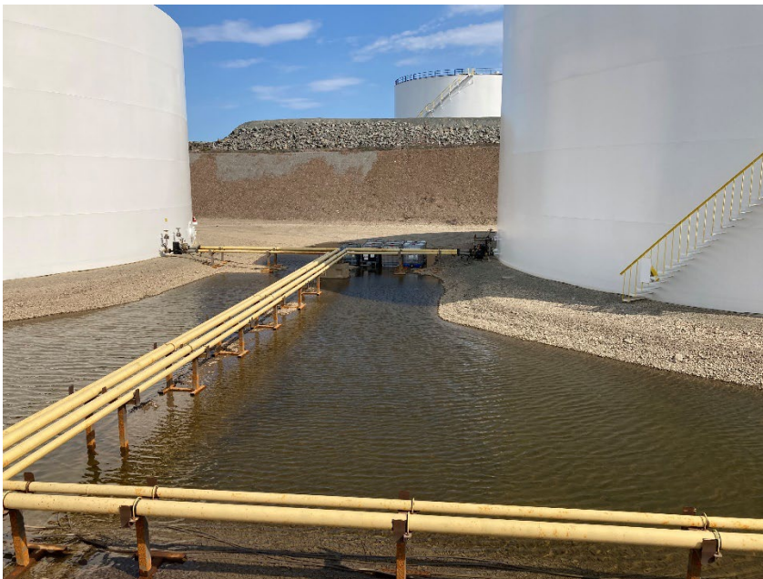
Photograph G1-14 Baker Lake Tank Farm
