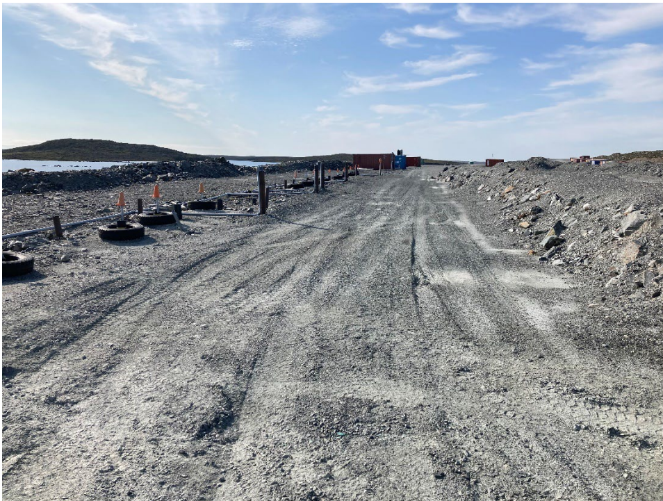
Photograph A1-2 East Dike
