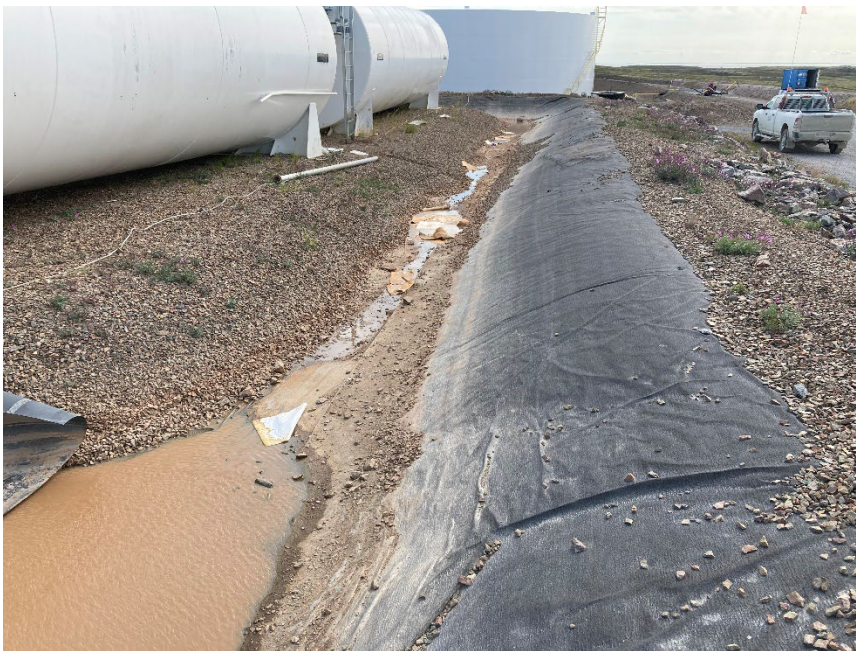
Photograph G1-22 Baker Lake Tank Farm
