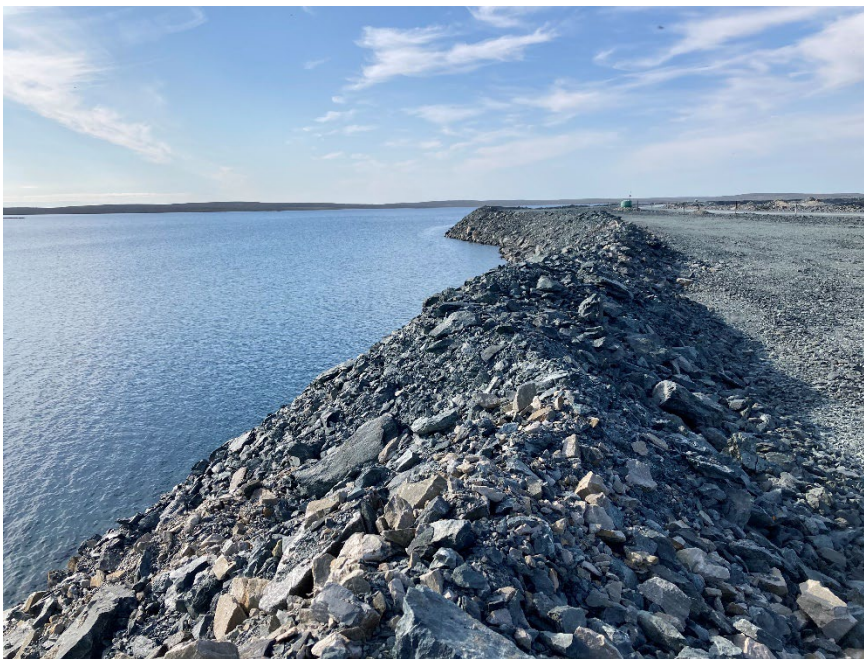
Photograph A3-6 Bay Goose Dike
