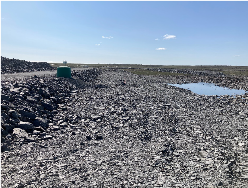
Photograph A8-5 Mammoth Dike
