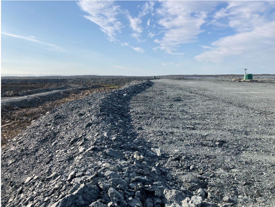
Photograph A3-30 Bay Goose Dike
