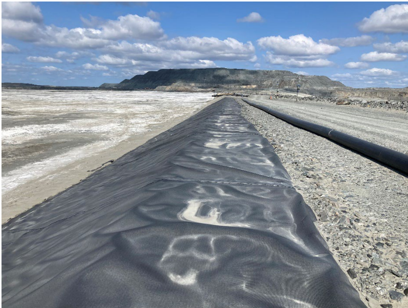
Photograph B7-8 Central Dike and Saddle Dam 5
