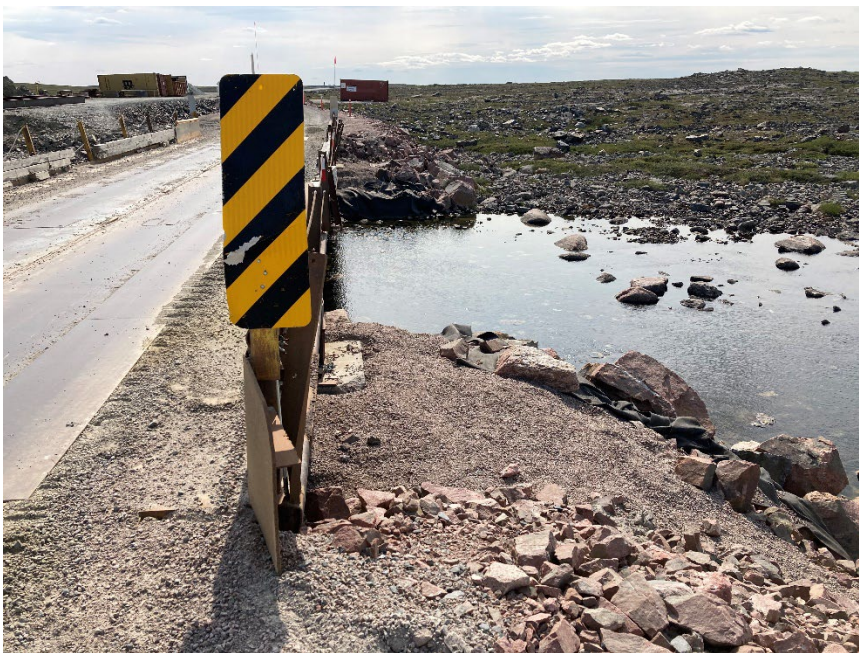
Photograph D3-12 Bridges 6 – R15 km 69+200
