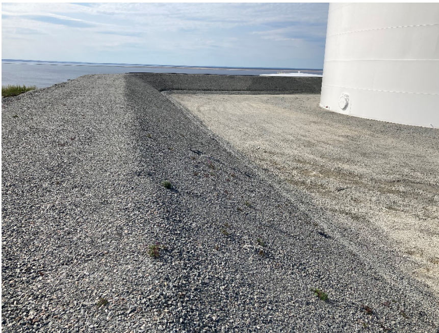
Photograph G1-20 Baker Lake Tank Farm
