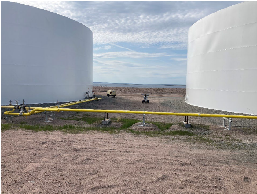
Photograph G1-12 Baker Lake Tank Farm
