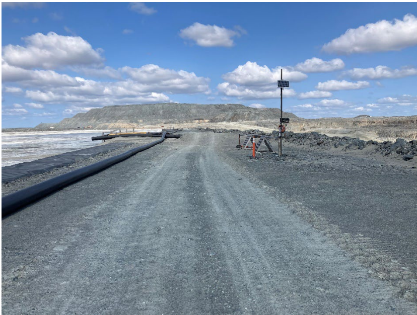
Photograph B7-4 Central Dike and Saddle Dam 5
