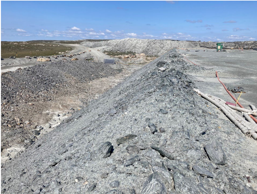
Photograph B5-1 Saddle Dam 3
