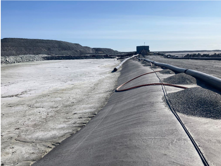
Photograph B4-10 Stormwater Dike
