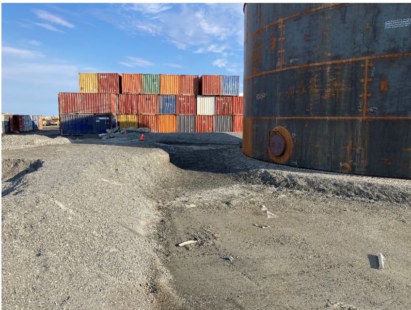
Photograph G2-6 Meadowbank Tank Farm
