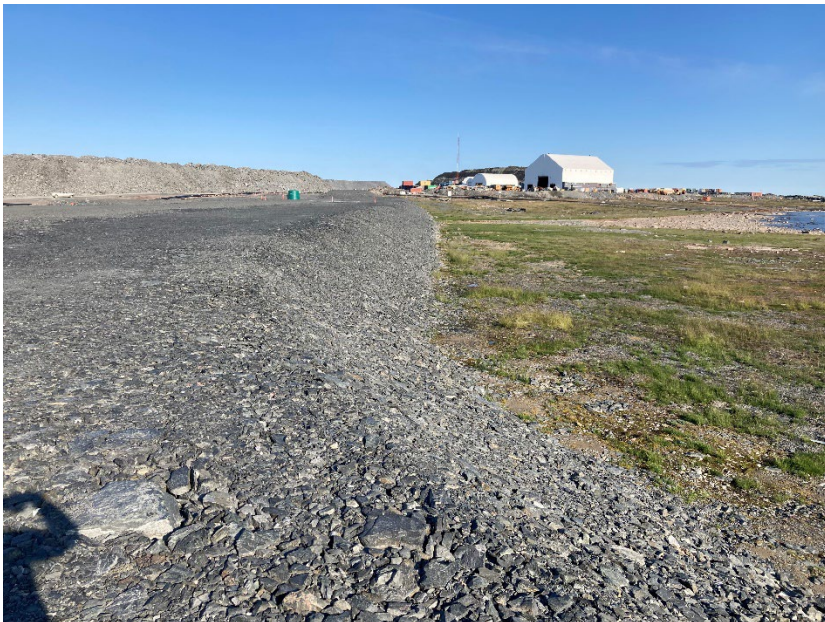
Photograph A6-6 IVR Dike D-1
