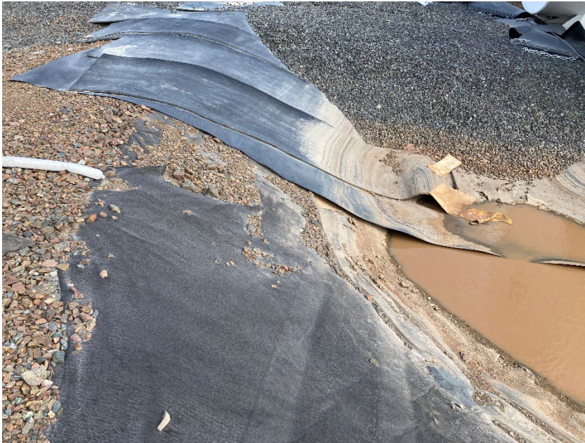
Photograph G1-21 Baker Lake Tank Farm
