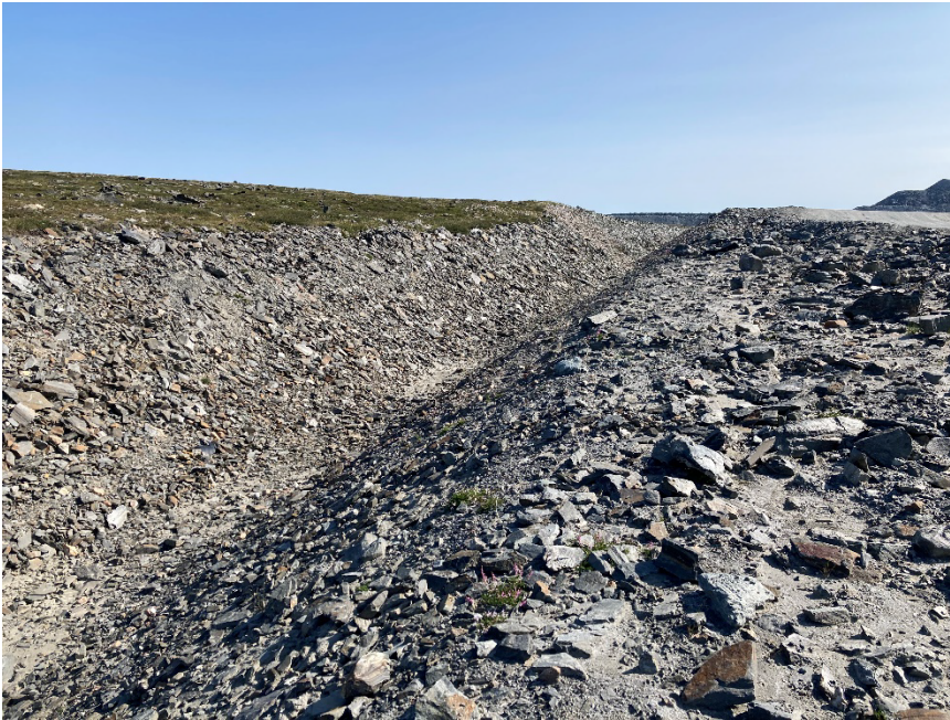
Photograph H2-17 Diversion Ditch and its Sediment and Erosion Protection Structure
