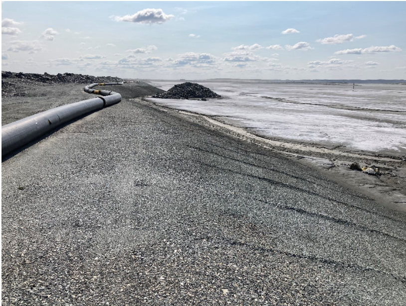
Photograph B1-11 Tailings Storage Facility
