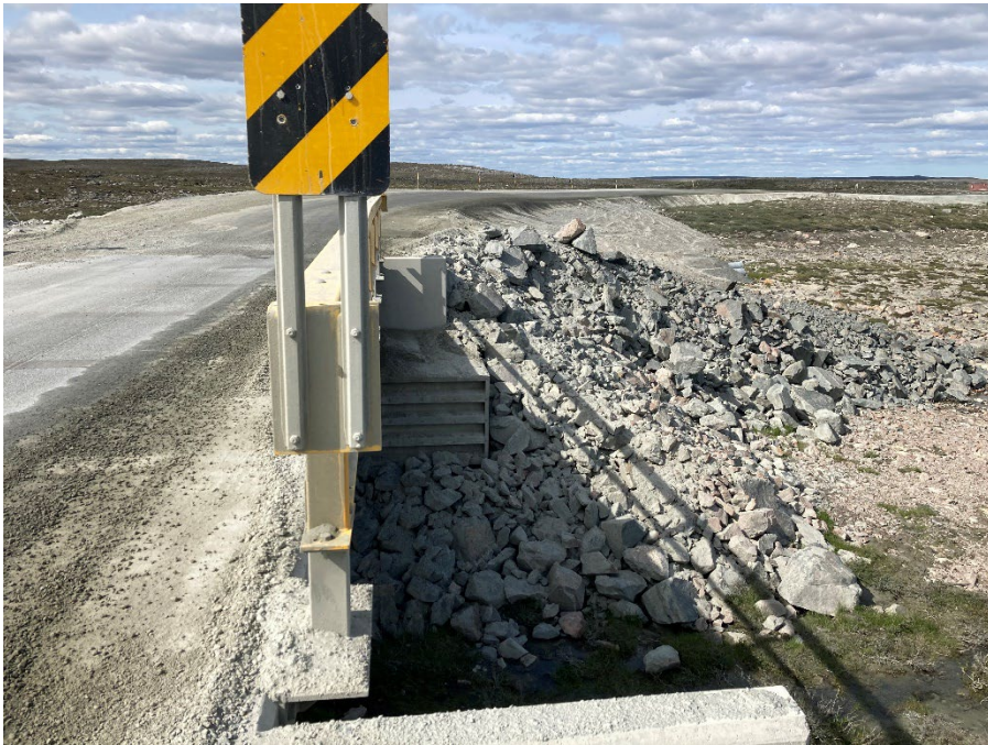
Photograph E2-16 Bridges 8 – km 159+500
