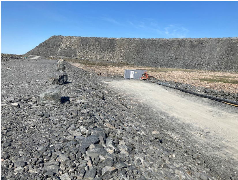
Photograph A7-6 WRSF Dike
