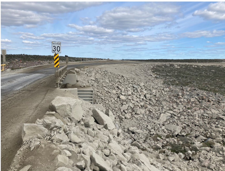
Photograph E2-12 Bridges 6 – km 142+100
