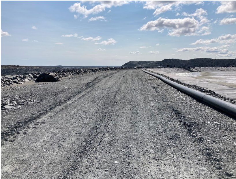
Photograph B7-3 Central Dike and Saddle Dam 5
