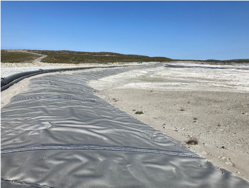
Photograph B2-7 Saddle Dam 1
