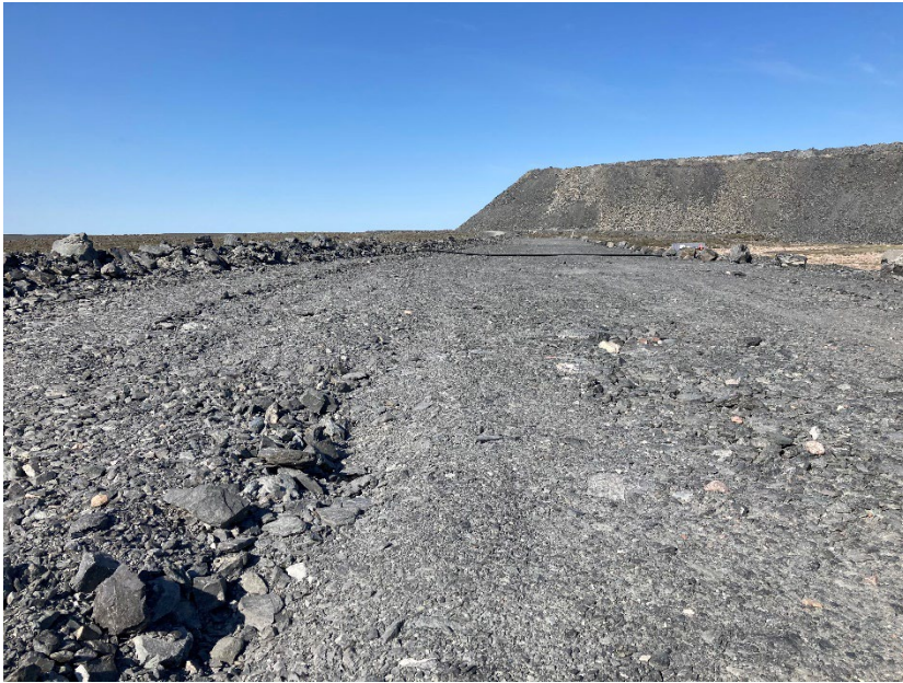
Photograph A7-3 WRSF Dike
