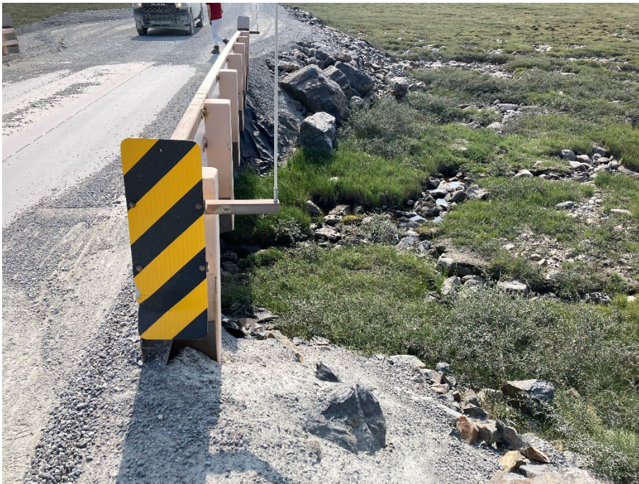
Photograph D3-14 Bridges 7 – R16 km 73+800
