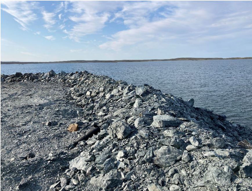
Photograph A3-25 Bay Goose Dike
