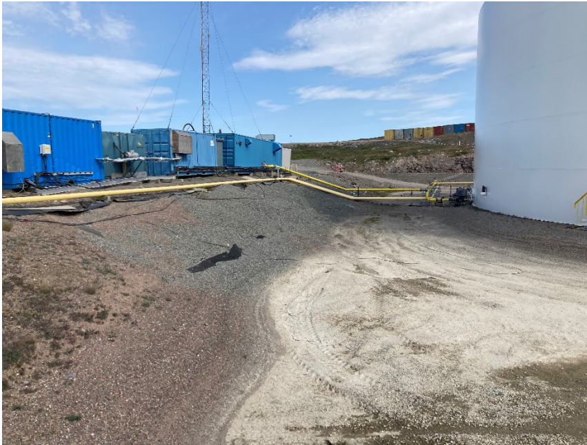
Photograph G1-1 Baker Lake Tank Farm
