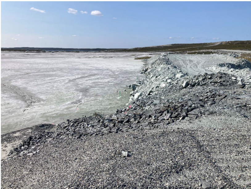
Photograph B1-14 Tailings Storage Facility
