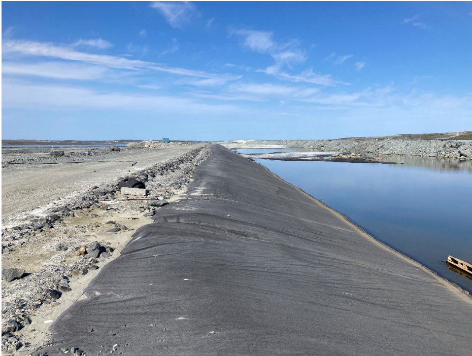
Photograph B4-5 Stormwater Dike
