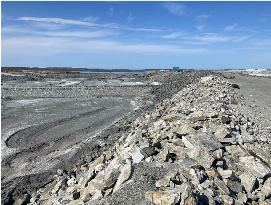
Photograph B4-9 Stormwater Dike
