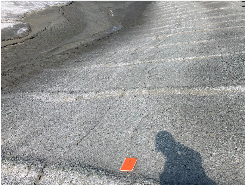
Photograph B1-13 Tailings Storage Facility
