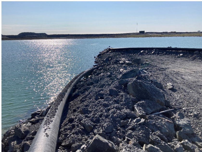
Photograph H8-3 IVR Attenuation Pond Jetty
