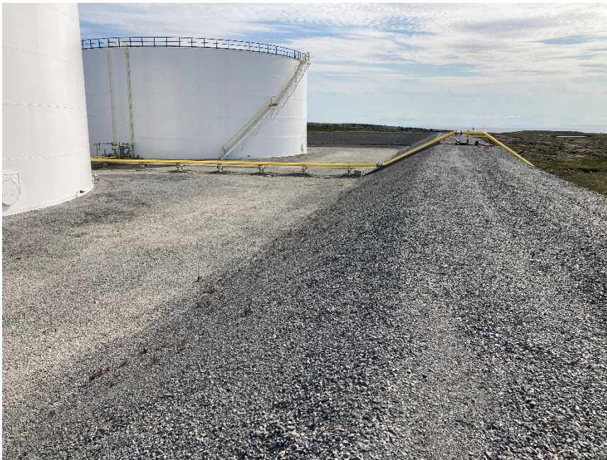
Photograph G1-26 Baker Lake Tank Farm
