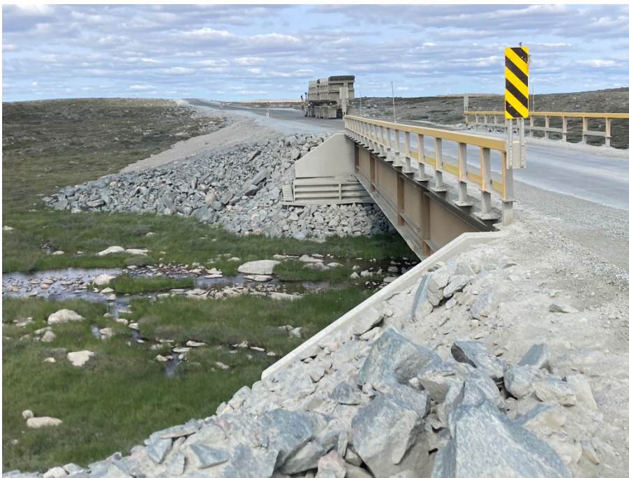
Photograph E2-18 Bridges 9 – km 160+800
