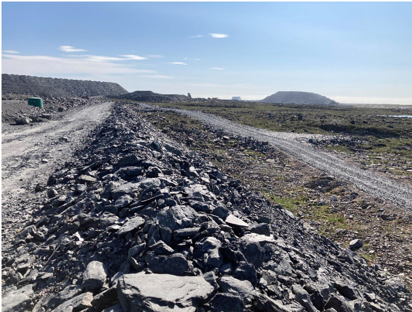
Photograph A7-10 WRSF Dike
