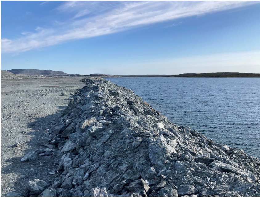
Photograph A3-9 Bay Goose Dike
