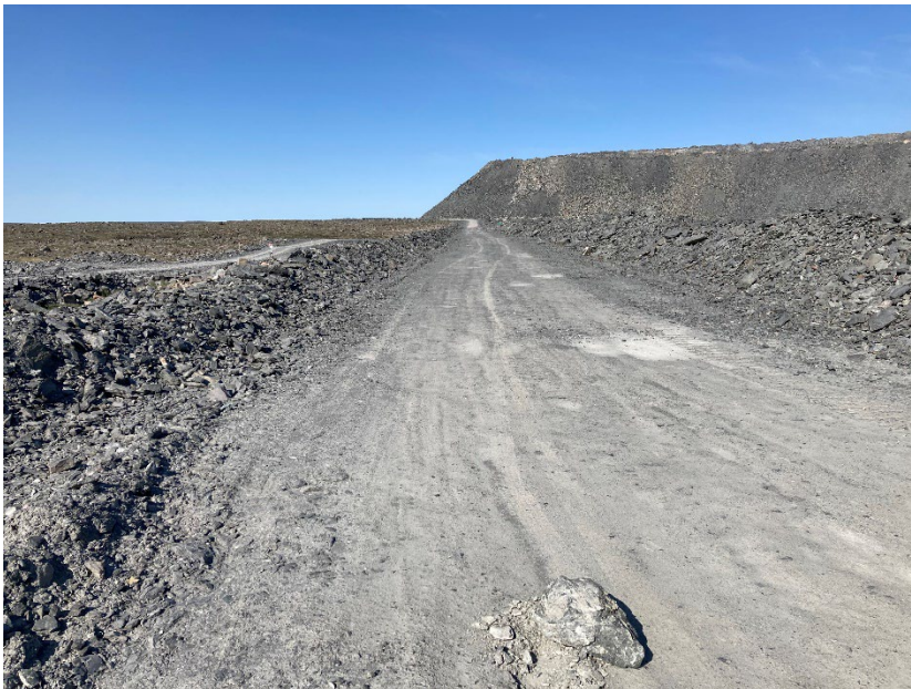
Photograph A7-2 WRSF Dike
