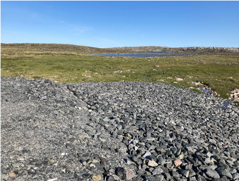
Photograph H13-5 IVR Diversion Channel
