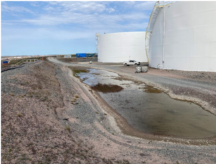
Photograph G1-4 Baker Lake Tank Farm
