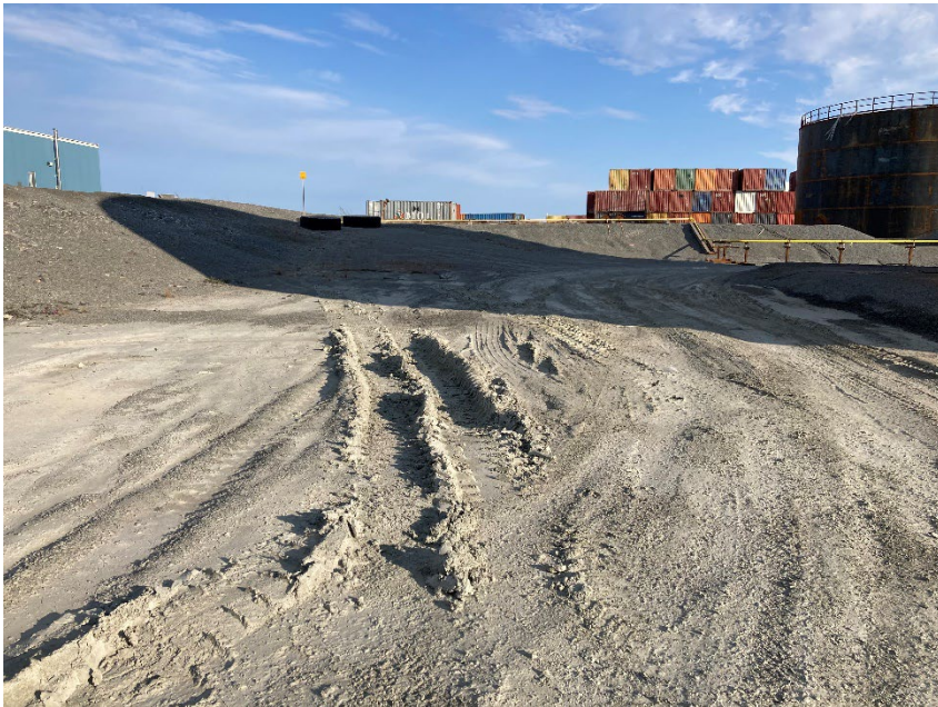
Photograph G2-4 Meadowbank Tank Farm
