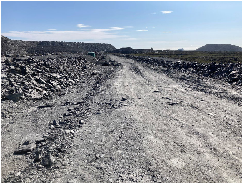
Photograph A7-9 WRSF Dike
