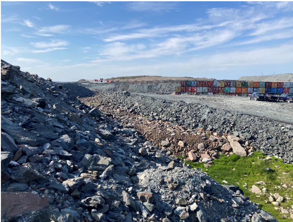
Photograph A1-10 East Dike
