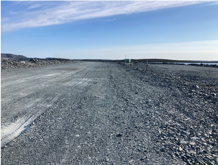
Photograph A3-17 Bay Goose Dike
