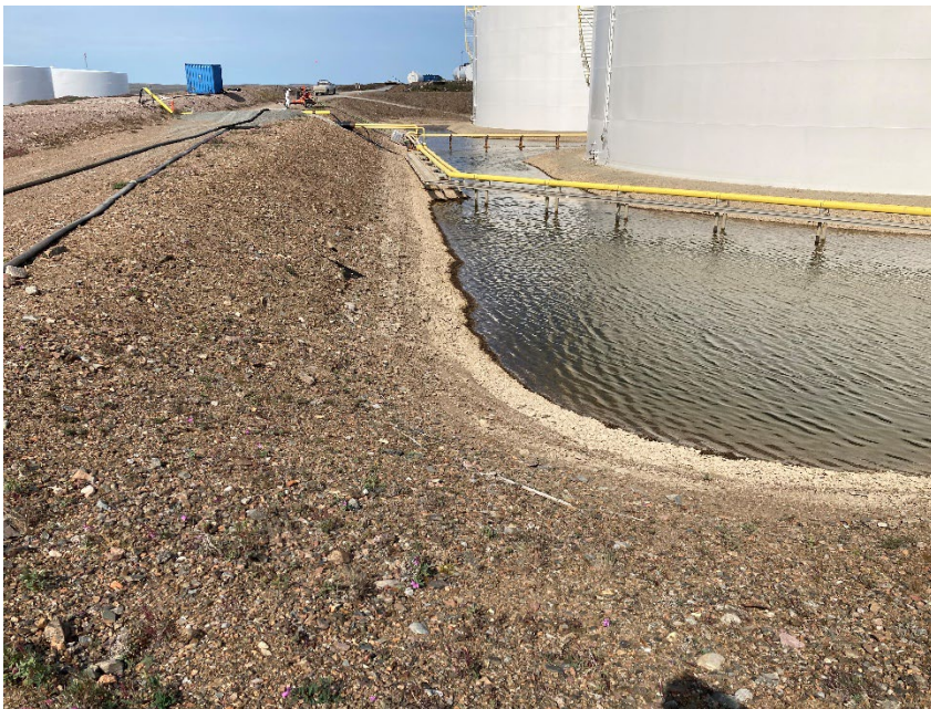
Photograph G1-16 Baker Lake Tank Farm
