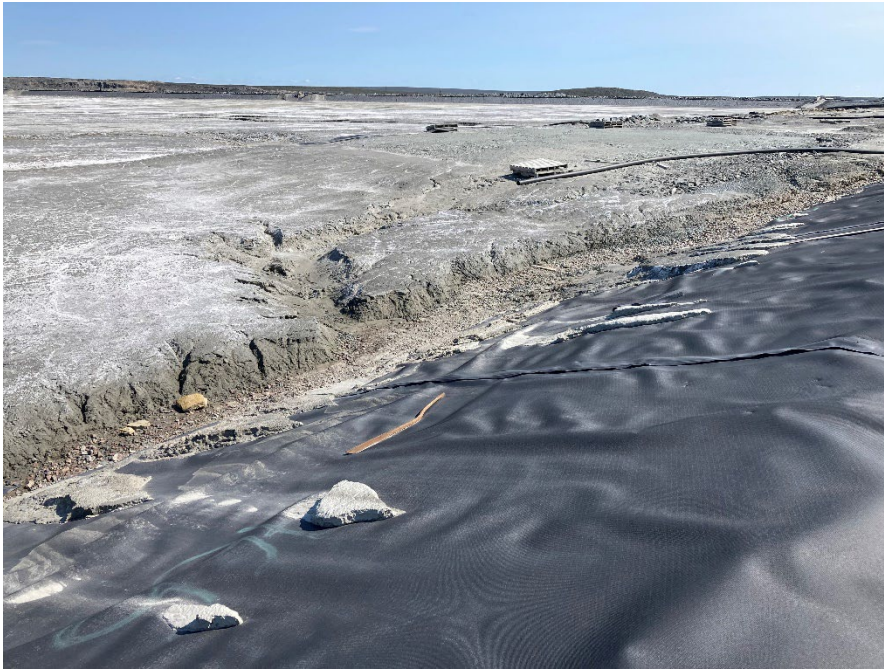
Photograph B6-9 Saddle Dam 4
