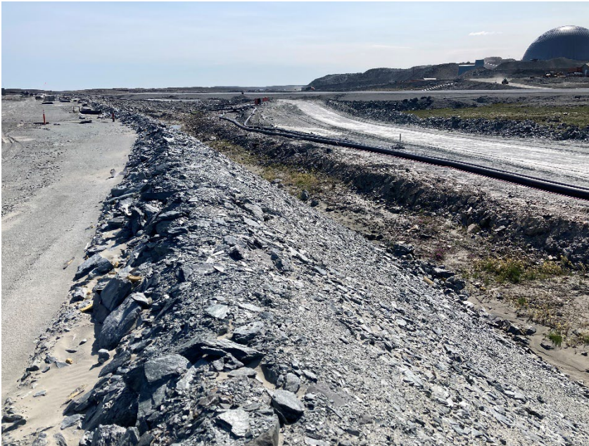
Photograph B6-1 Saddle Dam 4
