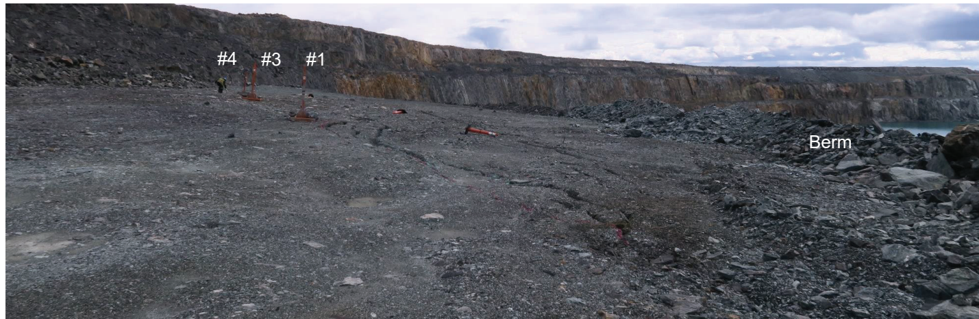
Tension Cracks on Dump, Looking Southeast
