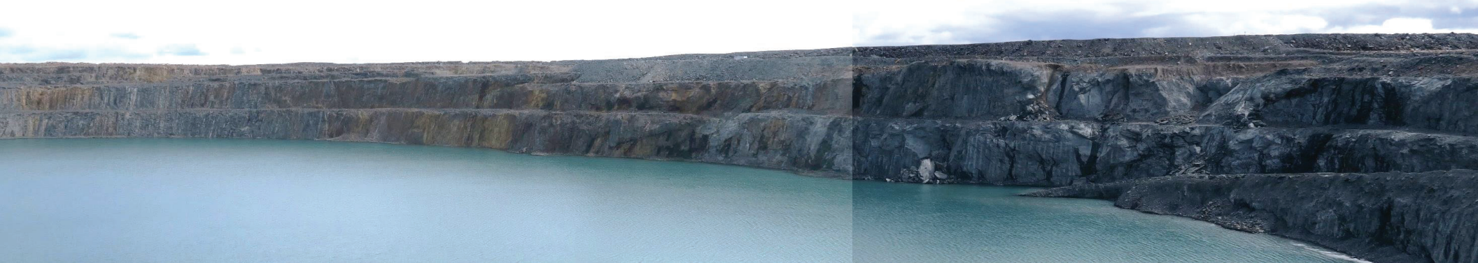
East and South Walls, Looking East
