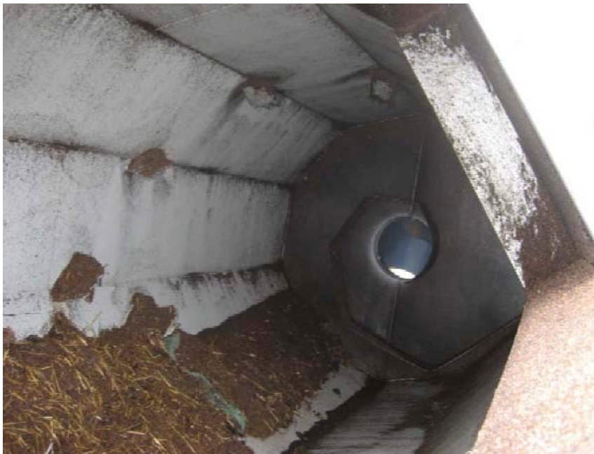
Figure 1 -- Interior view of the cylinder
