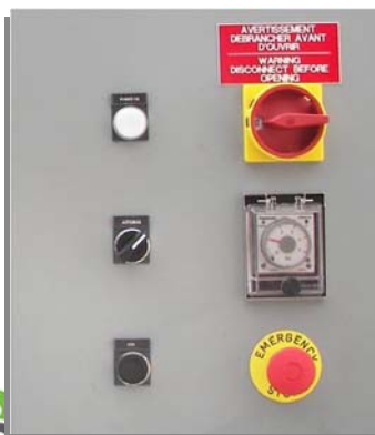
Figure 2 -- Brome Composter Control Panel
