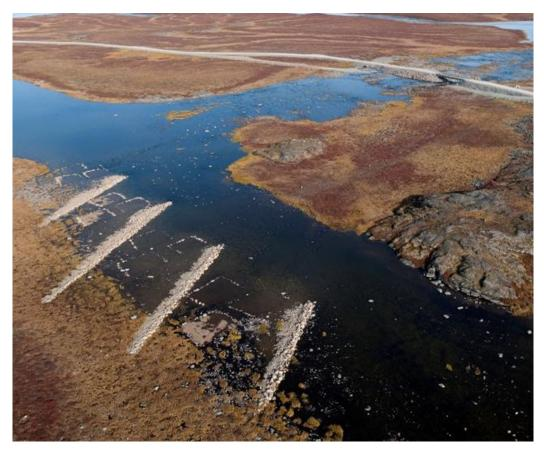
Figure 3. Arctic Grayling spawning pads constructed at Meadowbank all weather road crossing R02.
