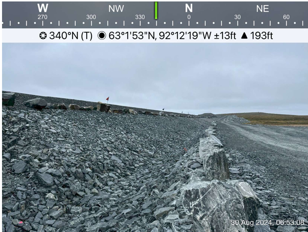
D-CP1 - Photo 9: Dike D-CP1: Dike downstream runoff/seepage collection north channel. Facing north.
