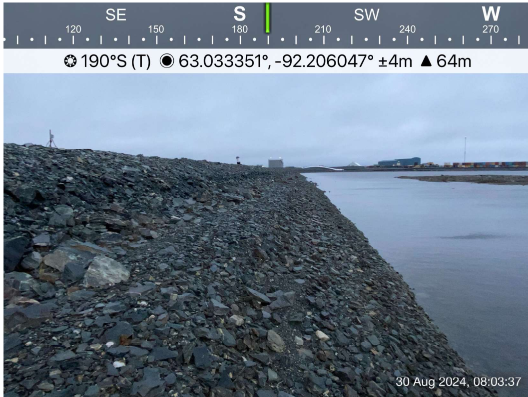
D-CP1 - Photo 1: Dike D-CP1: Upstream face– some wave erosion evident from 2019/2020 high water level event, no change from previous years. Facing south.
