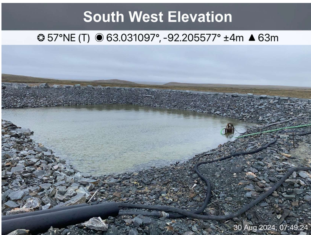
D-CP1 - Photo 12: Dike D-CP1: Dike downstream sump - rockfill berm. Facing northeast.
