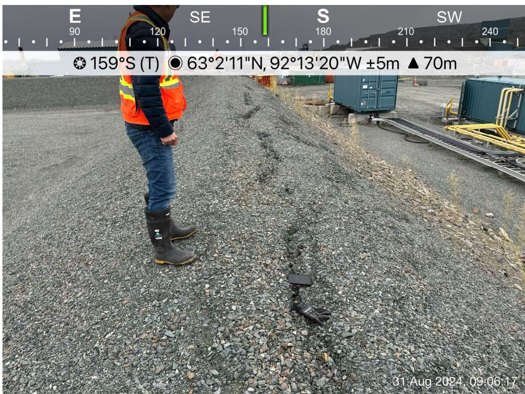
Industrial Fuel Tanks - Photo 22: Industrial Fuel Tanks - West side berm overview, cracking on crest. Facing south.
