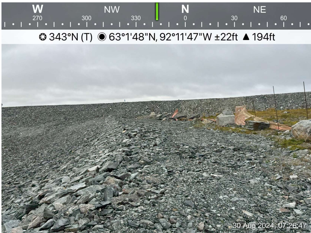
CP6 - Photo 6: CP6 - View of east side perimeter, thaw settlement and cracking observed. Facing north.
