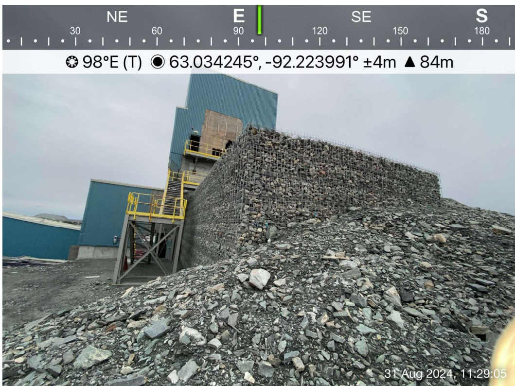
Crusher Pad - Photo 4: Crusher Pad - MSE retaining wall on the northwest corner. Facing east.
