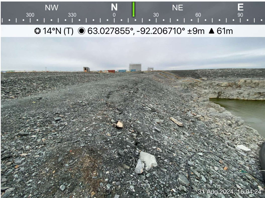
SP1 - Photo 6: SP1 Saline Pond - Deformation and cracking on top of overburden protected slope, southwestern side of SP1. Facing north.
