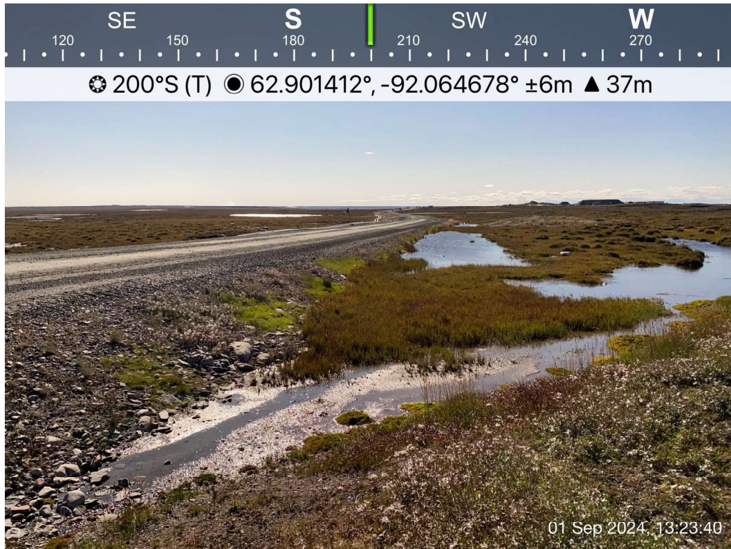
AWAR Road/ Culvert - Photo 31: KM 12.6 - No culvert installed, poor drainage condition, no sign of water flow.
