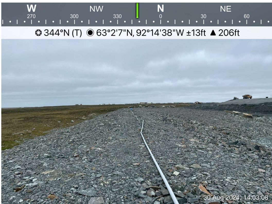
CP3 Thermal Berm Photo 4: CP3 Thermal Berm - Crest of CP3 Thermal Berm, minor thaw settlement observed, similar conditions to the previous year. Facing north.
