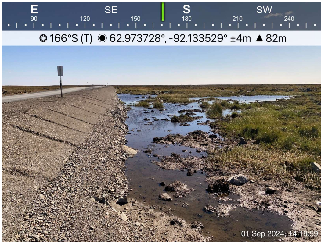
AWAR Road/ Culvert - Photo 48: KM 22.7 to 23.0 - No culvert installed, ponded water upstream.
