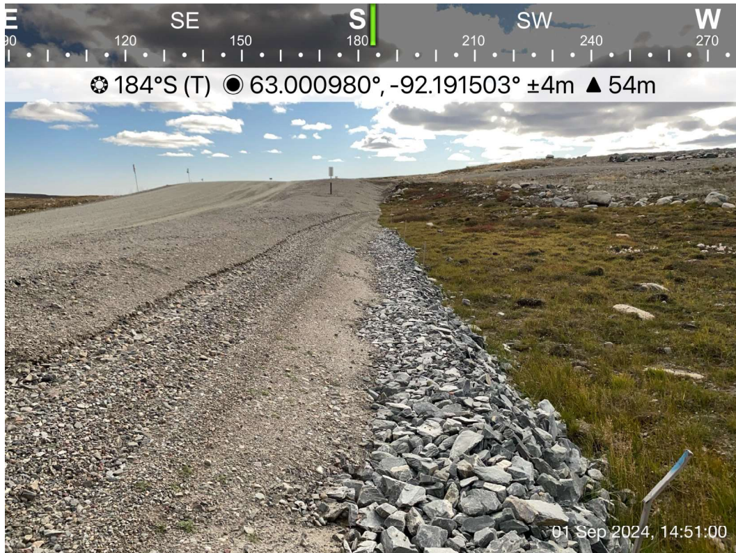
AWAR Road/ Culvert - Photo 59: KM 26.8 Culvert - Inlet has been blocked by new AWAR pipeline, high water marks from ponding water seen on pipeline bedding slope.
