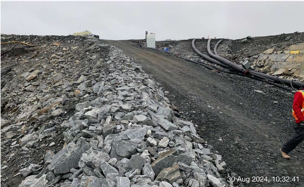
SP1 - Photo 4: SP1 Saline Pond - Access ramp, pipelines and safety berms. Facing east.
