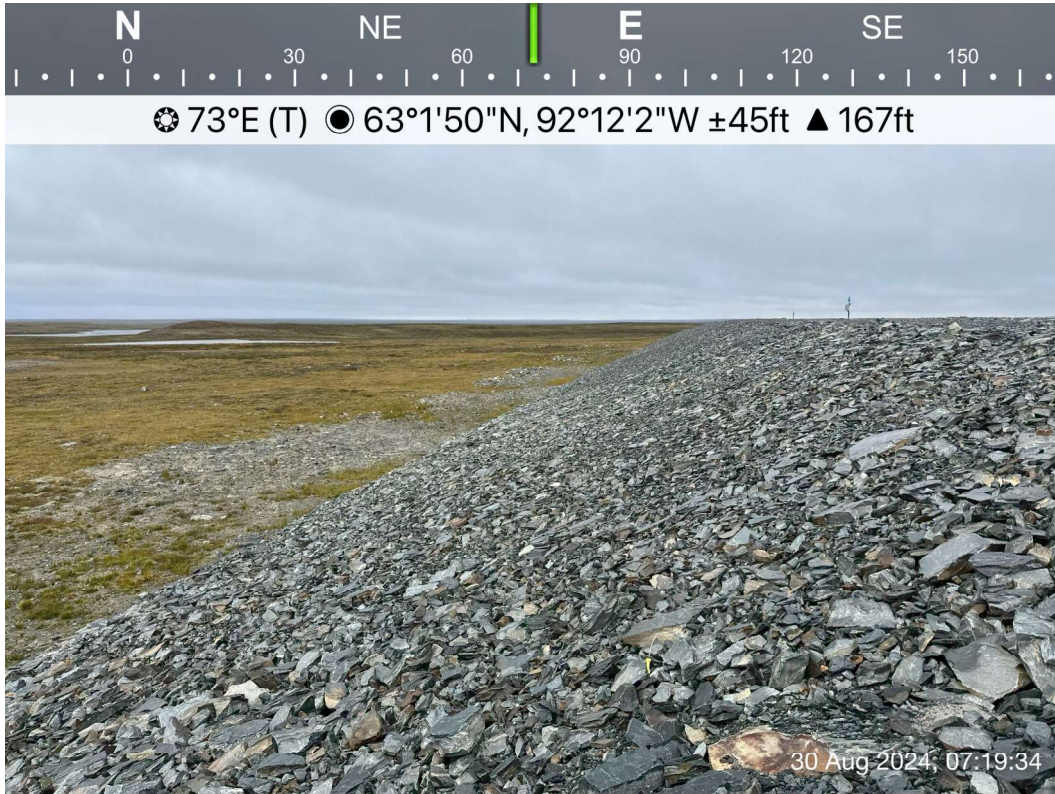
CP6 Thermal Berm - Photo 7: CP6 Thermal Berm - View of downstream and crest of berm, performing well, no stability concerns. Facing east.
