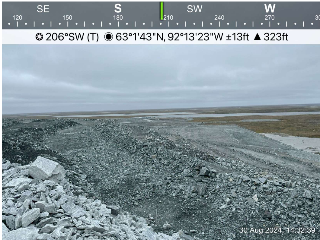
WRSF1 - Photo 3: WRSF1 - West side benches and slopes, CP4 and CP4 Thermal Berm in the background. Facing southwest.
