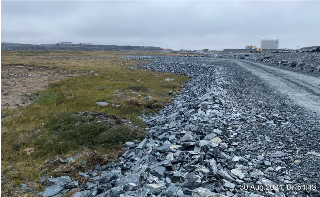
D-CP1 - Photo 13: Dike D-CP1: Downstream ROM cover. Facing southeast.
