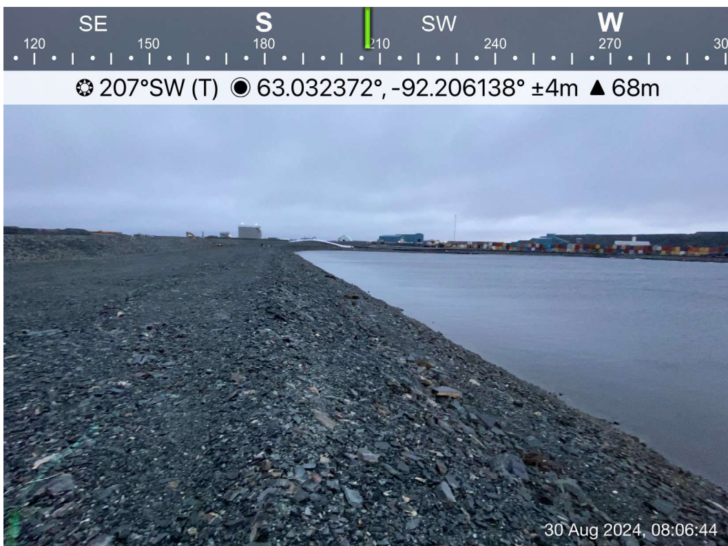
D-CP1 - Photo 6: Dike D-CP1: Dike upstream crest - minor cracking, no change from previous years. Facing southwest.
