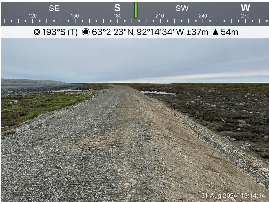
Berm 2 - Photo 10: Berm 2 - Berm 2 middle portion, slope and crest, performing well, no stability concern, ponded water on both sides. Facing south.
