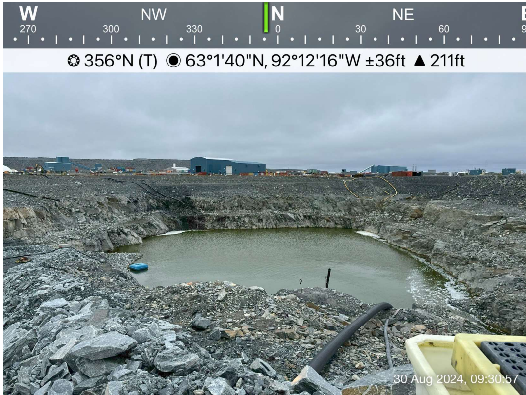
SP1 - Photo 1: SP1 Saline Pond - Overview of SP1, pond in bedrock, ROM covered overburden slopes. Facing North.
