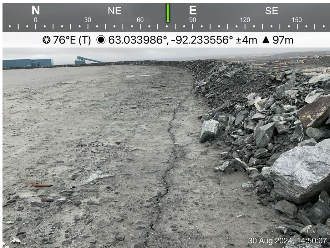
TSF - Photo 6: TSF - Crest of rockfill covered slope, minor cracking and settlement. Facing east.
