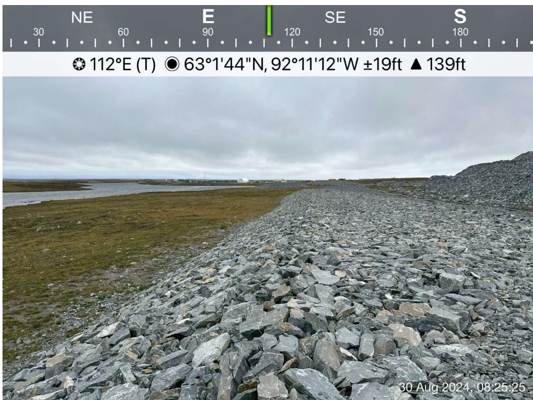
Channel 9 Berm - Photo 10: Channel 9 Berm: View of crest and downstream slope, performing well, no stability concern. Facing east.
