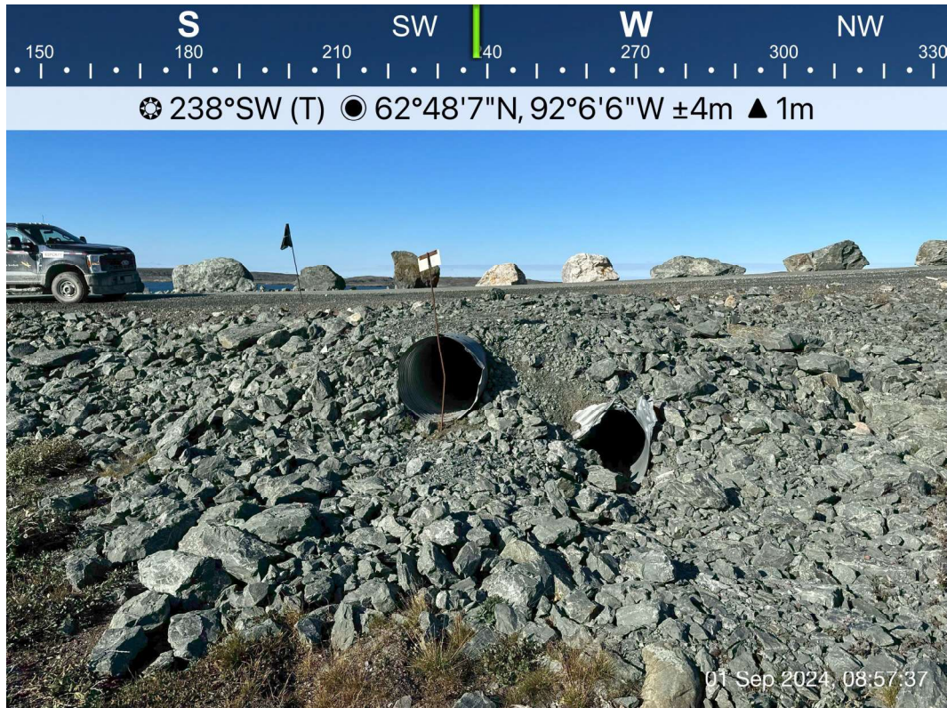
Itivia Bypass Road/ Culvert - Photo 1: Culvert C01 - KM 0.35 - Inlet.
