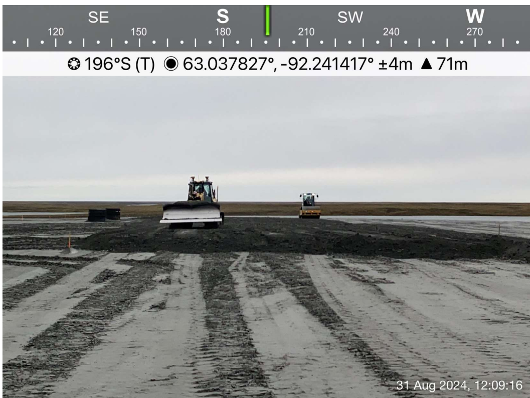
TSF - Photo 4: TSF - Placement and compaction of tailings in Cell 2. Facing south.
