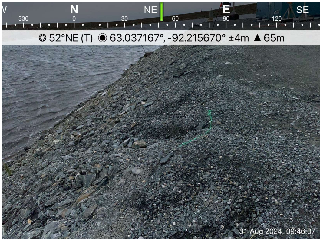
D-CP1 - Photo 18: Dike D-CP1: Jetty 1— side slope, minor erosion with similar conditions to the previous year. Facing northeast.
