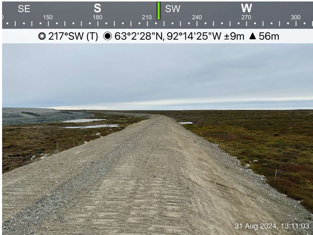
Berm 2 - Photo 9: Berm 2 - Berm 2 north portion, slope and crest, performing well, no stability concern. Facing southwest.
