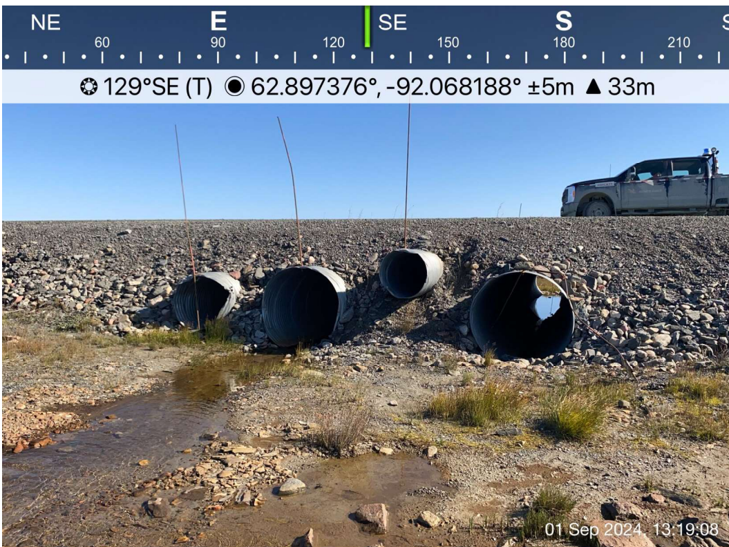
AWAR Road/ Culvert - Photo 30: Culvert KM 12.1 - Outlet.
