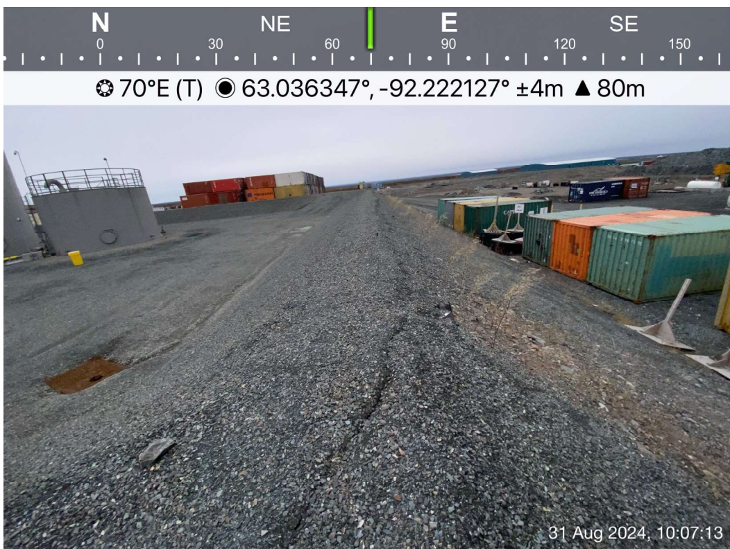
Industrial Fuel Tanks - Photo 24: Industrial Fuel Tanks - South side berm overview, cracking on crest. Facing east.
