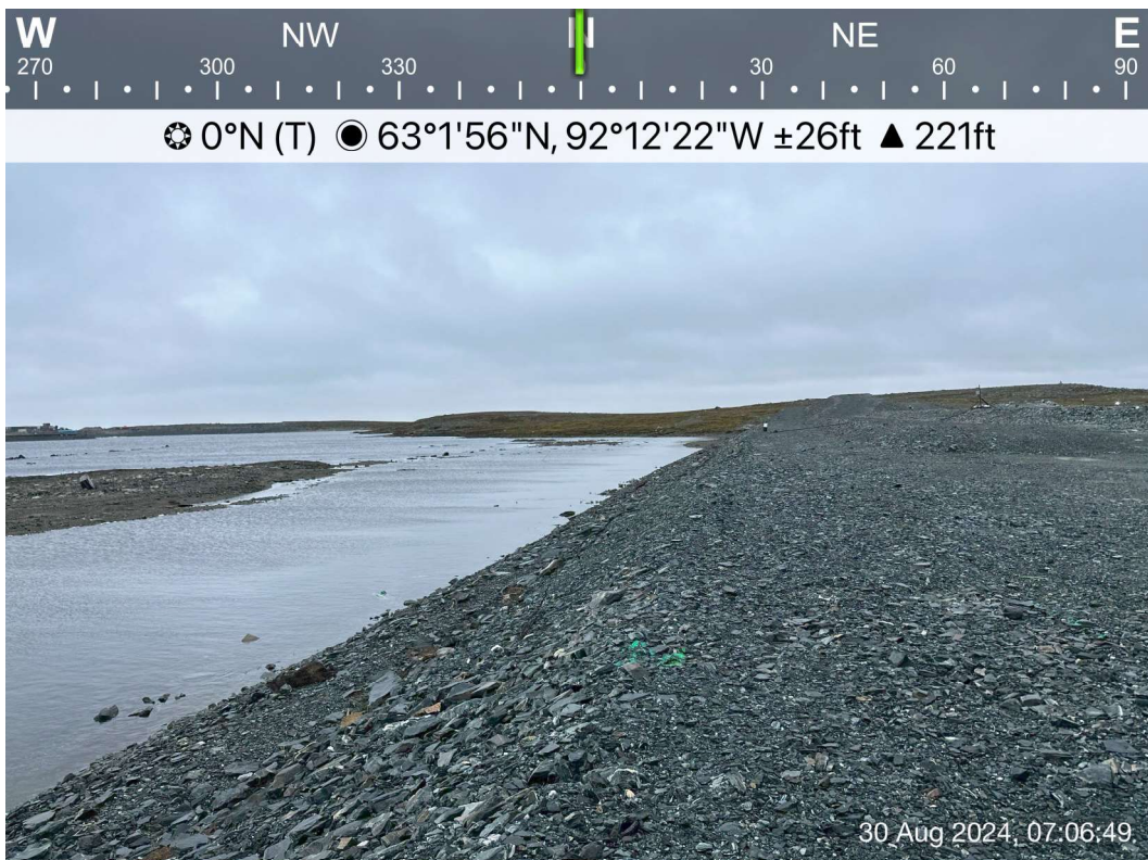
D-CP1 - Photo 2: Dike D-CP1: Upstream face– some wave erosion evident from 2019/2020 high water level event, no change from previous years. Facing north.
