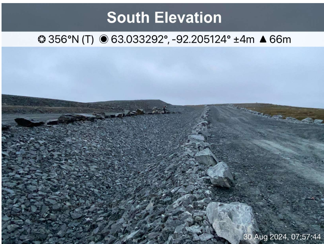
D-CP1 - Photo 8: Dike D-CP1: Dike downstream runoff/seepage collection north channel. Facing north.
