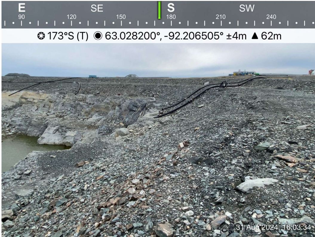
SP1 - Photo 5: SP1 Saline Pond - Deformation and cracking on top of overburden protected slope, southwestern side of SP1. Facing south.
