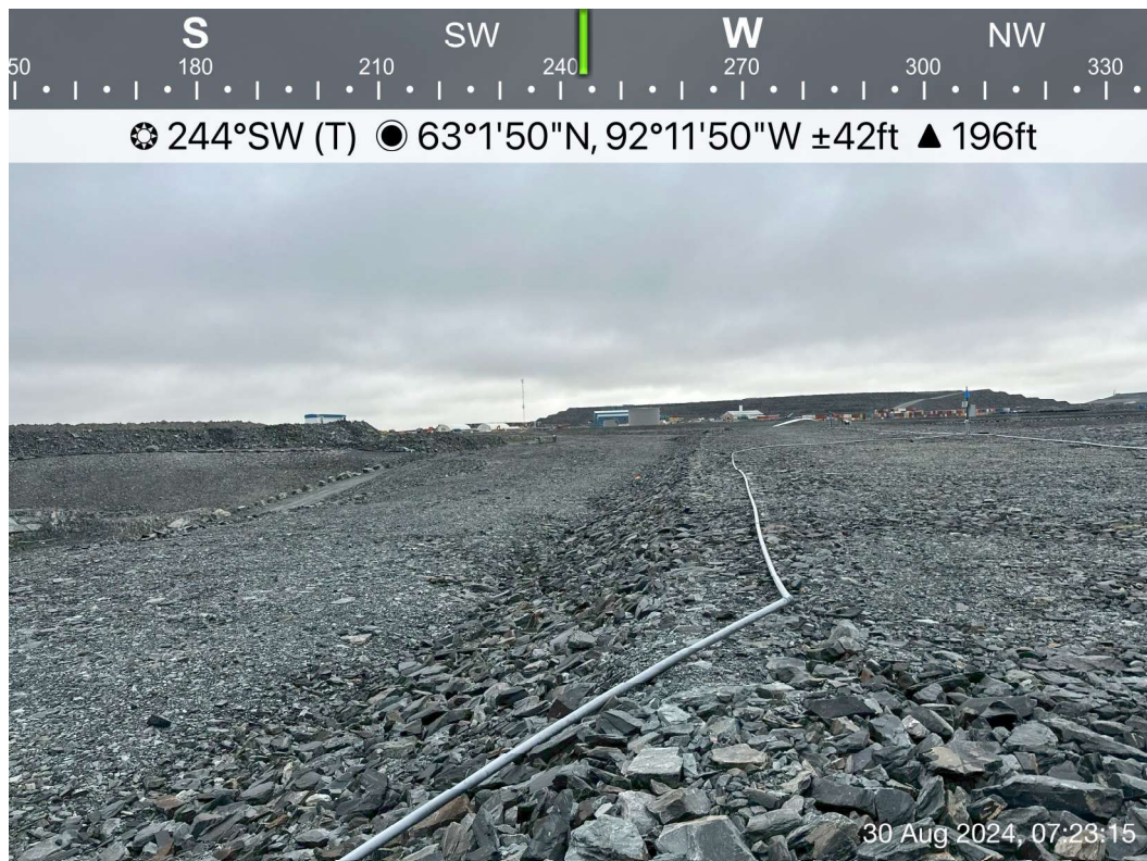
CP6 Thermal Berm - Photo 8: CP6 Thermal Berm - Crest view, thaw settlement observed at various areas. Facing southwest.
