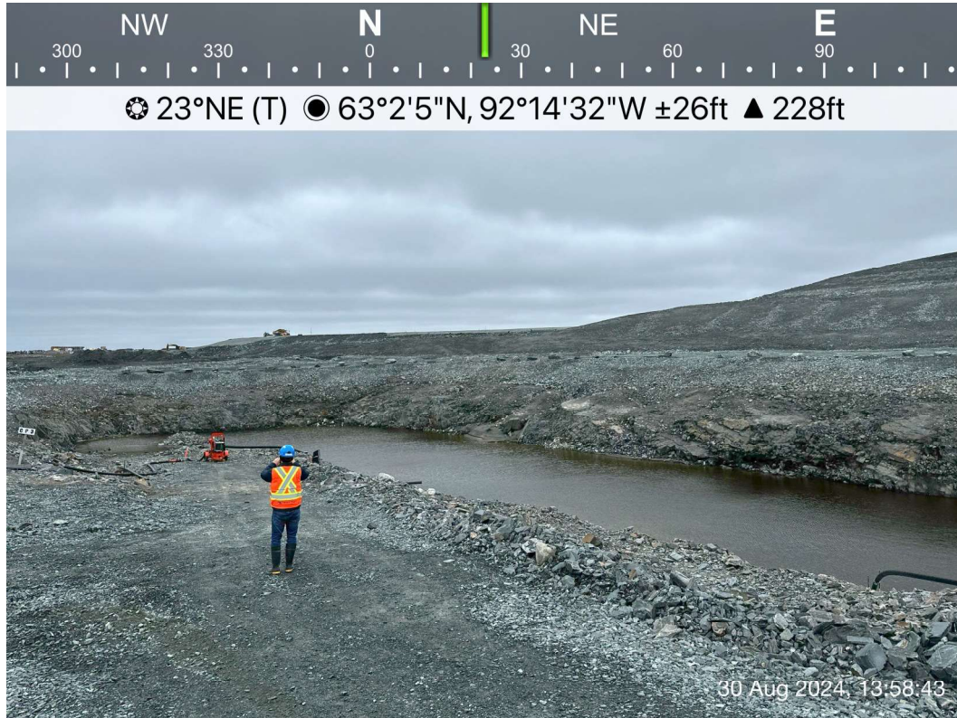
CP3 - Photo 1: CP3 - Small amount of water stored in CP3, bedrock slopes with fractured rock, no stability concern.
