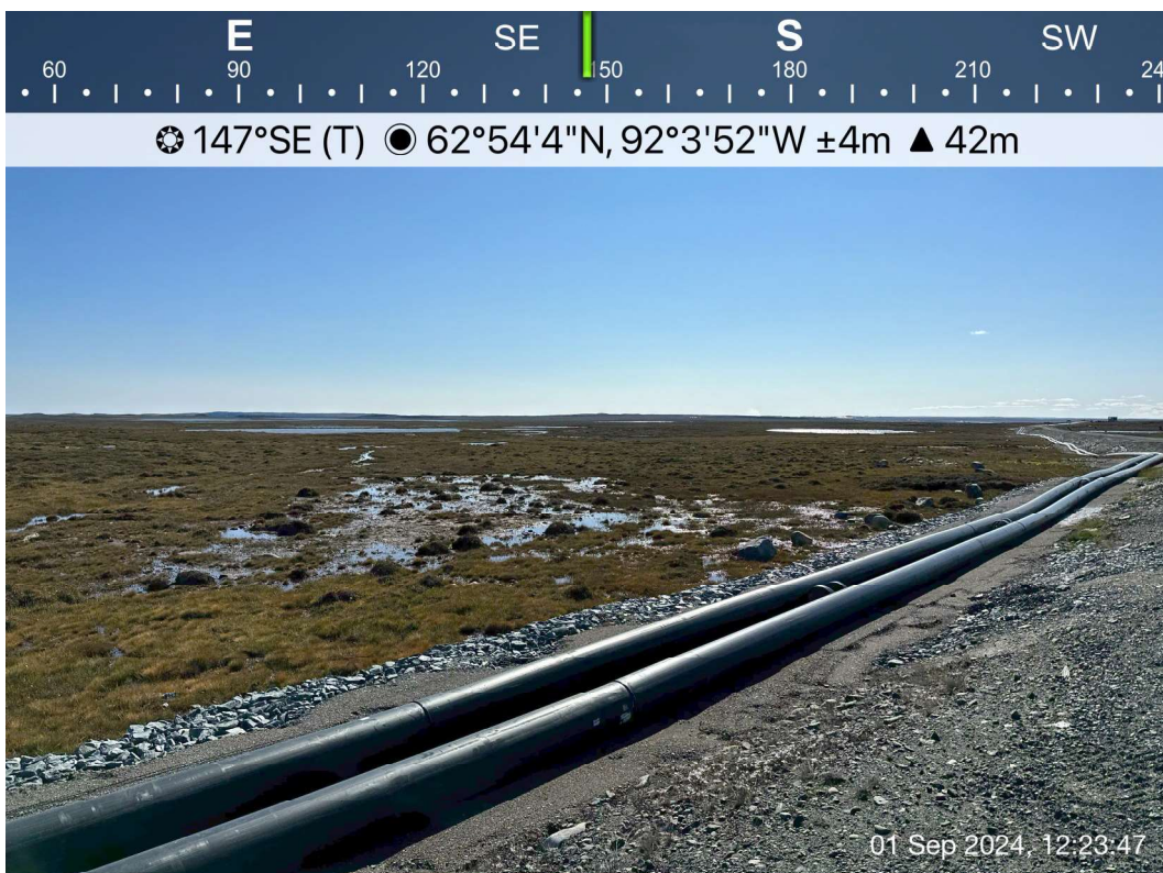
AWAR Road/ Culvert - Photo 32: KM 12.6 - No culvert installed, poor drainage condition, no sign of water flow.
