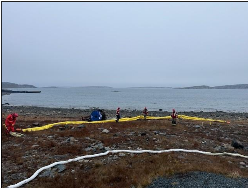
Photo 4: Marine booms installed along shore (in a real scenario these would be deployed in water)
