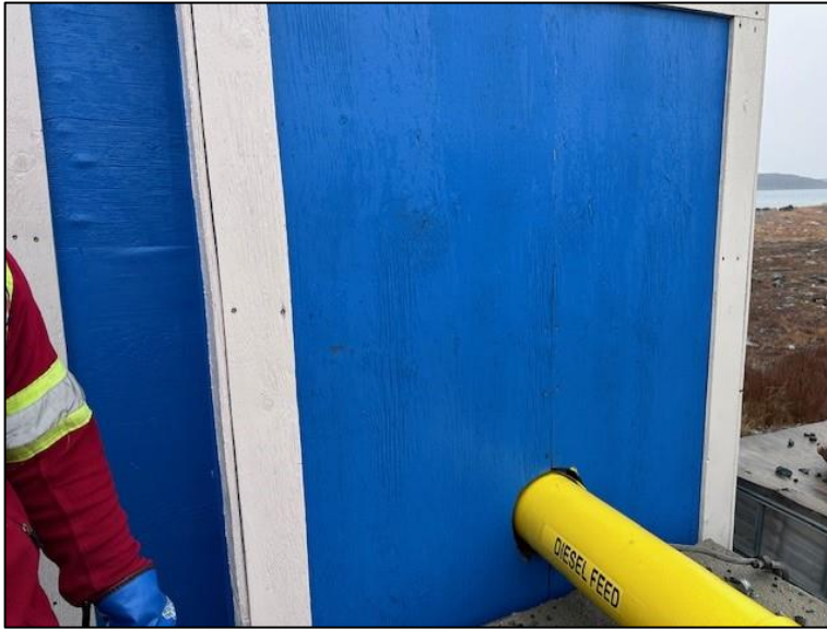
Photo 1: Hatch to be installed at the fuel transfer manifold to allow for better/alternative access.
